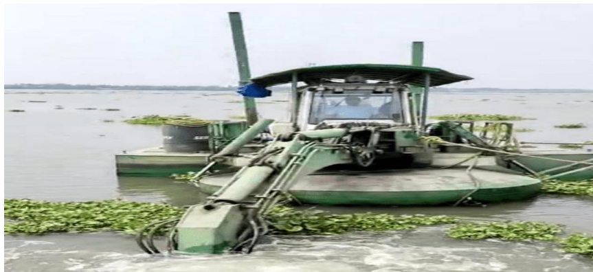
Dredging at Thevara
