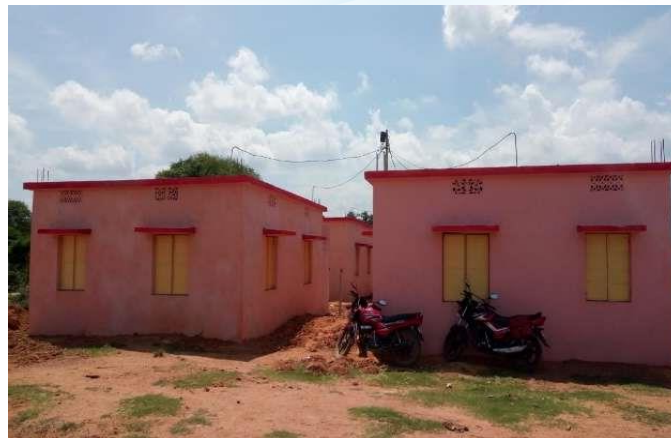
Construction of Houses in Relocation Site at Sahibganj
