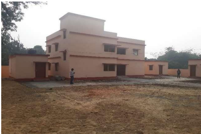
Construction of Primary School in Resettlement Site at Sahibganj
