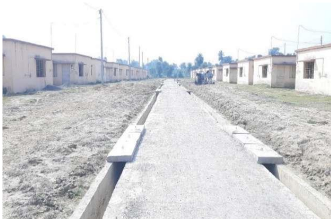
Construction of Road in Resettlement colony, Sahibganj
