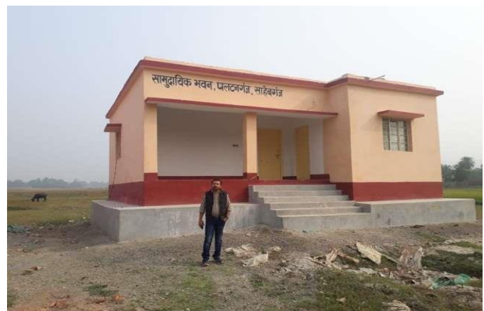
Community Hall in Paltanganj Relocation Site at Sahibganj
