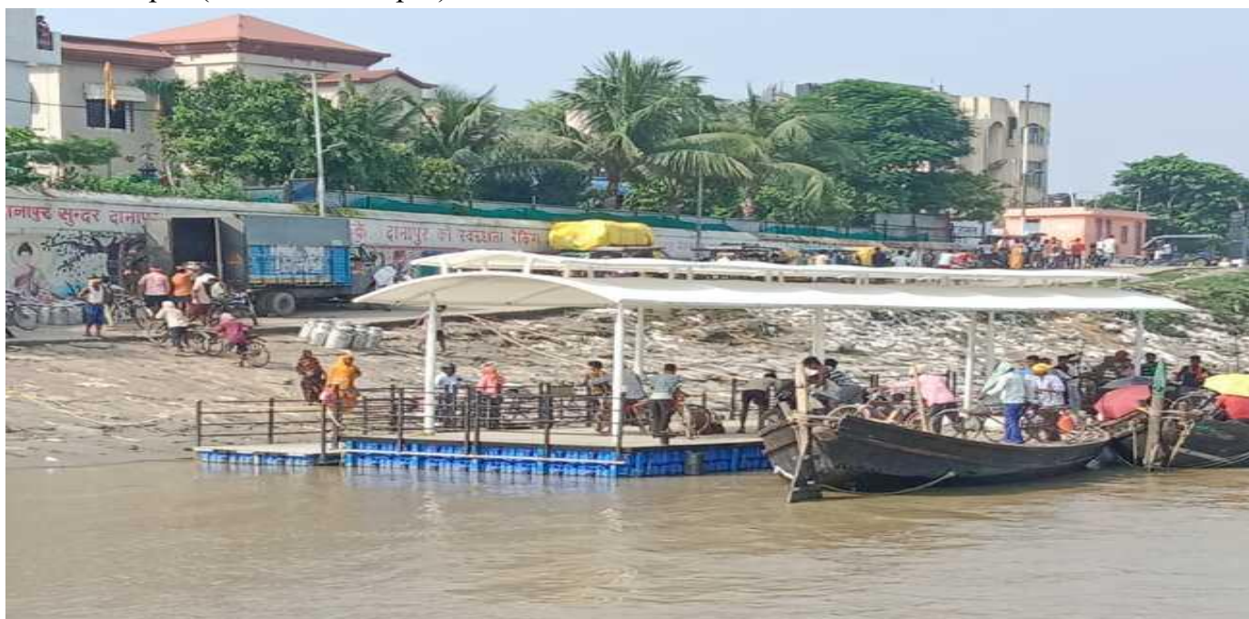
Community jetty installed in UP for public usage
