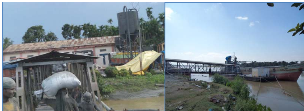
View of existing Badarpur terminal with manual cargo handling at Badarpur Terminal
