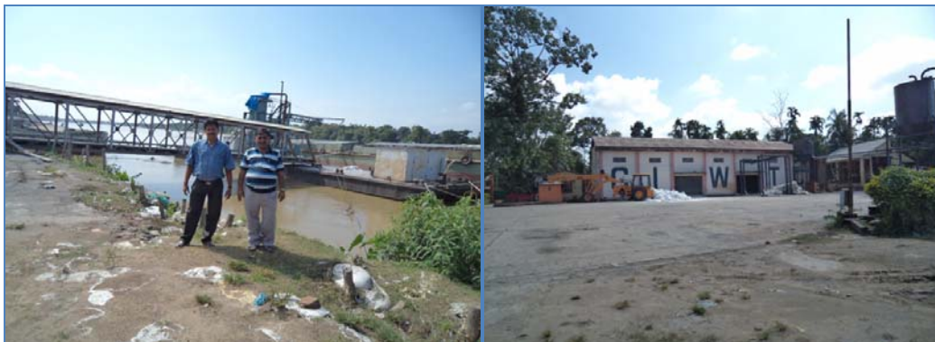
View of Gangway and Pontoon Jetty arrangement Godown facility at Badarpur Terminal
