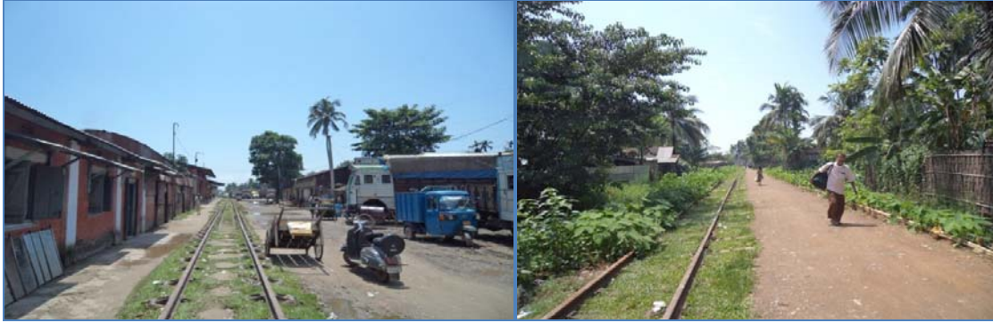
Old Railway line (MG) from Mall Godam to Karimganj Jn.
