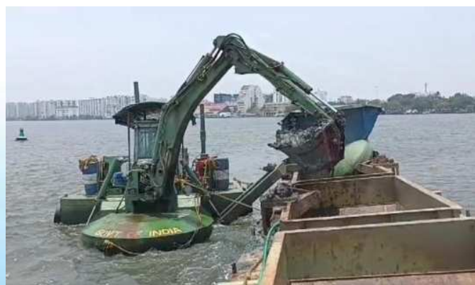
Maintenance dredging by dredgers AD Manimala & CSD Champakkara in NW – 3
