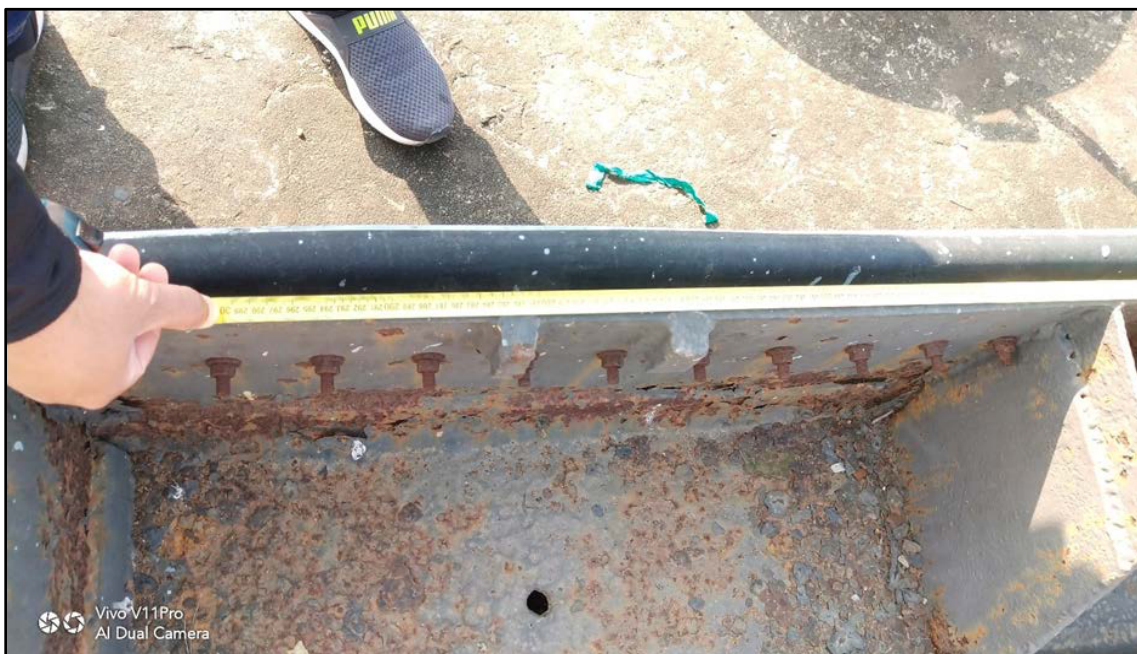
Figure 4.12 Dimensioning of Bulkhead Gates of Farakka Lock
