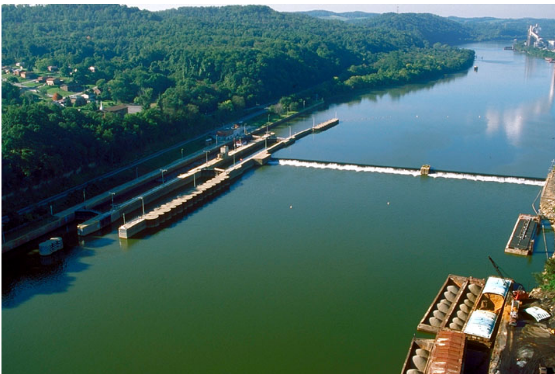
Figure 12.11 The Locks & Dam 3, Mon River
