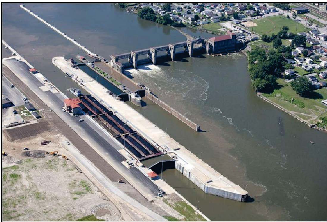
Figure 12.18 The Marmet Locks and Dam
