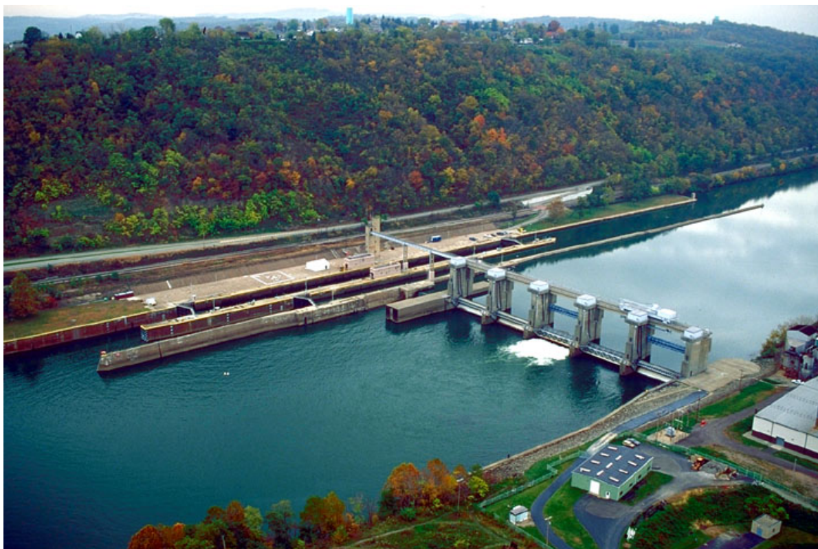
Figure 12.12 The Locks & Dam 4, Monongahela River Emsworth Locks & Dams
