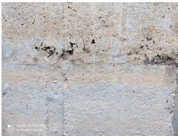
Figure 4.57 Lock Chamber side walls damaged
