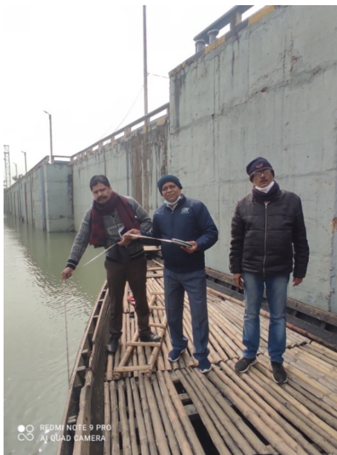
Figure 4.68 Depth measurement in lock chamber for silt deposition over base slab
