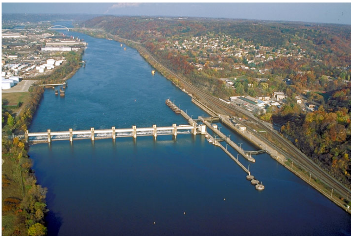
Figure 12.13 The Emsworth Locks & Dams
