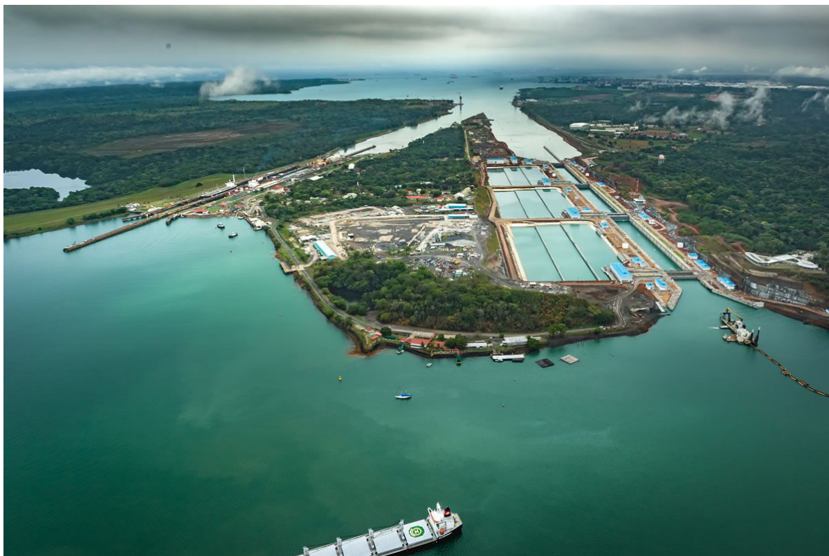
Figure 12.6 The Panama Canal Lock
