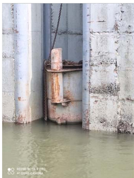
Figure 4.57 Lock Chamber side walls damaged
