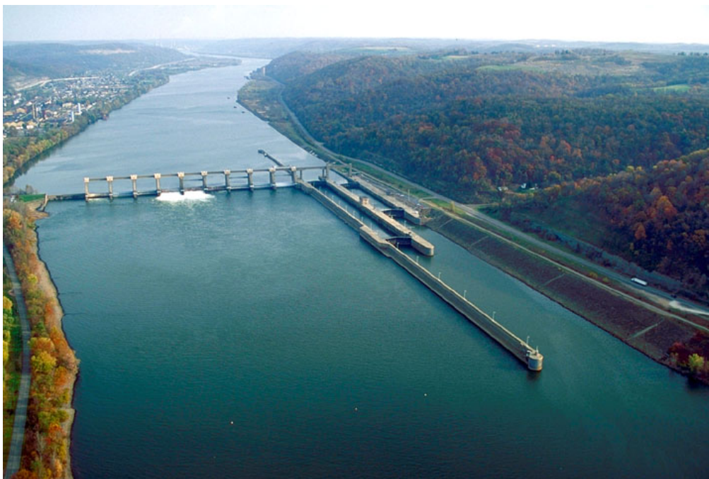
Figure 12.16 The Pike Island Locks & Dam
