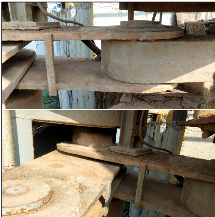
Figure 4.6 Top Bearing of Mitre Gates of Farakka Lock
