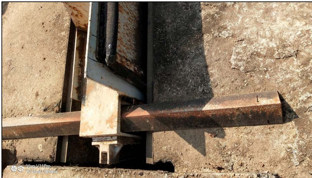
Figure 4.23 Rubber Seals of Bulkhead Gates of Farakka Lock
