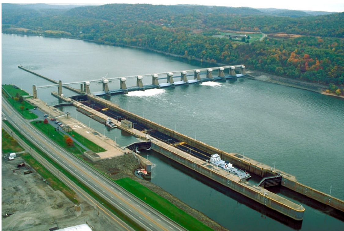
Figure 12.15 The New Cumberland Locks & Dam
