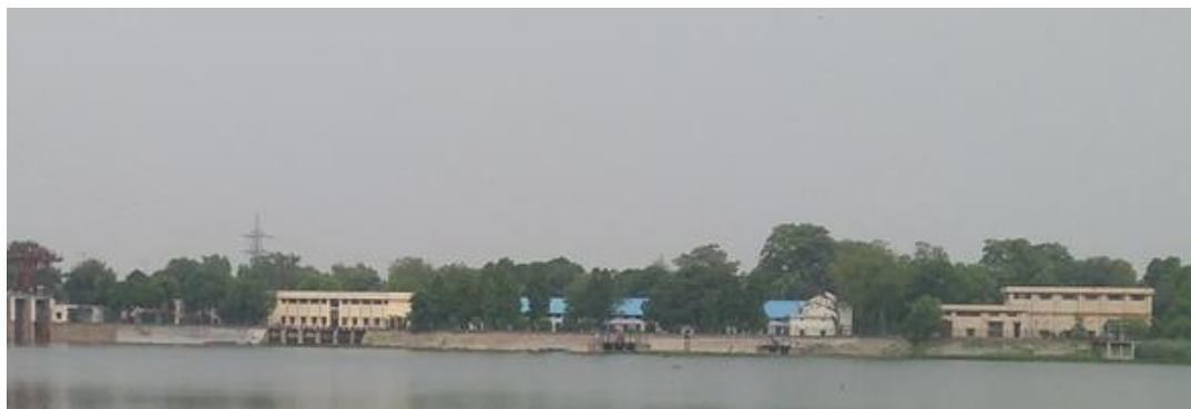
Fig. 2.26 View of Water works on the right bank of Yamuna river u/s of Wazirabad Barrage
