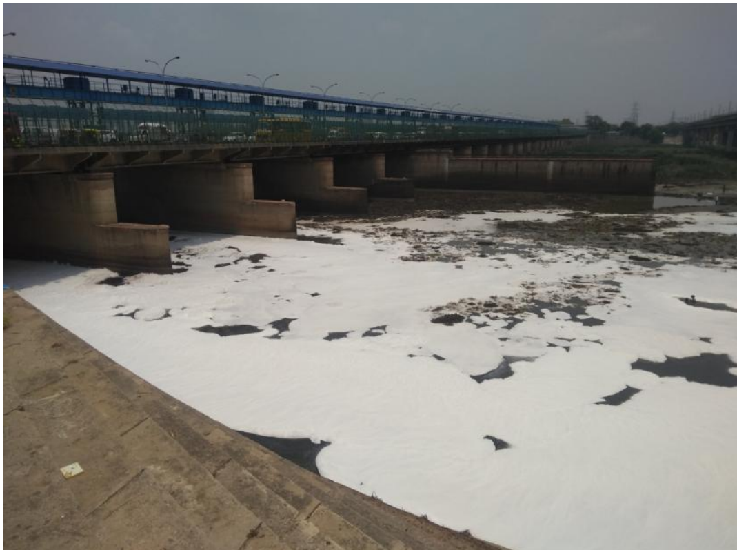
Fig. 2.34 Present view on the downstream of Okhla Barrage
