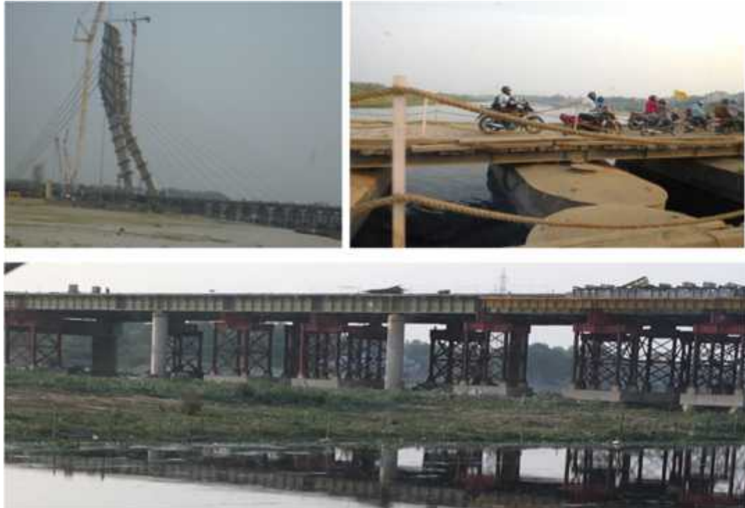
Fig. 6.45 Signature Bridge near Soniya Vihar
