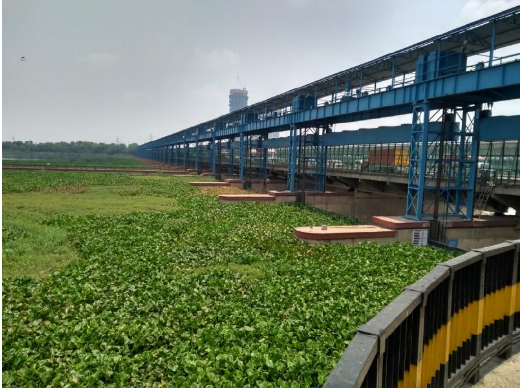
Fig. 2.33 Present view on the upstream of Okhla Barrage at CH 1052 KM
