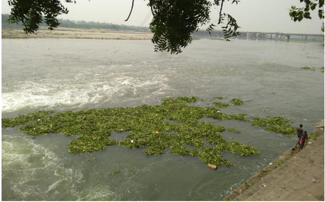
Fig. 2.22 Present view showing flow of Yamuna River on the downstream of Wazirabad Barrage
