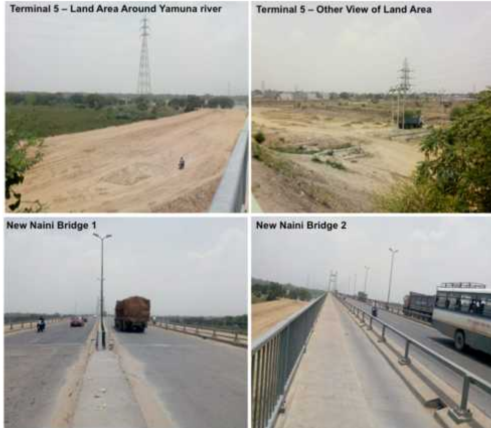
Fig. 7.5 Terminal 5 – Near Naini Bridge
