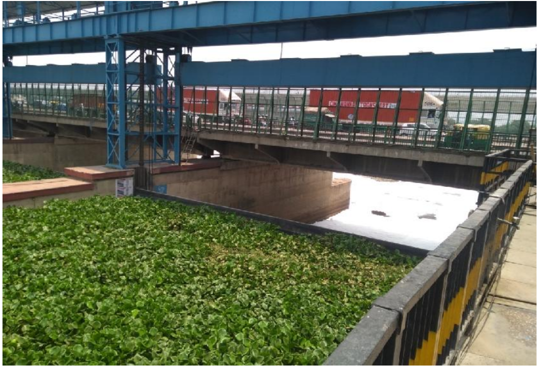
Fig. 2.37 Present condition of regulating platform and gates at Okhla barrage
