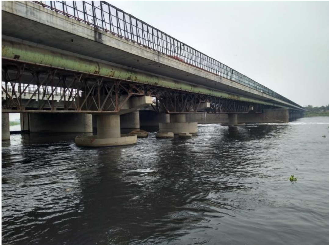
Fig. 2.28 Present view on the downstream of Yamuna Barrage at ITO
