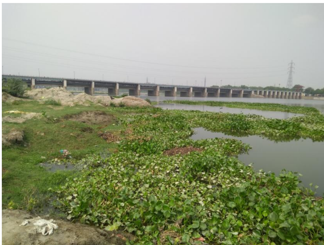
Fig. 2.19 Present view on the upstream of Wazirabad Barrage at CH 1074.1 KM
