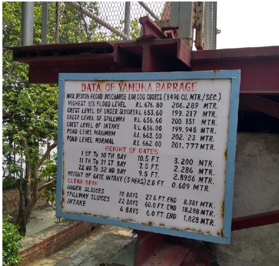
Fig. 2.31 Salient features of Yamuna Barrage at ITO, Delhi
