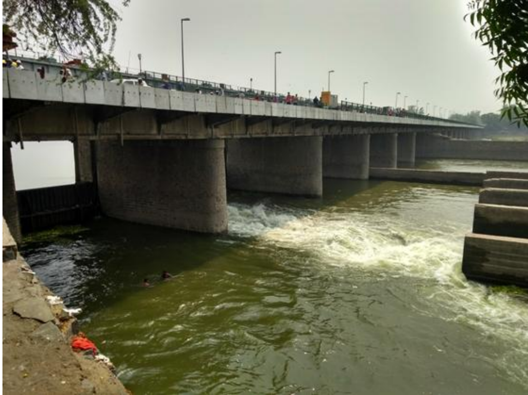
Fig. 2.20 Present view on the downstream of Wazirabad Barrage
