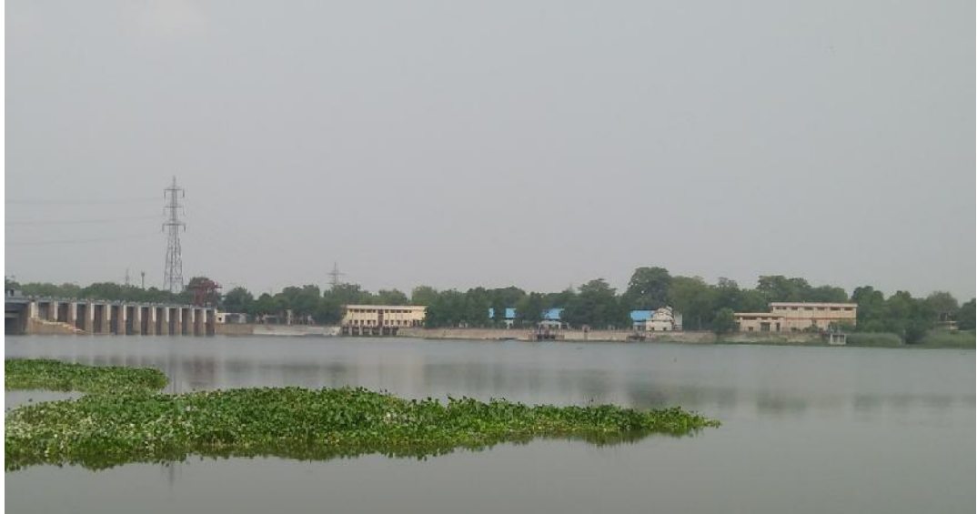
Fig. 2.24 Right Bank view on the upstream of Wazirabad Barrage
