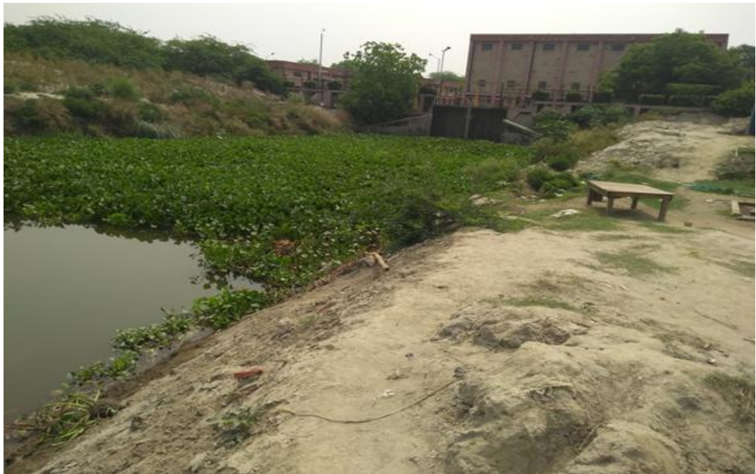
Fig. 2.25 Sangam Pump house on the left bank of Yamuna river u/s of Wazirabad Barrage
