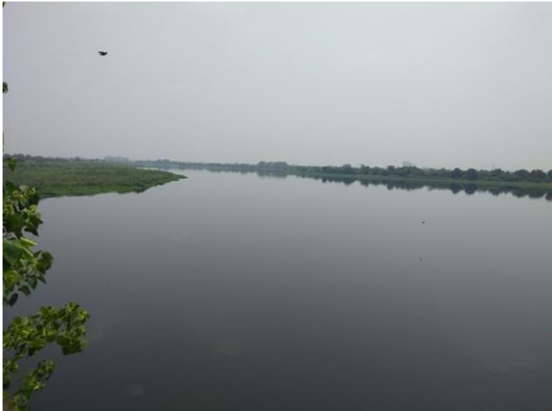
Fig. 2.29 Present view showing flow of Yamuna River on the upstream of Yamuna Barrage at ITO
