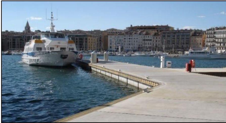
Figure 5.8: A passenger ship docked to a floating pontoon jetty
