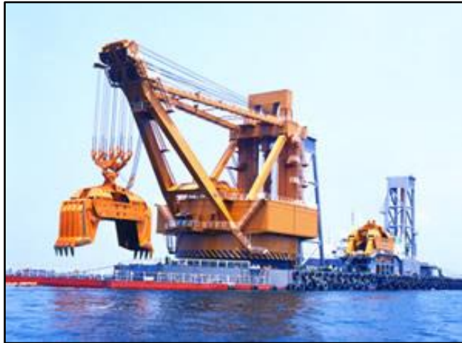
Figure 3.1: A typical grab dredger in operation
