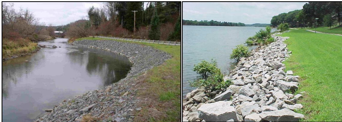
Figure 3.3: Embankment protection using stone riprap combined with vegetative cover
