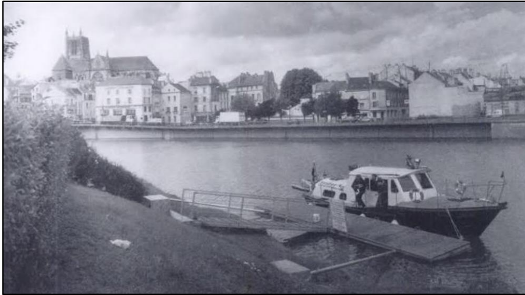
Figure 5.9: Floating pontoon quay with steel access supported on pedestals resting on open footing (Option 1)
