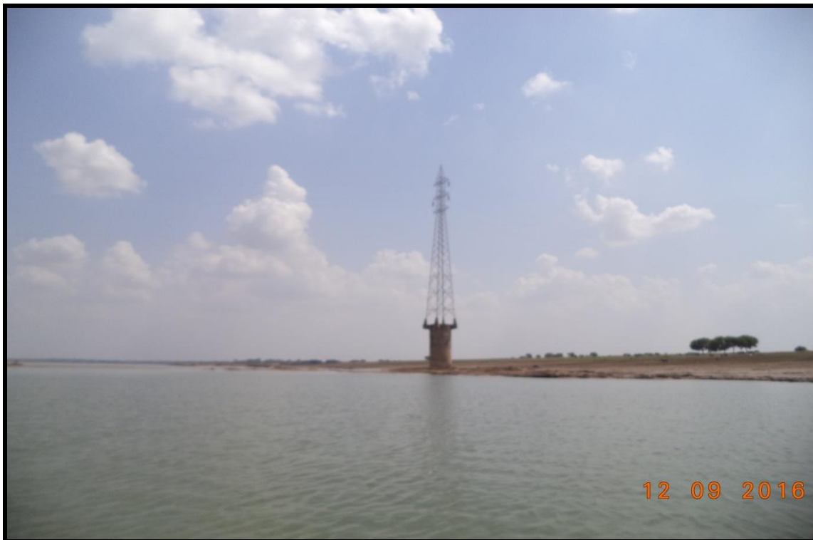
Fig No. 19 High Tension CH 7.530 km
