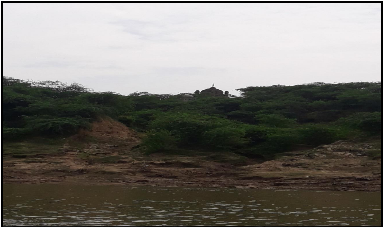
Fig No. 33 Temple Left side CH 60.220 km
