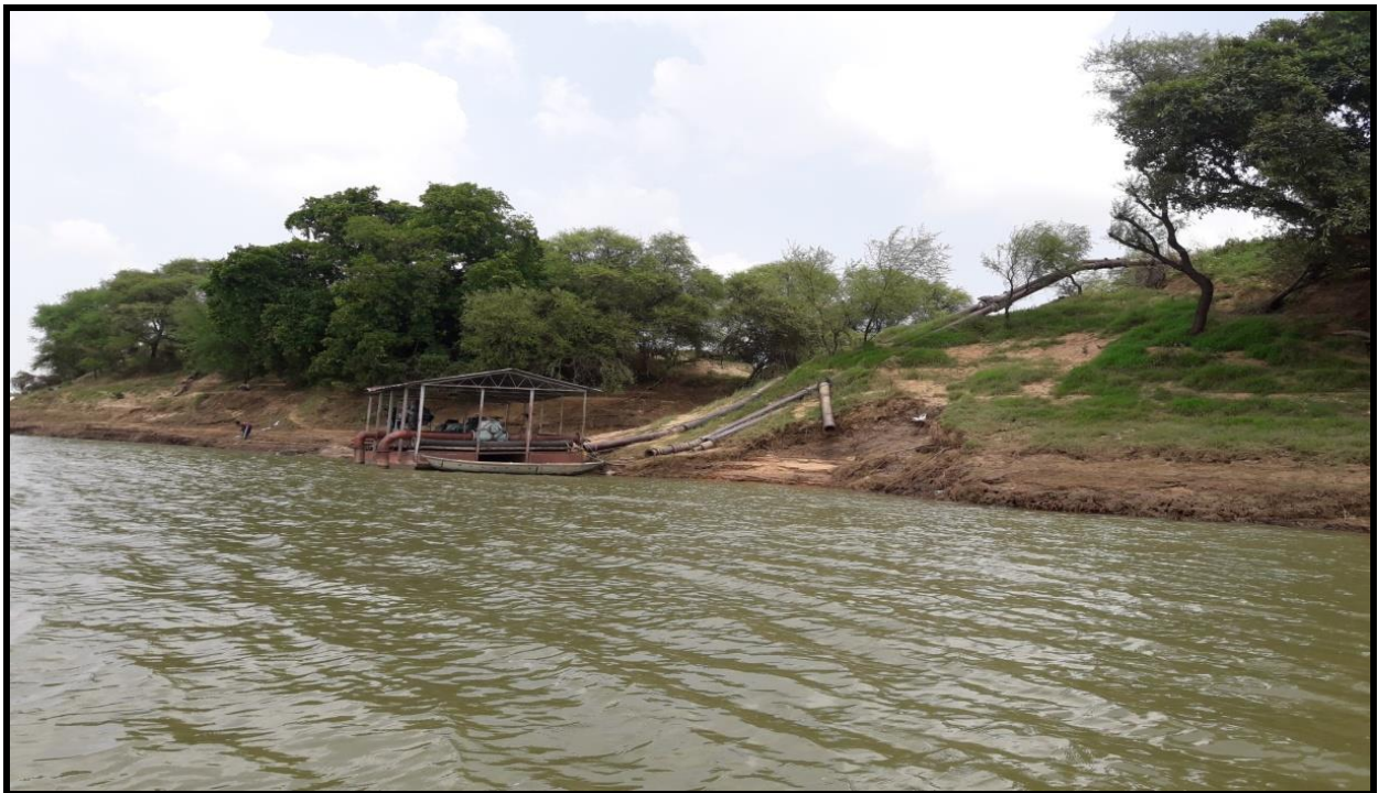
Fig No. 35 Pump House Left Side CH 65.000 km
