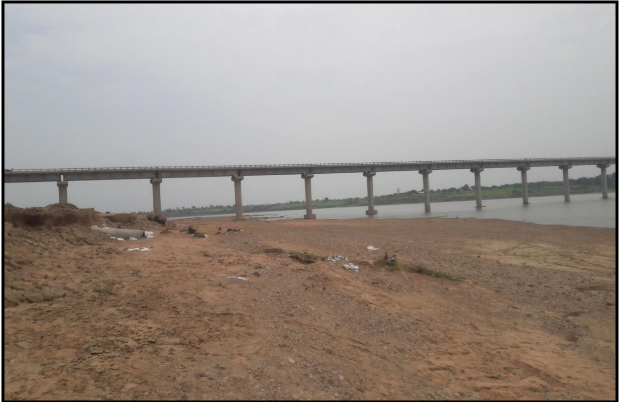
Fig No. 34 Jalalpur Bridge CH 59.282 km
