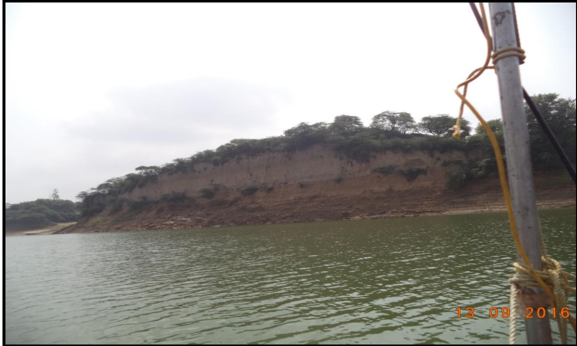
Fig No. 18 Steep cut Right side CH 2.000 to 2.700 km
