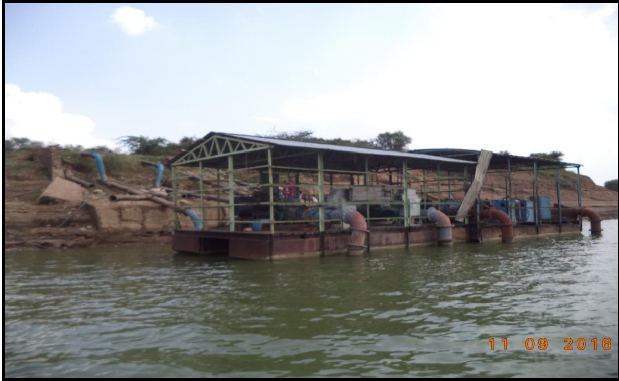
Fig No. 22 Pump House CH 25.000 km
