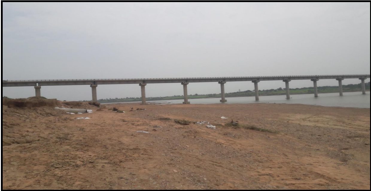
Figure No. - 08 Jalalpur Bridge CH 59.282 km
