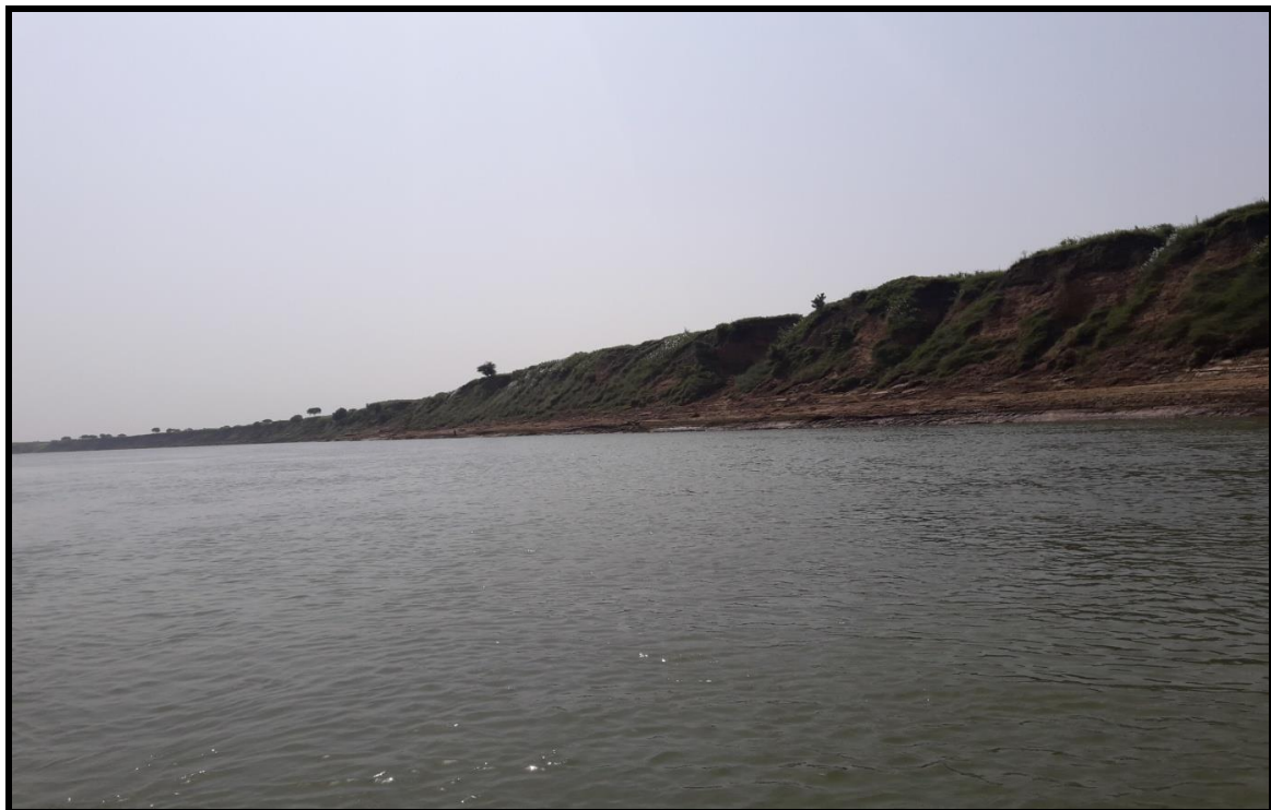
Fig No. 29 Steep cut Right side CH 46.500 to 48.000 km
