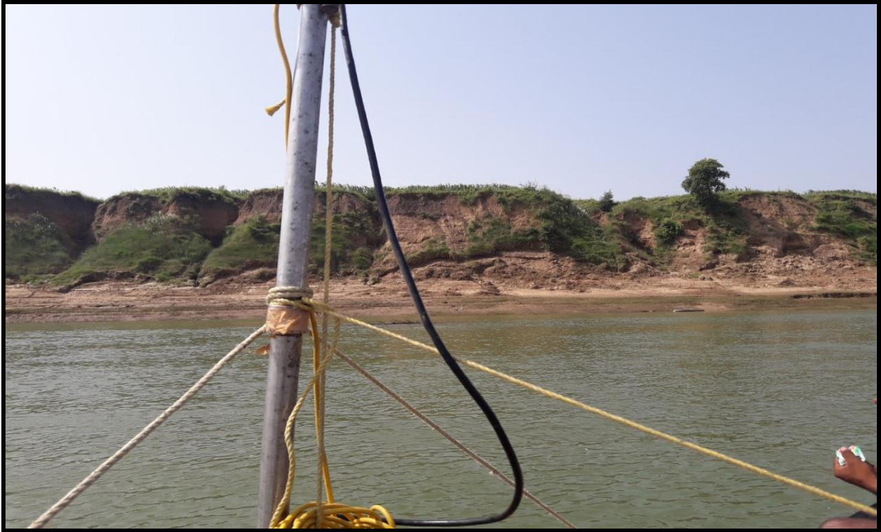
Fig No. 30 Steep cut Right side CH 48.000 km
