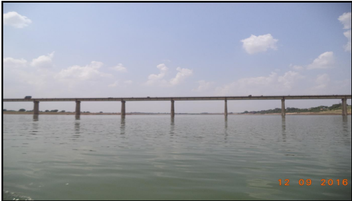
Figure No. - 07 Hamirpur Betwa Bridge CH 8.245 km
