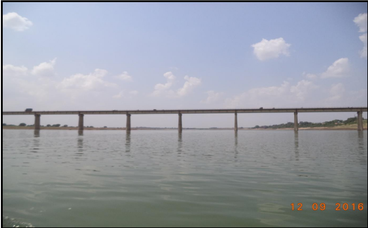
Fig No. 20 Hamirpur Betwa Bridge CH 8.245 km
