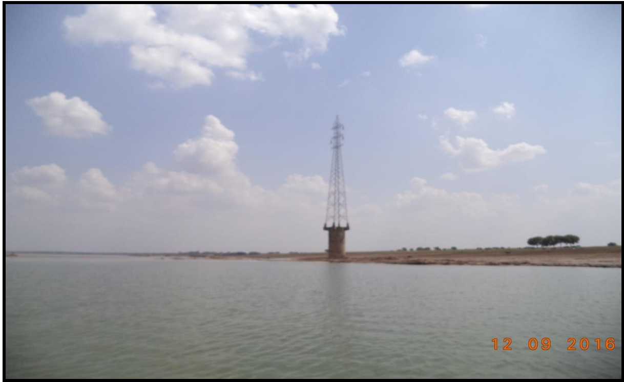
Figure No. - 06 High Tension Power Transmission Ch-7.530 km
