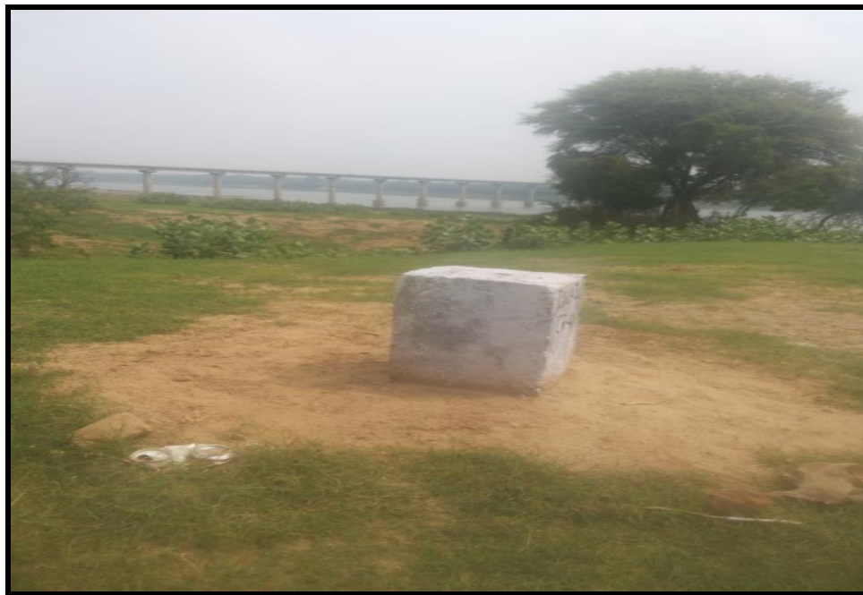
Bridge at chainage 27.312km
