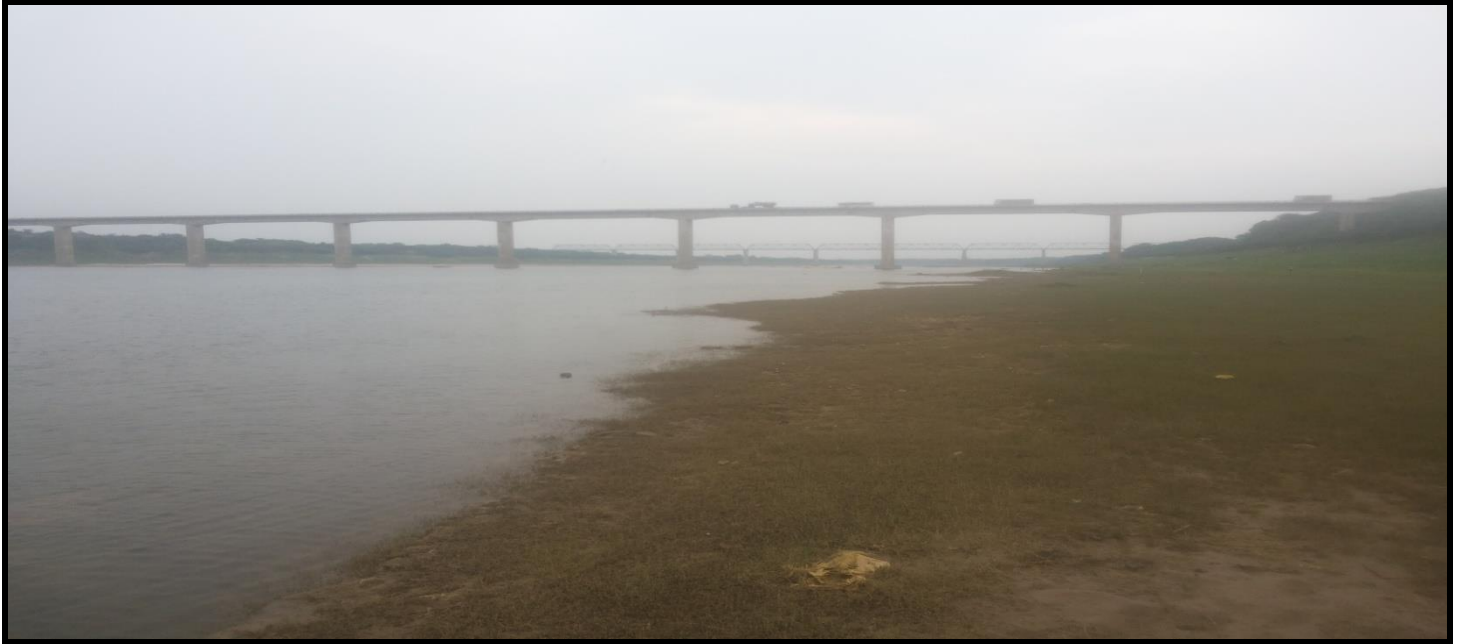
BRIDGE CH 60.953 km
