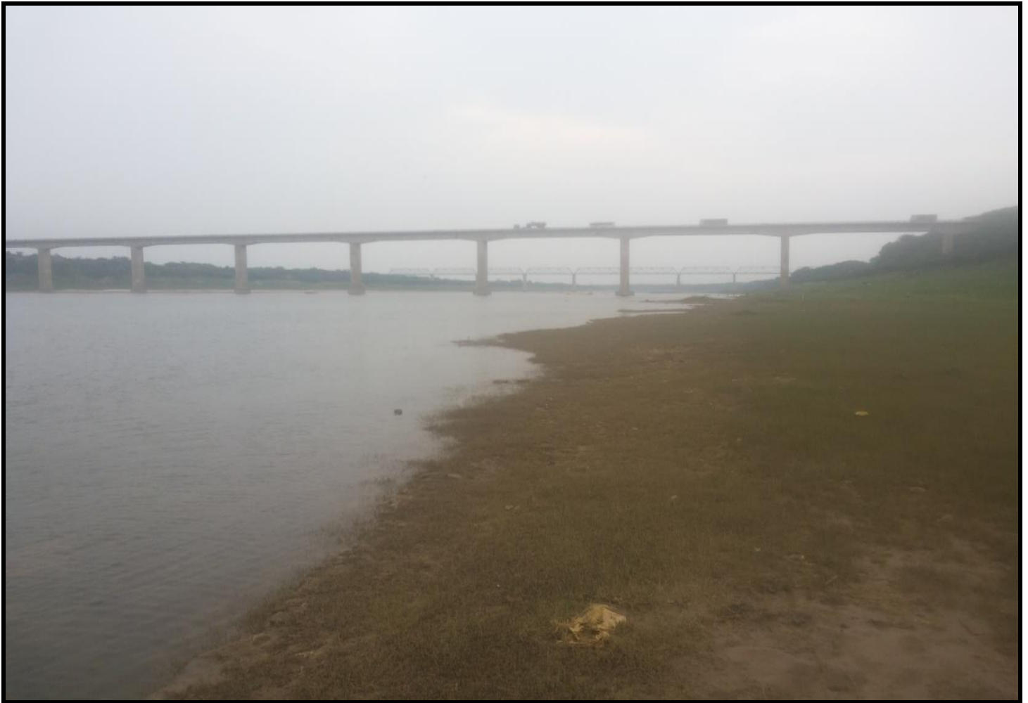
Bridge at chainage 60.954 km
