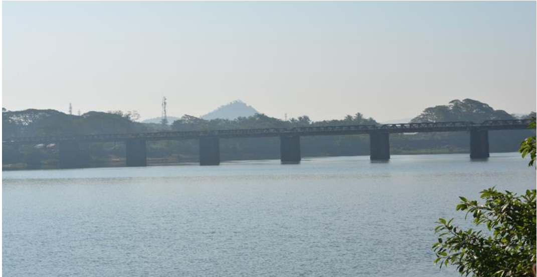
FIGURE 4.8: The Old Bridge on Netravathi River
