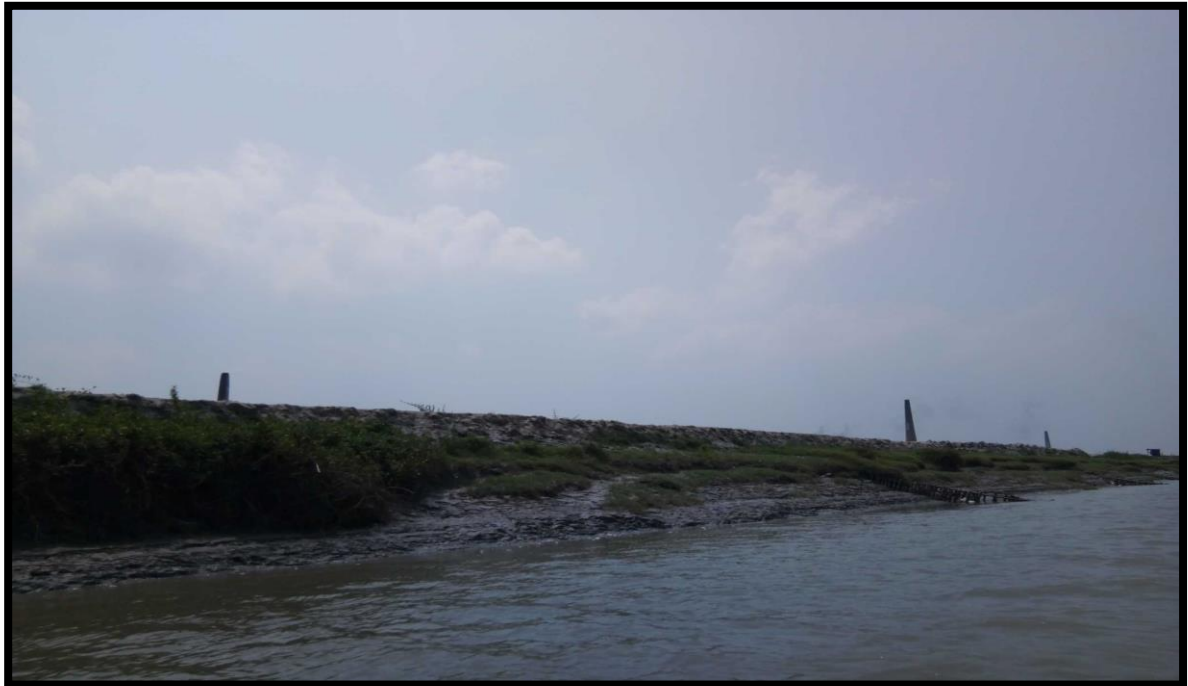
LEFT BANK AT CHAINAGE 21.5
