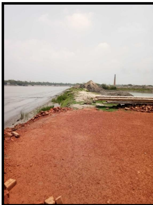
RIVER BANK AT CHAINAGE 3.5, LEFT BANK
