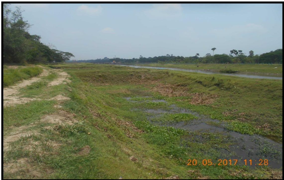
LEFT BANK AT CHAINAGE 61.6
