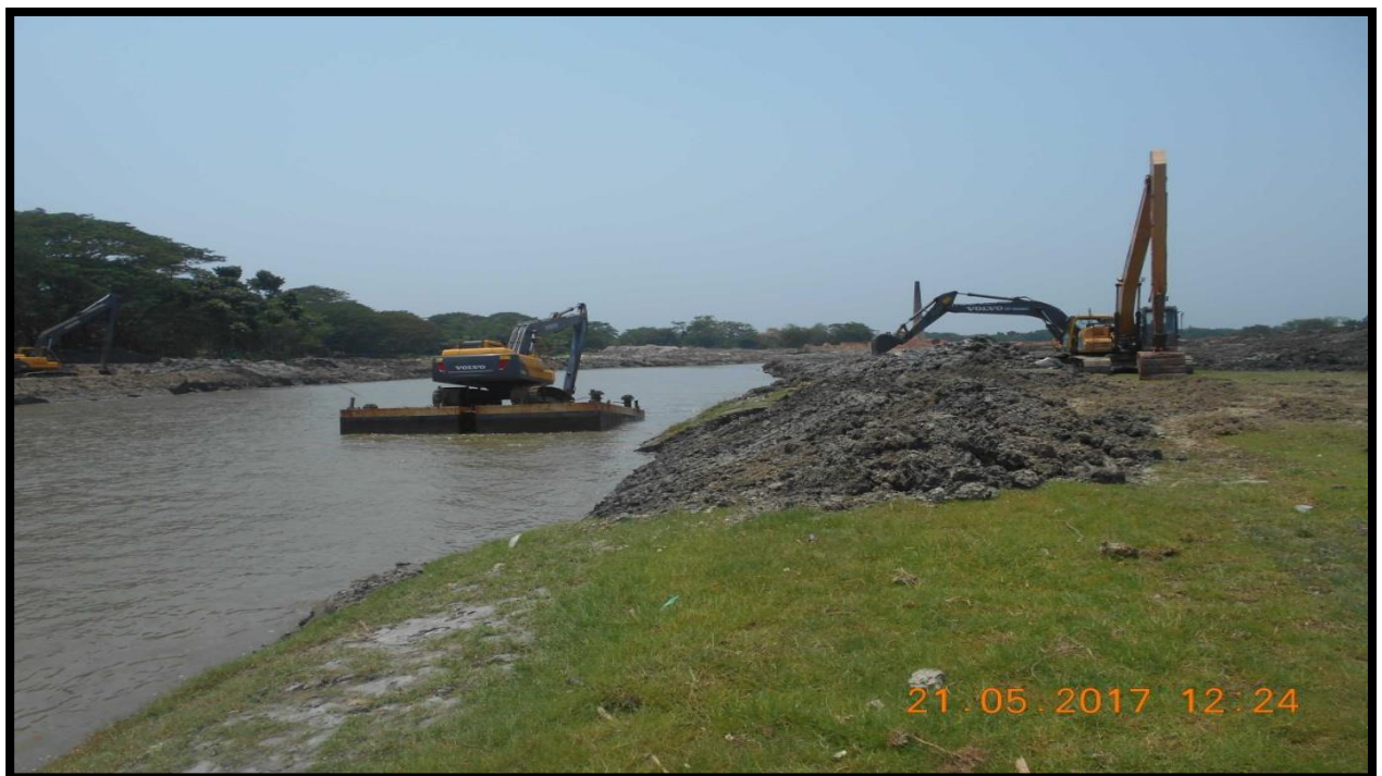
DREDGING AT RIGHT BANK CHAINAGE 45
