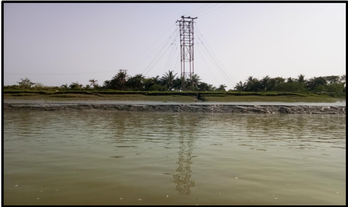
HIGH TENSION LINE AT LEFT BANK CHAINAGE 14.5
