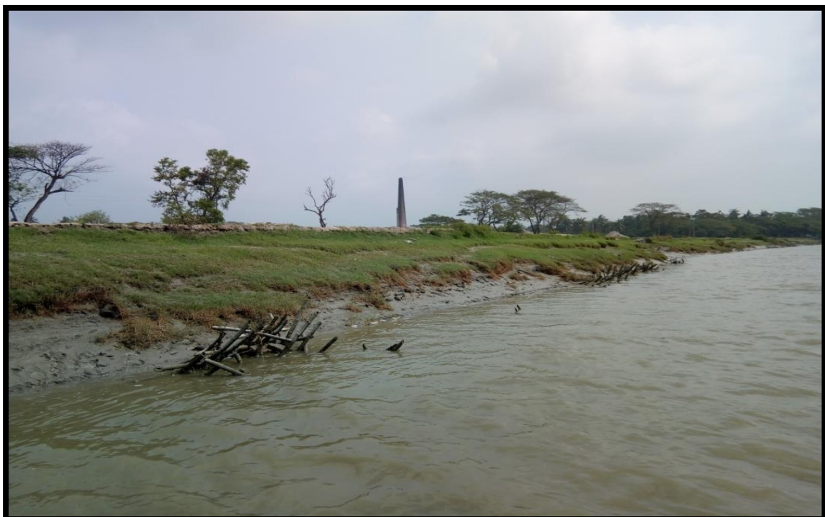
LEFT BANK AT CHAINAGE 28.9
