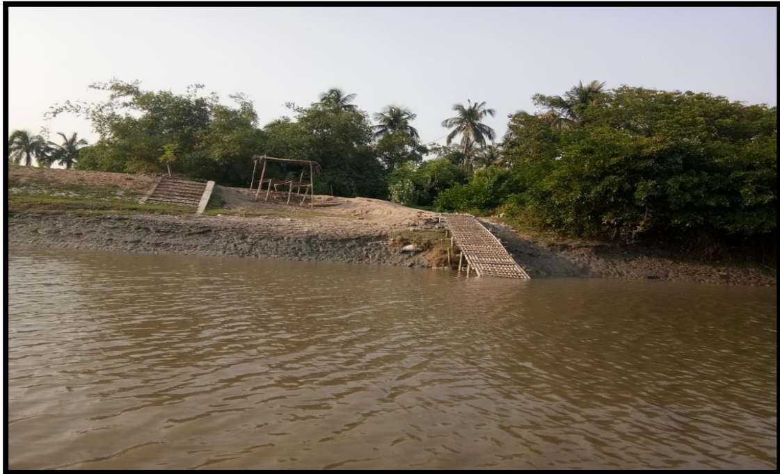
FERRY GHAT AT RIGHT BANK CHAINAGE 17.0
