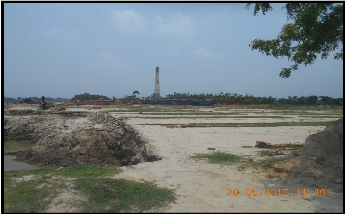
LEFT BANK AT CHAINAGE 60.7
