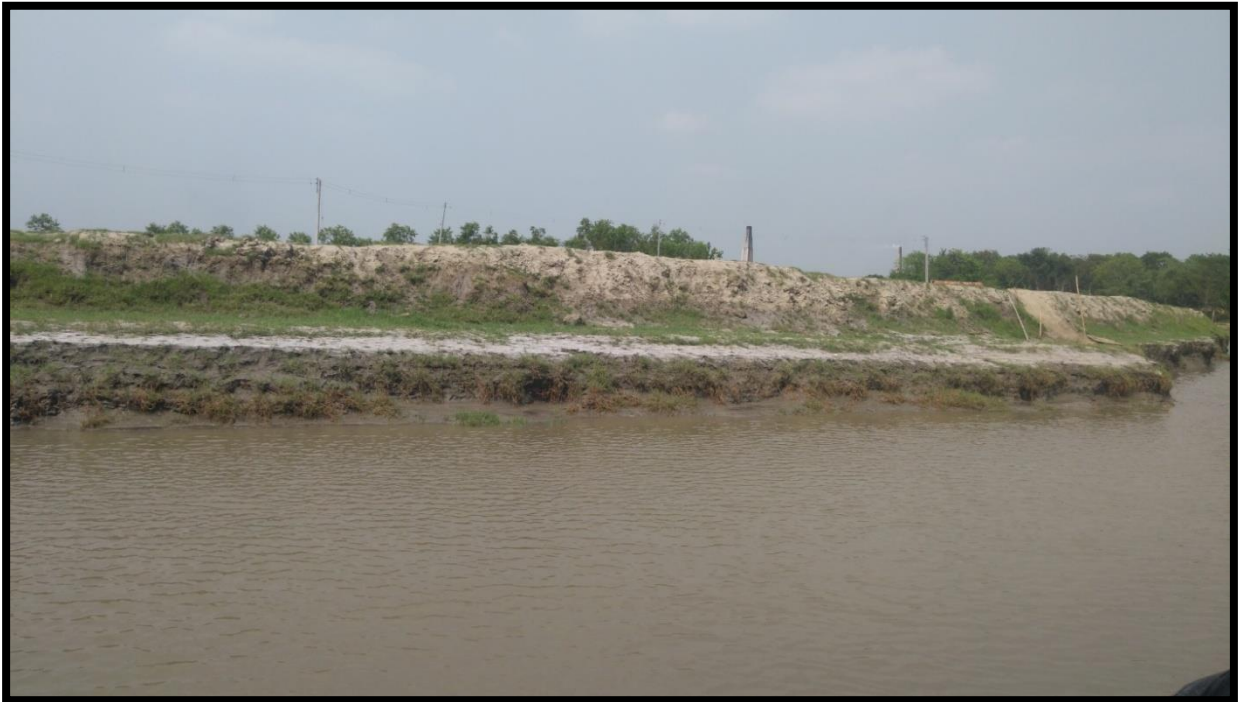
LEFT BANK AT CHAINAGE 29
