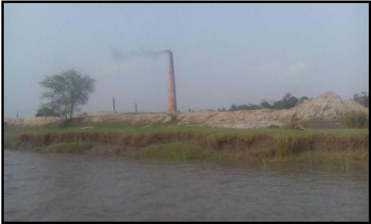
BRICK KLIN 8.4 CHAINAGE, RIGHT BANK
