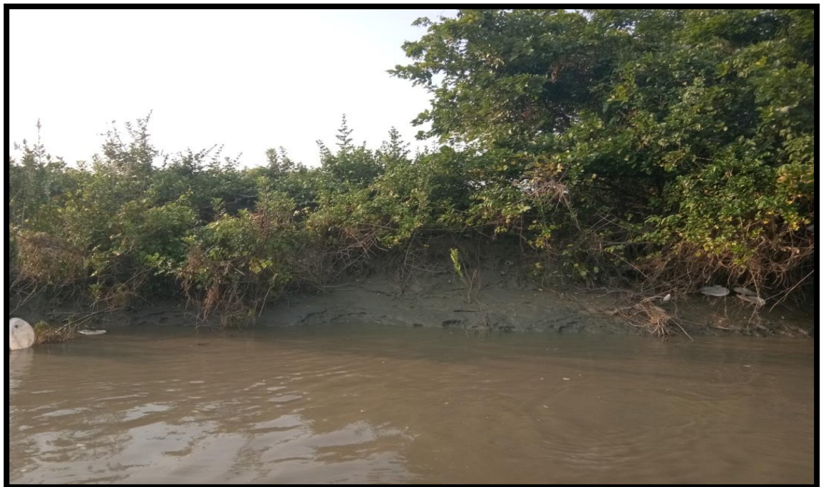
RIGHT BANK AT CHAINAGE 17.6
