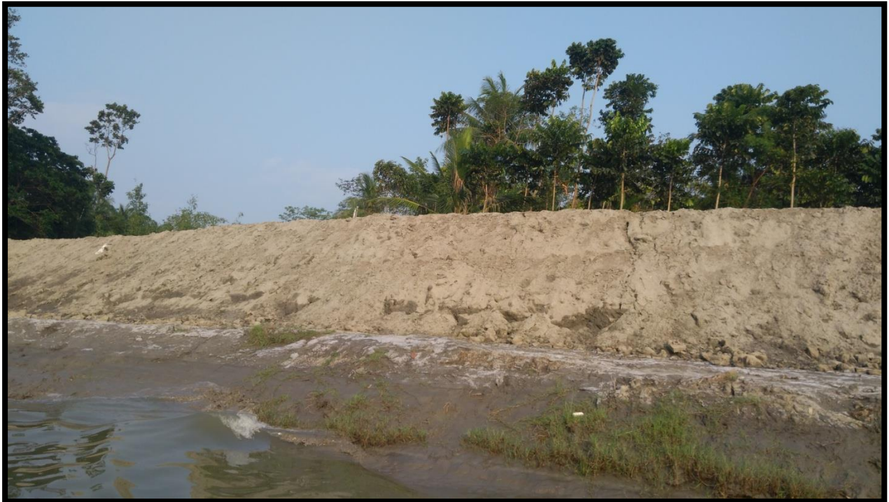
RIGHT BANK AT CHAINAGE 38.5
