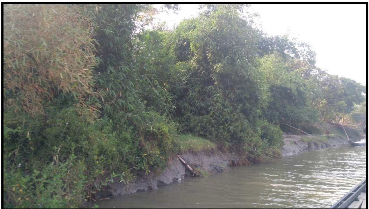
LEFT BANK AT CHAINAGE 37
