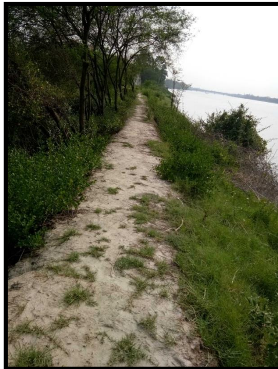
RIVER BANK AT CHAINAGE 6.2, LEFT BANK
