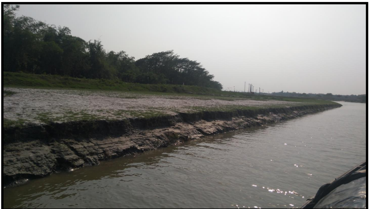
LEFT BANK AT CHAINAGE 35
