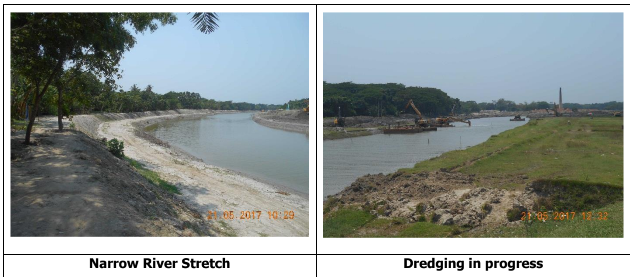
Figure 16: Photograph along Sub-Stretch 5
