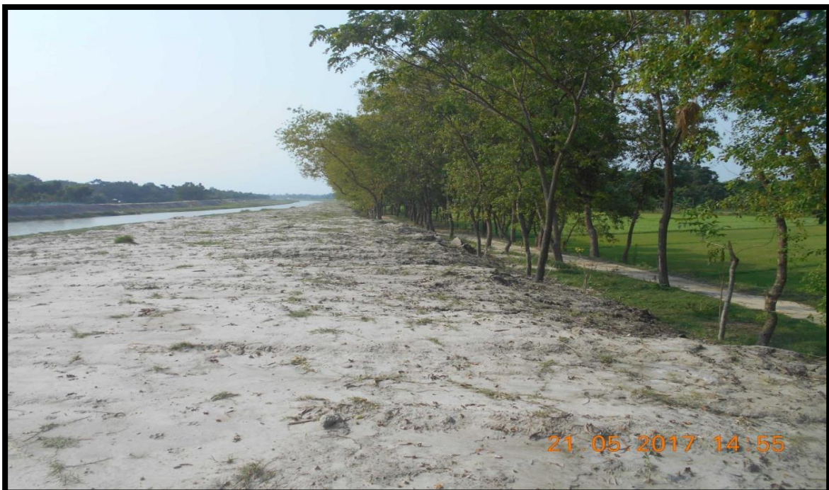
RIGHT BANK AT CHAINAGE 49.6
