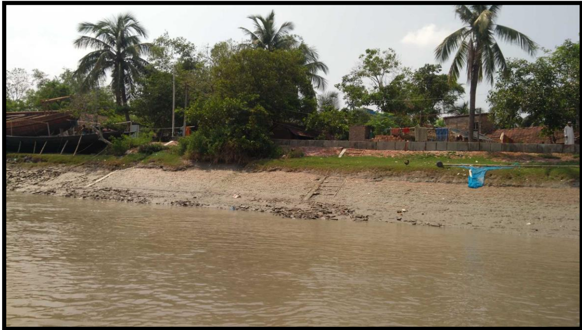
RIVER BANK PROTECTION AT 4.4 CHAINAGE, RIGHT BANK
