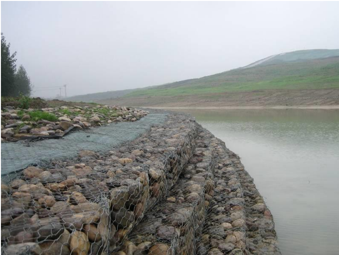
Figure 22: Photograph showing arrangement of Gabion Wall along River Bank
