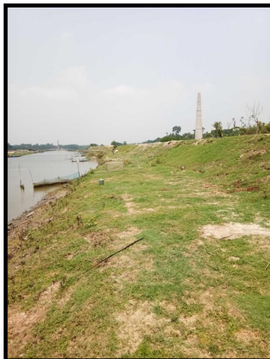
RIGHT BANK AT CHAINAGE 62.1
