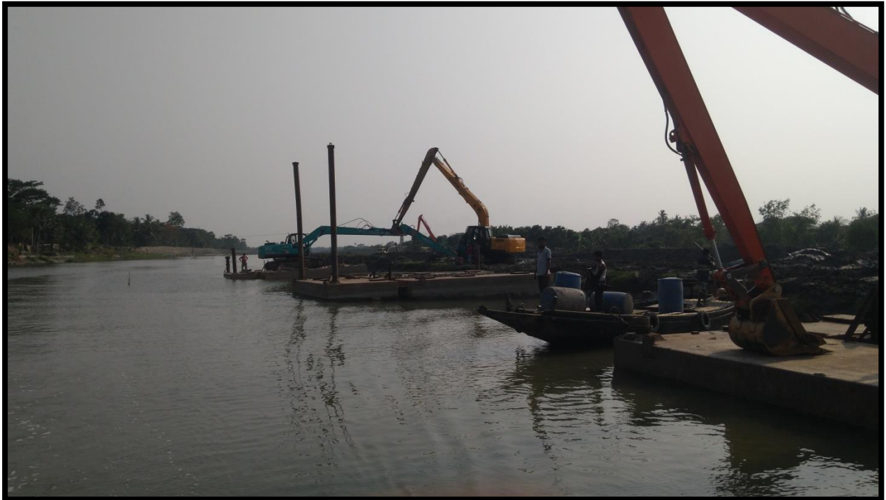
DREDGING AT LEFT BANK CHAINAGE 30
