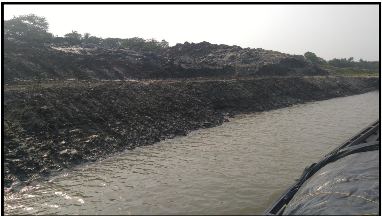
LEFT BANK AT CHAINAGE 36
