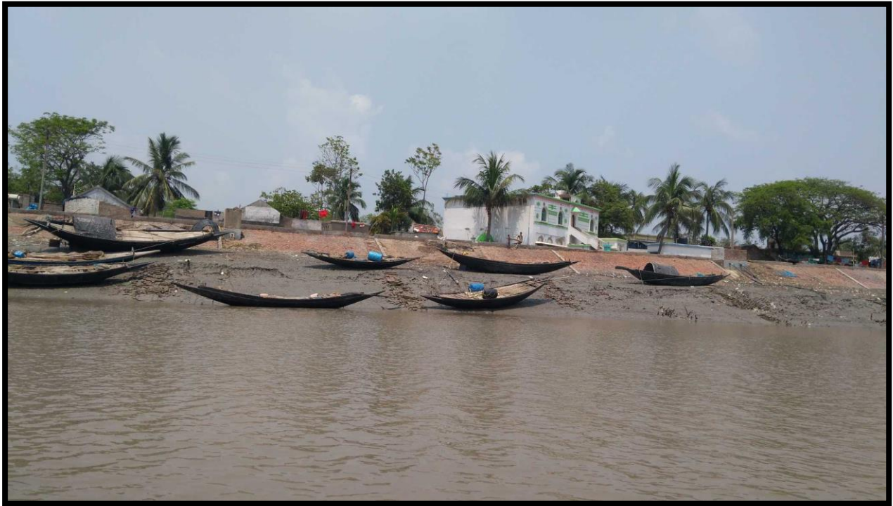
RIVER BANKPROTECTION, 2.5 CHAINAGE, RIGHT BANK
