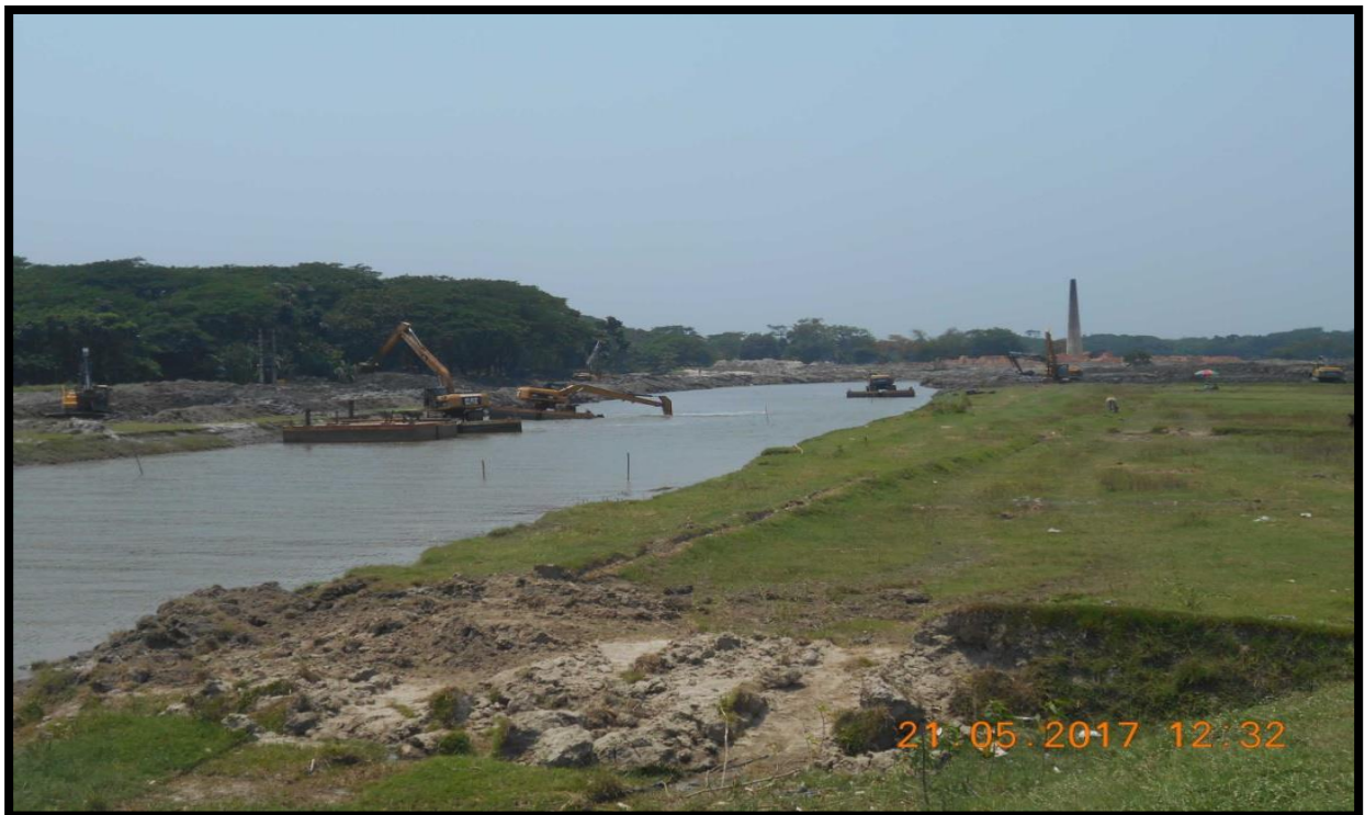
DREDGING AT RIGHT BANK CHAINAGE 45.5
