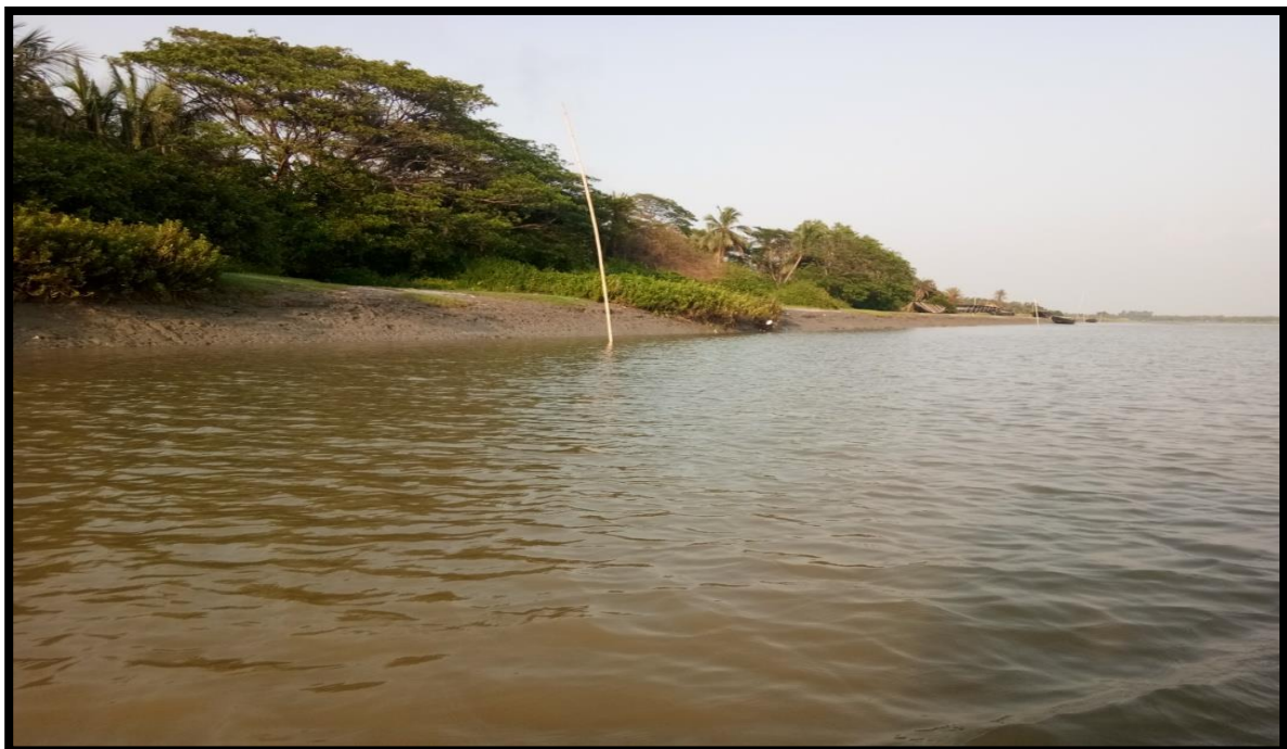
RIGHT BANK AT CHAINAGE 16.8
