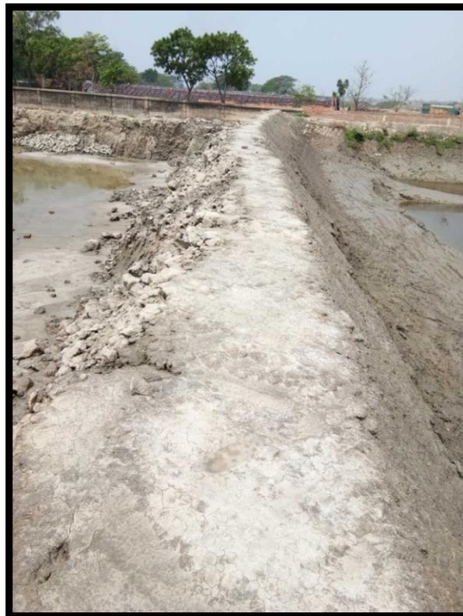
RIVER BANK AT CHAINAGE 3.3, LEFT BANK
