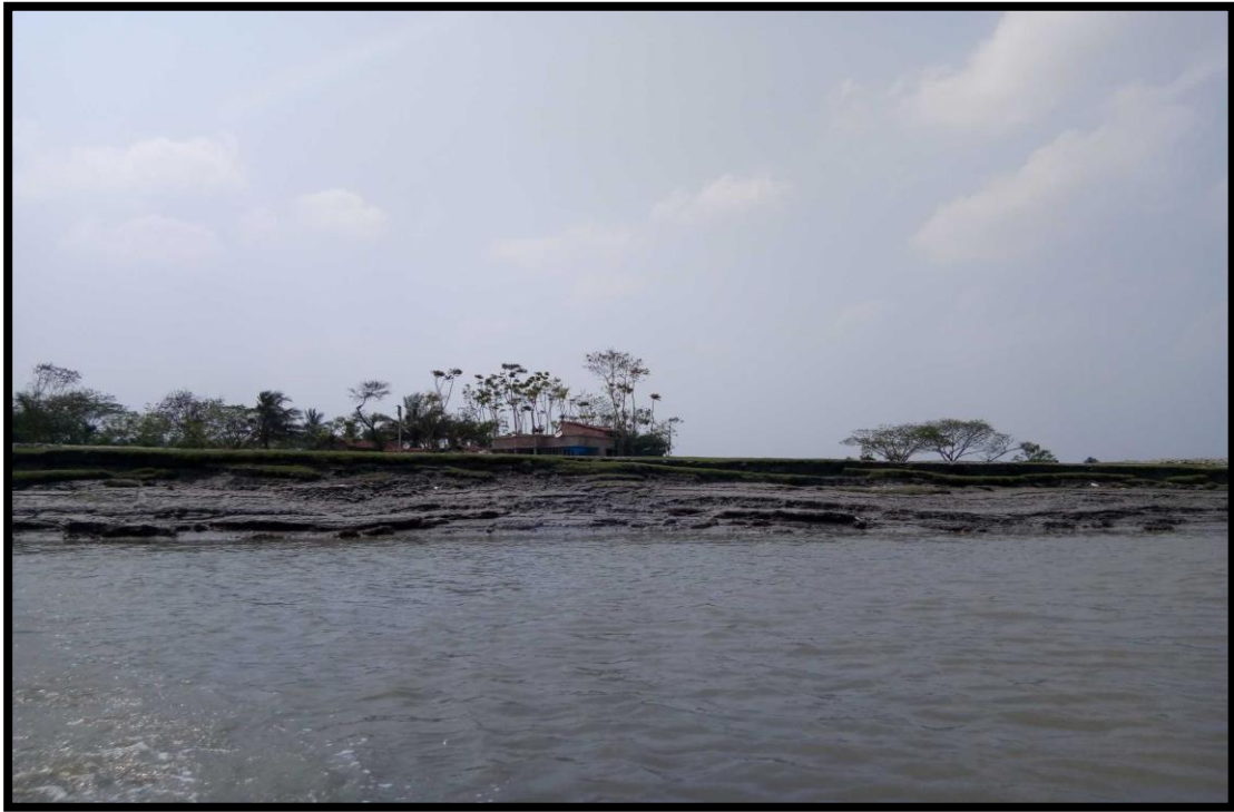
LEFT BANK AT CHAINAGE 22
