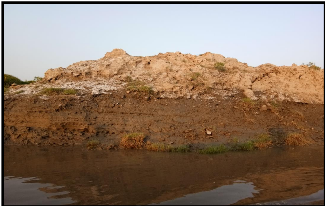
RIGHT BANK AT CHAINAGE 19.1
