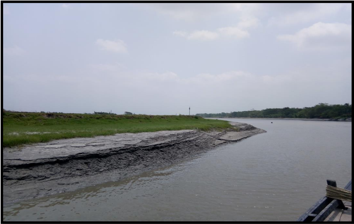
LEFT BANK AT CHAINAGE 27.2
