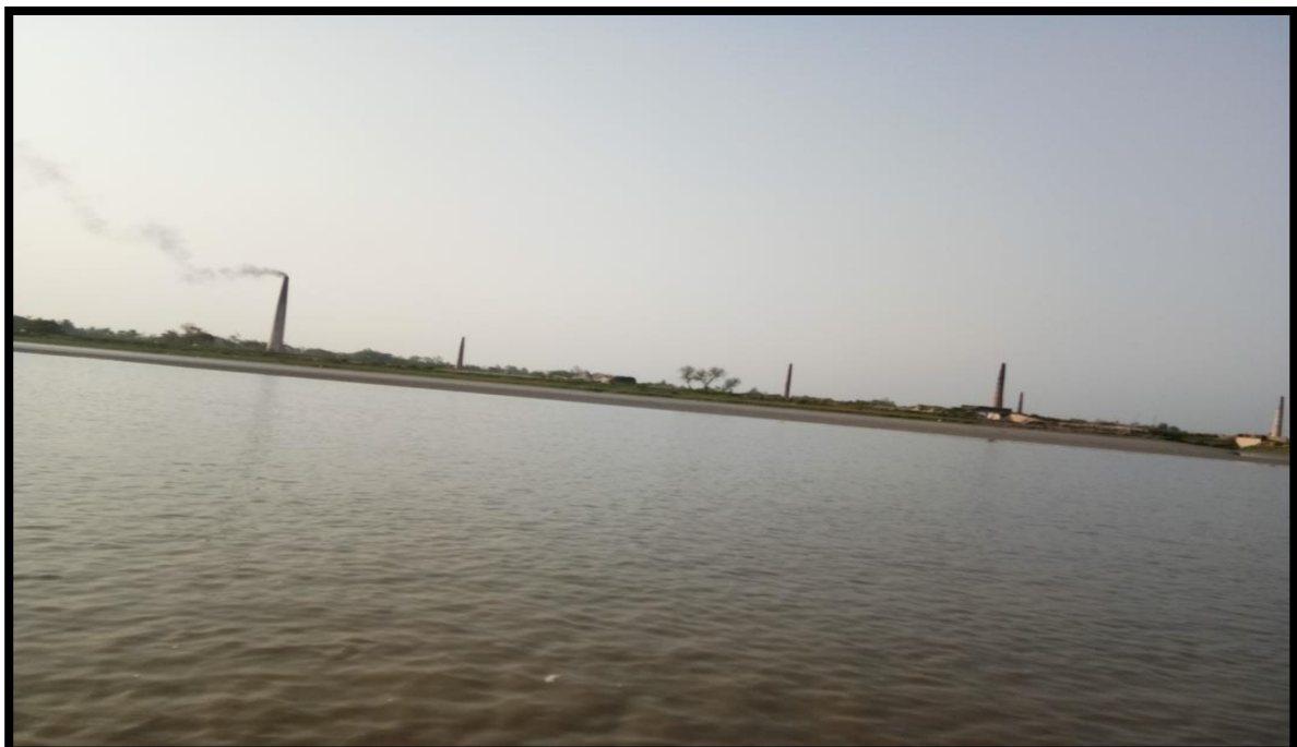
BRICK KLINS AT LEFT BANK CHAINAGE 16.3
