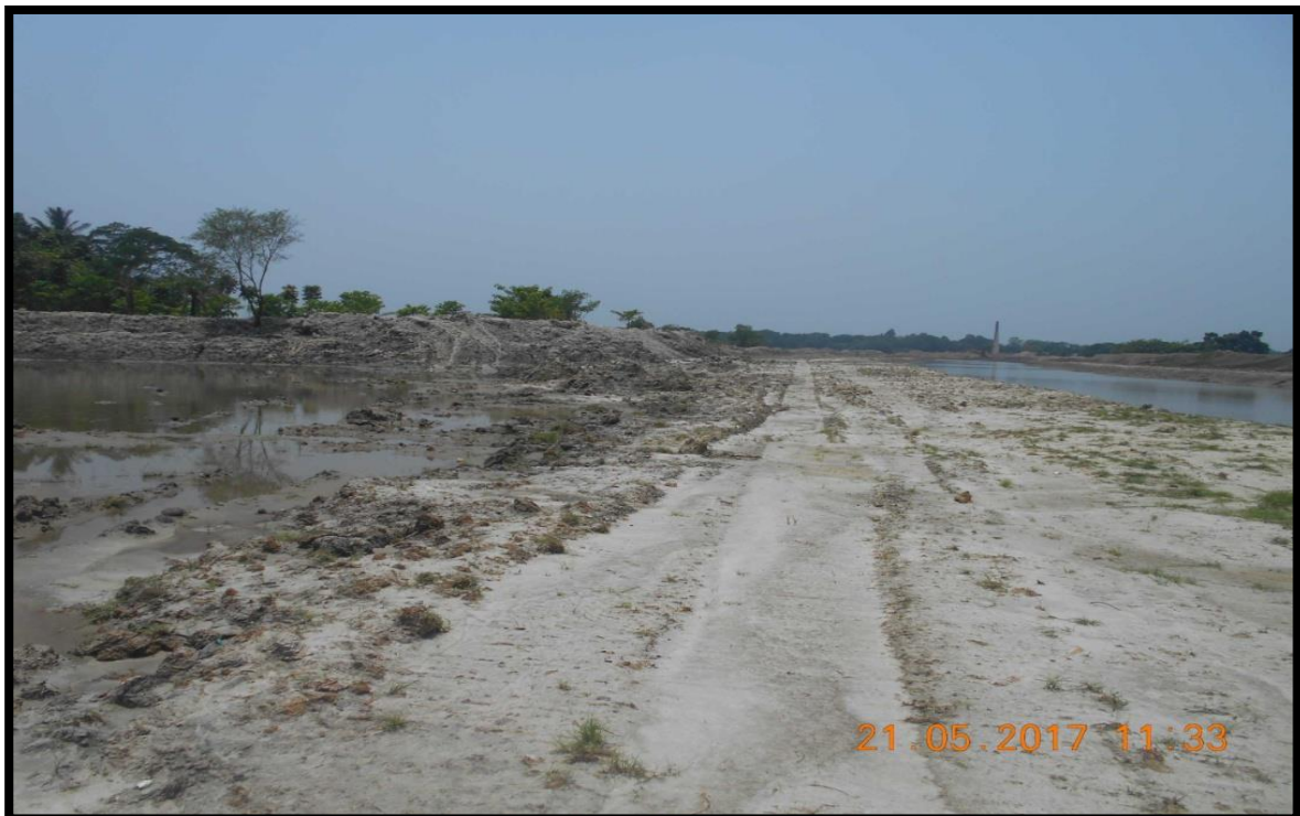
RIGHT BANK AT CHAINAGE 46.5
