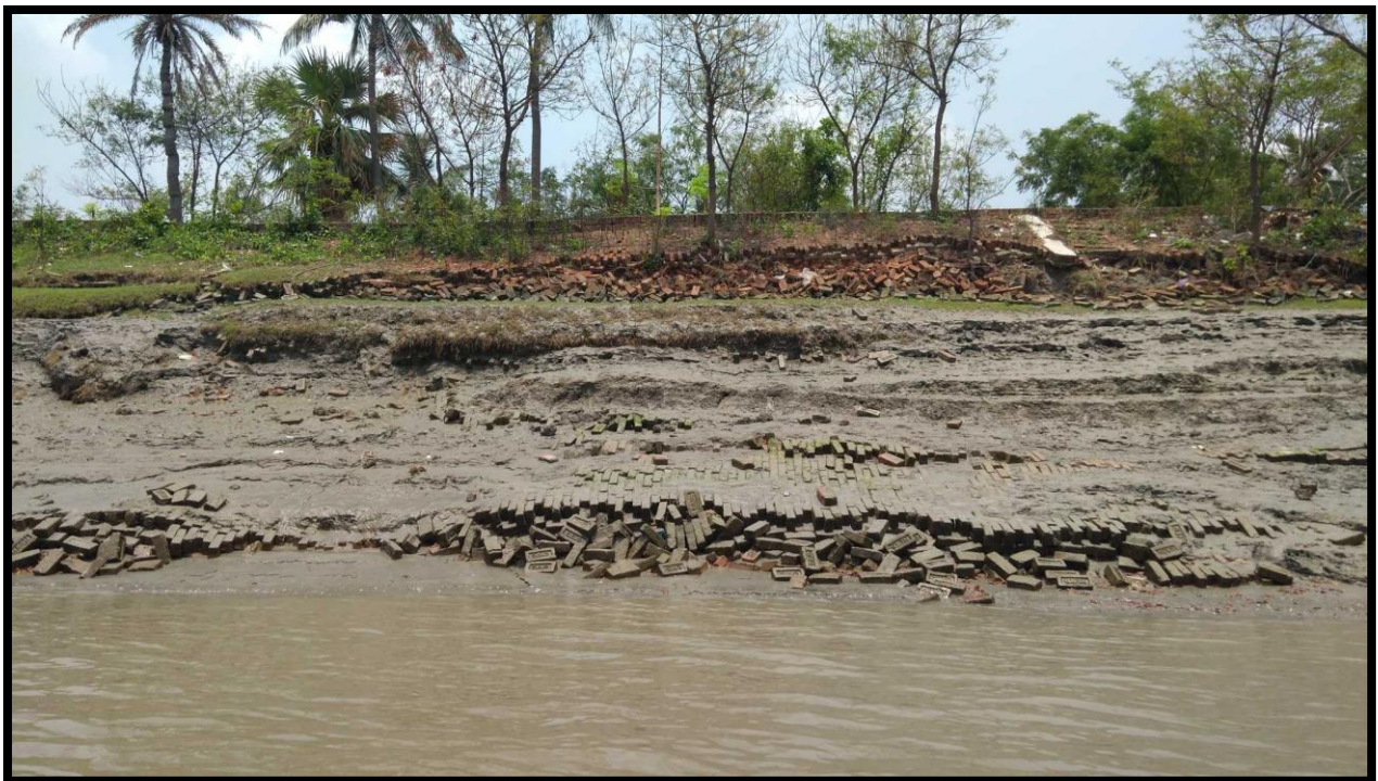
RIVER BANK PROTECTION, 1.5 CHAINAGE, RIGHT BANK
