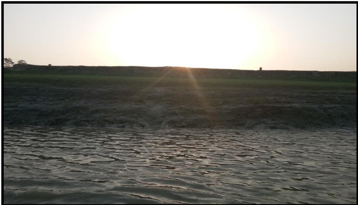
RIGHT BANK AT CHAINAGE 19.7
