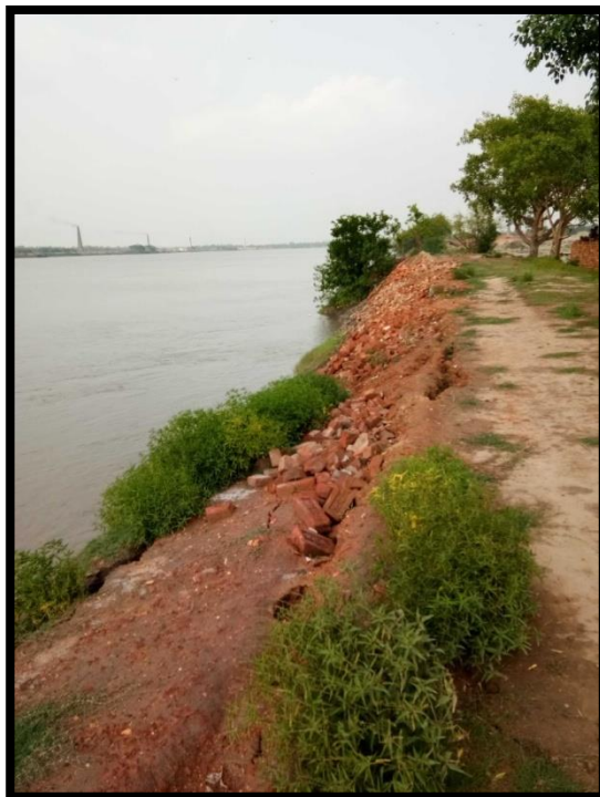
RIVER BANK AT CHAINAGE 4.7, LEFT BANK
