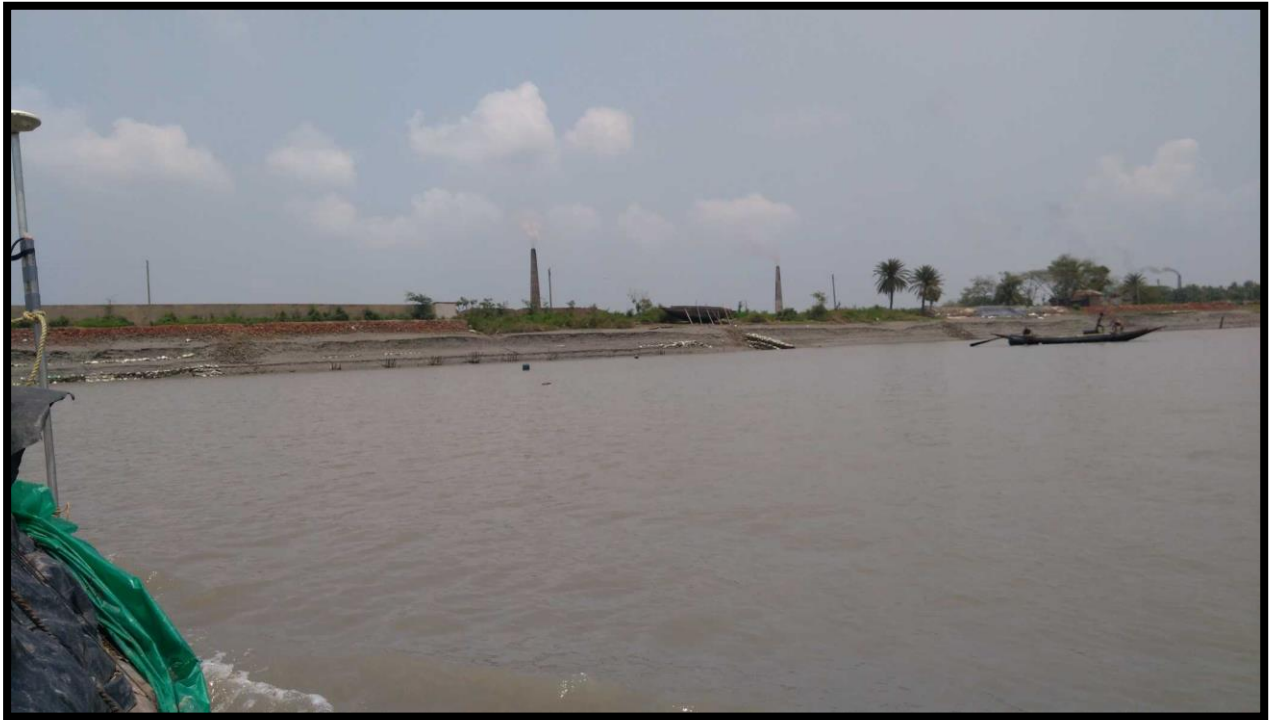
BRICK KLIN, 1.5 CHAINAGE, LEFT BANK
