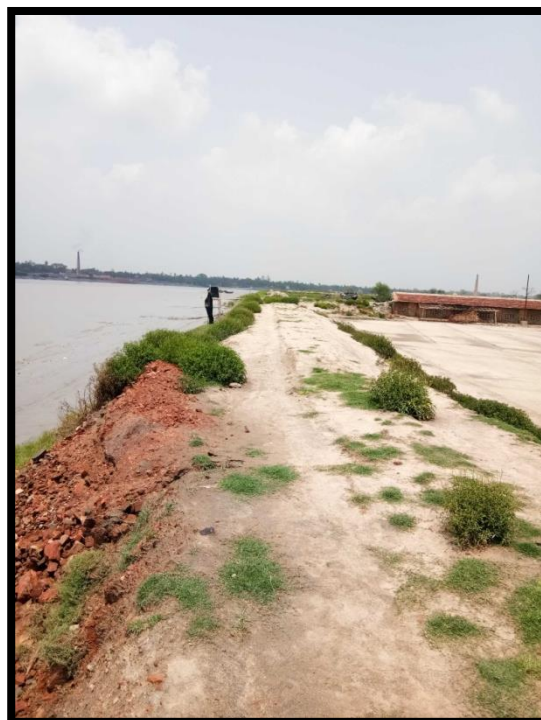
RIVER BANK AT CHAINAGE 4.1, LEFT BANK
