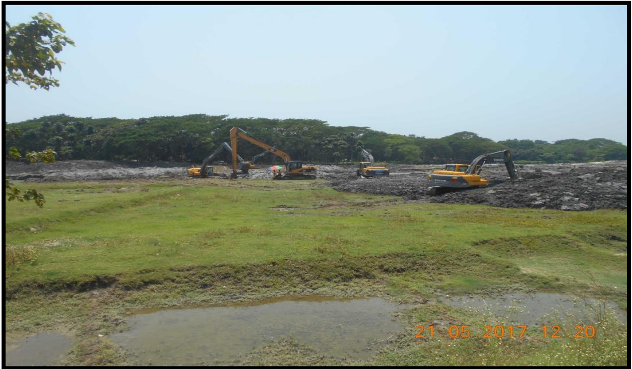
DREDGING AT RIGHT BANK CHAINAGE 45.6
