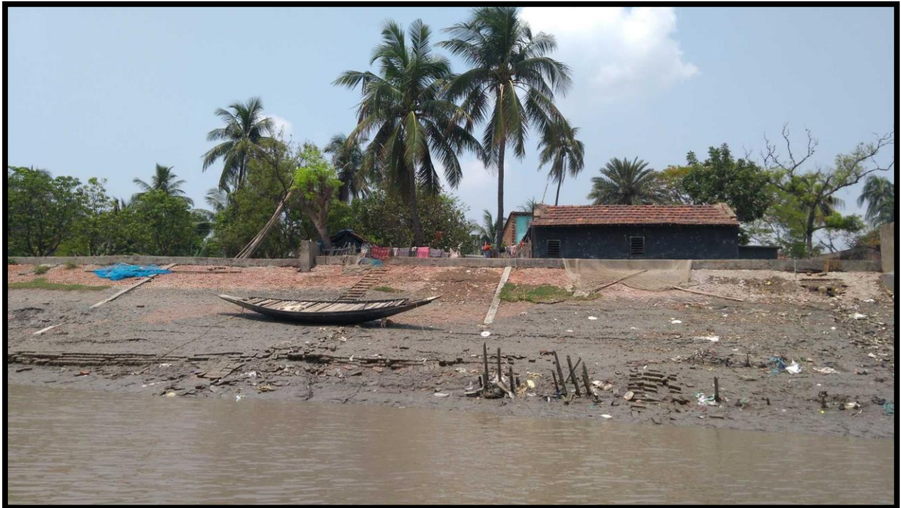
RIVER BANKPROTECTION, 3.3 CHAINAGE, RIGHT BANK
