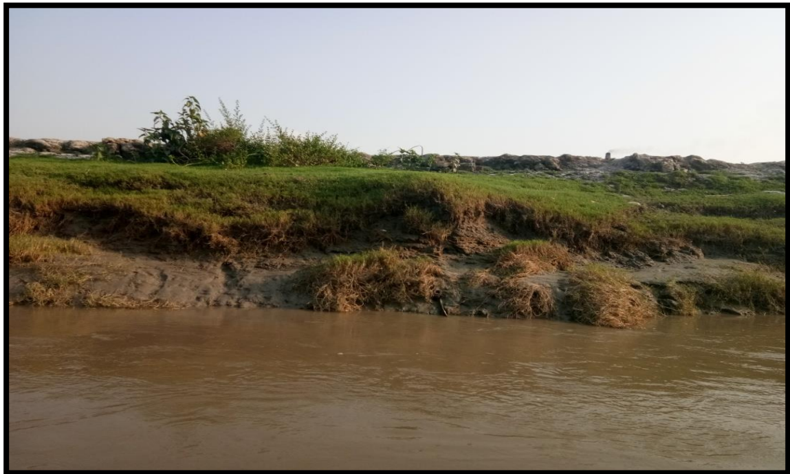
RIGHT BANK AT CHAINAGE 16.3
