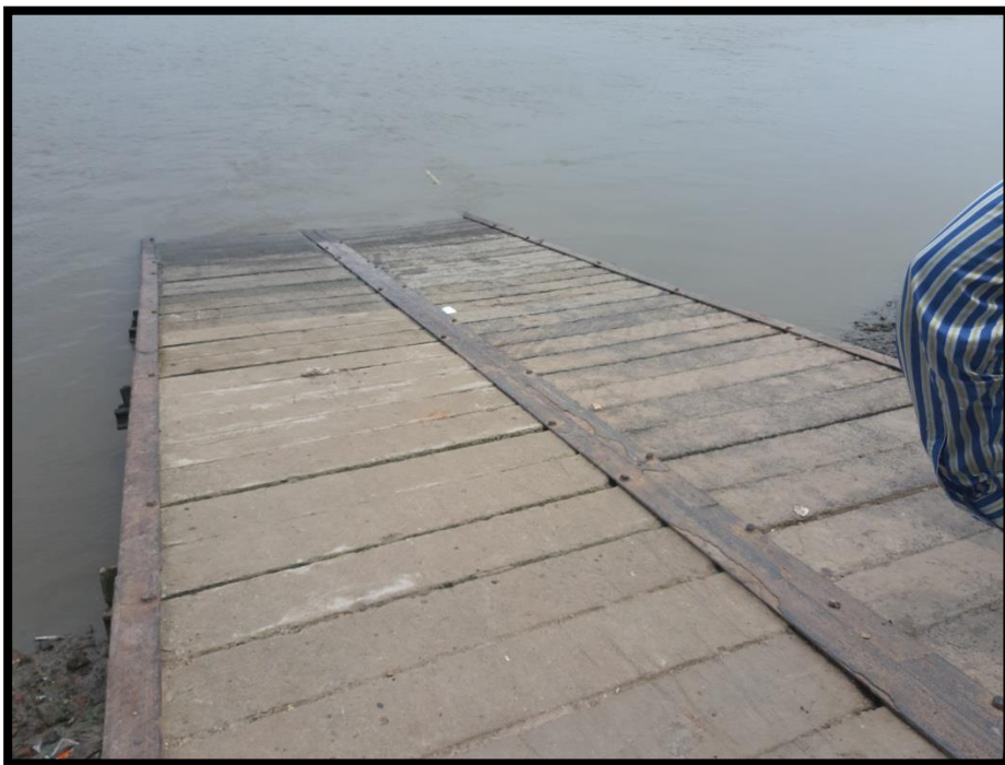
Existing jetty for ferry operations at Basirhat
