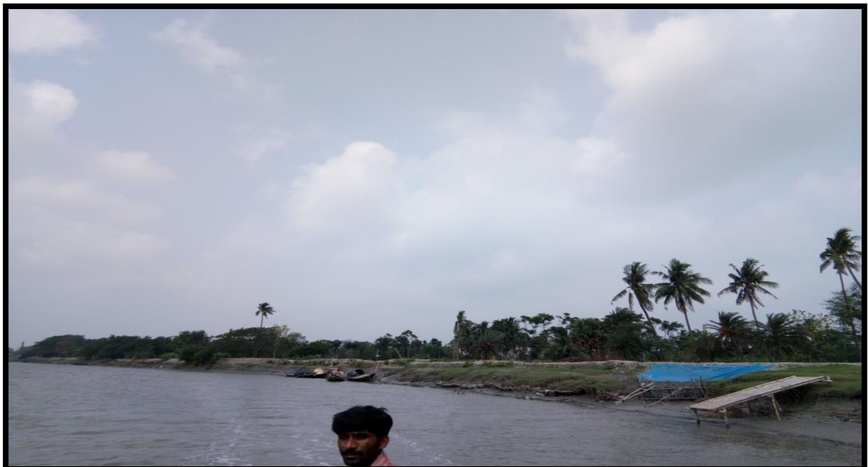
LEFT BANK AT CHAINAGE 29.5
