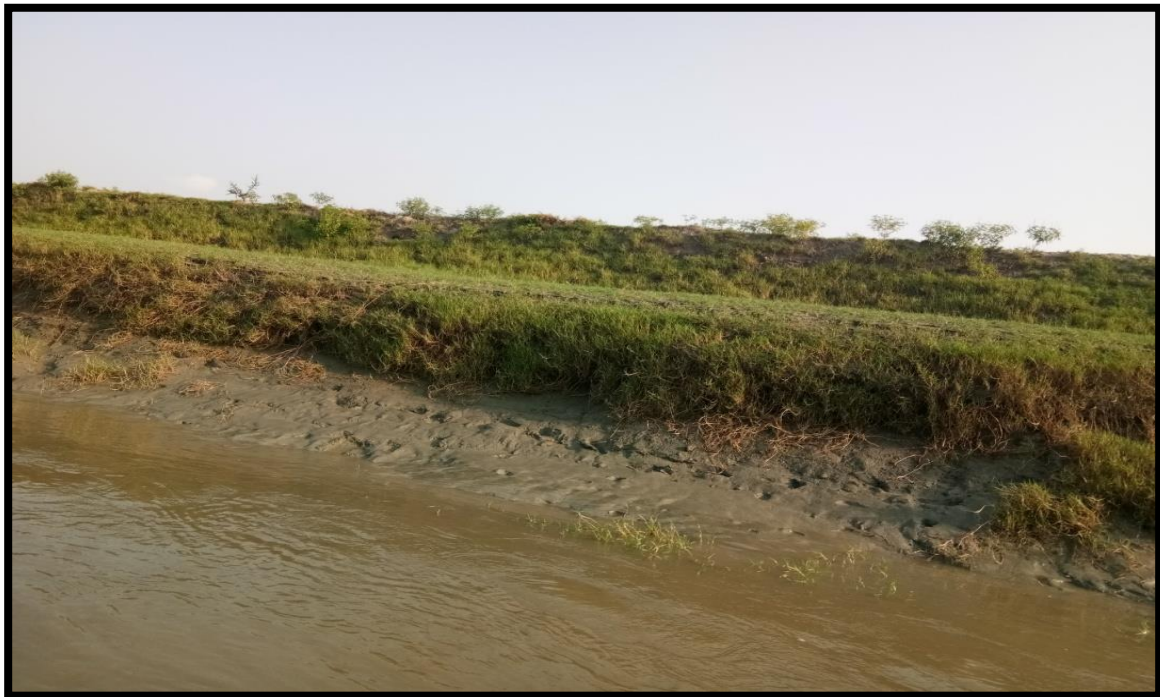
LEFT BANK AT CHAINAGE 16.2
