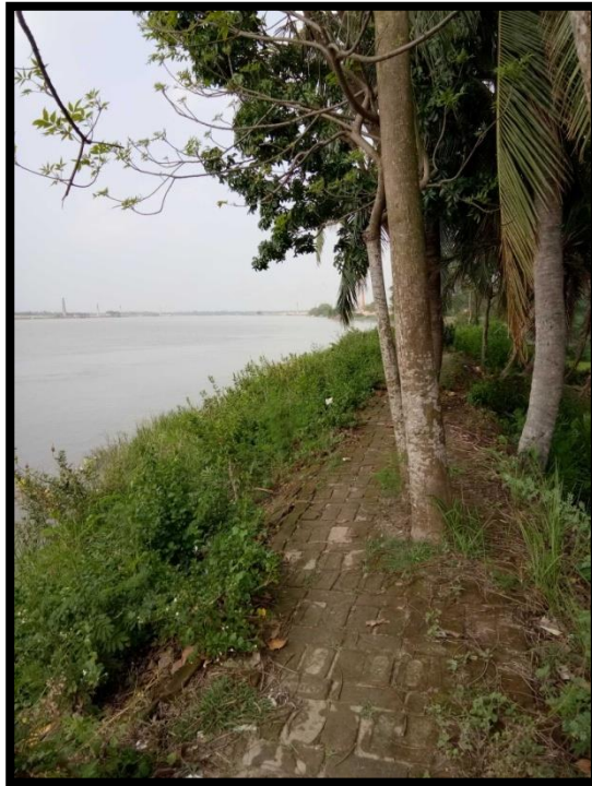
RIVER BANK AT CHAINAGE 6.4, LEFT BANK
