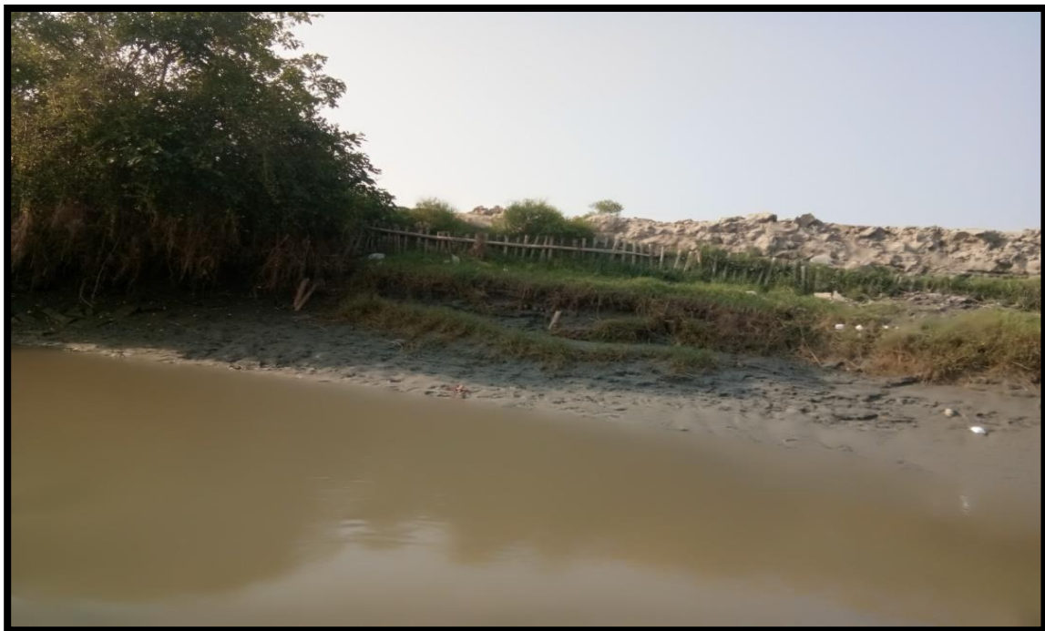
LEFT BANK AT CHAINAGE 15
