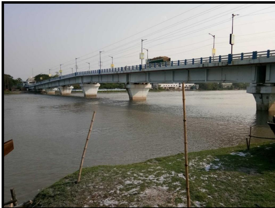
ICHAMATI BRIDGE AT CHAINAGE 7.4, LEFT BANK
