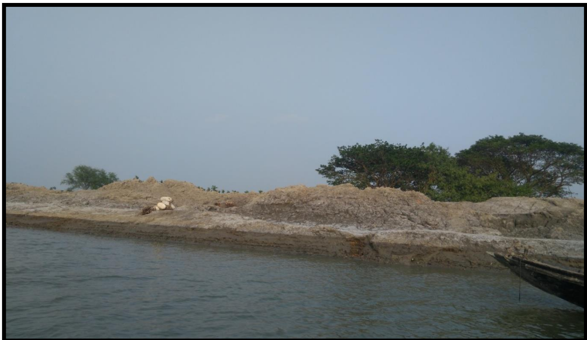
RIGHT BANK AT CHAINAGE 28
