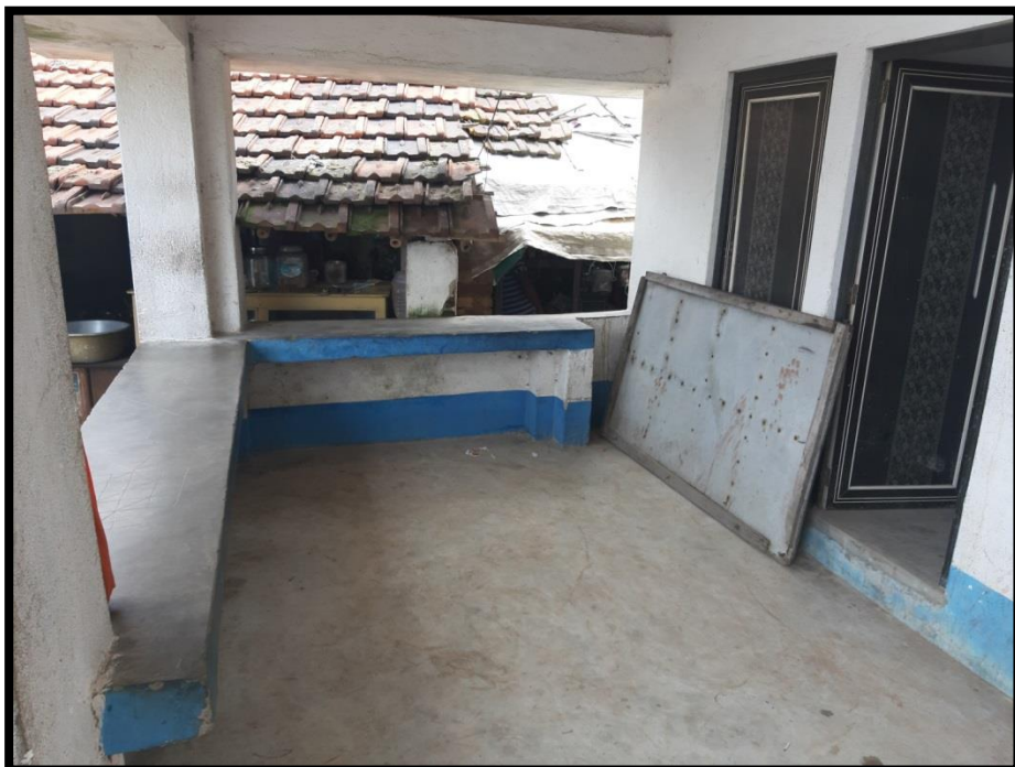
Existing building for passengers at Basirhat ferry Ghat (Pic 2)
