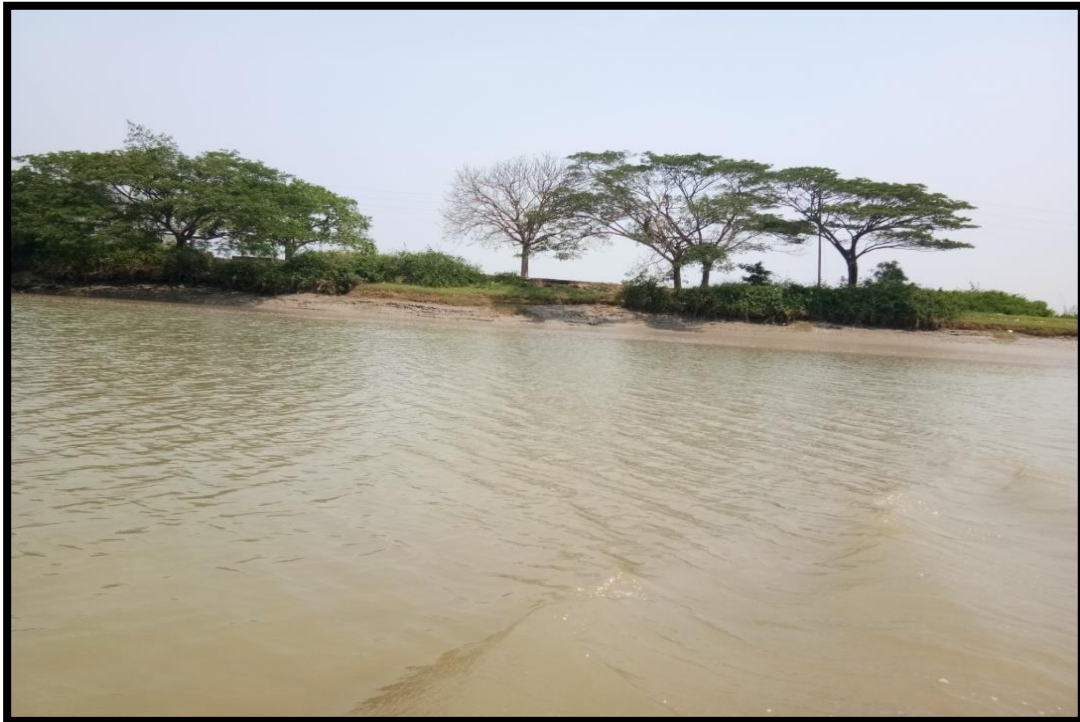
RIGHT BANK AT CHAINAGE 12.8
