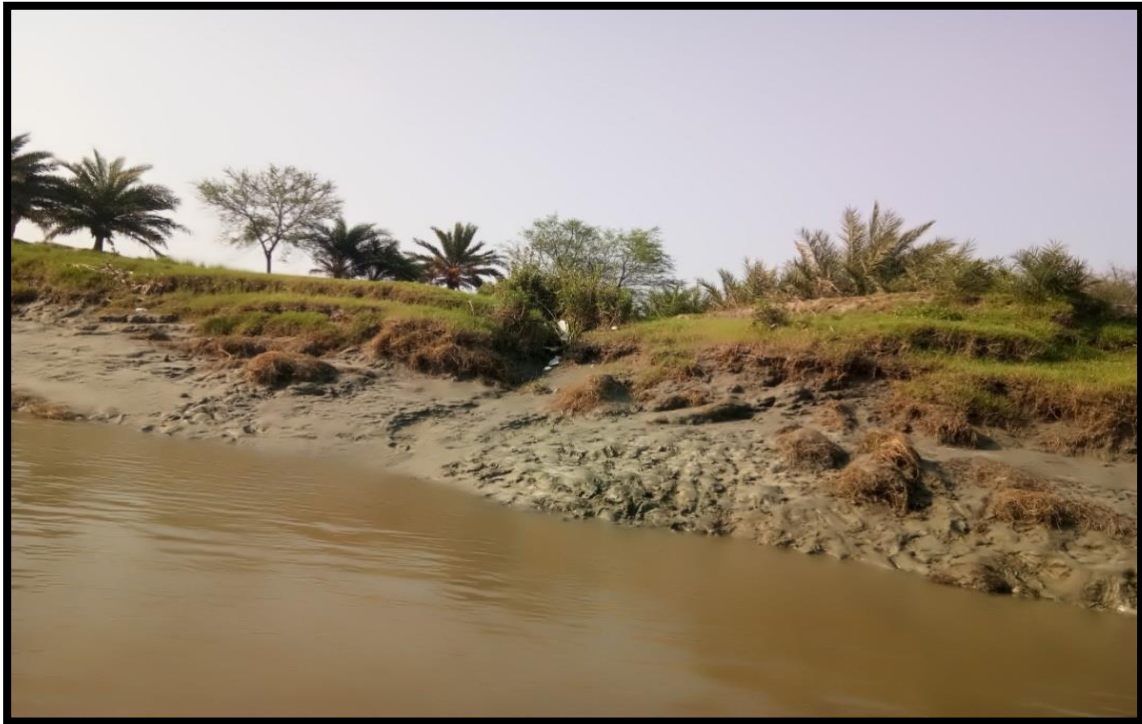
LEFT BANK AT CHAINAGE 14.9
