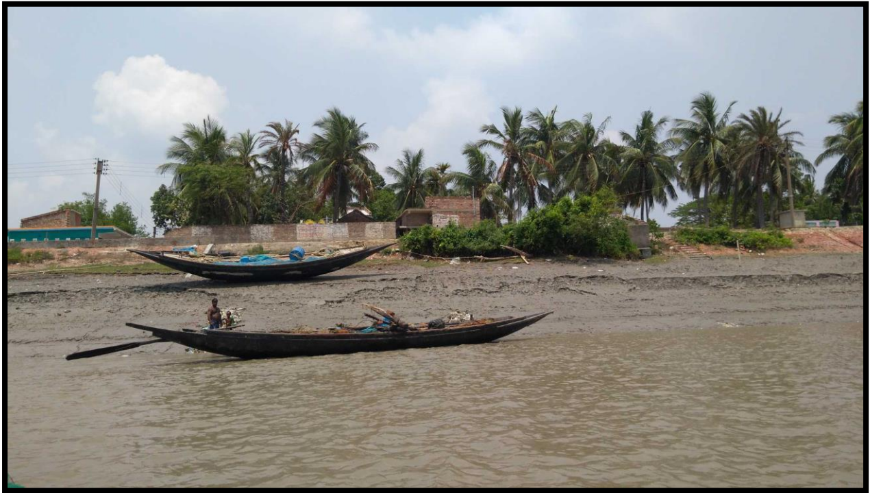
RIVER BANKPROTECTION, 2.3 CHAINAGE, RIGHT BANK
