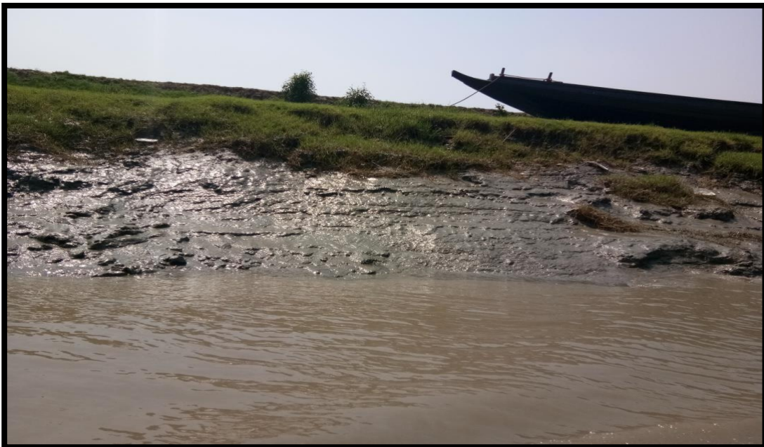
LEFT BANK AT CHAINAGE 11.2
