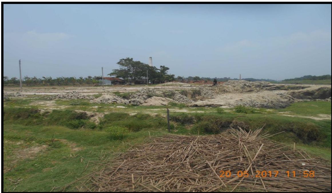
LEFT BANK AT CHAINAGE 60.8
