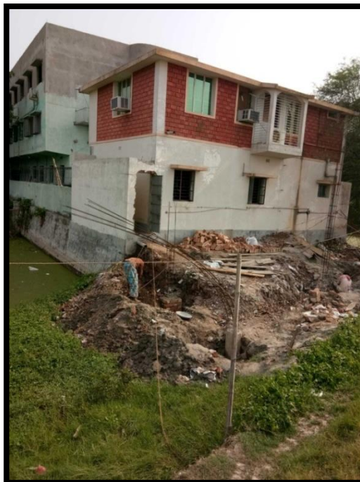
STRUCTURE AT CHAINAGE 6.4, LEFT BANK
