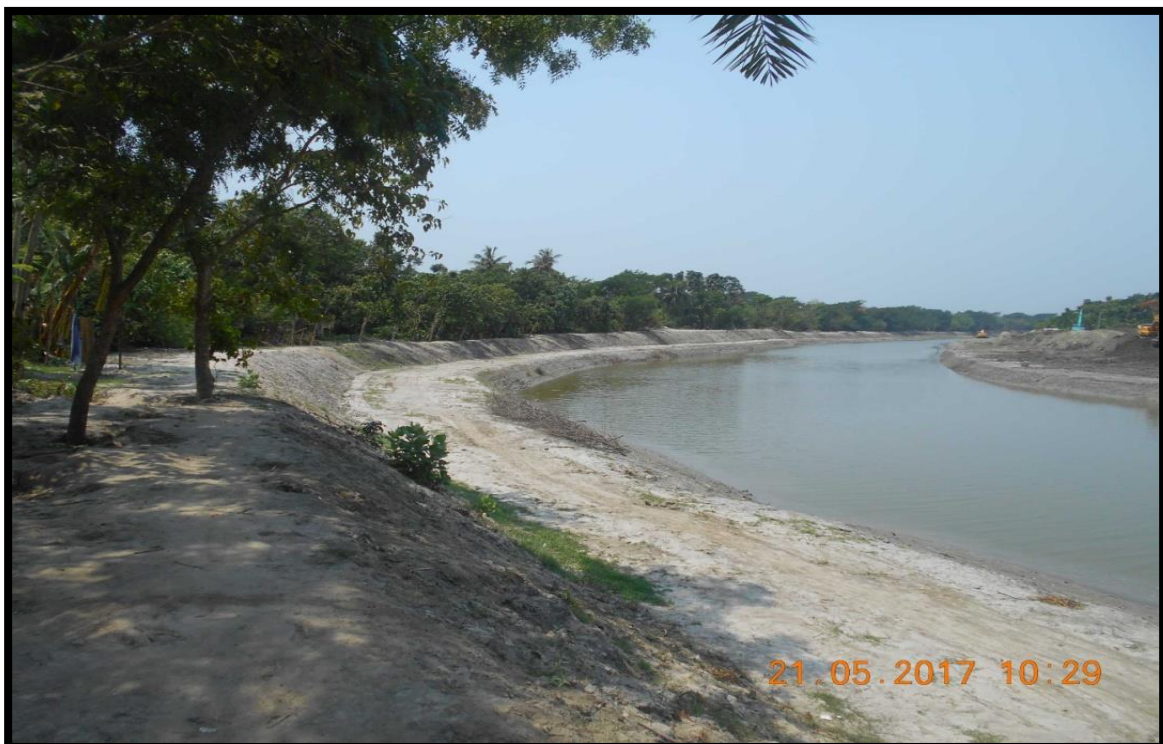
RIGHT BANK AT CHAINAGE 48.8
