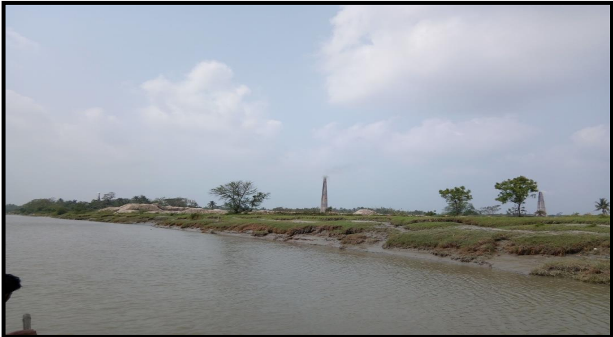
RIGHT BANK AT CHAINAGE 30.7
