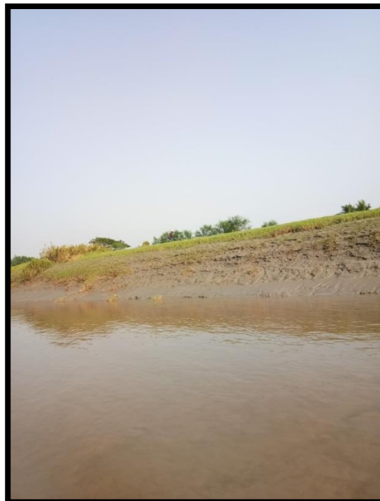
LEFT BANK AT CHAINAGE 15.2
