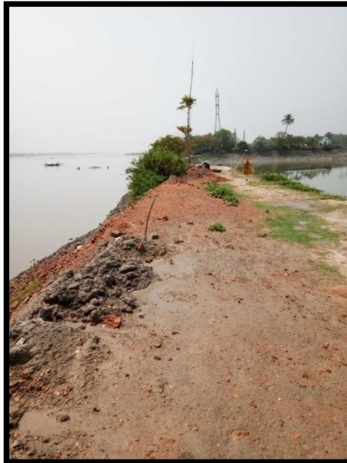
RIVER BANK AT CHAINAGE 3.1, LEFT BANK
