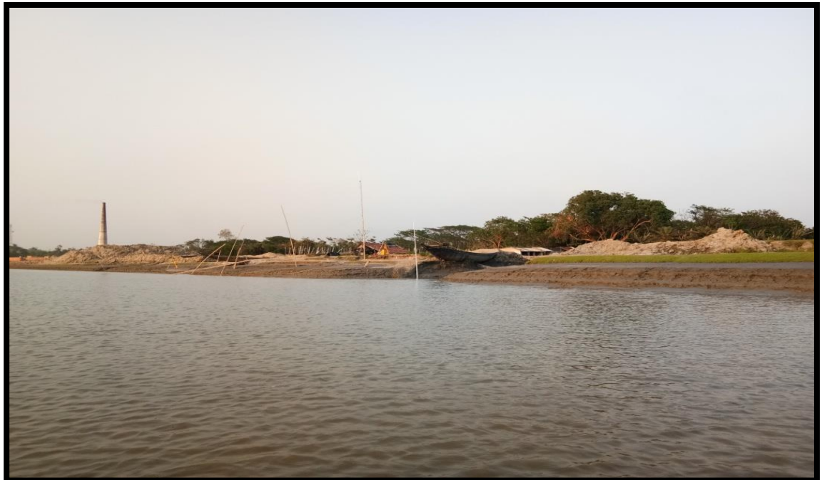
LEFT BANK AT CHAINAGE 19.6
