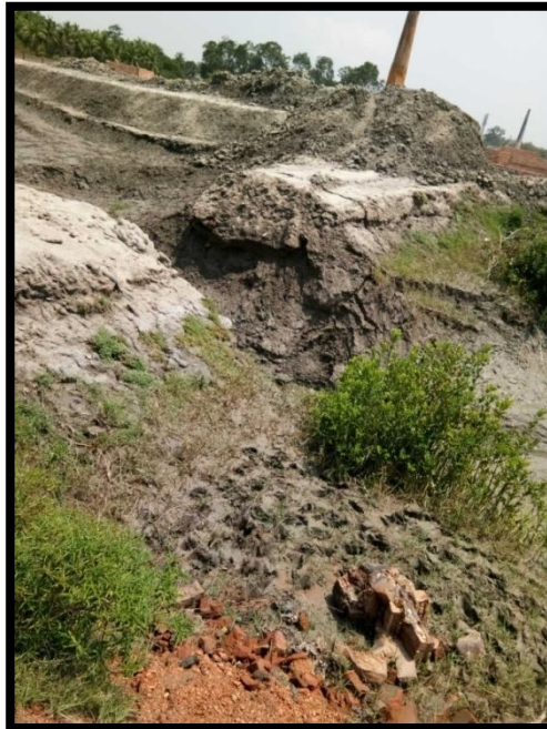
RIVER BANK BREAK AT CHAINAGE 4.5, LEFT BANK
