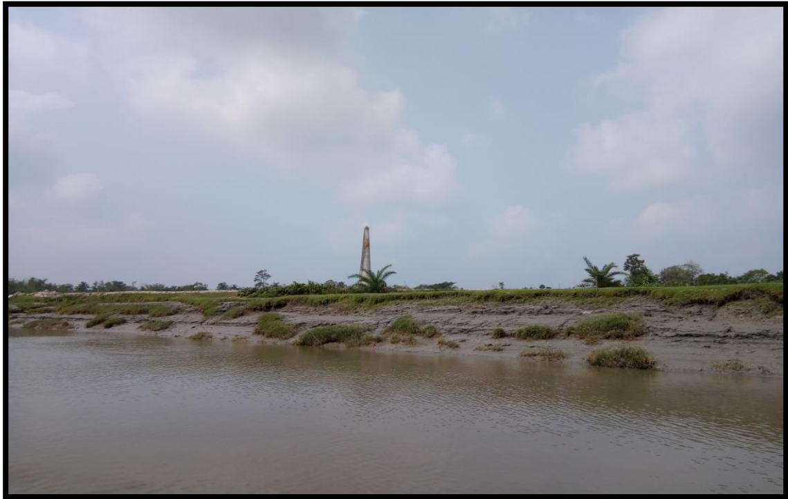
RIGHT BANK AT CHAINAGE 31.2
