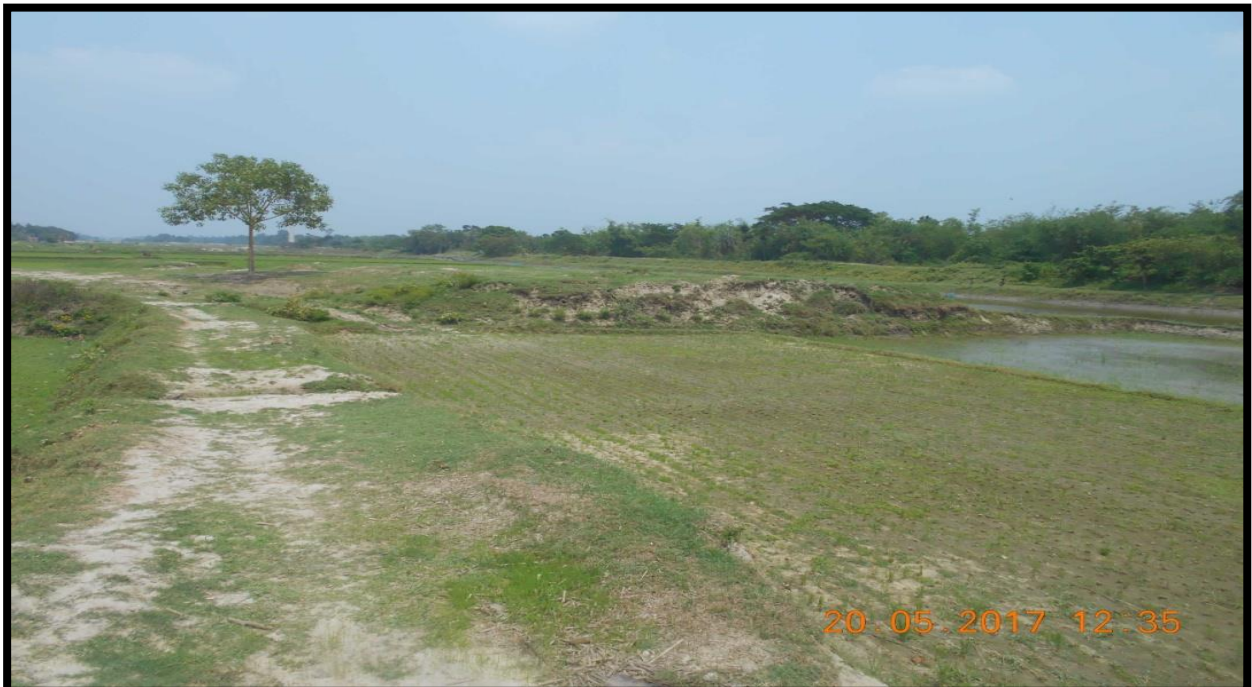
LEFT BANK AT CHAINAGE 59.7
