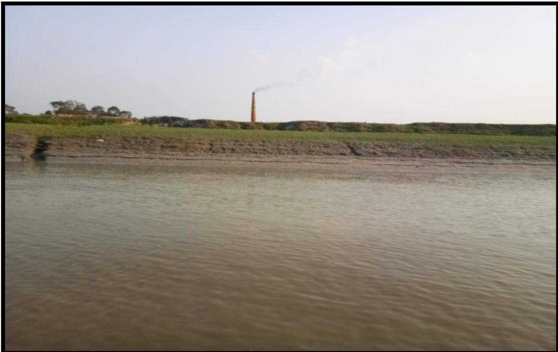
LEFT BANK AT CHAINAGE 17.1
