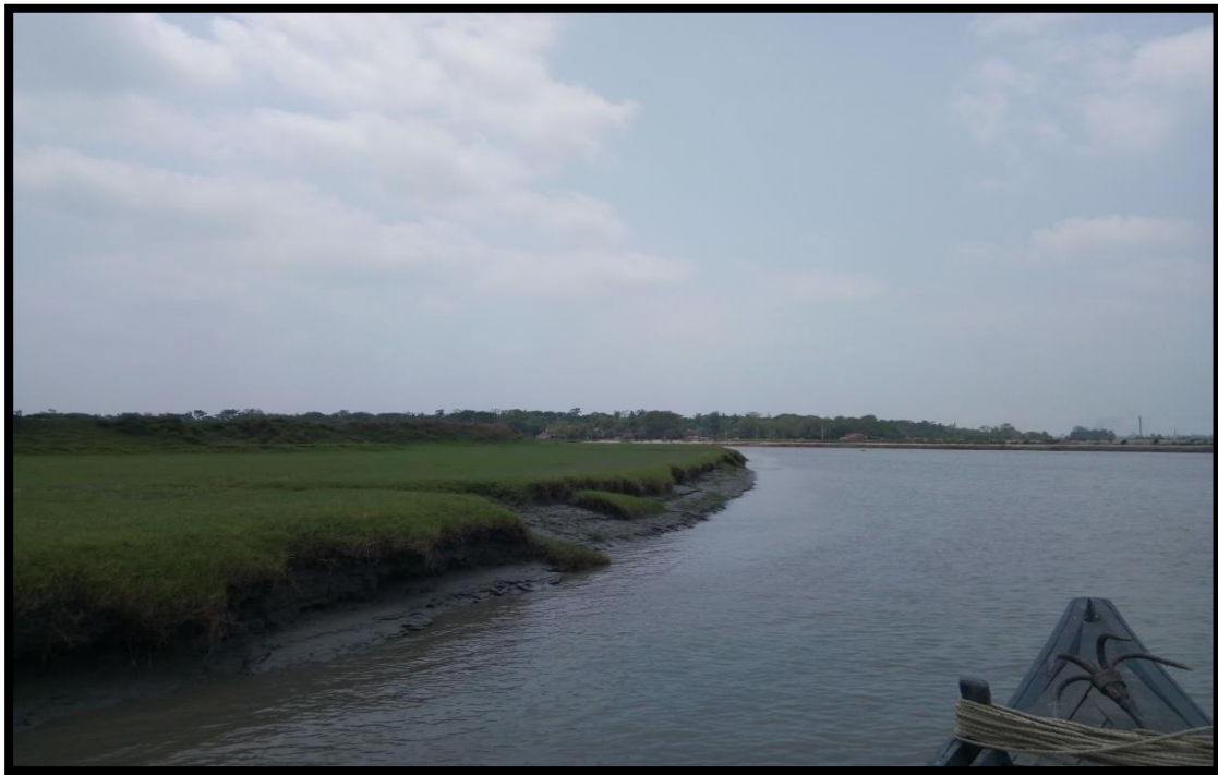
LEFT BANK AT CHAINAGE 26.7
