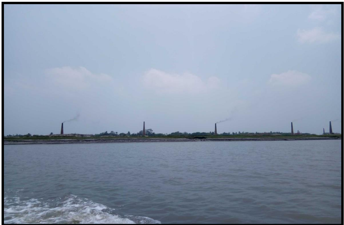
BRICK KILNS LEFT BANK AT CHAINAGE 21
