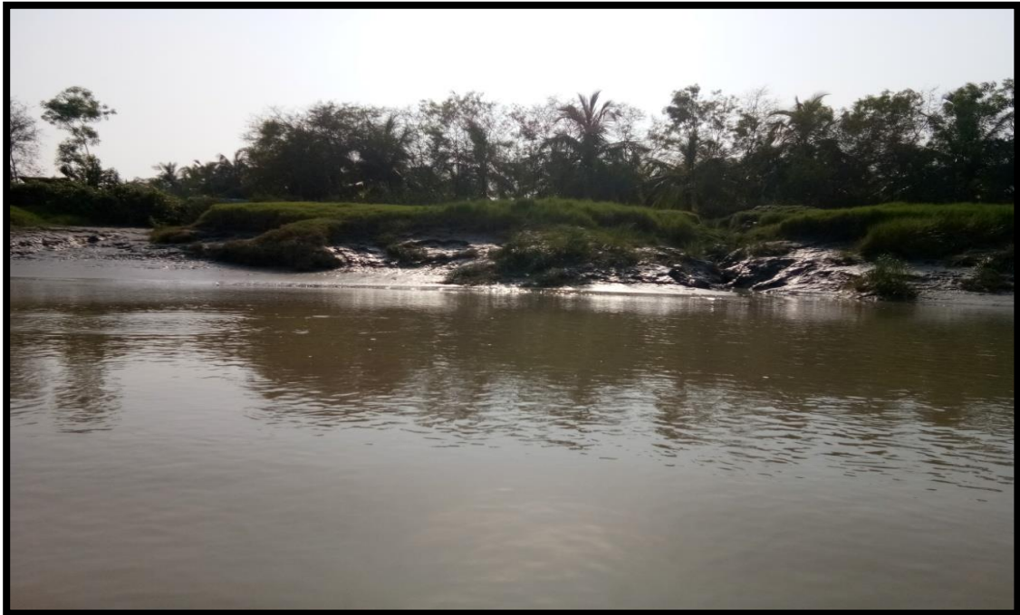
LEFT BANK AT CHAINAGE 14.4
