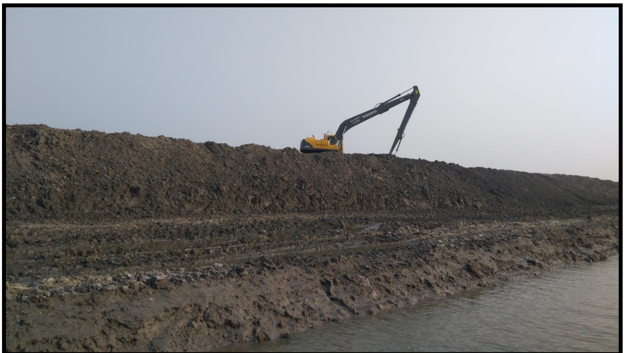
RIVER BANK CONSTRUCTION AT RIGHT BANK CHAINAGE 38
