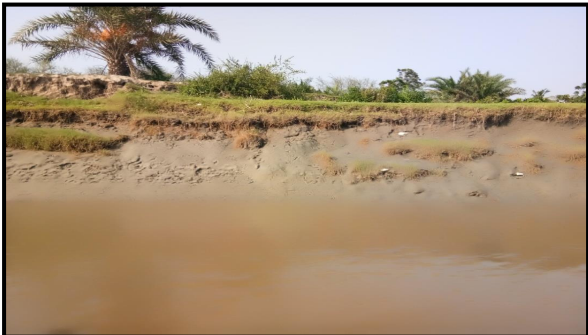
LEFT BANK AT CHAINAGE 14.8
