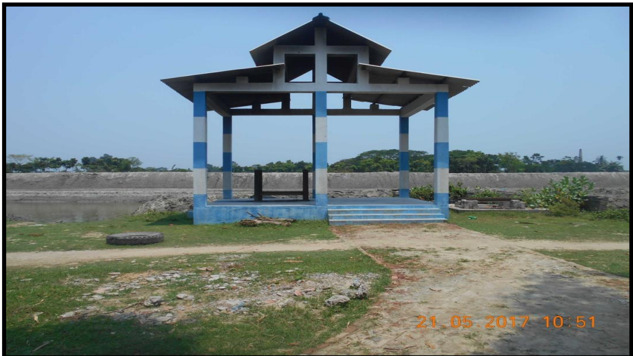
CEMETERY RIGHT BANK AT CHAINAGE 47.6
