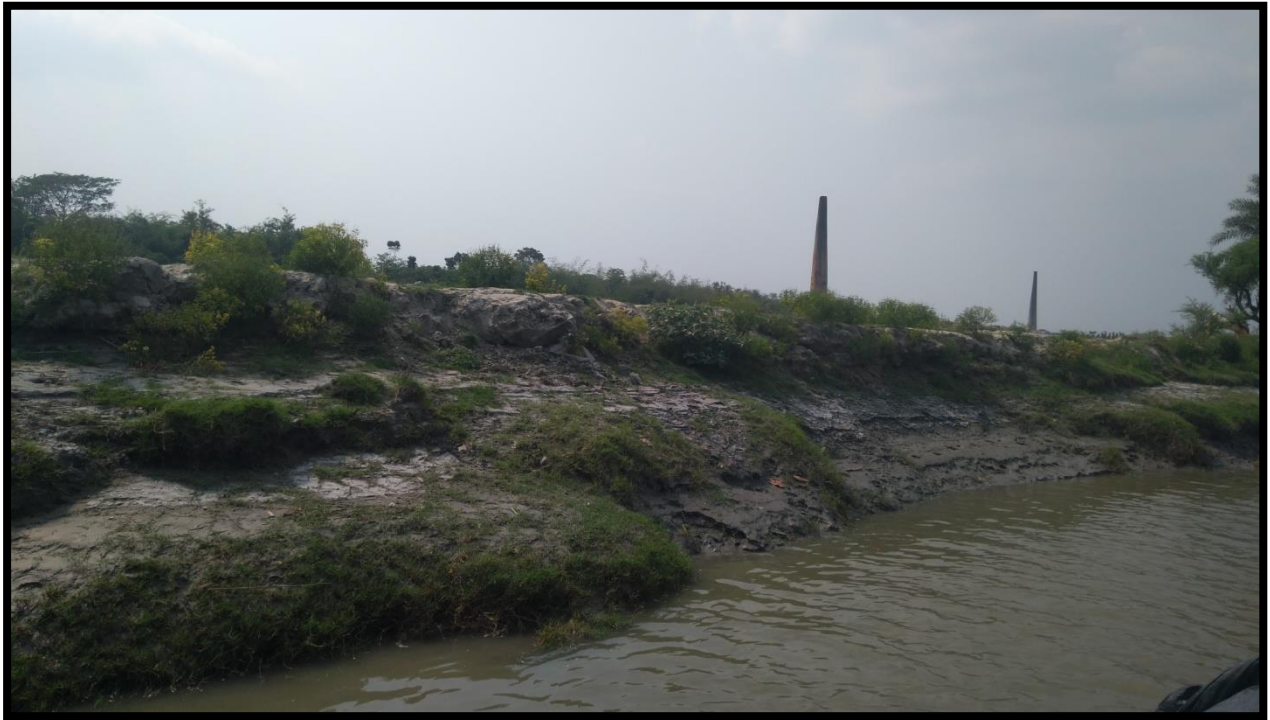
LEFT BANK AT CHAINAGE 33
