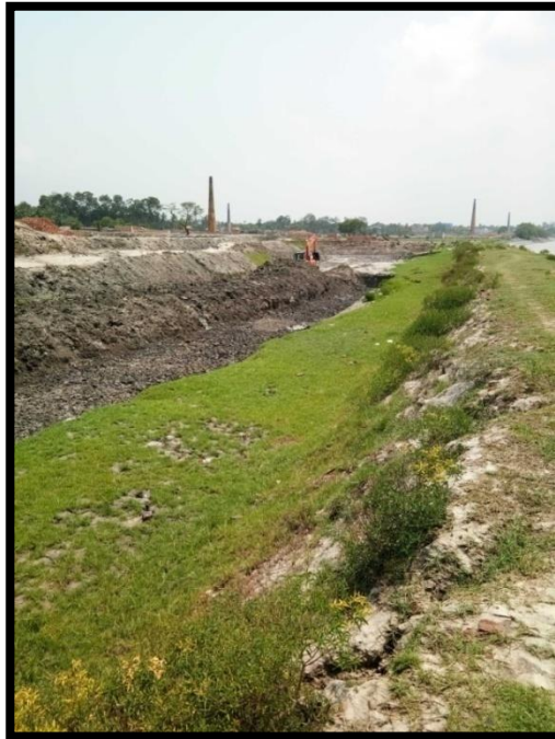
RIVER BANK AT CHAINAGE 4.5, LEFT BANK
