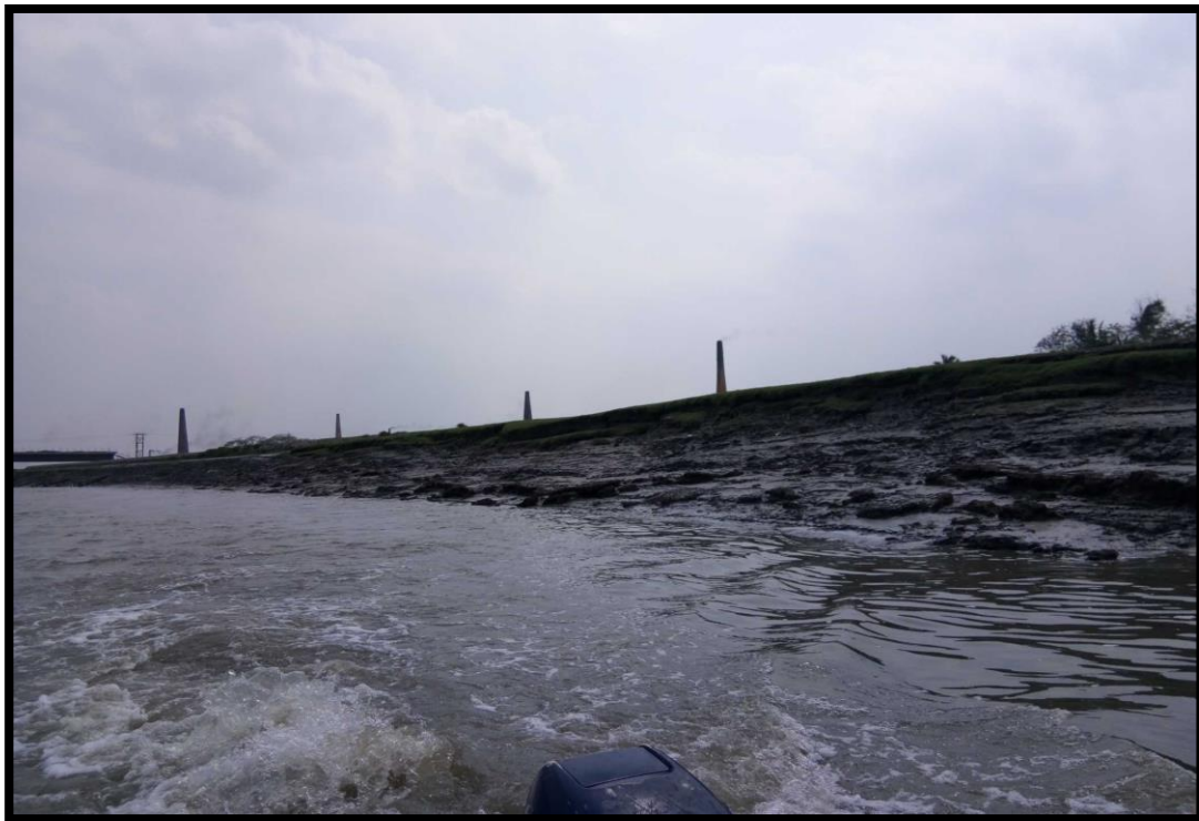
BRICK KLINS AT LEFT BANK CHAINAGE 21.9
