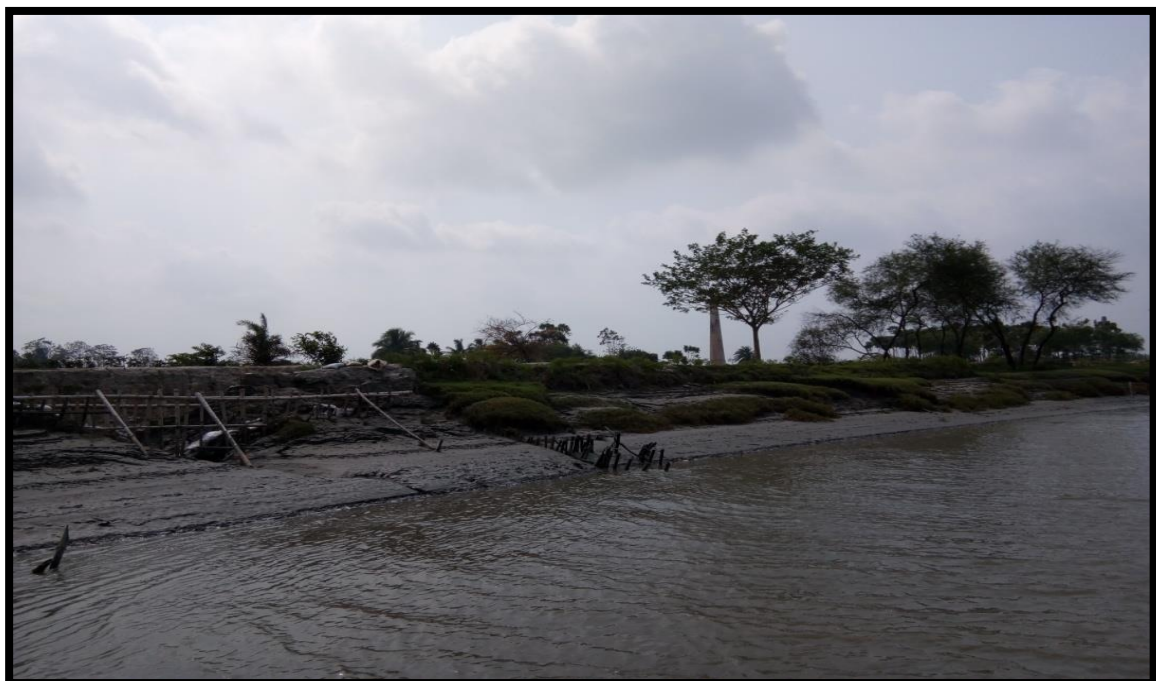
LEFT BANK AT CHAINAGE 30.2
