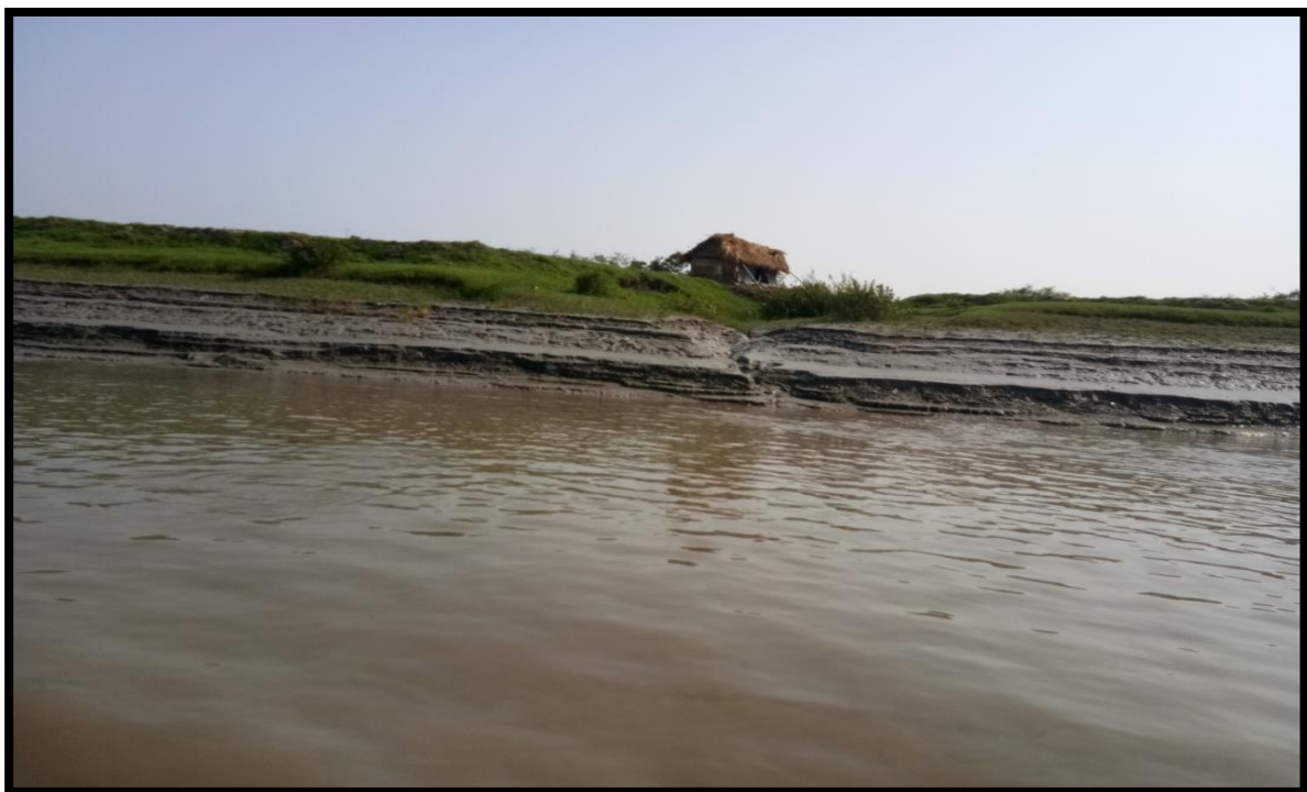
LEFT BANK AT CHAINAGE 13.2
