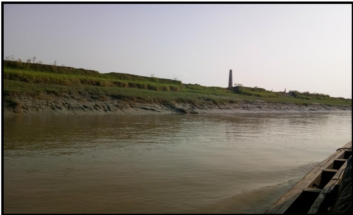
BRICK KLIN AT LEFT BANK CHAINAGE 15.2
