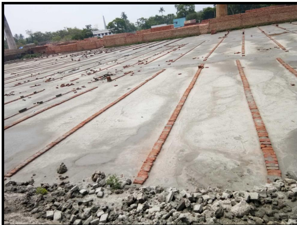
BRICK KLIN AT CHAINAGE 3.3, LEFT BANK
