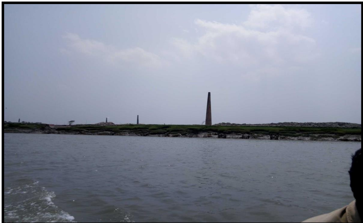
BRICK KILNS LEFT BANK AT CHAINAGE 21.6
