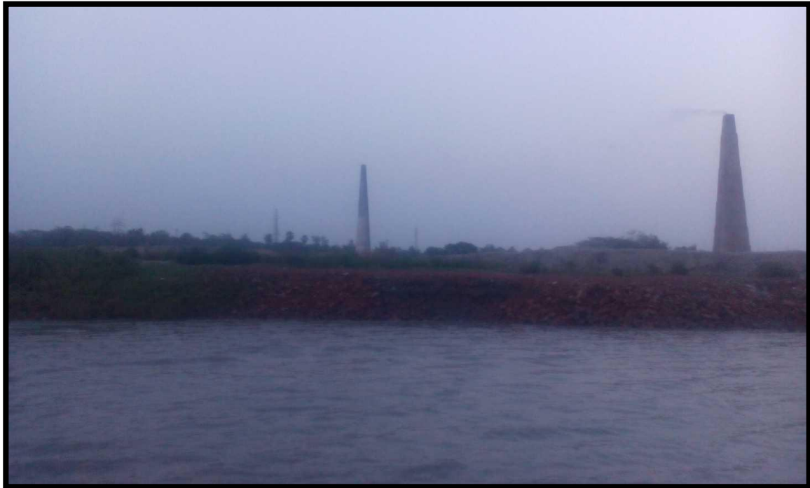
BRICK KLIN 10.3 CHAINAGE, RIGHT BANK
