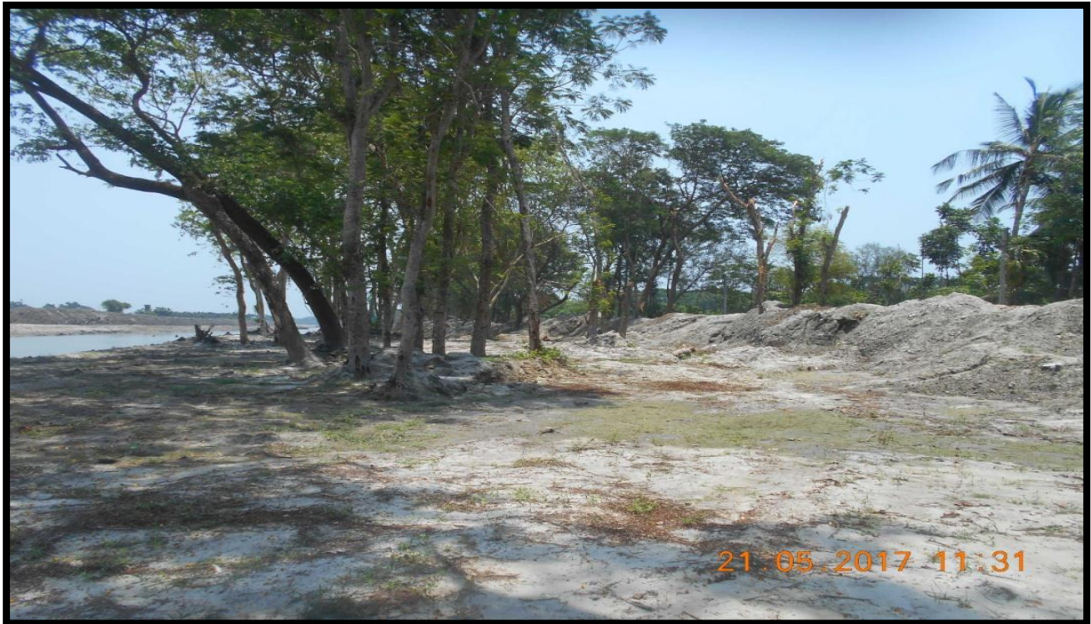
RIGHT BANK AT CHAINAGE 46.7
