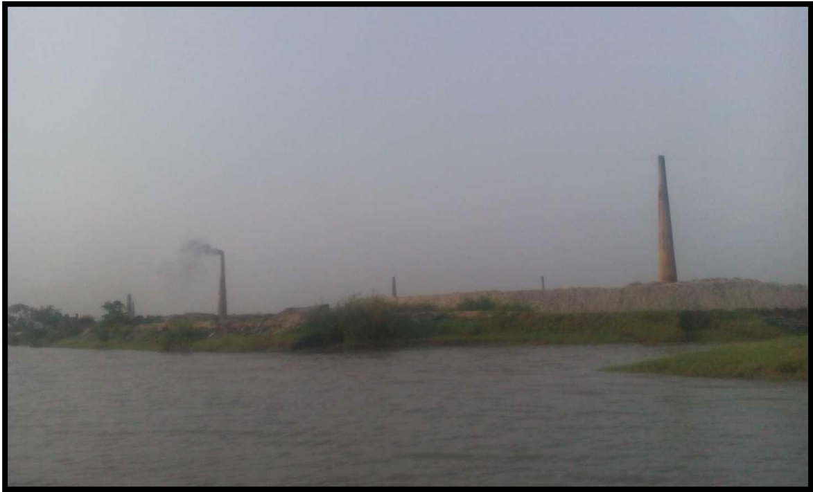
BRICK KLIN 9.5 CHAINAGE, RIGHT BANK
