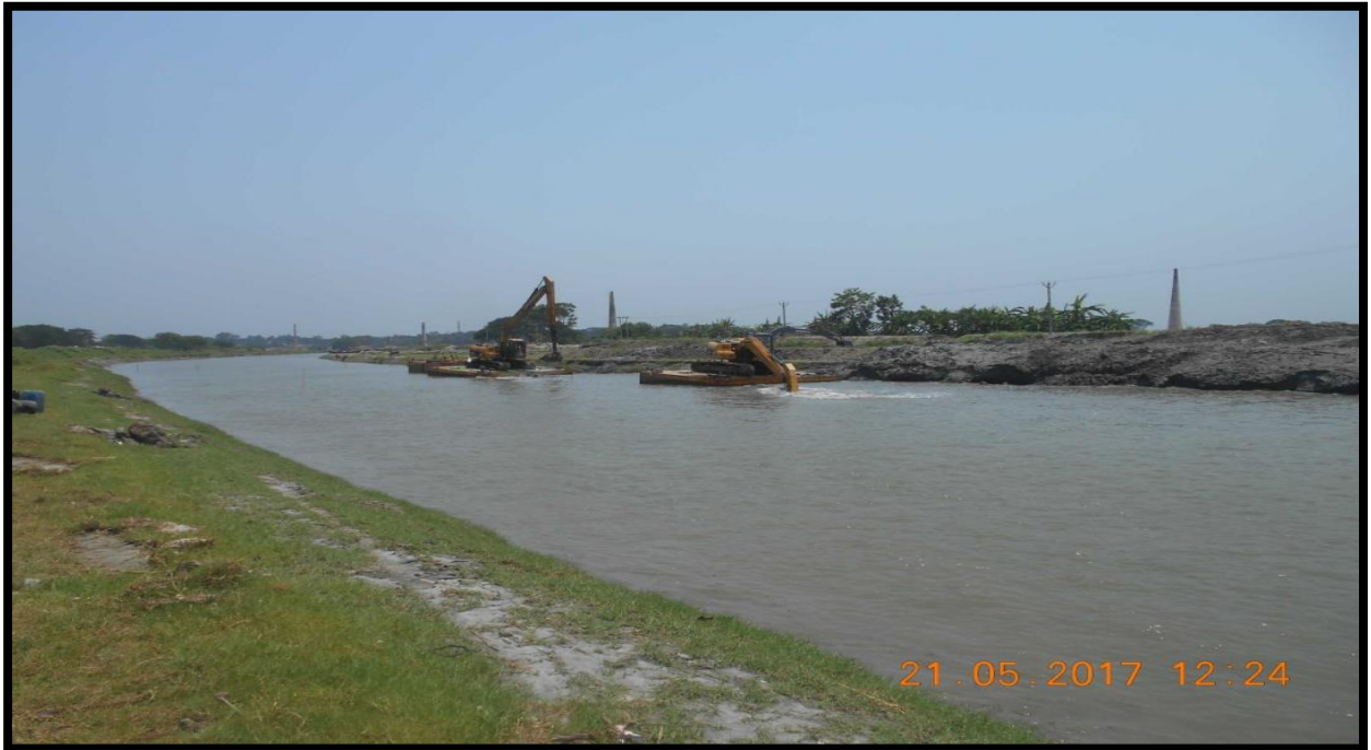
DREDGING AT LEFT BANK CHAINAGE 45
