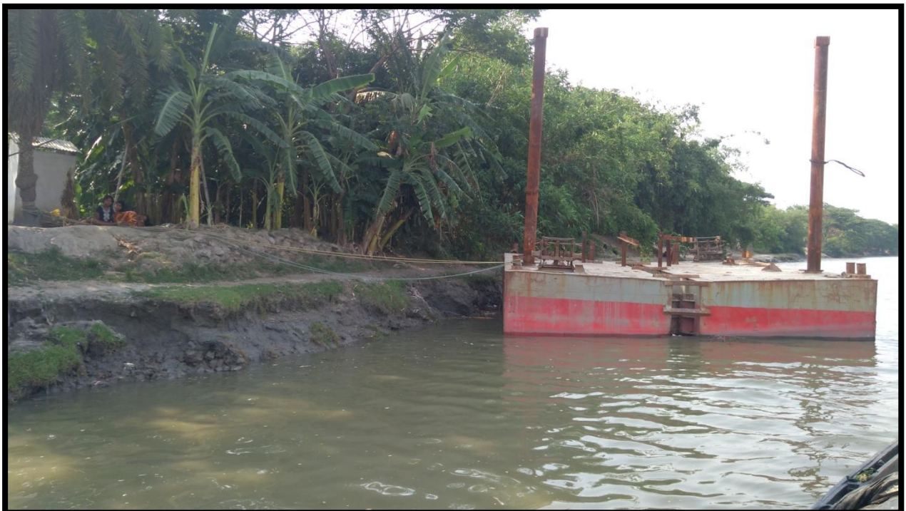
DREDGER AT LEFT BANK CHAINAGE 37.1
