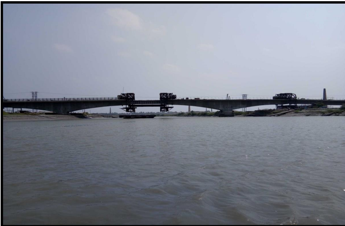
BRIDGE UNDER CONSTRUCTION AT CHAINAGE 21.8
