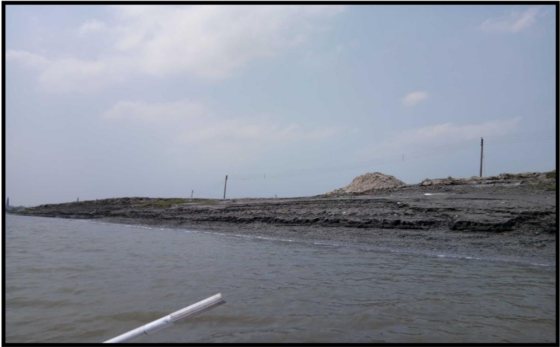
LEFT BANK AT CHAINAGE 21.1
