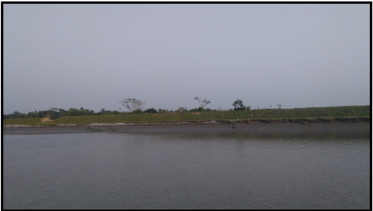
LEFT BANK AT CHAINAGE 34
