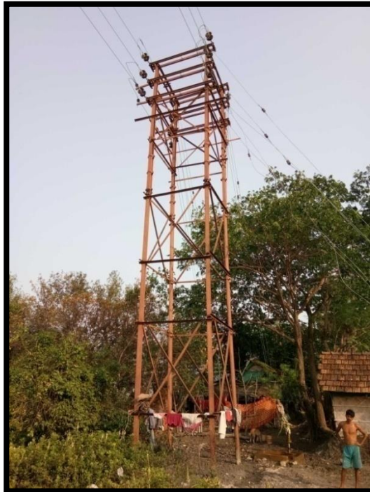
HIGH TENTION LINE AT CHAINAGE 7.4, LEFT BANK
