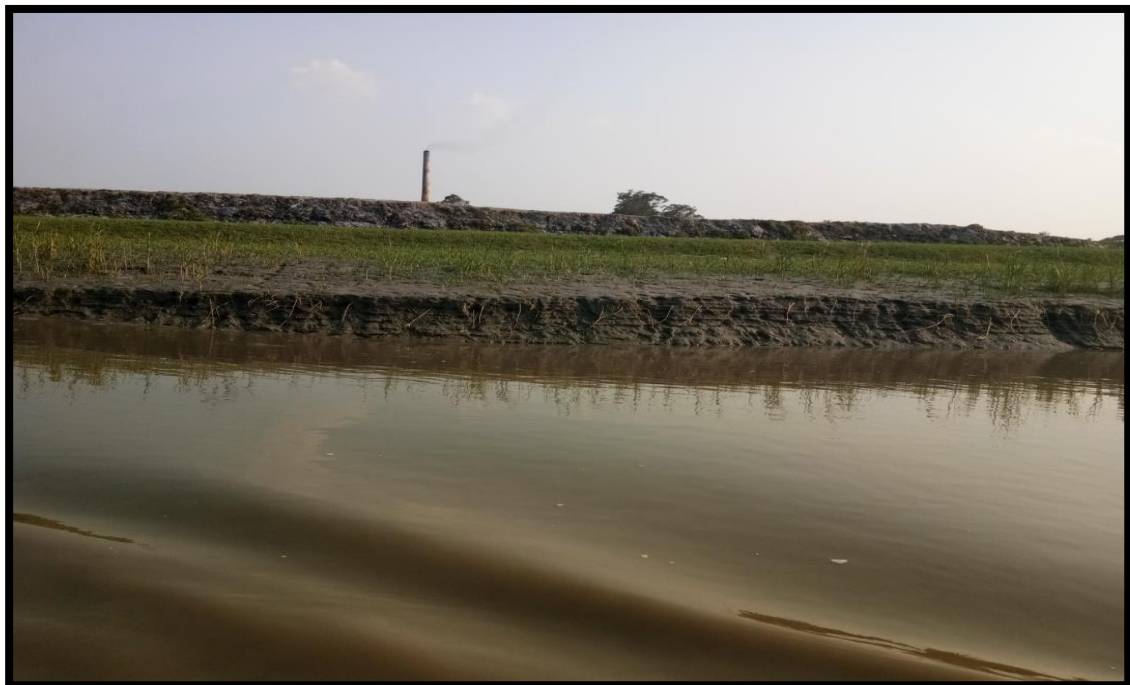
LEFT BANK AT CHAINAGE 17
