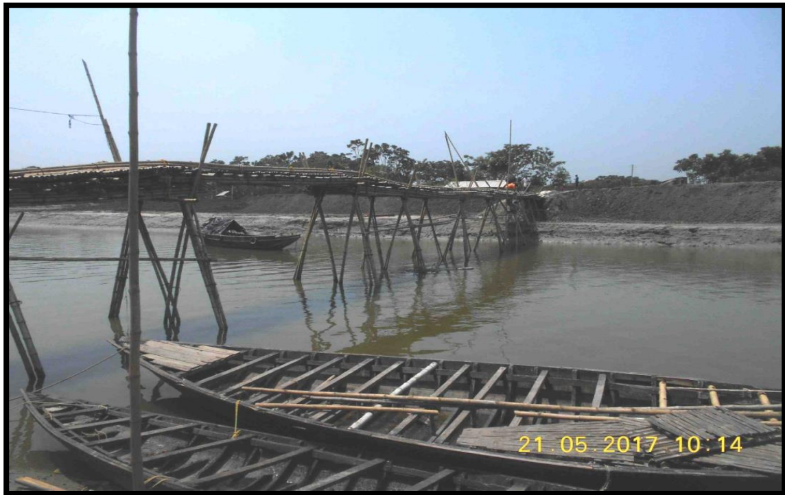
BAMBOO BRIDGE AT CHAINAGE 48.7
