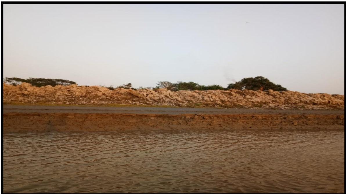
LEFT BANK AT CHAINAGE 19.8
