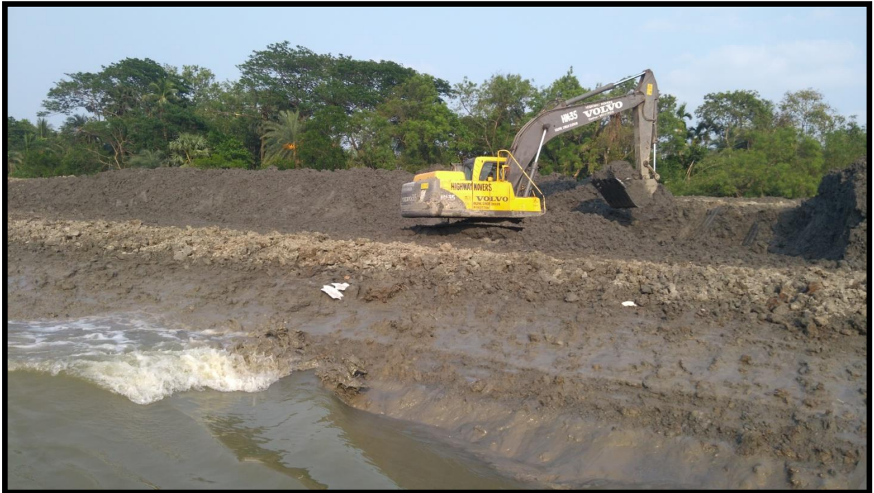
RIVER BANK CONSTRUCTION AT RIGHT BANK CHAINAGE 40.2
