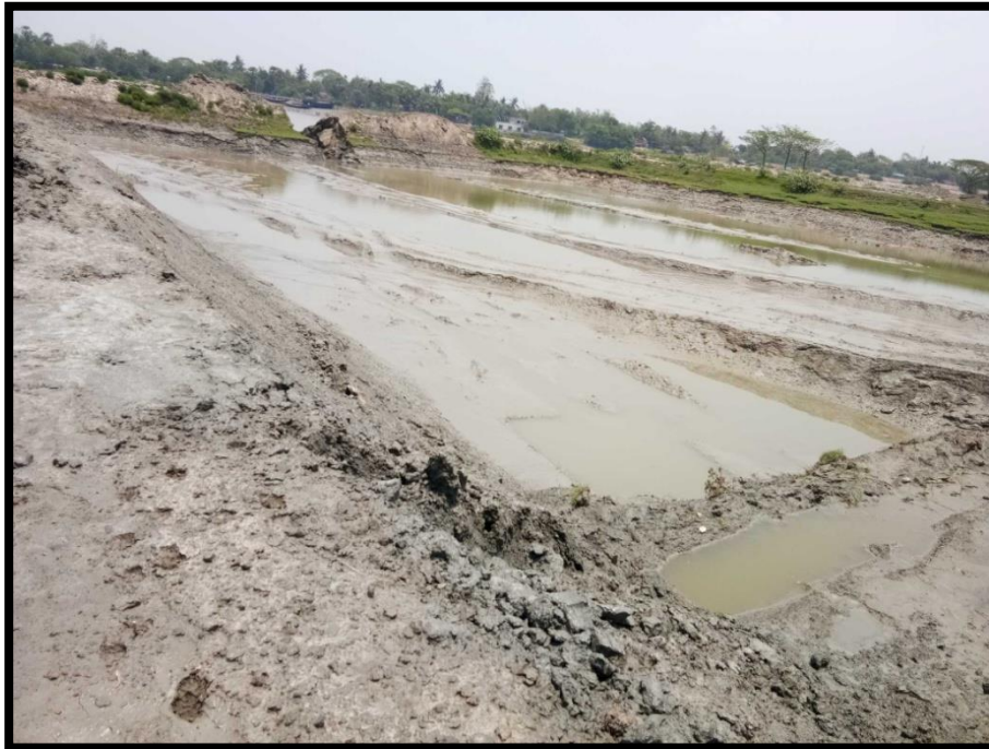
POND NEAR RIVER BANK AT CHAINAGE 3.5, LEFT BANK
