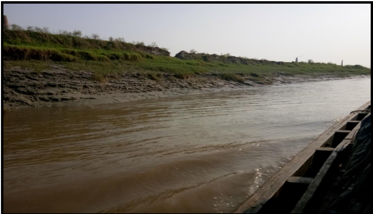
LEFT BANK AT CHAINAGE 15.6
