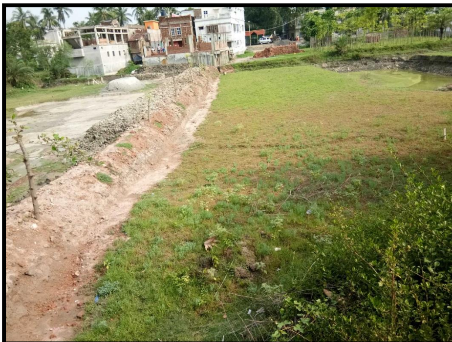
RIVER BANK AT CHAINAGE 6.3, LEFT BANK
