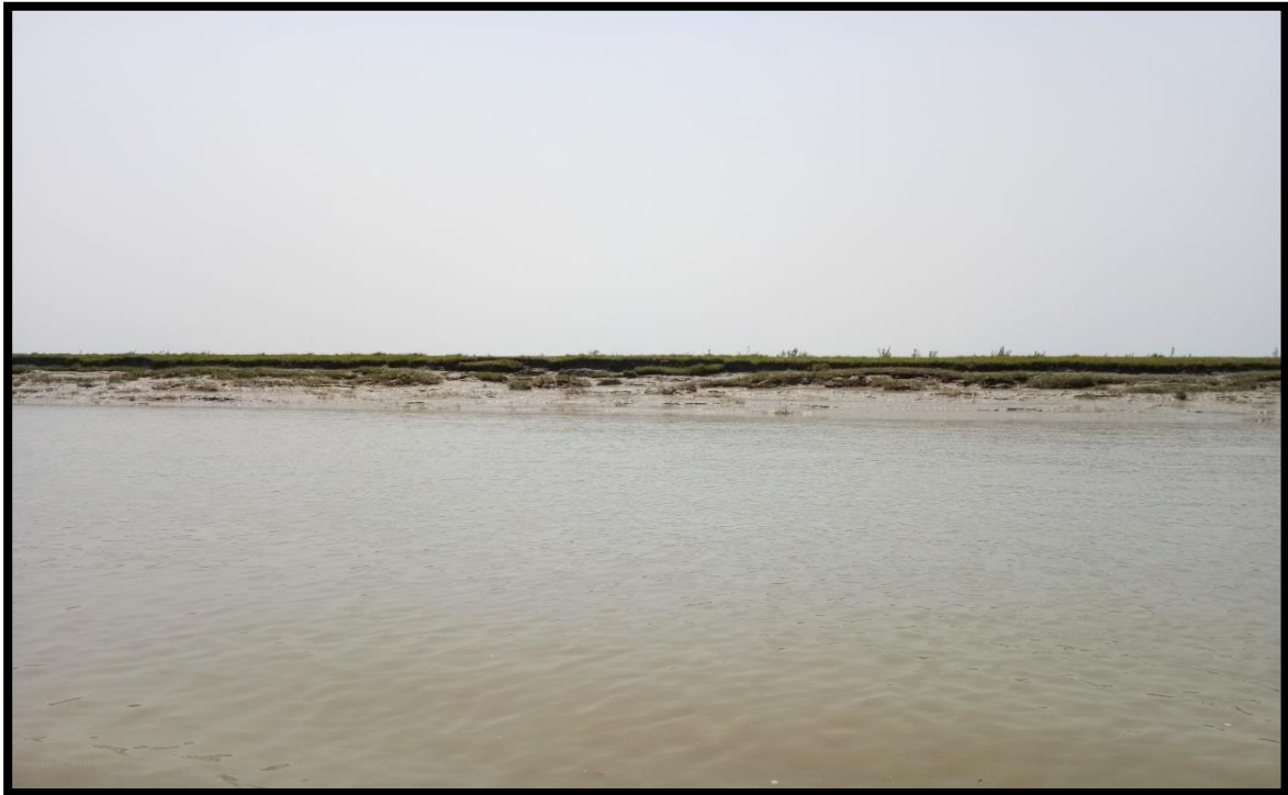
LEFT BANK AT CHAINAGE 13
