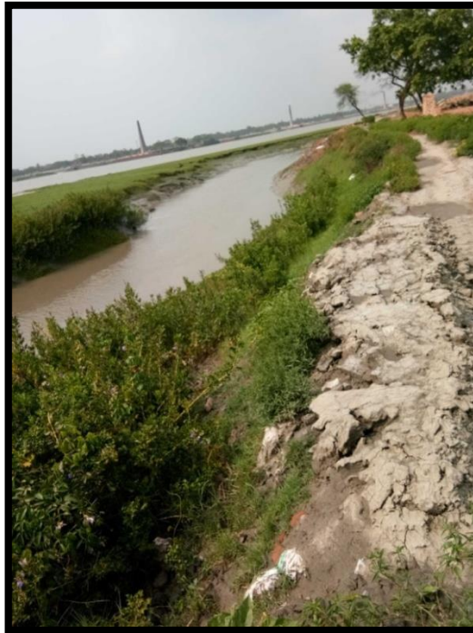
RIVER BANK AT CHAINAGE 4.7, LEFT BANK
