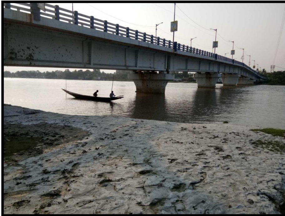
ICHAMATI BRIDGE AT CHAINAGE 7.4, LEFT BANK
