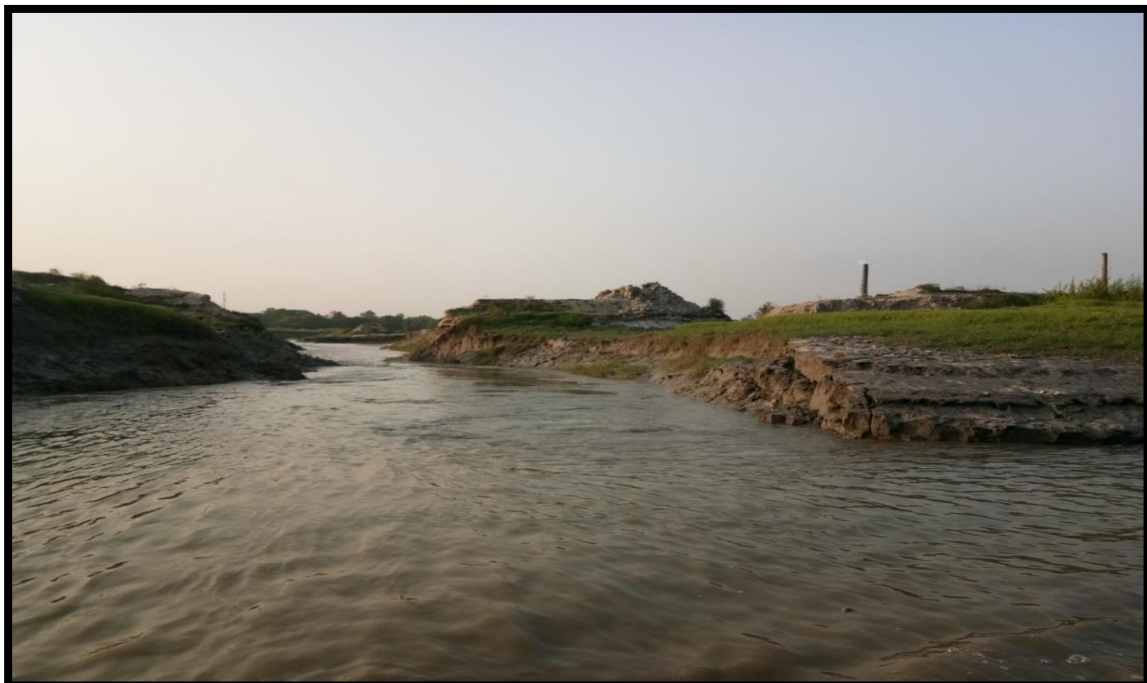
RIGHT BANK AT CHAINAGE 18.3
