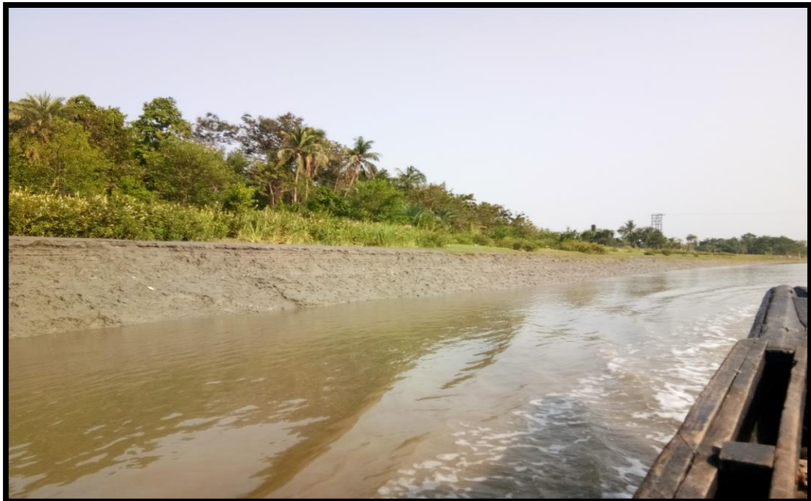
RIGHT BANK AT CHAINAGE 14.5
