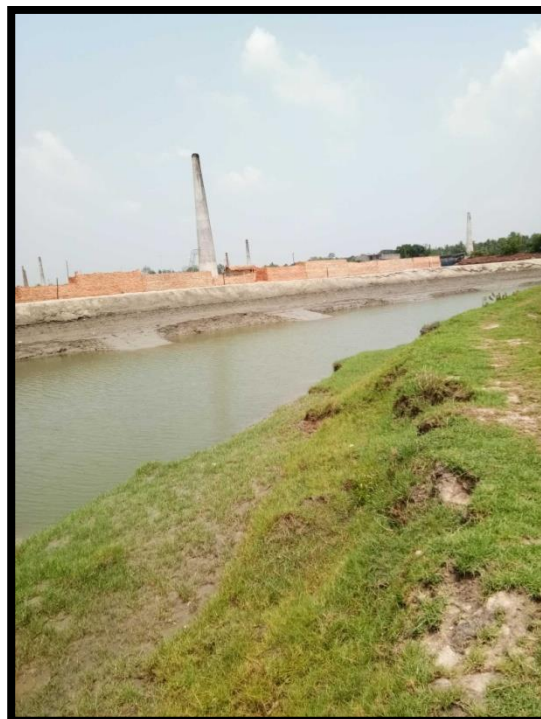
POND AT CHAINAGE 4.4, LEFT BANK
