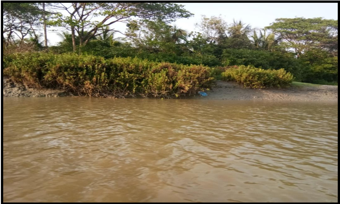
RIGHT BANK AT CHAINAGE 16.7
