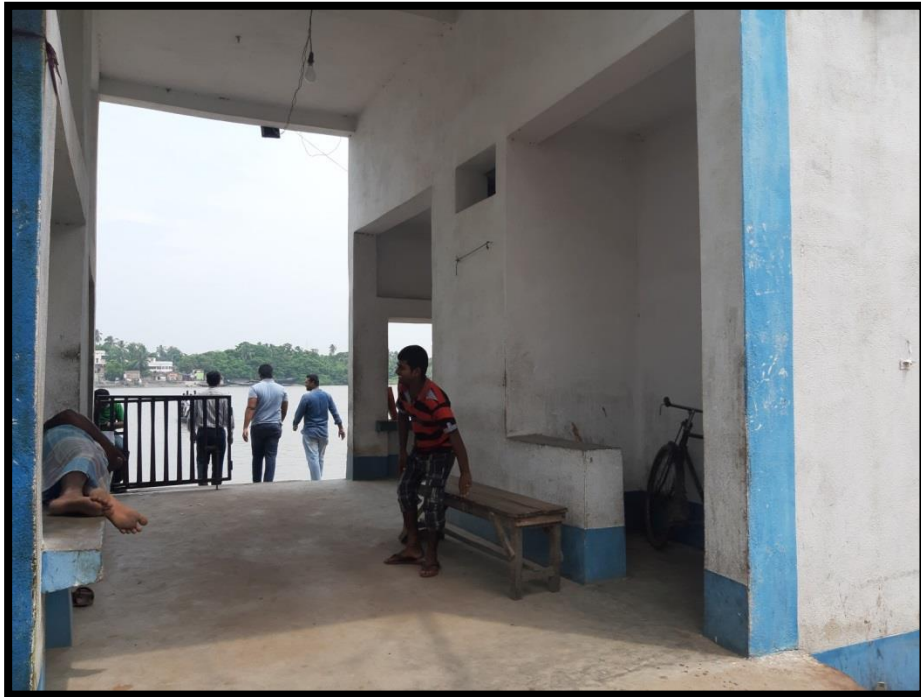
Existing building for passengers at Basirhat ferry Ghat (Pic 1)
