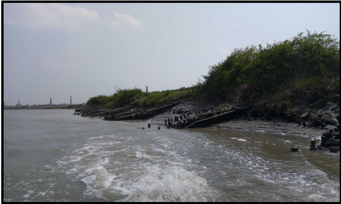
TEMPORARY RIVER BANK PROTECTION AT LEFT BANK CHAINAGE 21.7
