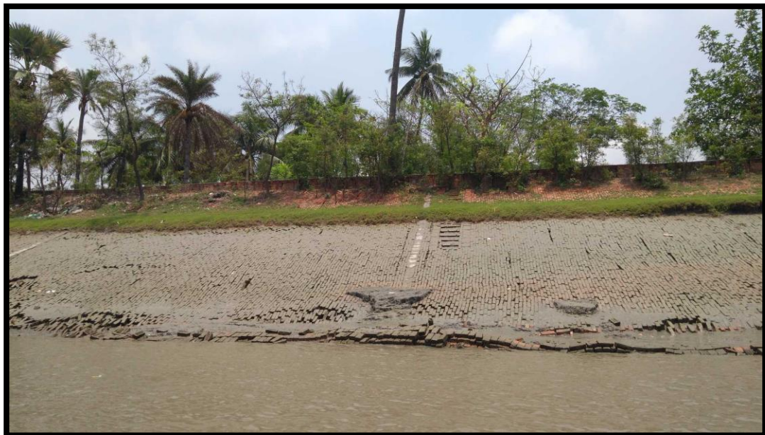
BANK PROTECTION, 1.2 CHAINAGE, RIGHT BANK
