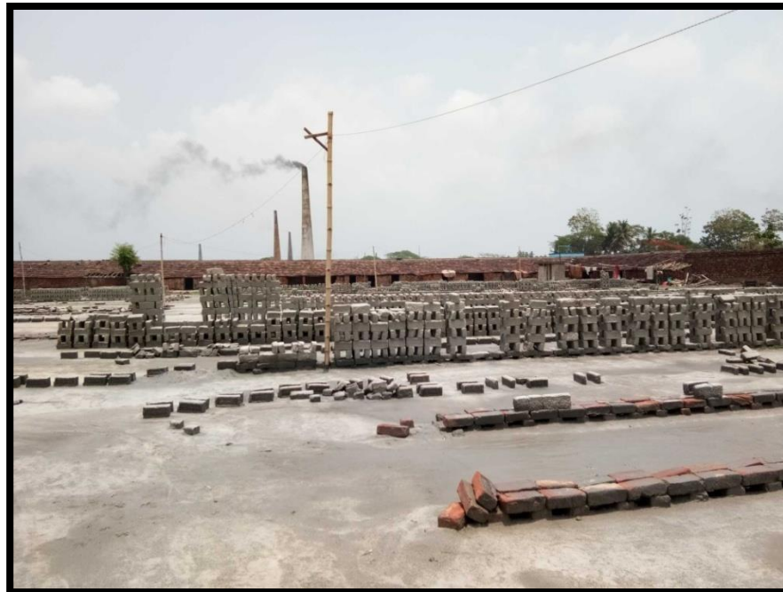
BRICK KLIN AT CHAINAGE 4, LEFT BANK
