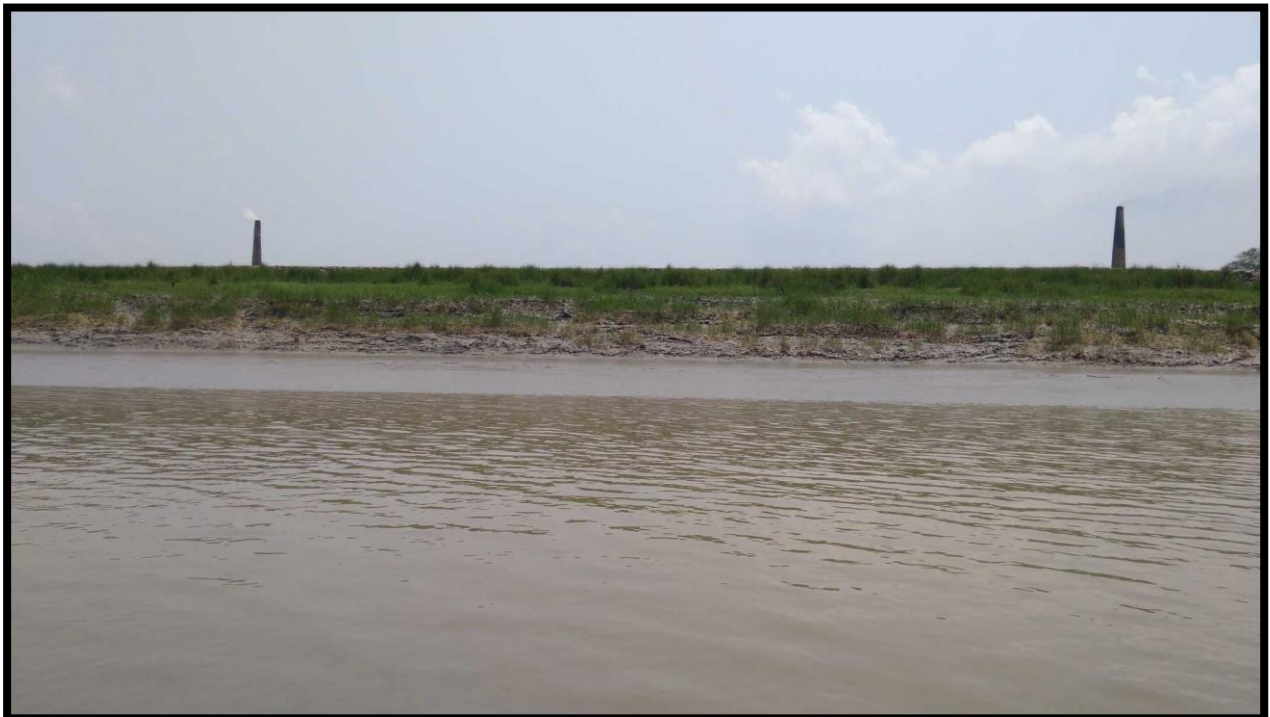
BRICK KLIN, 2.0 CHAINAGE, LEFT BANK
