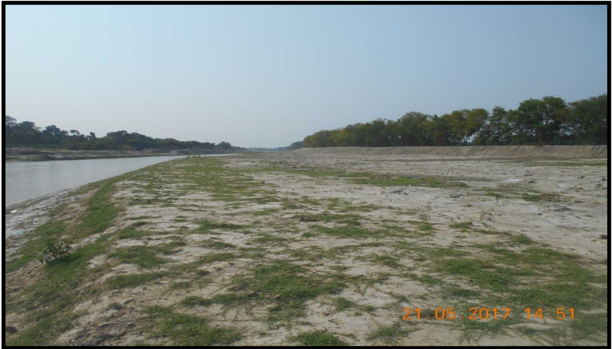
RIGHT BANK AT CHAINAGE 49.7
