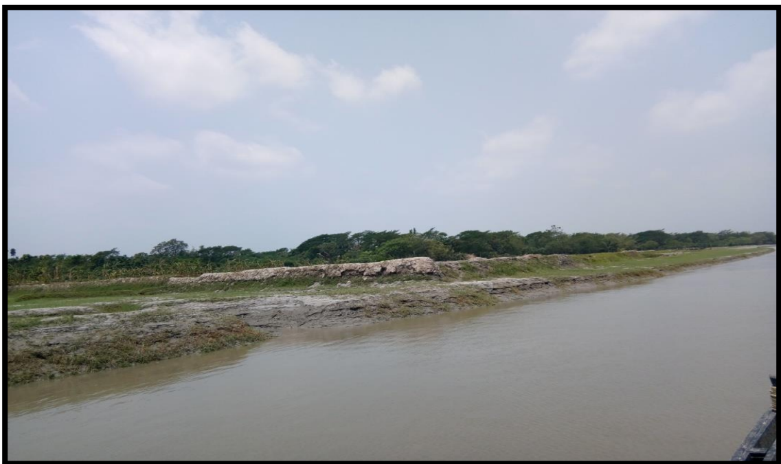
LEFT BANK AT CHAINAGE 27.5
