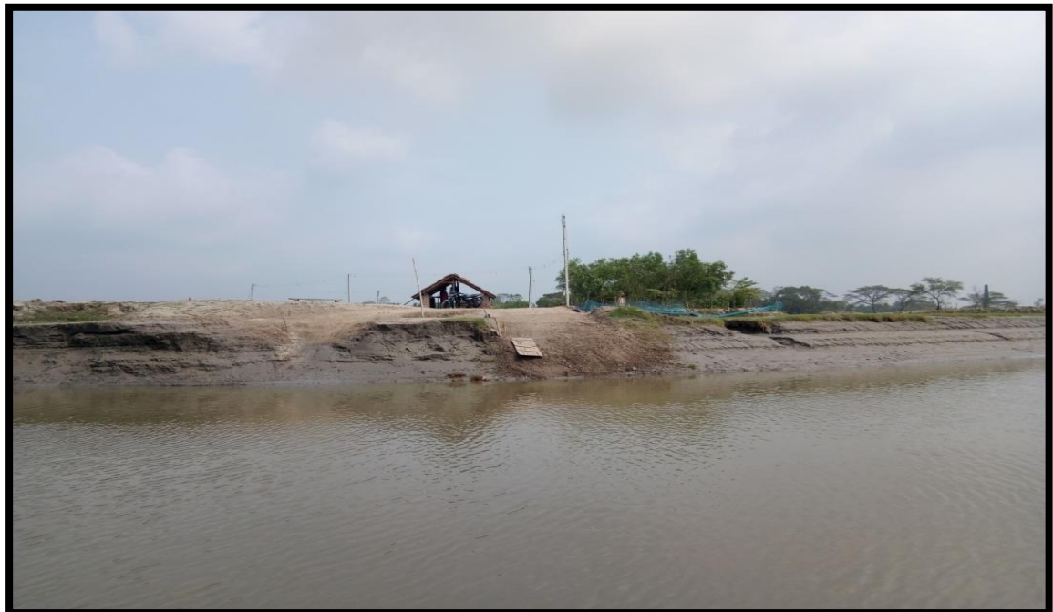
LEFT BANK AT CHAINAGE 28.6
