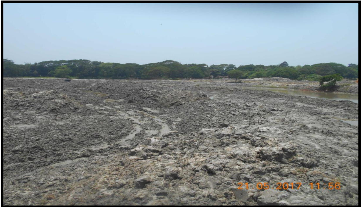
DREDGING AT RIGHT BANK CHAINAGE 46.1
