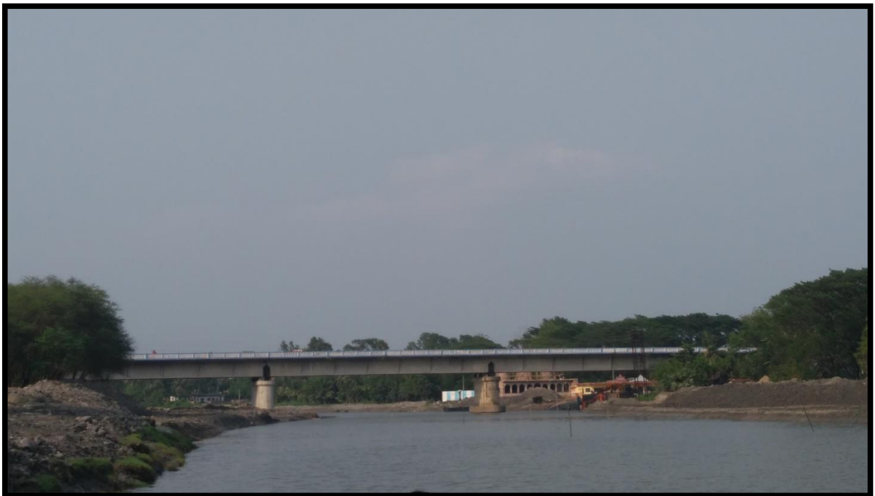
RIGHT BANK AT CHAINAGE 40.1
