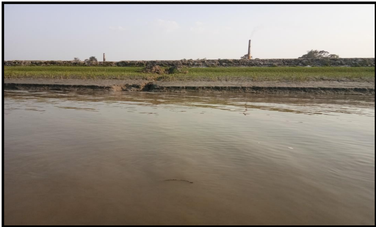
LEFT BANK AT CHAINAGE 16.7
