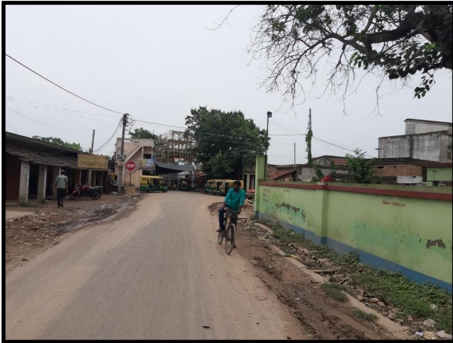
Existing road connecting to Basirhat ferry Ghat
