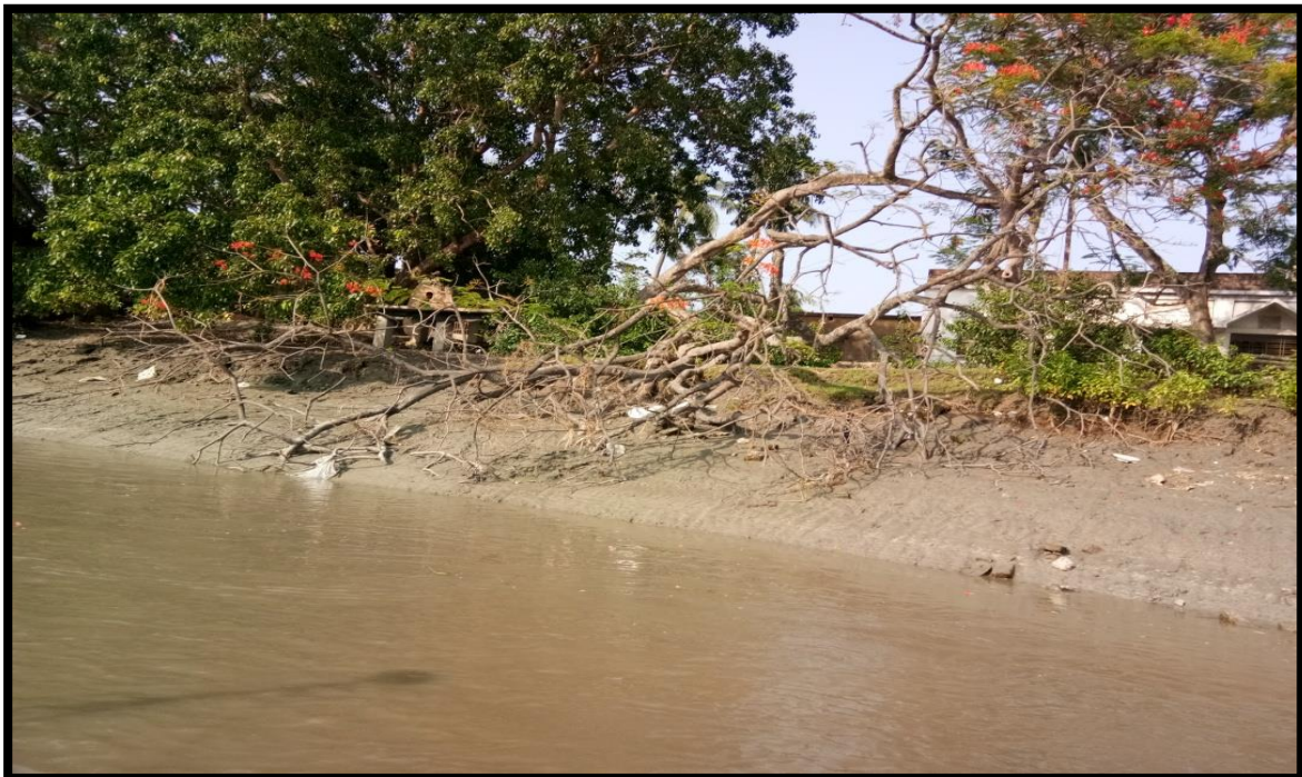
RIGHT BANK AT CHAINAGE 14.5
