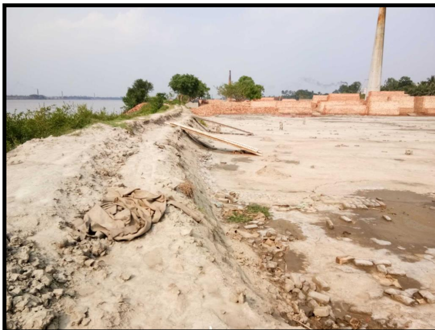
BRICK KLIN AT CHAINAGE 4.9, LEFT BANK
