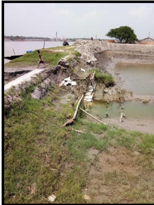
POND AT CHAINAGE 4.4, LEFT BANK
