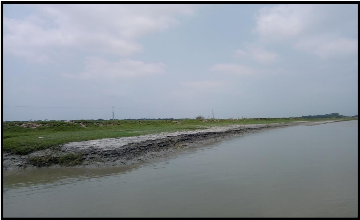
LEFT BANK AT CHAINAGE 26
