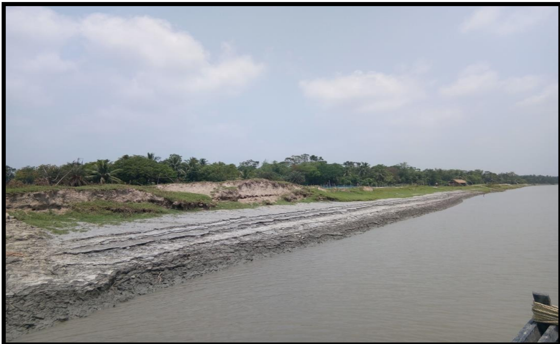
LEFT BANK AT CHAINAGE 23
