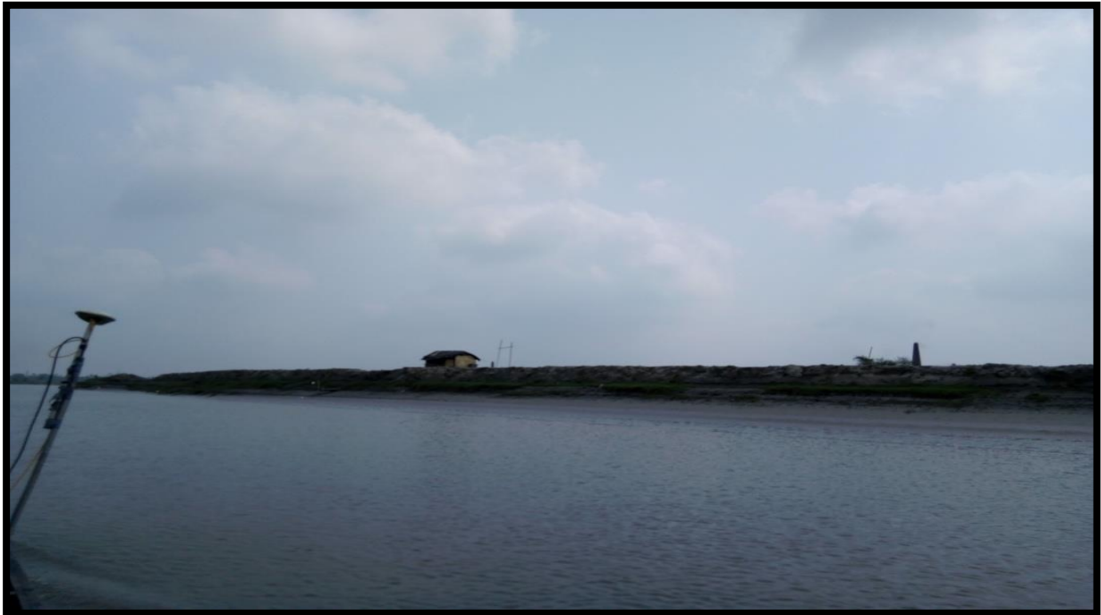
LEFT BANK AT CHAINAGE 31.7
