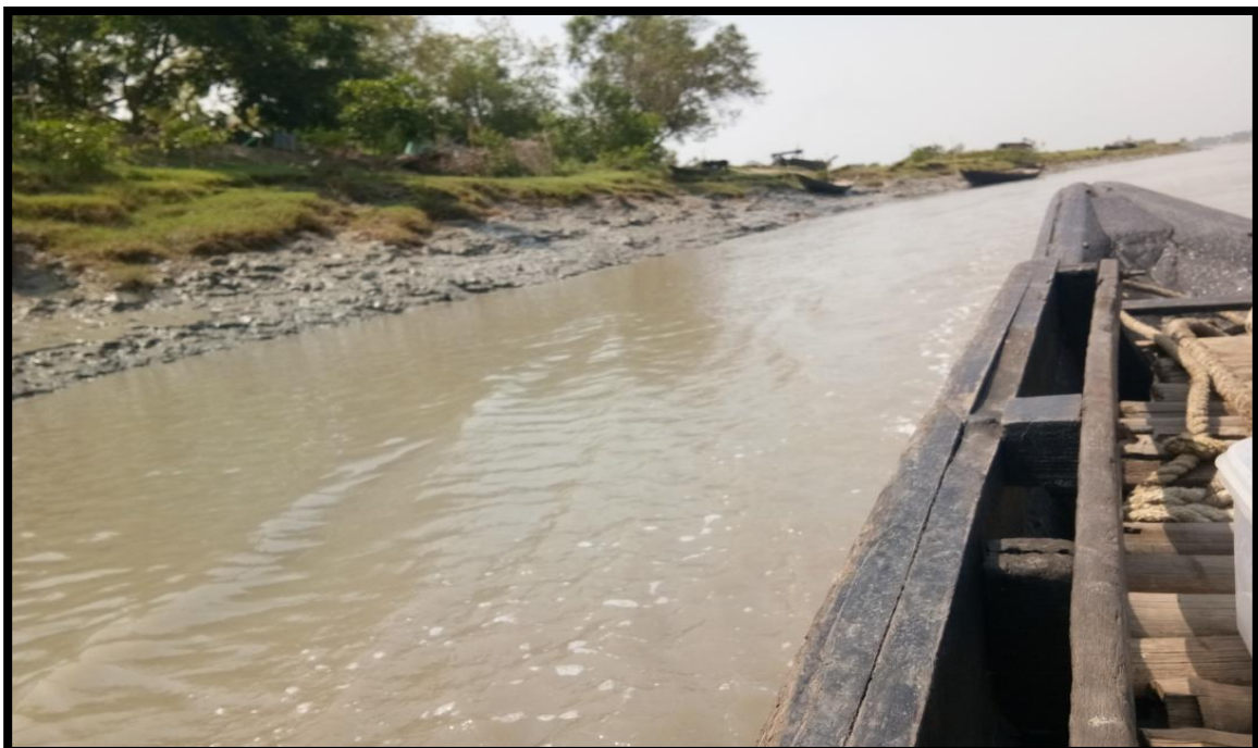
RIGHT BANK AT CHAINAGE 11
