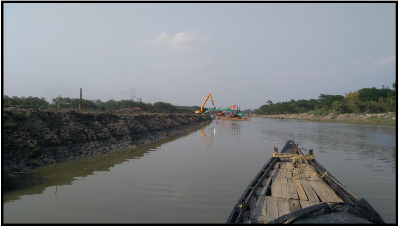
LEFT BANK AT CHAINAGE 30.3
