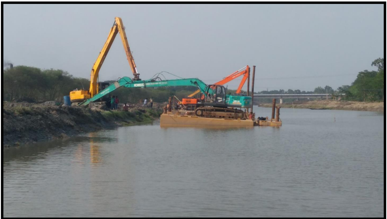
DREDGING AT LEFT BANK CHAINAGE 30
