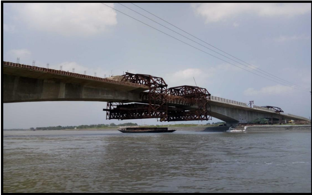
BRIDGE UNDER CONSTRUCTION AT CHAINAGE 21.8
