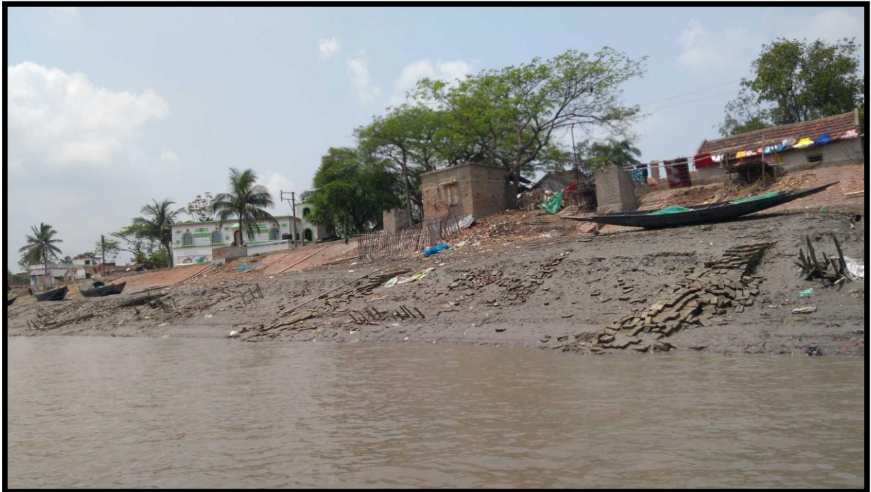
RIVER BANK PROTECTION, 2.0 CHAINAGE, RIGHT BANK
