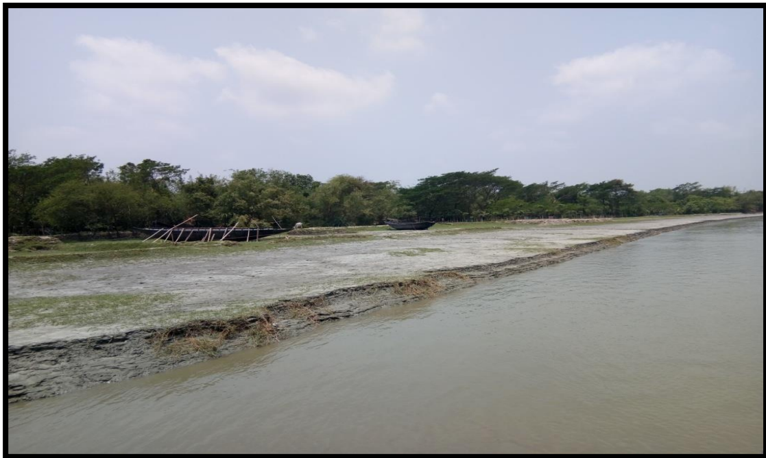
LEFT BANK AT CHAINAGE 27.3
