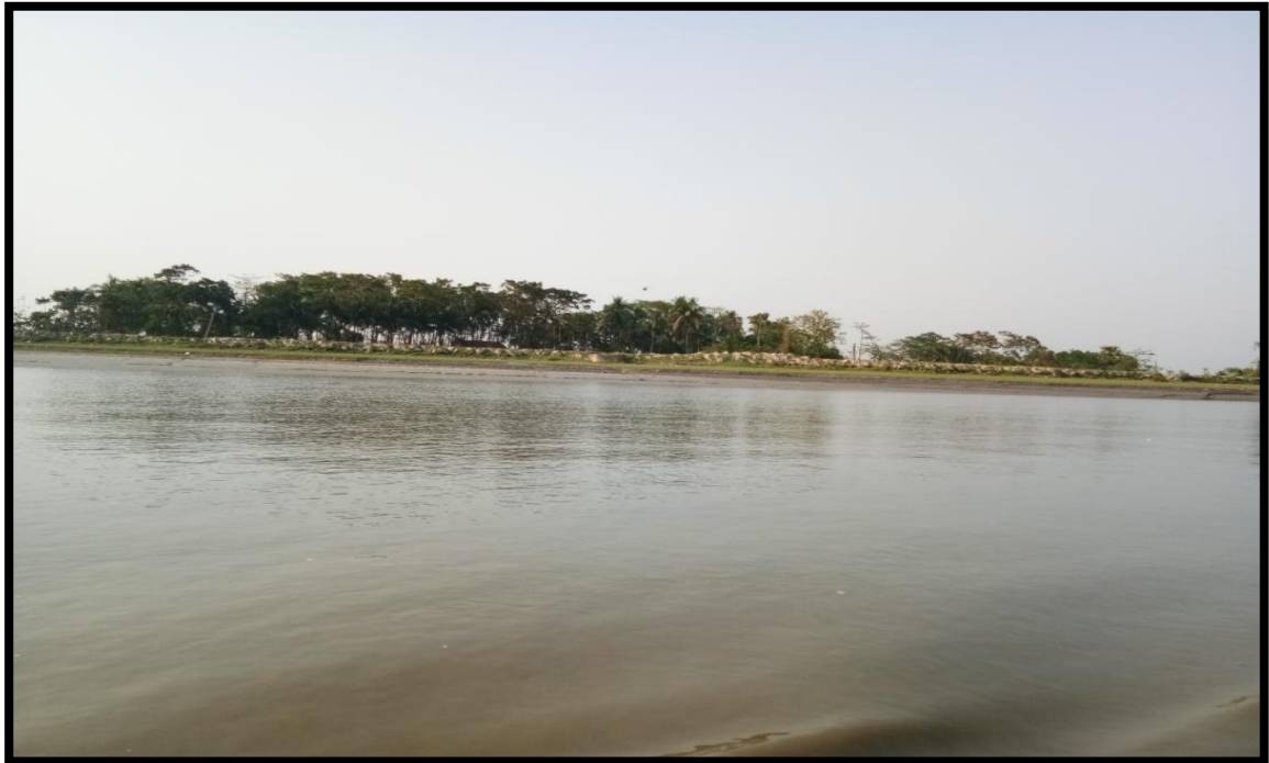
RIGHT BANK AT CHAINAGE 16.
