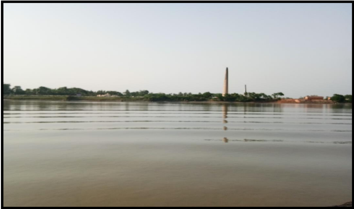
BRICK KLIN AT RIGHT BANK CHAINAGE 15.2
