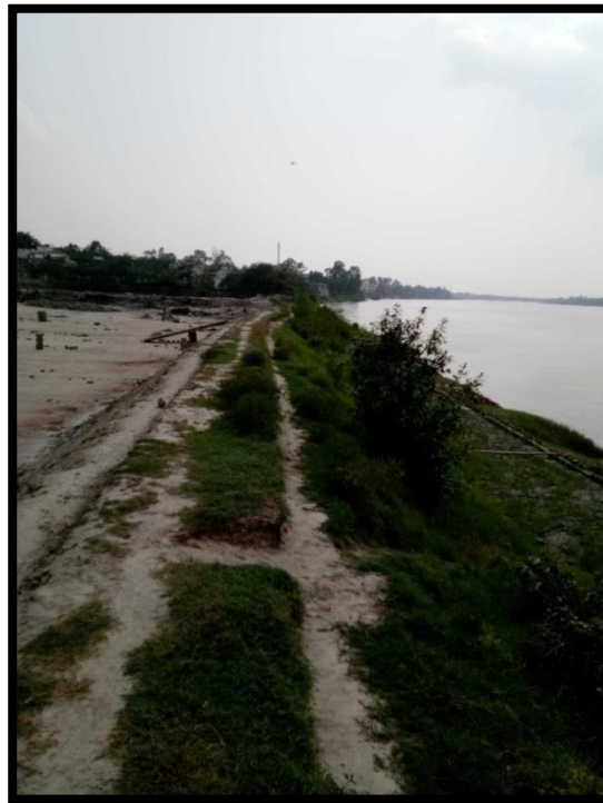
RIVER BANK AT CHAINAGE 4.8, LEFT BANK
