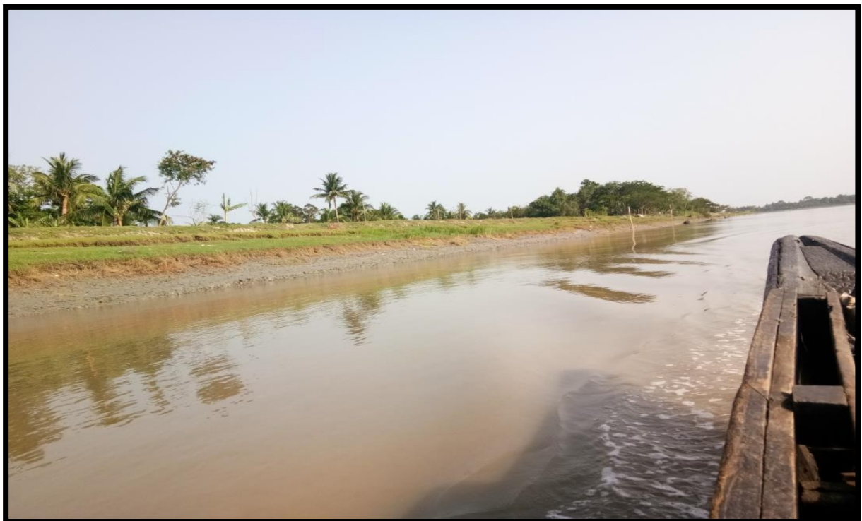
RIGHT BANK AT CHAINAGE 14.4
