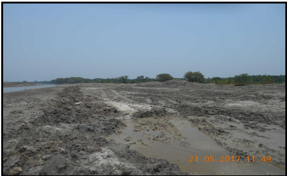
DREDGING AT RIGHT BANK CHAINAGE 46
