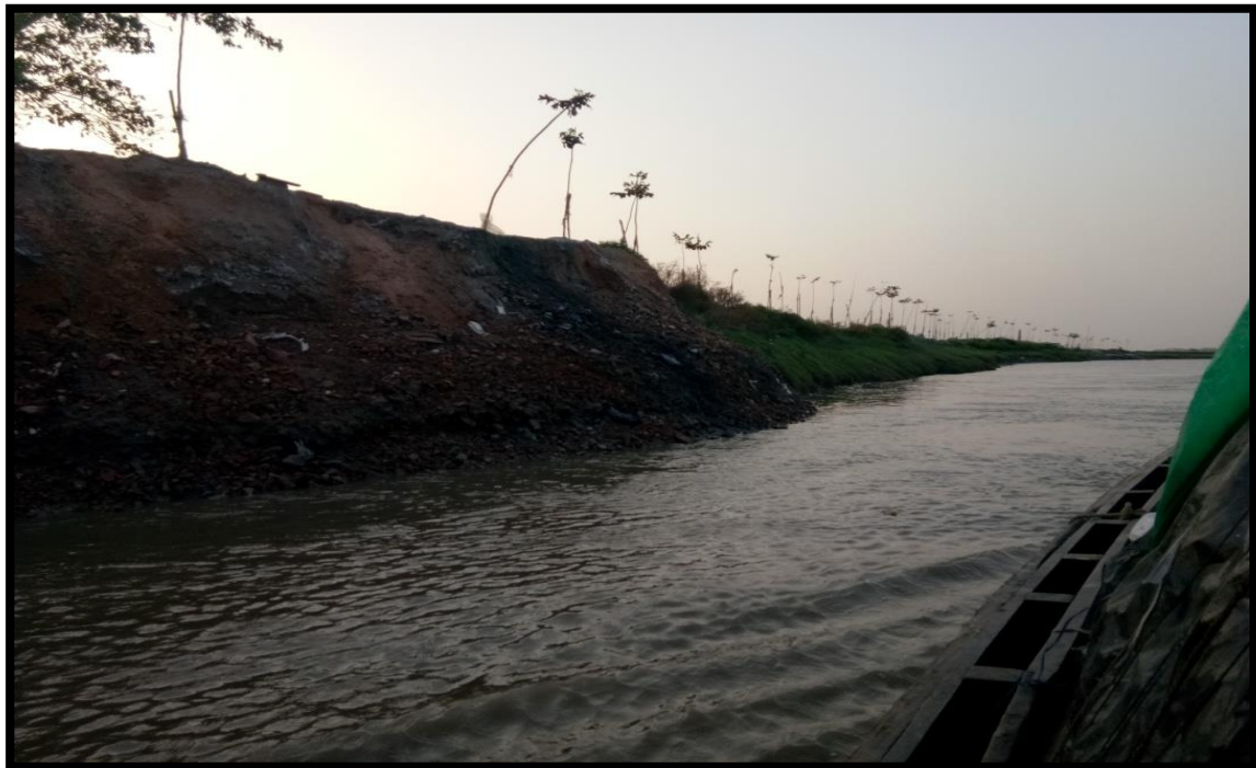
LEFT BANK AT CHAINAGE 19.4
