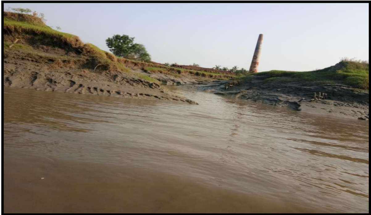
BRICK KLIN AT LEFT BANK CHAINAGE 15.6
