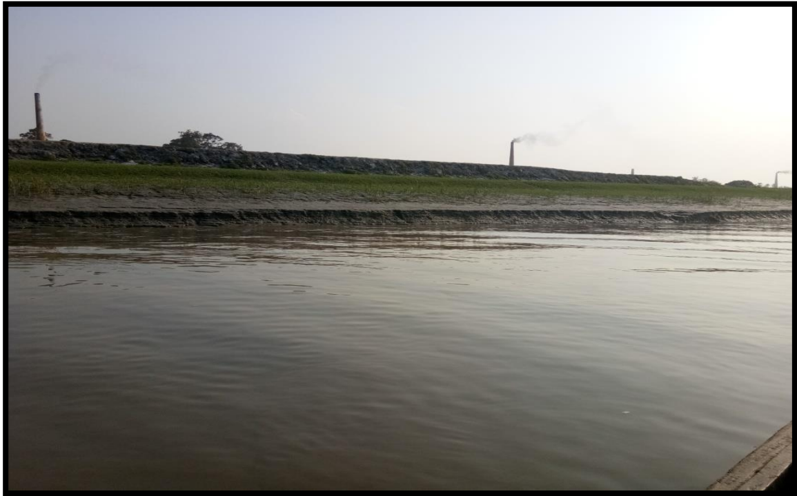
LEFT BANK AT CHAINAGE 16.9
