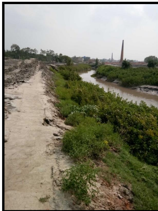
RIVER BANK AT CHAINAGE 4.7, LEFT BANK
