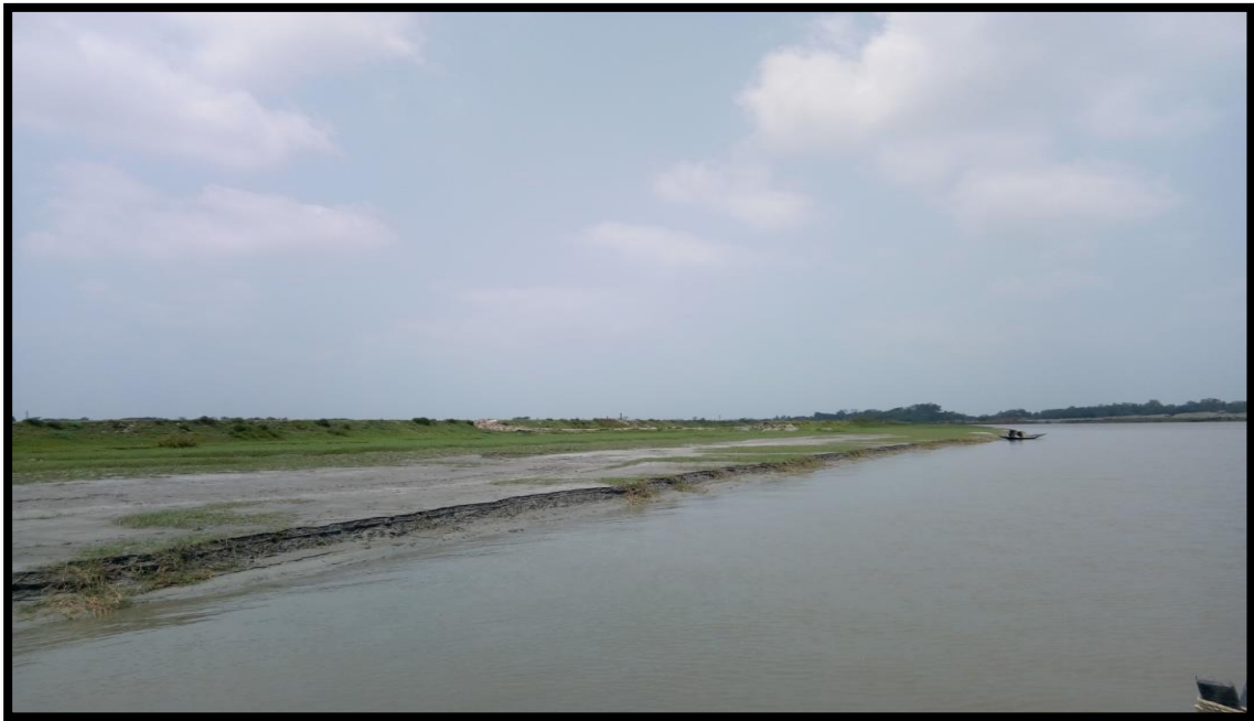
LEFT BANK AT CHAINAGE 26.5
