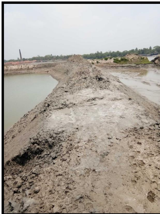
POND AT NEAR RIVER BANK CHAINAGE 3.5, LEFT BANK
