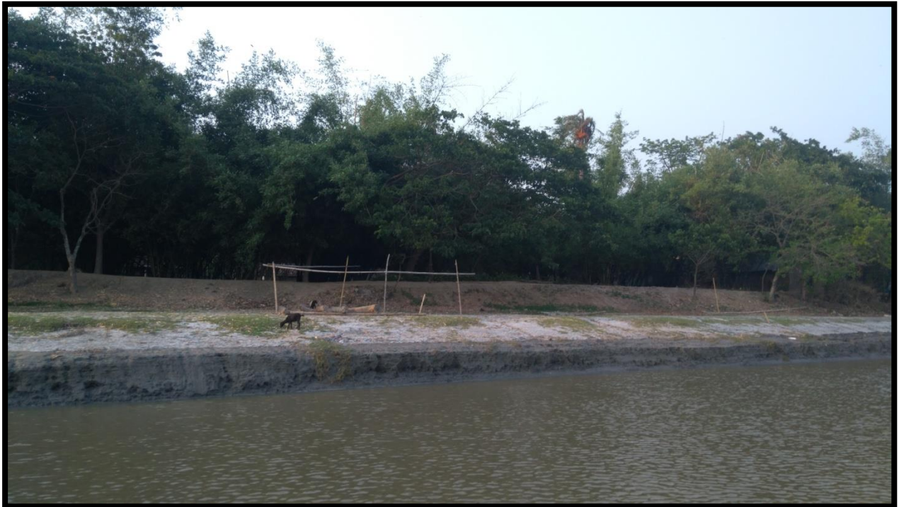
RIGHT BANK AT CHAINAGE 34
