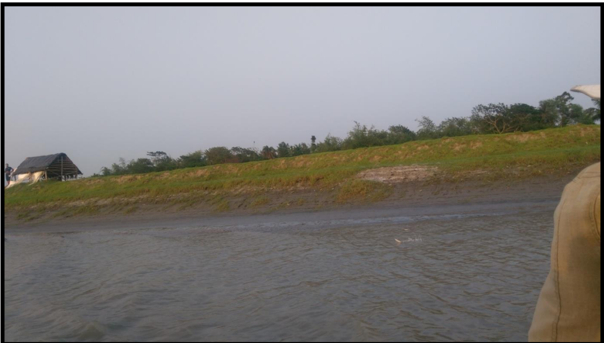
RIGHT BANK AT CHAINAGE 32.5
