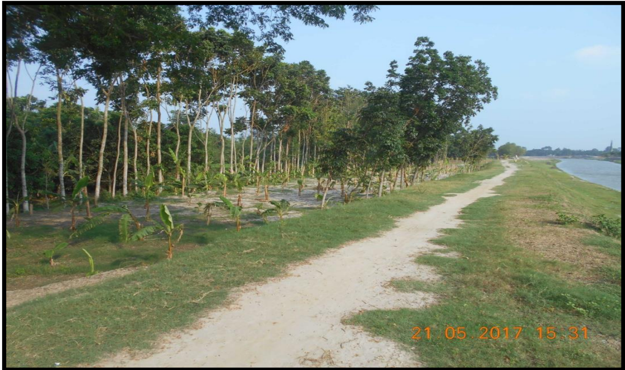
RIGHT BANK AT CHAINAGE 50.5
