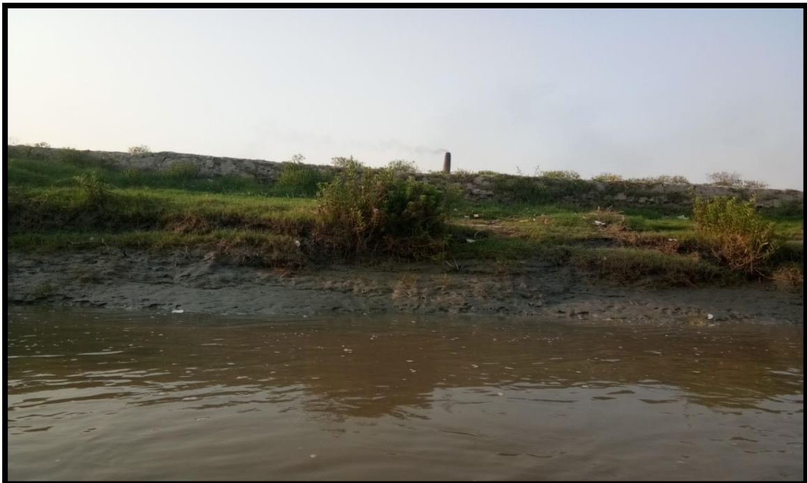
RIGHT BANK AT CHAINAGE 17.9
