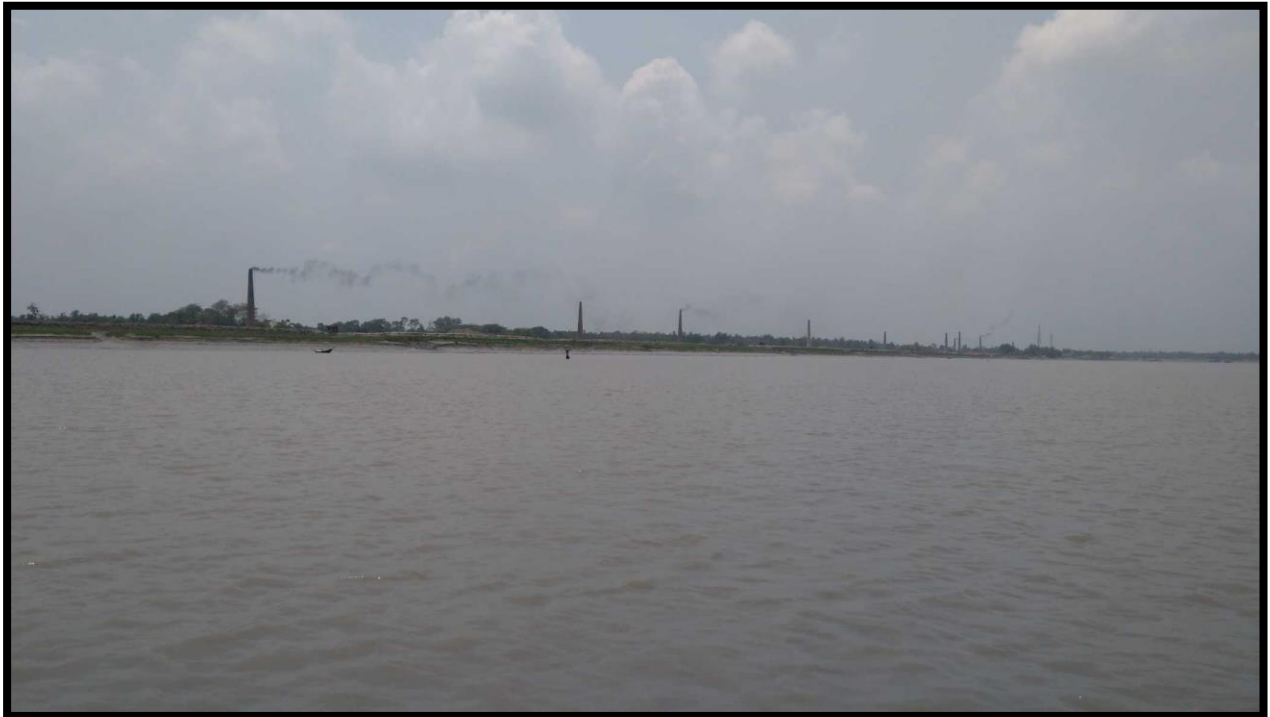
BRICK KLIN, 1.5 CHAINAGE, LEFT BANK
