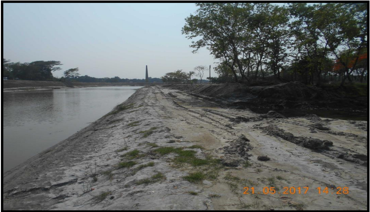
RIGHT BANK AT CHAINAGE 49
