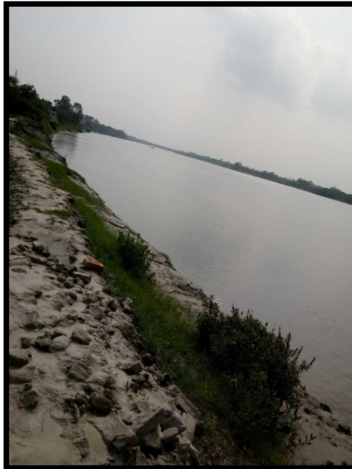
RIVER BANK AT CHAINAGE 6.0, LEFT BANK
