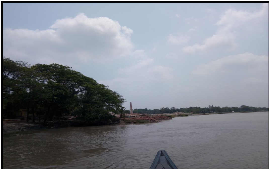
LEFT BANK AT CHAINAGE 24.5
