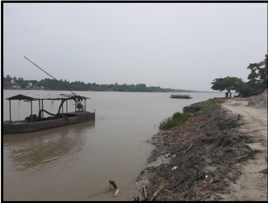
River Bank along the land acquired by M/s River Waterlink Pvt. Ltd. for RO-RO
