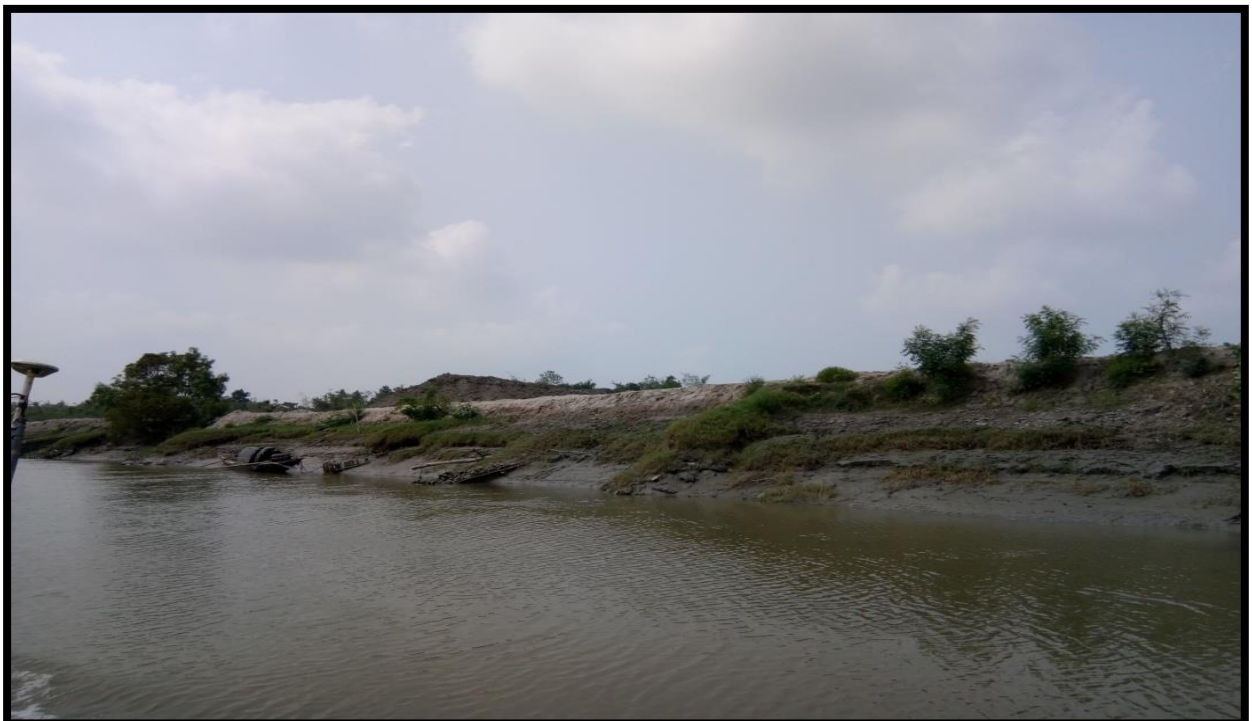
RIGHT BANK AT CHAINAGE 31.6
