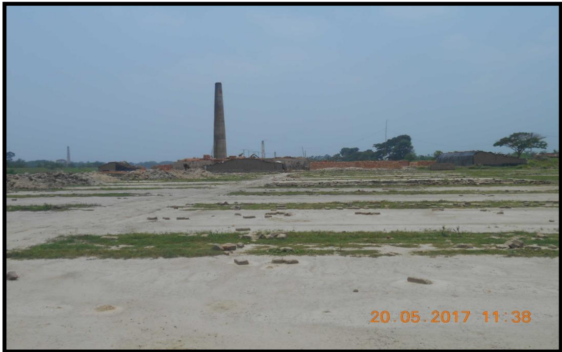
BRICK KLIN AT LEFT BANK CHAINAGE 61 .1
