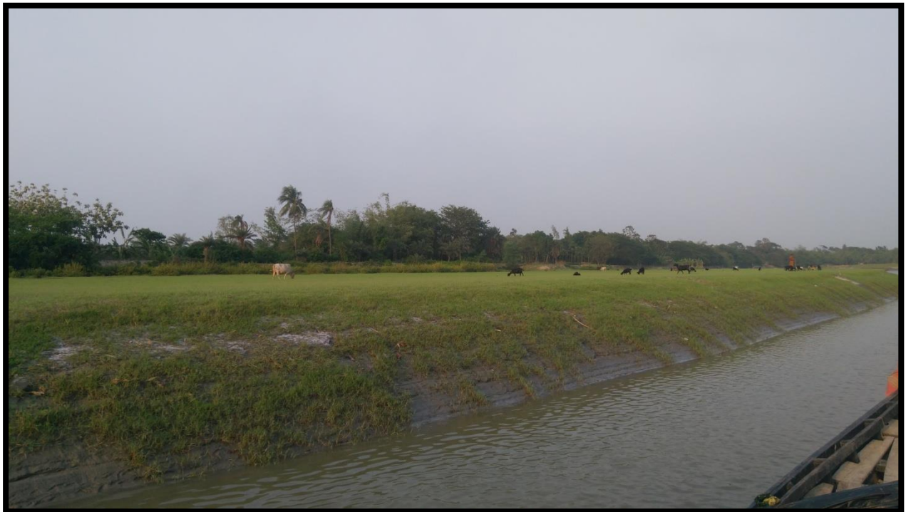
RIGHT BANK AT CHAINAGE 34.5
