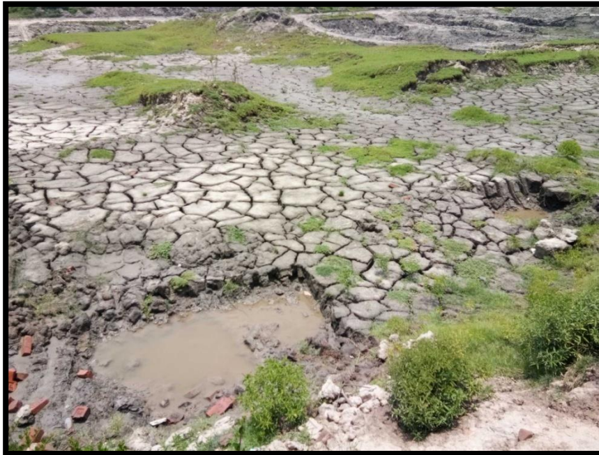
DRY POND NEAR RIVER BANK AT CHAINAGE 3.6, LEFT BANK
