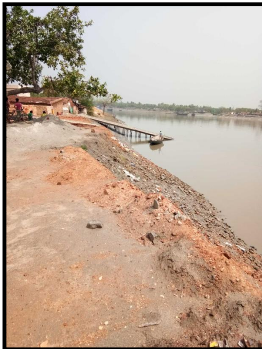
RIVER BANK AT CHAINAGE 3.1, LEFT BANK
