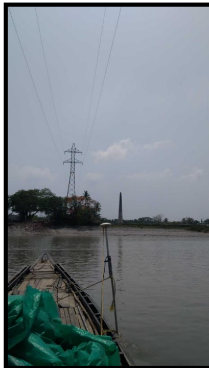
HIGH TENTION LINE, 3.1 CHAINAGE, LEFT BANK
