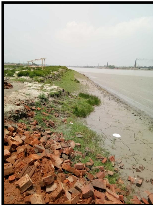
RIVER BANK AT CHAINAGE 3.6, LEFT BANK
