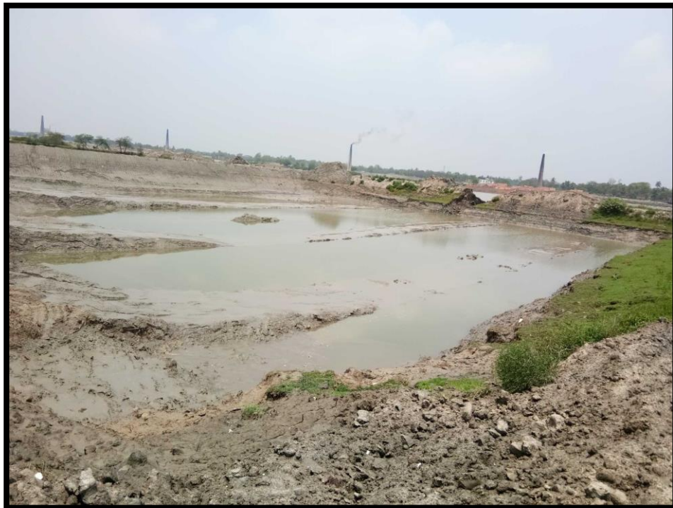
POND AT CHAINAGE 3.4, LEFT BANK
