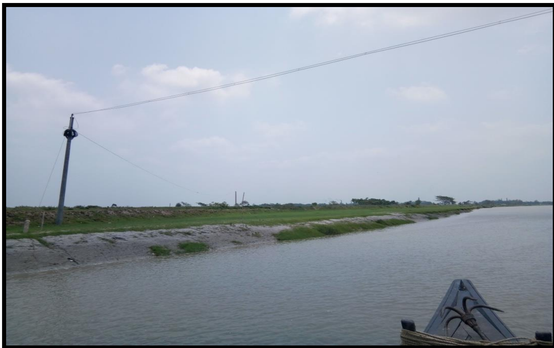
LEFT BANK AT CHAINAGE 27
