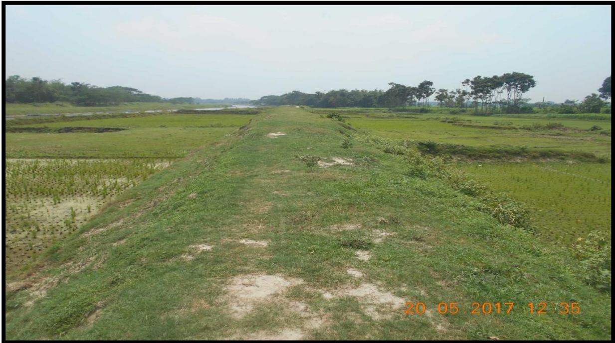
LEFT BANK AT CHAINAGE 59.8
