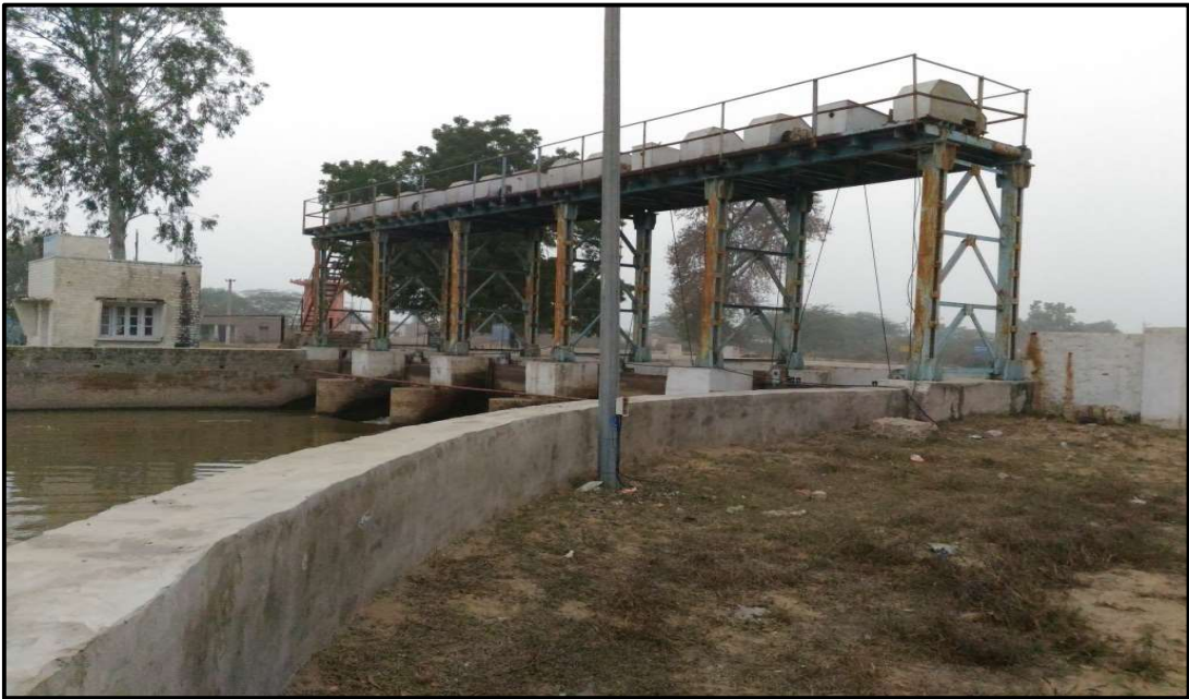
Figure 12 – Side Branch on Biradhwal Head, Anoopgarh Shakha (brnach CH: 2.20Km)
