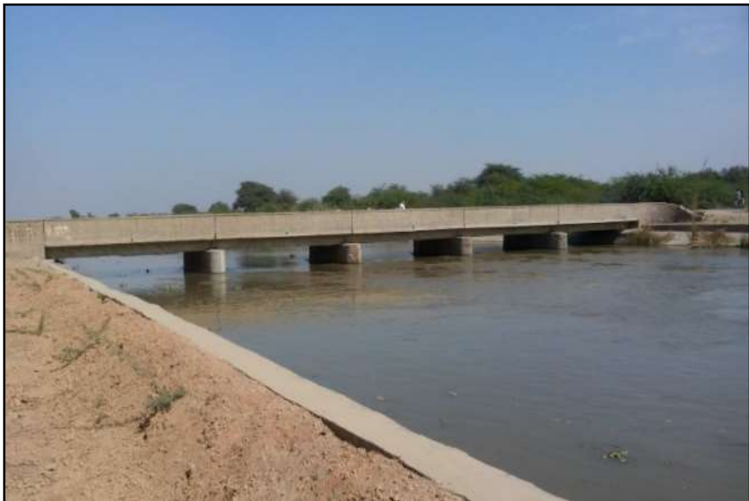
Figure 36 – Village Road Bridge RD 850 (Ch. 187.70 Km)
