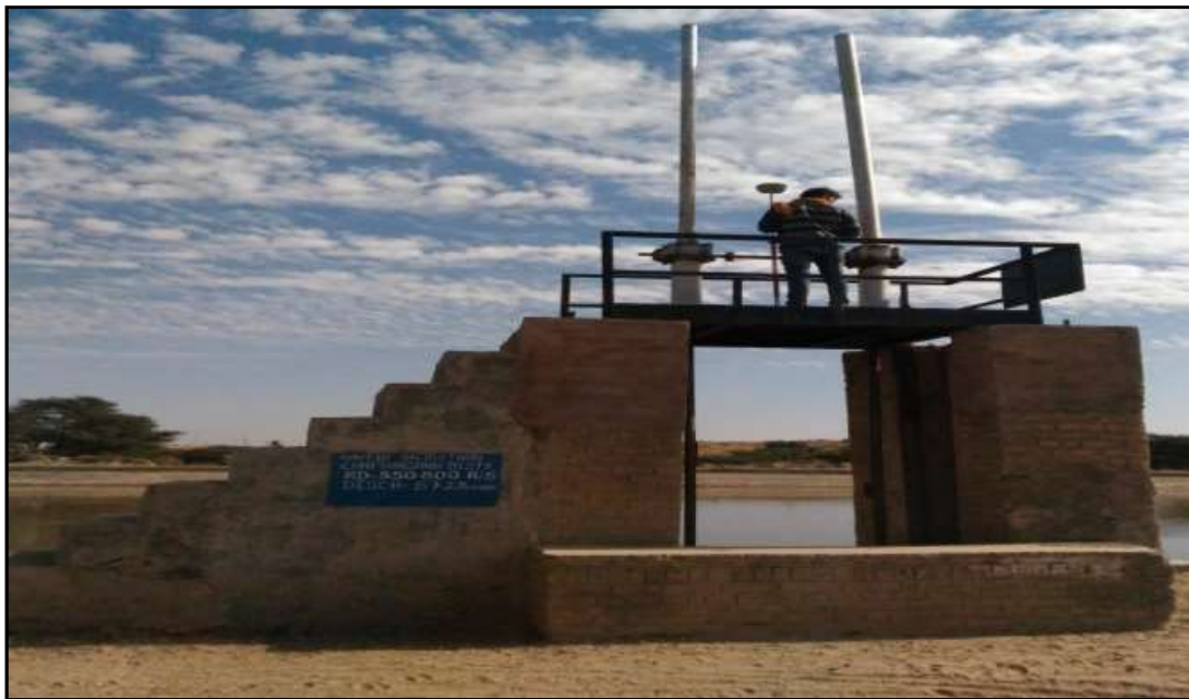
Figure 24 – Bridge on RD 550 (Ch. 96.25 Km)
