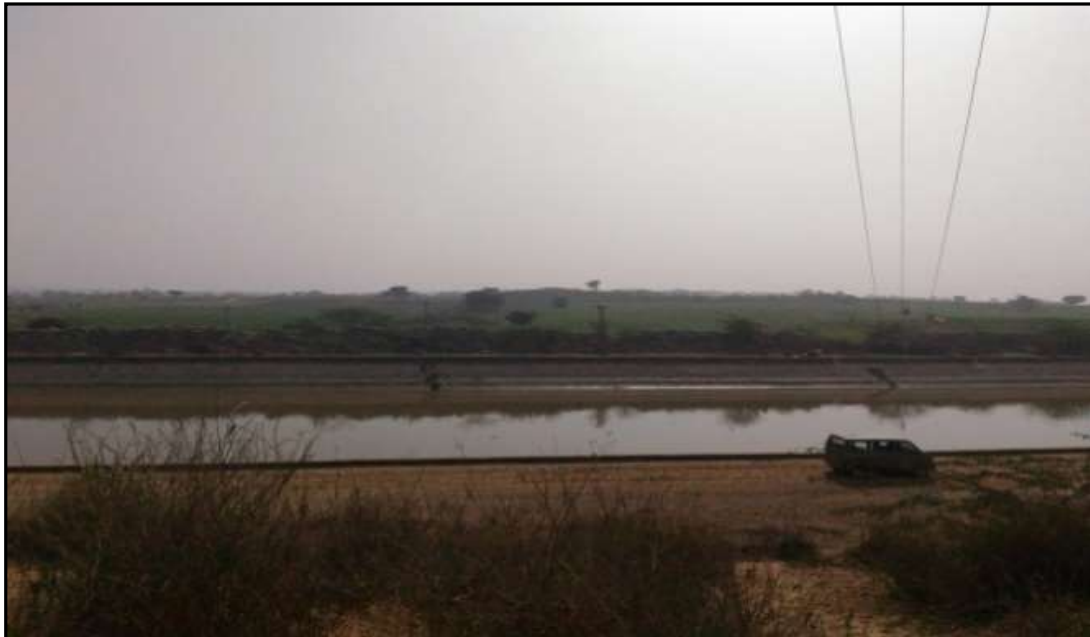
Figure 14 – Electric Line (Ch: 13.36 Km)
