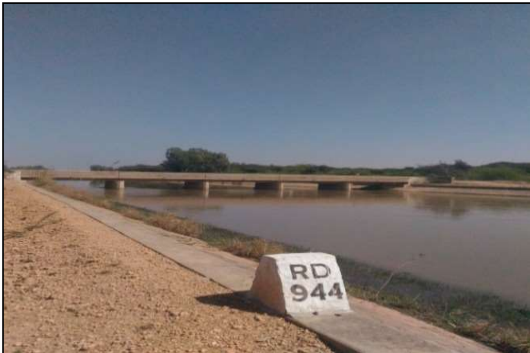
Figure 40 – Village Road Bridge RD 945 (Ch. 216.28 Km)
