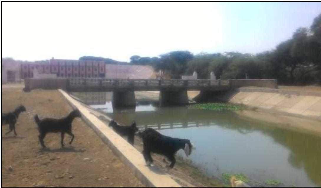
Figure 48 – Lift Irrigation Canal on Left bank of Canal RD 1205 (Ch. 294.80 Km)
