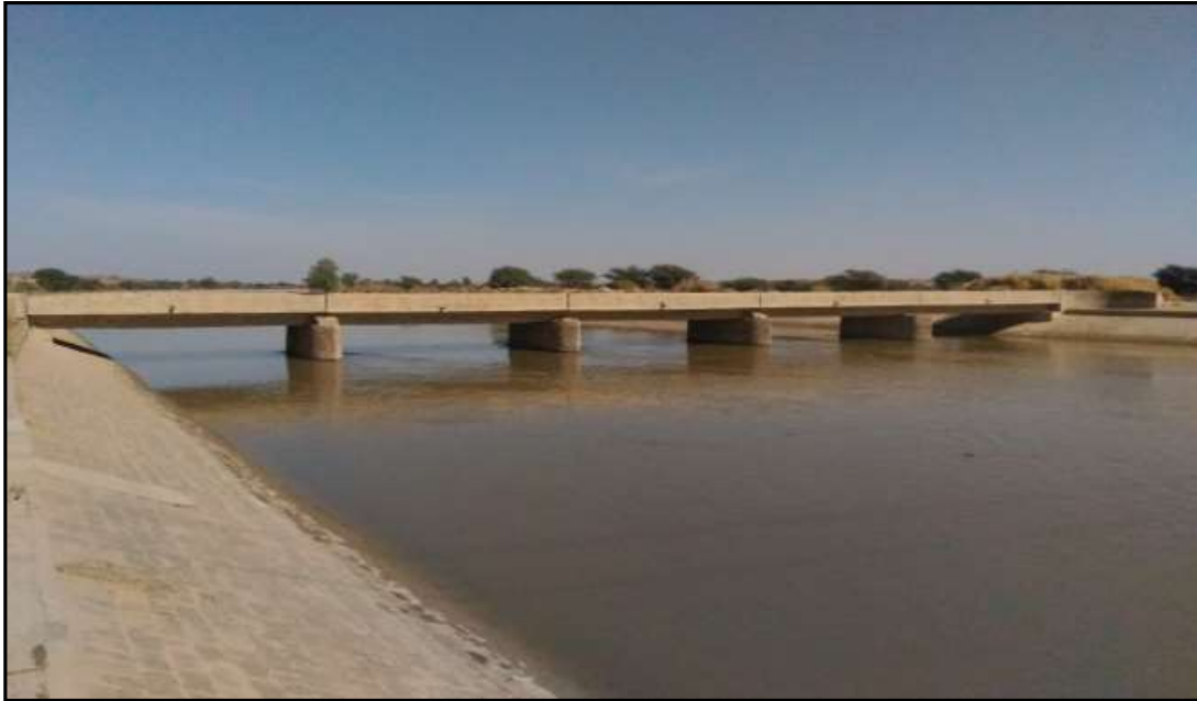
Figure 23 – Bridge on RD 528 (Ch.88.90 Km)
