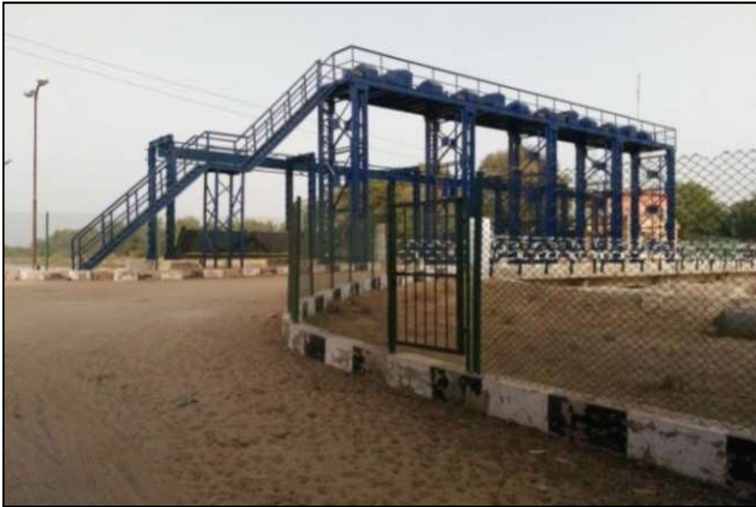
Figure 31 – Head Lock RD 750 (Ch. 157.02 Km)
