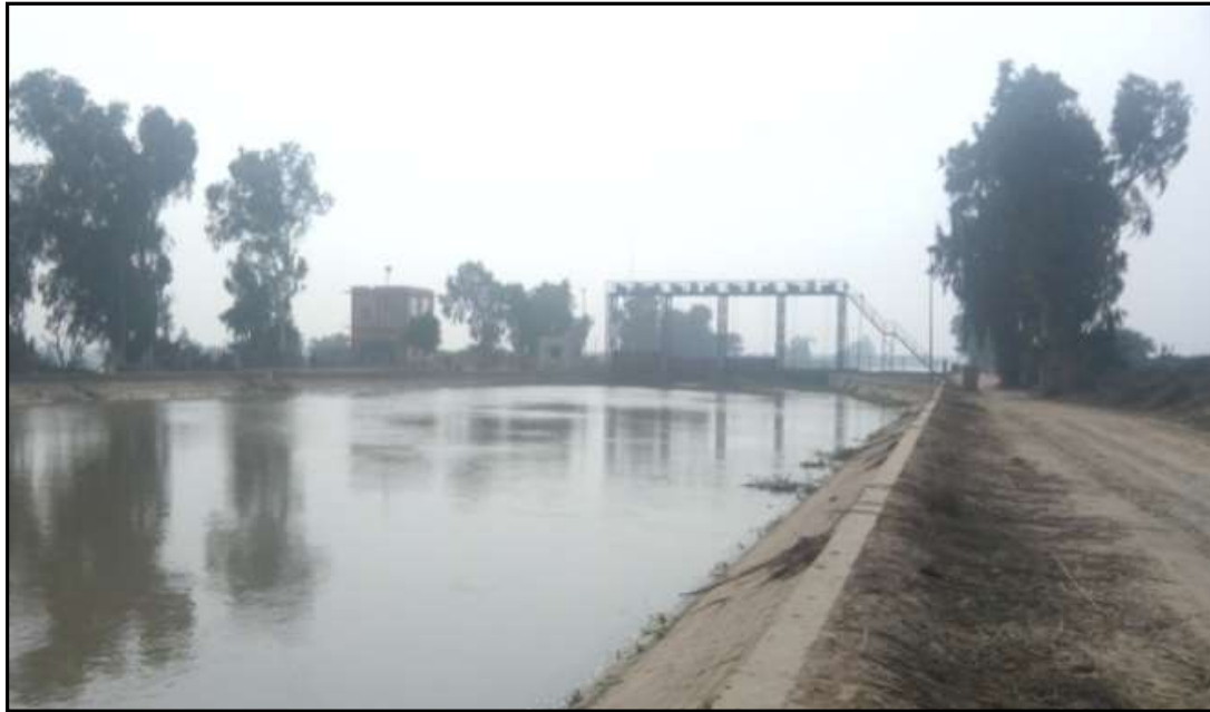
Figure 15 – Harinagar 415 RD Head Lock (Ch: 54.73 Km)
