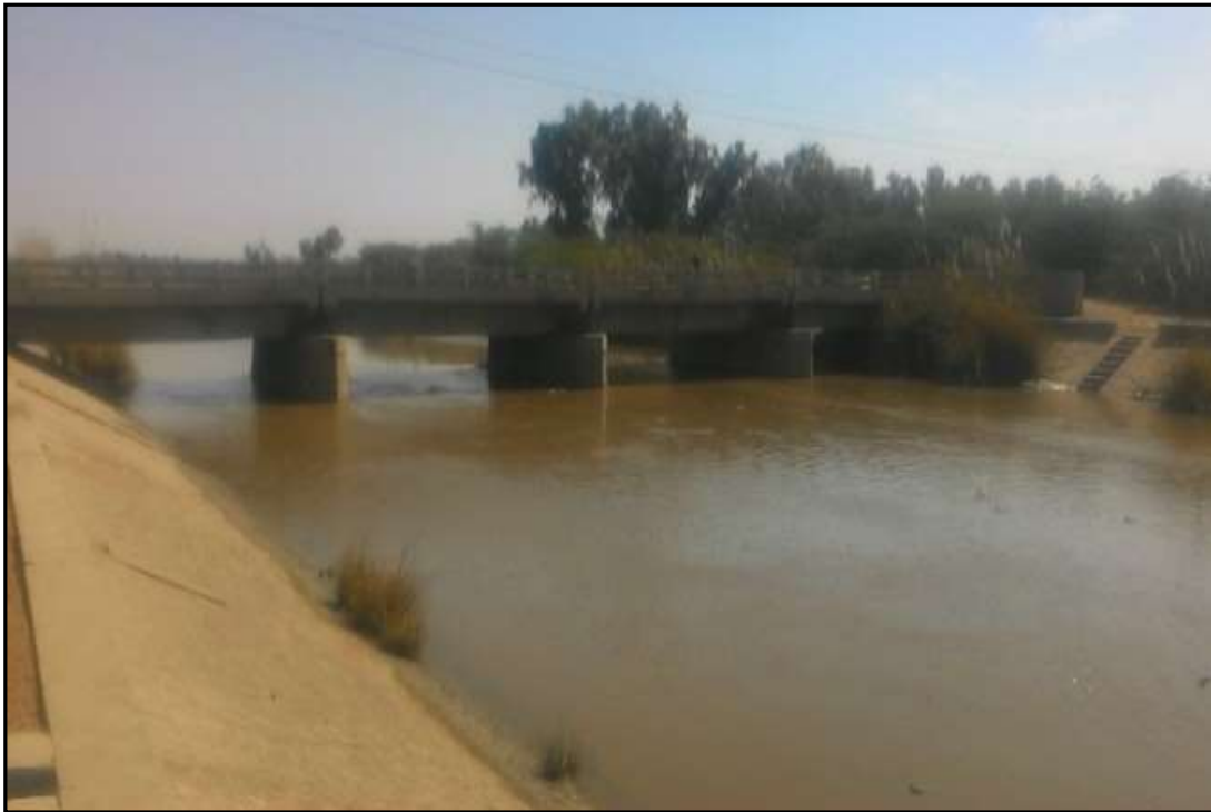
Figure 45 – Village Road Bridge RD 1058 (Ch. 251.10 Km)
