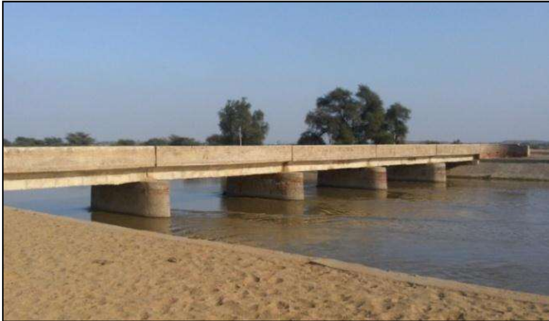
Figure 18 – Sherpur Bridge 445 RD (Ch.63.80 Km)
