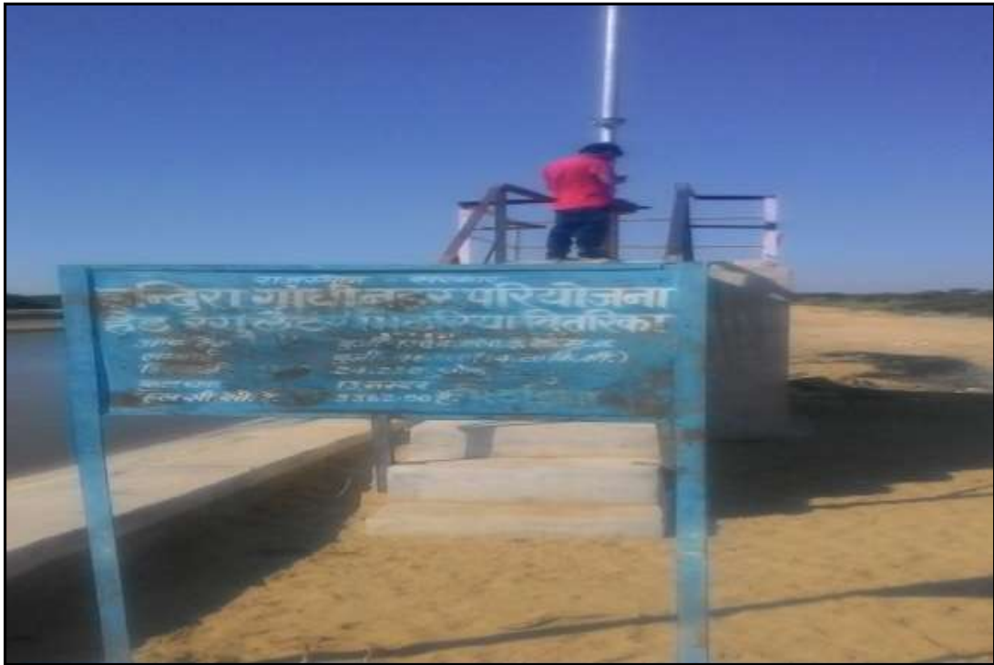
Figure 52 – RD 1304 Minor (Ch. 326.10 Km)
