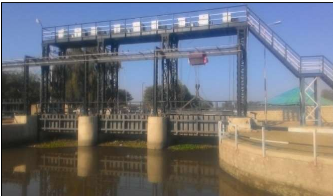
Figure 49 – RD 1254 Head Lock (Ch. 310.80 Km)
