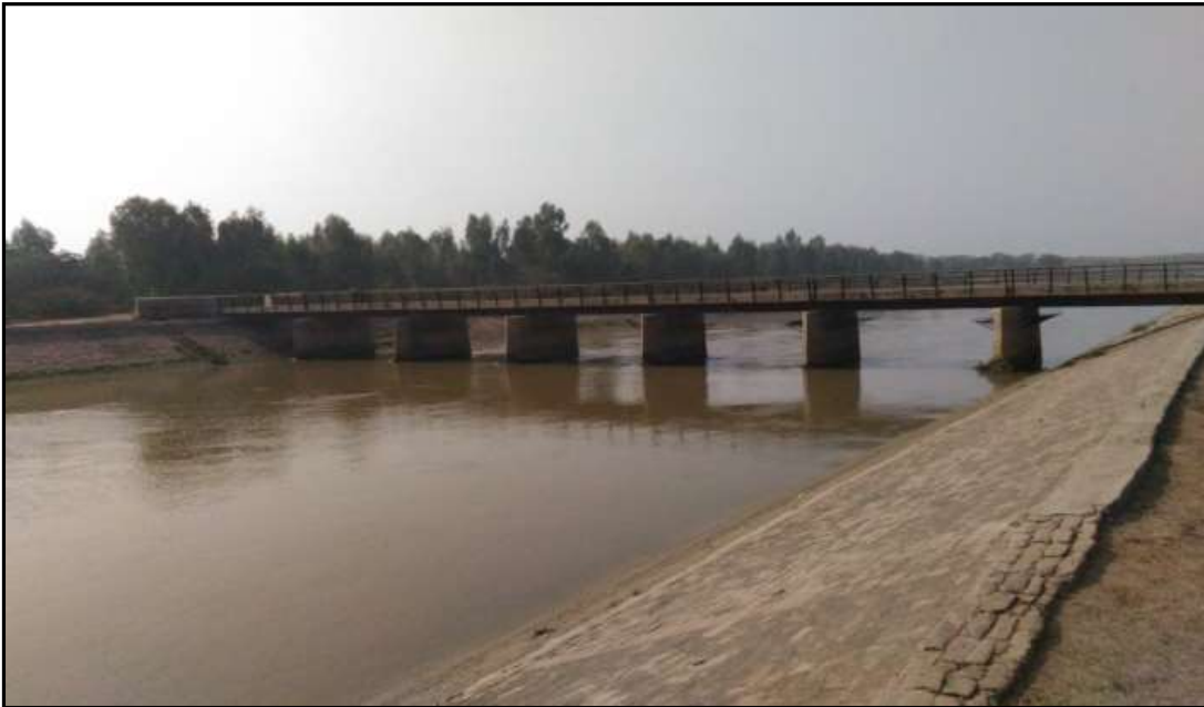
Figure 13 – Ladhana Bridge RD 253 (Ch: 5.11Km)
