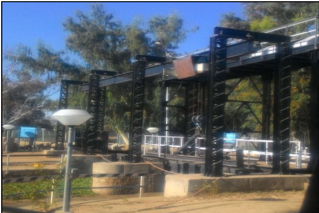
Figure 57 – RD 1458.5 Head Lock (Ch. 373.10 Km)
