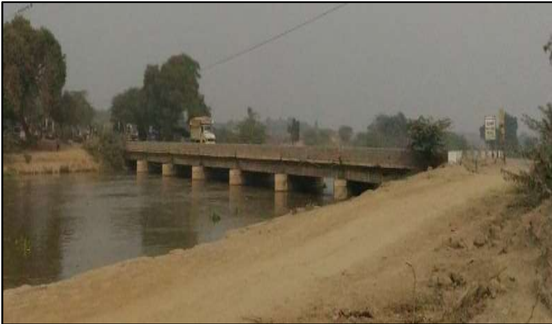
Figure 9 – Ch: 0.00 Km NH-15 Bridge Near Piperan villlage
