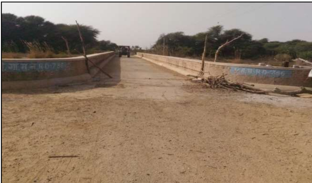
Figure 34 – Village Road Bridge RD 786 (Ch. 168.09 Km)
