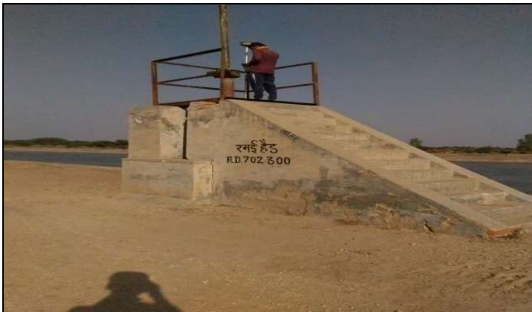
Figure 30 – Ramal Head at IG Canal at RD 702.30 (Ch. 142.38 Km)
