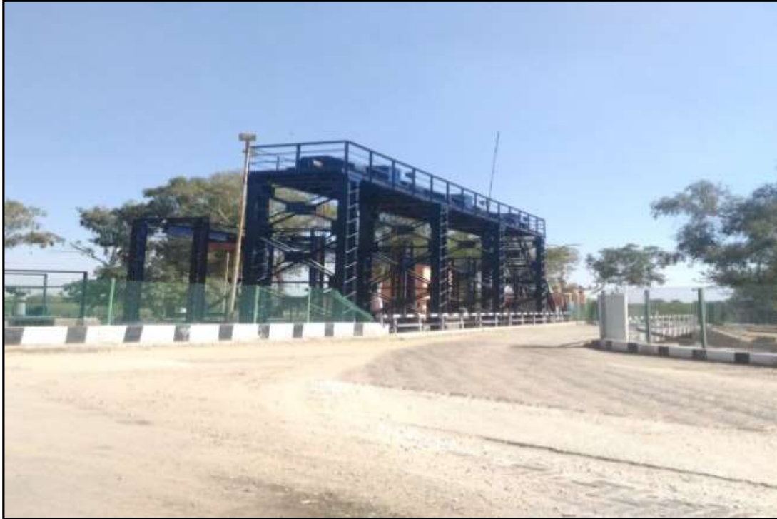
Figure 41 – RD 961 Head Lock and Lock Bridge (Ch. 221.66 Km)
