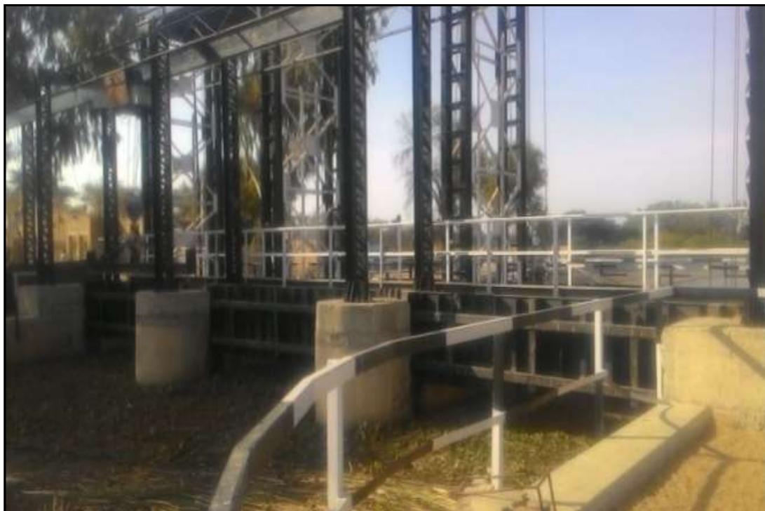
Figure 53 – RD 1365 Head Lock (Ch. 344.36 Km)
