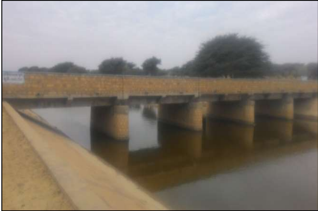
Figure 56 – Village Road Bridge RD 1405 (Ch. 356.85 Km)
