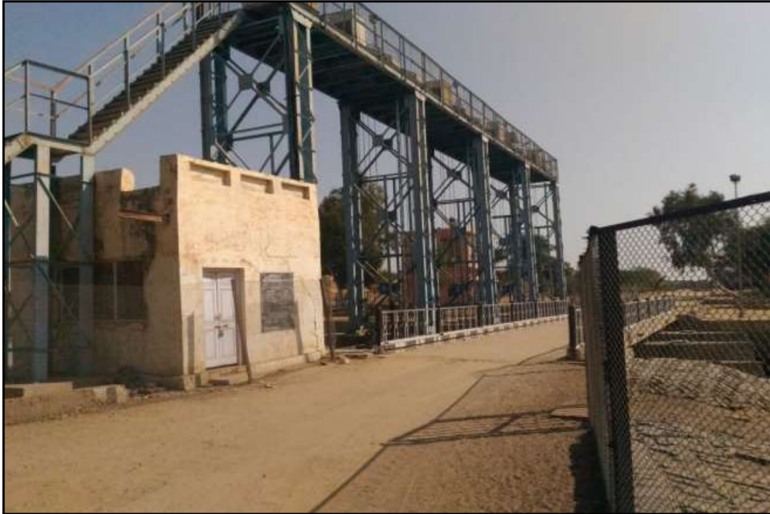
Figure 26 – 620 RD Head Lock and Lock Bridge (Ch. 117.02 Km)
