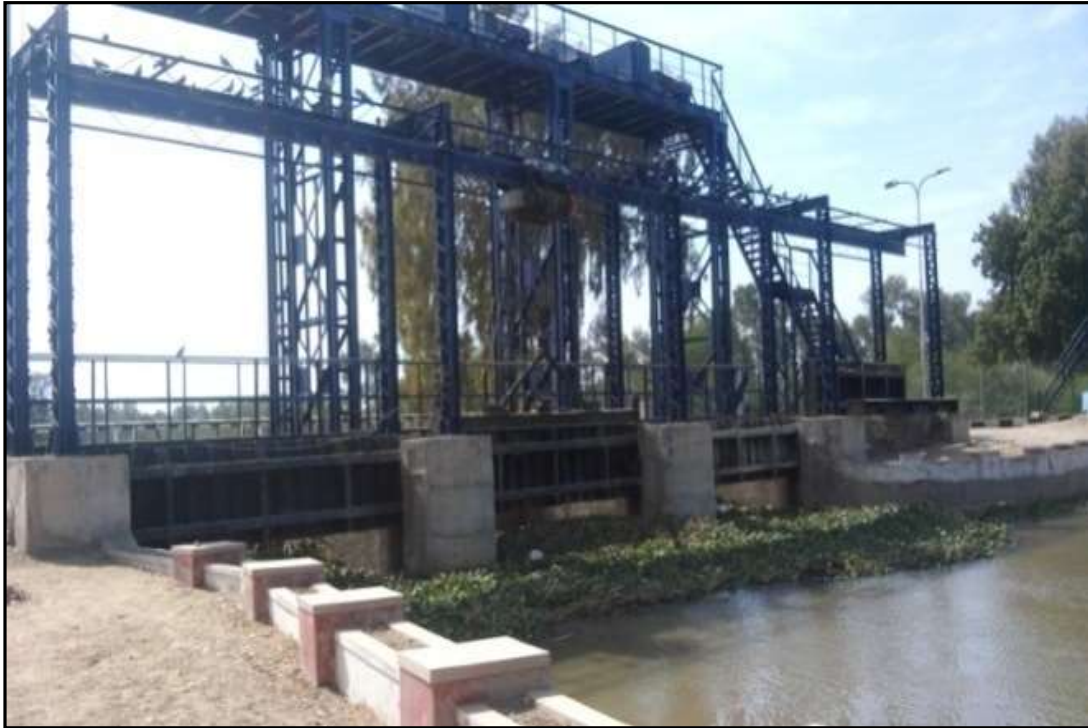
Figure 37 – RD 860 Head Lock (Ch. 190.04 Km)
