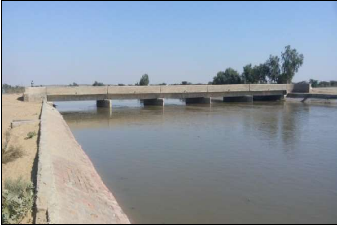
Figure 25 – Bridge on RD 587 (Ch. 107.80 Km)
