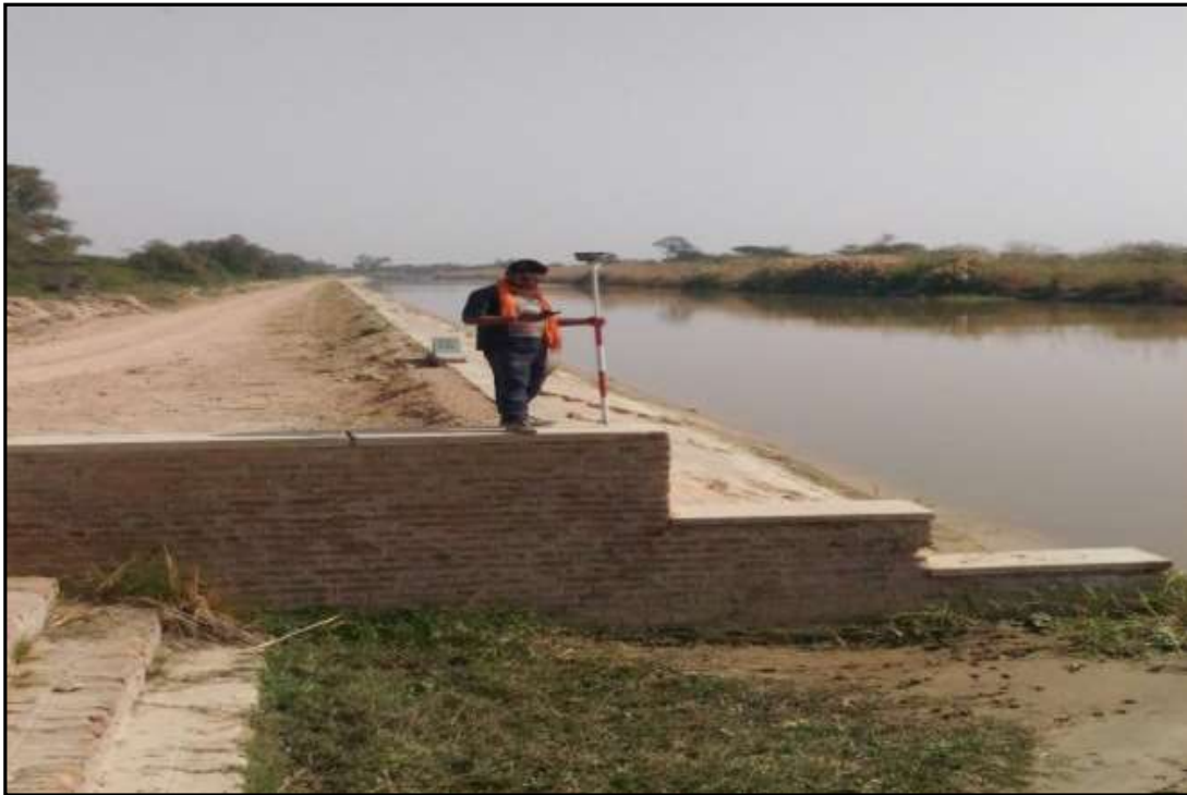
Figure 35 – Spot Level Acquisition RD 800 (Ch. 172.35 Km)
