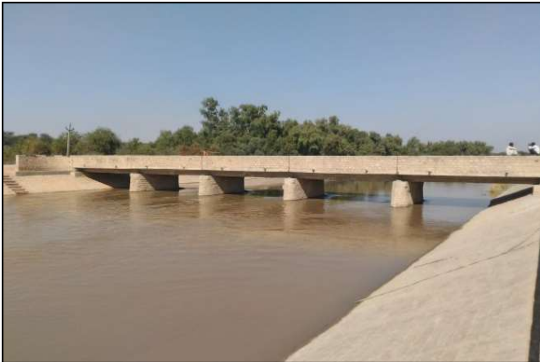
Figure 44 – Village Road Bridge RD 1041 (Ch. 246.10 Km)
