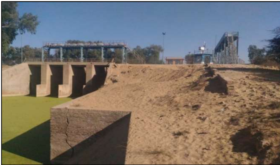
Figure 20 – Escape Canal at 507 RD Head (Ch. 82.82 Km)
