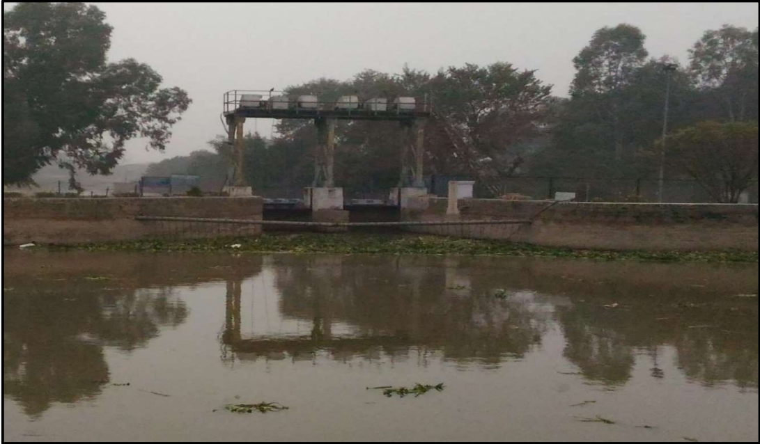
Figure 11 – Side Branch n Biradhwal Head, Lunaksar Shakha (branch CH:2.20Km)
