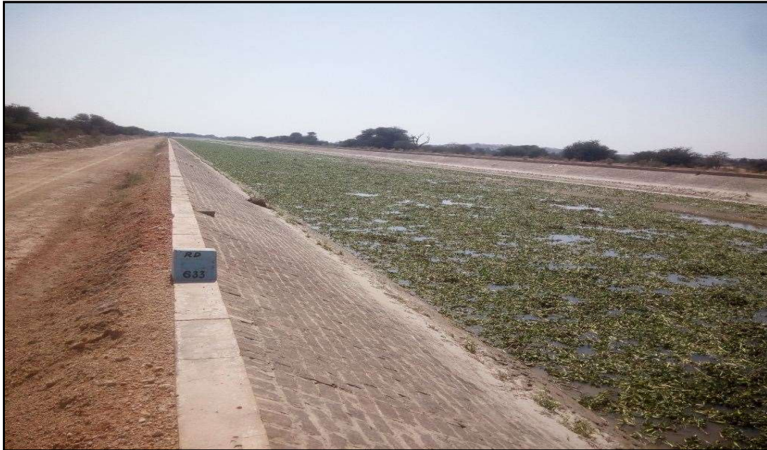
Figure 29 – Weeds floating over water in IG Canal at RD 633 (Ch. 121 Km)
