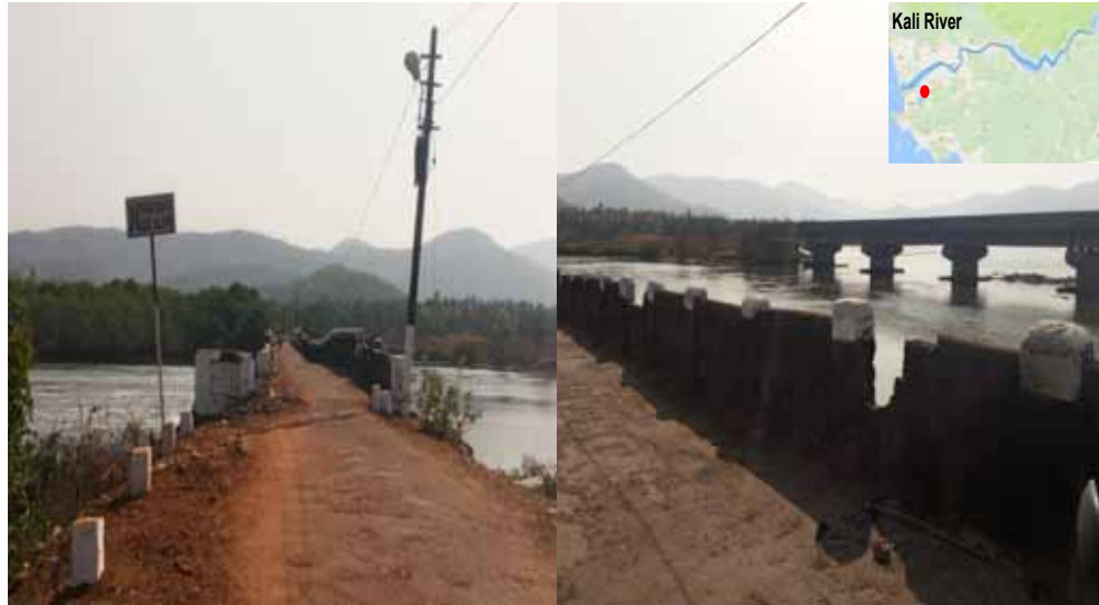
FIGURE 4-3: Expansion of Kadwad Bridge (Under Construction)
