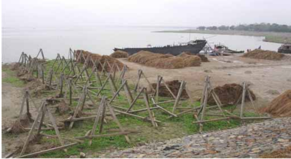
Figure 6-8: Porcupine Arrangement
