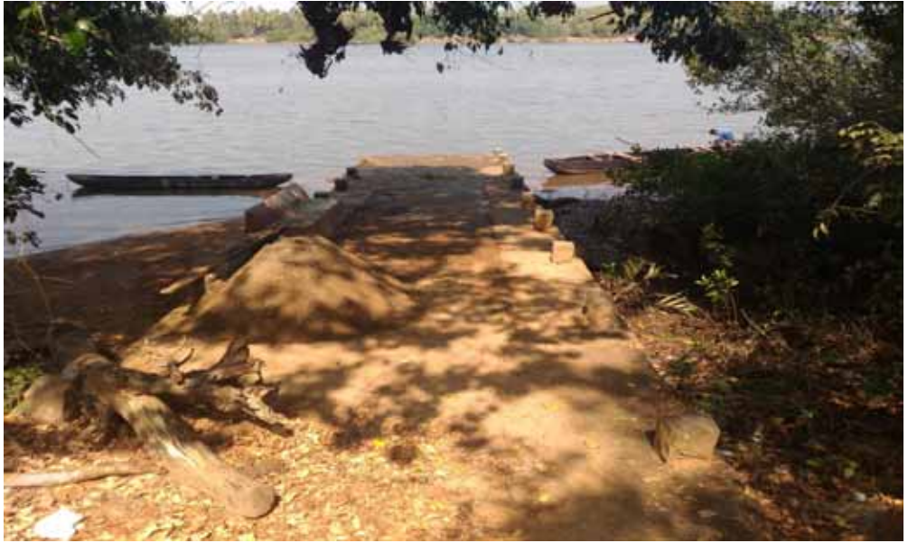
FIGURE 4-18: Passenger Jetty at Wailwada near Siddar
