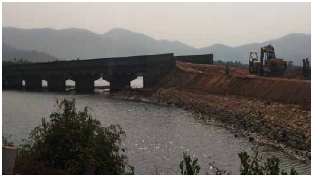
FIGURE 4-4: Kadwad Bridge on Kali River (Fully Functional)
