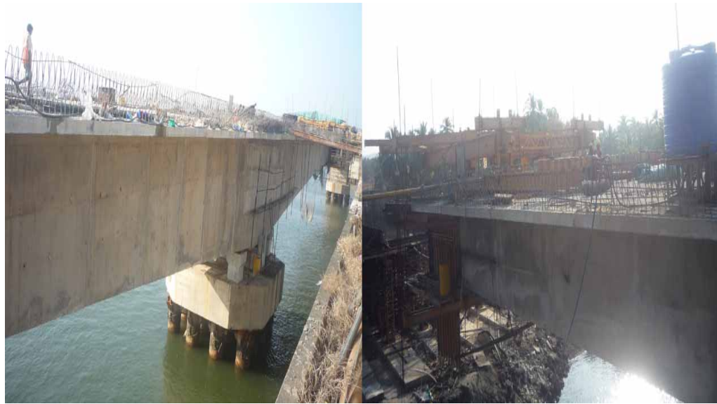
FIGURE 4-5: Under Construction Bridge on Kali River
