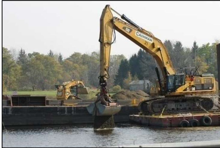
Figure 3.1: Dredging a river
