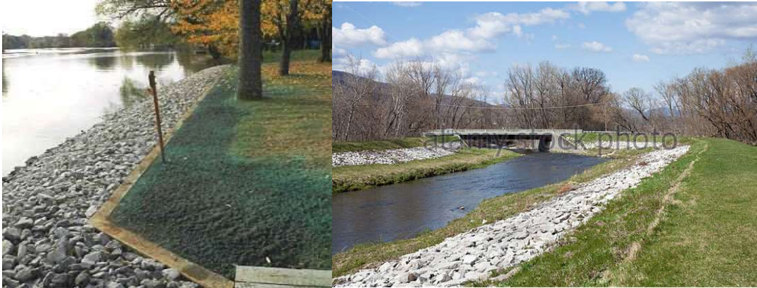
Figure 3.3: A typical protected bank using rip-rap and vegetation
