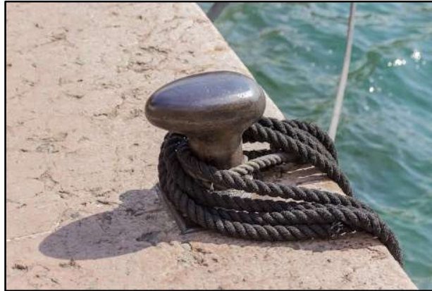
Figure 5.8: A typical bollard fixed to a quay
