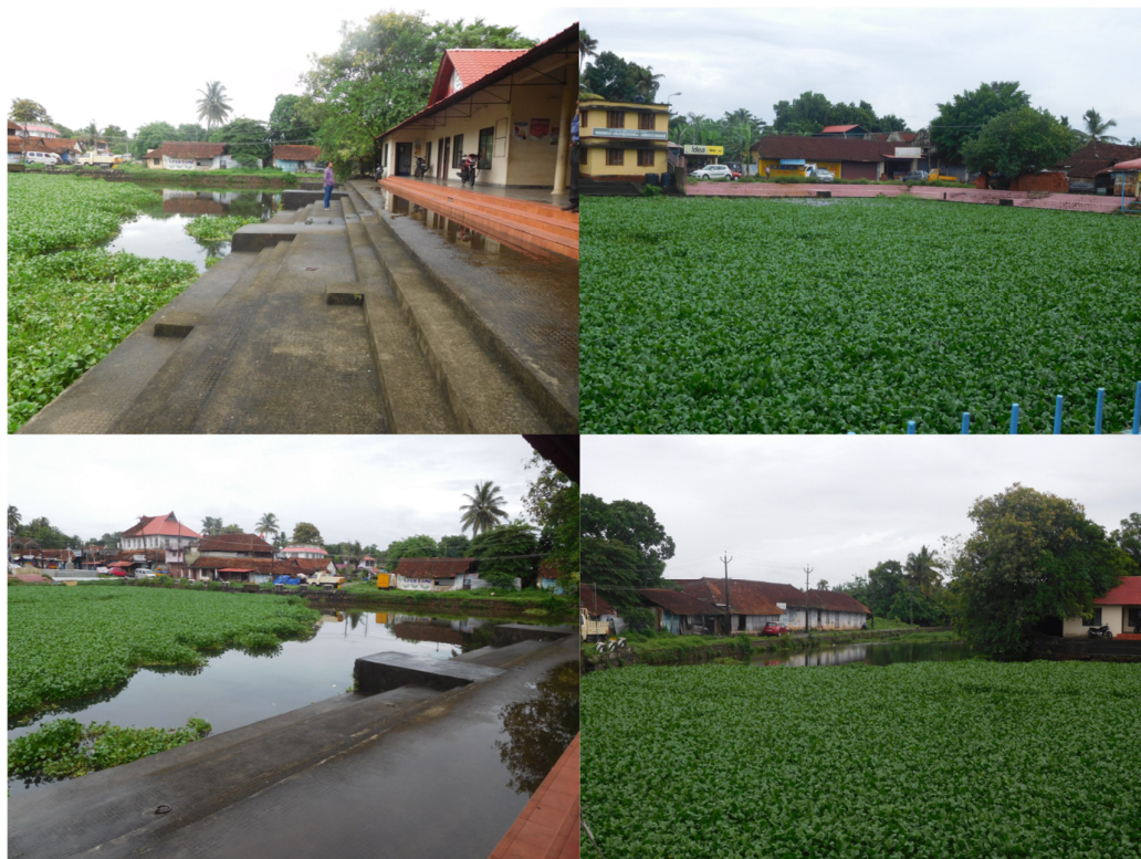
Figure 4-9 Changanassery ferry terminal
