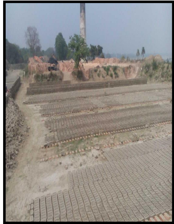
Brick Kline At Bykandapur Chainage 9.5
