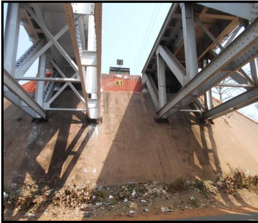
Railway Bridge 2 Kolaghat
