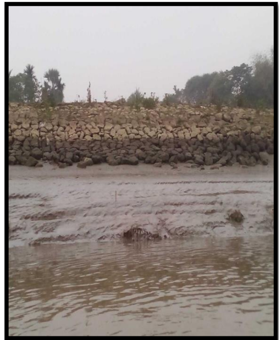
Protected River Bank at Chainage 9.4
