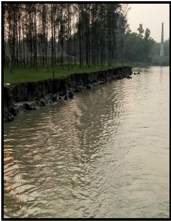
River Bank At Chainage 1.2
