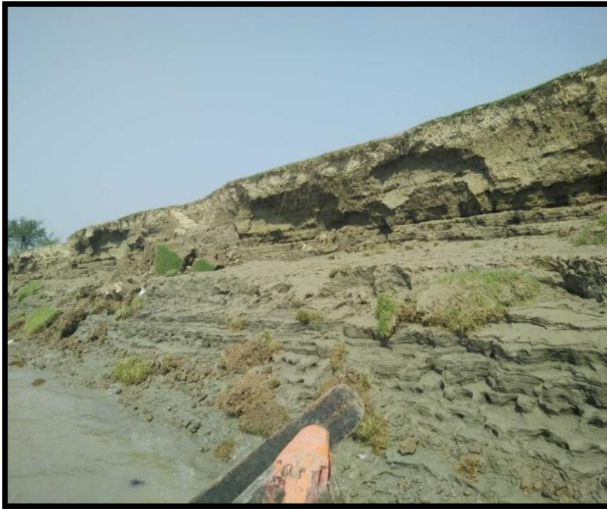
River Bank At Chainage 22.7
