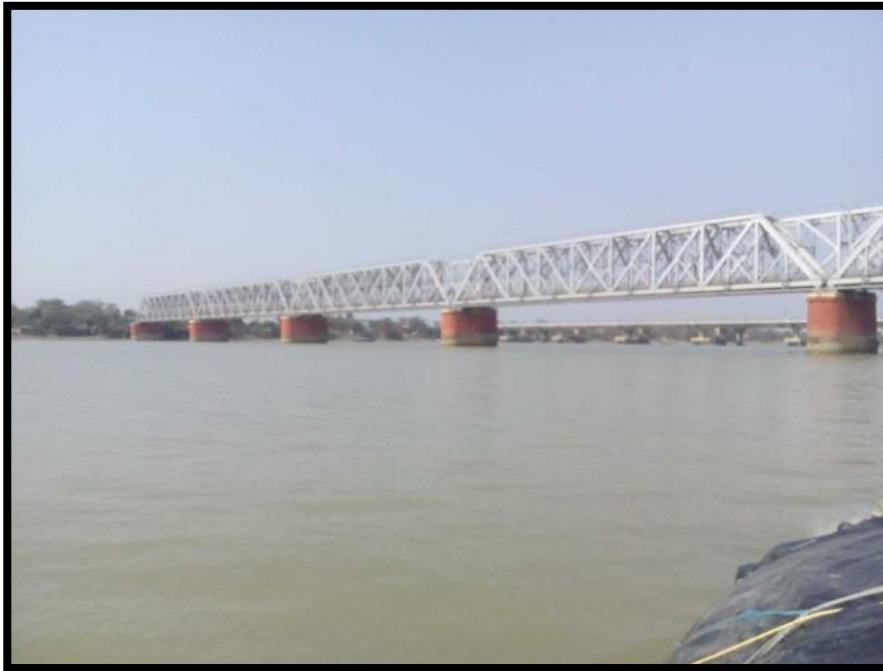
Kolaghat Railway Over Bridge
