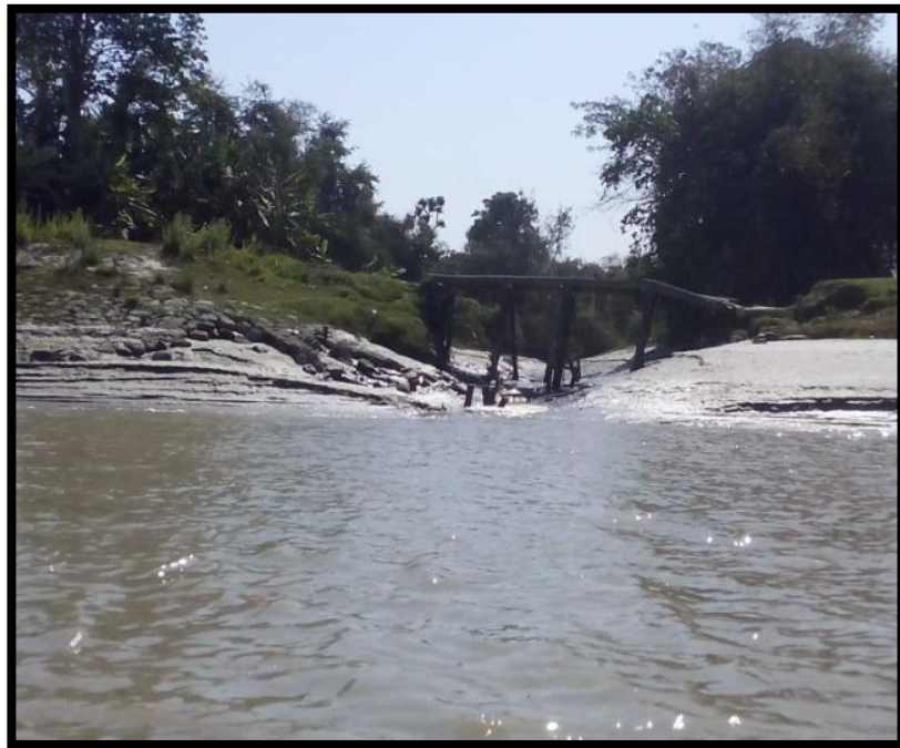
Wooden Bridge A Chainage 35.5
