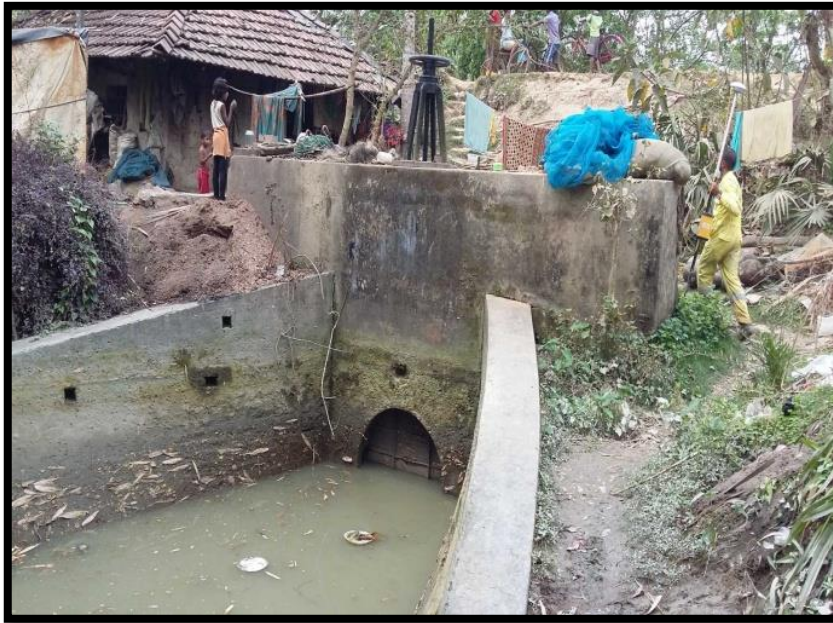
Culvert at Natshal
