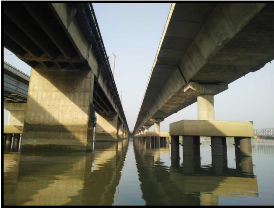
Kolaghat Bridge at Chainage 35.76
