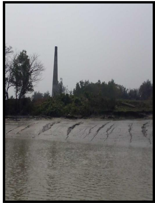
Brickline at Chainage 4.6
