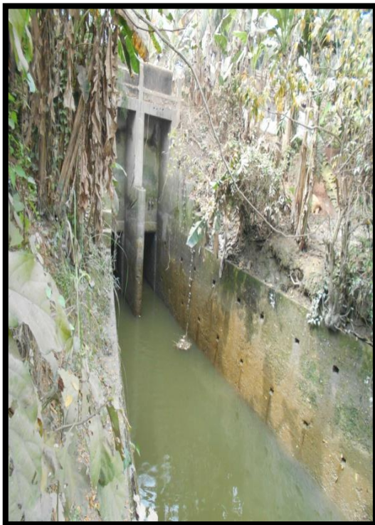
Aqueducts at Nanpur Village
