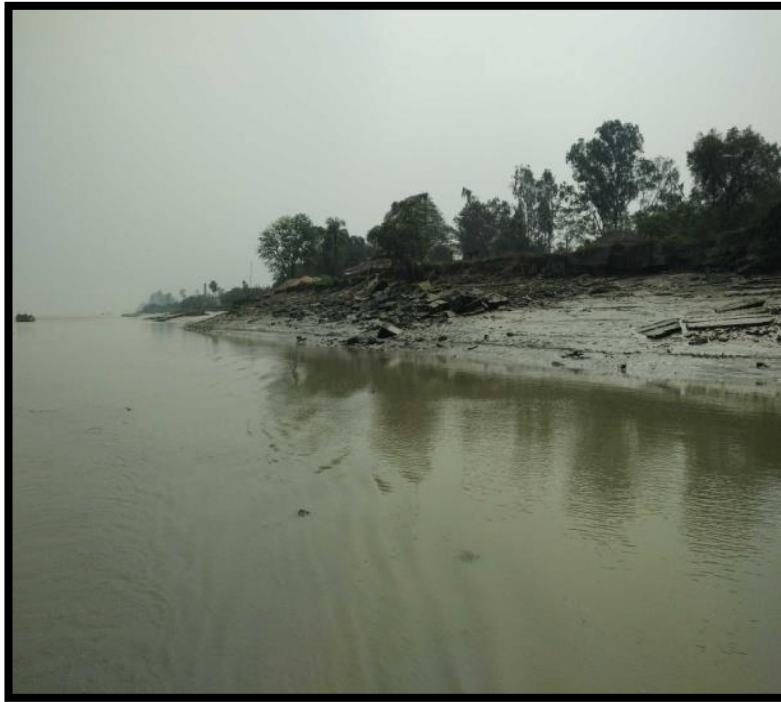
River Bank At Chainage 8.3
