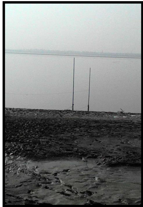
Erection of Tide Pole at Geonkhali
