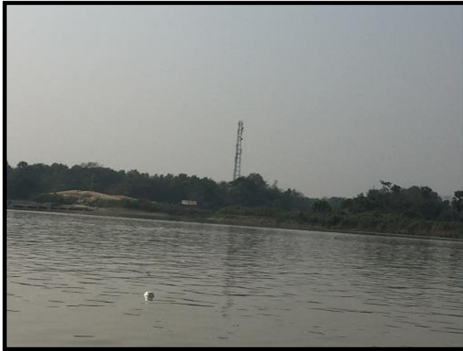
Mobile Tower At Chainage 34.5
