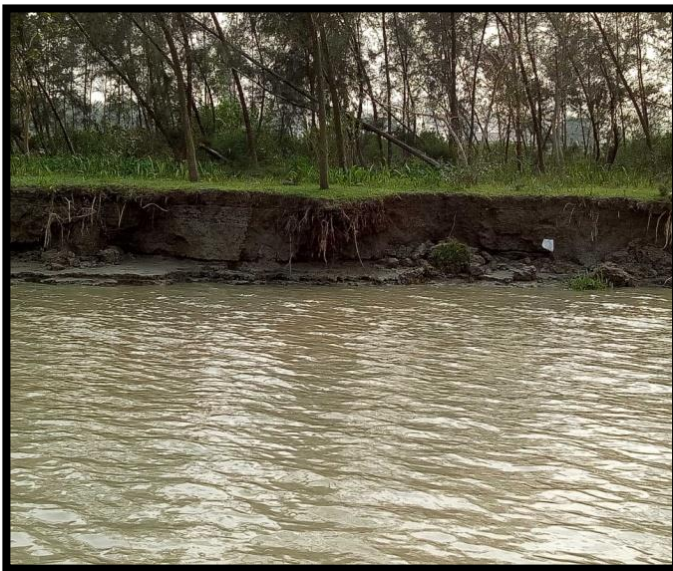
River Bank at Chainage 1.0
