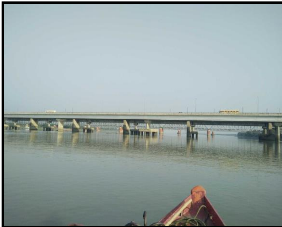
Kolaghat Road Bridge at Chainage 35.76
