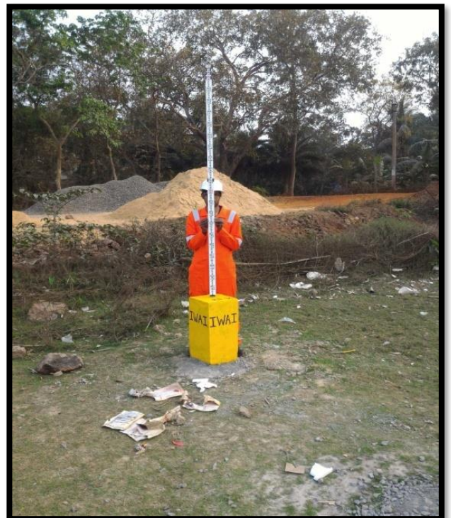
Levelling at RN 5
