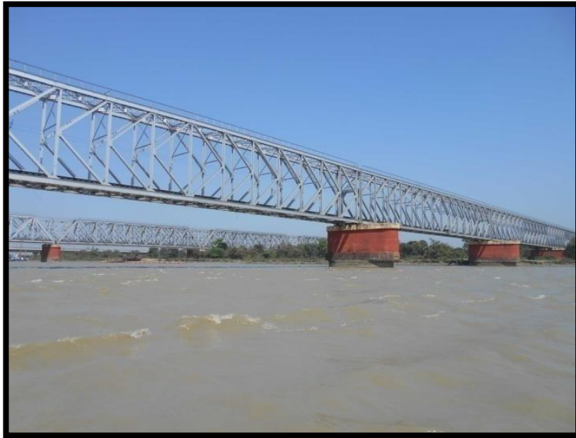
Railway Bridge At Kolghat Chainage 35.2
