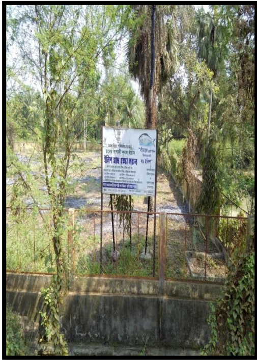
Compound wall fishery department at chainage 37.5
