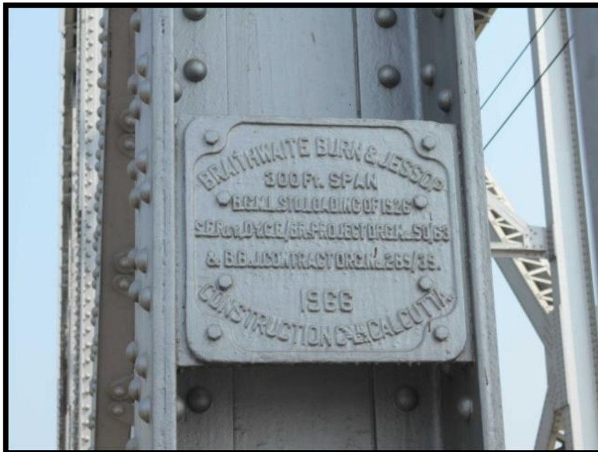
Kolaghat Railway Bridge NO.1
