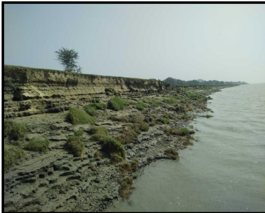
River Bank At Chainage 22.7
