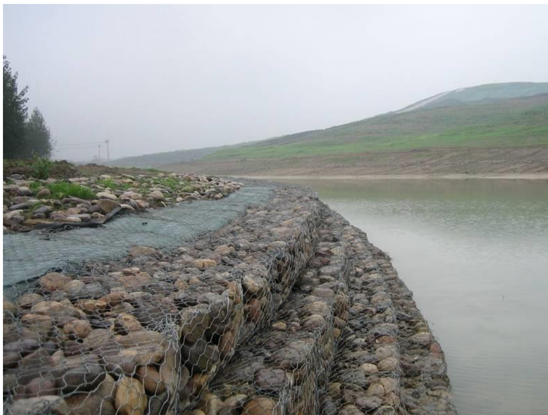
Figure 17: Photograph showing arrangement of Gabion Wall along River Bank
