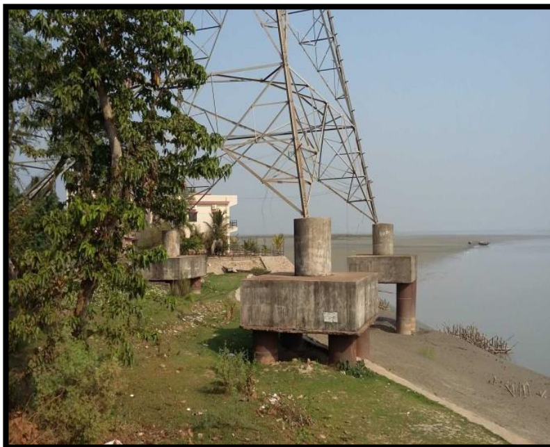
High Tension Line At Orphuli Chainage 34.4
