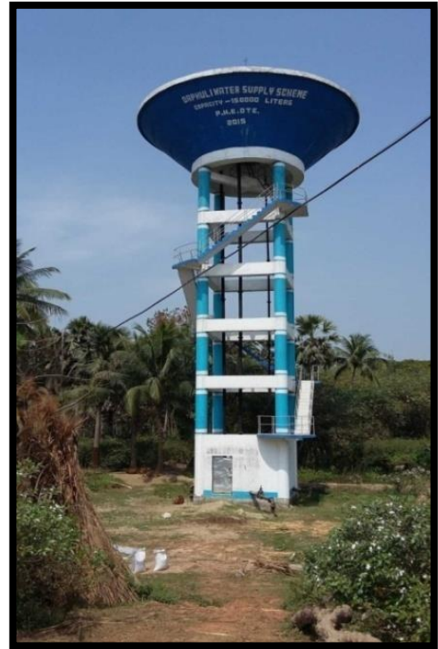
Water Tank at Orphuli
