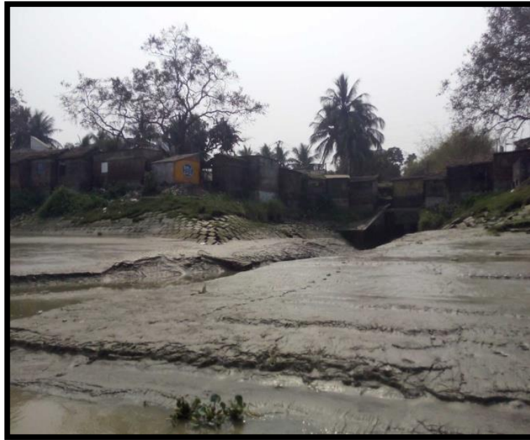
River bank at Chainage 2.8
