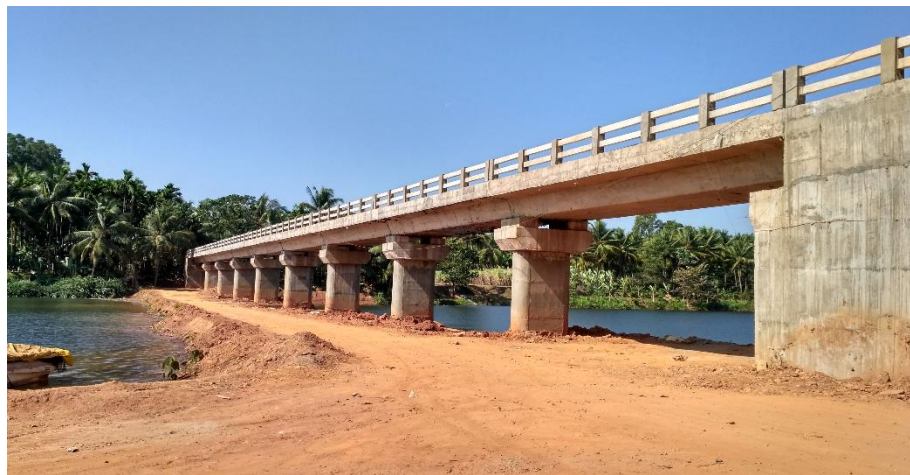
FIGURE 4.9: Haigund Island Bridge
