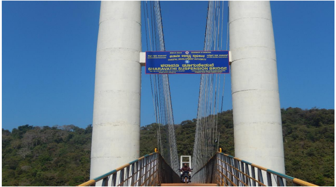
FIGURE 4.10: Suspension Bridge in Upponi, Honnavar
