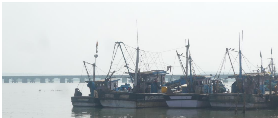
FIGURE 4.7: Edapally-Panvel Highway Bridge on Sharavati River at Honnavar
