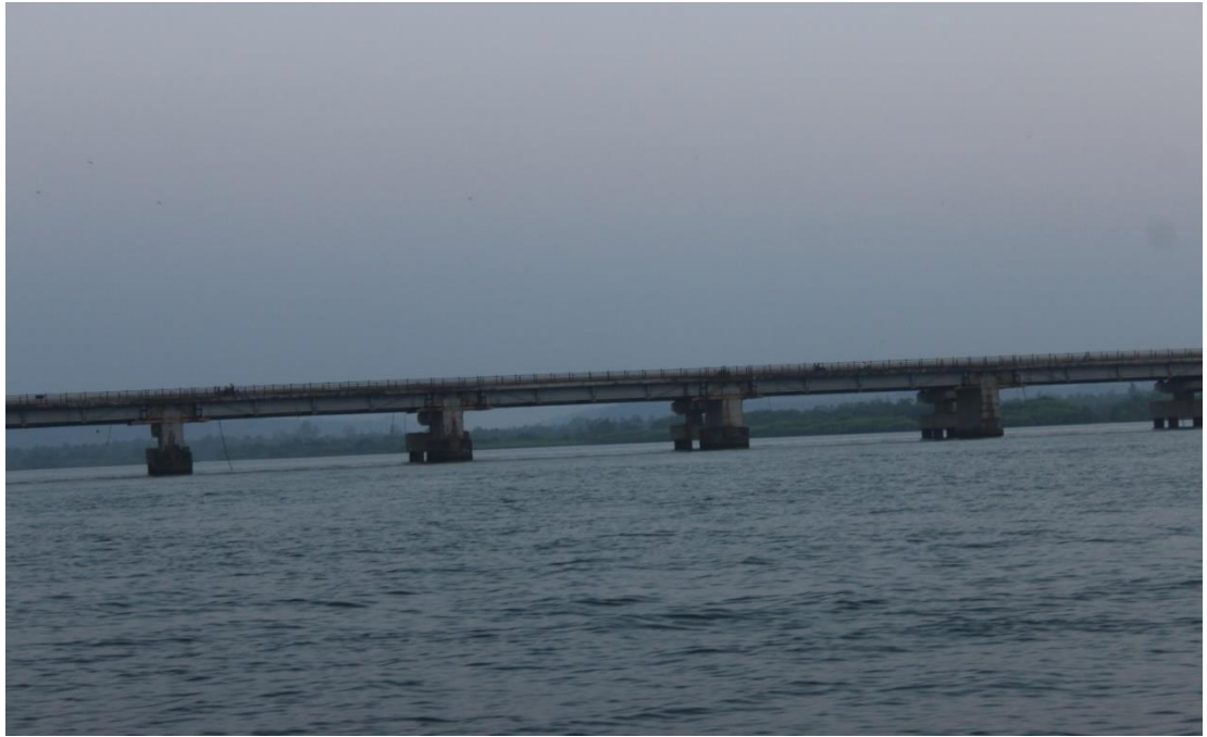
FIGURE 4.8: Edapally-Panvel Highway Bridge on Sharavati River
