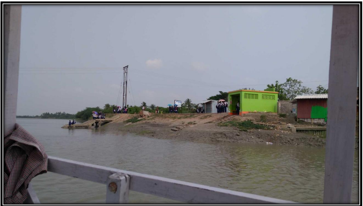
Transmission Line near left bank of river at CHAINAGE 19.5
