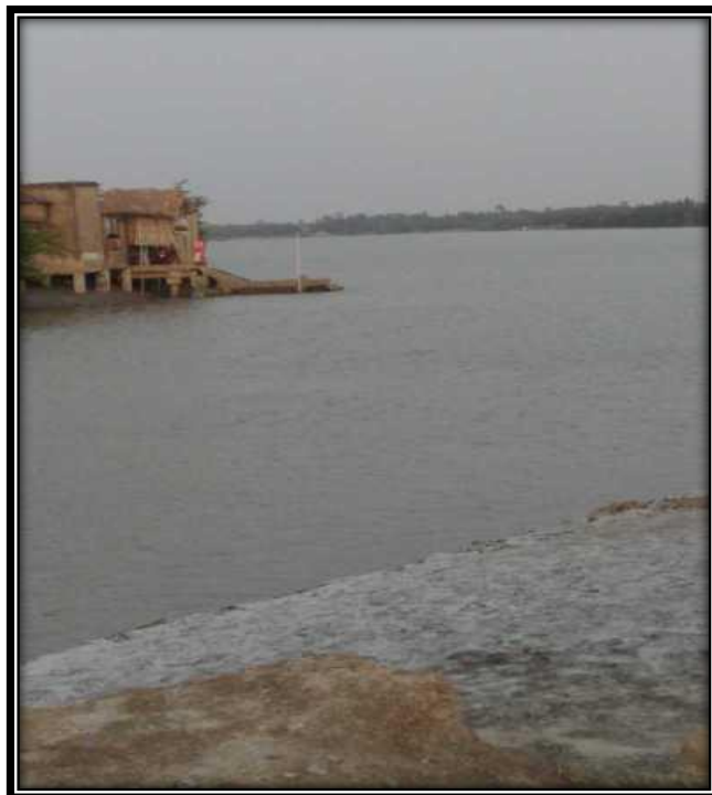
Tide observation on jetty
