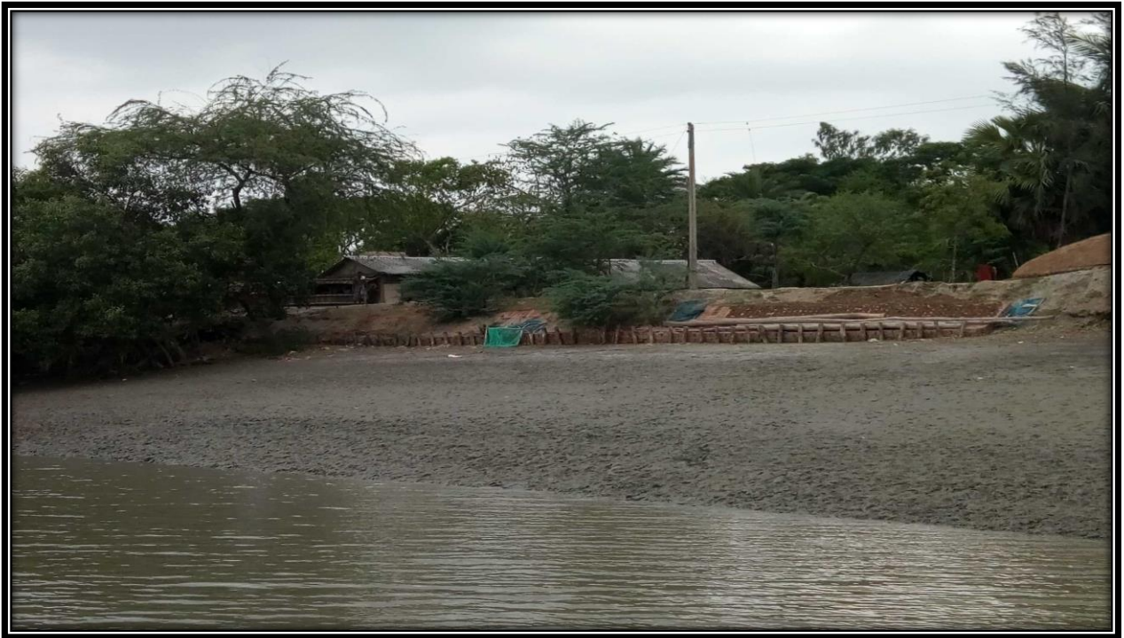
Left bank of river at CHAINAGE 25
