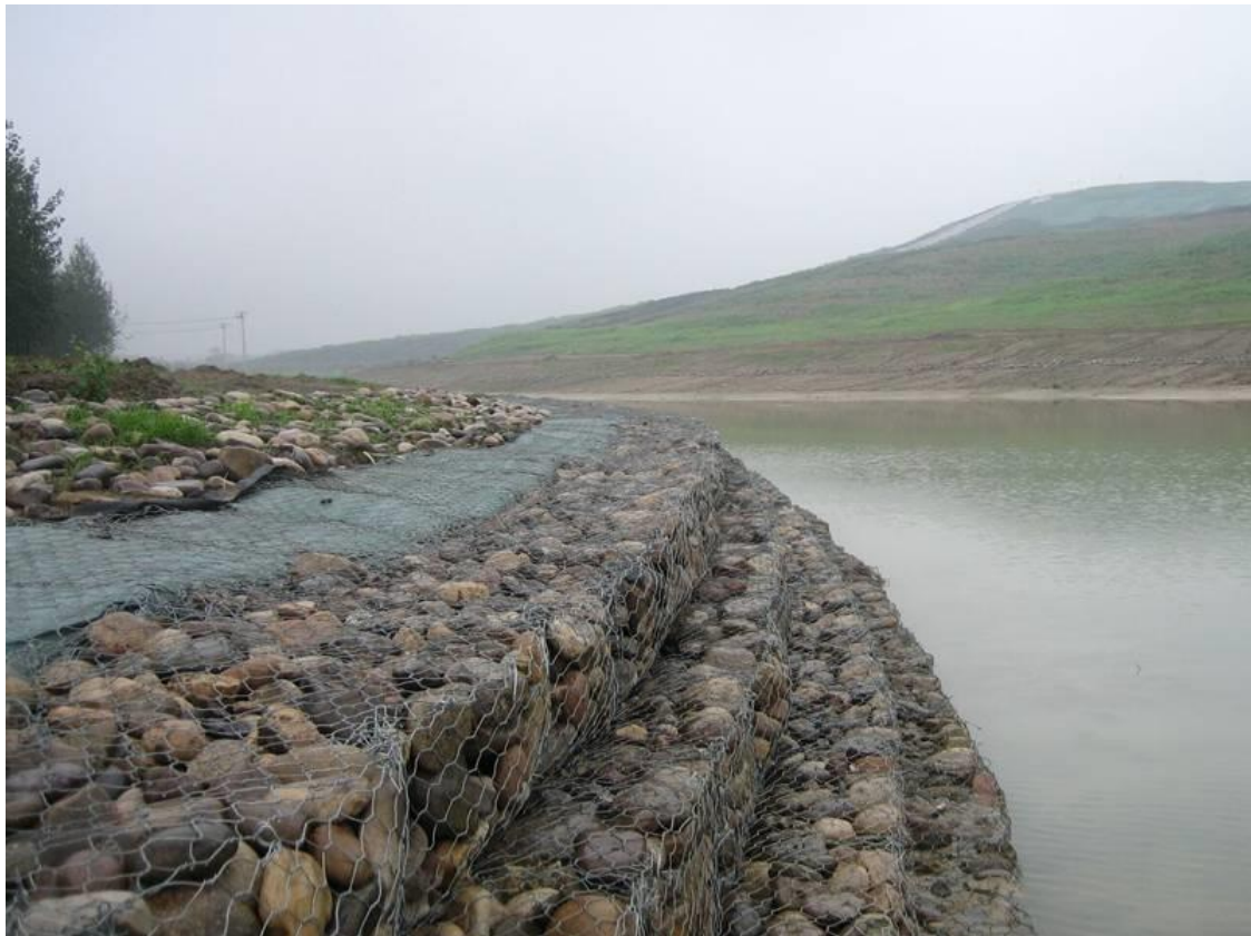
Figure 18: Photograph showing arrangement of Gabion Wall along River Bank
