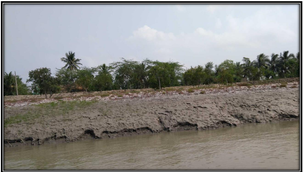
Left Bank of river at CHAINAGE 15.5
