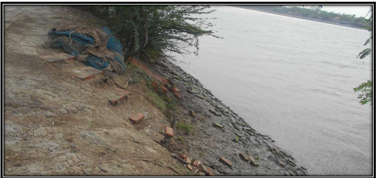
Right Side of River Bank at 23.9 CHAINAGE
