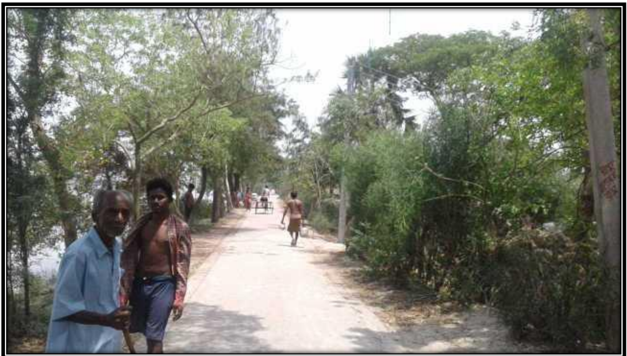
Electric pole & road at 30.7 CHAINAGE
