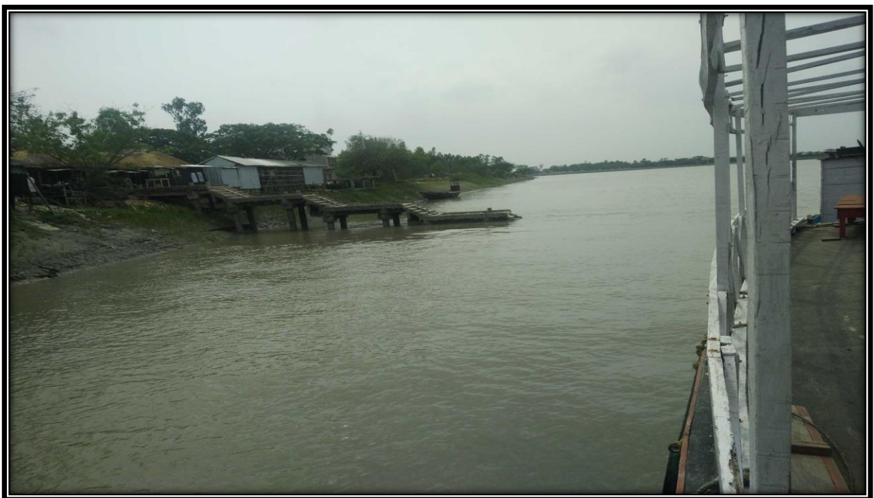
Jetty on right bank of river at CHAINAGE 31.5
