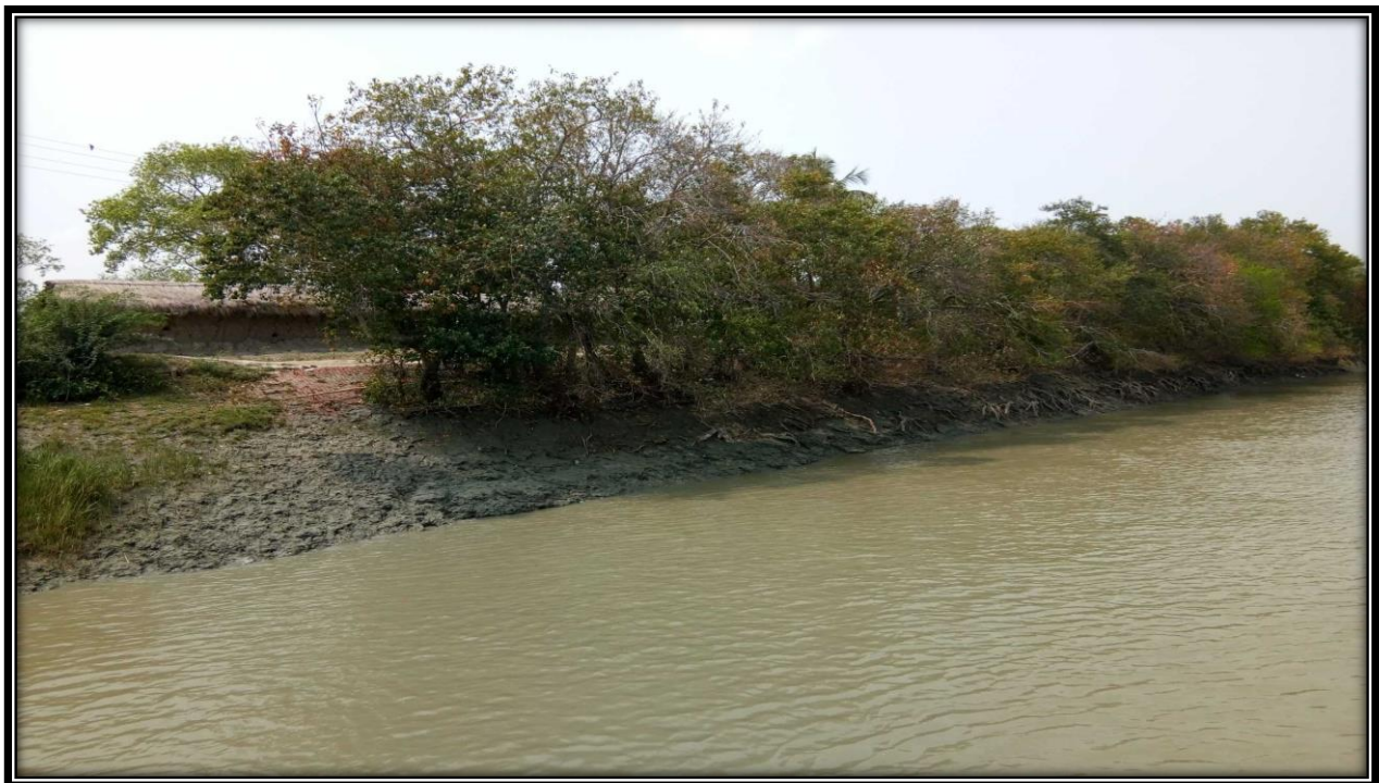
Right bank of river at CHAINAGE 29.5
