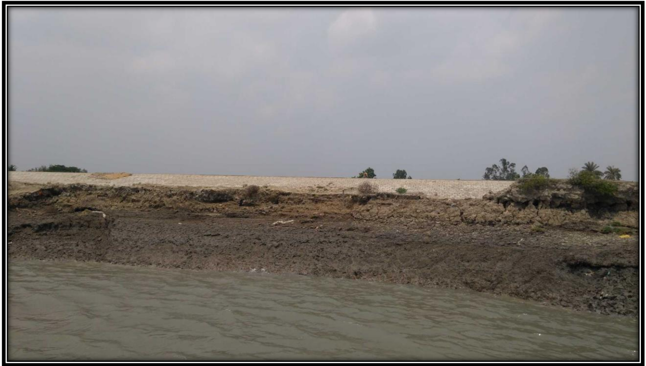
Bank Protection Wall near left bank of river at CHAINAGE 1.5
