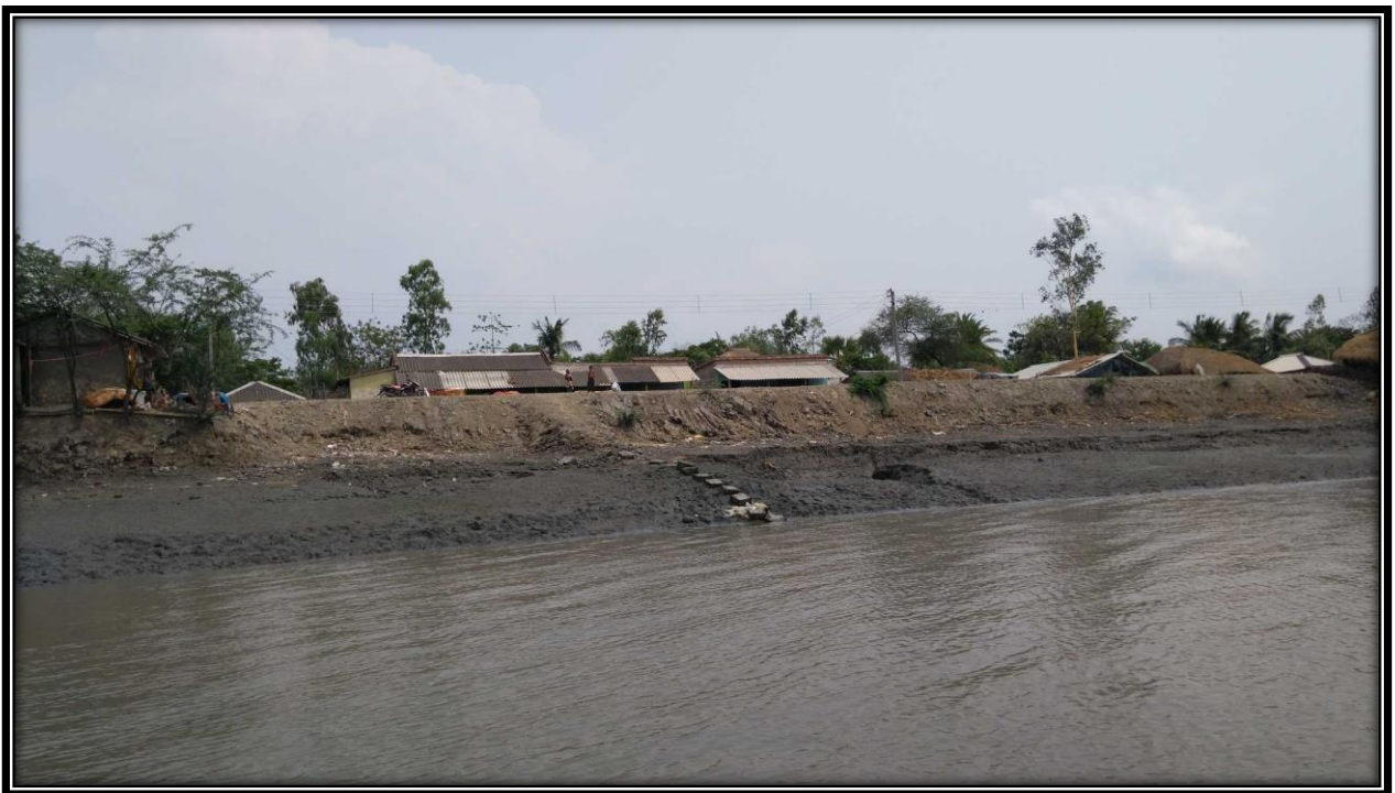
Left Bank of river at CHAINAGE 13
