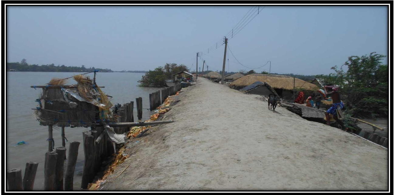
River bank 31.9Chainage Left river bank
