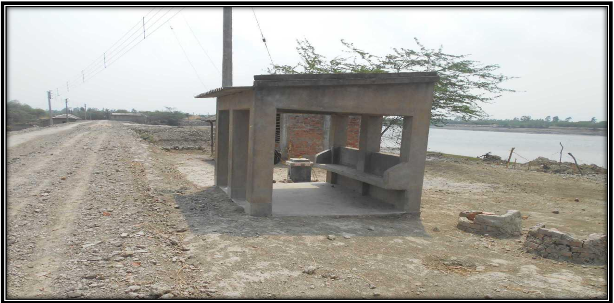
Structure near 13 CHAINAGE of Right Side Of River Bank
