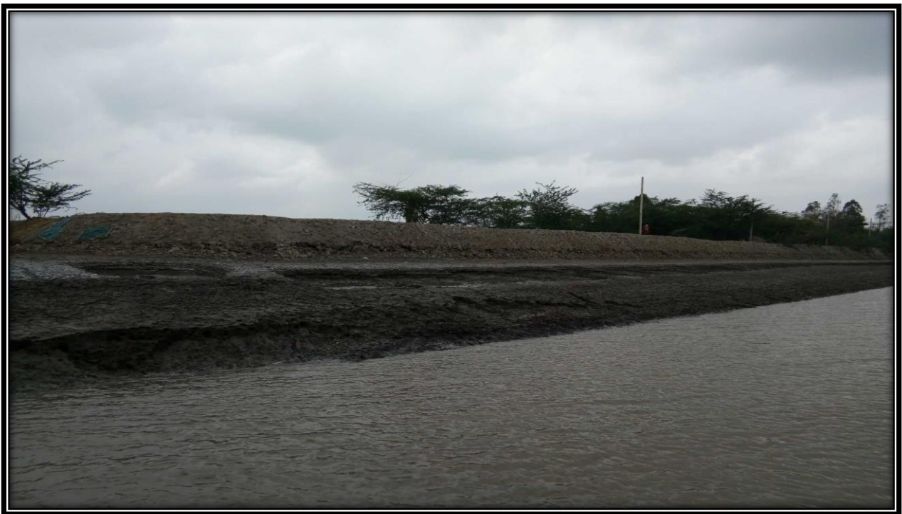
Left bank of river at CHAINAGE 23.5
