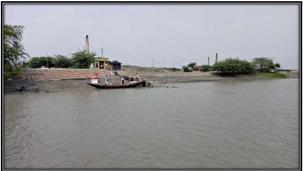
Jetty on right bank of river at CHAINAGE 35
