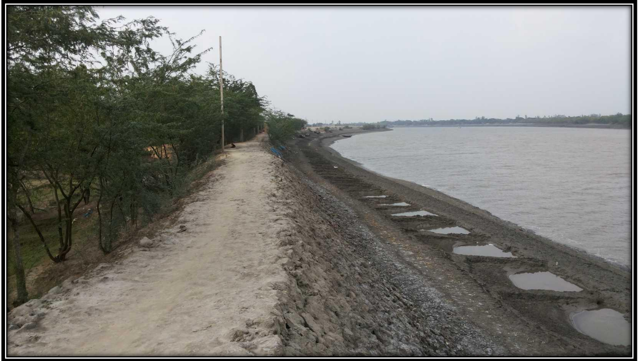
River Bank near 23.5 CHAINAGE of Left Side Of River Bank
