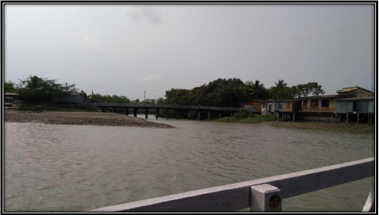
Concrete bridge near right bank of river at 19.5 CHAINAGE
