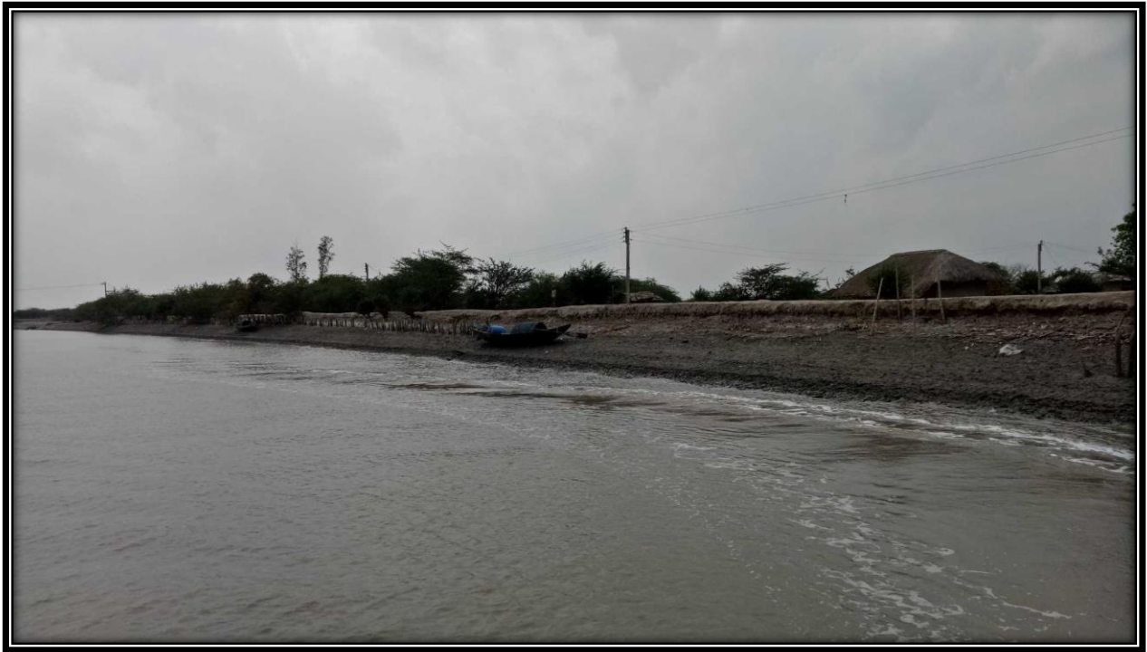
Electric pole near right bank of river at CHAINAGE 33.5
