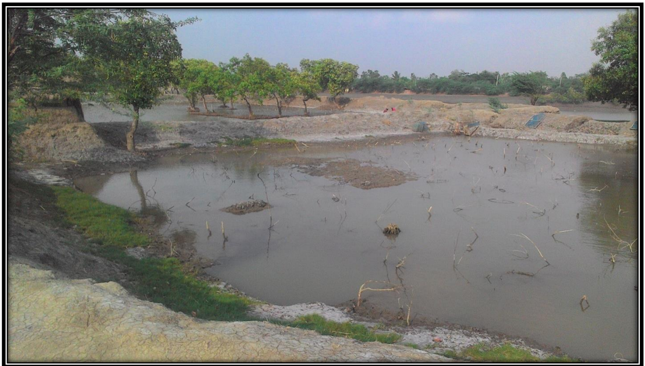
River Bank near 27 CHAINAGE of Left Side of River Bank
