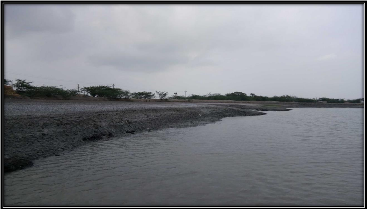
Left bank of river at CHAINAGE 26.5
