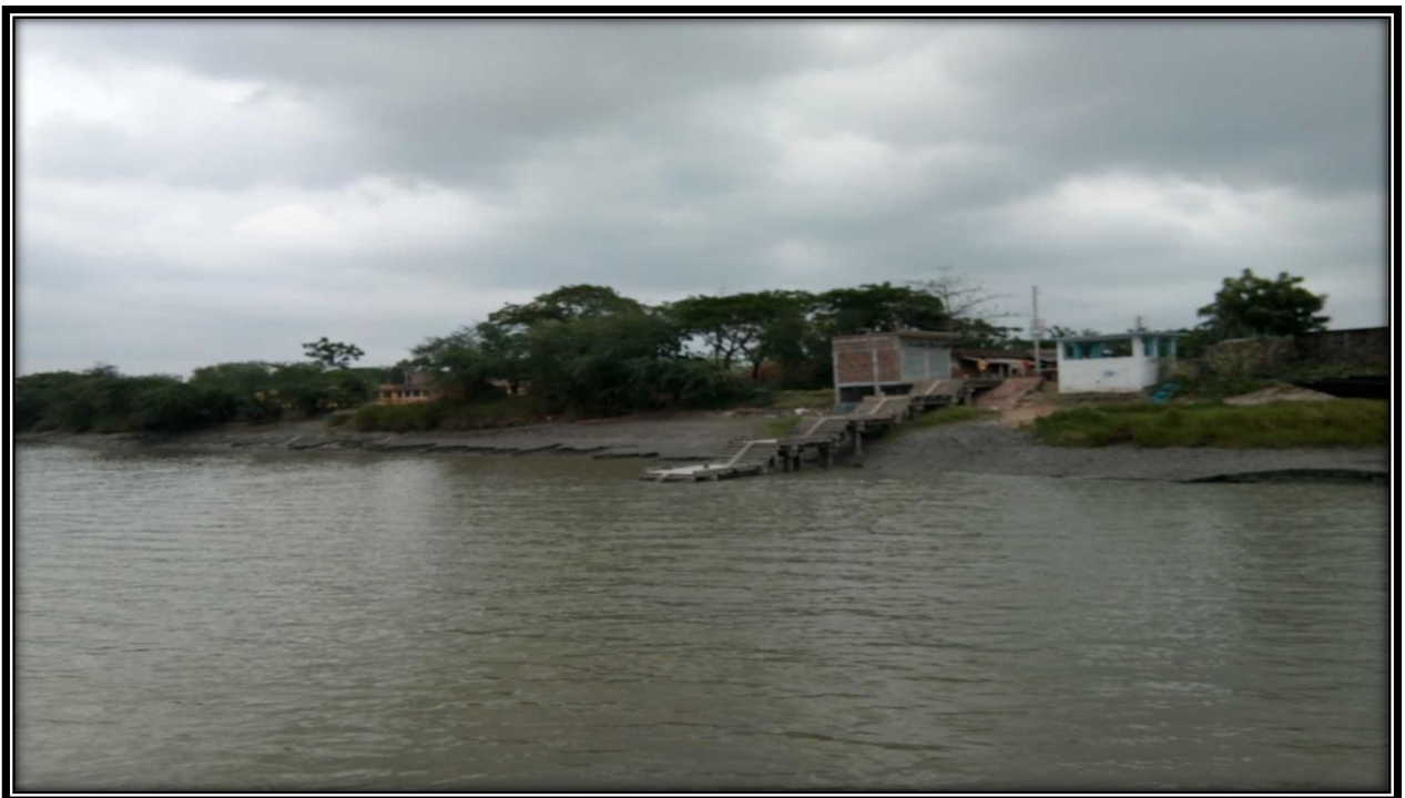
Jetty on left bank of river at CHAINAGE 23
