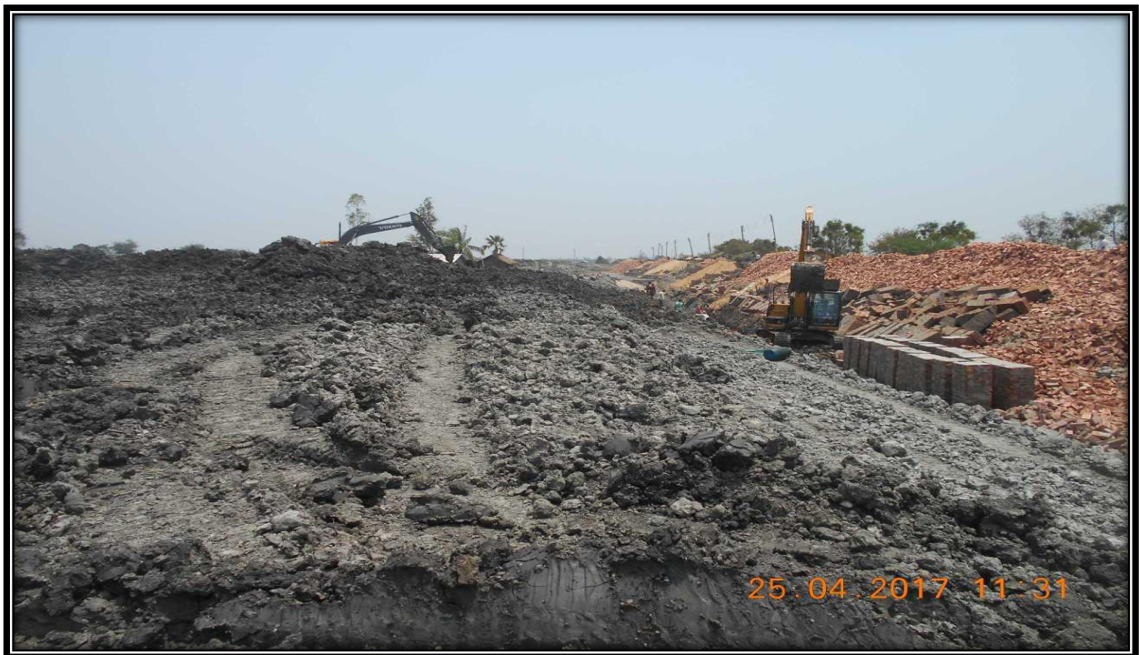
River bank protection construction at 30.8Chainage Left river bank
