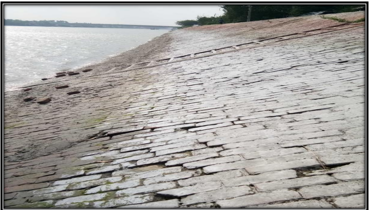
Left Side River Bank at CHAINAGE 4.8
