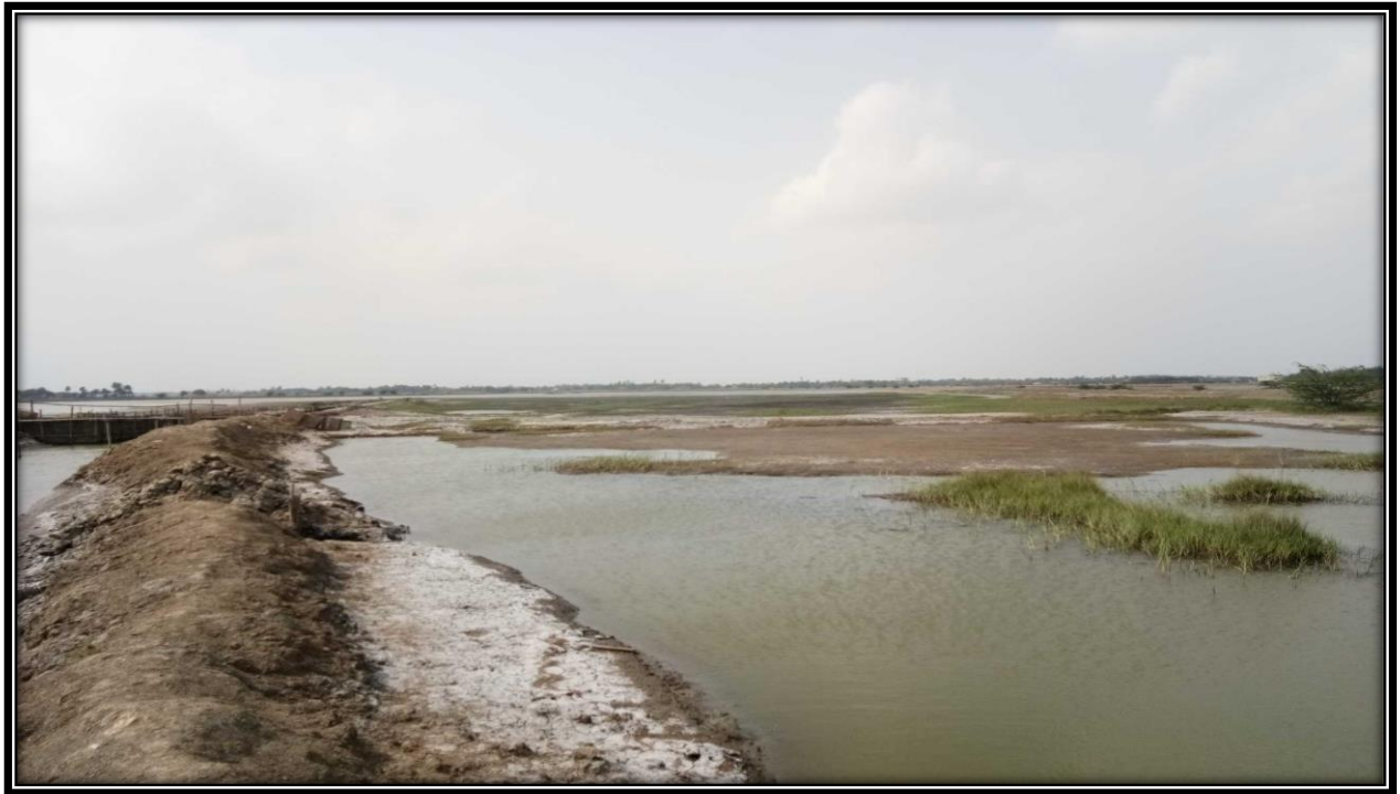
Pond near Left Bank of river at CHAINAGE 7.3
