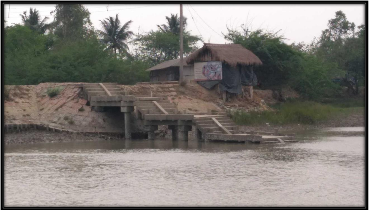
Jetty on right bank of river at CHAINAGE 6
