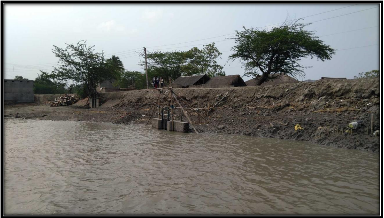
Water Lock on right bank of river at CHAINAGE 19.5
