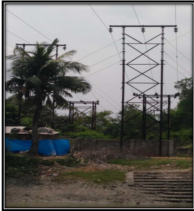
High Tension Line near right bank of river at CHAINAGE 4
