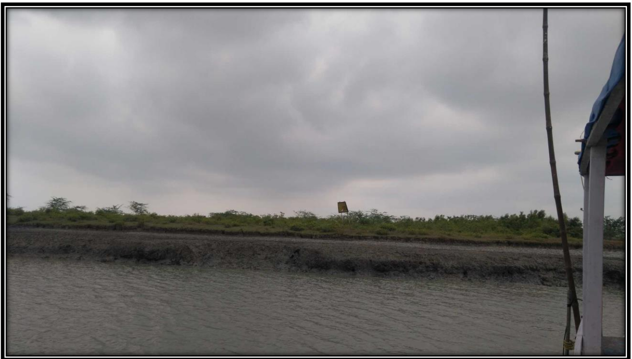
Right bank of river at CHAINAGE 6.5
