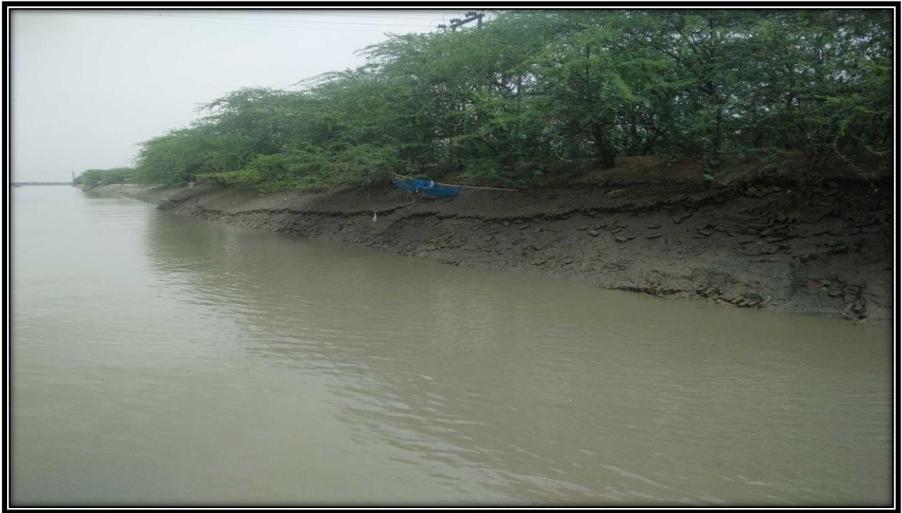
Right bank of river at CHAINAGE 32.5
