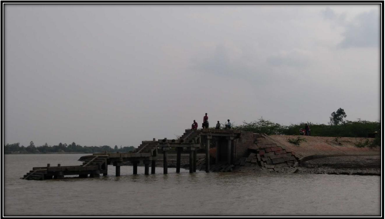
Jetty on left bank at CHAINAGE 21
