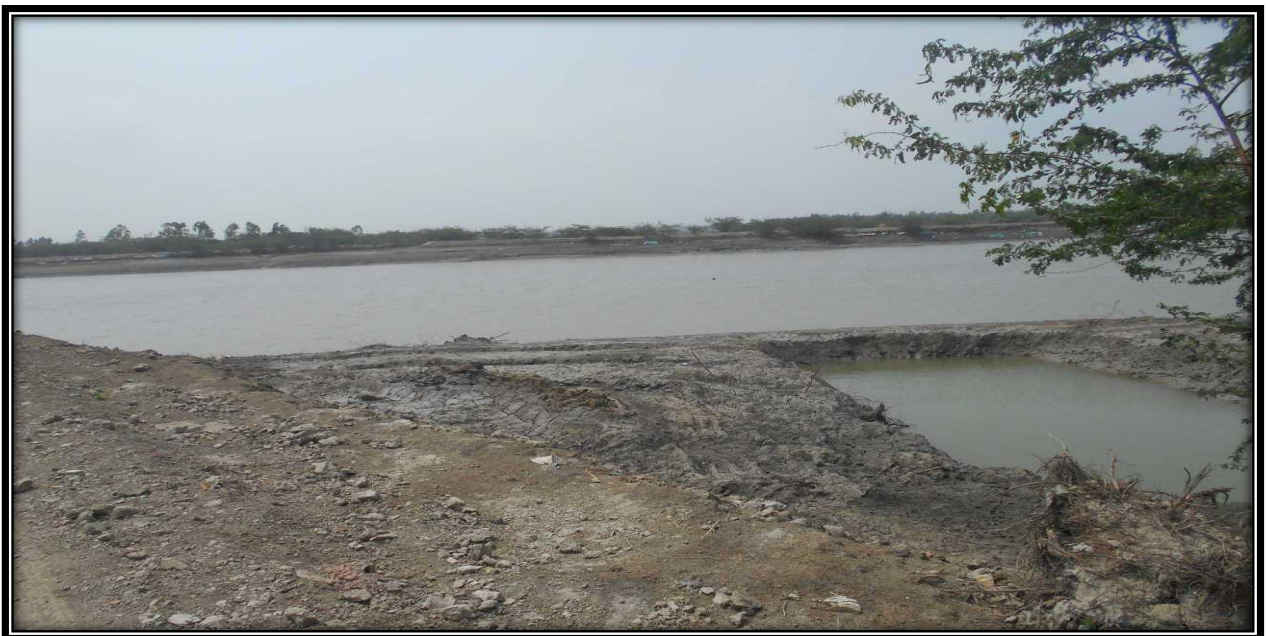
River Bank near 12.5 CHAINAGE of Right Side Of River Bank
