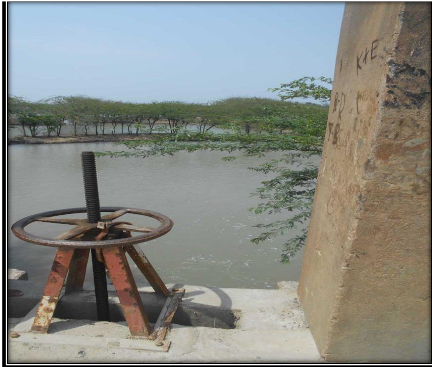
Water lock at 32.8 Chainage Left river bank
