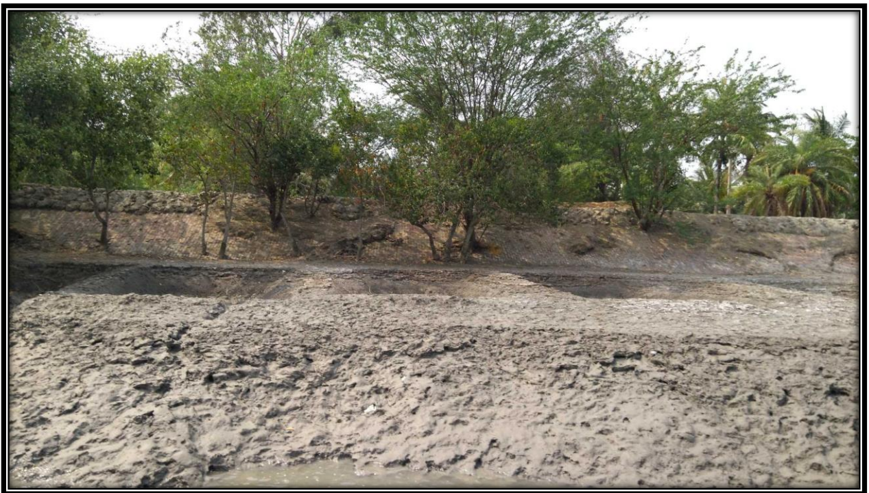
Right Bank of river at CHAINAGE 16.5
