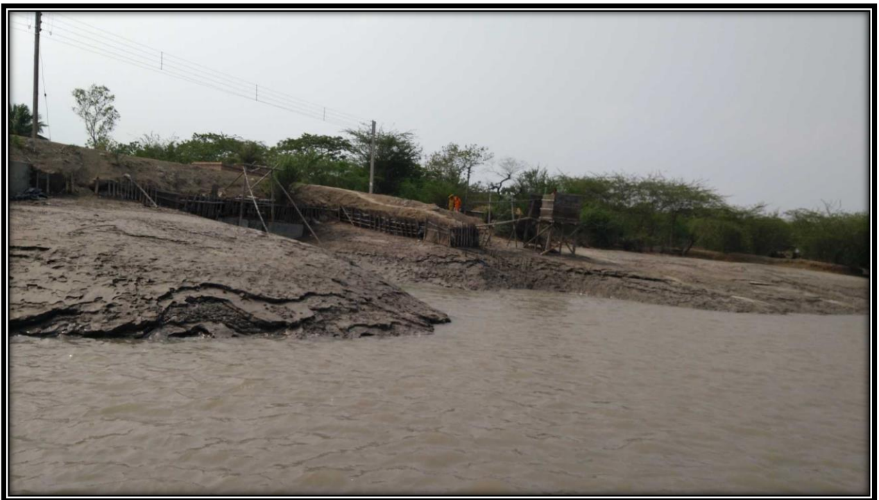
Bank protection wall near left bank of river at CHAINAGE 20
