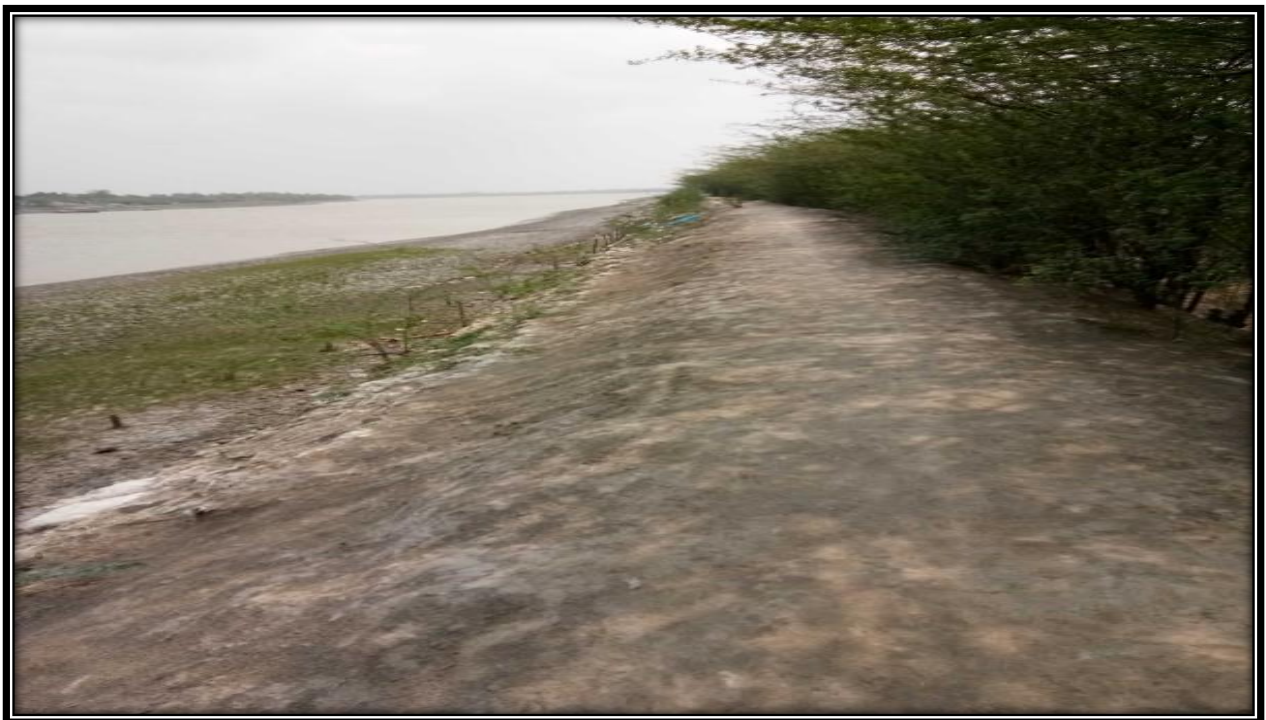
River Bank-11.8 CHAINAGE Left Bank
