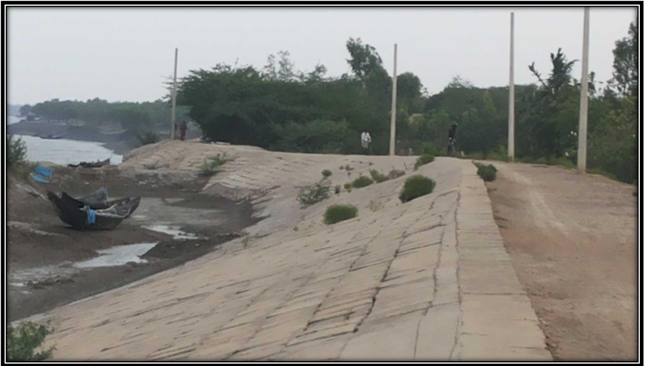
River Bank Protection near 24 CHAINAGE of Left Side Of River Bank
