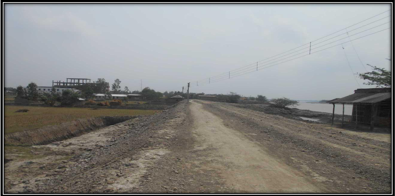
Road near 13 CHAINAGE Of right Side of River Bank
