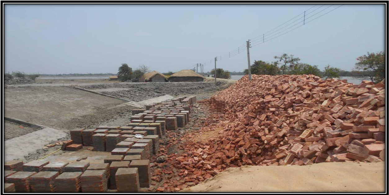
River bank protection construction at 31Chainage Left river bank
