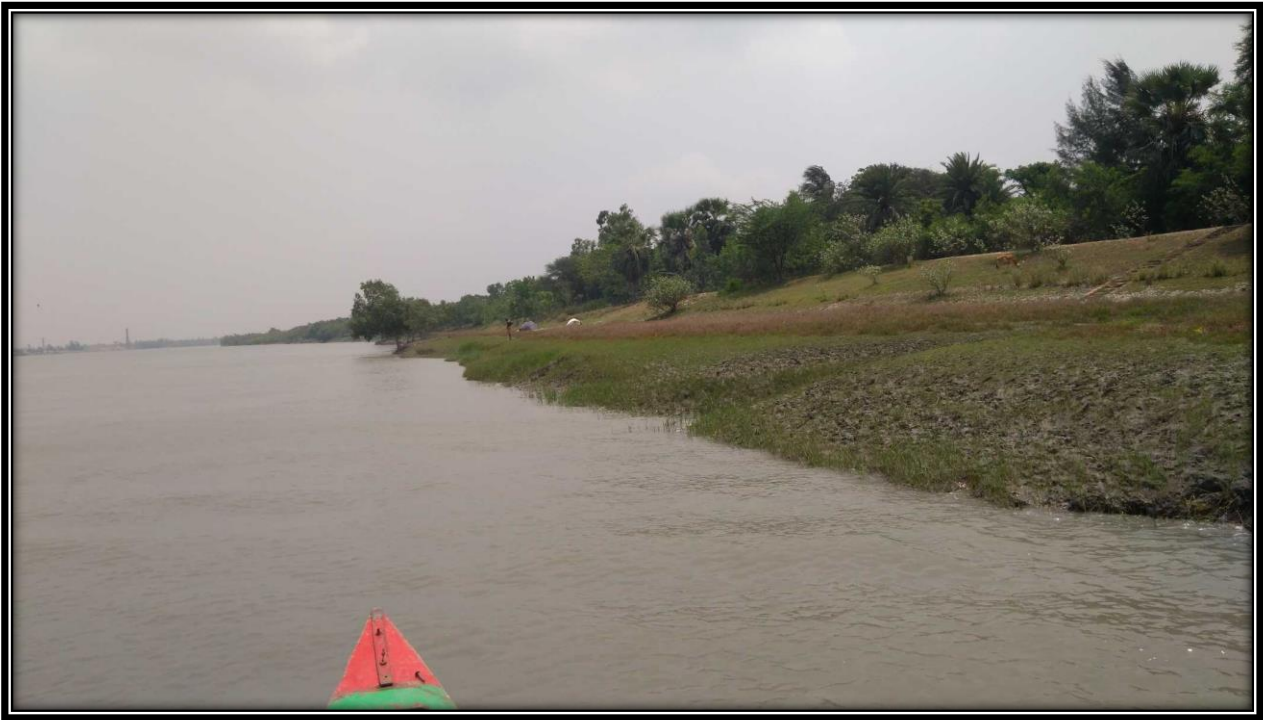
Bank protection wall near right bank of river at CHAINAGE 0.5
