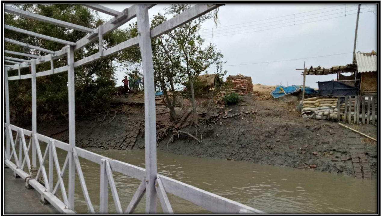
Right bank of river at CHAINAGE 31.5
