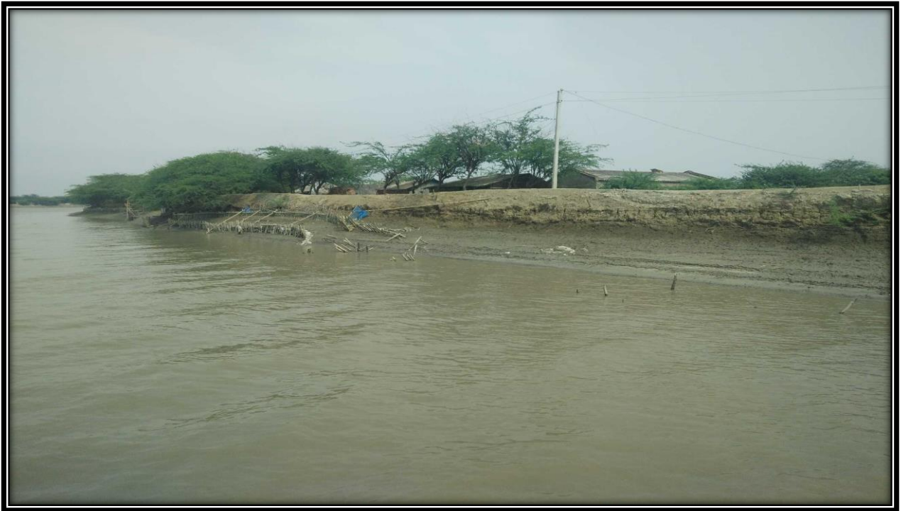
Right bank of river at CHAINAGE 36
