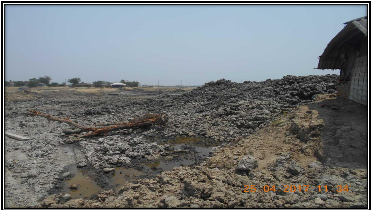
River bank protection construction at 30.9Chainage Left river bank
