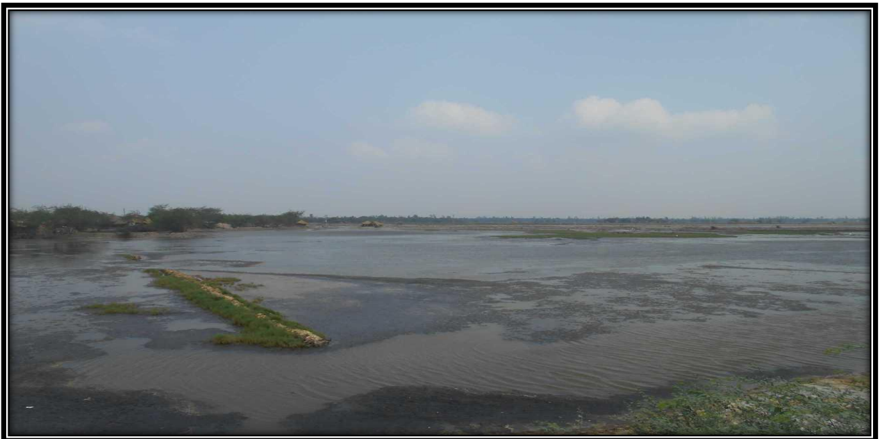
Pond Ahead Near Right Side of River Bank at 24.5 CHAINAGE
