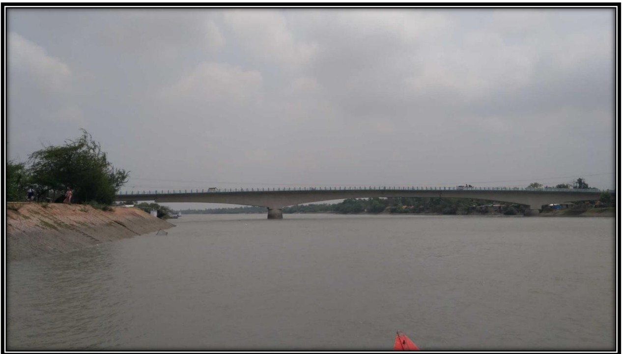
Basanti Bridge at CHAINAGE 4
