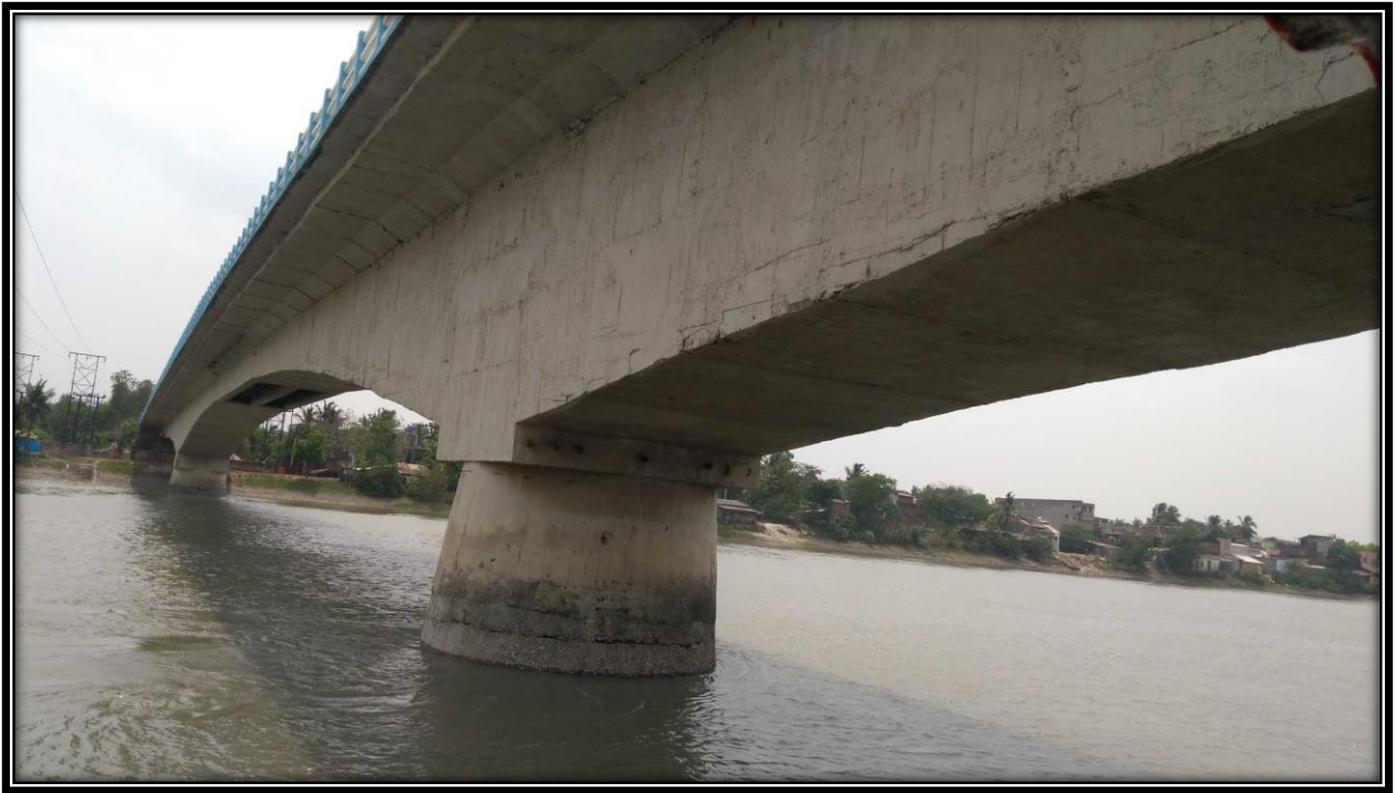
Basanti Bridge at CHAINAGE 4
