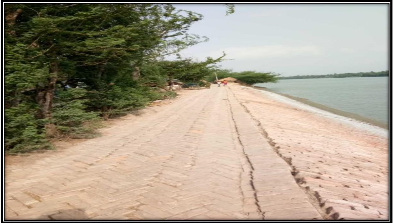
Left Bank at CHAINAGE 4.7
