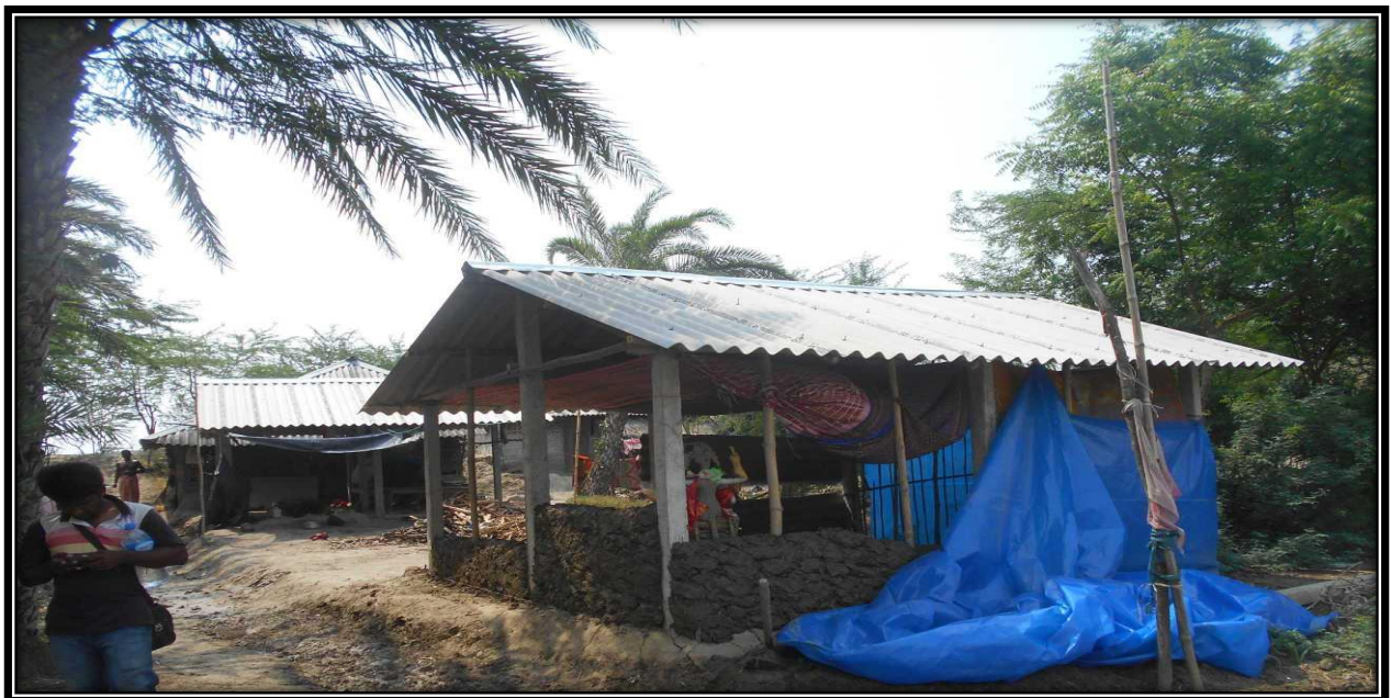
Structure near river bank at CHAINAGE 25
