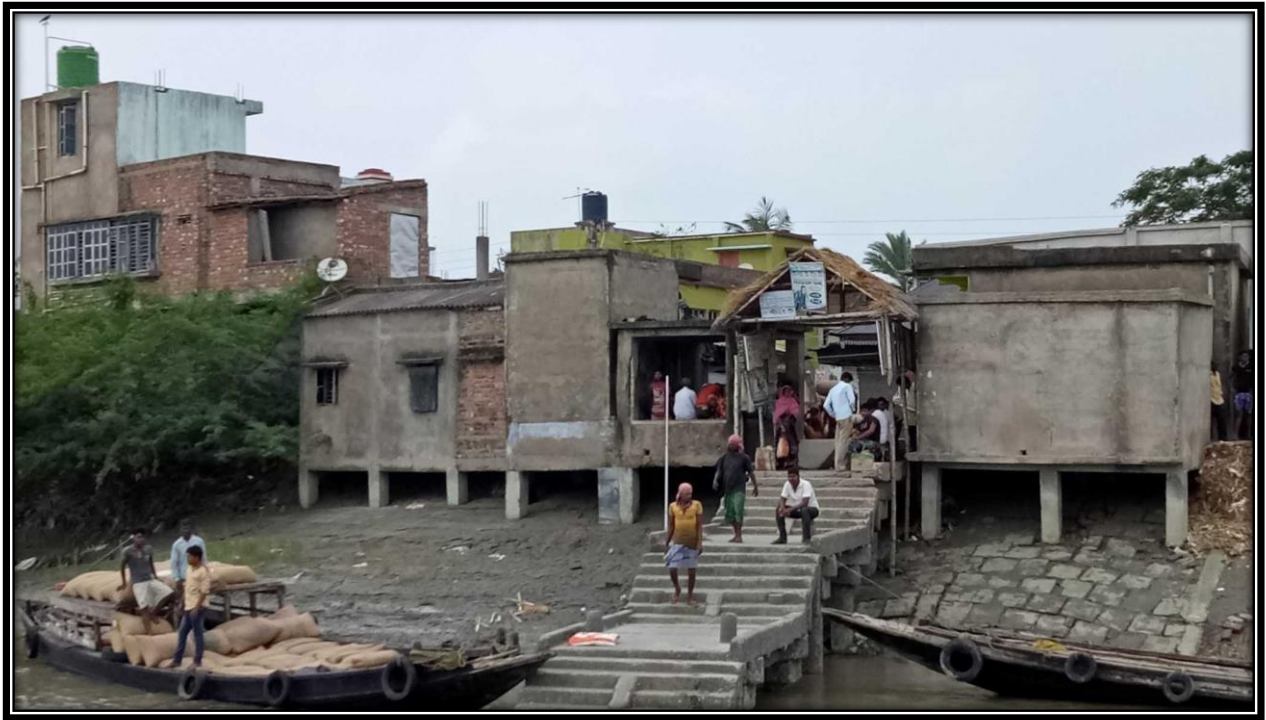
Jetty on left bank of river at CHAINAGE 31
