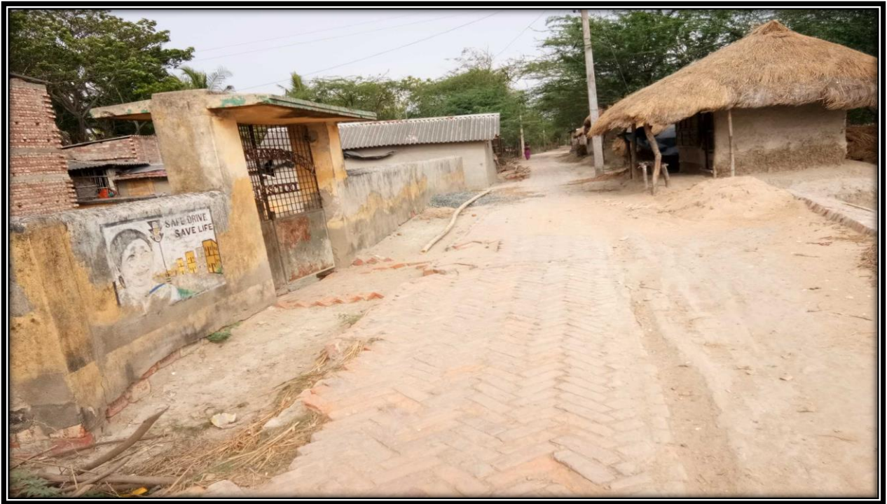
Structure at CHAINAGE 4.8
