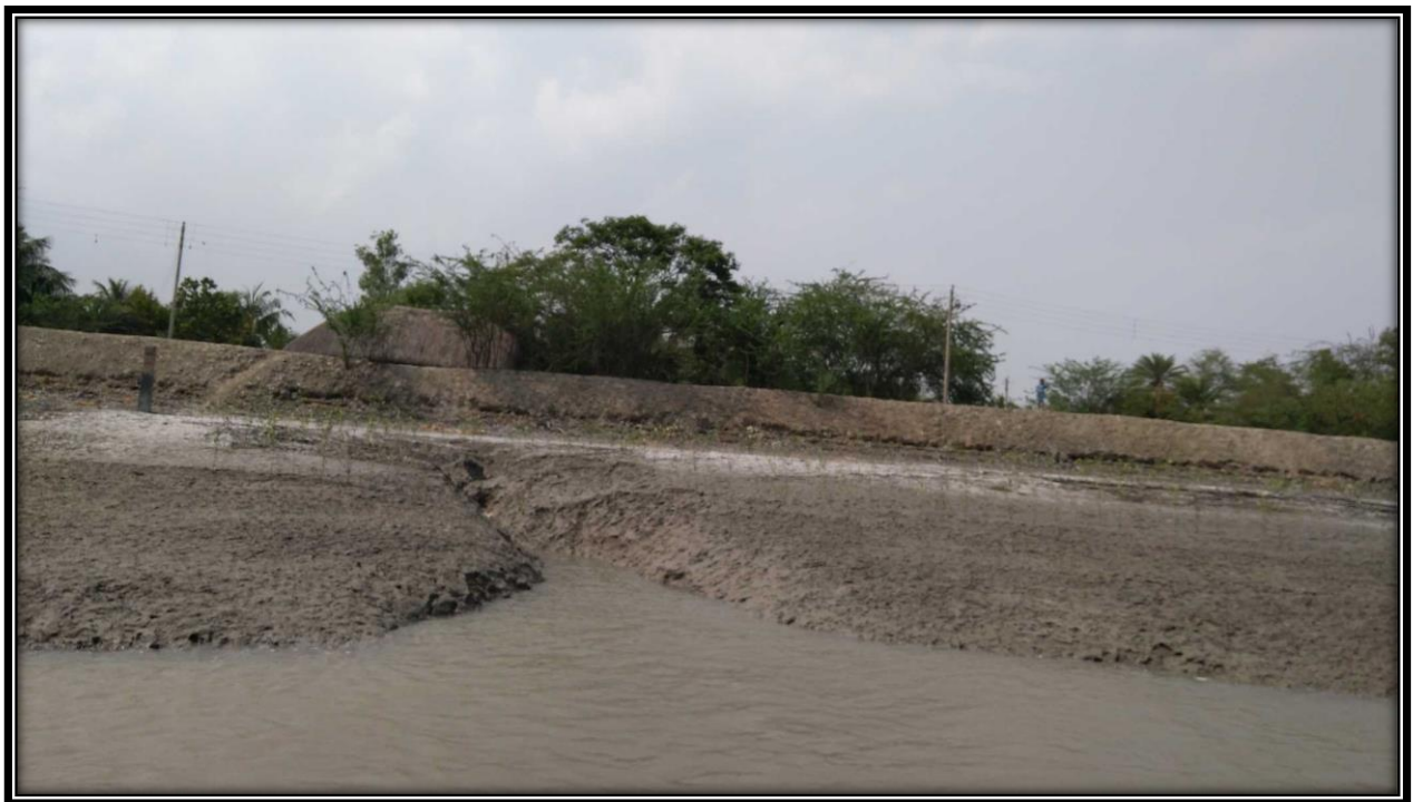
Right Bank of river at CHAINAGE 16
