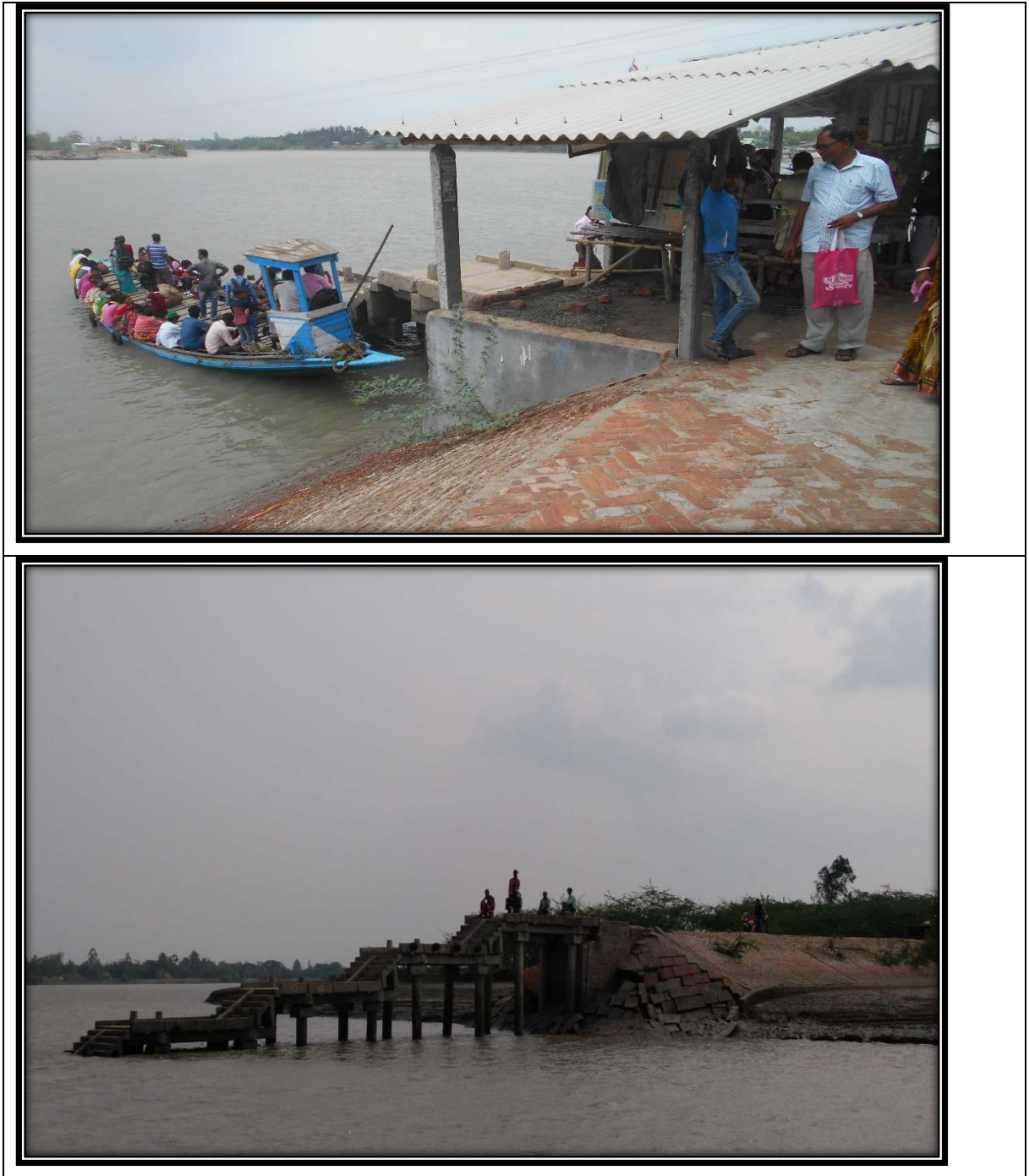
Figure 26: Photographs of Jettiy located along Hogla Waterway
