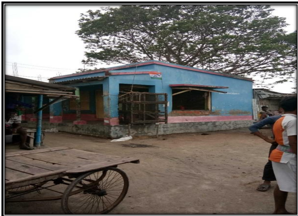
Structure at 19.5 CHAINAGE
