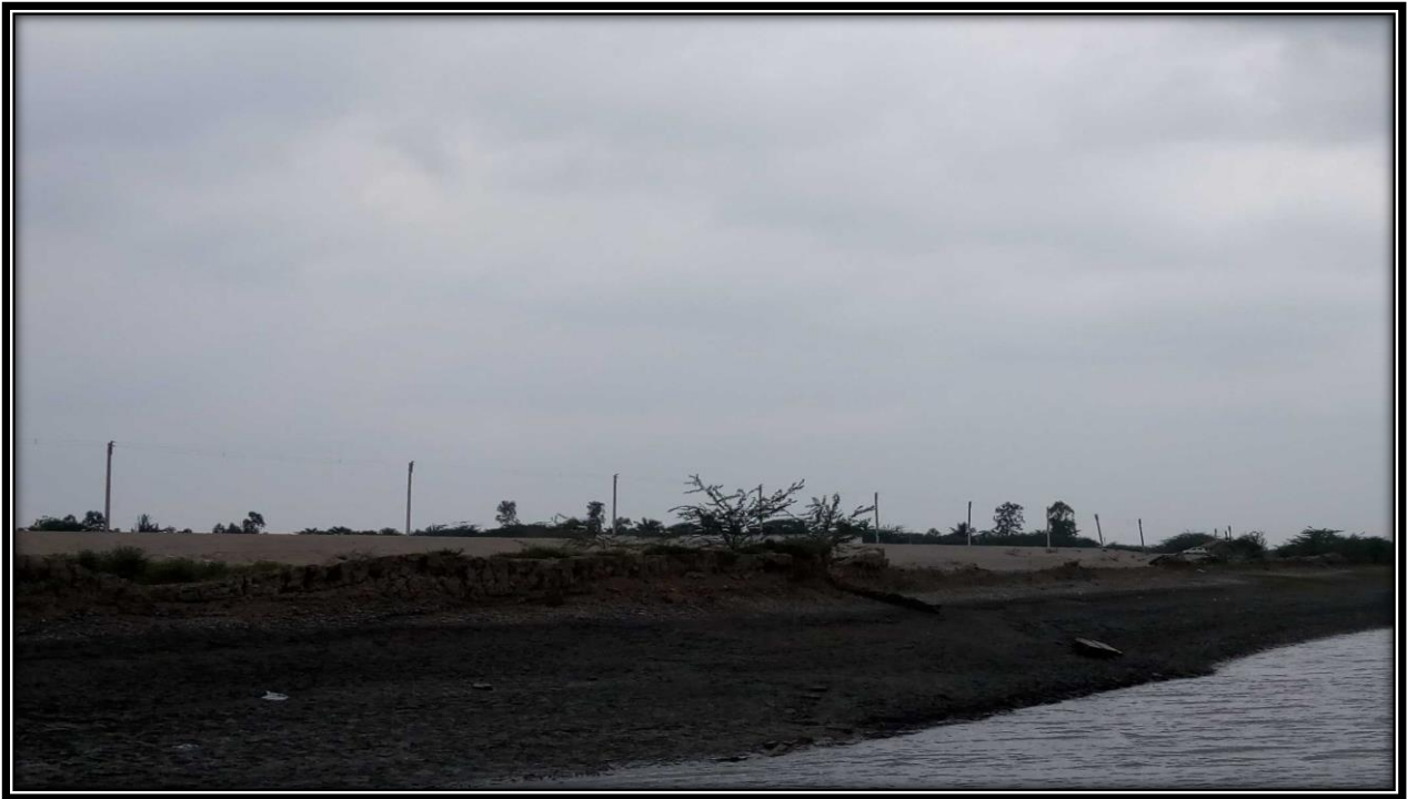
Right bank of river at CHAINAGE 24.5
