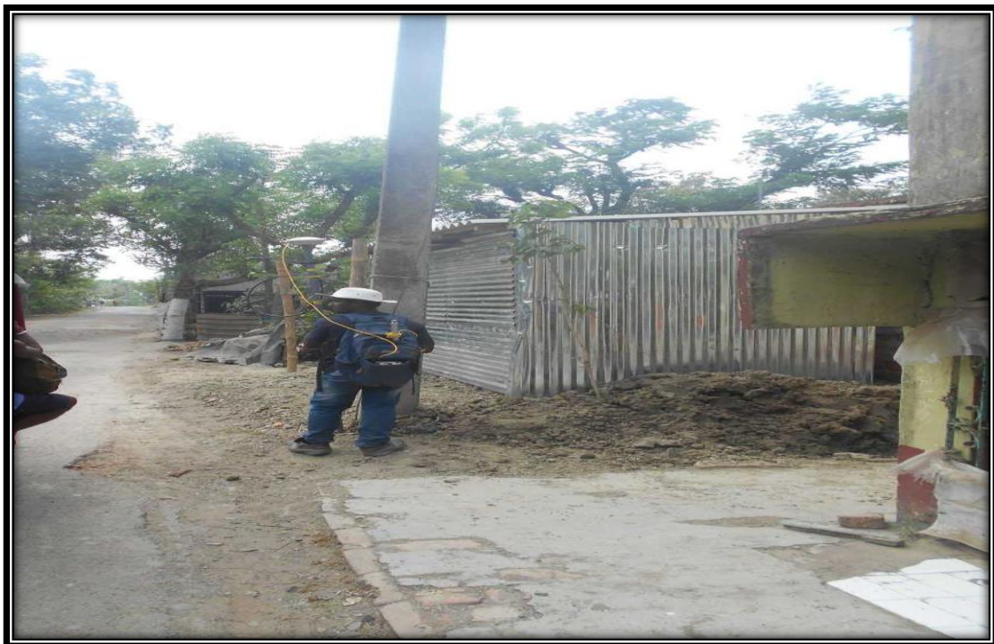
Structure near 2.5 CHAINAGE of Right Side of River Bank
