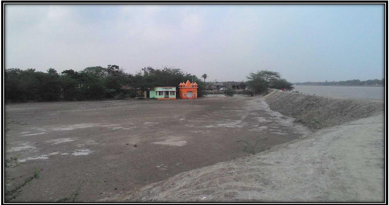
Temple near 22.5 CHAINAGE of Left Side Of River Bank
