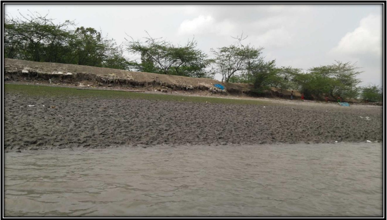
Right Bank of river at CHAINAGE 12.5
