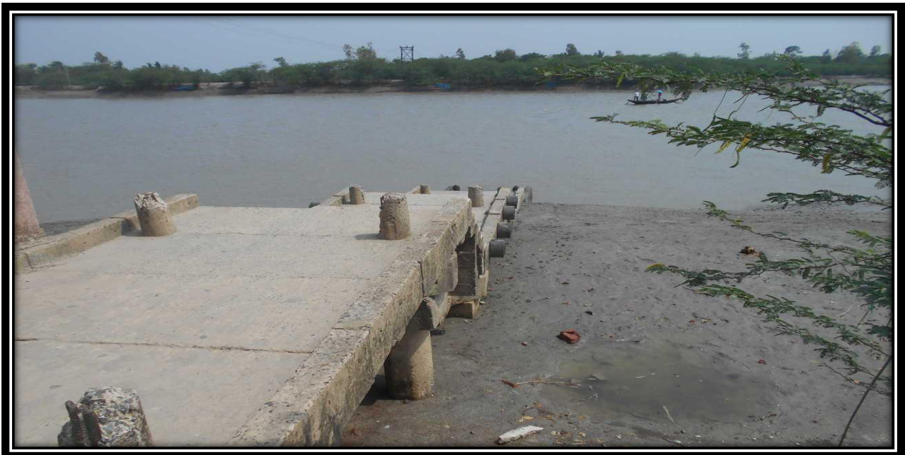
Sakhali ferry ghat at 32 Chainage-Left river bank
