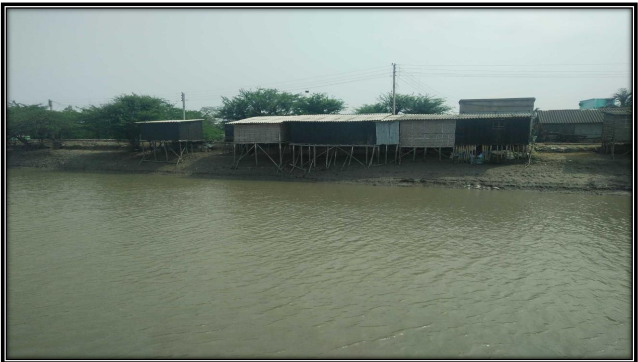
Right bank of river at CHAINAGE 35.5
