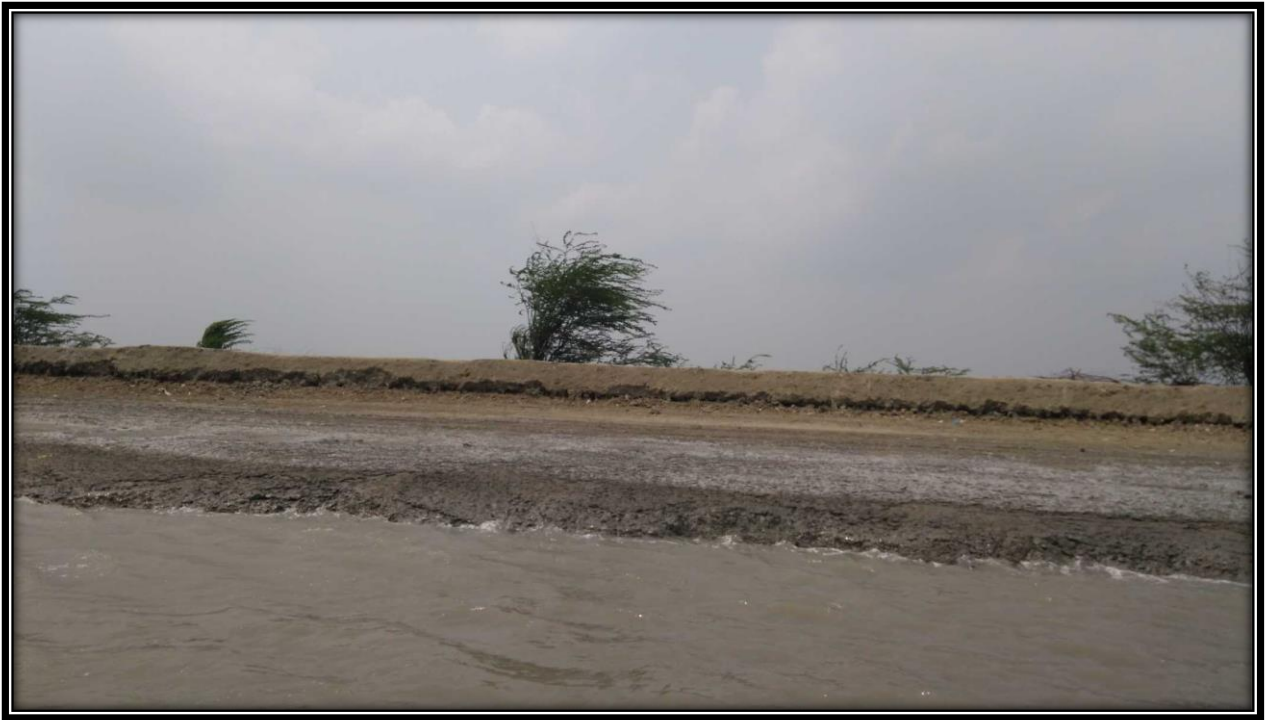
Left bank of river at CHAINAGE 6
