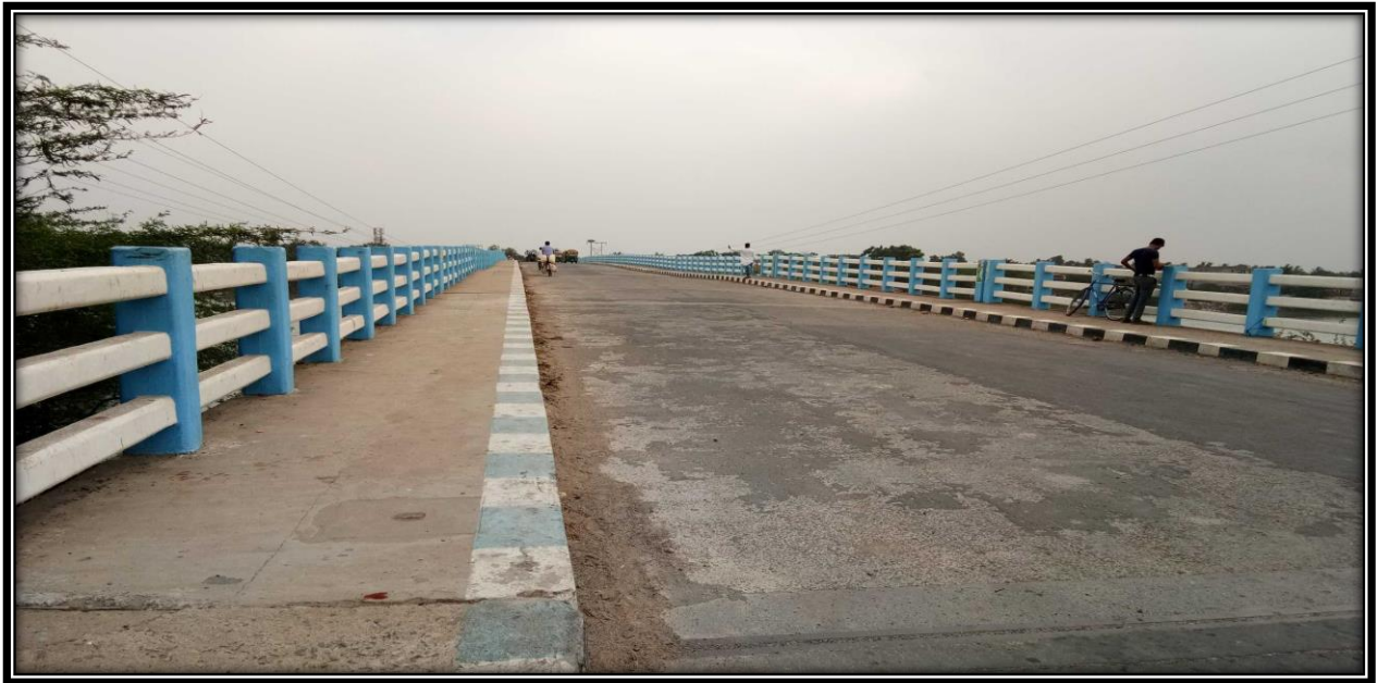
Bridge at CHAINAGE 4.1
