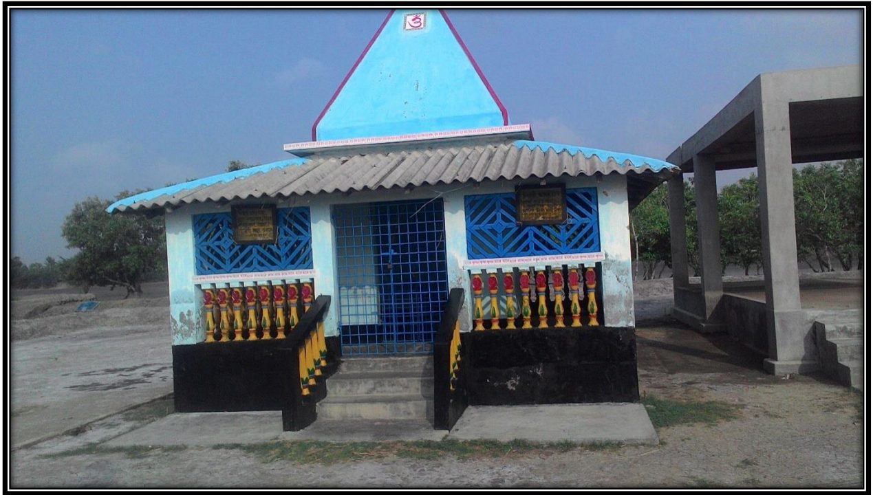
Temple near 27 CHAINAGE of Left Side of River Bank
