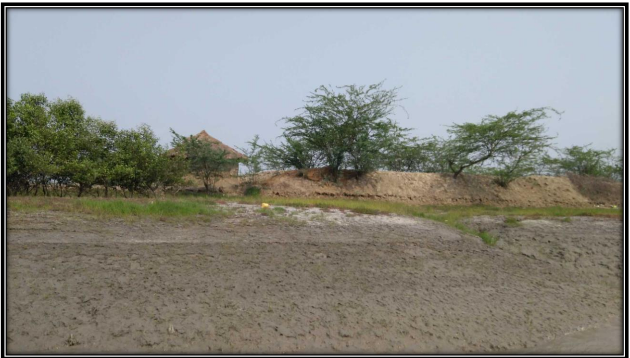
Left Bank of river at CHAINAGE 17.5
