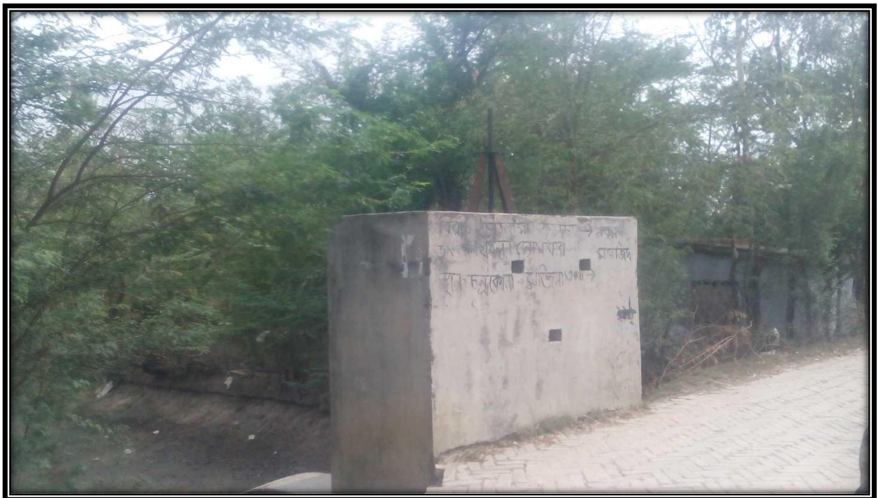
Water Lock CHAINAGE-5.9
