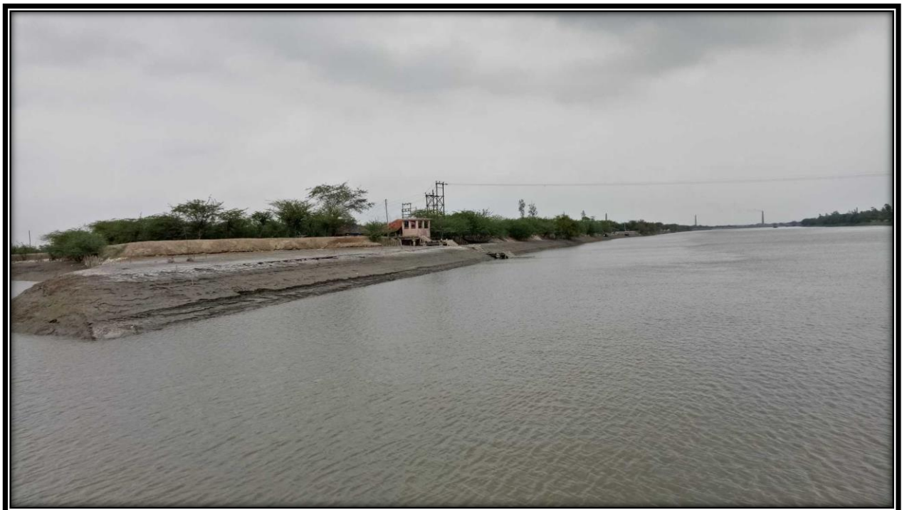
Jetty bank of river at CHAINAGE 32.5
