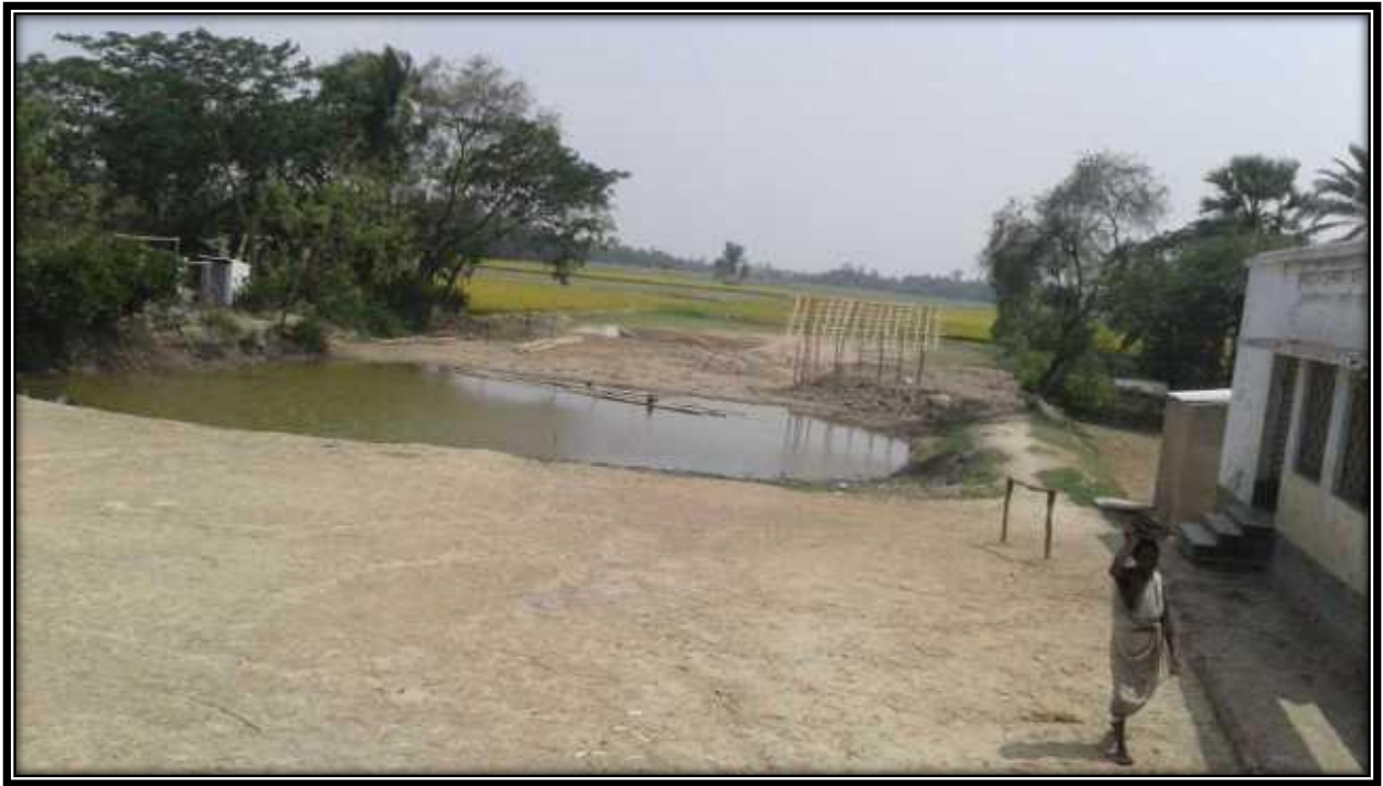
Pond at 31.7 CHAINAGE of right side of river bank
