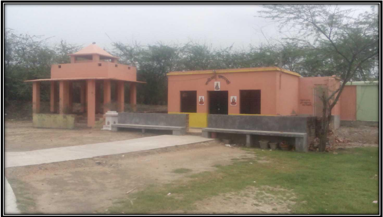
Structure at CHAINAGE 4.5
