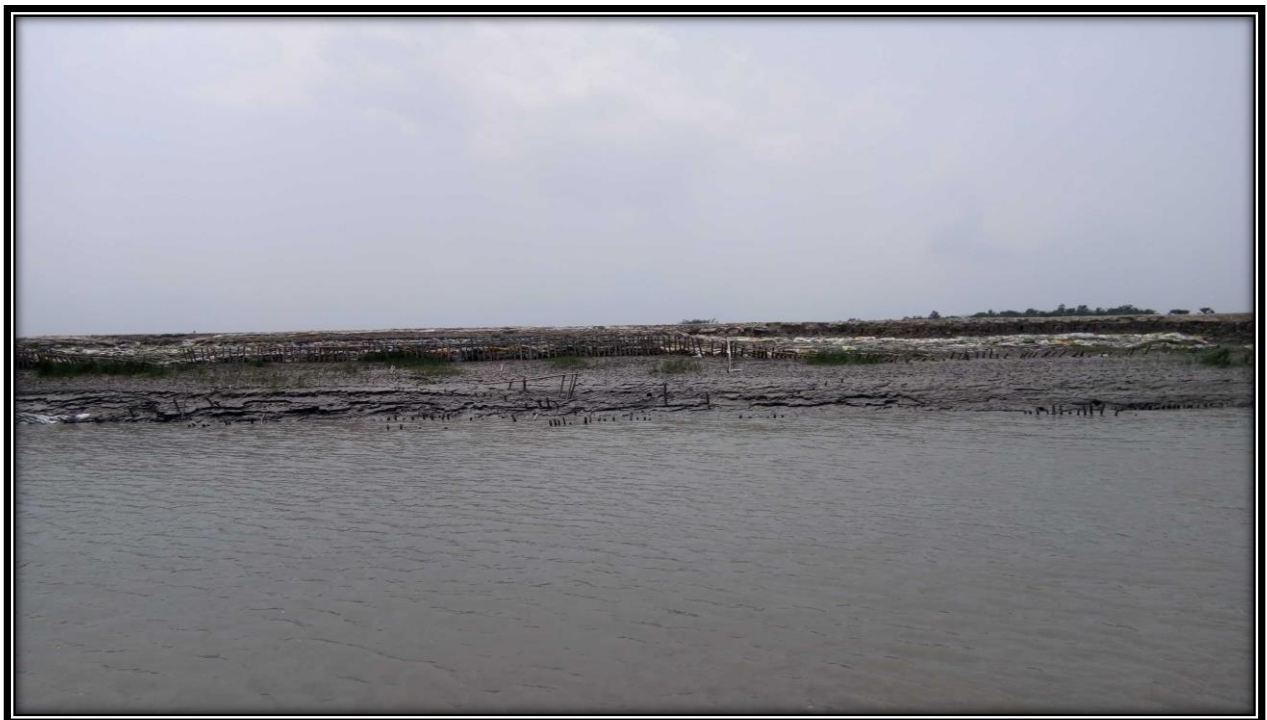
Left bank of river at CHAINAGE 28.5
