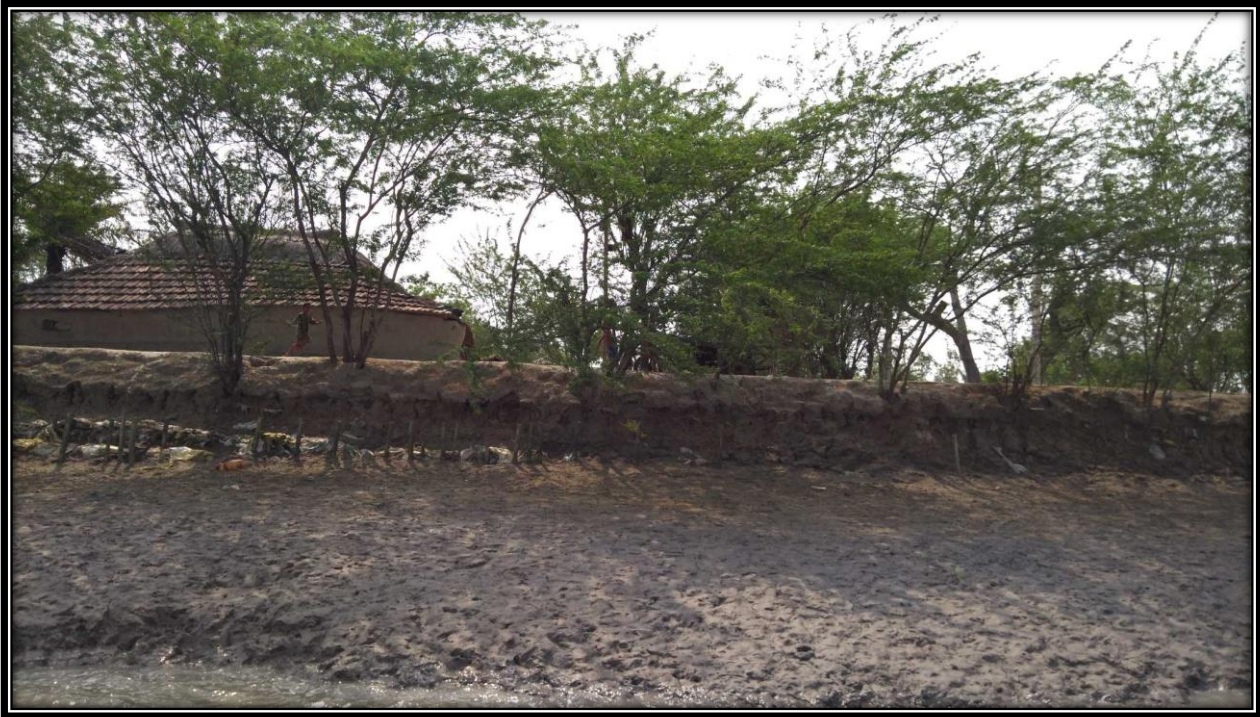
Left Bank of river at CHAINAGE 18
