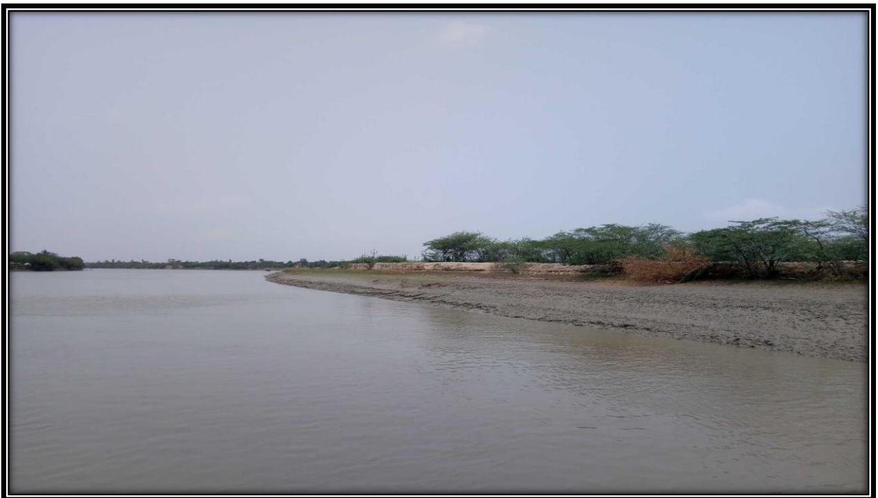
Left bank of river at CHAINAGE 29
