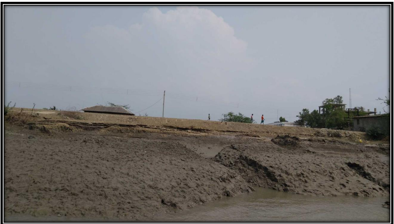
Right Bank of river at CHAINAGE 13
