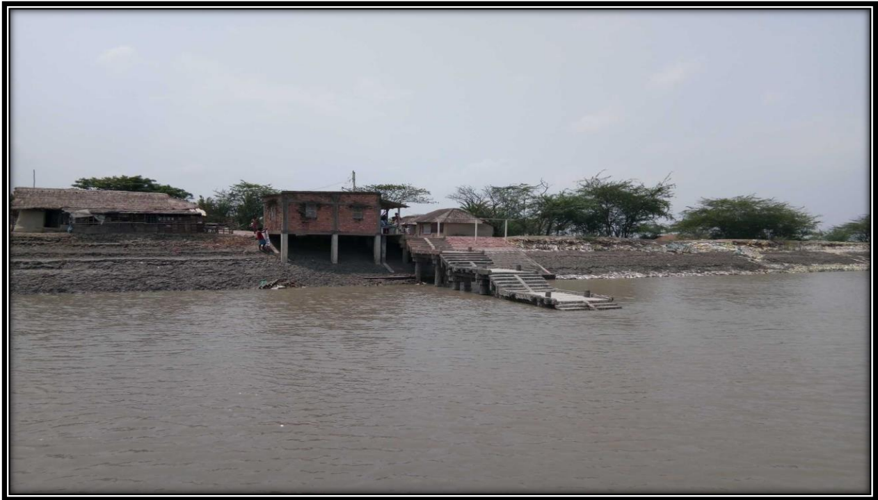
Jetty on right bank of river at CHAINAGE 28
