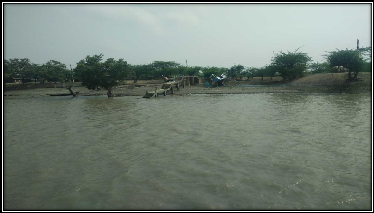
Jetty on right bank of river at CHAINAGE 37
