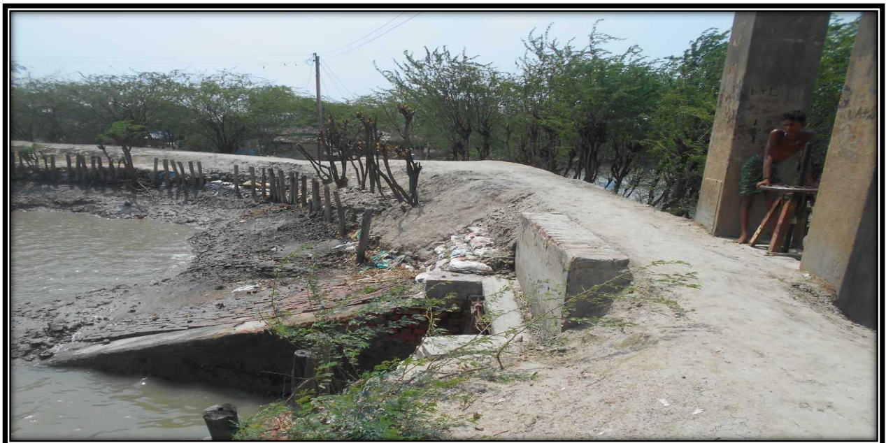
Water lock at 32.8 Chainage Left river bank
