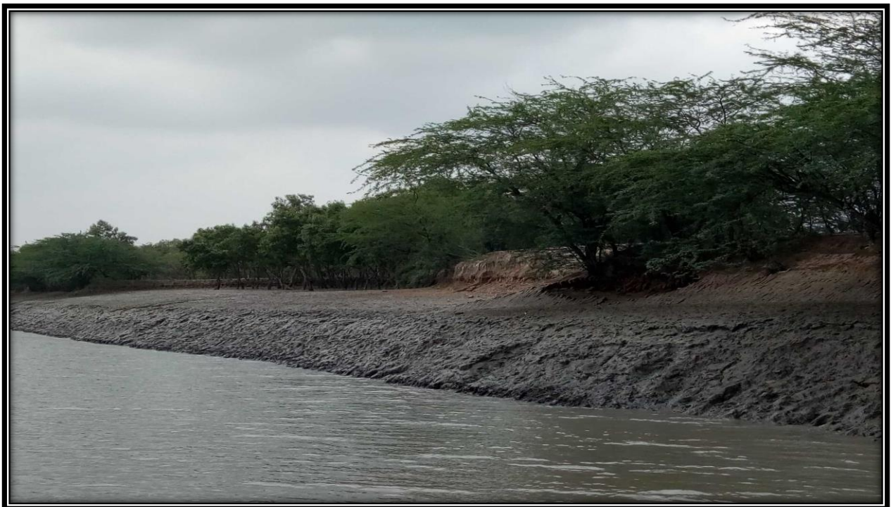
Right bank of river at CHAINAGE 24
