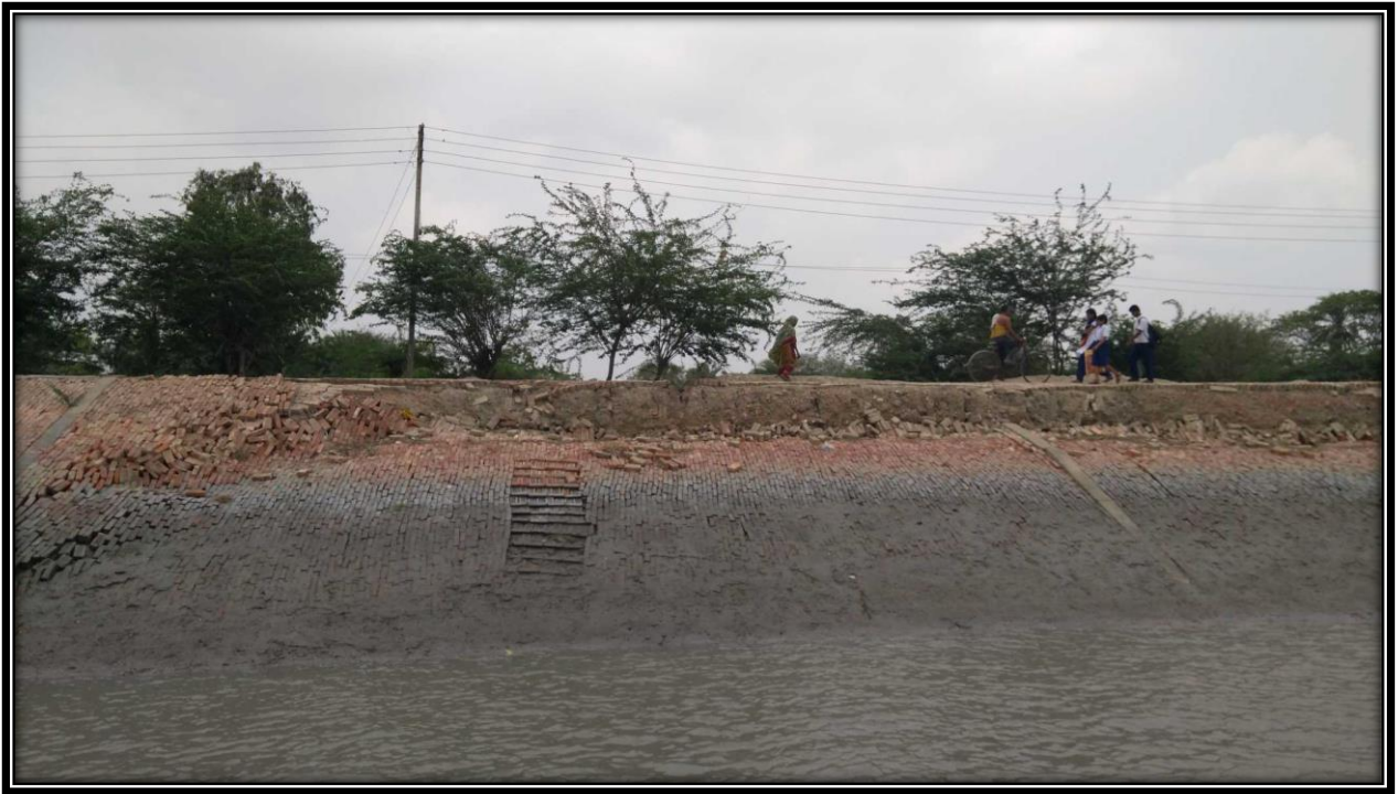
Bank Protection Wall near left bank of river at CHAINAGE 3.5
