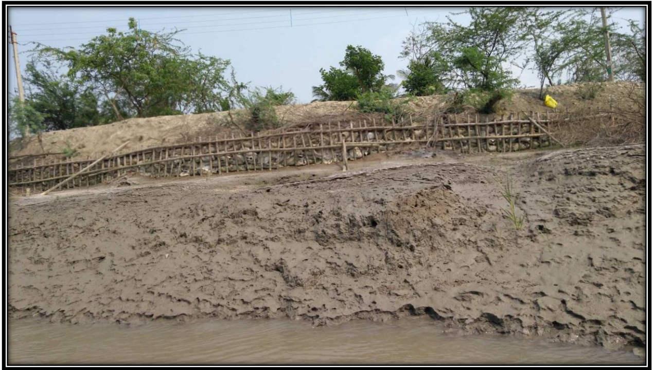
Bank Protection near left bank of river at CHAINAGE 15.5
