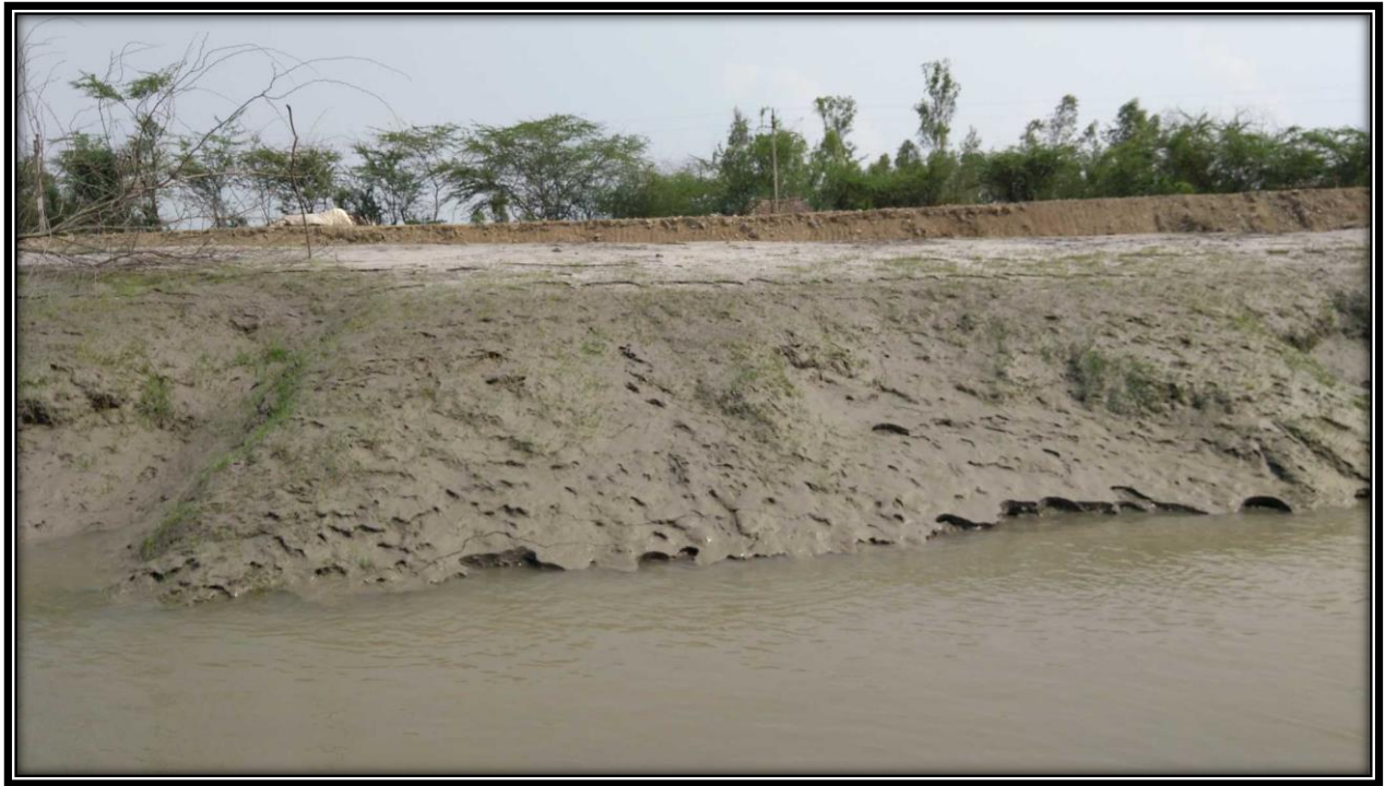
Right Bank of river at CHAINAGE 17
