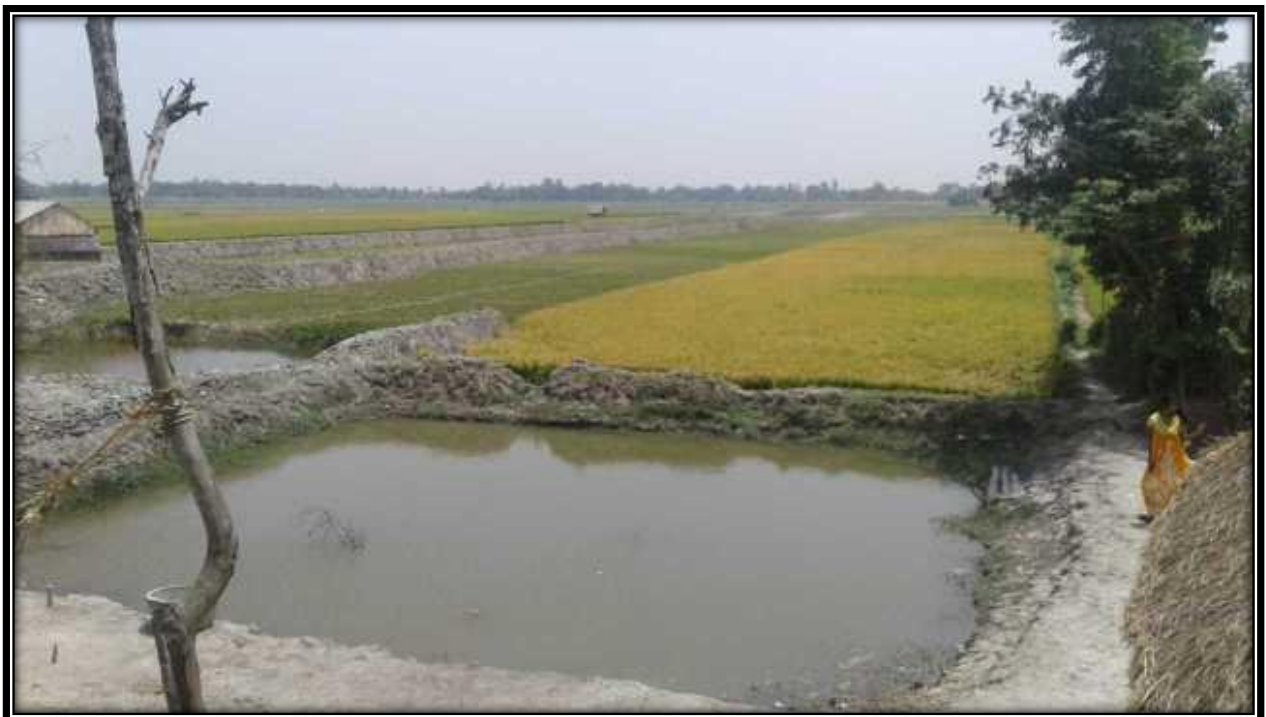
Pond& forming area at 31.2 CHAINAGE
