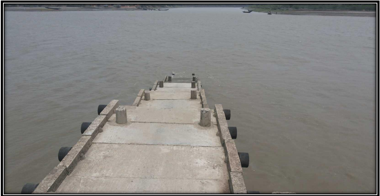
Jetty near 21 CHAINAGE of Left Side Of River Bank
