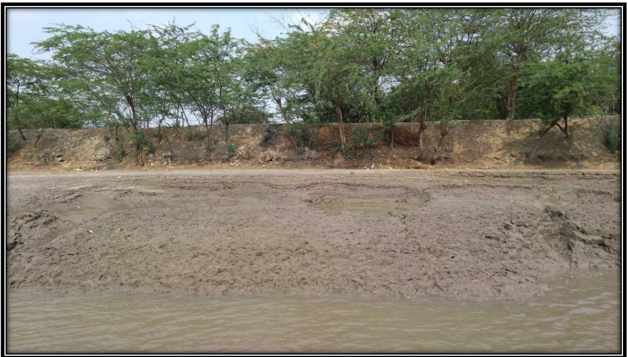
Left Bank of river at CHAINAGE 18.5
