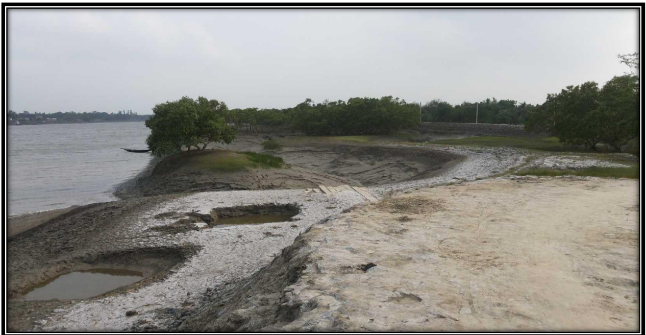
River Bank near 23.5 CHAINAGE of Left Side Of River Bank
