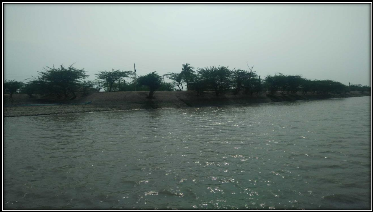
Left bank of river at CHAINAGE 37
