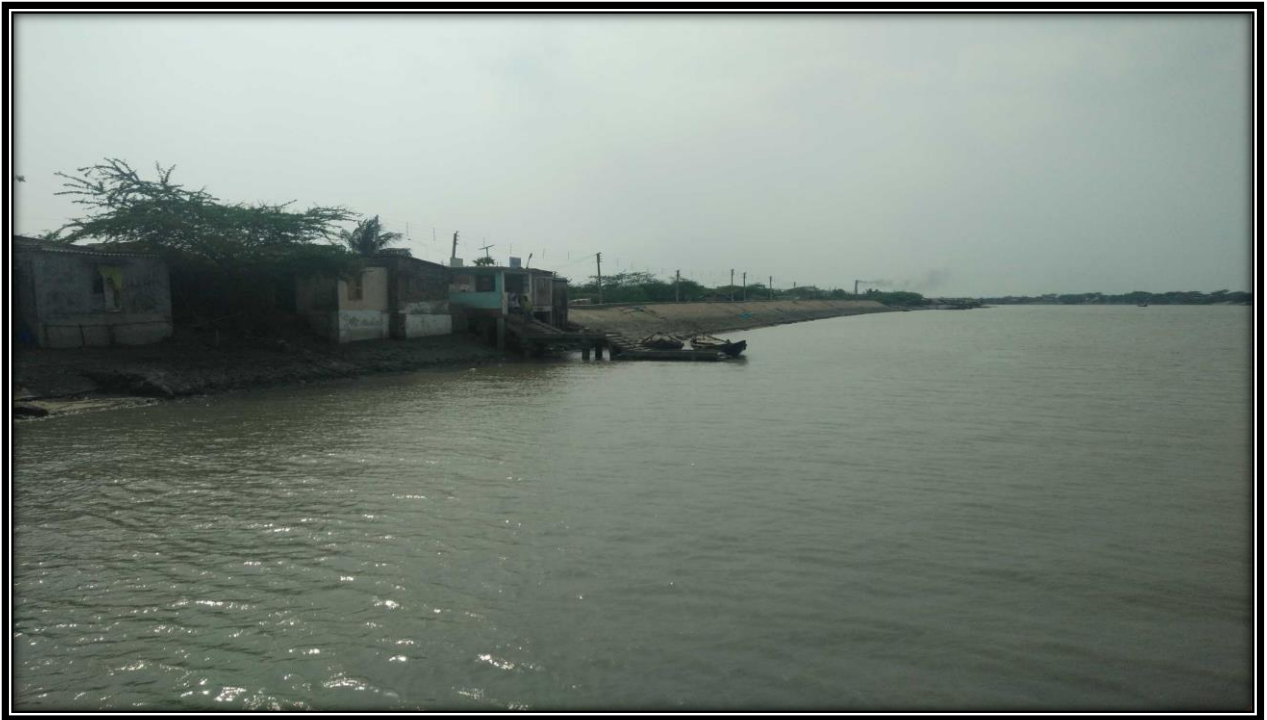
Jetty on left bank of river at CHAINAGE 36.5
