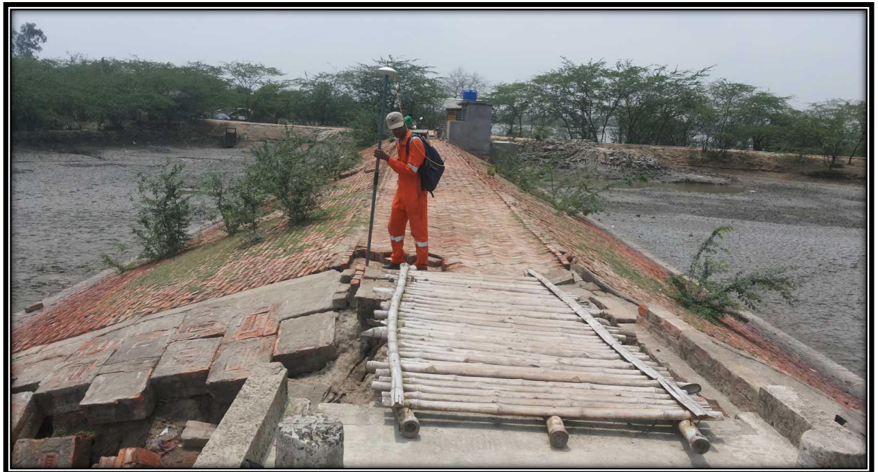
Jetty near 21 CHAINAGE of Left Side Of River Bank
