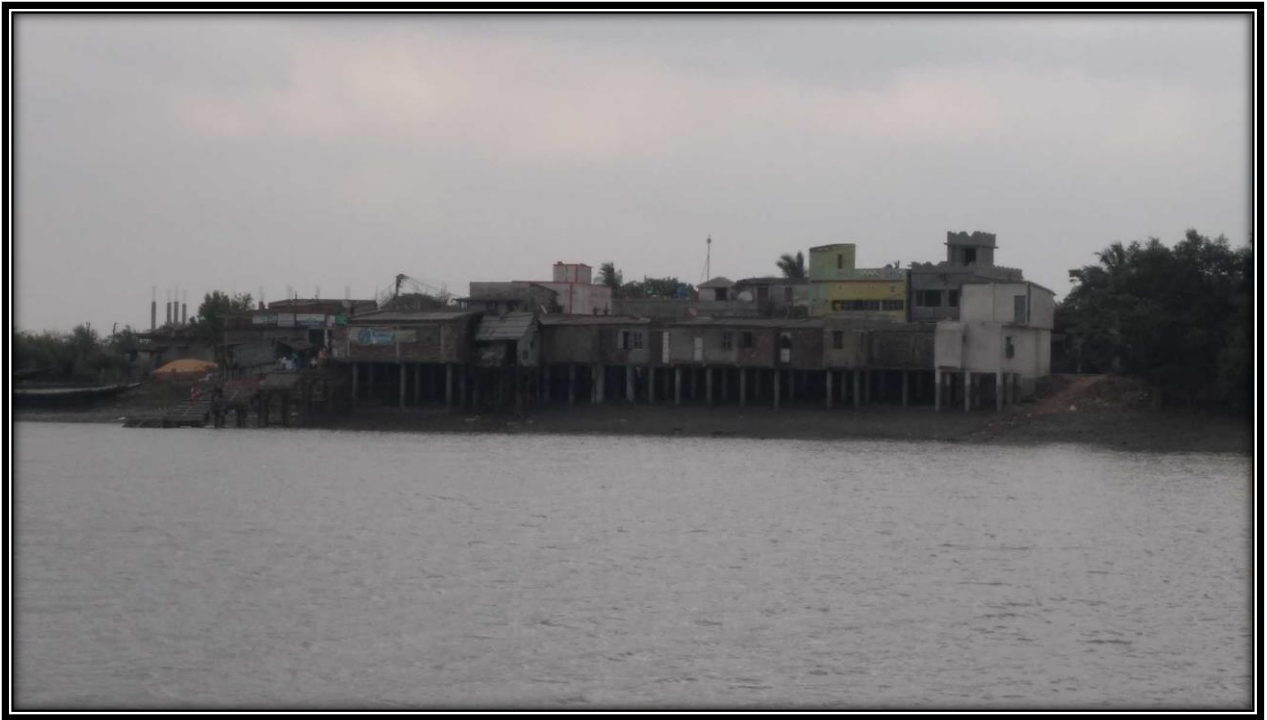
Buildings on right bank of river at CHAINAGE 8.5
