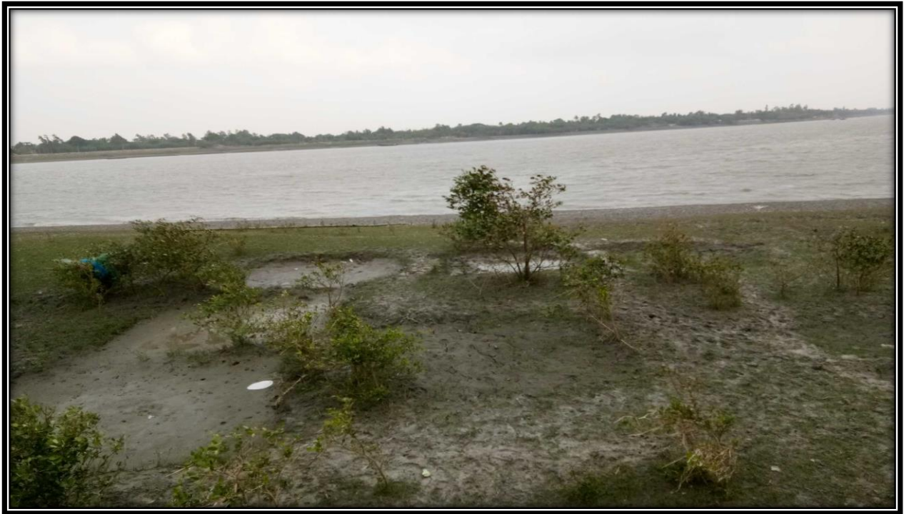
River Bank-10.1 CHAINAGE Left Bank
