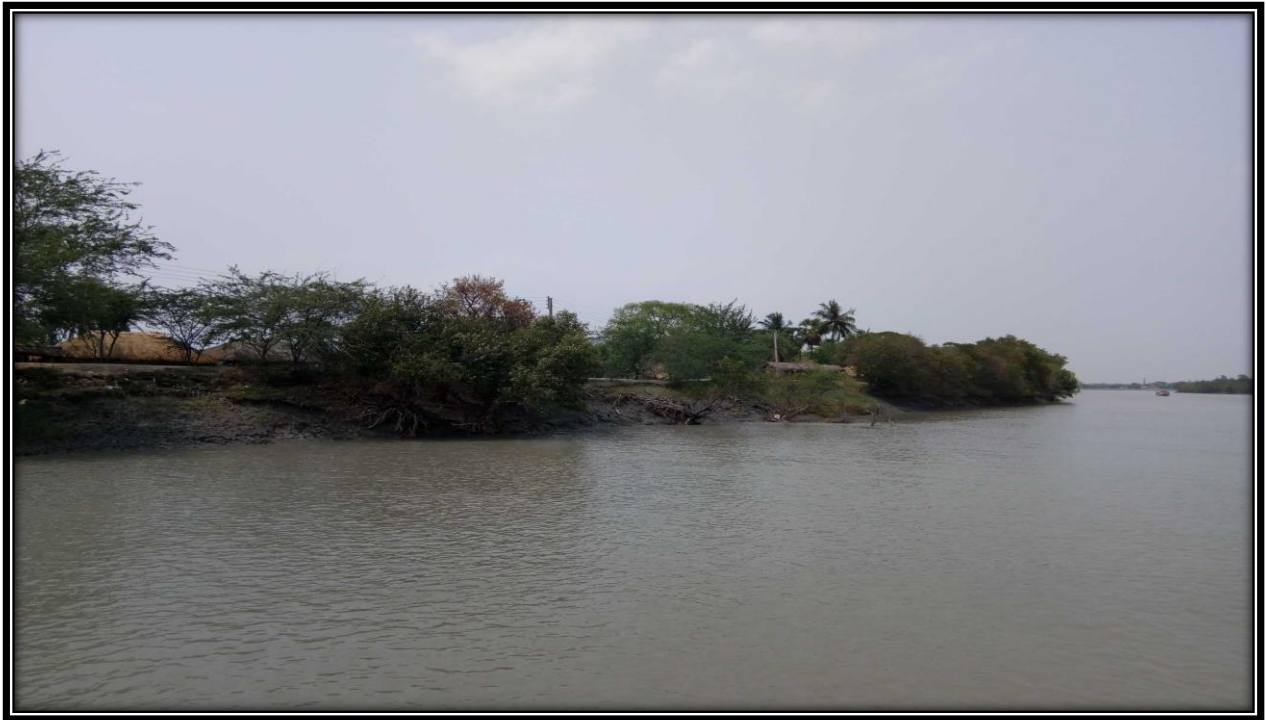
Right bank of river at CHAINAGE 29.5
