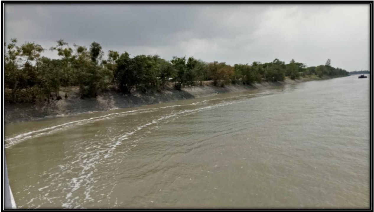
Left bank of river at CHAINAGE 32
