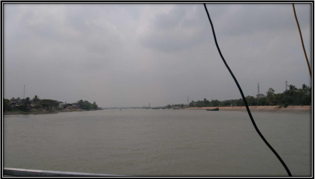
River Bank Protection Wall at CHAINAGE 4
