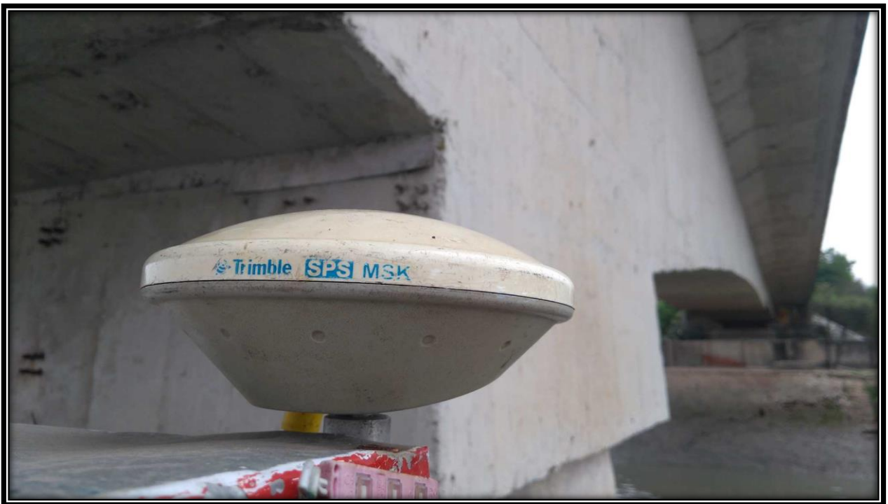
Basanti Bridge Pillar Fixing at CHAINAGE 4
