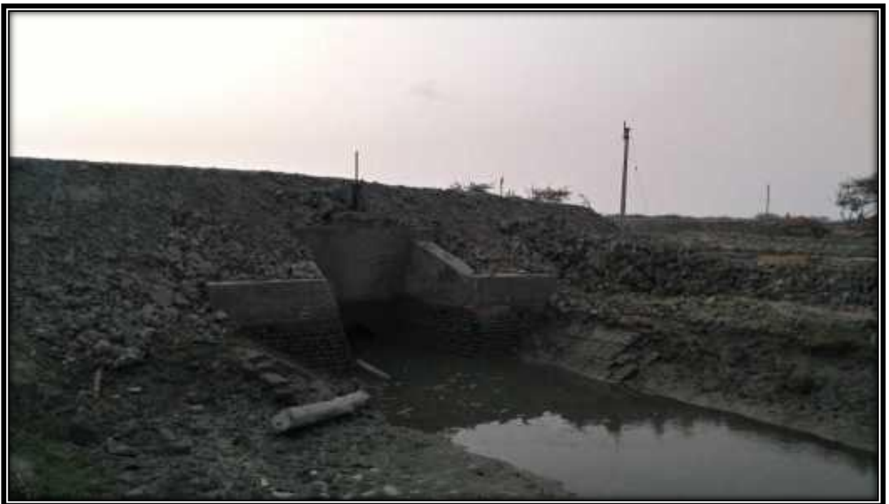
Water Lock CHAINAGE-15
