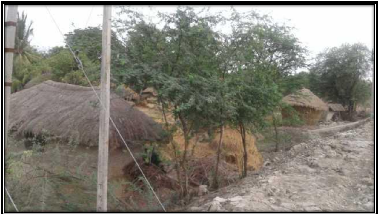
Electric Pole & Structure at 14.5 CHAINAGE
