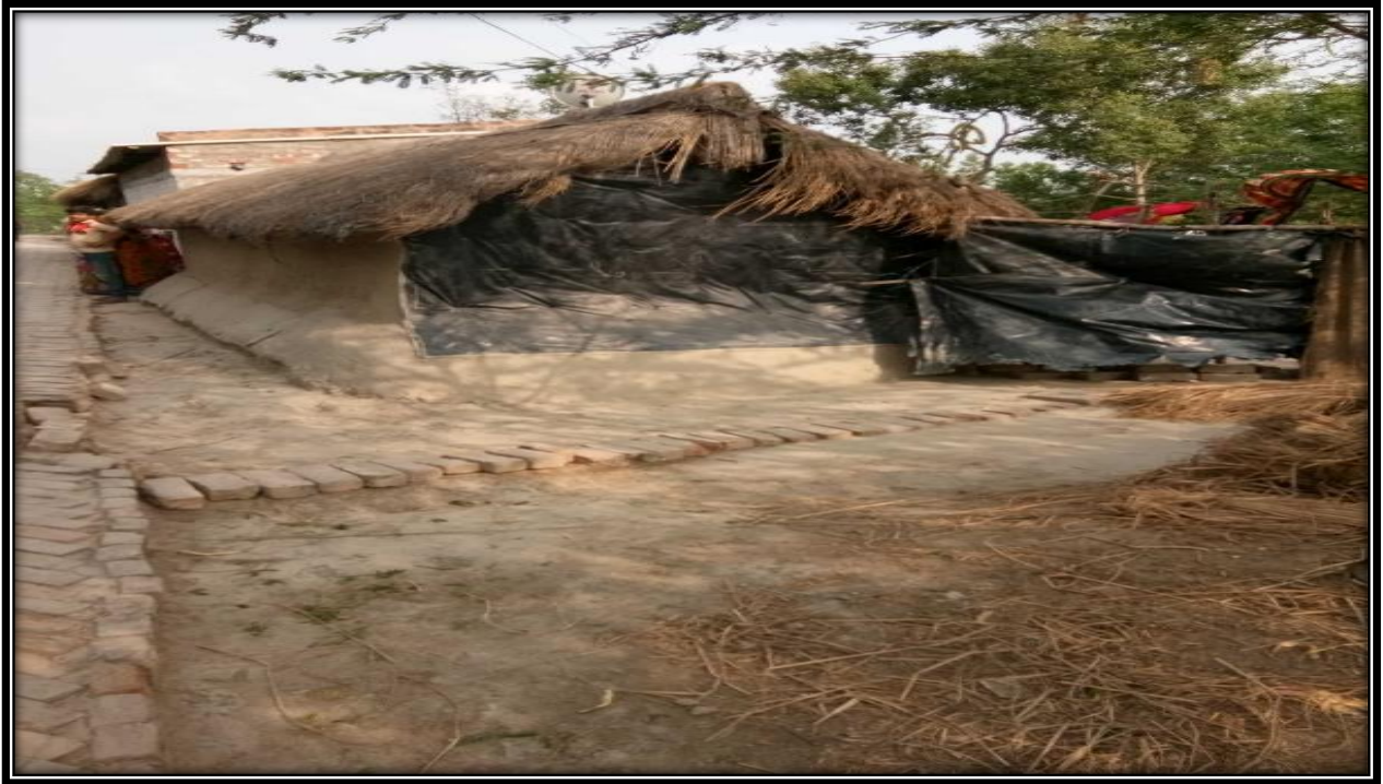
Structure AT 3.8 CHAINAGE
