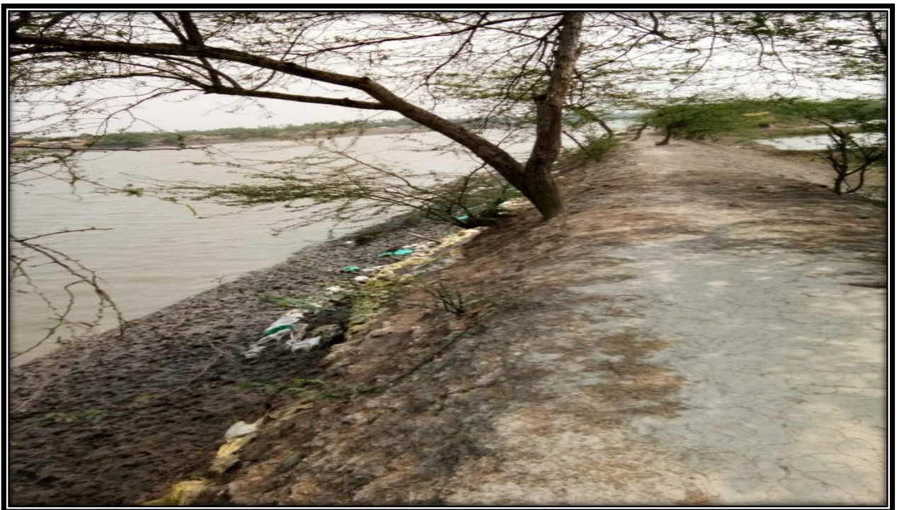
River Bank-12.2 CHAINAGE-Left Bank
