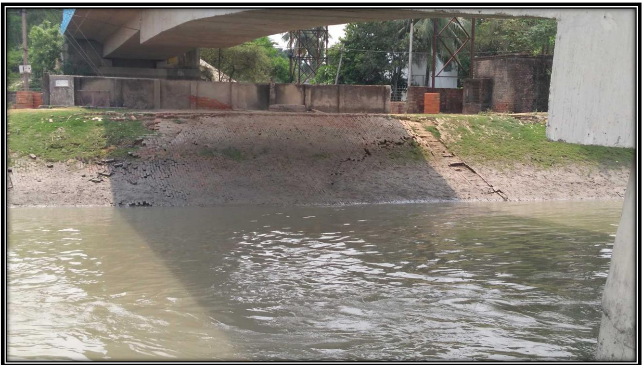
Bank Protection Wall on left bank of river at CHAINAGE 4
