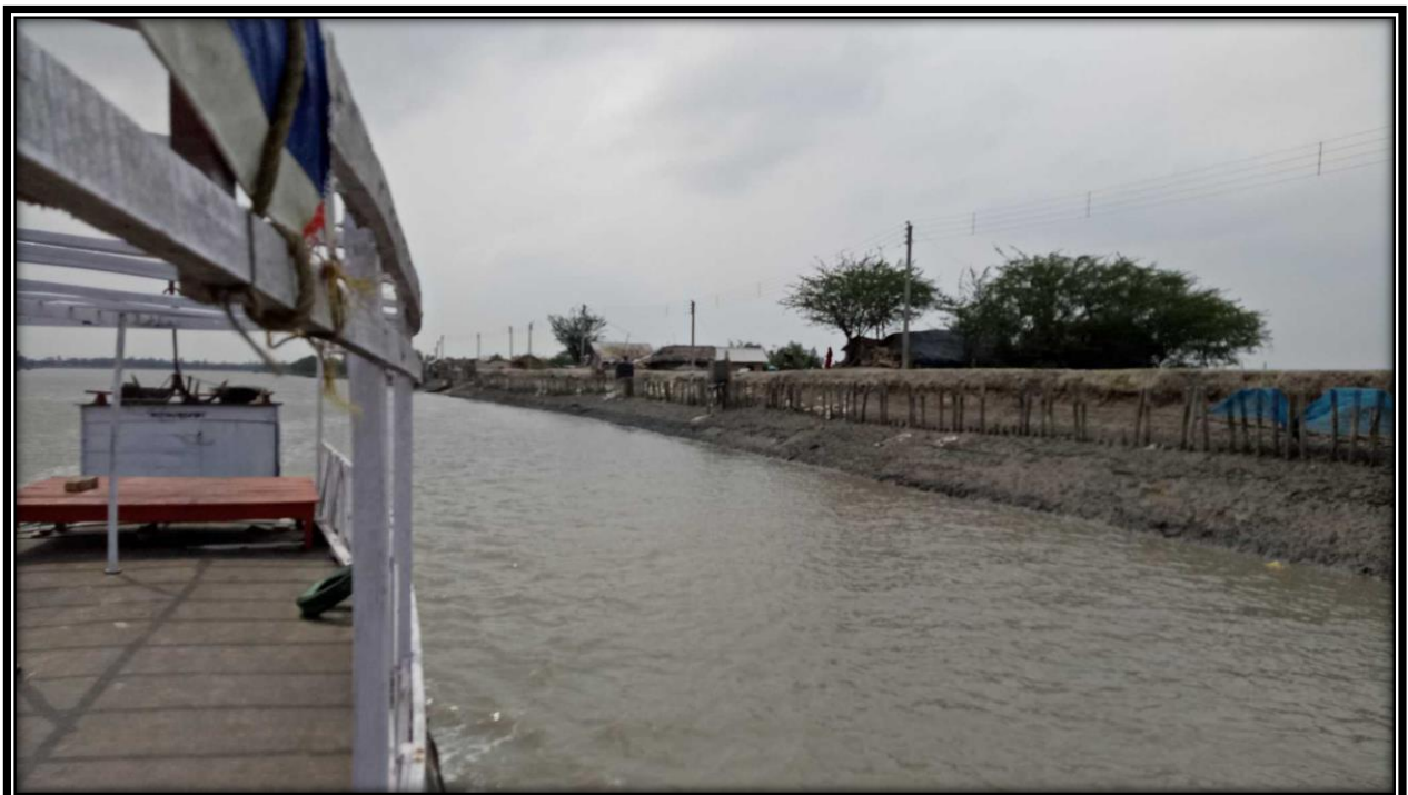
Left bank of river at CHAINAGE 32
