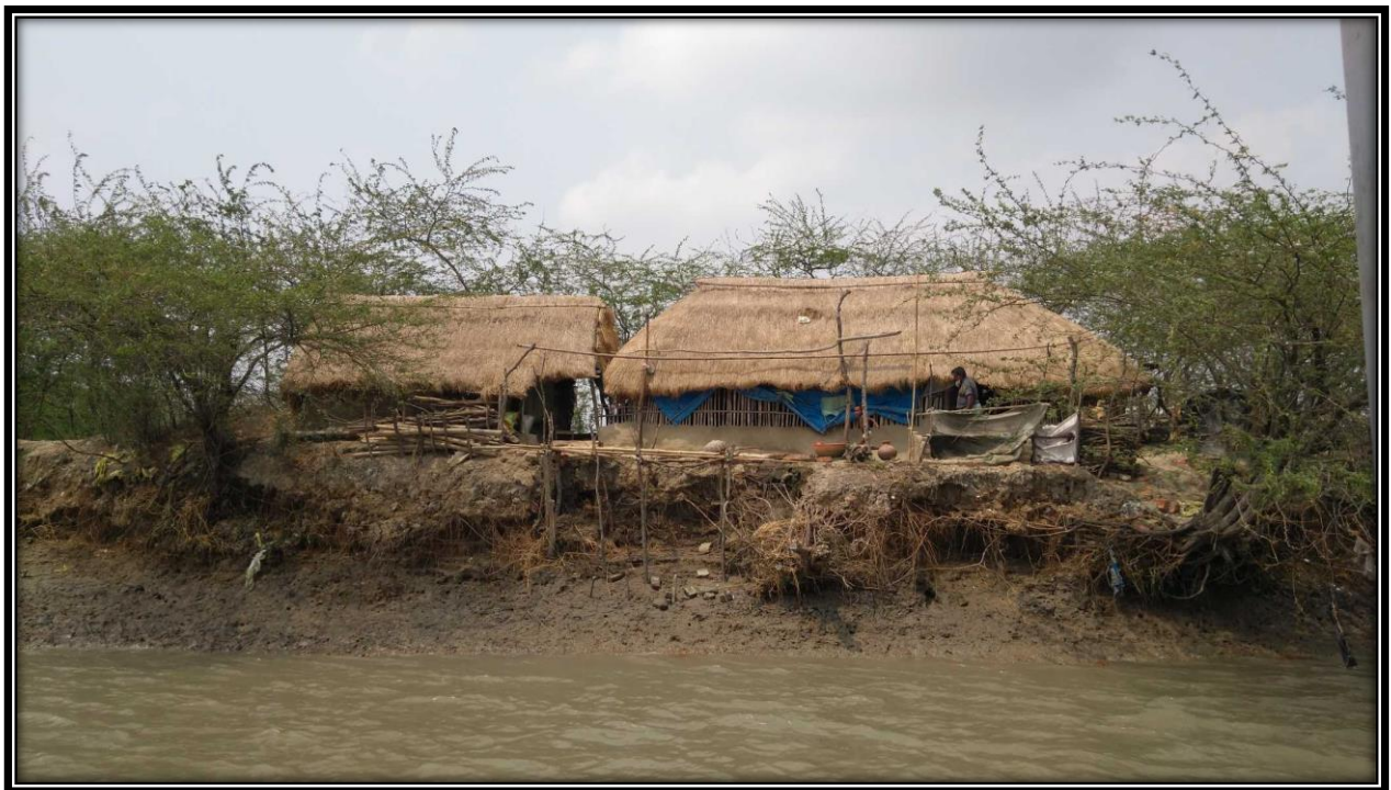
Left bank of river at CHAINAGE 7
