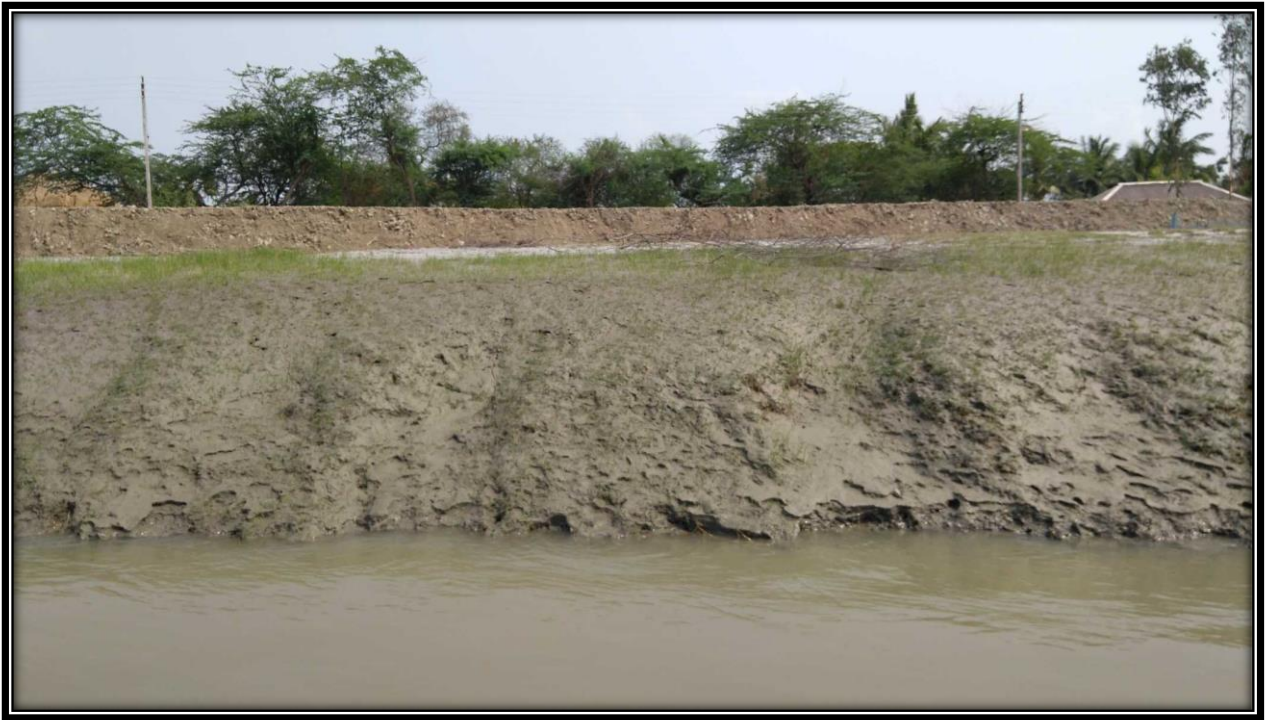
Right Bank of river at CHAINAGE 16.5
