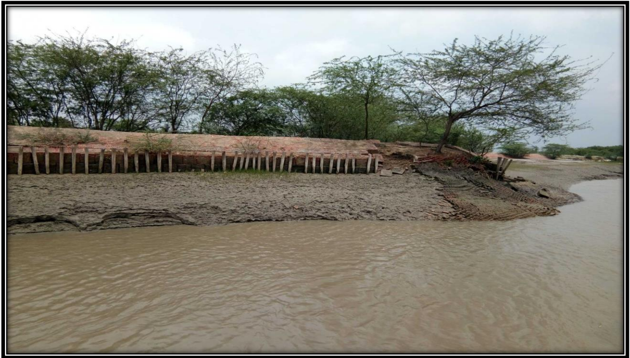
Bank protection wall near right bank of river at CHAINAGE 26
