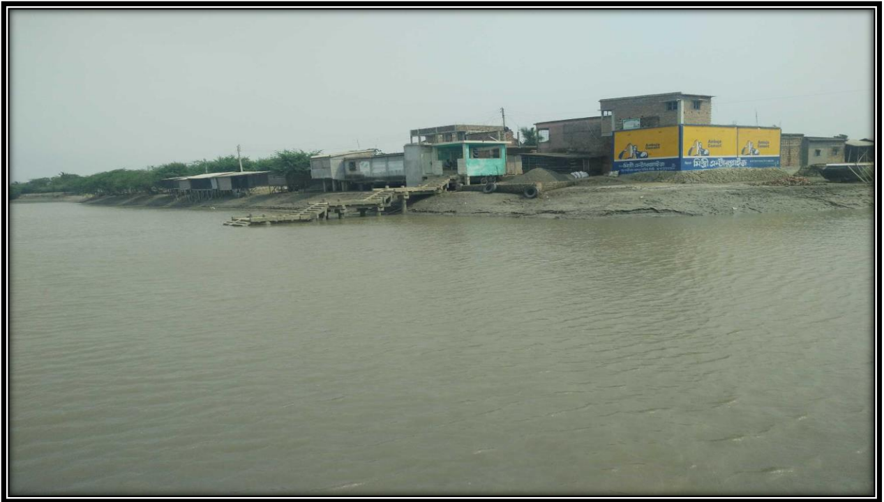
Jetty on left bank of river at CHAINAGE 35
