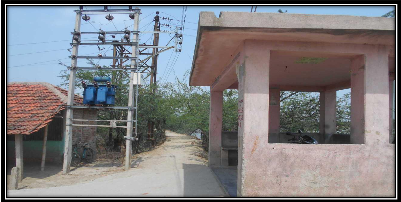
Sakhali ferry ghat at 32 Chainage-Left river bank
