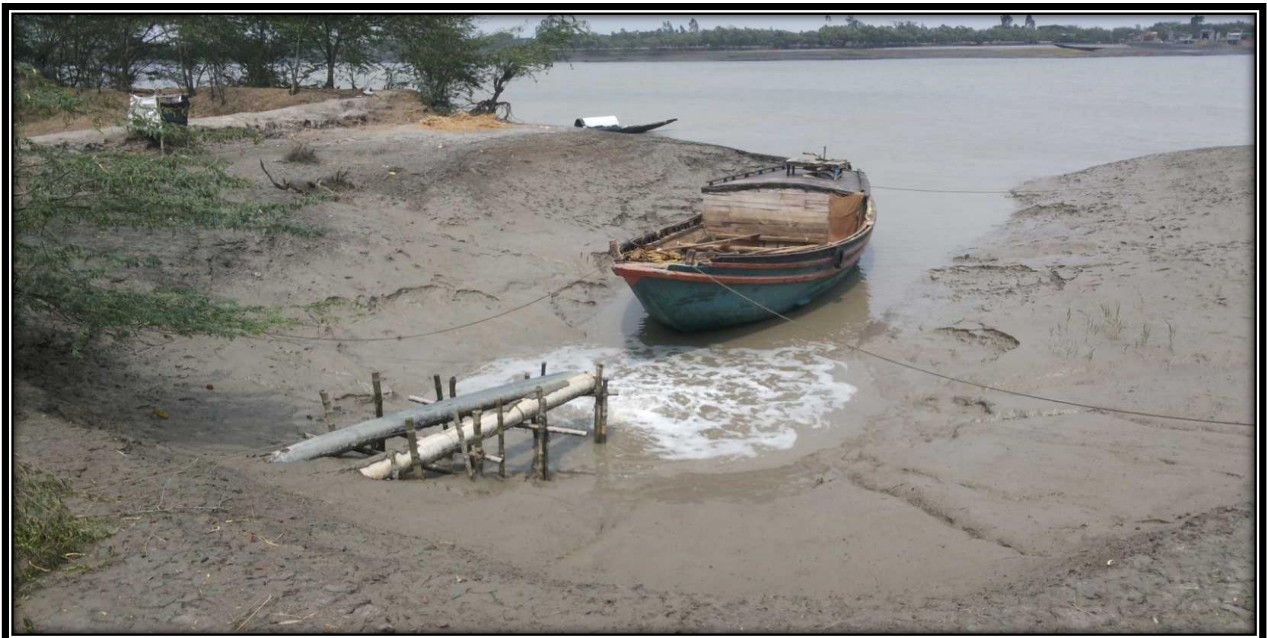
River Bank near 19.7 CHAINAGE of Left Side Of River Bank
