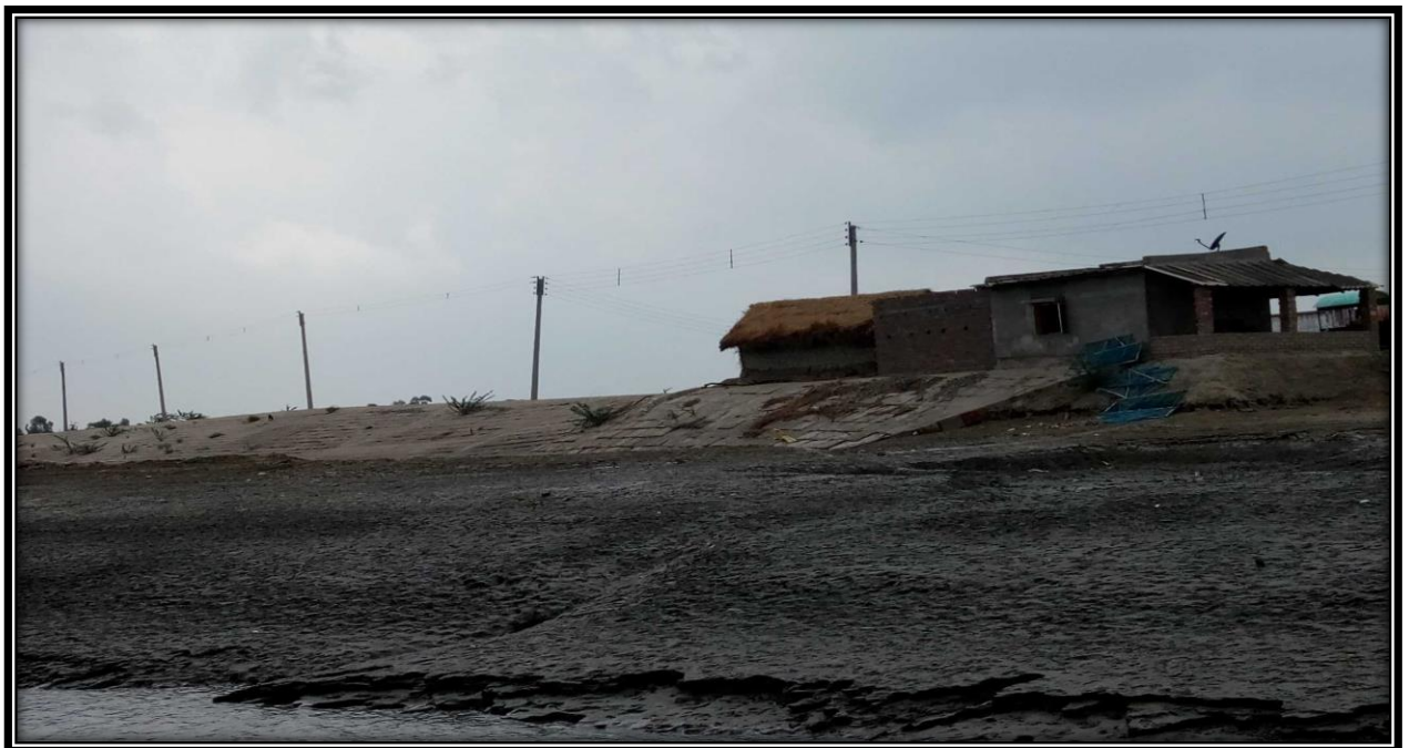
Right bank of river at CHAINAGE 25.5
