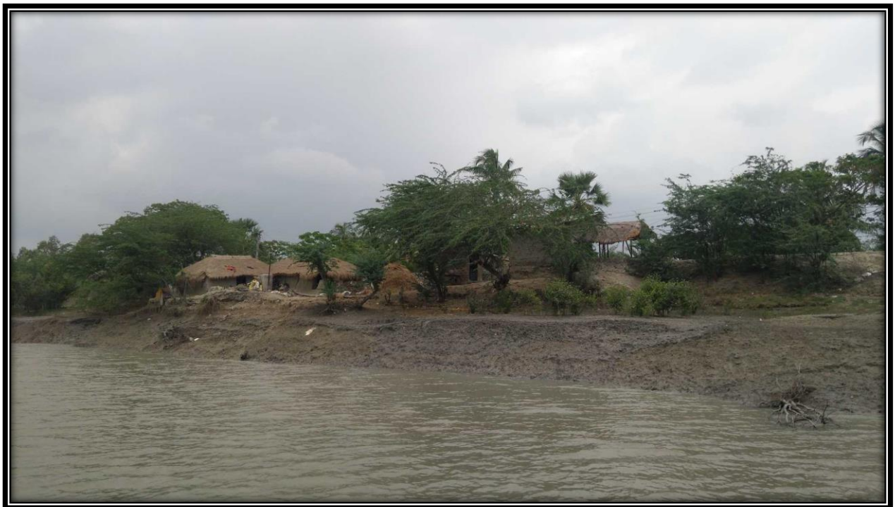
Right Bank of river at CHAINAGE 10
