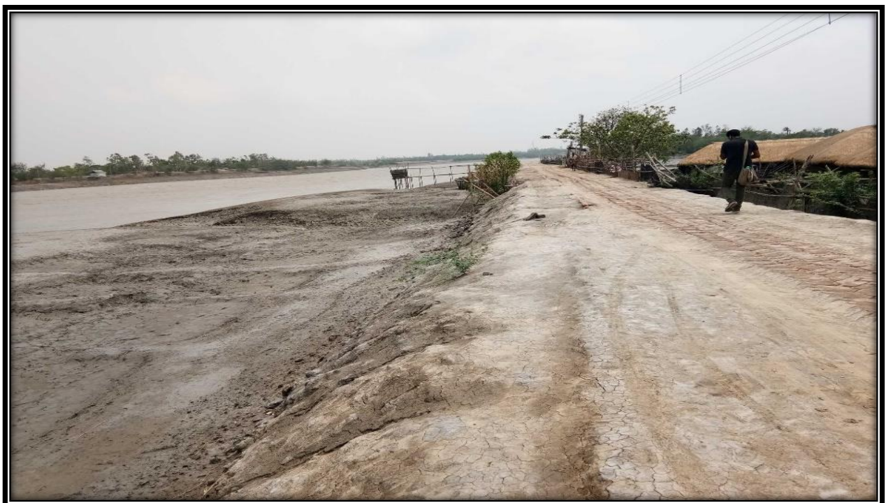
Left Side River Bank at 17 CHAINAGE
