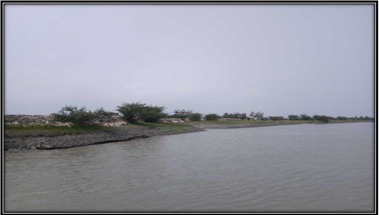
Right bank of river at CHAINAGE 28.5
