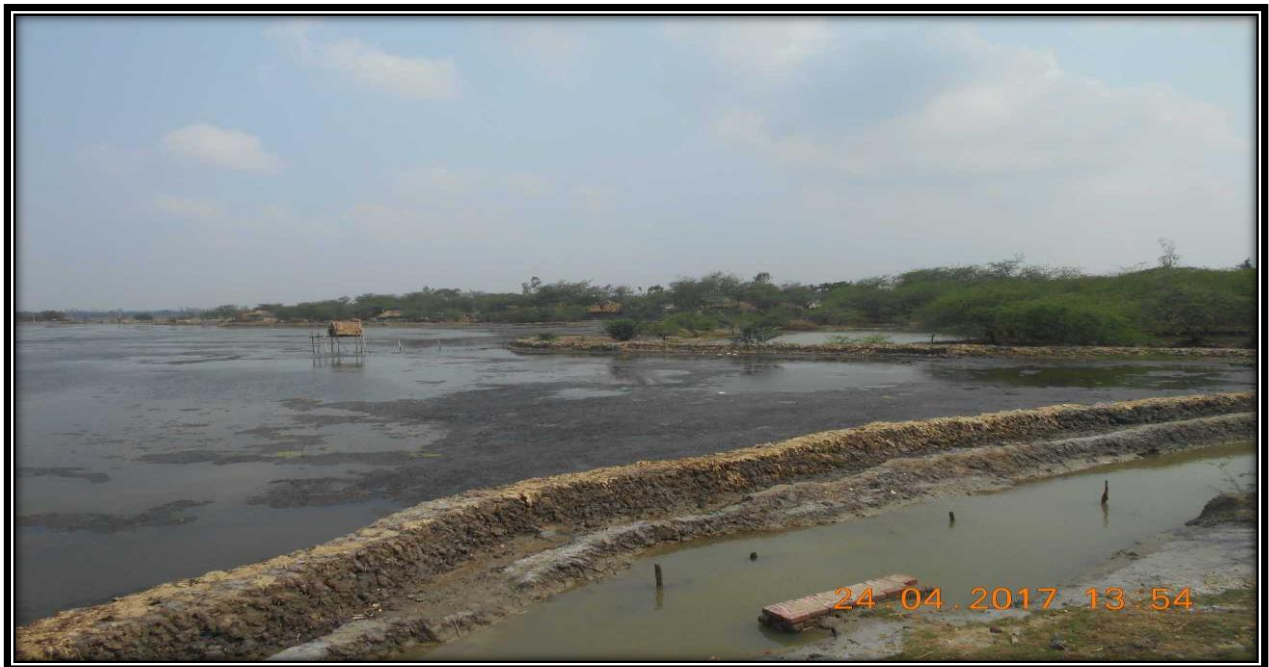
Pond a head Right Side of River Bank at 24 CHAINAGE
