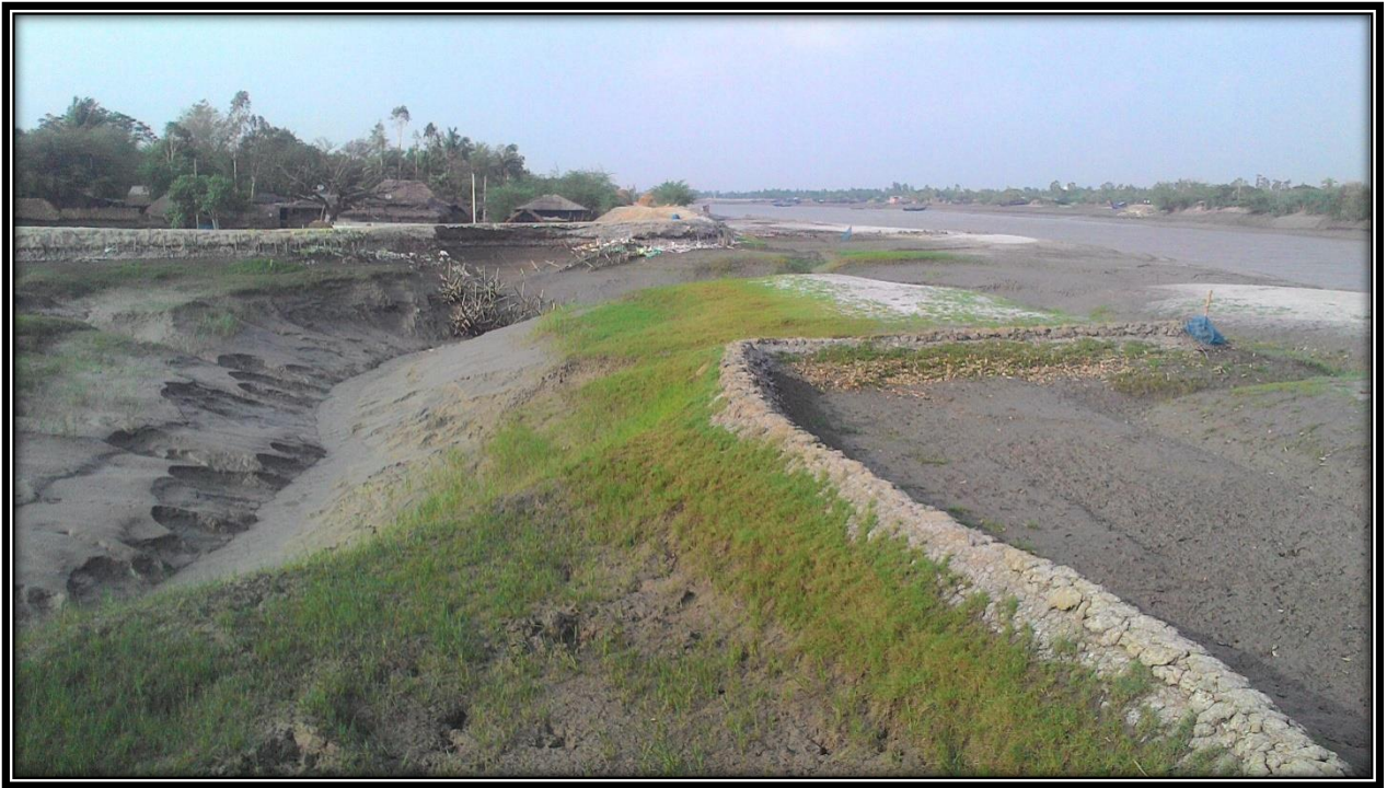
River Bank near 27.2 CHAINAGE of Left Side of River Bank
