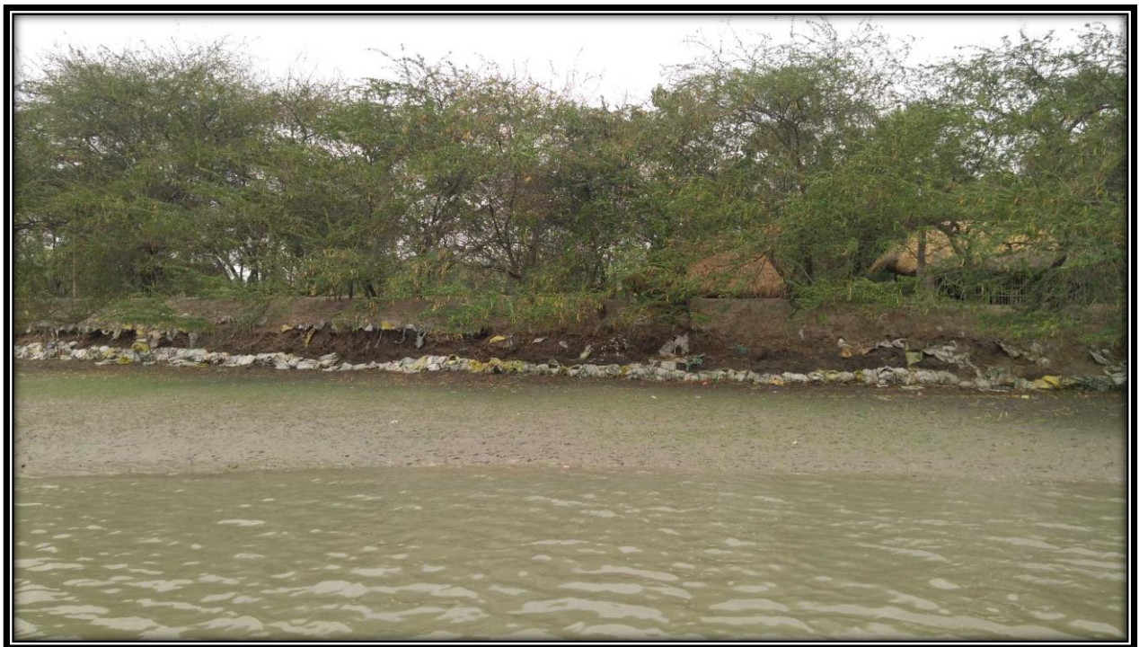
Left bank of river at CHAINAGE 5
