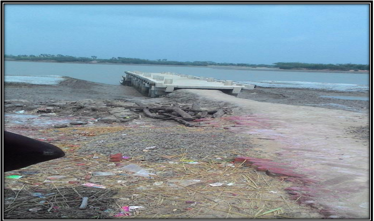
Jetty near 25 CHAINAGE of Left Side of River Bank
