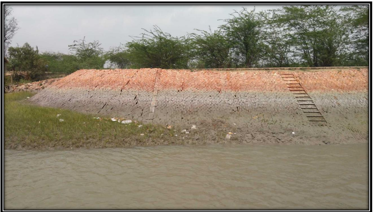
Bank protection wall near left bank of river at CHAINAGE 4.5
