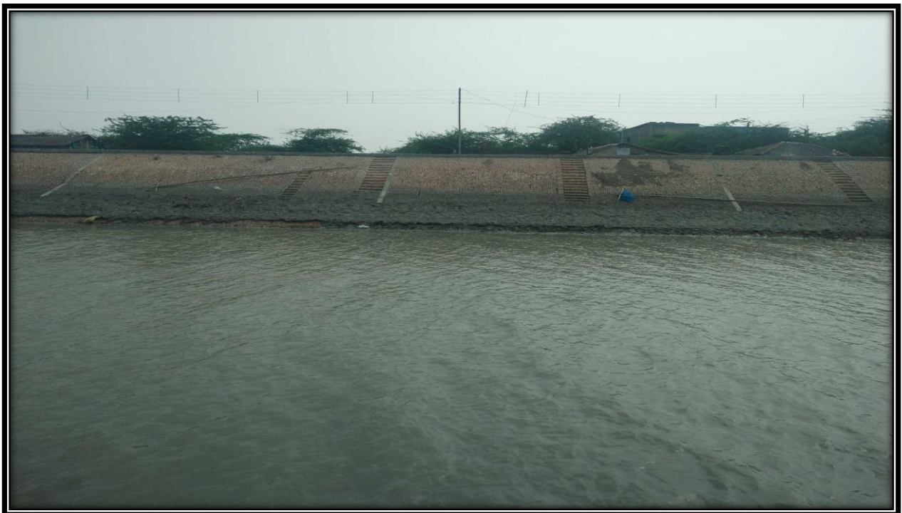
Right bank of river at CHAINAGE 36.5
