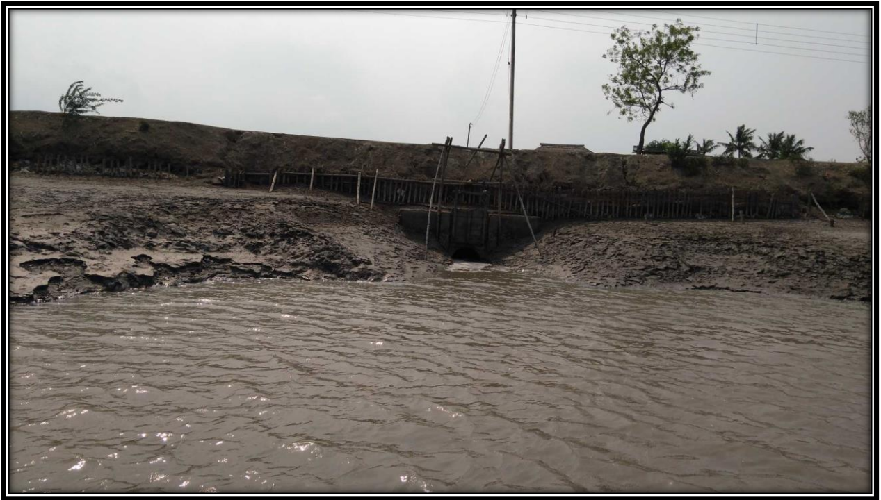
Water Lock on Left Bank at CHAINAGE 19
