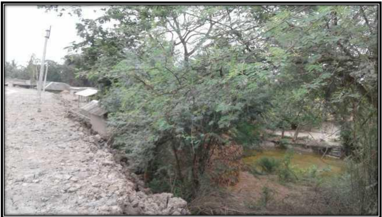
Structure Area at 14 CHAINAGE
