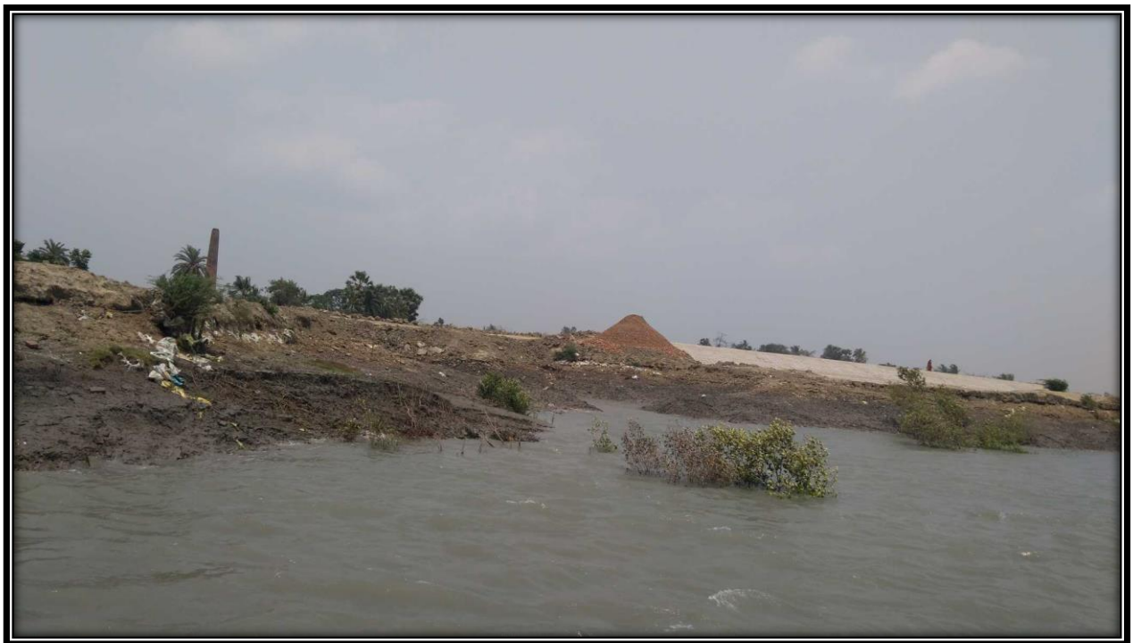
Bank Protection Wall near left bank of river at CHAINAGE 2
