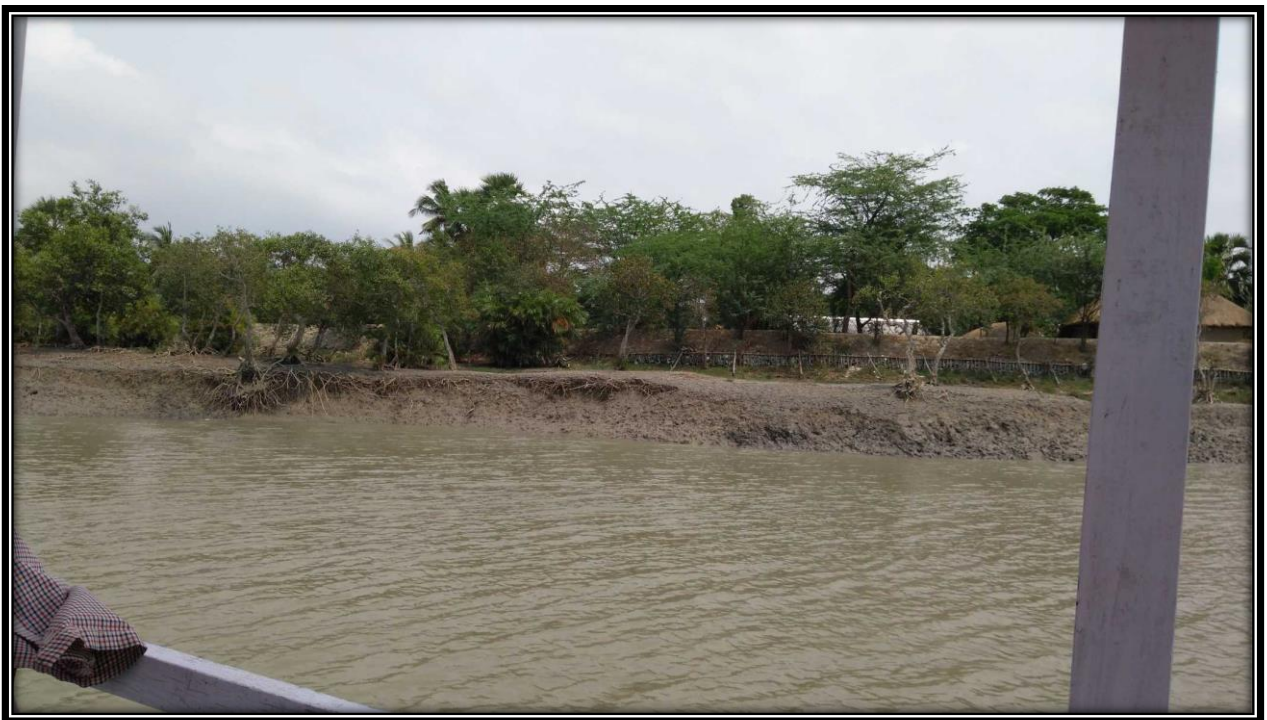
Right Bank of river at CHAINAGE 11.5
