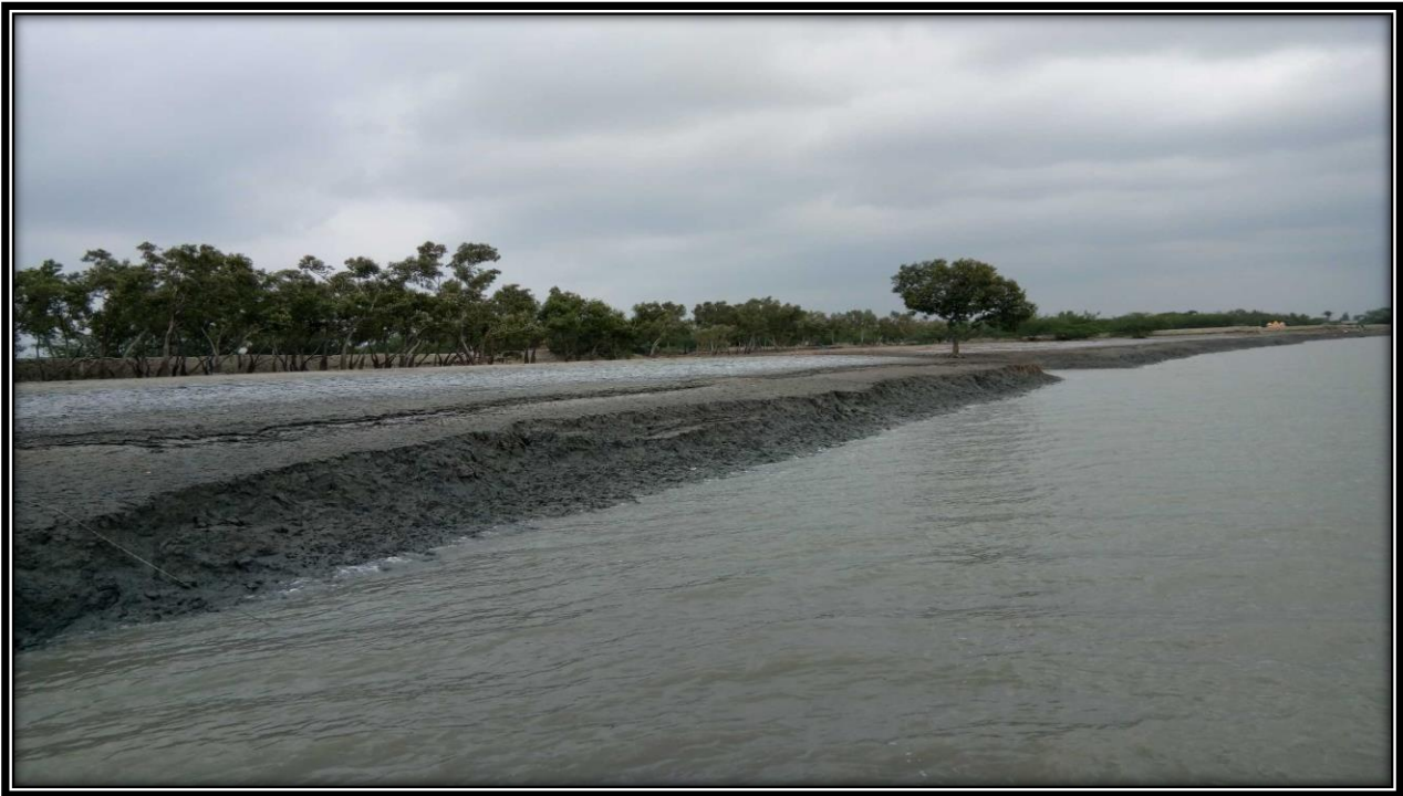
Left bank of river at CHAINAGE 22.5
