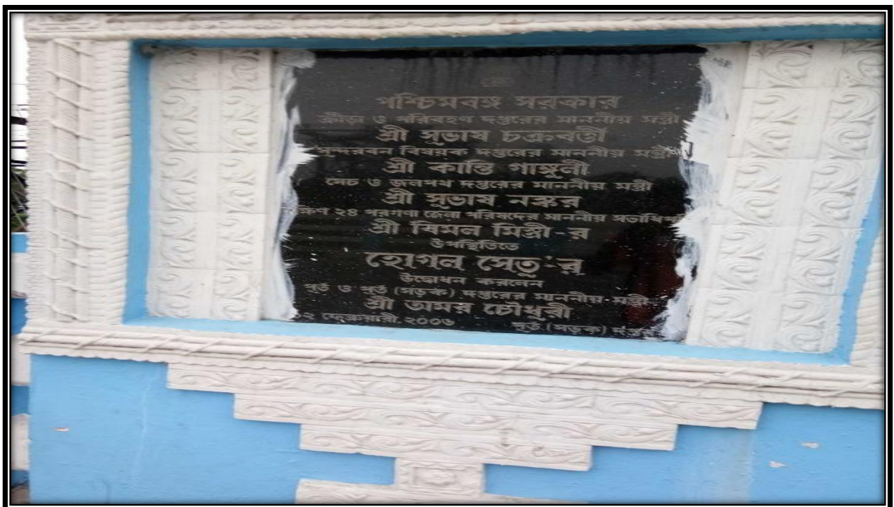
Bridge at 4.1 Chainage
