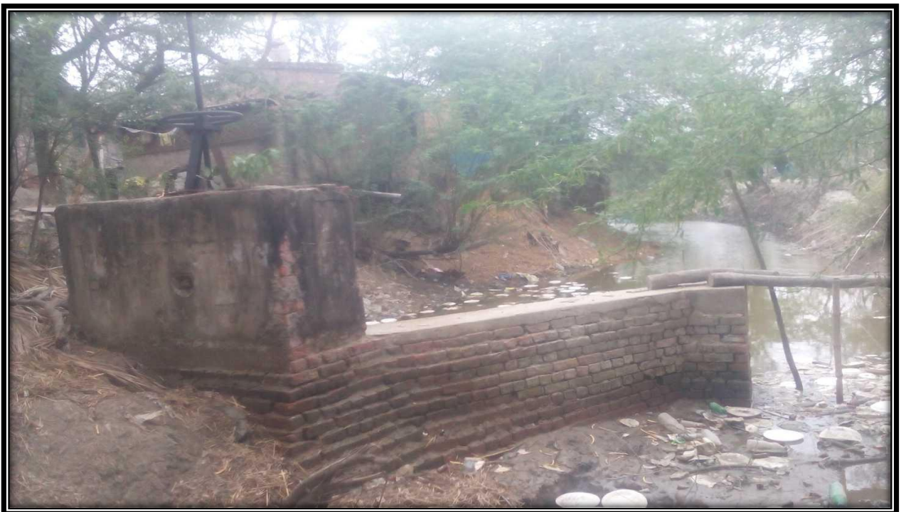
Water Lock at CHAINAGE 4.6
