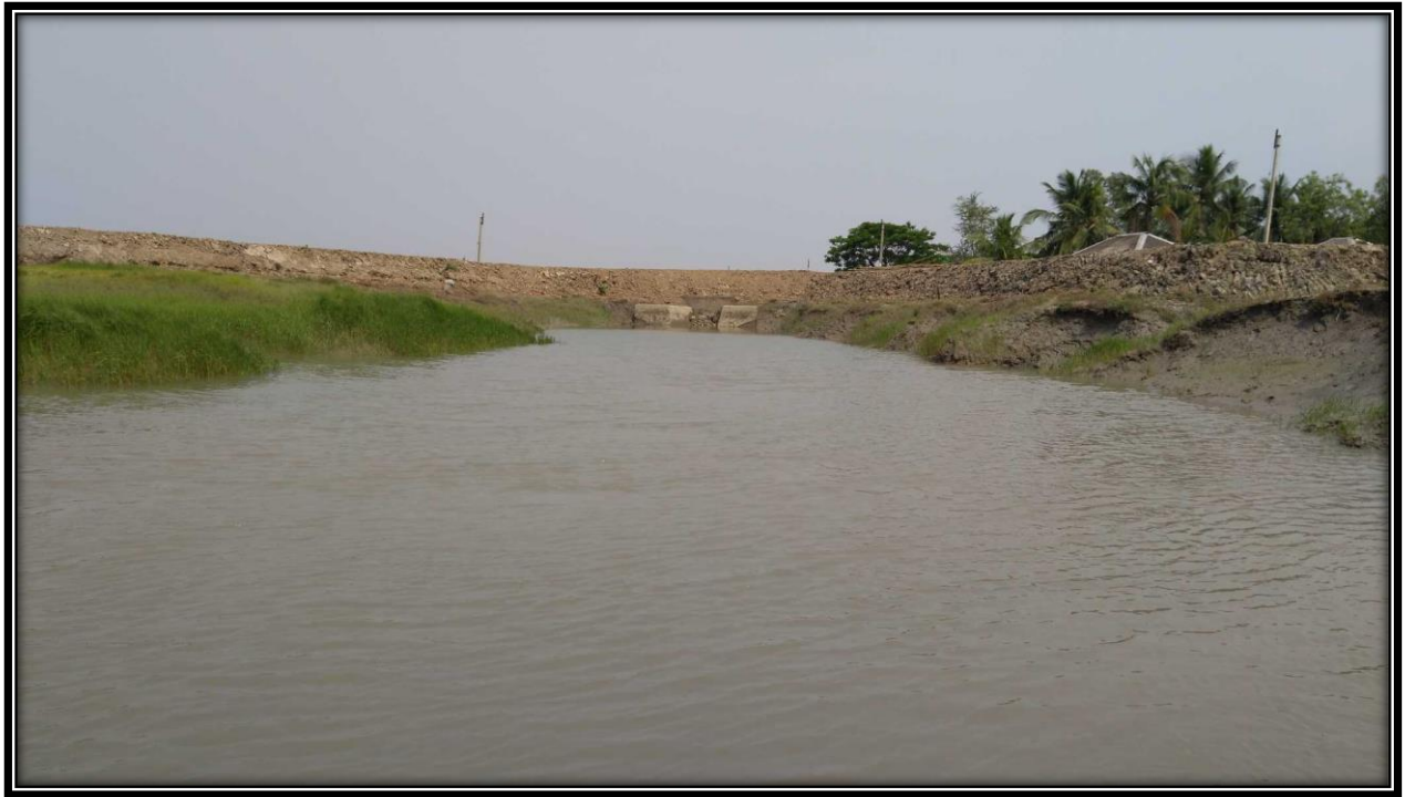
Water Lock on left bank of river at CHAINAGE 15
