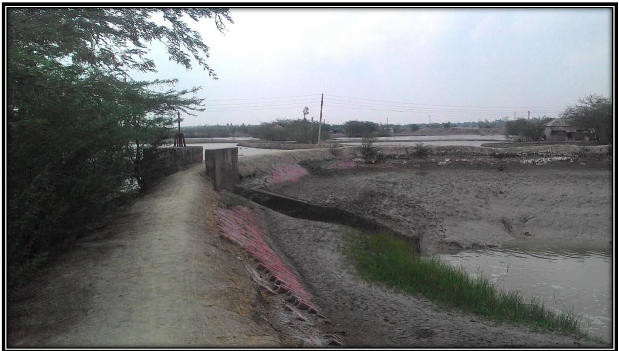
Water Lock near 25.5 CHAINAGE of Left Side of River Bank
