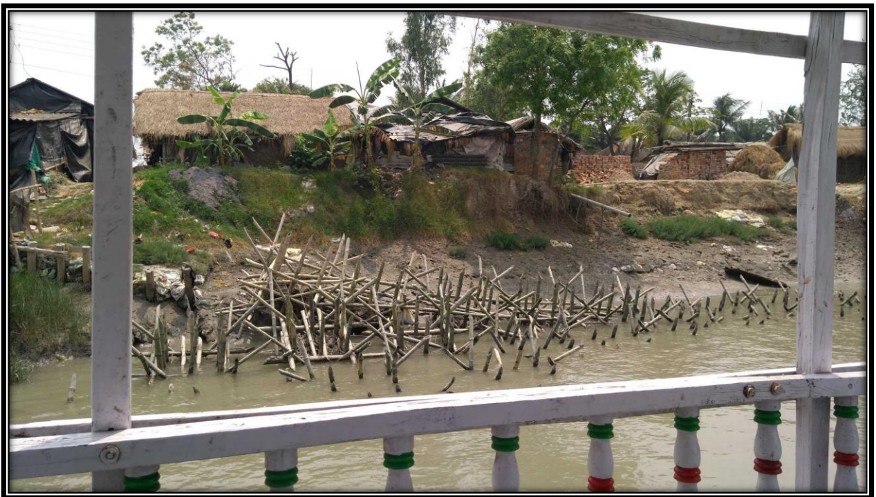
Right bank of river at CHAINAGE 5.5
