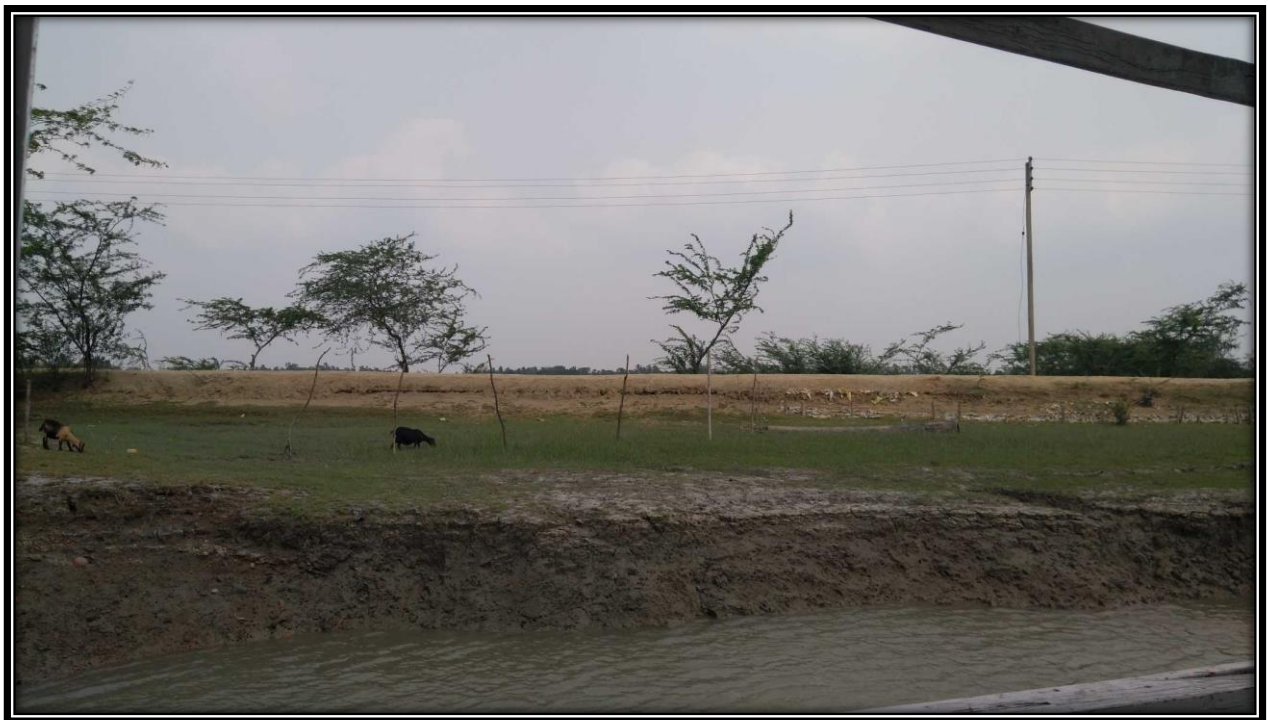
Right bank of river at CHAINAGE 6.5
