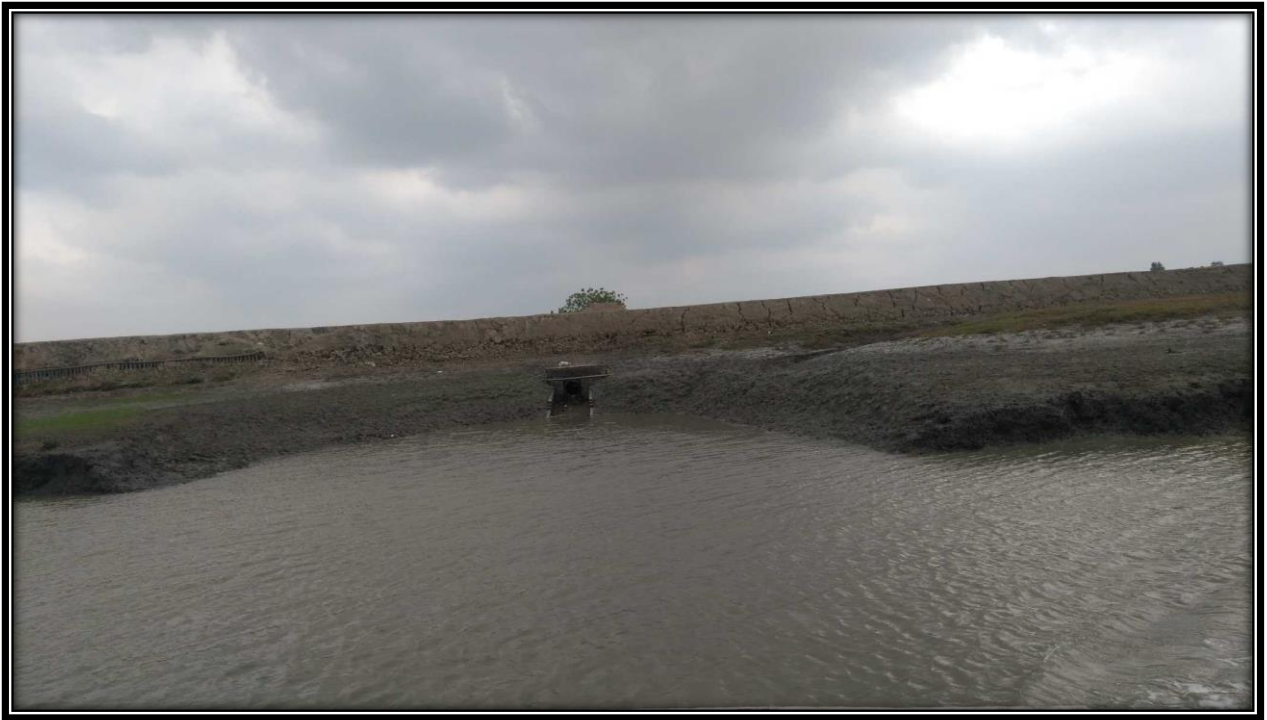
Water Lock on right bank at CHAINAGE 9
