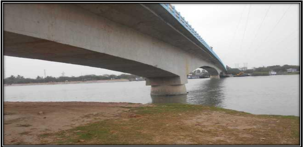
Basanti Bridge near 4 CHAINAGE of Right Side of River Bank
