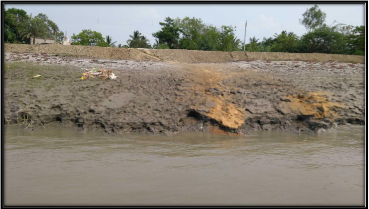
Left Bank of river at CHAINAGE 16
