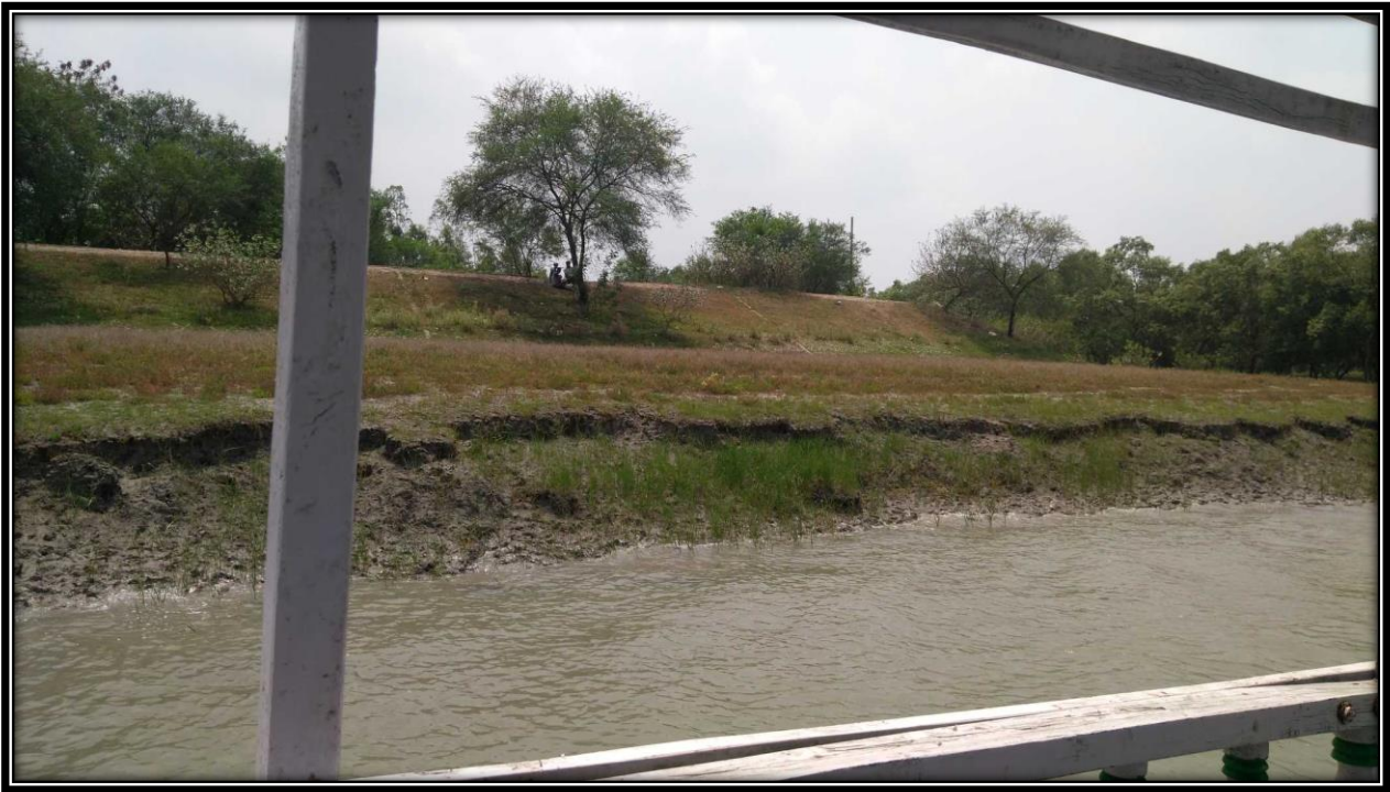
Right bank of river at CHAINAGE 0.5
