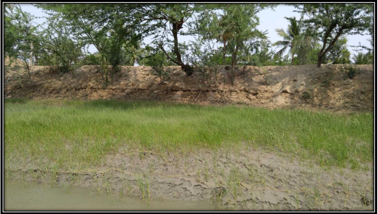
Left Bank of river at CHAINAGE 14
