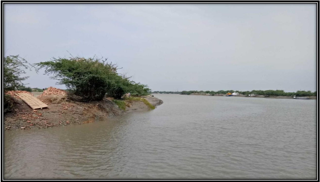
Left bank of river at CHAINAGE 35.5
