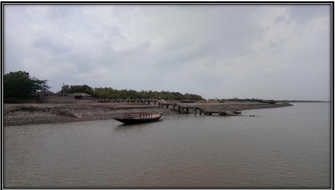
Jetty on left bank of river at CHAINAGE 25
