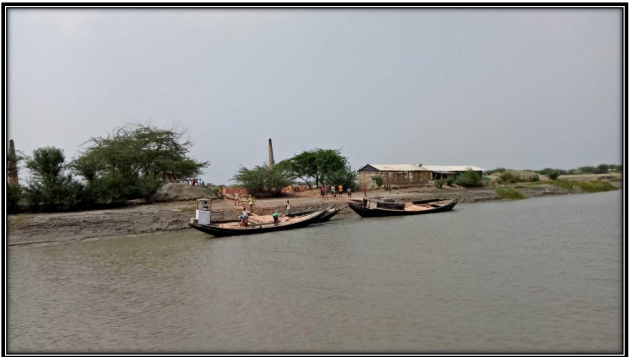
Brick loading point of brick kiln at CHAINAGE 36
