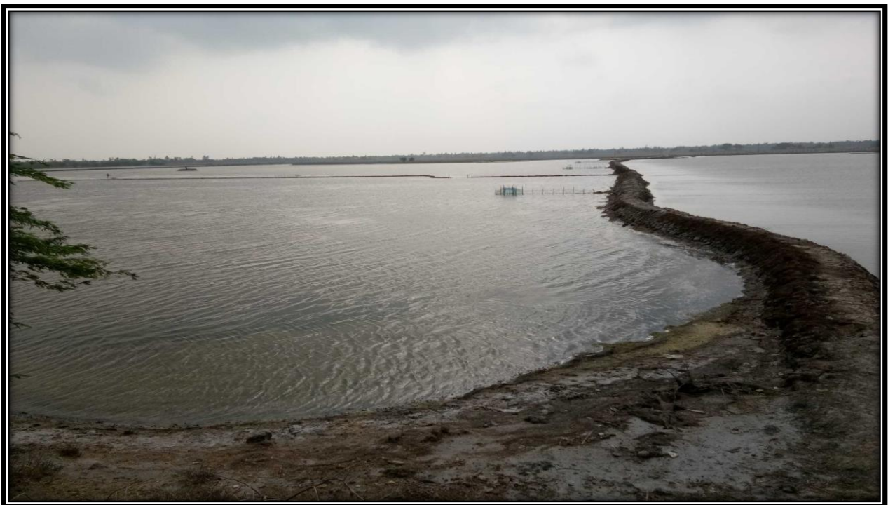
Pond near left bank of river at CHAINAGE 9.9
