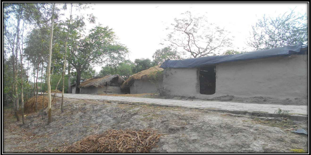
Structure at 23.6 CHAINAGE
