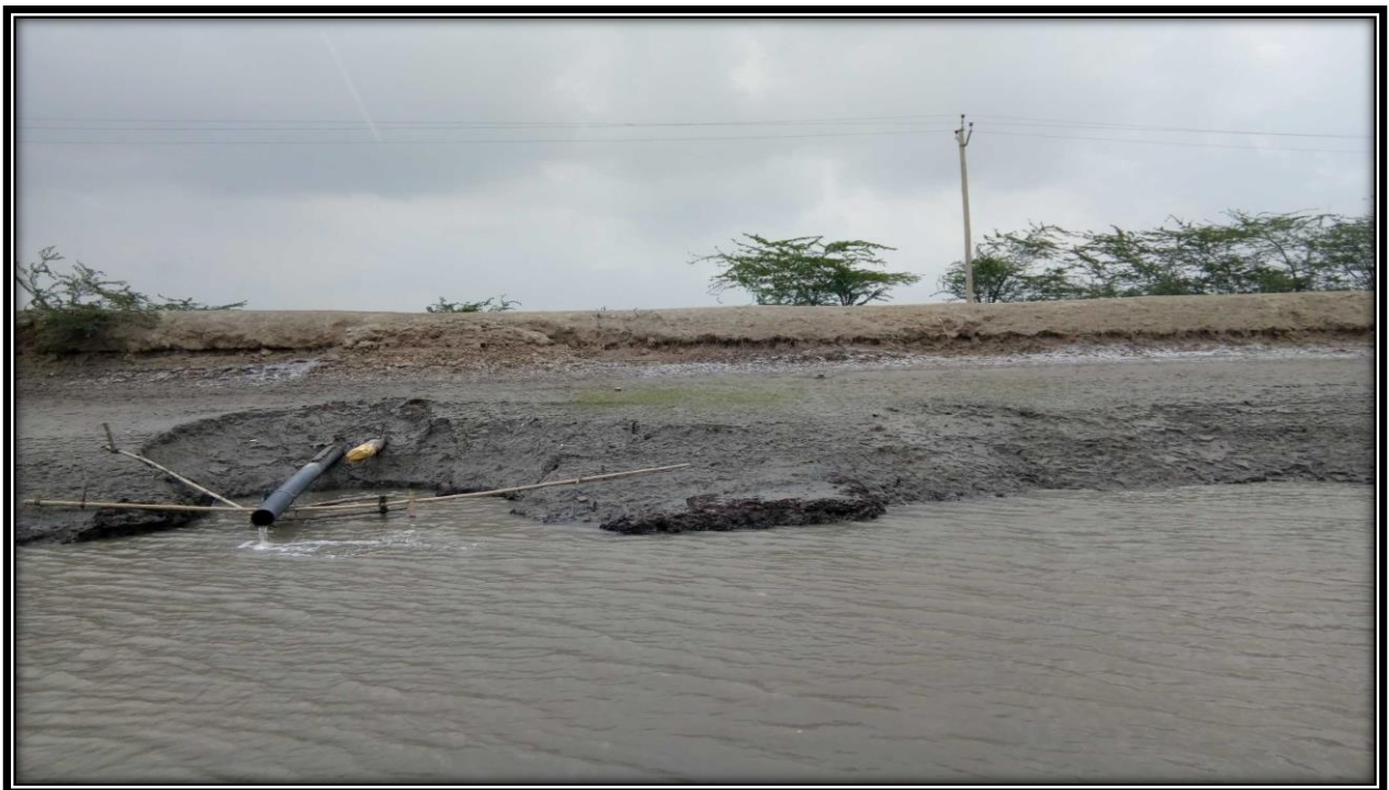
Left bank of river at CHAINAGE 26
