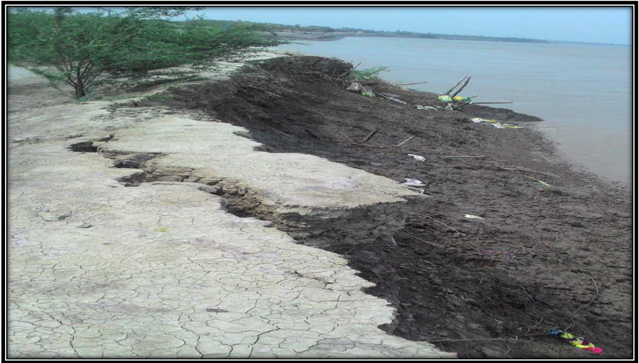
River Bank Erosion near 22 CHAINAGE Of Left Side Of River Bank
