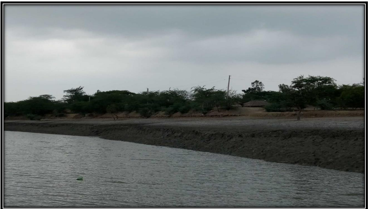
Left bank of river at CHAINAGE 24.5
