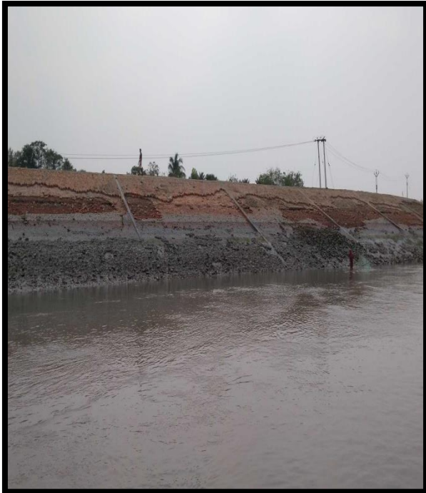
RIVER BANK PROTECTION AT CHAINAGE 95, LEFT BANK
