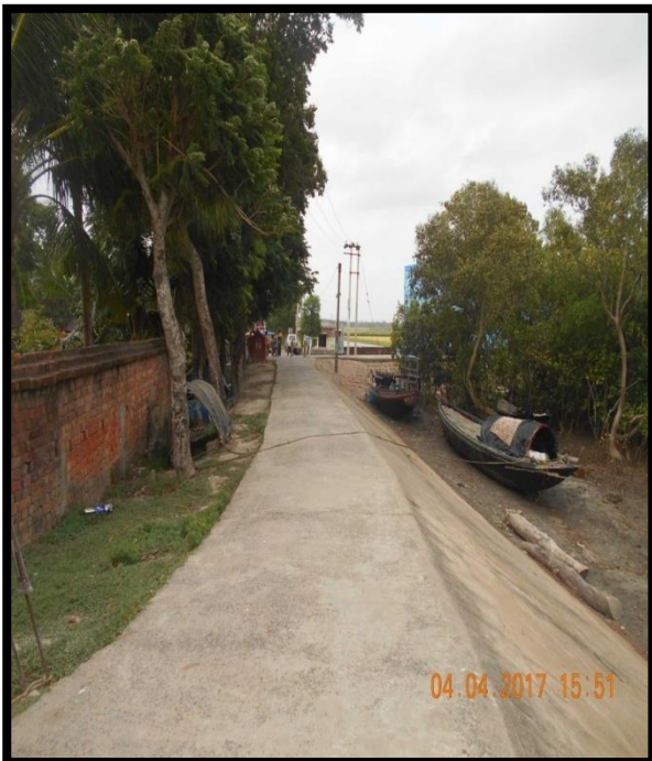
ROAD OF KAIKHALI JETTY AT CHAINAGE 57.5, LEFT BANK
