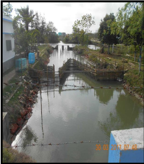
WATER LOCK NEAR ML-01 AT CHAINAGE 58, RIGHT BANK
