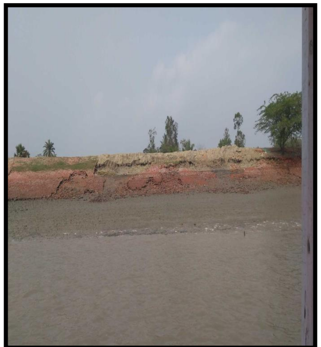
BANK PROTECTION WALL AT CHAINAGE 82.5, RIGHT BANK
