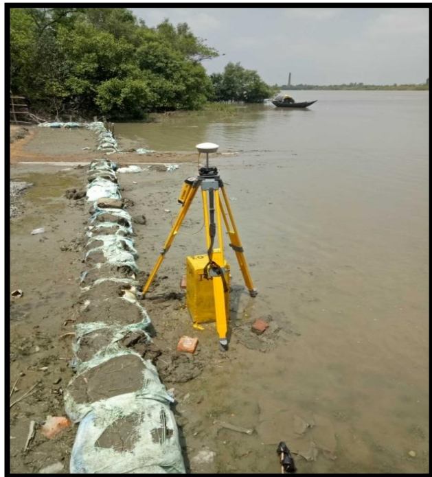
BASE OBSERVATION AT CHAINAGE 80.5, RIGHT BANK
