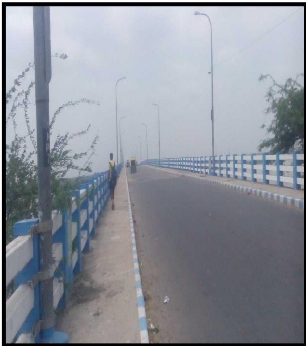
BRIDGE AT CHAINAGE 98.5, CANNING
