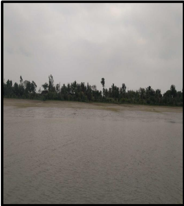
RIVER BANK AT CHAINAGE 71, RIGHT BANK
