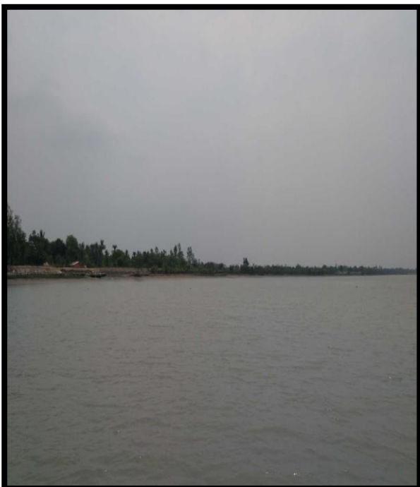
MANGROVES AT CHAINAGE 73.5, RIGHT BANK
