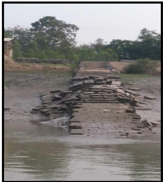
JETTY AT CHAINAGE 58.5, RIGHT BANK
