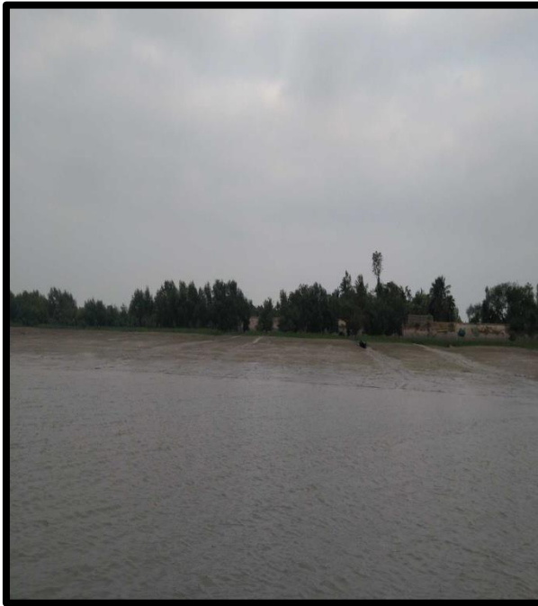
RIVER BANK AT CHAINAGE 71.5, LEFT BANK
