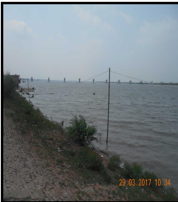
UNDER CONSTRUCTION BRIDGE PILLAR AT CHAINAGE 98
