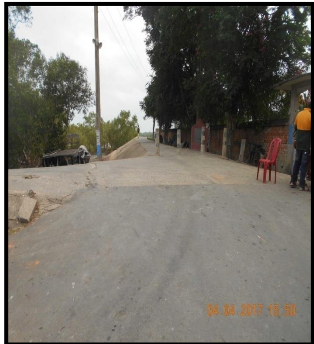
ROAD TOWARD KAIKHALI JETTY AT CHAINAGE 57.5, LEFT BANK
