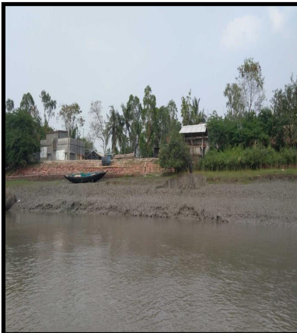
RIVER BANK PROTECTION AT CHAINAGE 99, RIGHT BANK
