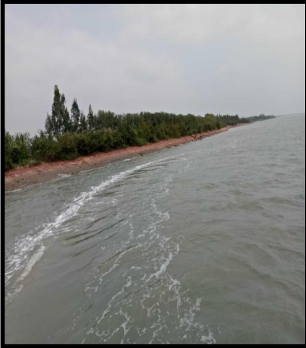
RIVER BANK PROTECTION AT CHAINAGE 55.7, LEFT BANK
