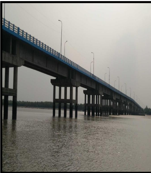
BRIDGE AT CHAINAGE 98.5, CANNING
