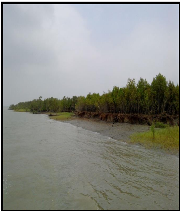
MANGROVES AT CHAINAGE 49, RIGHT BANK
