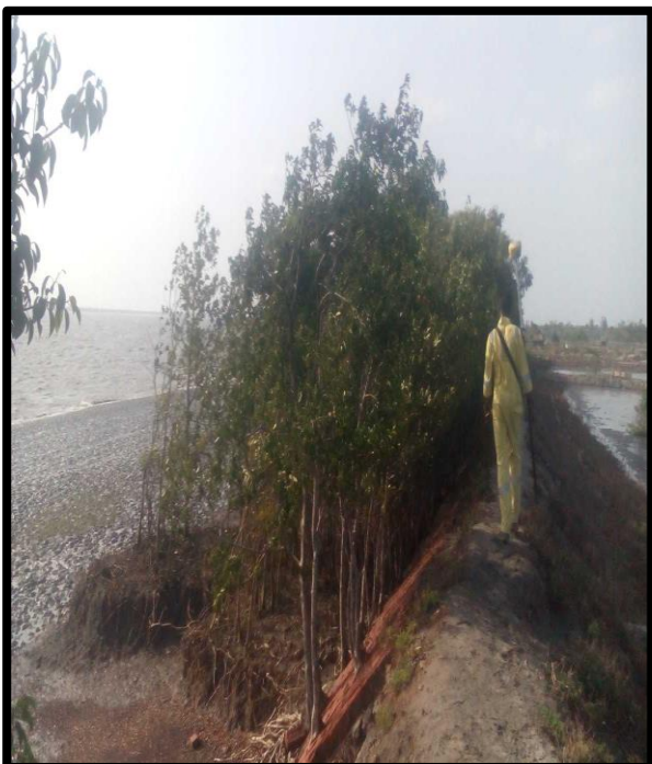
RIVER BANK AT CHAINAGE 65, RIGHT BANK
