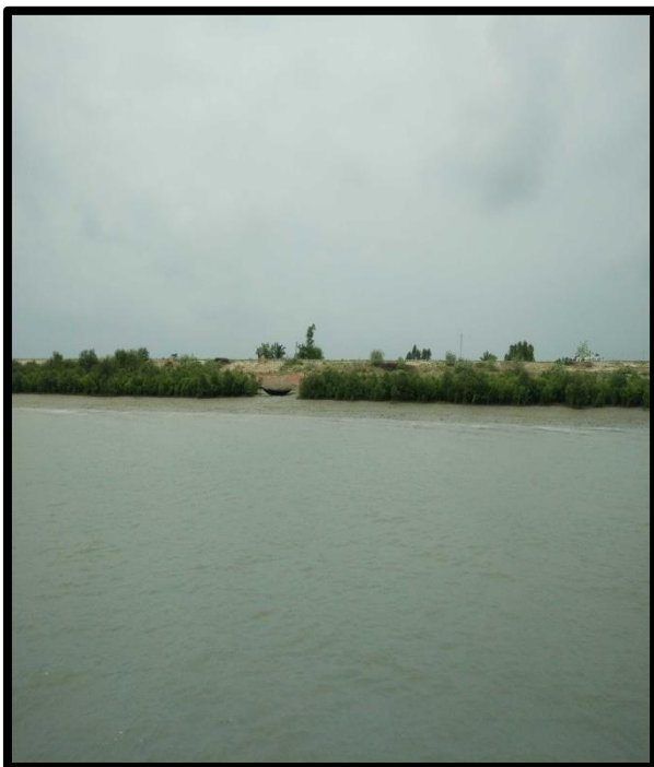
RIVER BANK AT CHAINAGE 58.5, LEFT BANK
