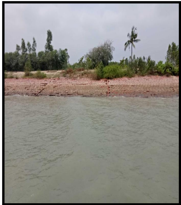
RIVER BANK PROTECTION AT CHAINAGE 54.7, LEFT BANK
