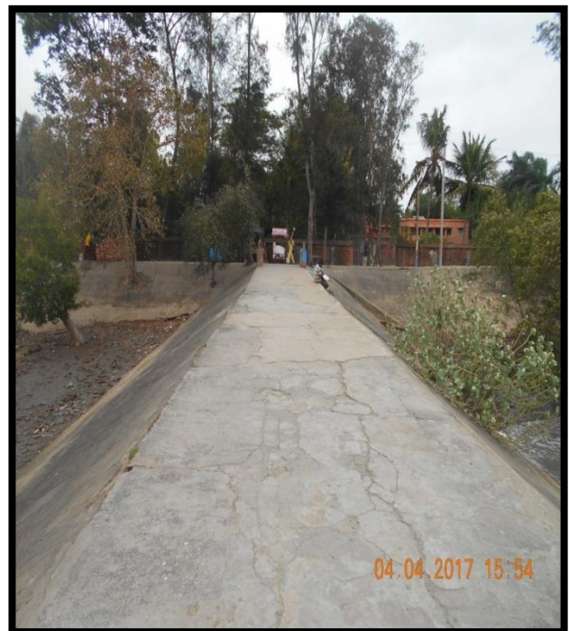
RIVER BANK PROTECTION AT CHAINAGE 57.5, LEFT BANK
