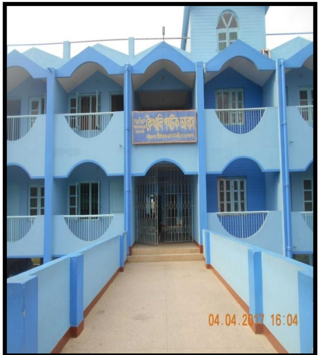
KAIKHALI GUEST HOUSE AT CHAINAGE 57.5, LEFT BANK
