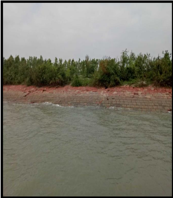
RIVER BANK PROTECTION AT CHAINAGE 55, LEFT BANK
