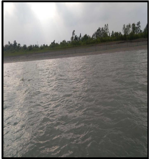
RIVER BANK PROTECTION AT CHAINAGE 71.5, RIGHT BANK
