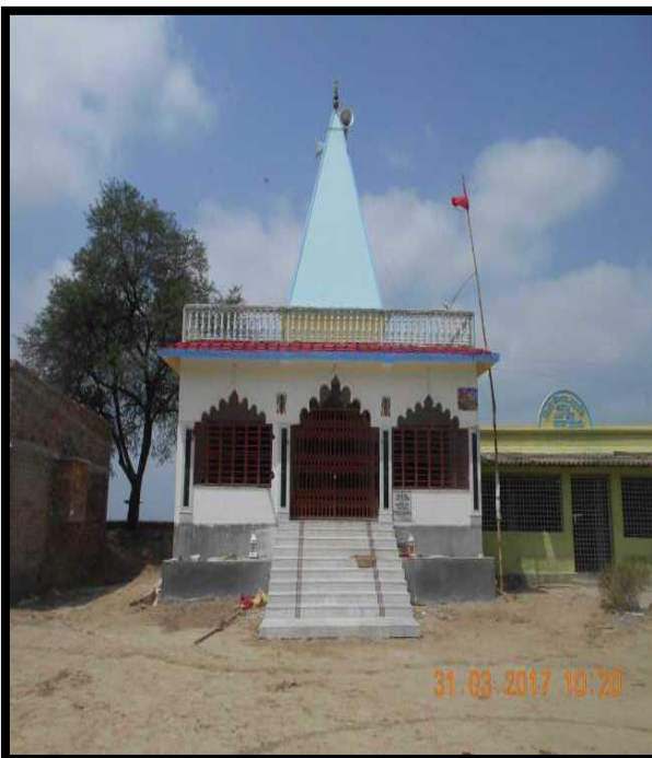
TEMPLE AT CHAINAGE 74.5, RIGHT BANK
