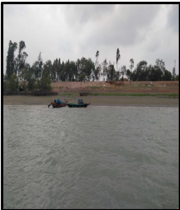
RIVER BANK PROTECTION AT CHAINAGE 71, LEFT BANK
