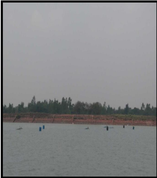
BANK PROTECTION WALL AT CHAINAGE 76.5, LEFT BANK
