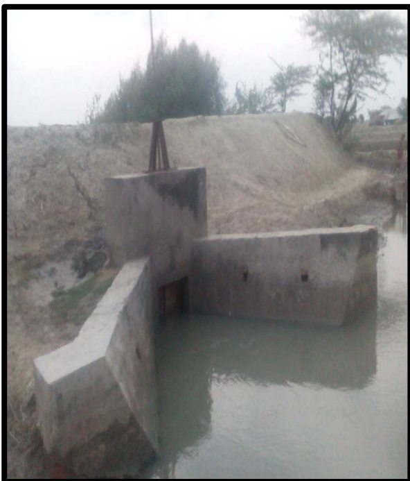
WATER LOCK AT CHAINAGE 63, RIGHT BANK
