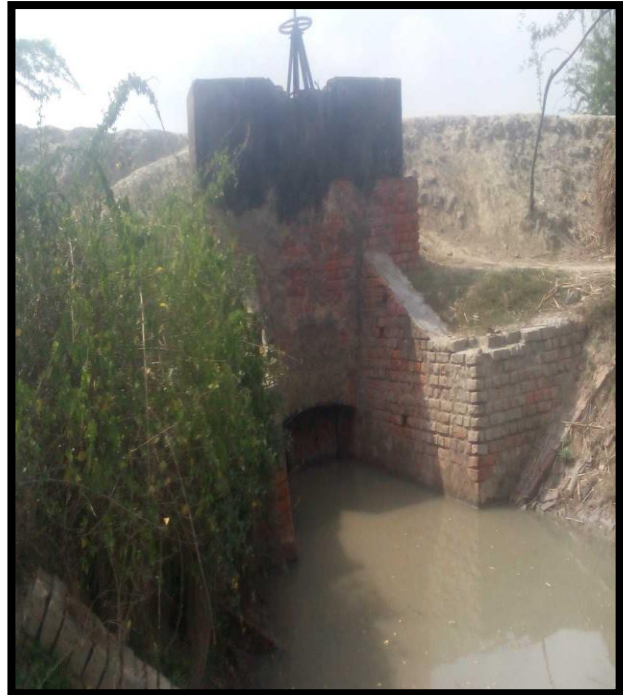
WATER LOCK NALIAKHALI AT CHAINAGE 92.3, LEFT BANK
