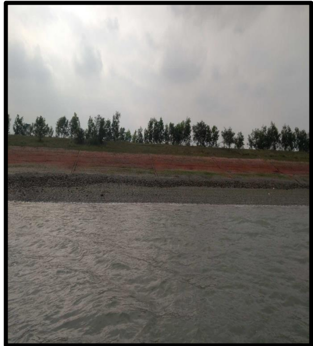
RIVER BANK PROTECTION AT CHAINAGE 70.5, LEFT BANK
