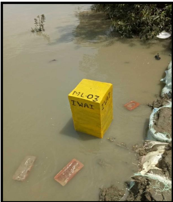
BM ML-03 AT CHAINAGE 80.5, RIGHT BANK
