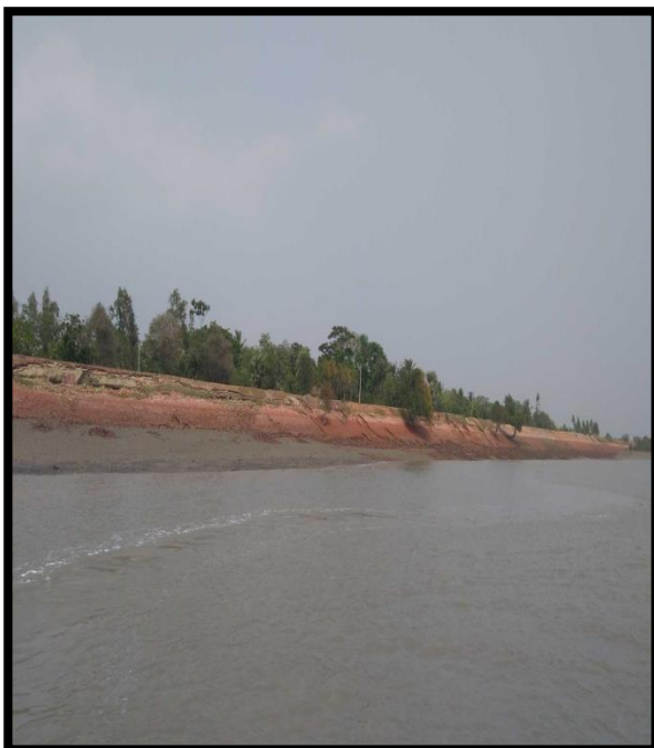
BANK PROTECTION WALL AT CHAINAGE 82, RIGHT BANK
