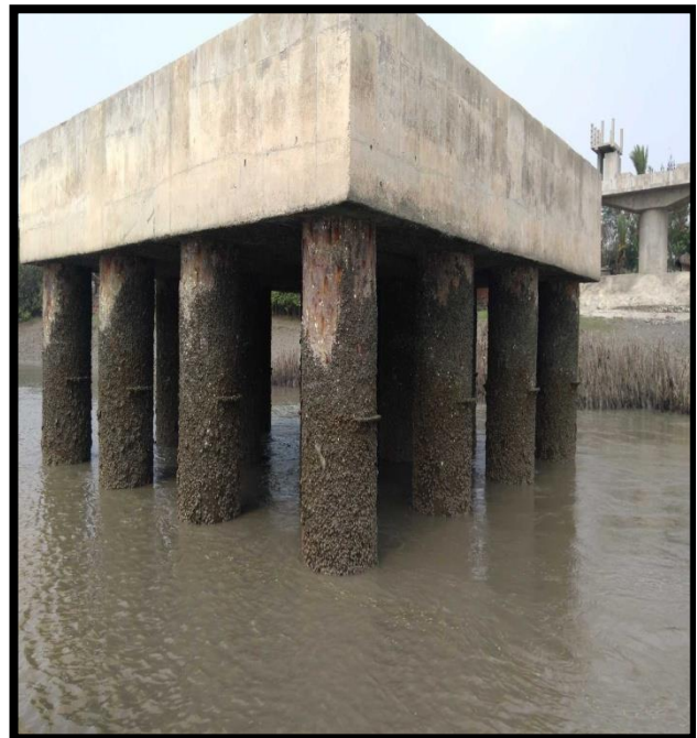
UNDER CONSTRUCTION BRIDGE PILLAR AT CHAINAGE 98
