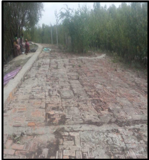
RIVER BANK PROTECTION AT CHAINAGE 64.5, RIGHT BANK
