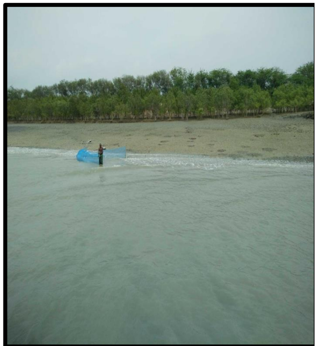
RIVER BANK AT CHAINAGE 63.5, RIGHT BANK
