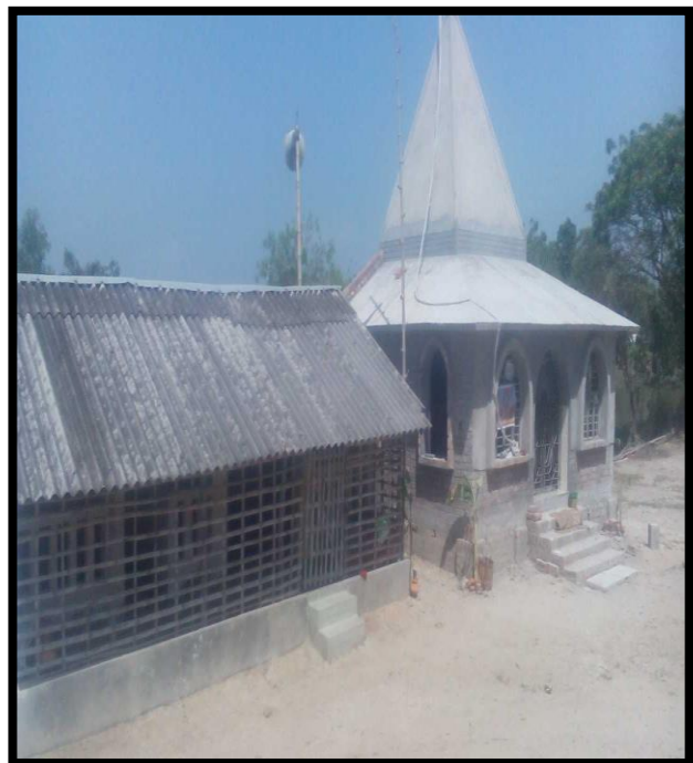
TEMPLE AT CHAINAGE 71, RIGHT BANK
