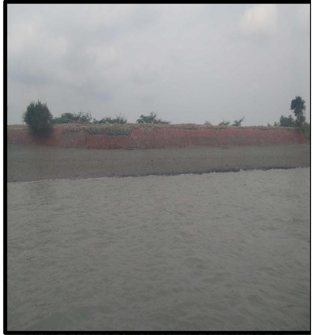
RIVER BANK PROTECTION AT CHAINAGE 67, RIGHT BANK
