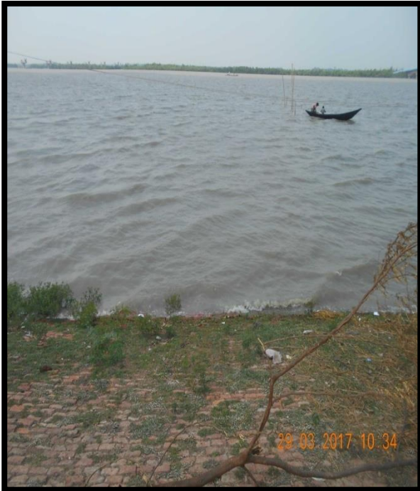
RIVER BANK PROTECTION AT CHAINAGE 98.5, RIGHT BANK
