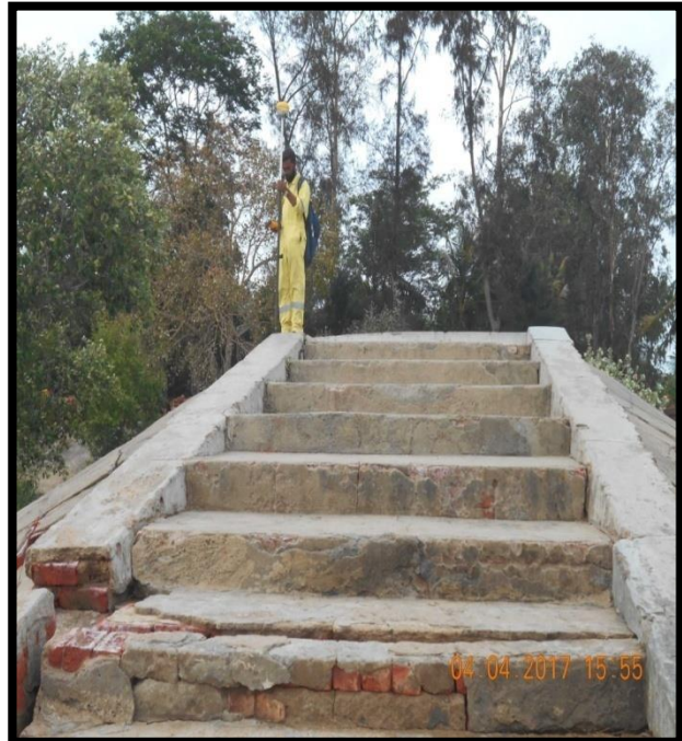
KAIKHALI JETTY AT CHAINAGE 57.5, LEFT BANK
