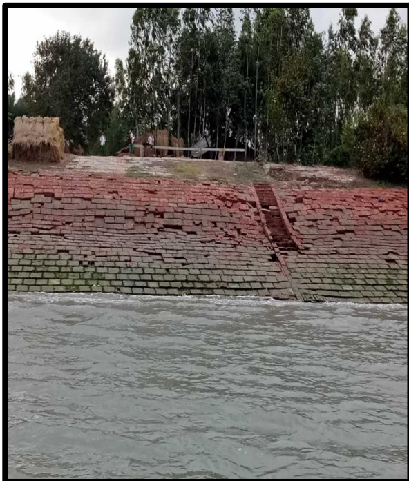
RIVER BANK PROTECTION AT CHAINAGE 55.7, LEFT BANK
