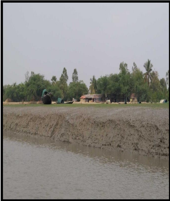
SHALLOW PATCH ON LOW WATER AT CHAINAGE 97.5, RIGHT BANK
