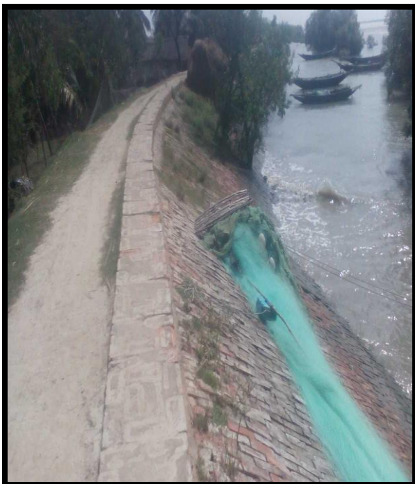
RIVER BANK PROTECTION AT CHAINAGE 70, RIGHT BANK
