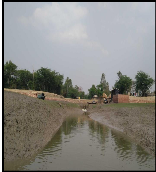
CULVERT AT CHAINAGE 98, RIGHT BANK
