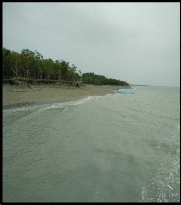
RIVER BANK AT CHAINAGE 63.5, RIGHT BANK
