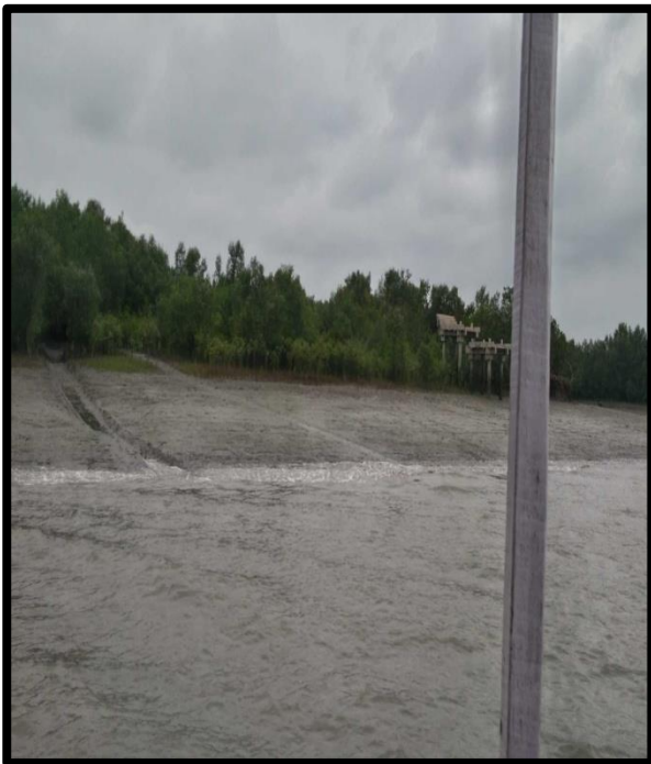
JETTY UNDER CONSTRUCTION AND MANGROVES AT CHAINAGE 60, LEFT BANK
