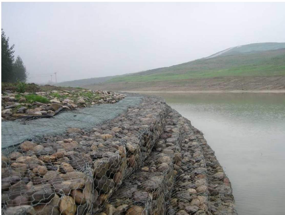
Figure 26: Photograph showing arrangement of Gabion Wall along River Bank
