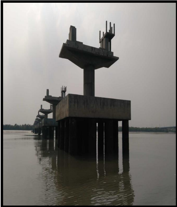
UNDER CONSTRUCTION BRIDGE PILLAR AT CHAINAGE 98
