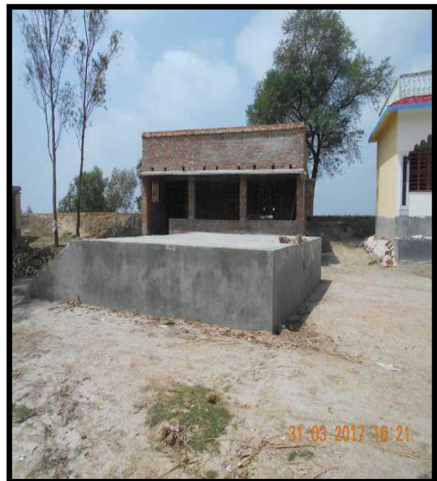
TEMPLE AUDITORIUM AT CHAINAGE 74.5, RIGHT BANK
