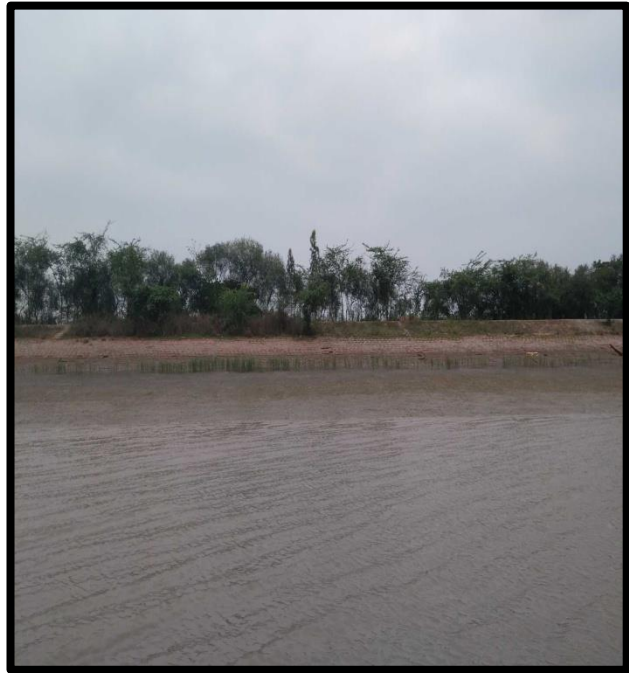
RIVER BANK PROTECTION AT CHAINAGE 72, RIGHT BANK
