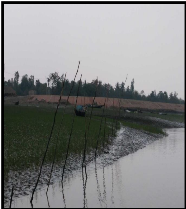
RIVER BANK AT CHAINAGE 94.5, LEFT BANK
