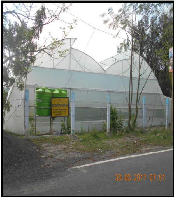
BOTANICAL GARDEN NEAR ML-01 AT CHAINAGE 58, RIGHT BANK
