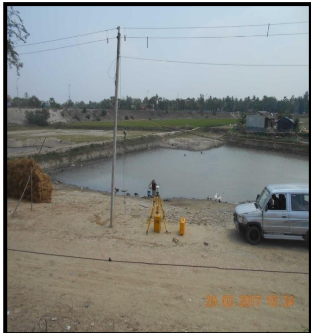
BASE OBSERVATION ON ML-05 AT CHAINAGE
