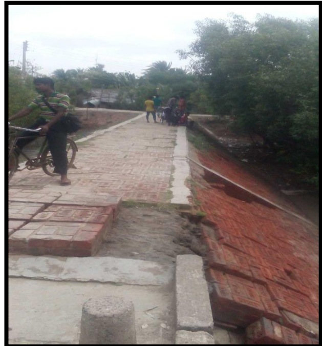
RIVER BANK PROTECTION AT CHAINAGE 74.5, RIGHT BANK
