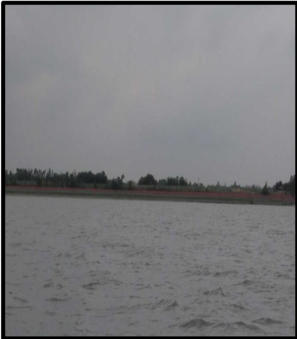
RIVER BANK PROTECTION AT CHAINAGE 60.5, LEFT BANK
