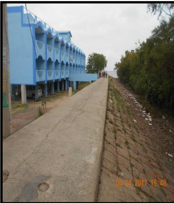
KAIKHALI GUEST HOUSE AT CHAINAGE 57.5, LEFT BANK
