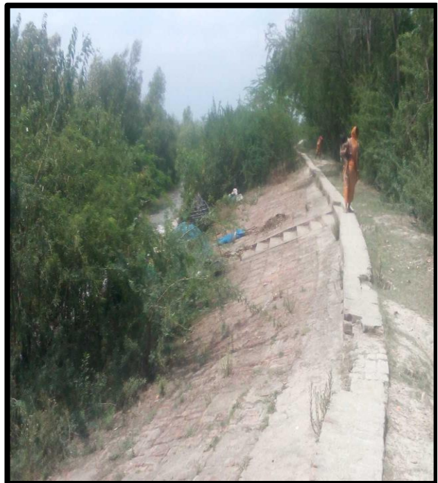
RIVER BANK PROTECTION WALL AT CHAINAGE 65, RIGHT BANK
