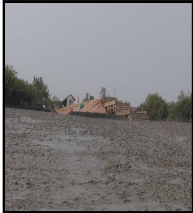
JETTY AT CHAINAGE 84.5, RIGHT BANK
