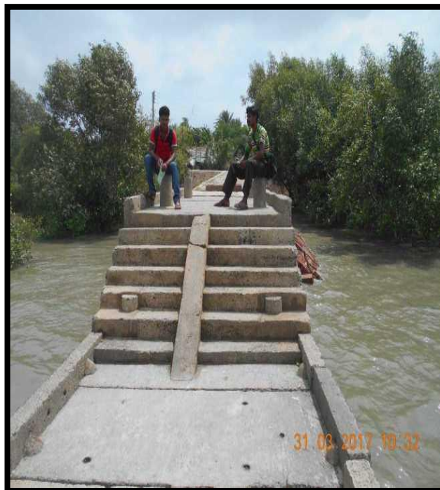
GARANBOSE JETTY NO.1 AT CHAINANGE 74.5, RIGHT BANK
