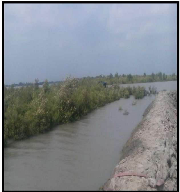
MANGROVE START NALIAKHALI AT CHAINAGE 93.2, LEFT BANK
