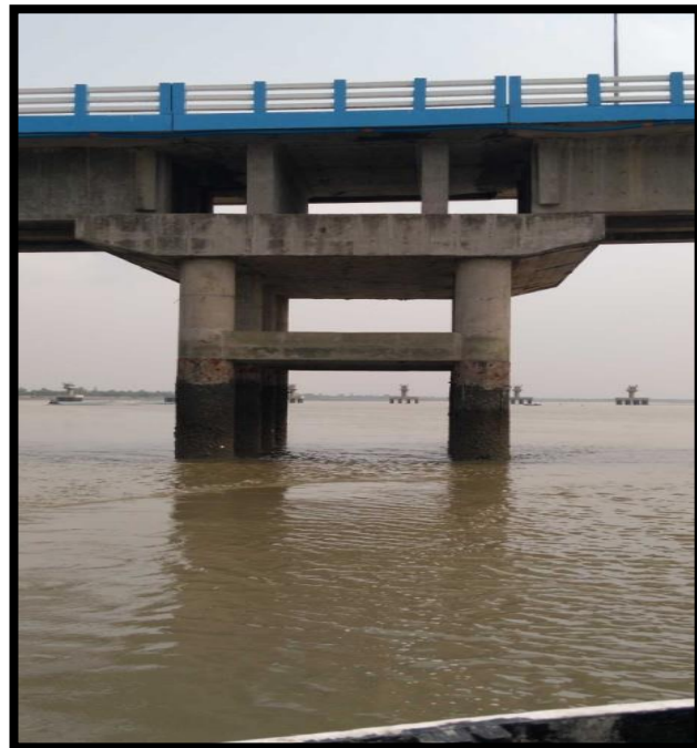
BRIDGE PILLAR AT CHAINAGE 98.5, CANNING
