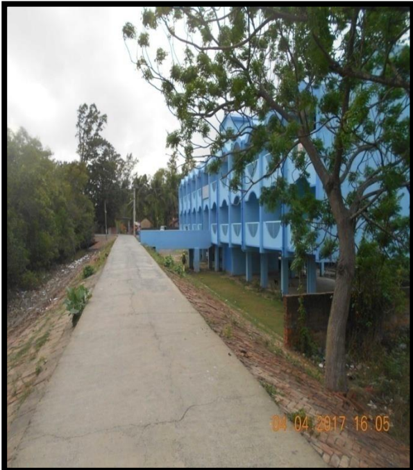
KAIKHALI GUEST HOUSE AT CHAINAGE 57.5, LEFT BANK
