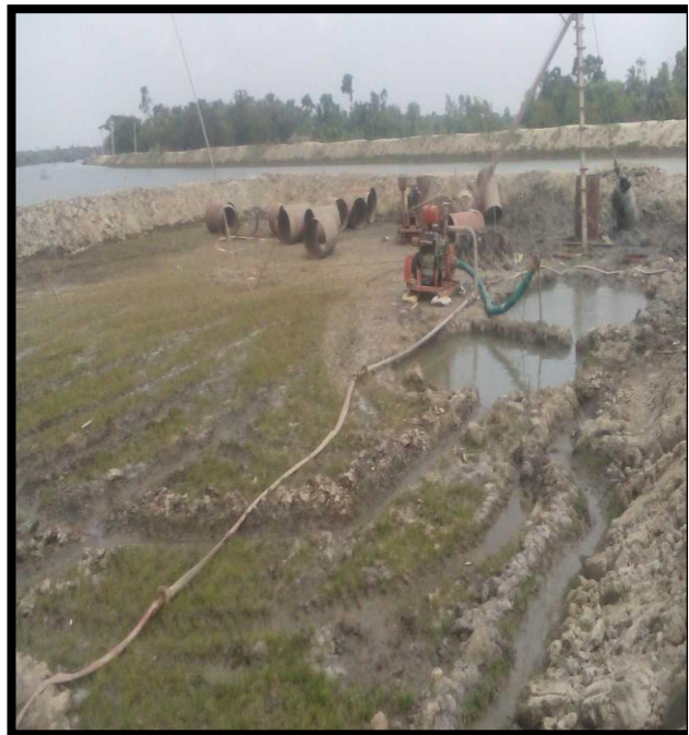
PYLON NEW CONSTRUCTION SITE NALIAKHALI AT CHAINAGE 93.2, LEFT BANK
