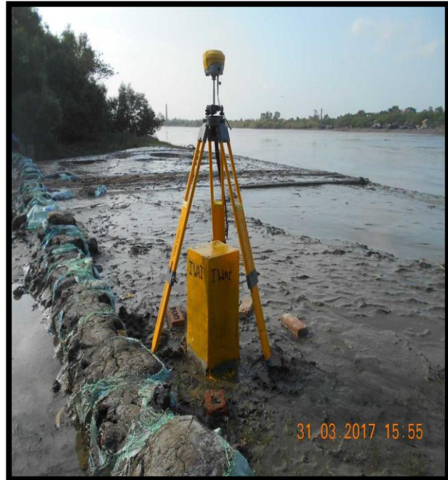
BASE STATION ML-03 AT CHAINAGE 80.5, RIGHT BANK
