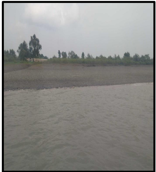
RIVER BANK AT CHAINAGE 67.5, RIGHT BANK
