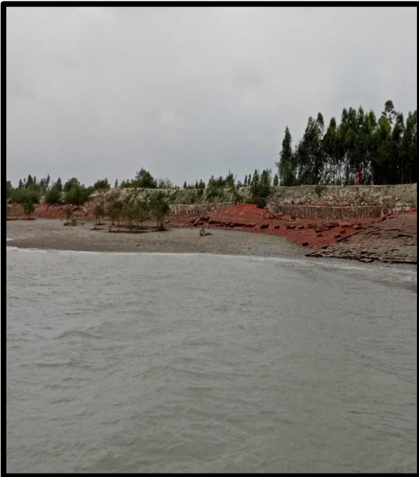
RIVER BANK PROTECTION AT CHAINAGE 56, LEFT BANK
