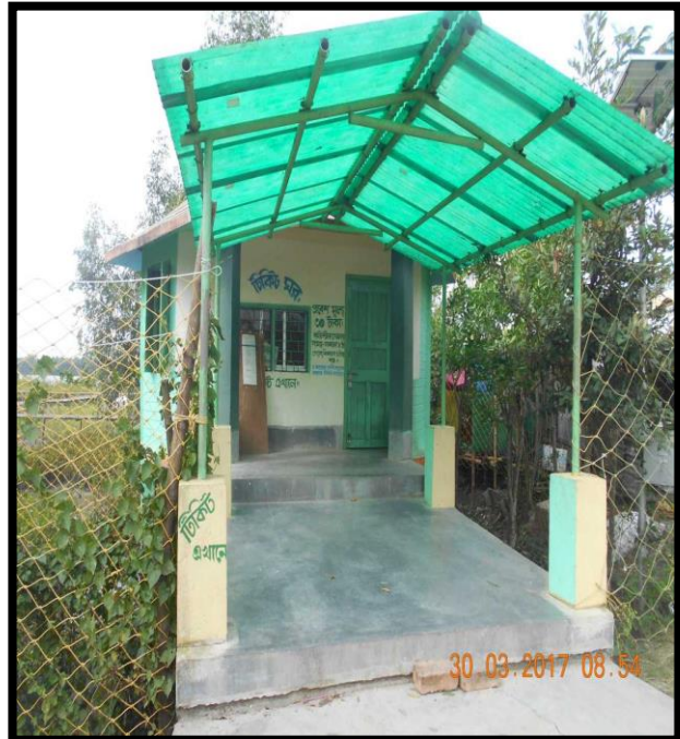
TICKET COUNTER BOTANICAL GARDEN NEAR ML-01 AT CHAINAGE 58, RIGHT BANK
