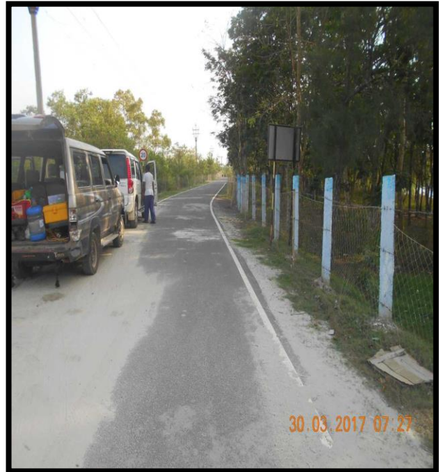
ROAD NEAR BM-01 AT CHAINAGE 58, RIGHT BANK
