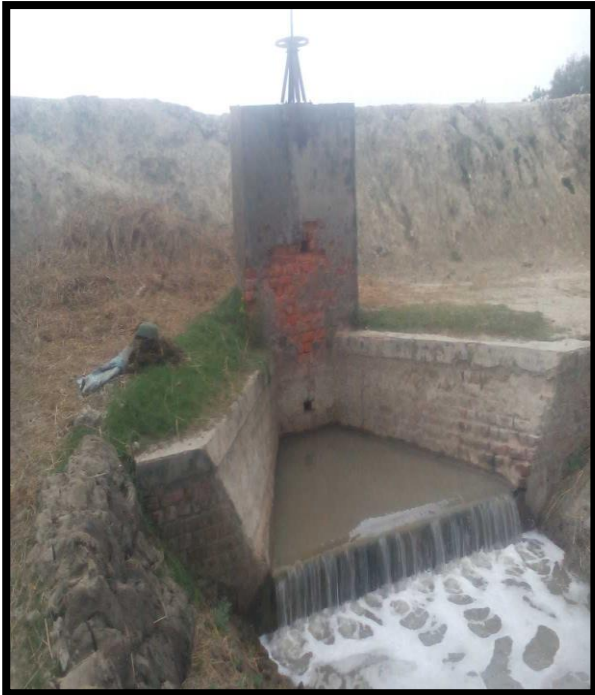
WATER LOCK NALIAKHALI AT CHAINAGE 92.2, LEFT BANK
