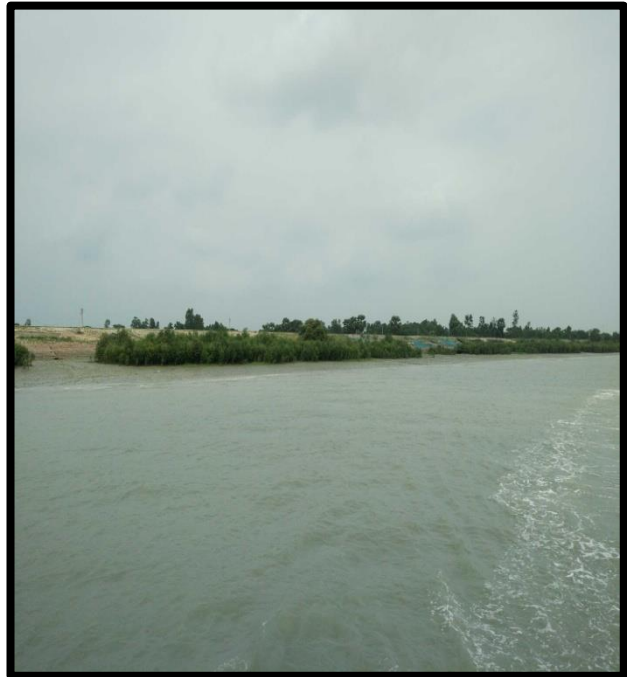
RIVER BANK AT CHAINAGE 58.5, LEFT BANK
