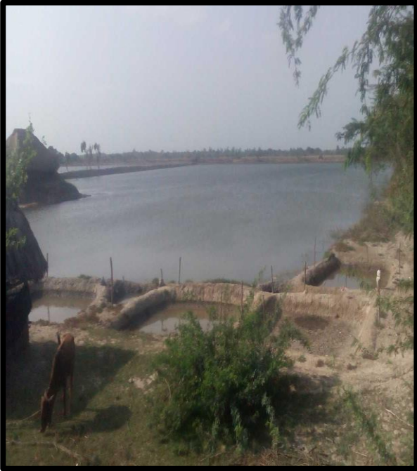
FISHING POND AT CHAINAGE 64.9, RIGHT BANK
