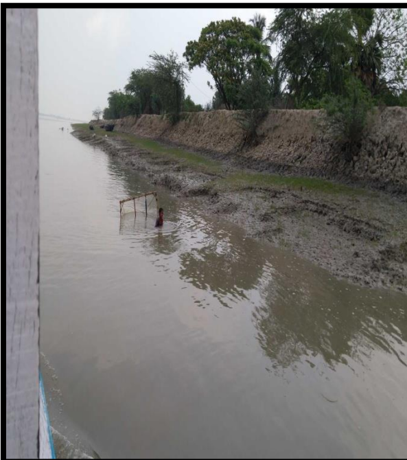
RIVER BANK AT CHAINAGE 91.5, RIGHT BANK
