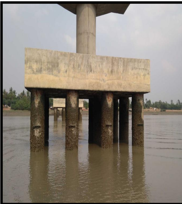
UNDER CONSTRUCTION BRIDGE PILLAR AT CHAINAGE 98
