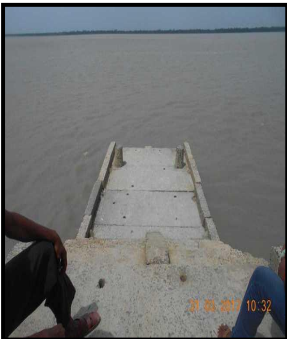
GARANBOSE JETTY NO.1 AT CHAINANGE 74.5, RIGHT BANK
