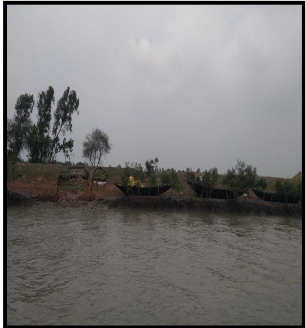
BANK PROTECTION WALL AT CHAINAGE 77.5, LEFT BANK
