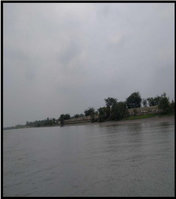
BANK PROTECTION AT CHAINAGE 73, LEFT BANK
