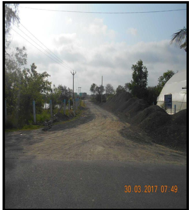
ECO TOURISM HUB ROAD AT CHAINAGE 58, RIGHT BANK
