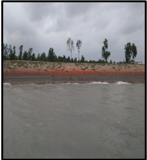
RIVER BANK PROTECTION AT CHAINAGE 57, LEFT BANK
