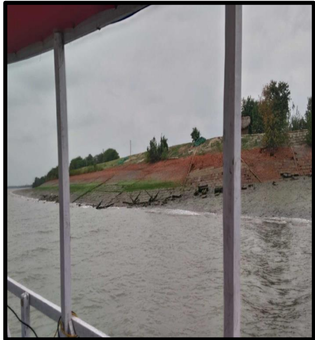
RIVER BANK PROTECTION AT CHAINAGE 60.5, LEFT BANK
