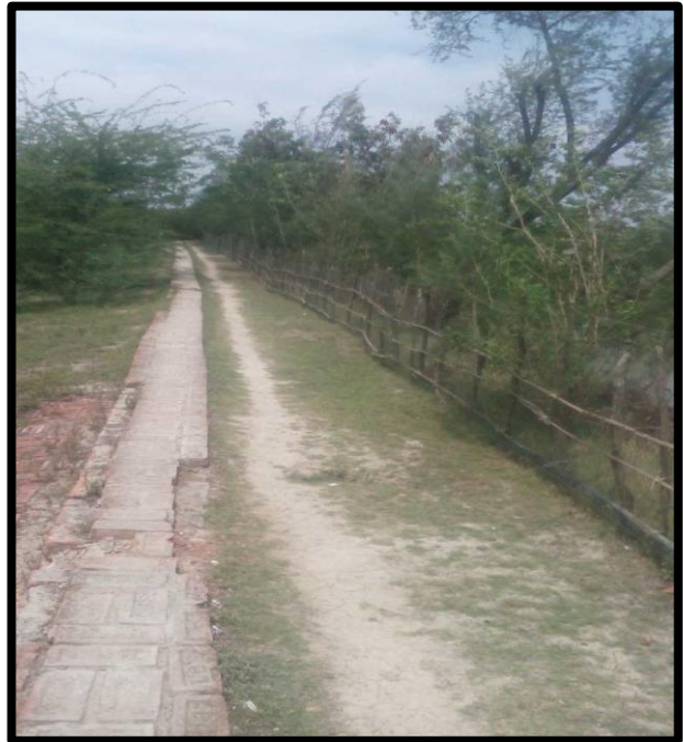
FENCE AT CHAINAGE 63, RIGHT BANK
