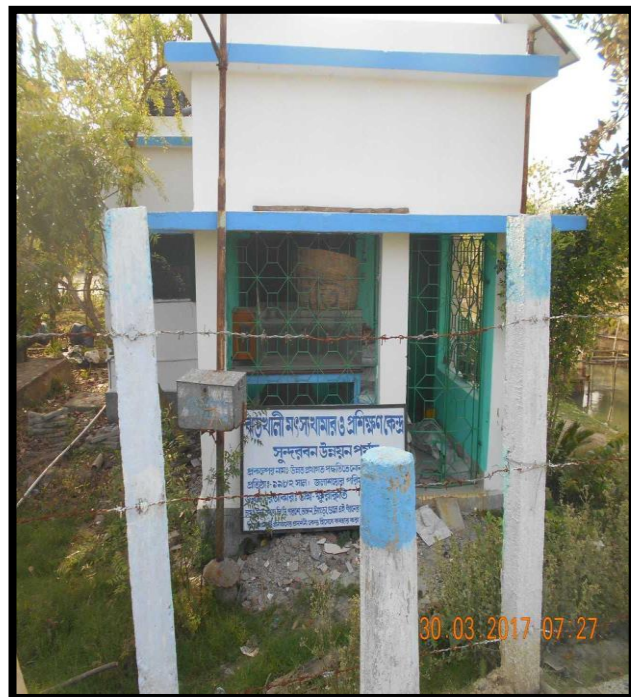
FISHERY PROJECT AND TRAINING CENTER AT CHAINAGE 58, RIGHT BANK
