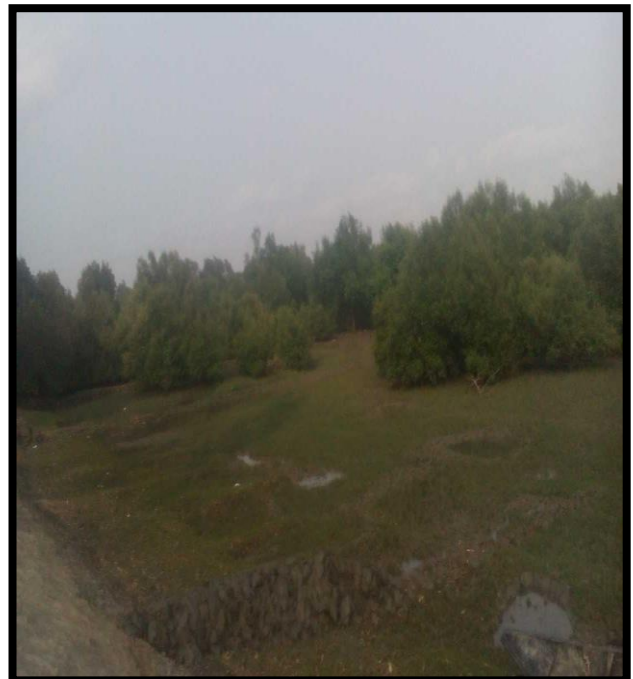
MANGROVE END GARKHALI AT CHAINAGE 87.3, RIGHT BANK
