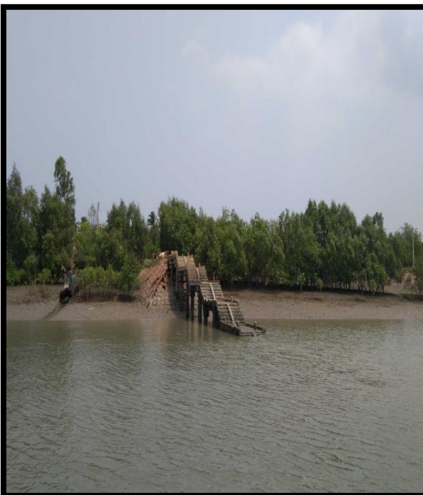
JETTY AT CHAINAGE 75, RIGHT BANK
