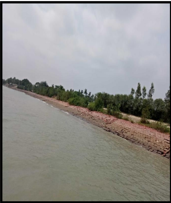
RIVER BANK PROTECTION AT CHAINAGE 54.7, LEFT BANK
