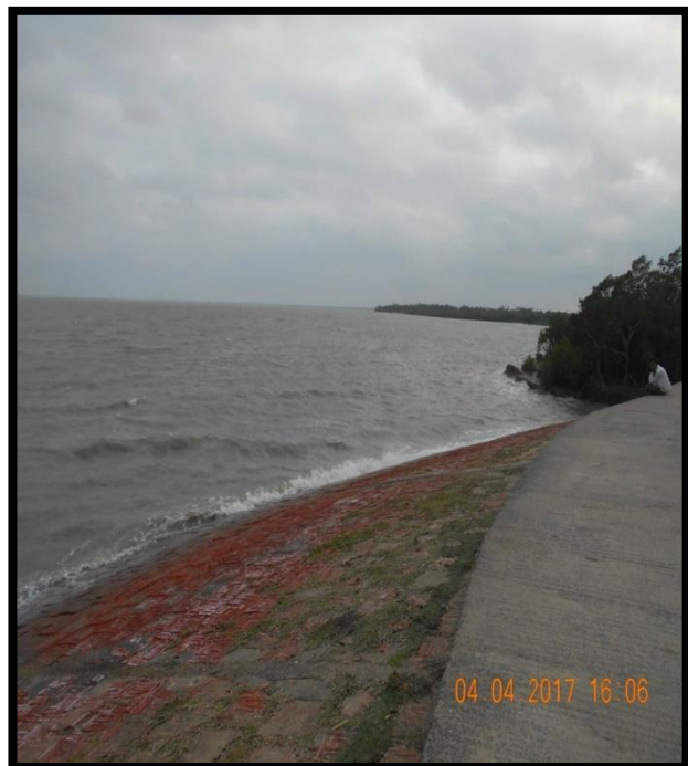
RIVER BANK PROTECTION CHAINAGE 57.5, LEFT BANK
