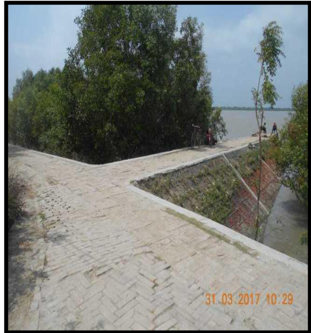
GARANBOSE JETTY NO.1 AT CHAINANGE 74.5, RIGHT BANK
