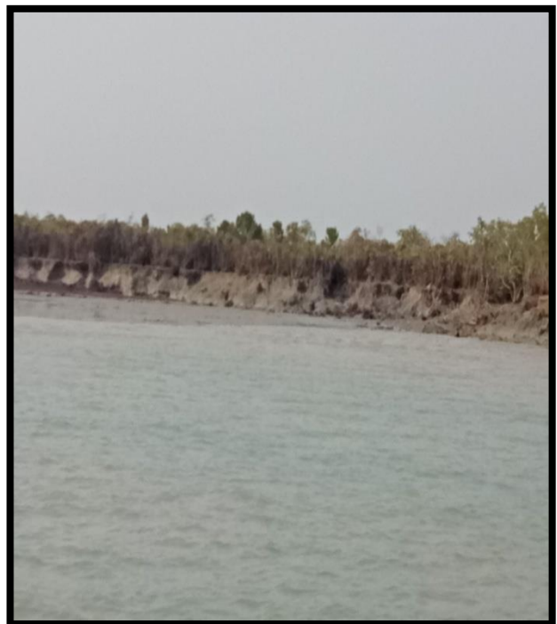
RIVER BANK AT CHAINAGE 45, RIGHT BANK
