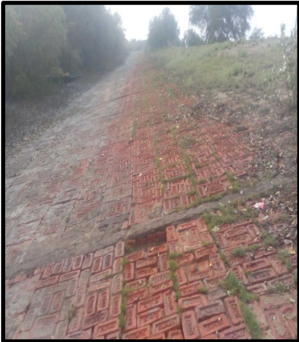
RIVER BANK PROTECTION AT CHAINAGE 63, RIGHT BANK GONGAMALA
