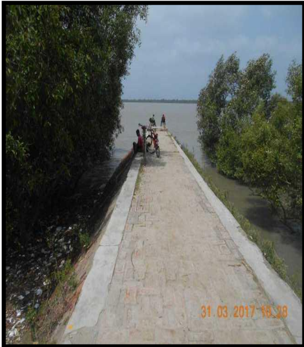
GARANBOSE JETTY NO.1 AT CHAINANGE 74.5, RIGHT BANK
