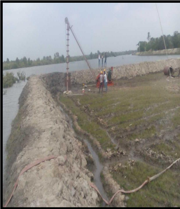
PYLON NEW CONSTRUCTION SITE NALIAKHALI AT CHAINAGE 93.2, LEFT BANK
