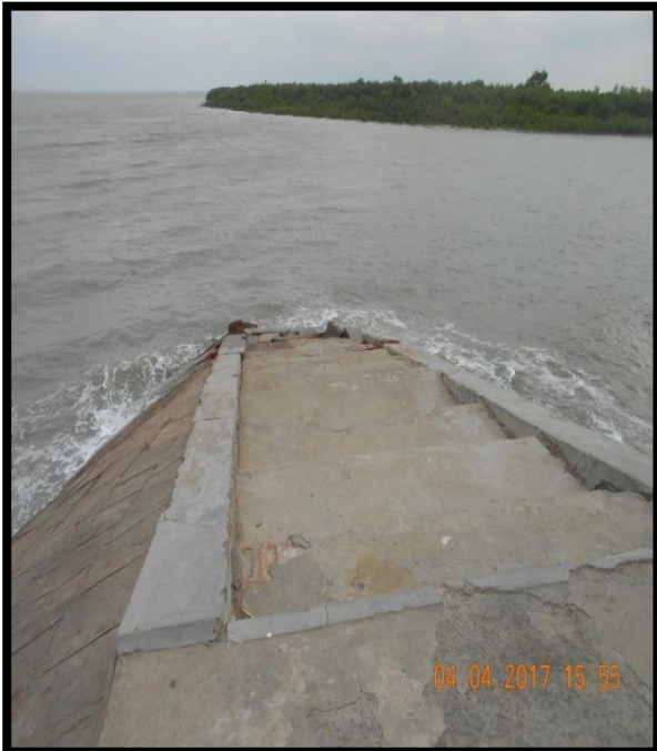
KAIKHALI JETTY AT CHAINAGE 57.5, LEFT BANK
