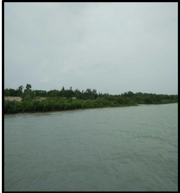
RIVER BANK AT CHAINAGE 59, LEFT BANK
