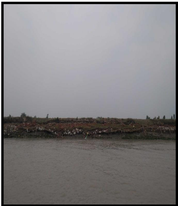
BANK PROTECTION AT CHAINAGE 77.5, LEFT BANK
