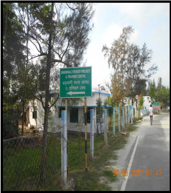
FISHERY PROJECT AND TRINING CENTER AT CHAINAGE 58, RIGHT BANK
