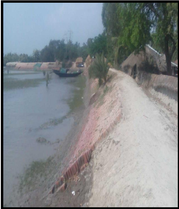
RIVER BANK PROTECTION AMRATALA 90.3, LEFT BANK
