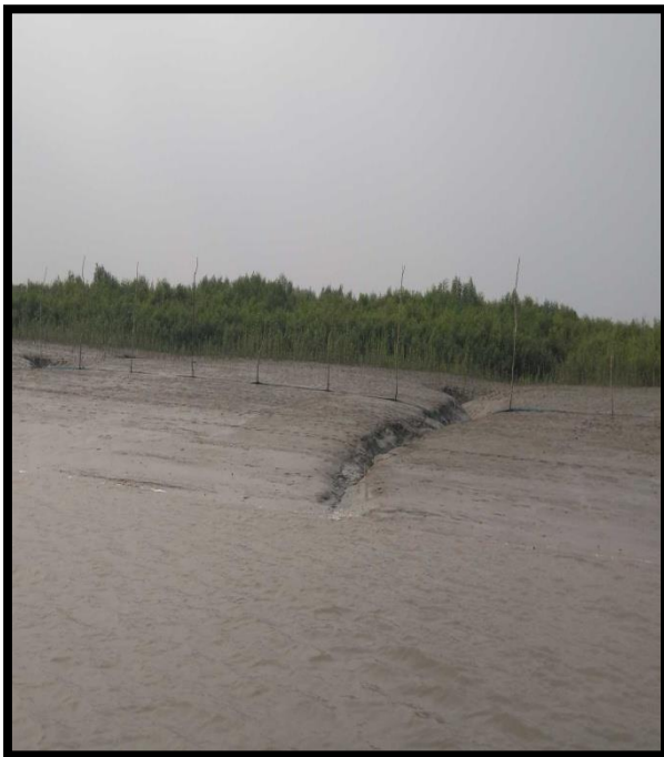
RIVER BANK AT CHAINAGE 85, RIGHT BANK
