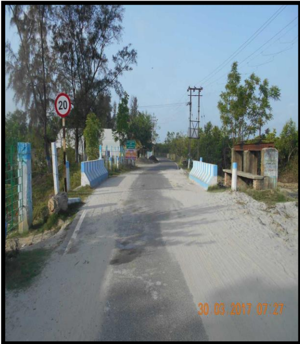
ROAD NEAR TBM-01 AT CHAINAGE 58, RIGHT BANK
