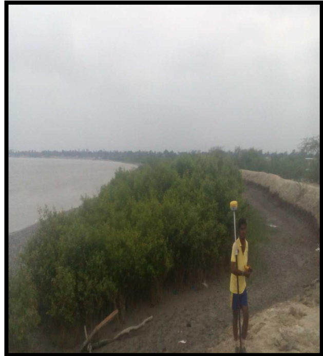
MANGROVE START AT CHAINAGE 88.1, RIGHT BANK
