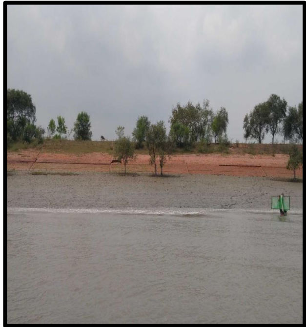
RIVER BANK PROTECTION AT CHAINAGE 69, RIGHT BANK
