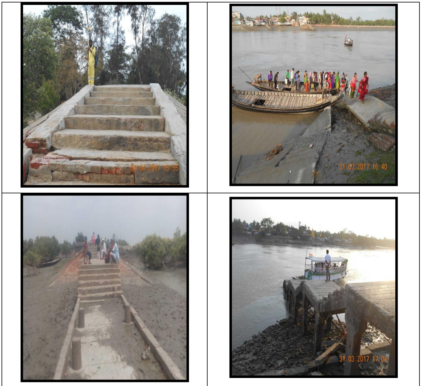
Figure 42: Photographs of Jetties located along Matla Waterway
