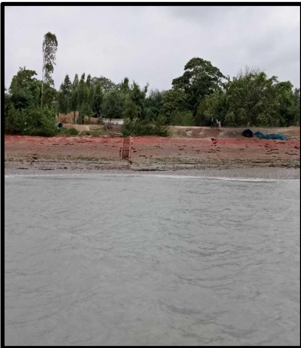
RIVER BANK PROTECTION AT CHAINAGE 56, LEFT BANK
