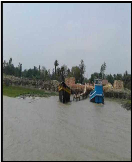
Wooden Jetty at Chainage 10.0
