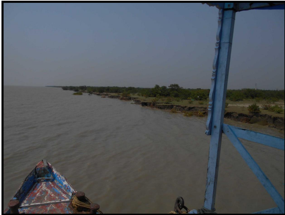
Un Protected Bank at Chainage 23.2
