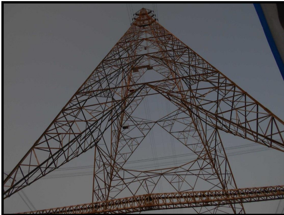
High Tension Wire Crossing at Kakdwip
