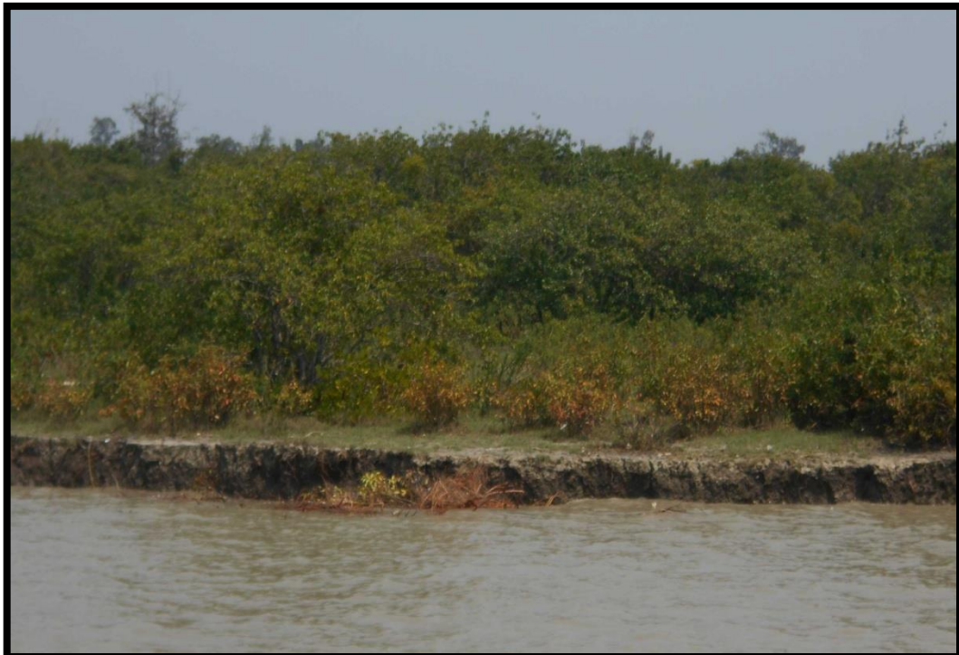
River Bank at Chainage 22.2
