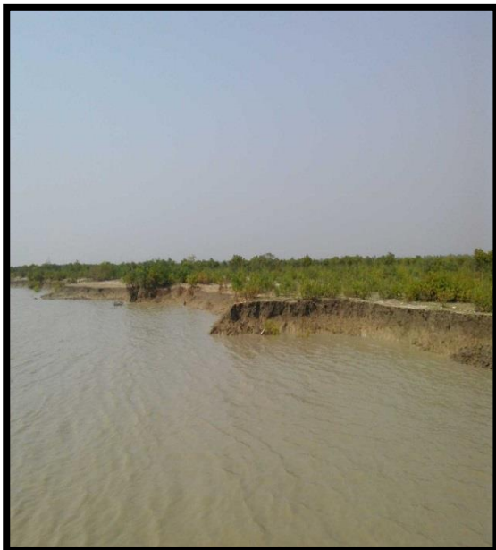
Unprotected River Bank At Chainage 25
