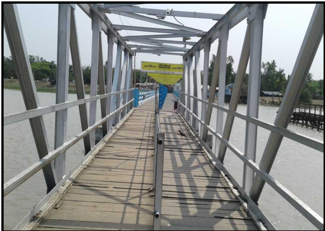
Jetty at Kachuberia (near Kastala) at Chainage 26.5
