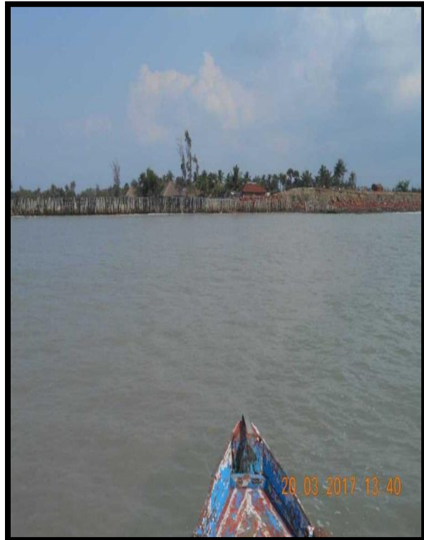
Left Bank Protection at Chainage 3.0
