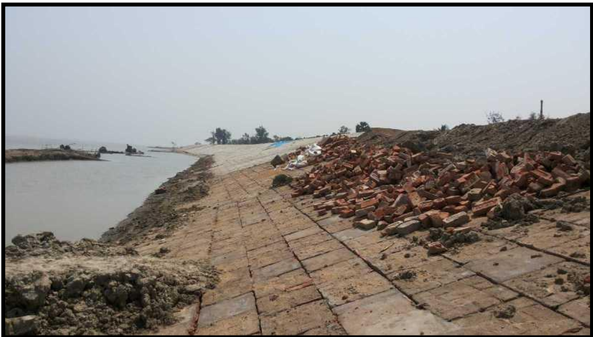
Protected Bank at Chainage 21.5
