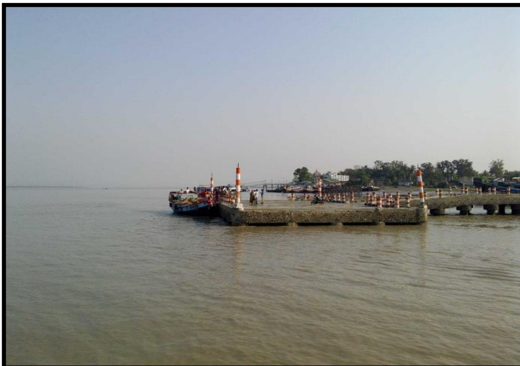
Ferry Berthing Point at Chainage 26.9
