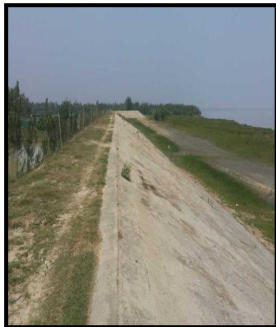
Bank Protection at Chainage 12.7
