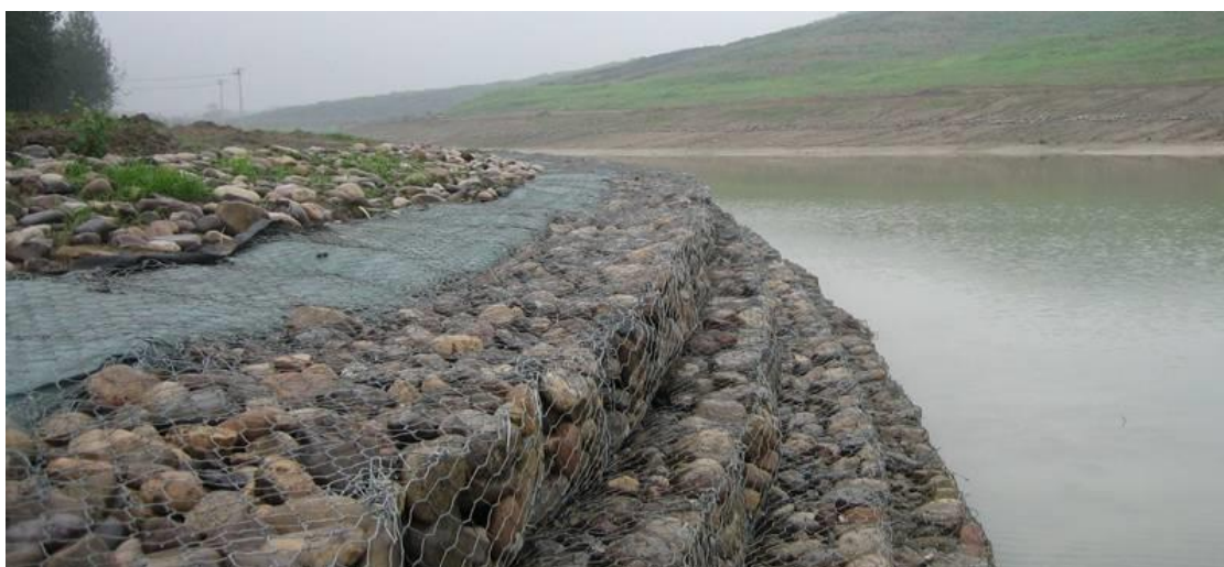
Figure 15: Photograph showing arrangement of Gabion Wall along River Bank
