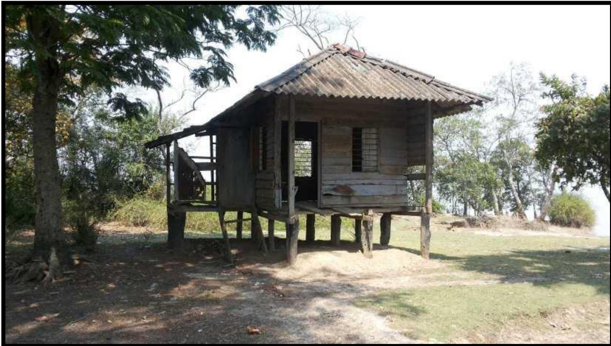
Old Forest Office at Shikarpur at Chainage 20.7
