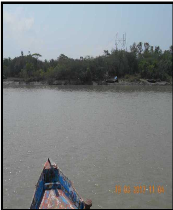
Pylon Construction at Chainage 3.0
