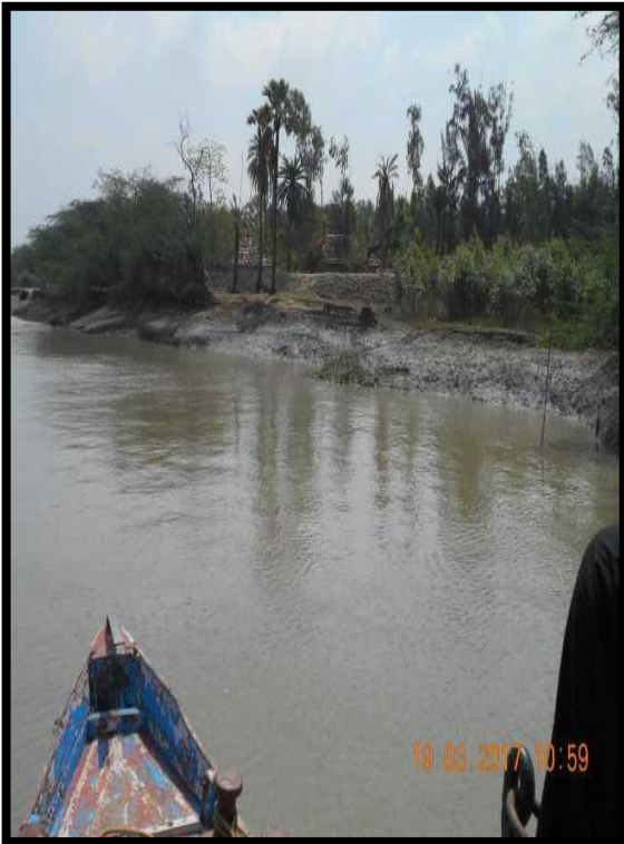
Un protected Right Bank at Chainage 3.0
