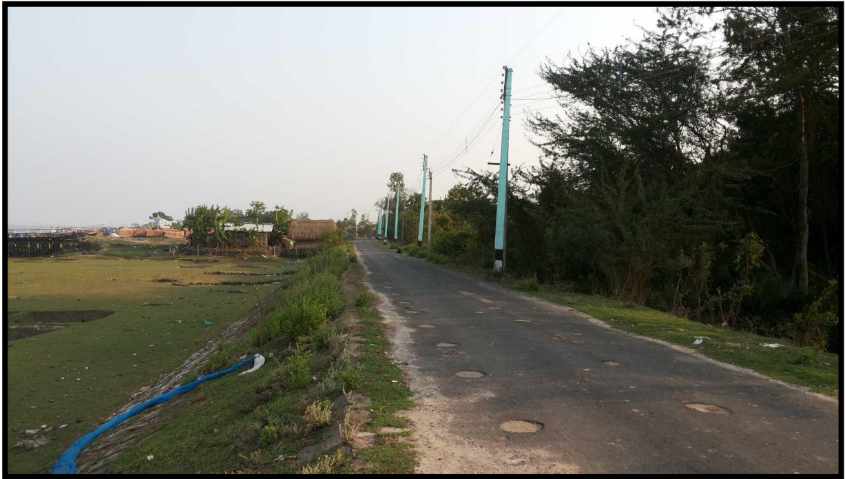
Road near Kachuberia Villaage at Chainage 26.3
