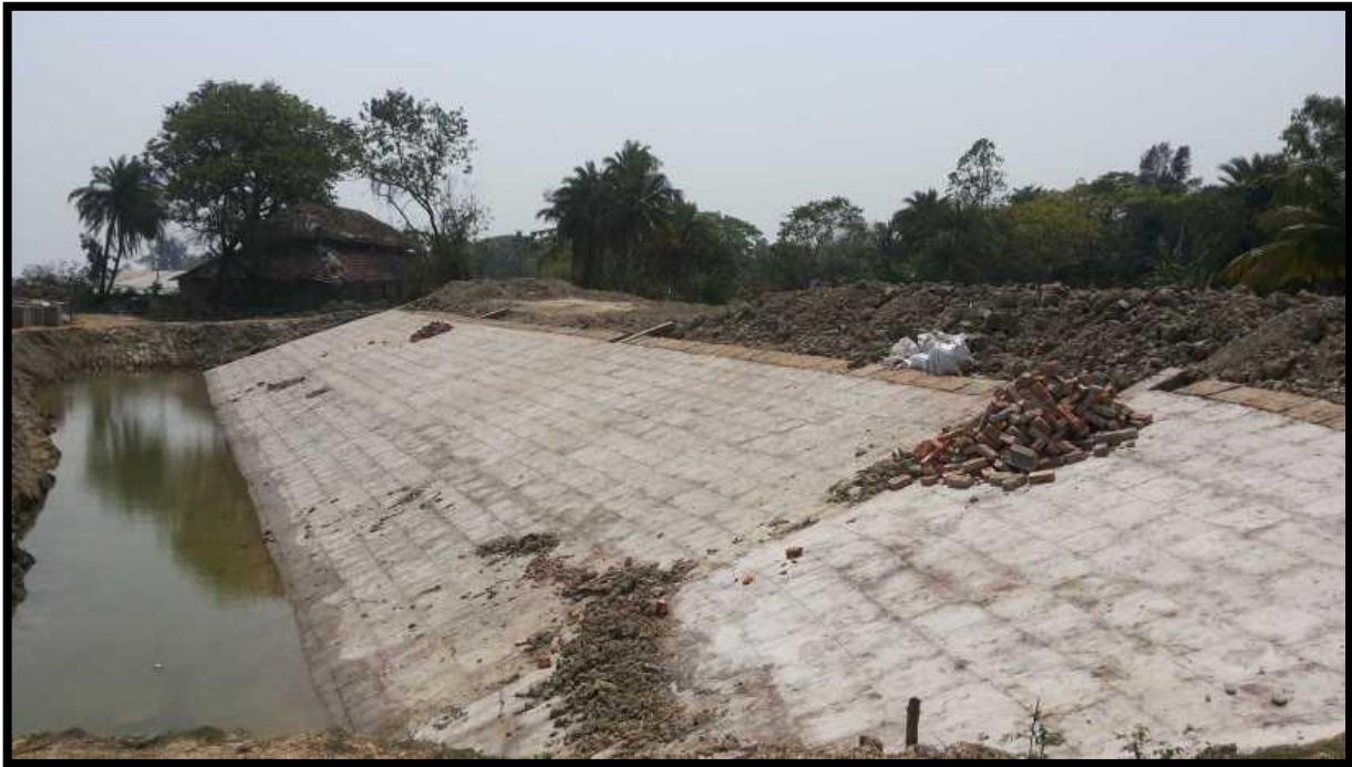
Protected Bank at Chainage 22
