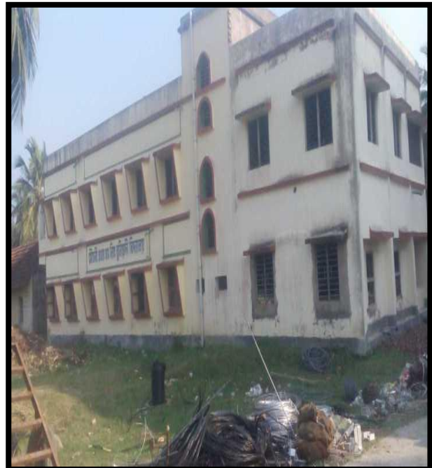
School at Mousani Chainage 7.5
