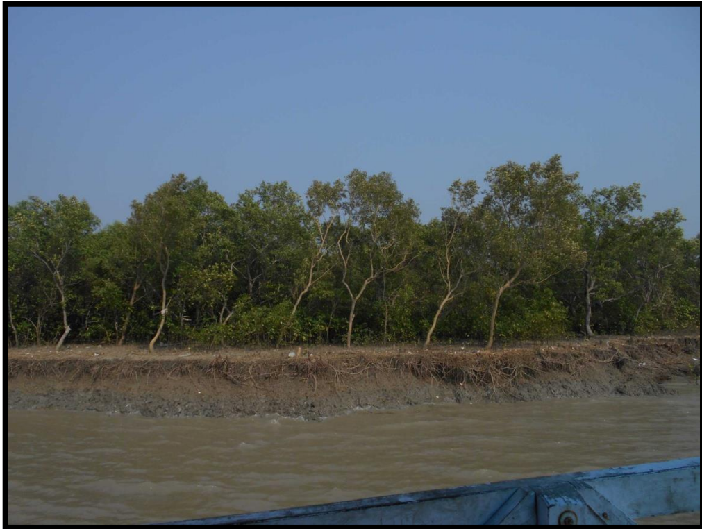
River Bank at Chainage 20.9
