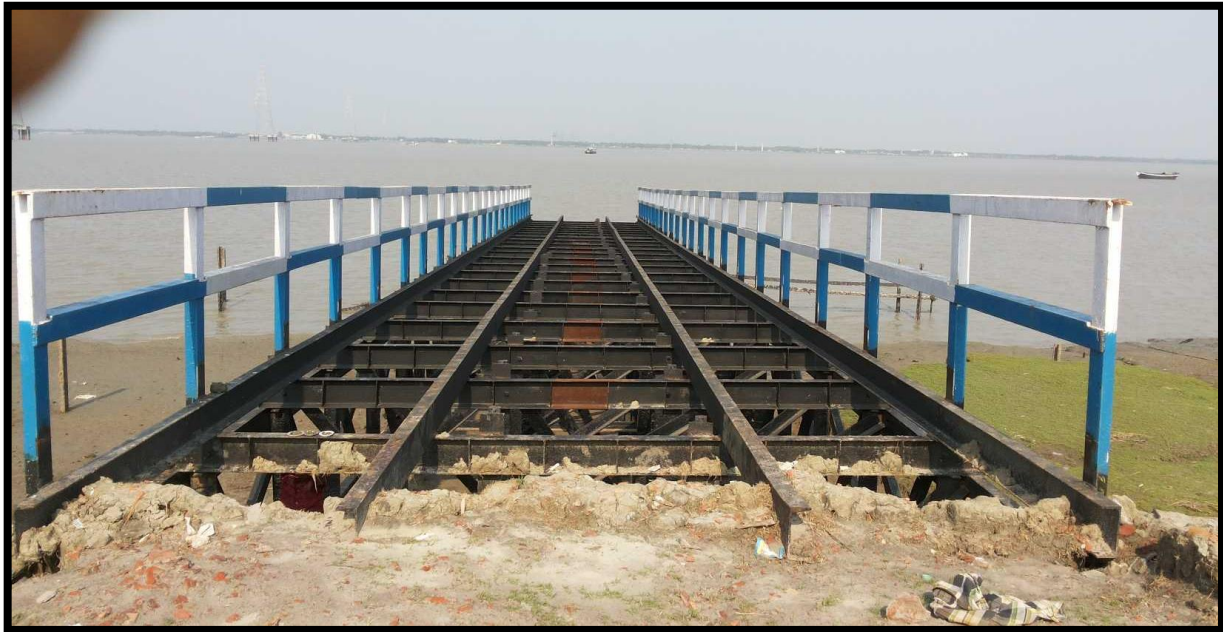
Jetty Under Construction at Chainage 26.2
