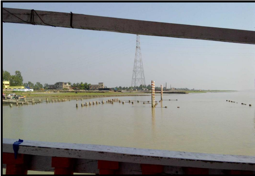
High Tension Wire Crossing at Kakdwip
