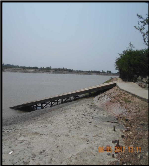
PANCHI GHAT JETTY AT CHAINAGE 44, RIGHT BANK
