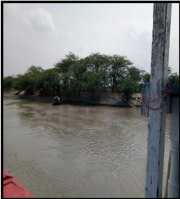
RIVER BANK AT CHAINAGE 47.5, RIGHT BANK
