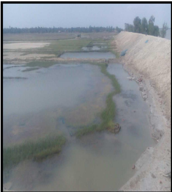
POND AT CHAINAGE 11, LEFT BANK
