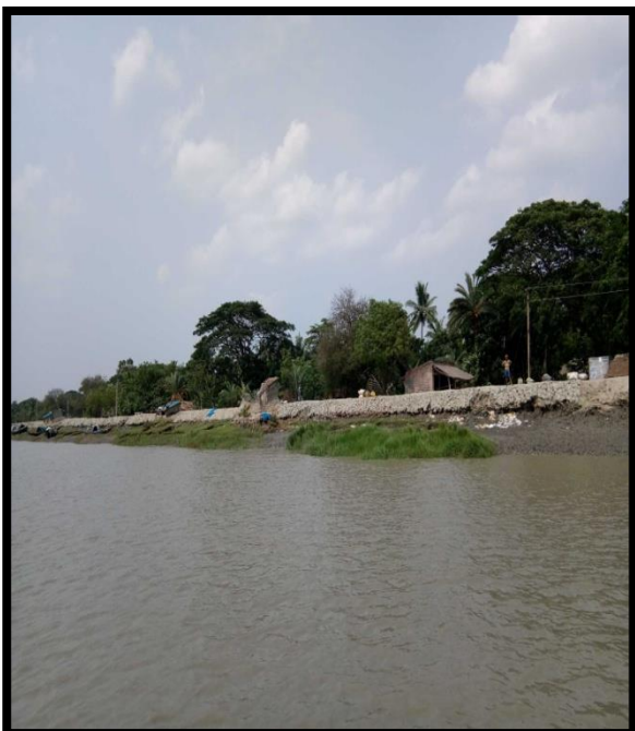
RIGHT RIVER BANK AT CHAINAGE 34.5
