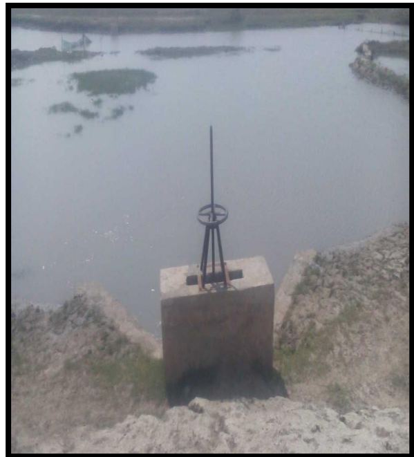
WATER LOCK AT CHAINAGE 9.2, LEFT BANK
