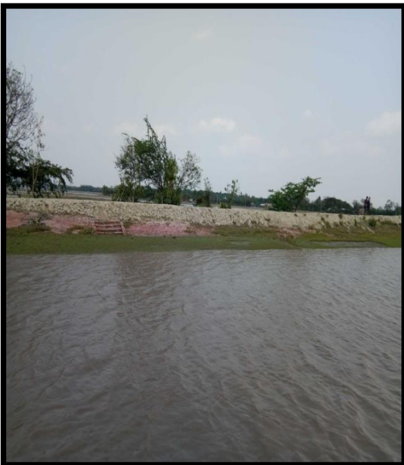
RIVER BANK AT CHAINAGE 43.5, LEFT BANK
