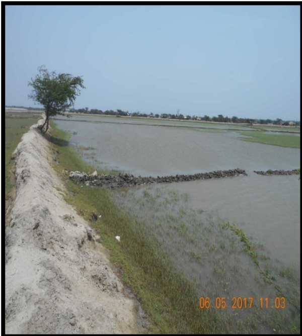
FISHING POND AT CHAINAGE 41.8, RIGHT BANK
