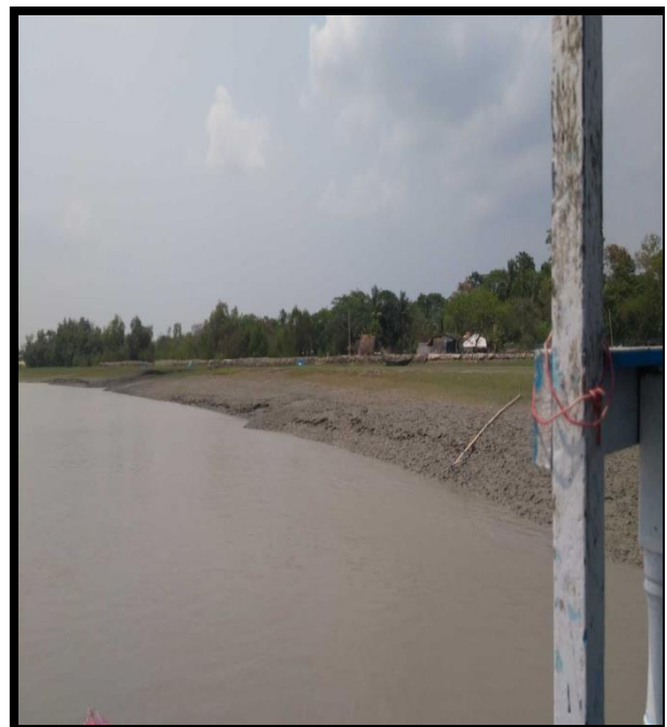
RIGHT RIVER BANK AT CHAINAGE 33
