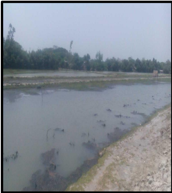
POND AT CHAINAGE 30.5, LEFT BANK
