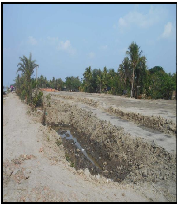
RIGHT RIVER BANK GROUND LEVEL AT CHAINAGE 49.3
