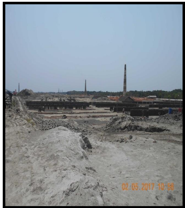
RIGHT RIVER BANK BRICKLIN AT CHAINAGE 51.5
