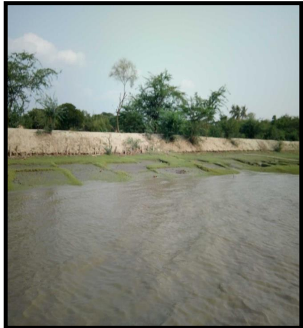
RIVER BANK AT CHAINAGE 40, LEFT BANK
