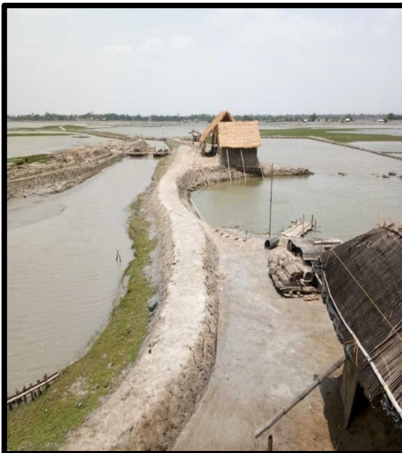
POND AT CHAINAGE 41.1, LEFT BANK
