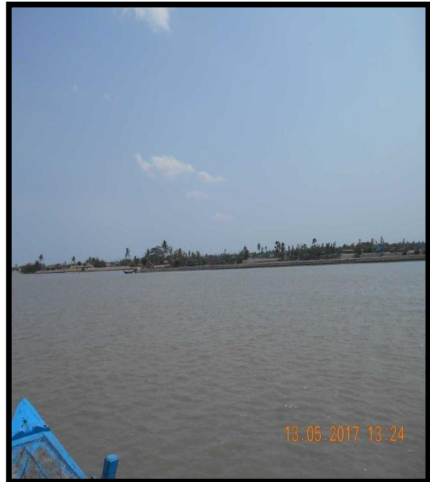
RIVER BANK AT CHAINAGE 17, RIGHT BANK
