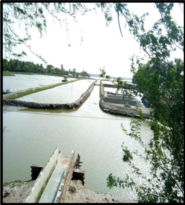
POND AT CHAINAGE 45, LEFT BANK
