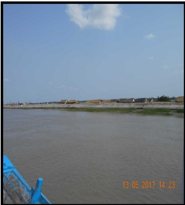
RIVER BANK AT CHAINAGE 15, RIGHT BANK
