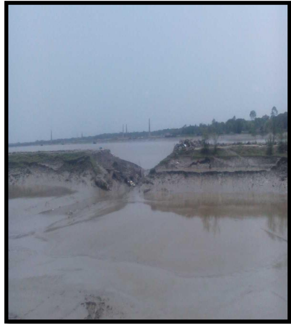
RIGHT RIVER BANK POND AT CHAINAGE
