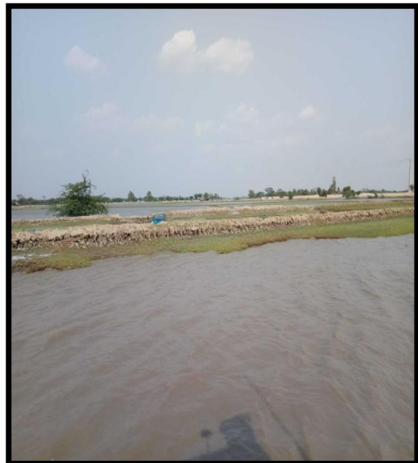
RIVER BANK AT CHAINAGE 41.5, LEFT BANK
