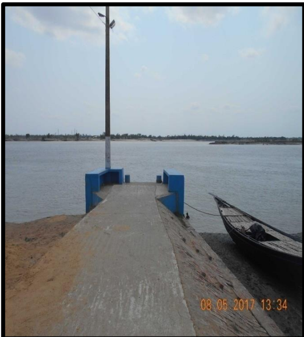
JETTY AT CHAINAGE 20.8, RIGHT BANK
