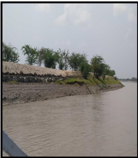
LEFT RIVER BANK AT CHAINAGE 32.5
