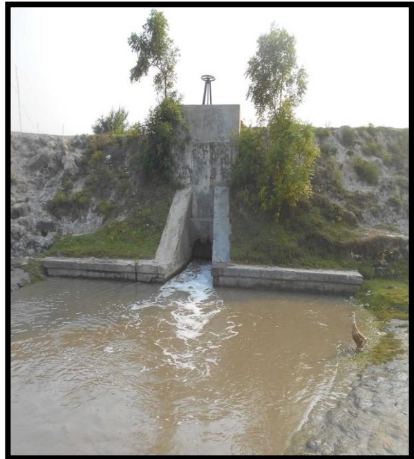
RIGHT RIVER BANK WATER LOCK AT CHAINAGE 47.1
