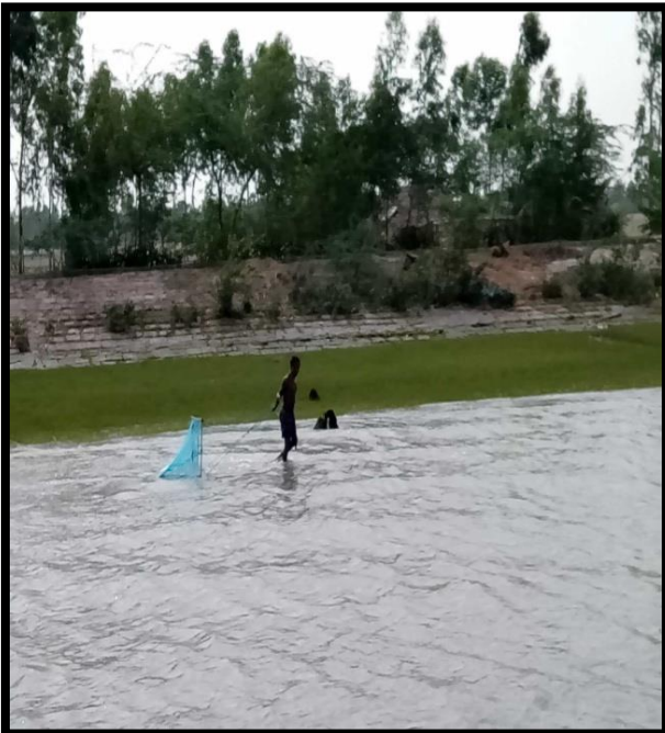
RIVER BANK AT CHAINAGE 4, LEFT BANK
