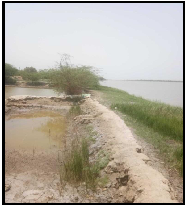
RIVER BANK AT CHAINAGE 34.3, LEFT BANK
