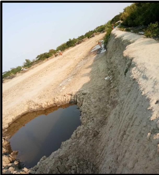
RIVER BANK AT CHAINAGE 5.2, RIGHT BANK
