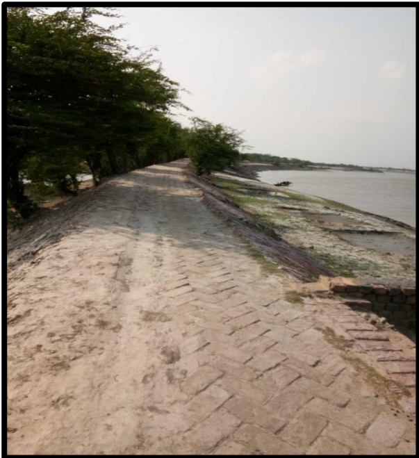
RIVER BANK AT CHAINAGE 44, LEFT BANK
