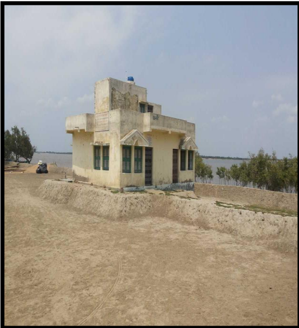
SCHOOL AT CHAINAGE 11.3, LEFT BANK
