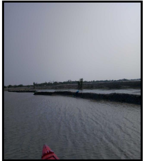
RIVER BANK AT CHAINAGE 41, RIGHT BANK
