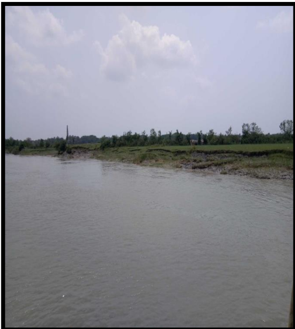
RIVER BANK AT CHAINAGE 52.5, RIGHT BANK
