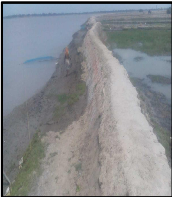
RIVER BANK AT CHAINAGE 29.5, LEFT BANK
