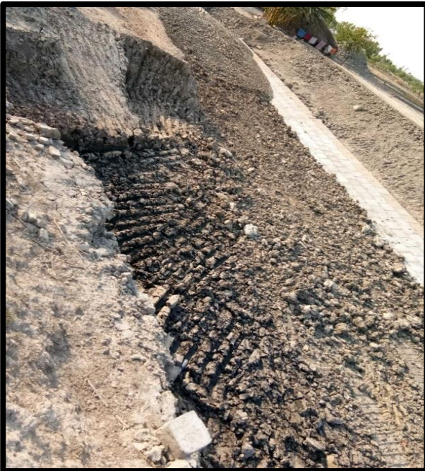
NEW CONSTRUCTION FOR RIVER BANK AT CHAINAGE 5.3, RIGHT BANK
