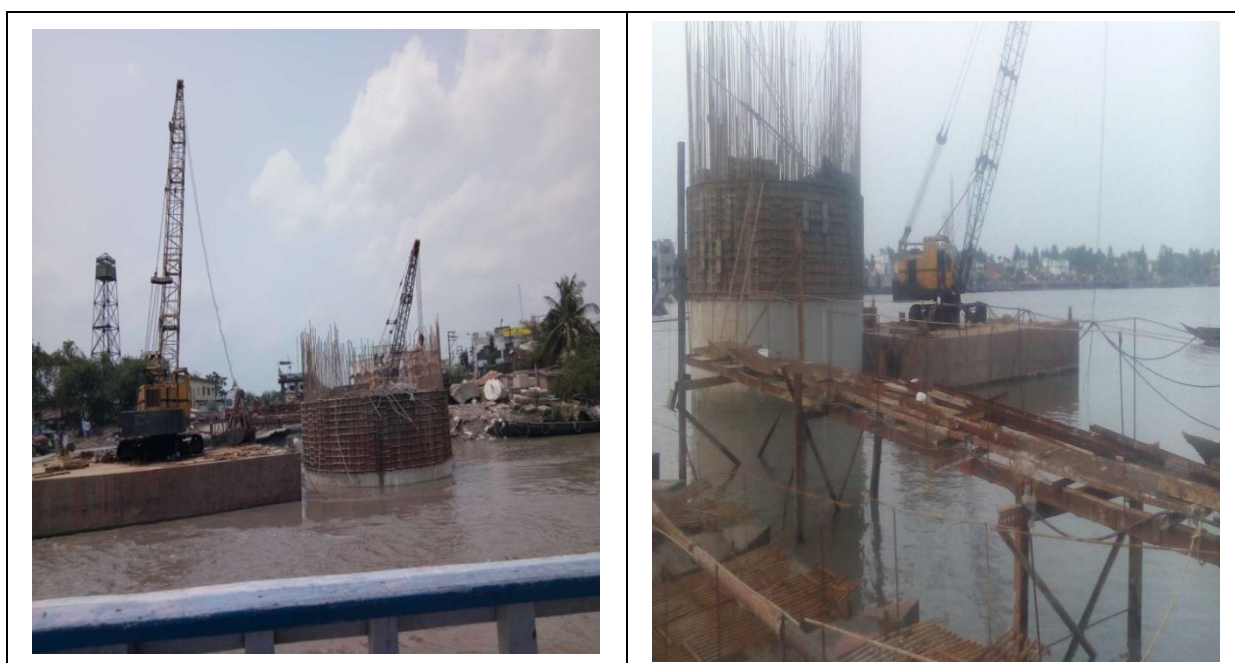
Figure 36: Photographs of Road Bridge under construction at Hasnabad
