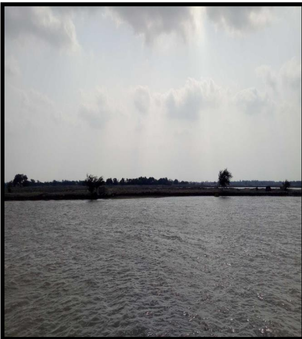
RIVER BANK AT CHAINAGE 22.5, RIGHT BANK
