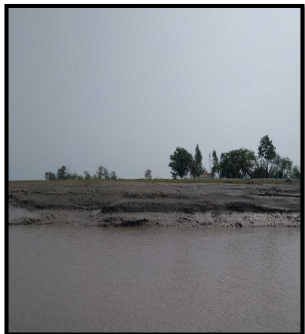
RIGHT RIVER BANK AT CHAINAGE 30
