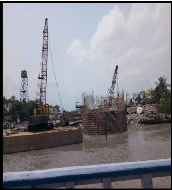
BRIDGE IN CONSTRUCTION AT CHAINAGE 50, RIGHT BANK
