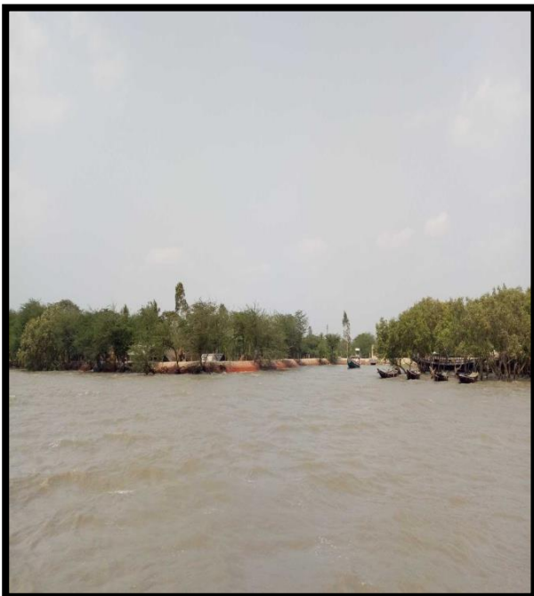
RIVER BANK AT CHAINAGE 19.5, RIGHT BANK
