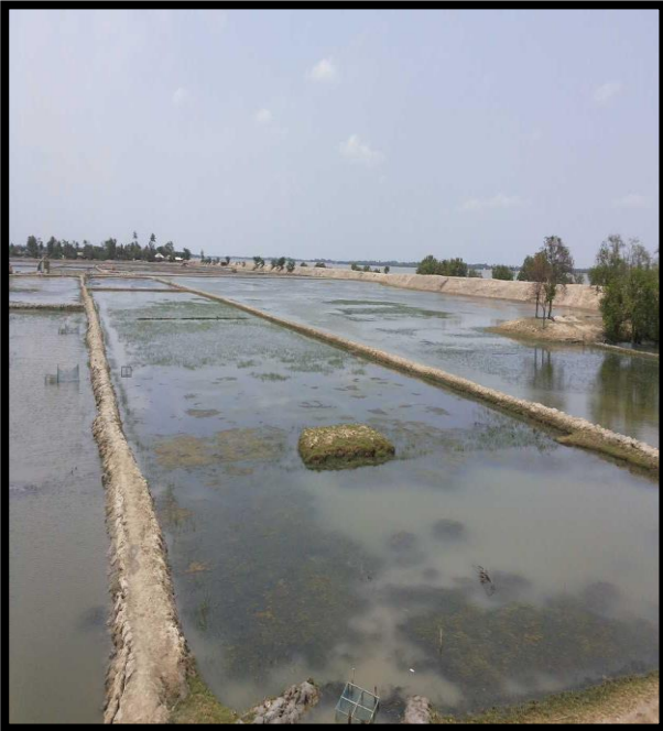
FISHING POND CHAINAGE 13, LEFT BANK
