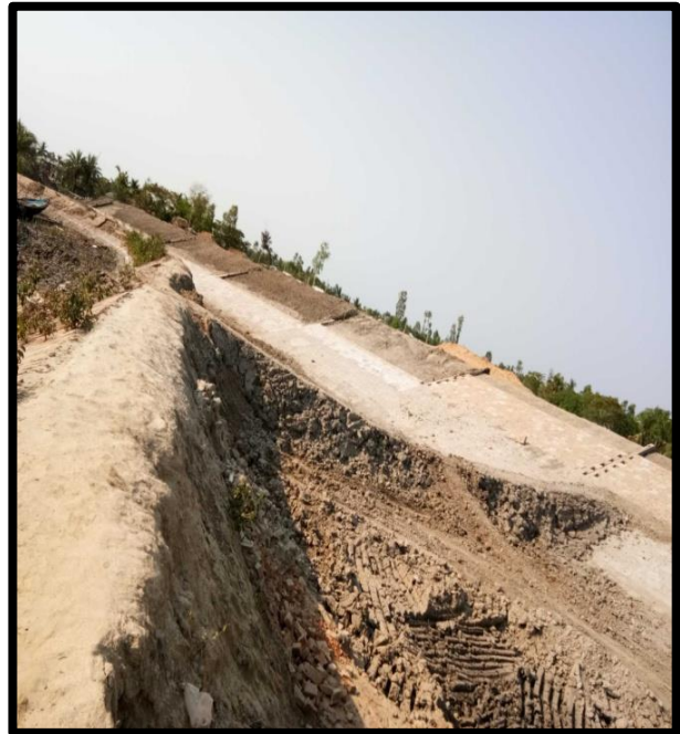
NEW CONSTRUCTION FOR RIVER BANK AT CHAINAGE 6, RIGHT BANK
