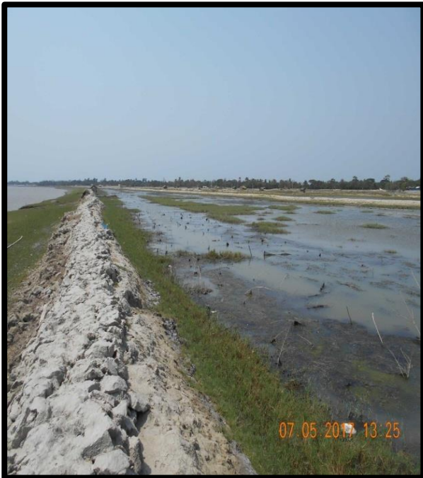
FISHING POND AT CHAINAGE 32, RIGHT BANK
