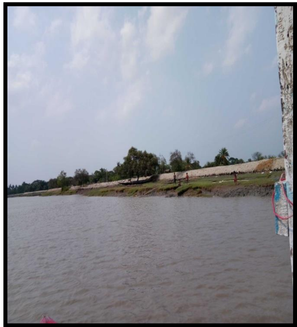
RIGHT RIVER BANK AT CHAINAGE 35.5
