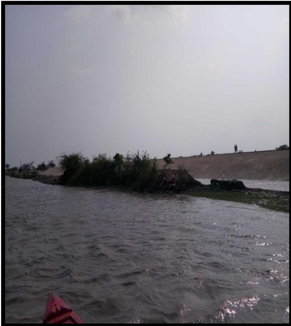
RIVER BANK AT CHAINAGE 42, RIGHT BANK
