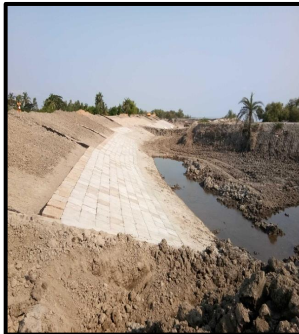
NEW CONSTRUCTION FOR RIVER BANK AT CHAINAGE 6.5, RIGHT BANK
