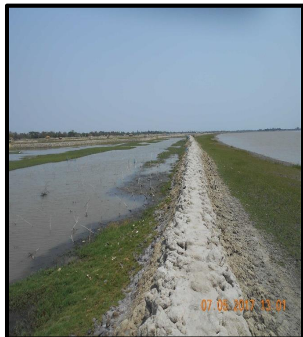
RIVER BANK AT CHAINAGE 32, RIGHT BANK
