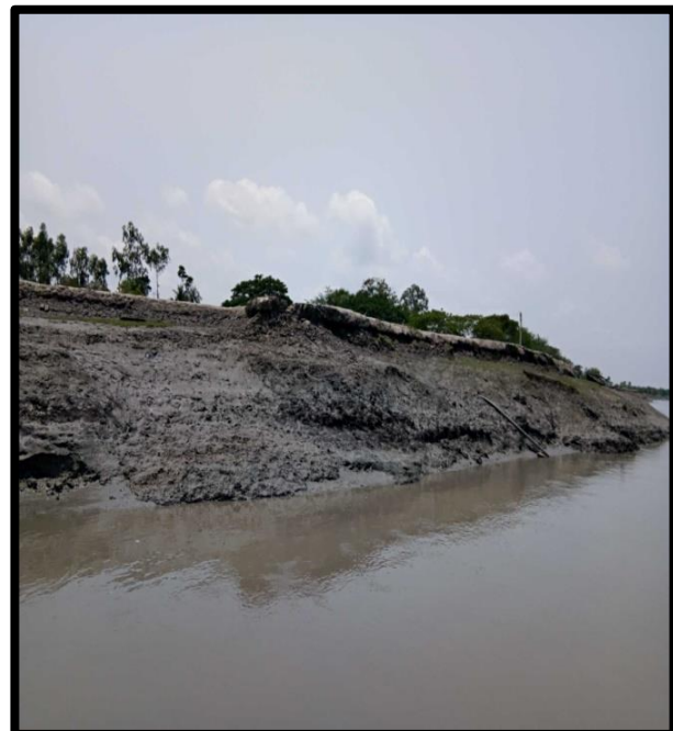
RIGHT RIVER BANK AT CHAINAGE 25.5
