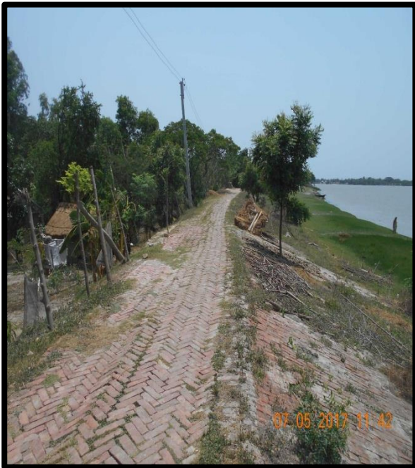
RIVER BANK PROTECTION AT CHAINAGE 34.5, RIGHT BANK
