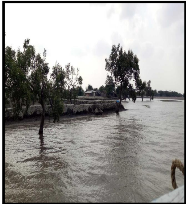
RIVER BANK AT CHAINAGE 21.5, RIGHT BANK
