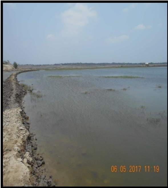
FISHING POND AT CHAINAGE 42.1, RIGHT BANK
