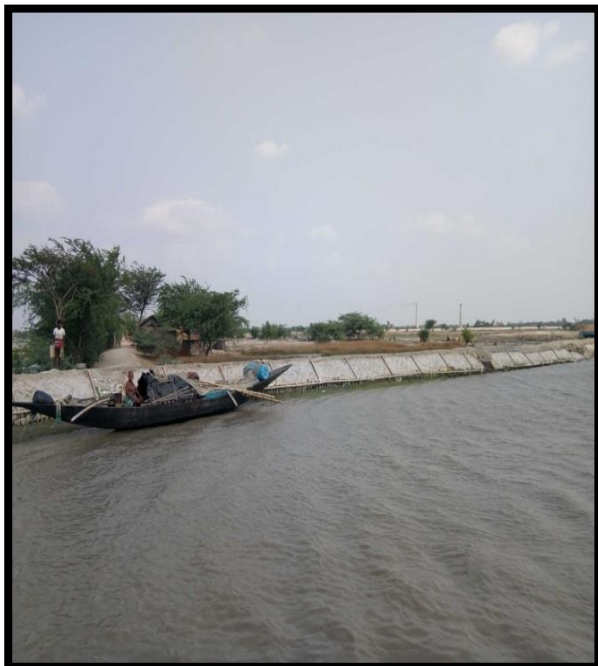
RIVER BANK AT CHAINAGE 41.5, LEFT BANK
