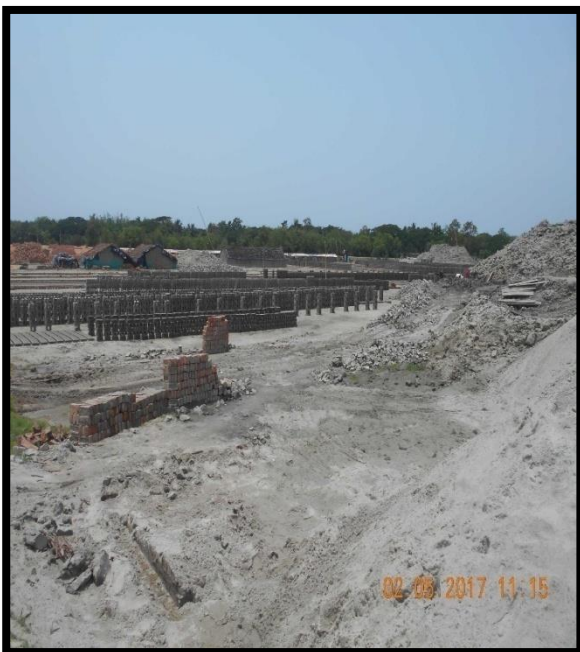
RIGHT RIVER BANK BRICKLIN AT CHAINAGE 51.7
