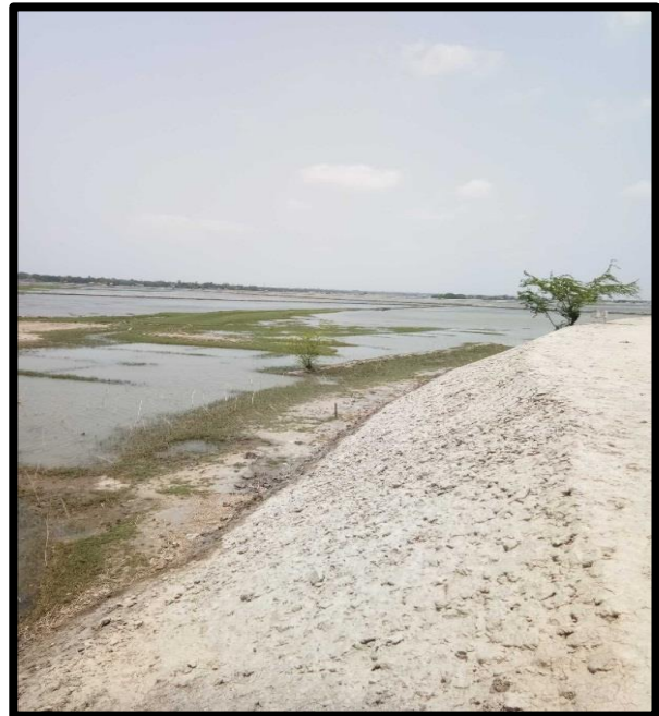
POND AT CHAINAGE 41, LEFT BANK
