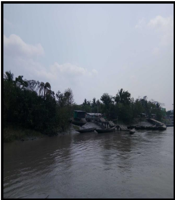
HASNABAD FERRY GHAT NO.2 AT CHAINAGE 50, LEFT BANK
