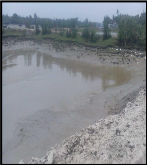
RIGHT RIVER BANK POND AT CHAINAGE
