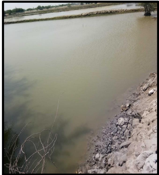
POND AT CHAINAGE 43.8, LEFT BANK
