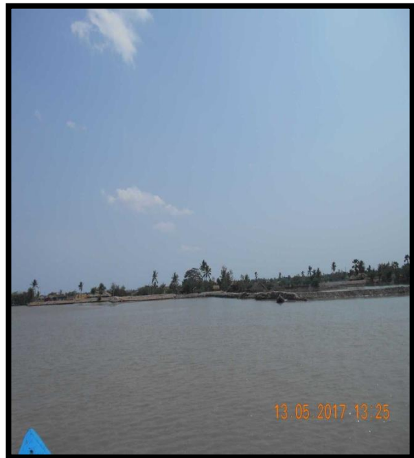
RIVER BANK AT CHAINAGE 17, LEFT BANK
