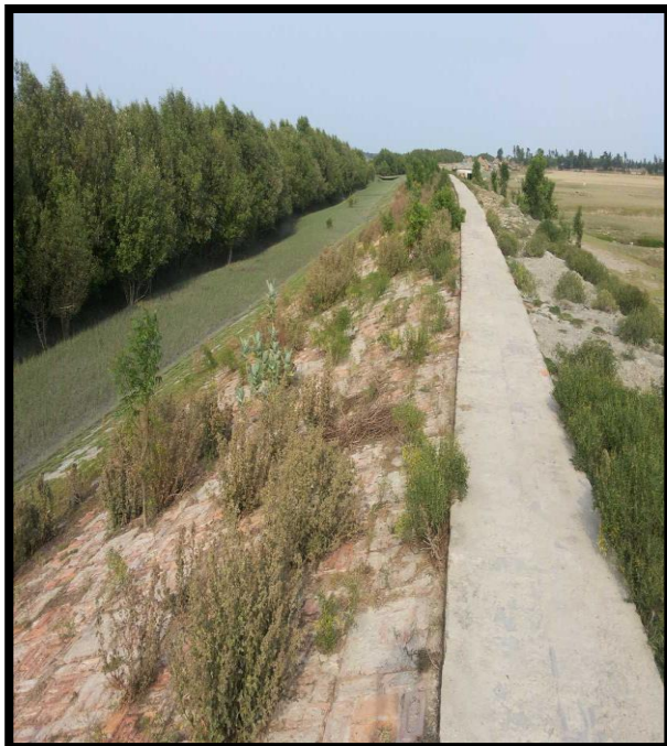
RIVER BANK PROTECTION AT CHAINAGE 6.5, LEFT BANK
