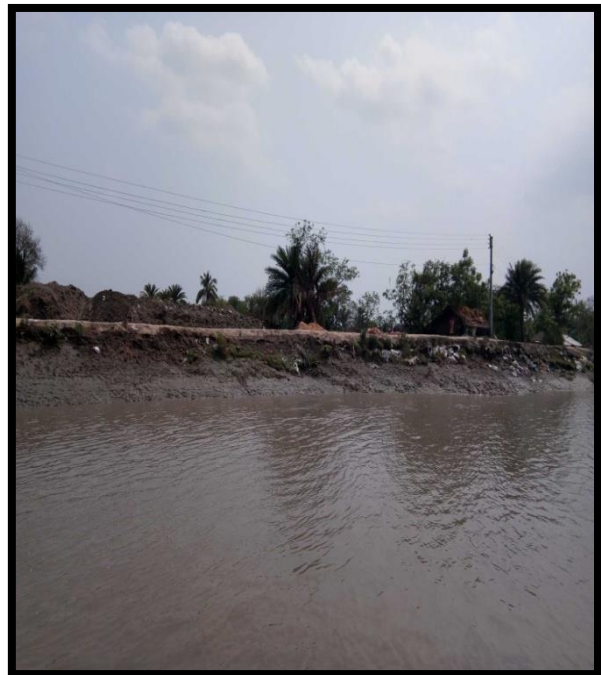
RIVER BANK AT CHAINAGE 49, LEFT BANK
