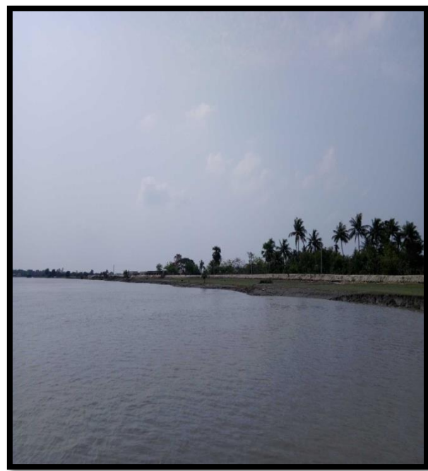
LEFT RIVER BANK AT CHAINAGE 36
