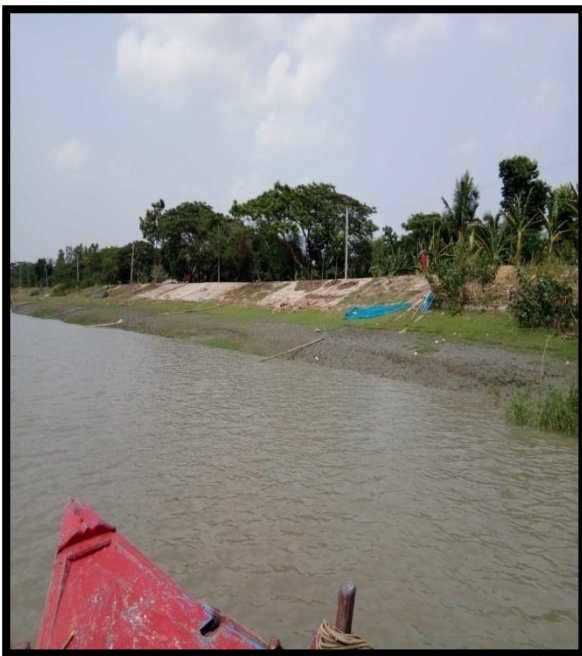
RIGHT RIVER BANK AT CHAINAGE 34
