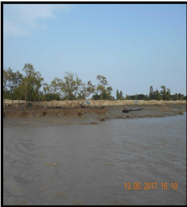
RIVER BANK AT CHAINAGE 12.5, RIGHT BANK
