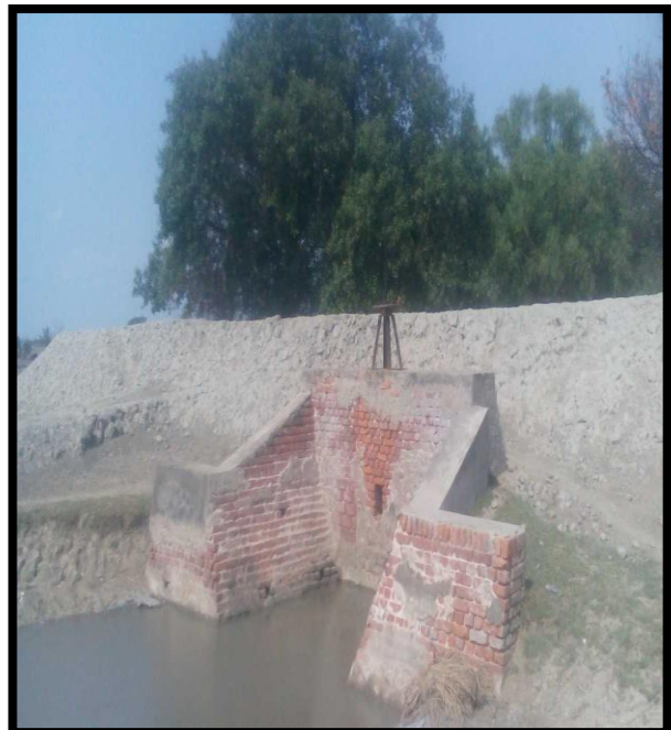
WATER LOCK AT CHAINAGE 10.2, LEFT BANK
