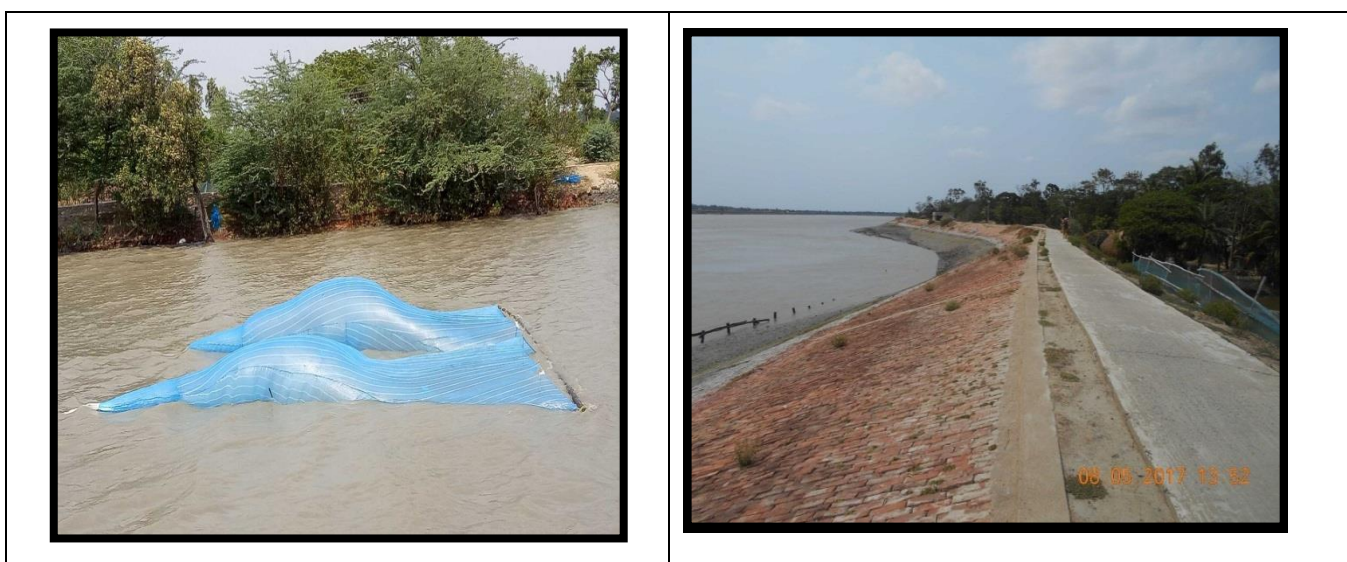
Figure 11: Photograph along Sub-Stretch 3
