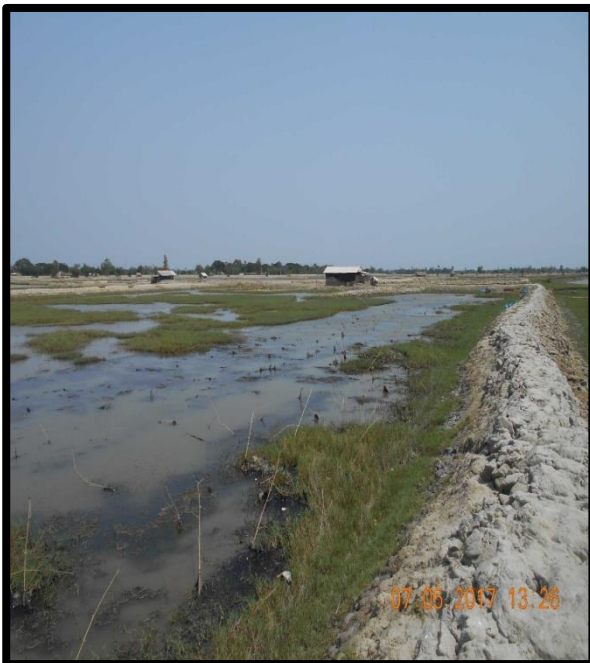
FISHING POND AT CHAINAGE 33, RIGHT BANK
