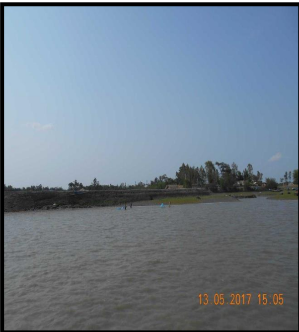
RIVER BANK AT CHAINAGE 13.5, LEFT BANK
