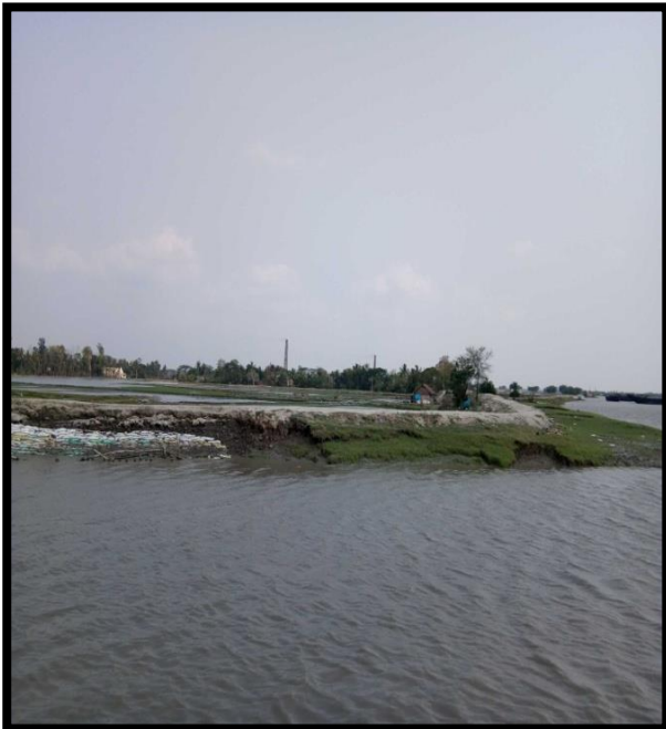
RIVER BANK AT CHAINAGE 44.5, LEFT BANK
