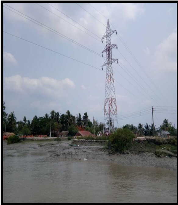
HIGH TENSION LINE AT CHAINAGE 49, RIGHT BANK
