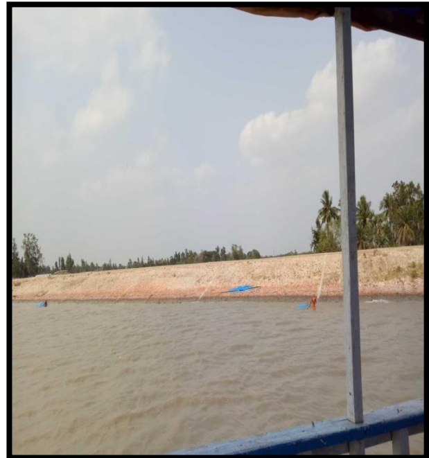
RIVER BANK PROTECTION AT CHAINAGE 22, LEFT BANK
