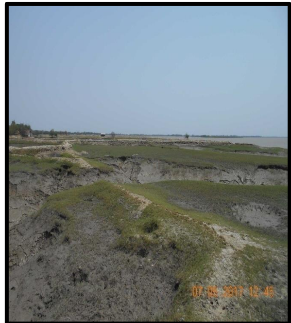
RIVER BANK AT CHAINAGE 33, RIGHT BANK
