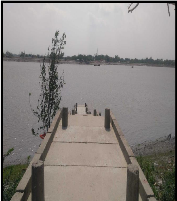
BAILANY JETTY AT CHAINAGE 38.4, RIGHT BANK
