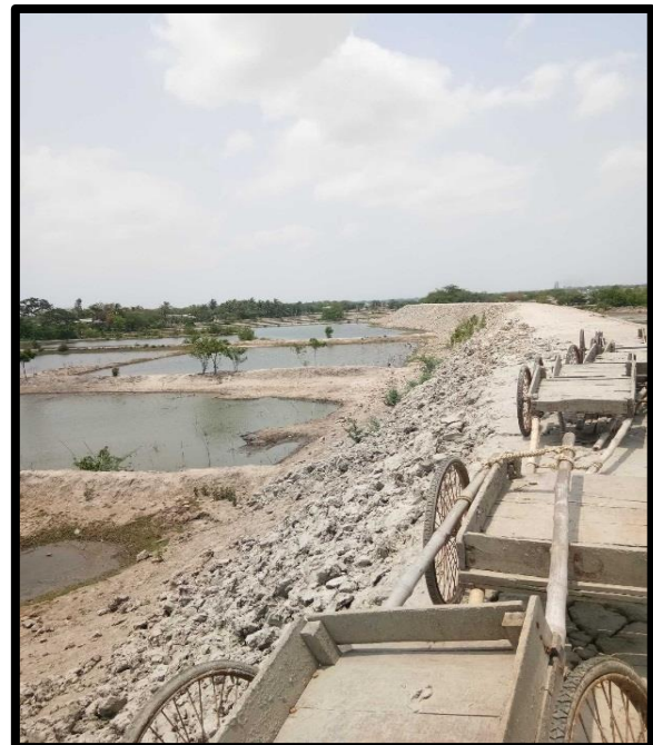
POND AT CHAINAGE 42, LEFT BANK
