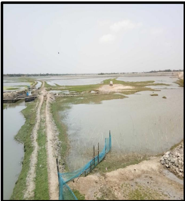
POND AT CHAINAGE 40.8, LEFT BANK
