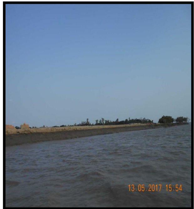
RIVER BANK AT CHAINAGE 12.5, LEFT BANK
