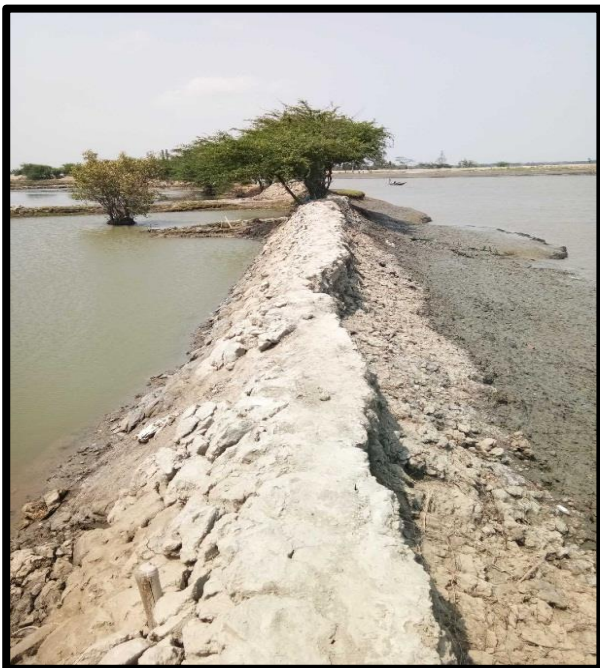
RIVER BANK AT CHAINAGE 43, LEFT BANK
