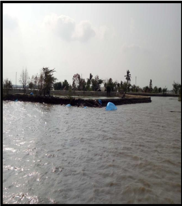
RIVER BANK AT CHAINAGE 23.5, LEFT BANK
