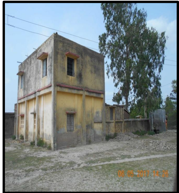
SCHOOL AT CHAINAGE 22.8, RIGHT BANK
