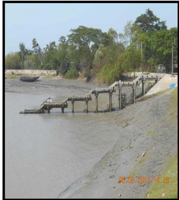
CHAK KHAPUKUR JETTY AT CHAINAGE 46, RIGHT BANK
