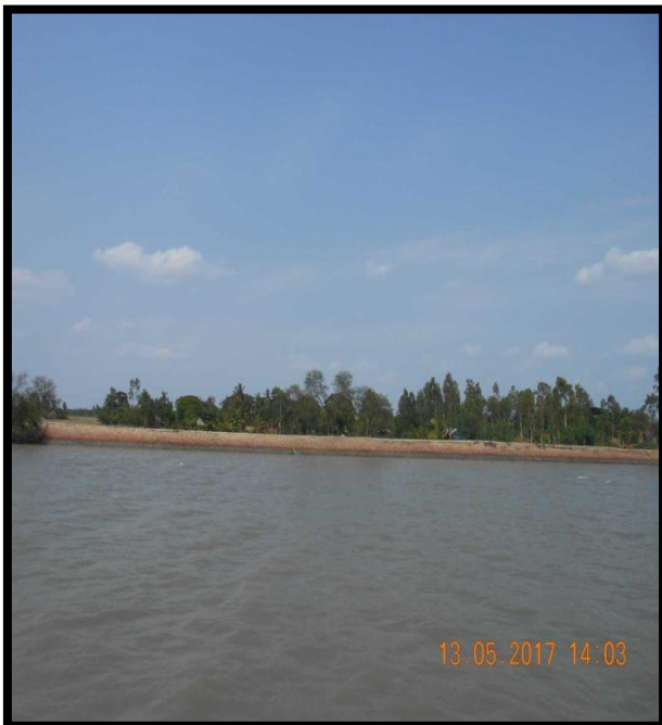
RIVER BANK AT CHAINAGE 15.5, RIGHT BANK
