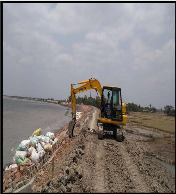
RIVER BANK CONSTRUCTION AT CHAINAGE 40.8, RIGHT BANK
