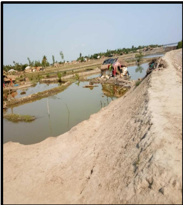
RIVER BANK AT CHAINAGE 7.5, RIGHT BANK
