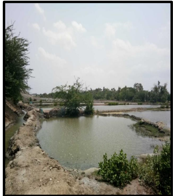
POND AT CHAINAGE 42.9, LEFT BANK
