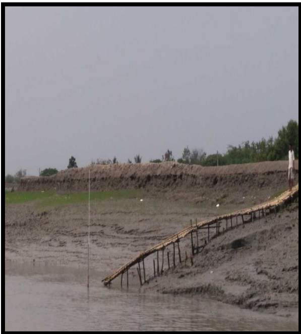
WOODEN JETTY AT CHAINAGE 30.5, LEFT BANK
