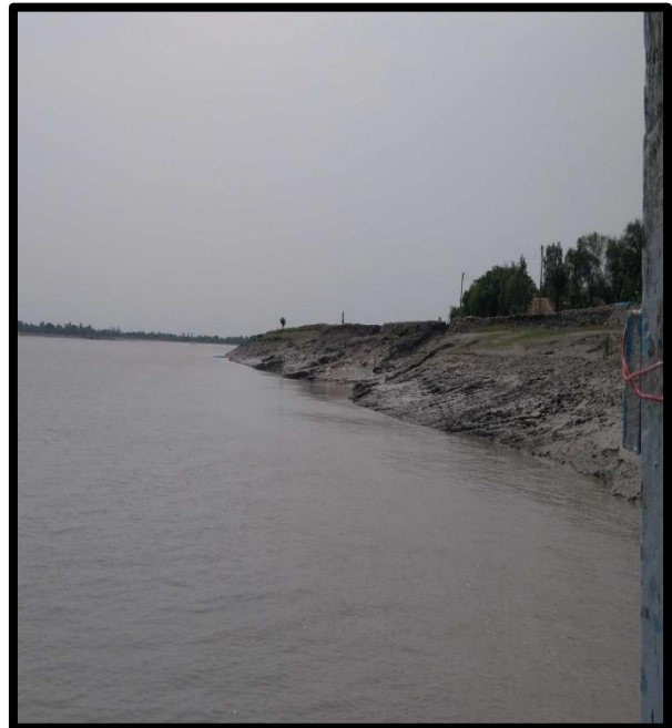
LEFT RIVER BANK AT CHAINAGE 29
