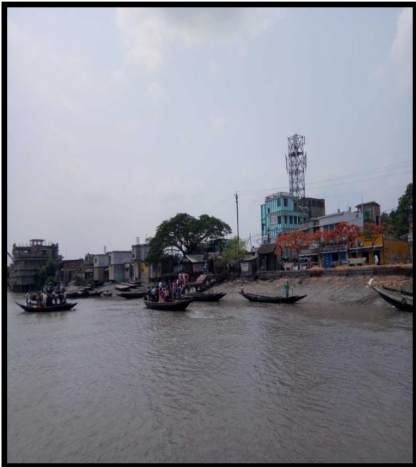
HASNABAD FERRY GHAT AT CHAINAGE 50, LEFT BANK
