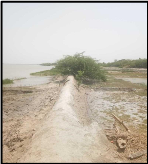
RIVER BANK AT CHAINAGE 34, LEFT BANK
