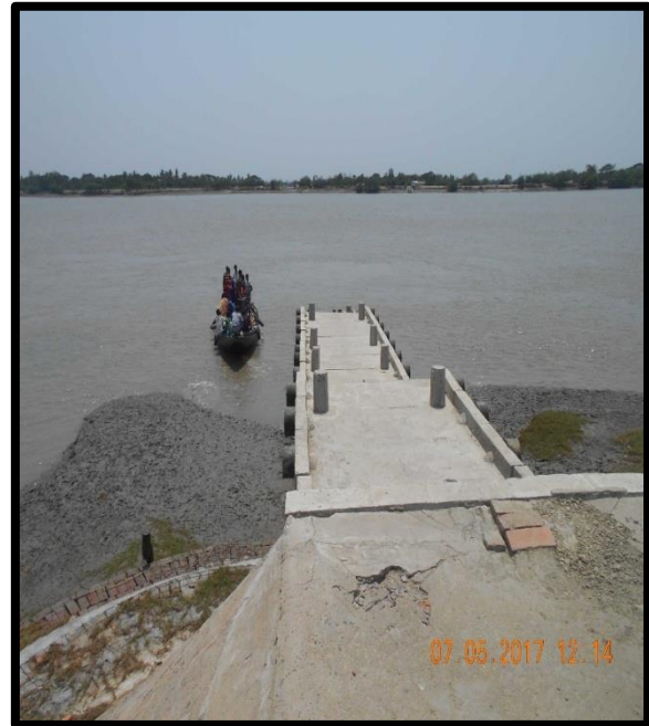
BINDADA JETTY AT CHAINAGE 33.5, RIGHT BANK
