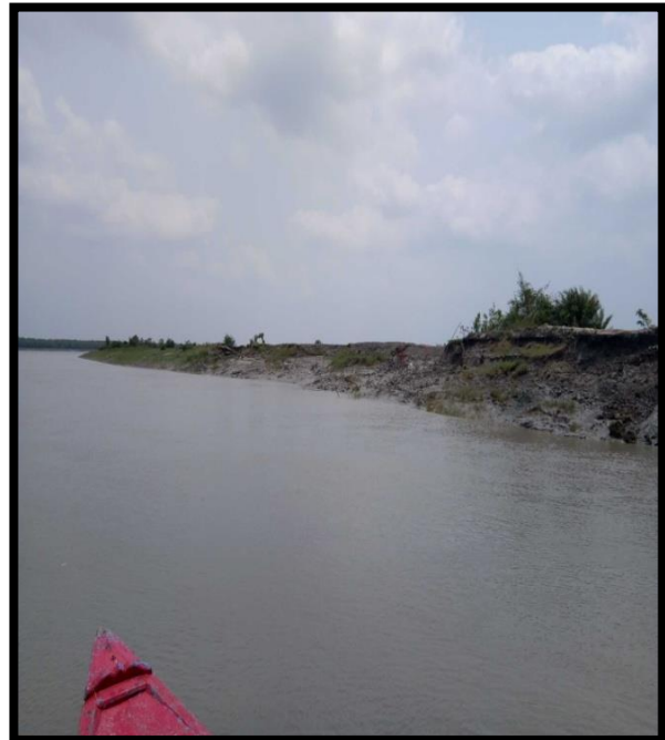
RIVER BANK AT CHAINAGE 52.5, RIGHT BANK
