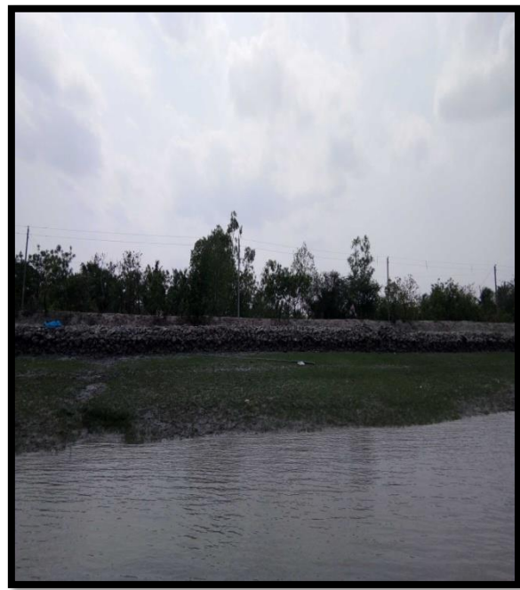
LEFT RIVER BANK AT CHAINAGE 34.5
