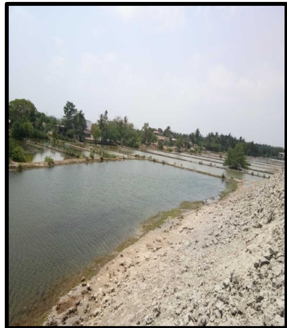
POND AT CHAINAGE 42.3, LEFT BANK
