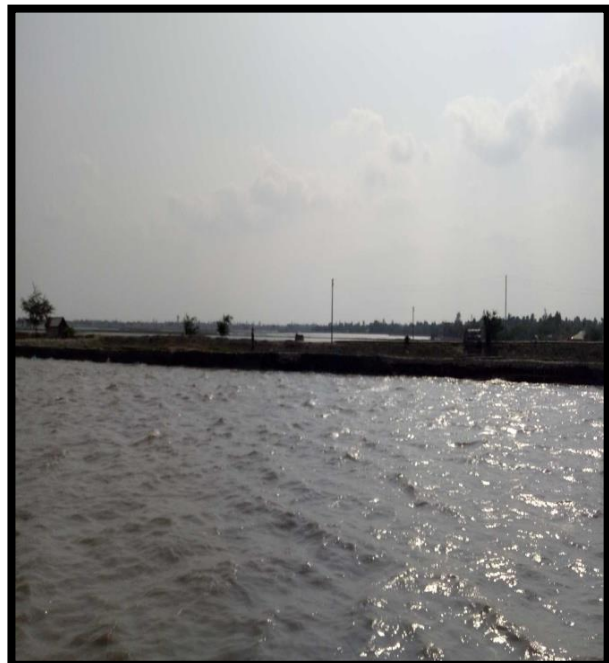
RIVER BANK AT CHAINAGE 23.5, LEFT BANK
