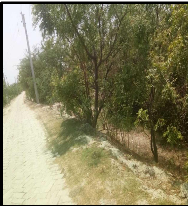
ROAD AT CHAINAGE 34.5, LEFT BANK
