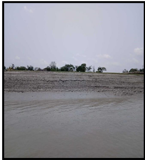
RIGHT RIVER BANK AT CHAINAGE 26
