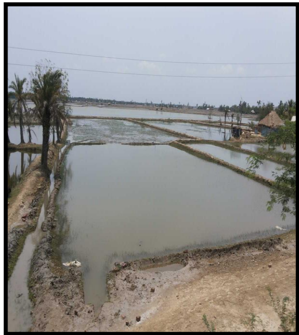
FISHING POND CHAINAGE 13.5, LEFT BANK
