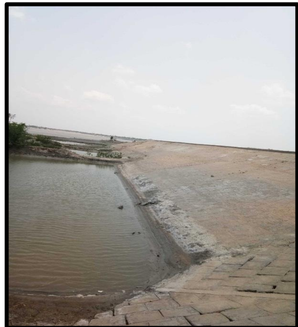
POND AT CHAINAGE 42.5, LEFT BANK
