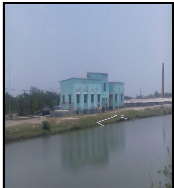
RIGHT RIVER BANK WATER TREATMENT PLANT CHAINAGE 52
