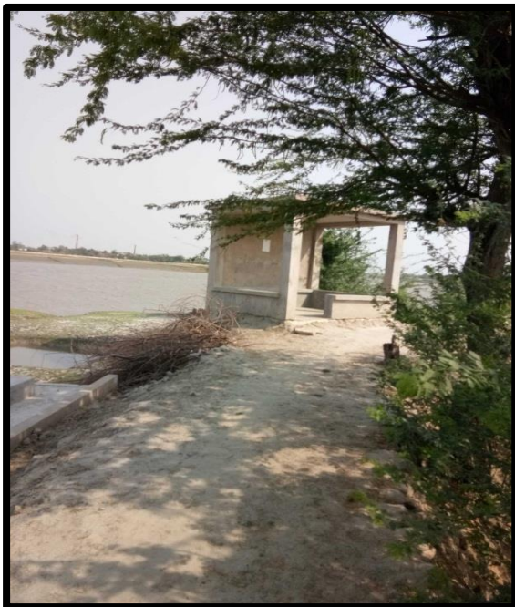
STRUCTURE AT CHAINAGE 45, LEFT BANK
