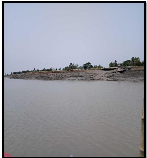
LEFT RIVER BANK AT CHAINAGE 26.5
