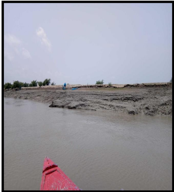
RIVER BANK AT CHAINAGE 25.5, LEFT BANK
