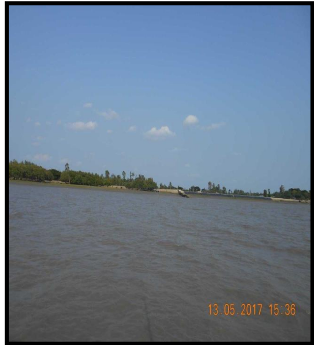
RIVER BANK AT CHAINAGE 12.5, RIGHT BANK
