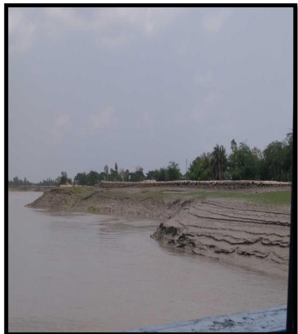
RIGHT RIVER BANK AT CHAINAGE 31
