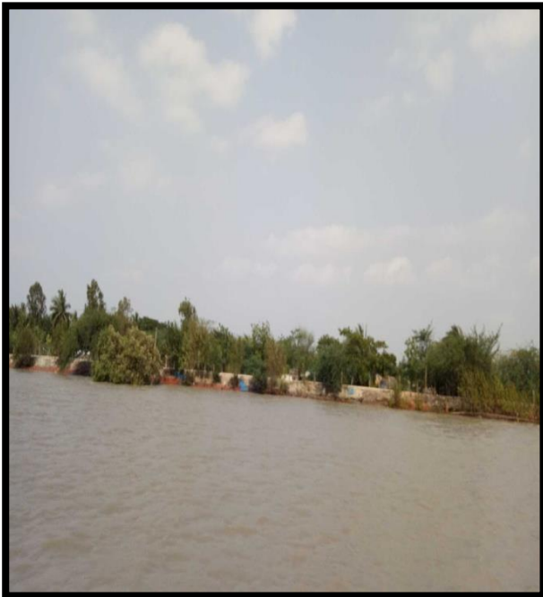
RIVER BANK AT CHAINAGE 19.5, RIGHT BANK
