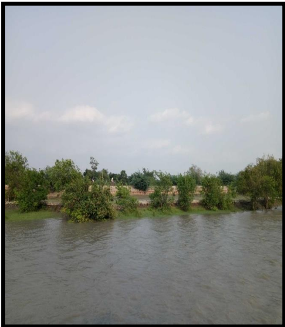
RIVER BANK AT CHAINAGE 38.5, LEFT BANK
