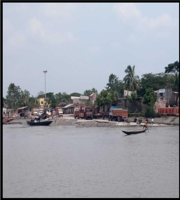
HASNABAD VESSEL JETTY AT CHAINAGE 51, LEFT BANK
