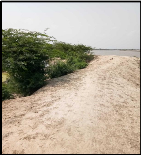
POND AT CHAINAGE 42.4, LEFT BANK
