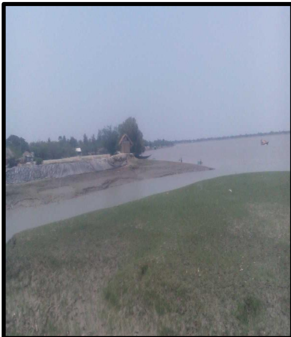
CREEK AT CHAINAGE 30.7, LEFT BANK
