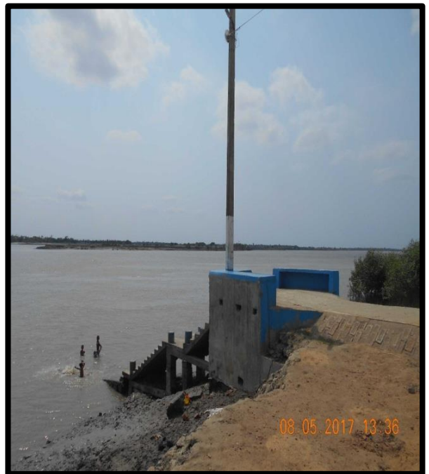
JETTY AT CHAINAGE 20.8, RIGHT BANK
