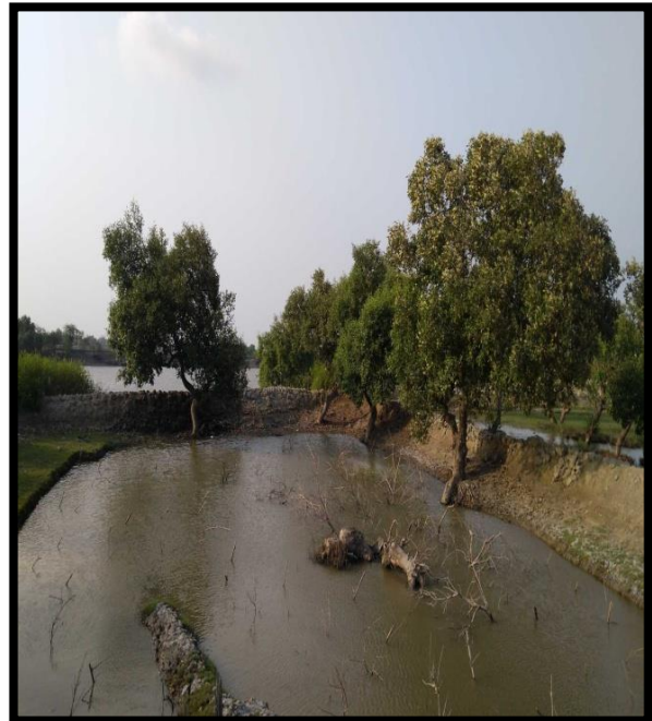
POND AT CHAINAGE 36.5, RIGHT BANK
