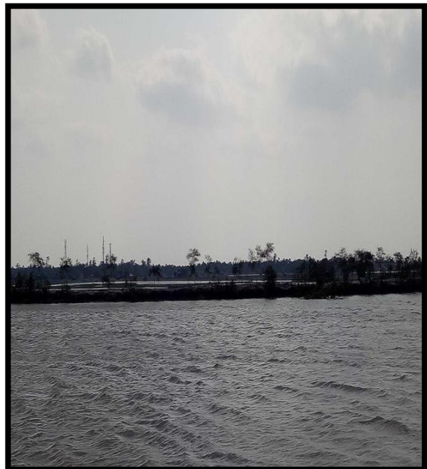
RIVER BANK AT CHAINAGE 21.5, LEFT BANK
