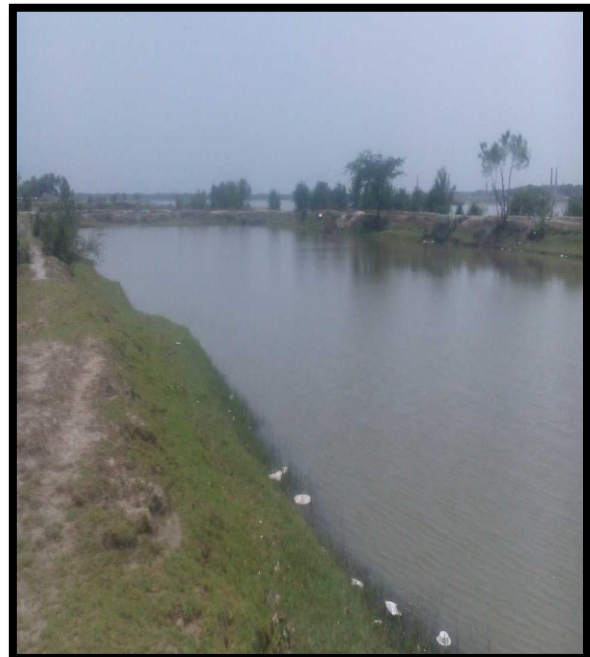
RIGHT RIVER BANK POND AT CHAINAGE 52
