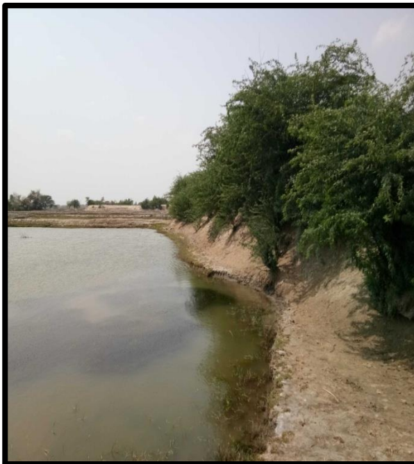
RIVER BANK AT CHAINAGE 44.2, LEFT BANK
