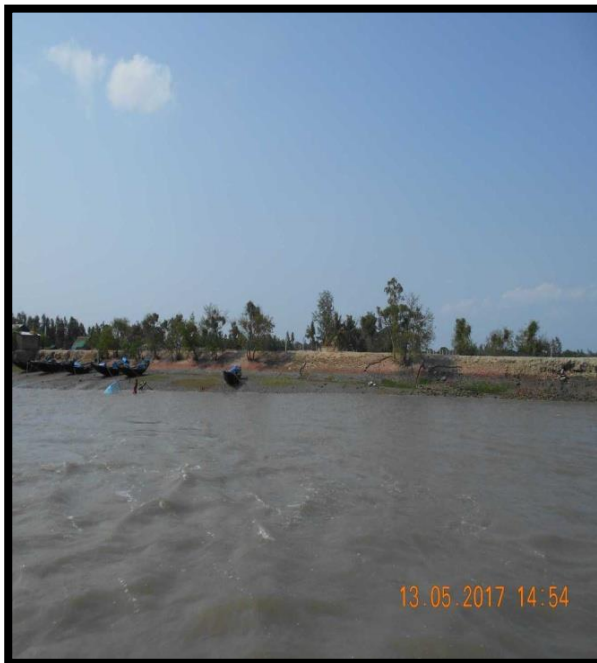
RIVER BANK AT CHAINAGE 14, RIGHT BANK
