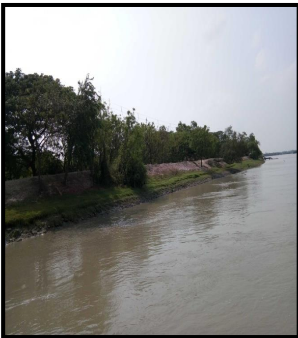
LEFT RIVER BANK AT CHAINAGE 35.5
