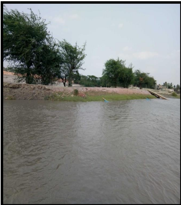
RIVER BANK AT CHAINAGE 44, LEFT BANK
