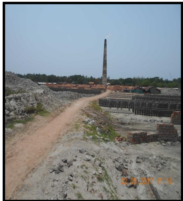
RIGHT RIVER BANK BRICKLIN AT CHAINAGE 51.8
