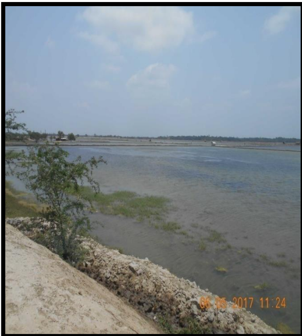
FISHING POND AT CHAINAGE 42.3, RIGHT BANK
