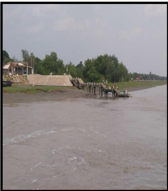
JETTY AT CHAINAGE 33.5, RIGHT BANK
