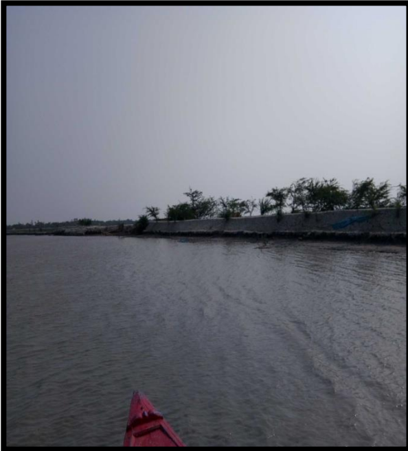
RIVER BANK AT CHAINAGE 41.5, RIGHT BANK
