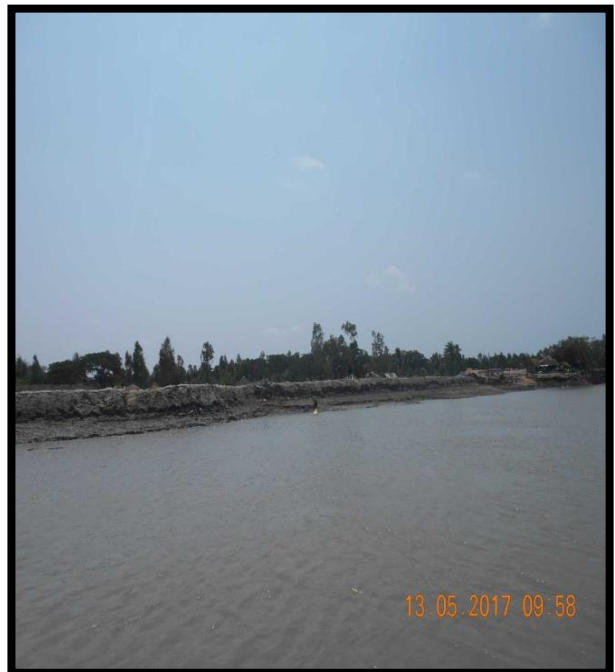
RIVER BANK AT CHAINAGE 5, LEFT BANK
