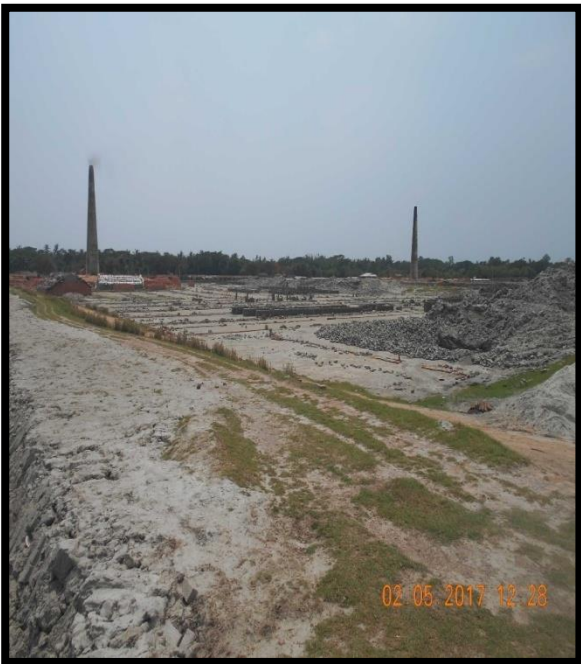
RIGHT RIVER BANK BRICKLIN AT CHAINAGE 51.8
