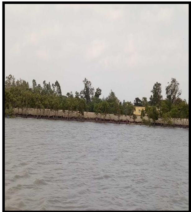
RIVER BANK AT CHAINAGE 22.5, RIGHT BANK
