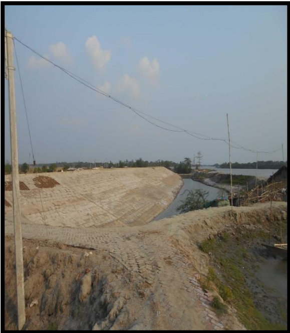
RIGHT RIVER BANK PROTECTION AT CHAINAGE 47
