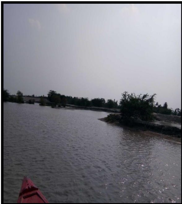
RIVER BANK AT CHAINAGE 42.5, RIGHT BANK
