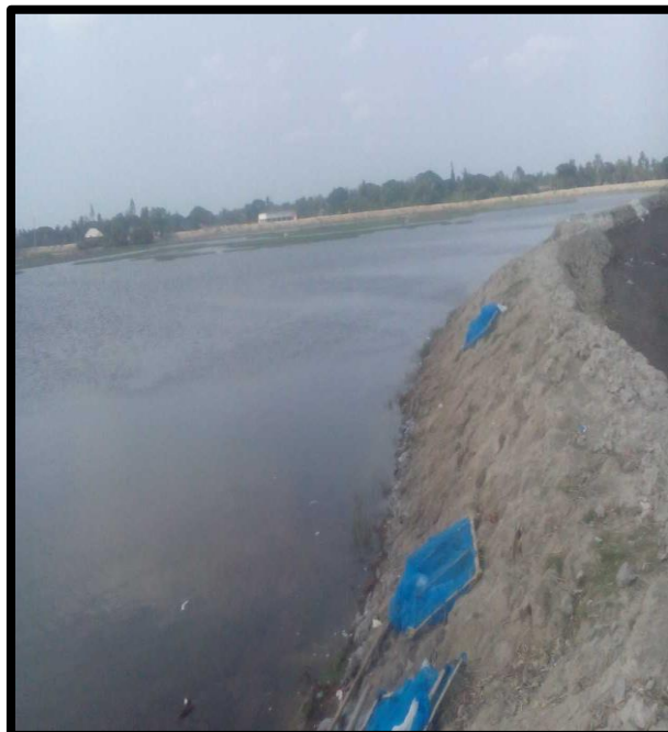
RIVER BANK AT CHAINAGE 25, RIGHT BANK
