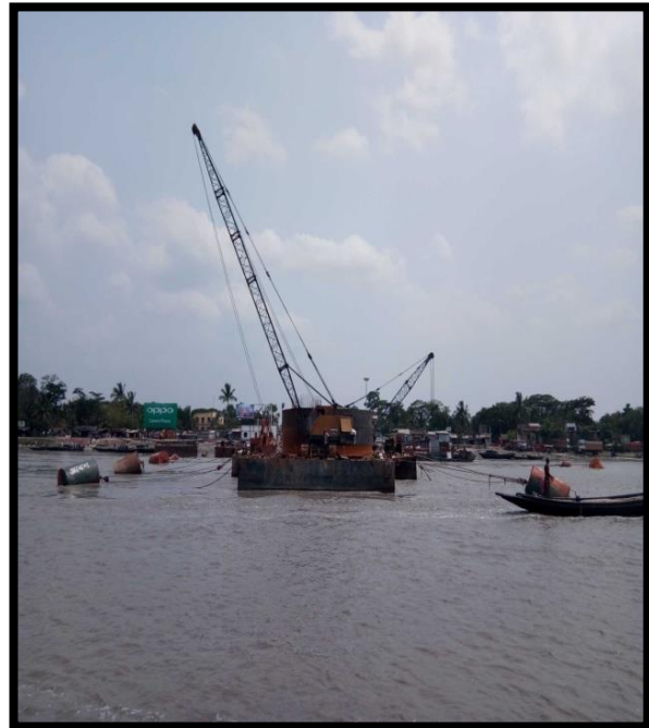
BRIDGE IN CONSTRUCTION AT CHAINAGE 50, RIGHT BANK
