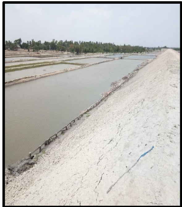
POND AT CHAINAGE 41.7, LEFT BANK
