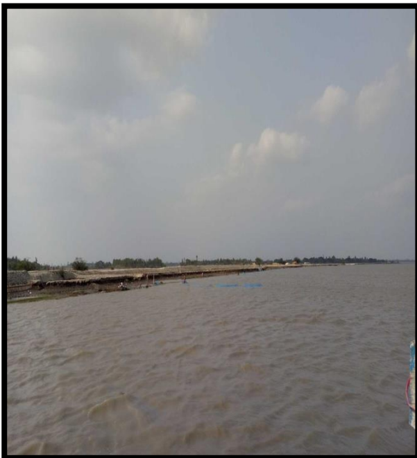
RIVER BANK AT CHAINAGE 24.5, RIGHT BANK
