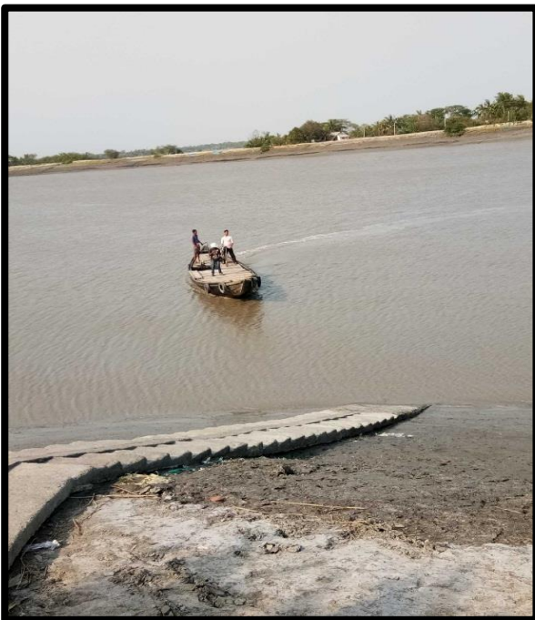
JETTY GHAT AT CHAINAGE 46, LEFT BANK
