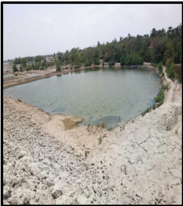
POND AT CHAINAGE 41.9, LEFT BANK
