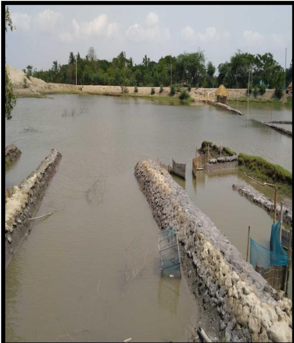
POND AT CHAINAGE 40, RIGHT BANK
