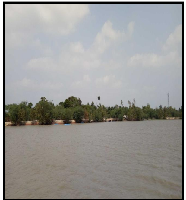
RIVER BANK AT CHAINAGE 20.5, RIGHT BANK
