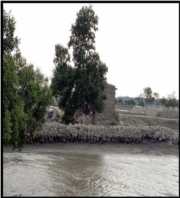
RIVER BANK AT CHAINAGE 21.5, RIGHT BANK
