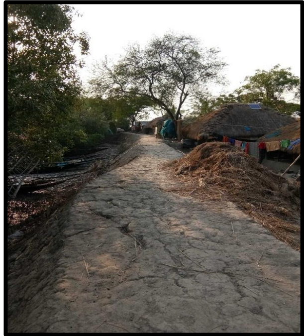
TREE COVER AREA AT CHAINAGE 5.1, RIGHT BANK
