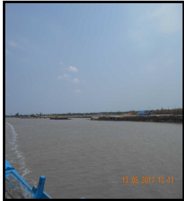
RIVER BANK AT CHAINAGE 17, LEFT BANK
