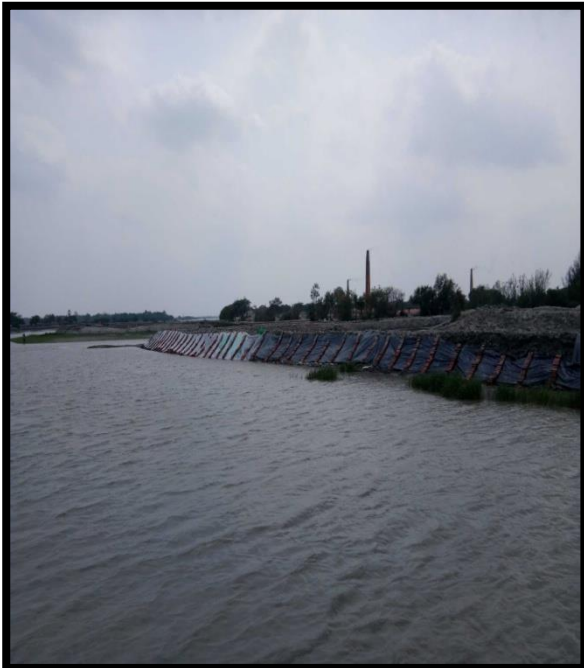
RIVER BANK AT CHAINAGE 48, LEFT BANK
