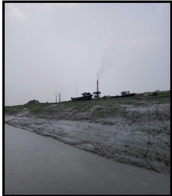
RIVER BANK AT CHAINAGE 52, LEFT BANK
