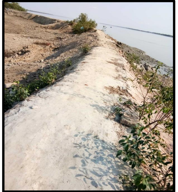
RIVER BANK AT CHAINAGE 6, RIGHT BANK
