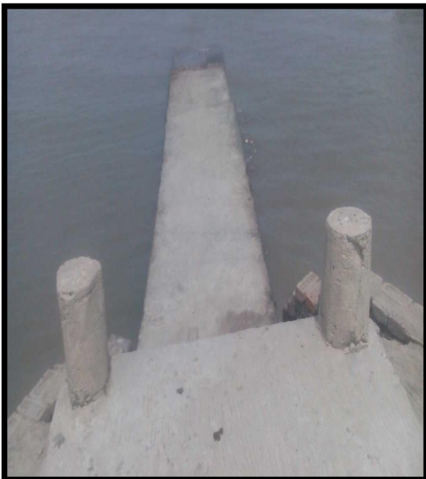
JETTY GHAT AT CHAINAGE 11.5, LEFT BANK
