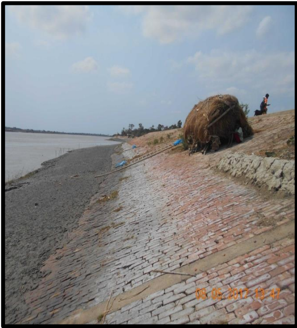
RIVER BANK PROTECTION AT CHAINAGE 22.2, RIGHT BANK
