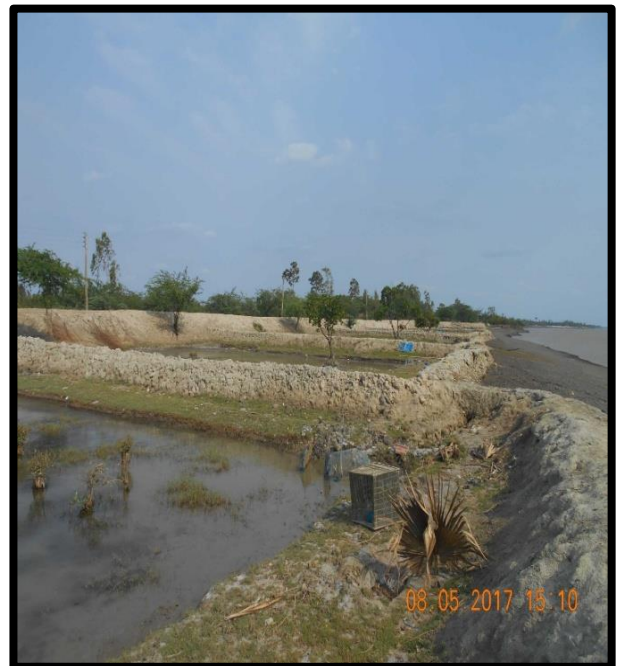
POND AT CHAINAGE 23.4, RIGHT BANK
