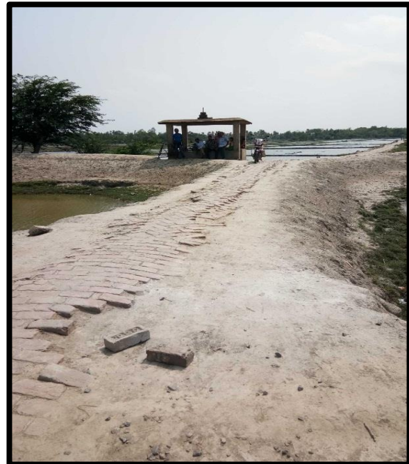
JETTY HOUSE AT CHAINAGE 43.9, LEFT BANK
