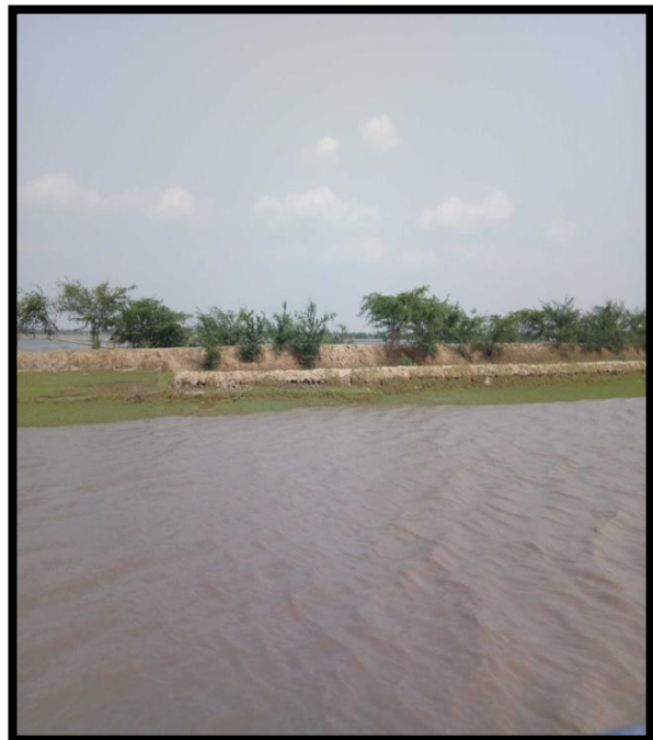
RIVER BANK AT CHAINAGE 42, LEFT BANK
