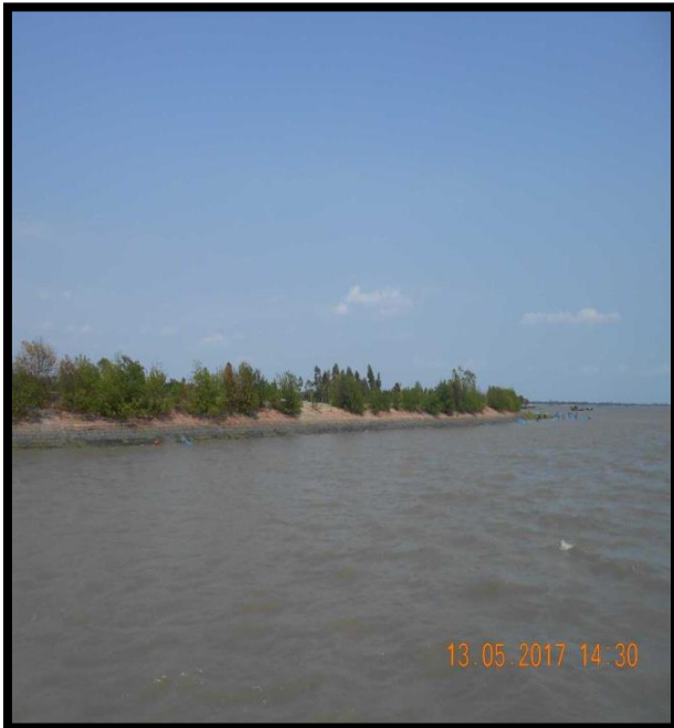
RIVER BANK AT CHAINAGE 15, RIGHT BANK
