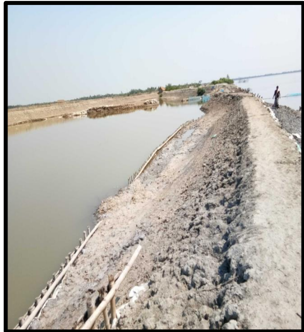
RIVER BANK AT CHAINAGE 9.5, RIGHT BANK
