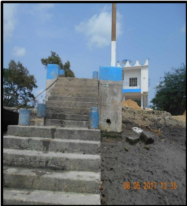
JETTY AT CHAINAGE 20.8, RIGHT BANK
