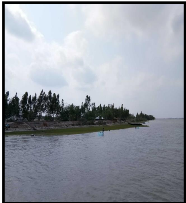
RIVER BANK CHAINAGE 4, LEFT BANK
