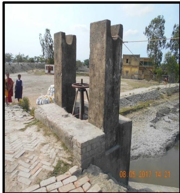
WATER LOCK AT CHAINAGE 22.7, RIGHT BANK
