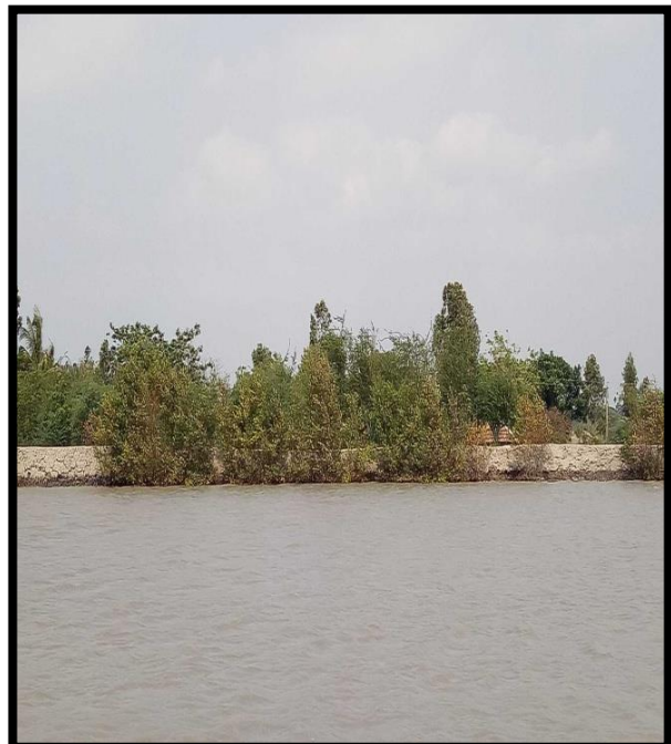
RIVER BANK AT CHAINAGE 21, LEFT BANK
