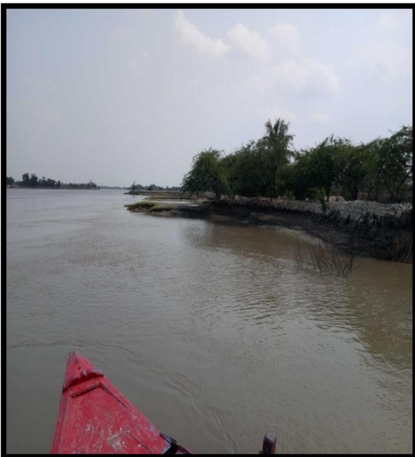
RIVER BANK AT CHAINAGE 46.5, RIGHT BANK
