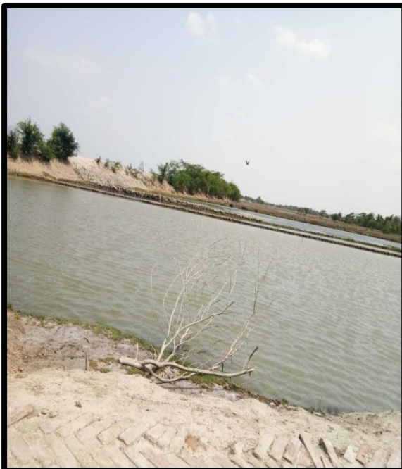
RIVER BANK AT CHAINAGE 44.3, LEFT BANK
