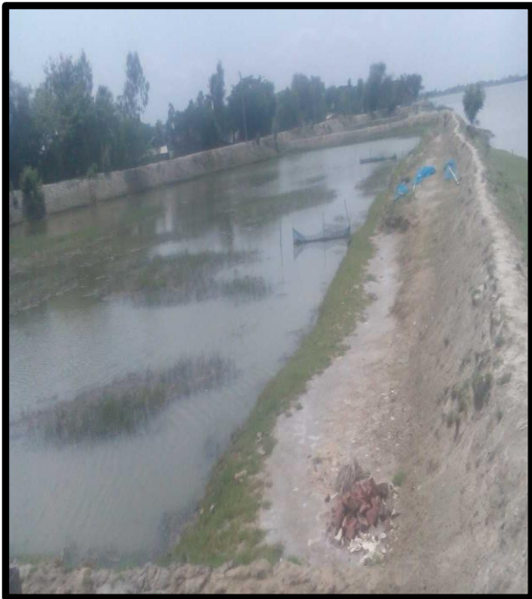
POND AT CHAINAGE 26.8, RIGHT BANK
