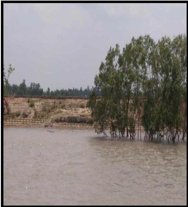
RIVER BANK AT CHAINAGE 1, LEFT BANK
