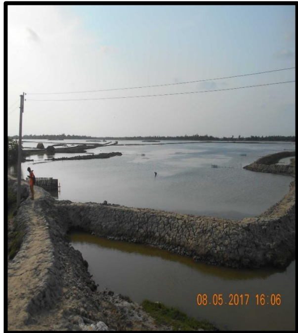
FISHING POND AT CHAINAGE 24, LEFT BANK
