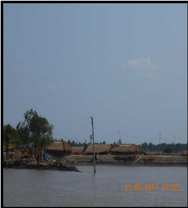
RIVER BANK AT CHAINAGE 15.5, LEFT BANK
