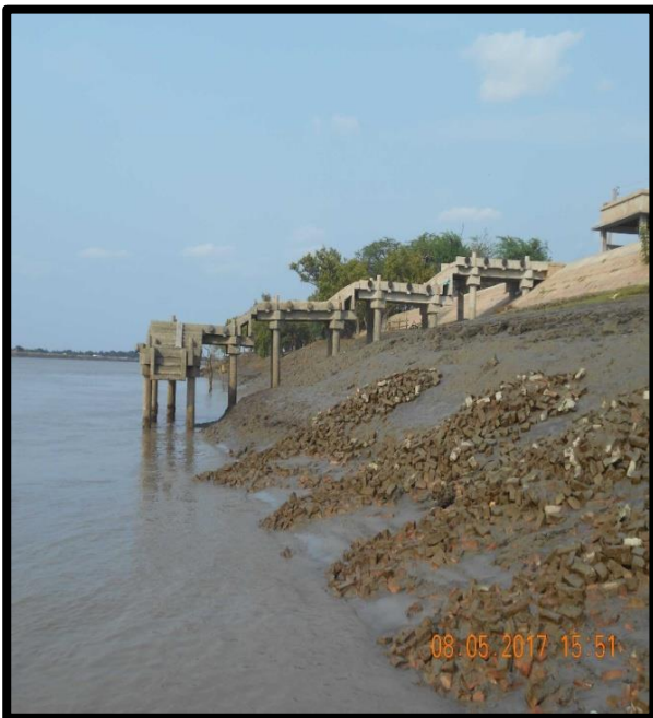
MALAPADA FERRY GHAT AT CHAINAGE 24, RIGHT BANK
