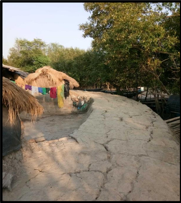
STRUCTURE AT CHAINAGE 5.1, RIGHT BANK
