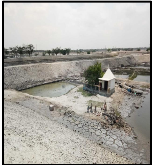
POND AT CHAINAGE 41.8, LEFT BANK
