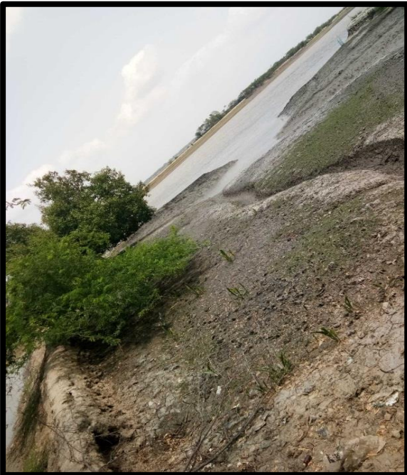
POND AT CHAINAGE 43, LEFT BANK
