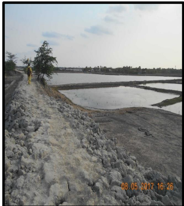
FISHING POND AT CHAINAGE 23, LEFT BANK
