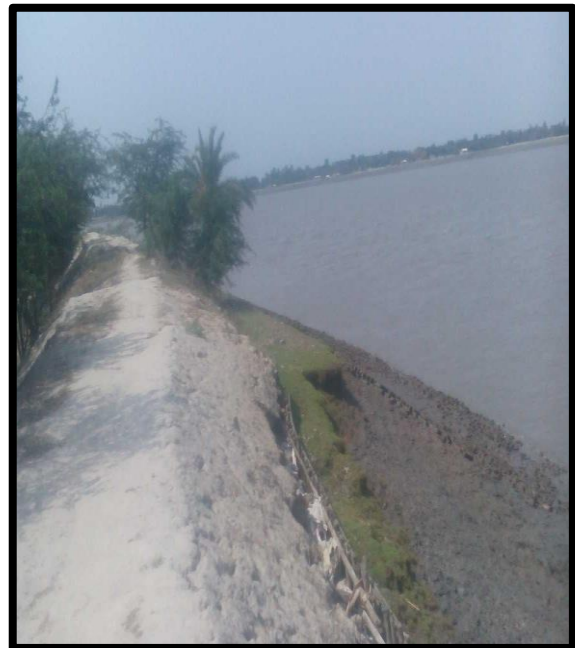
RIVER BANK AT CHAINAGE 31 LEFT BANK
