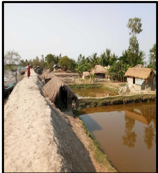
STRUCTURE AT CHAINAGE 8, RIGHT BANK
