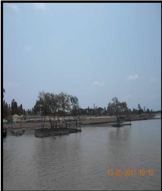
RIVER BANK AT CHAINAGE 0, RIGHT BANK
