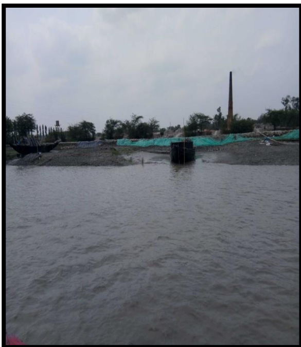
RIVER BANK AT CHAINAGE 49.5, RIGHT BANK
