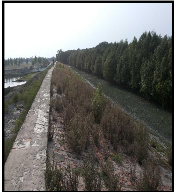
RIVER BANK PROTECTION AT CHAINAGE 6.5, LEFT BANK
