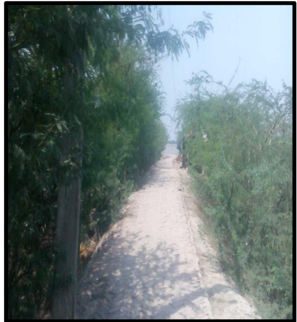
ROAD AT CHAINAGE 30.9, LEFT BANK
