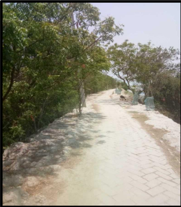
RIVER BANK AT CHAINAGE 35, LEFT BANK
