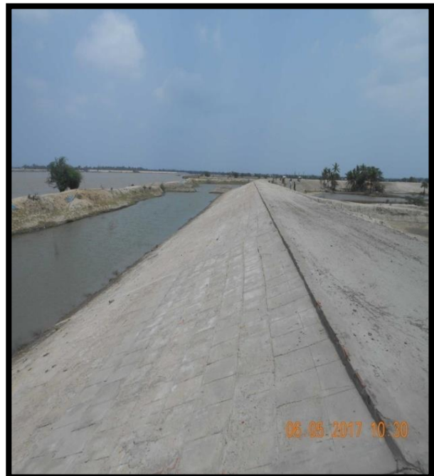
RIVER BANK PROTECTION AT CHAINAGE 41, RIGHT BANK
