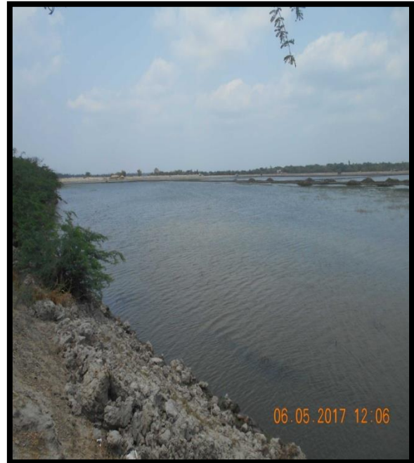
FISHING POND AT CHAINAGE 42.7, RIGHT BANK
