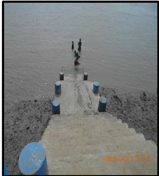
JETTY AT CHAINAGE 20.8, RIGHT BANK
