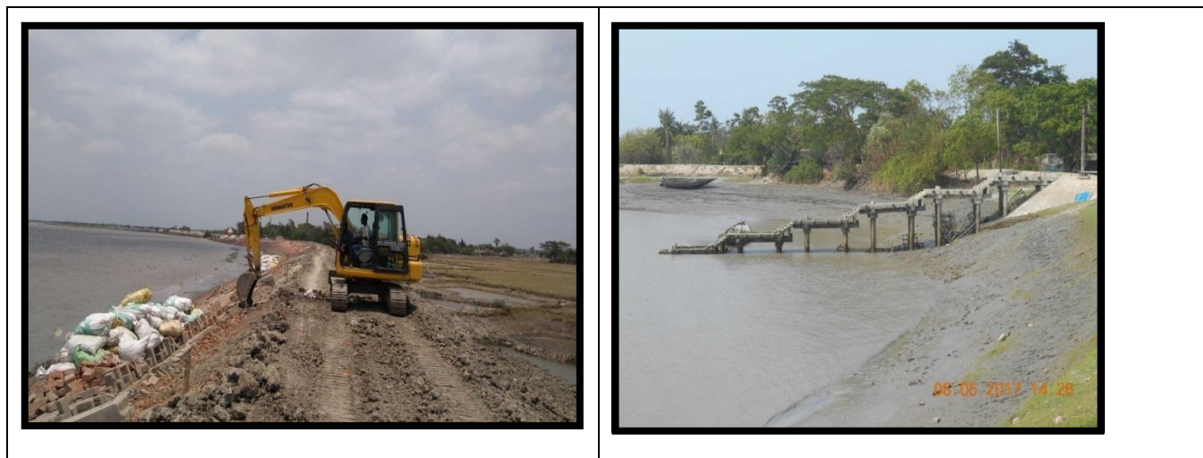
Figure 16: Photograph along Sub-Stretch 4
