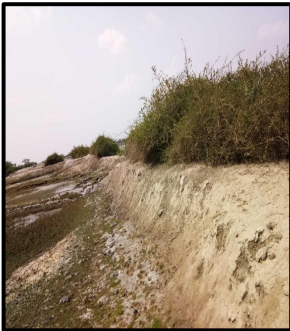
RIVER BANK AT CHAINAGE 43.8, LEFT BANK
