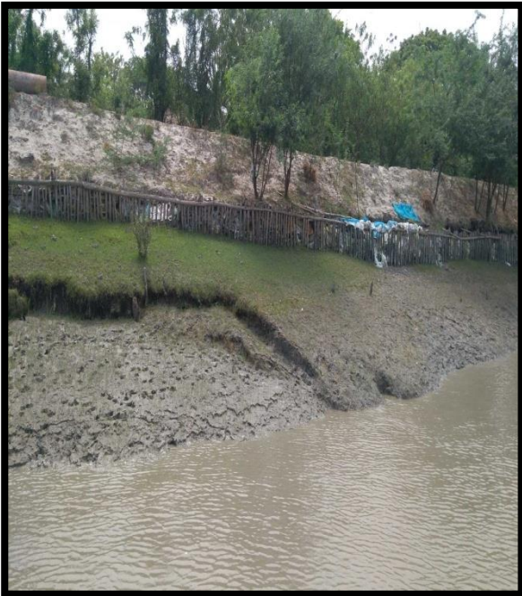
LEFT RIVER BANK AT CHAINAGE 33
