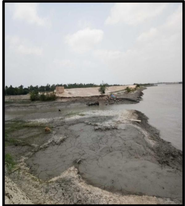
POND AT CHAINAGE 41.6, LEFT BANK
