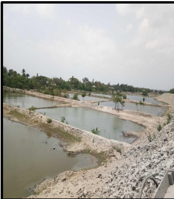
POND AT CHAINAGE 42, LEFT BANK
