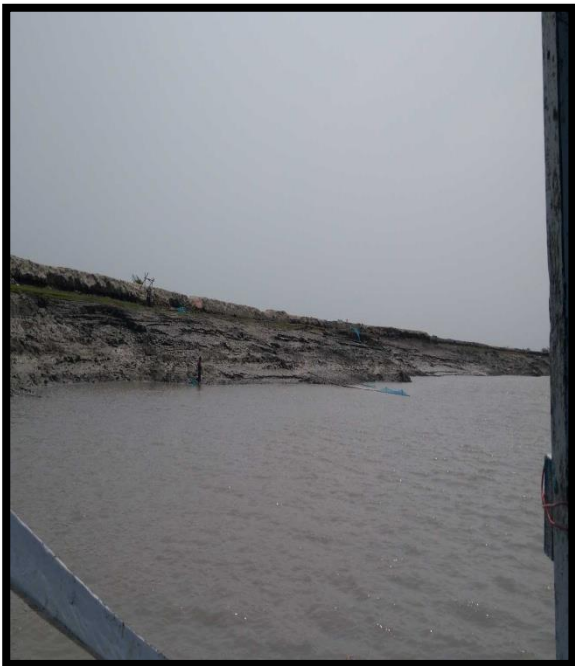
RIGHT RIVER BANK AT CHAINAGE 28.5
