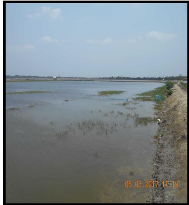
FISHING POND AT CHAINAGE 42, RIGHT BANK
