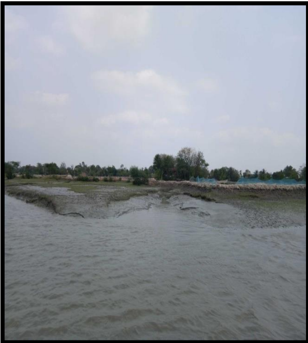
RIVER BANK AT CHAINAGE 48.5, RIGHT BANK
