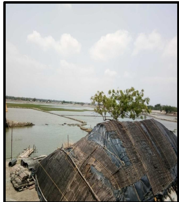
POND AT CHAINAGE 41.2, LEFT BANK
