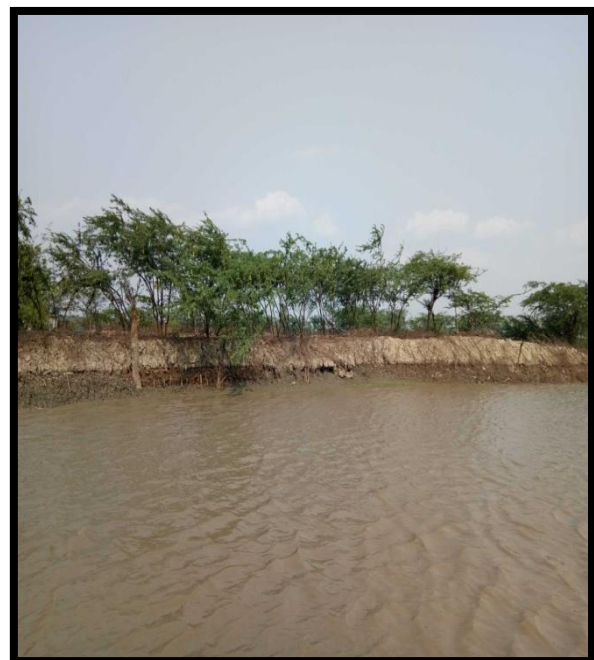
RIVER BANK AT CHAINAGE 43, LEFT BANK
