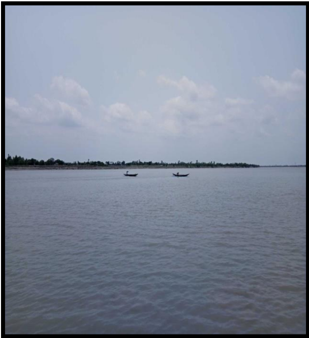
LEFT RIVER BANK AT CHAINAGE 25
