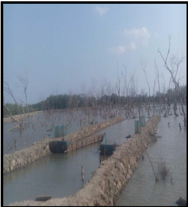
POND AT CHAINAGE 9, LEFT BANK
