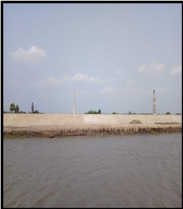
RIVER BANK PROTECTION AT CHAINAGE 41, RIGHT BANK
