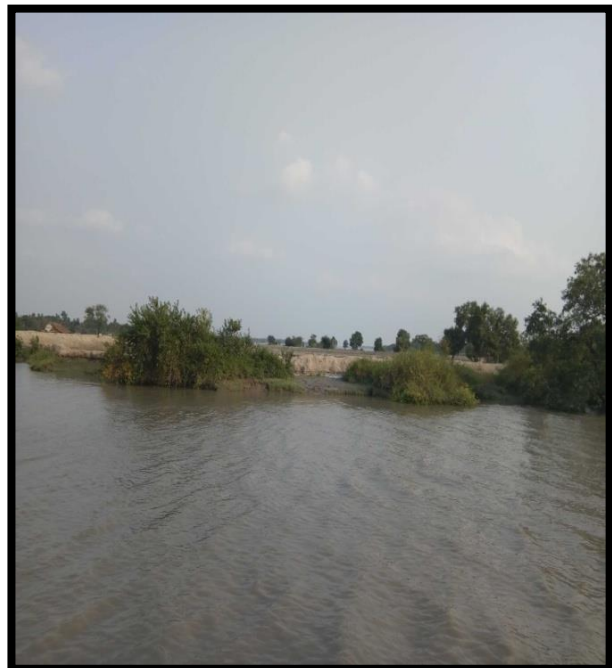
RIVER BANK AT CHAINAGE 36.5, LEFT BANK
