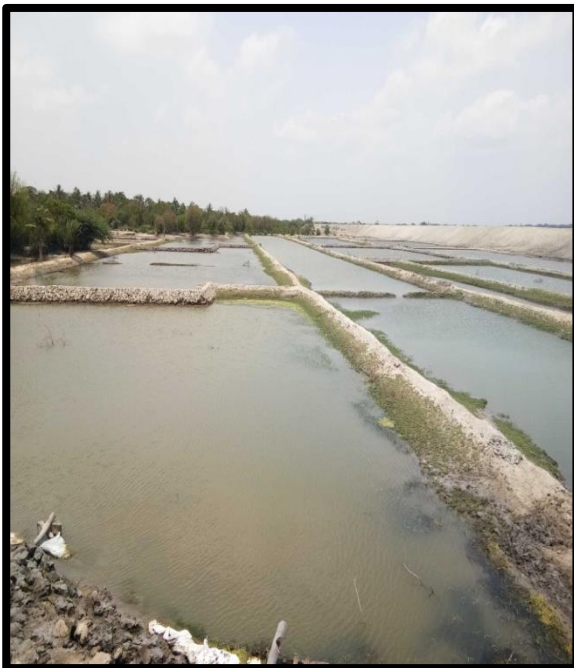
POND AT CHAINAGE 41.7, LEFT BANK
