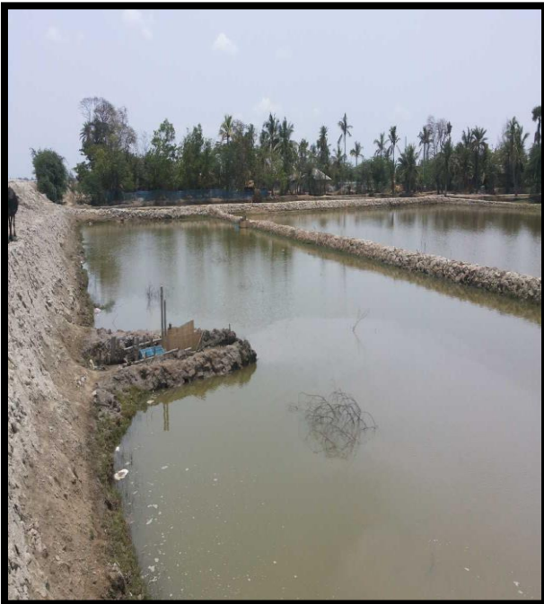
FISHING POND CHAINAGE 14, LEFT BANK
