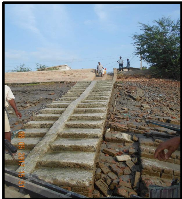
MALAPADA FERRY GHAT AT CHAINAGE 24, RIGHT BANK
