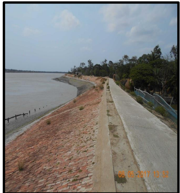
RIVER BANK PROTECTION AT CHAINAGE 22.2, RIGHT BANK
