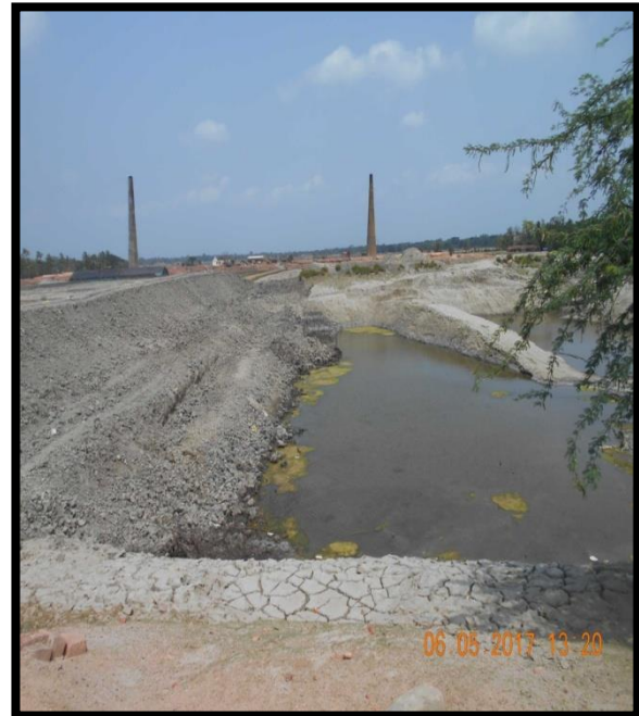
BRICKKILN AT CHAINAGE 44.2, RIGHT BANK
