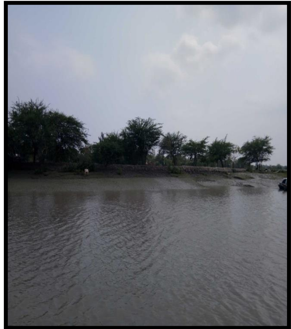
RIVER BANK AT CHAINAGE 48.5, RIGHT BANK
