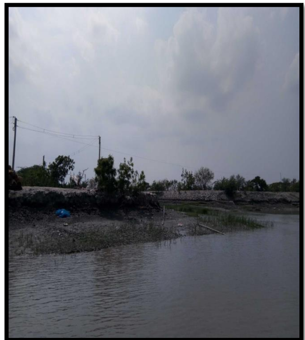
LEFT RIVER BANK AT CHAINAGE 35
