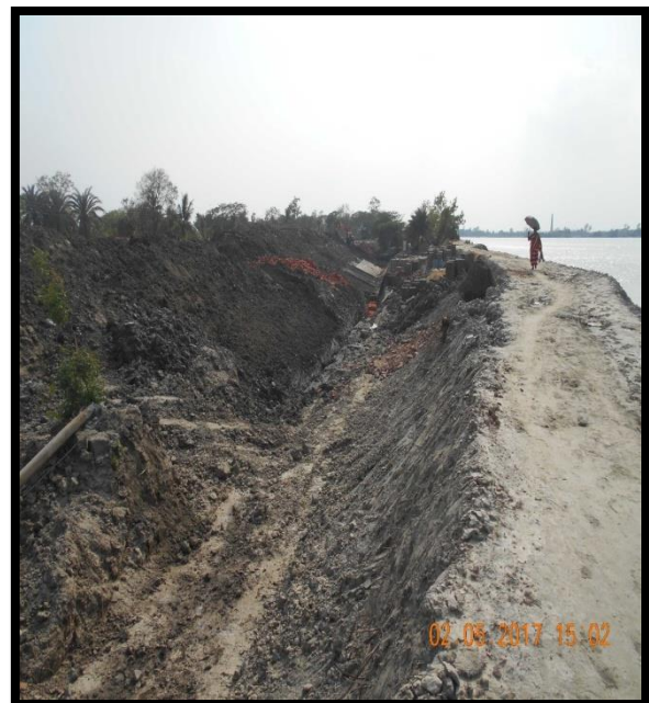
RIGHT RIVER BANK PROTECTION AT CHAINAGE 49.3
