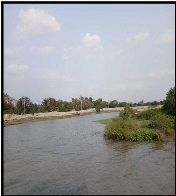
RIVER BANK AT CHAINAGE 37, LEFT BANK
