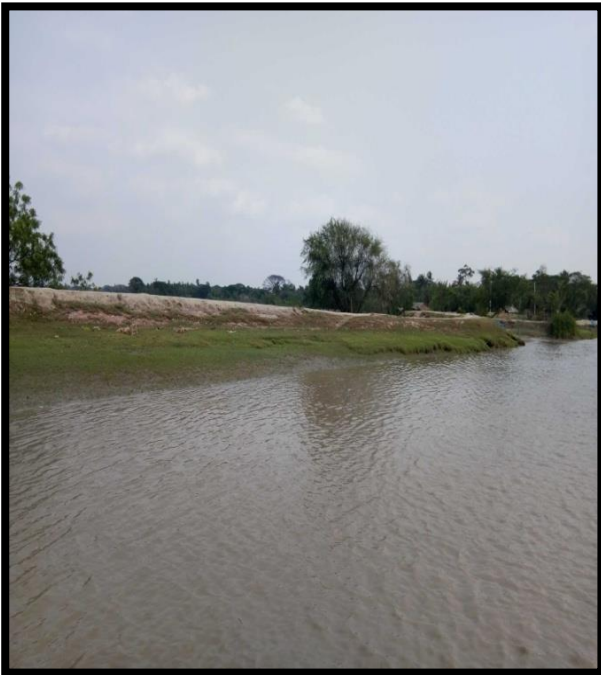
RIVER BANK AT CHAINAGE 46.5, LEFT BANK
