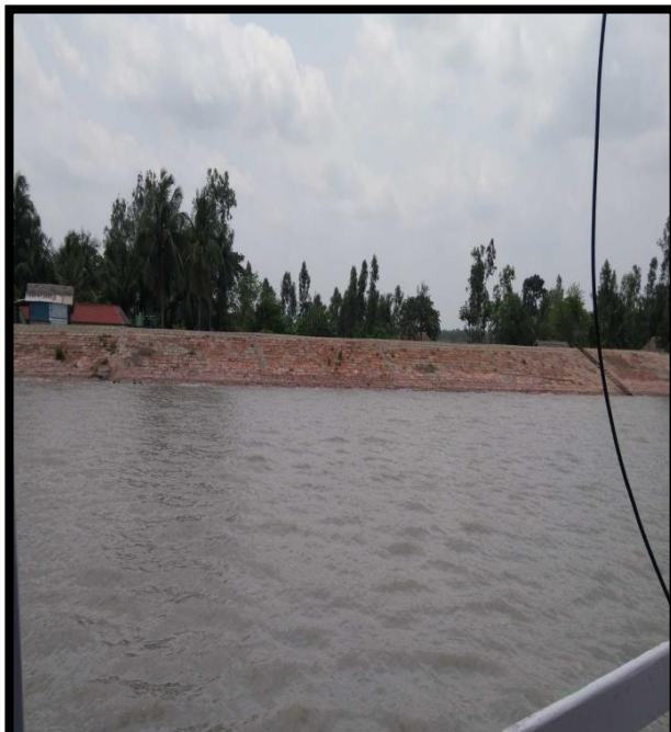
RIVER BANK AT CHAINAGE 0, LEFT BANK
