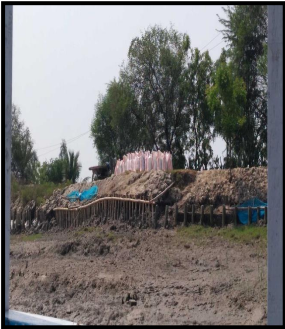
LEFT RIVER BANK AT CHAINAGE 29
