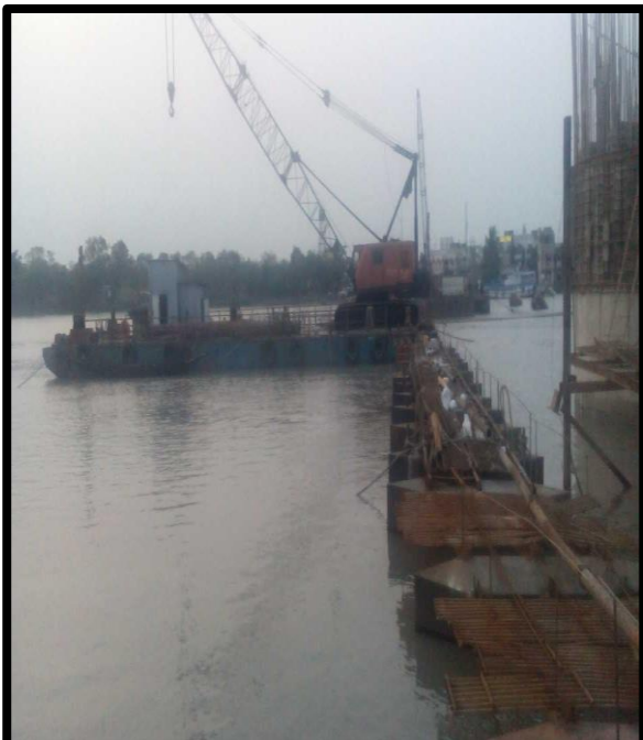
RIGHT RIVER BANK BRIDGE CONSTRUCTION AT CHAINAGE 50
