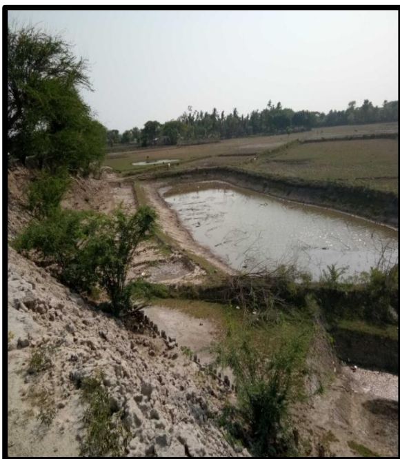
POND AT CHAINAGE 44.9, LEFT BANK
