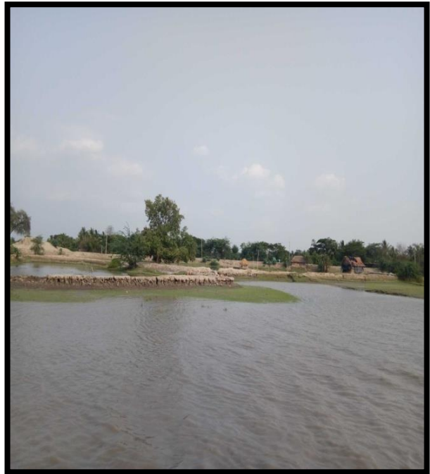
RIVER BANK AT CHAINAGE 39, LEFT BANK
