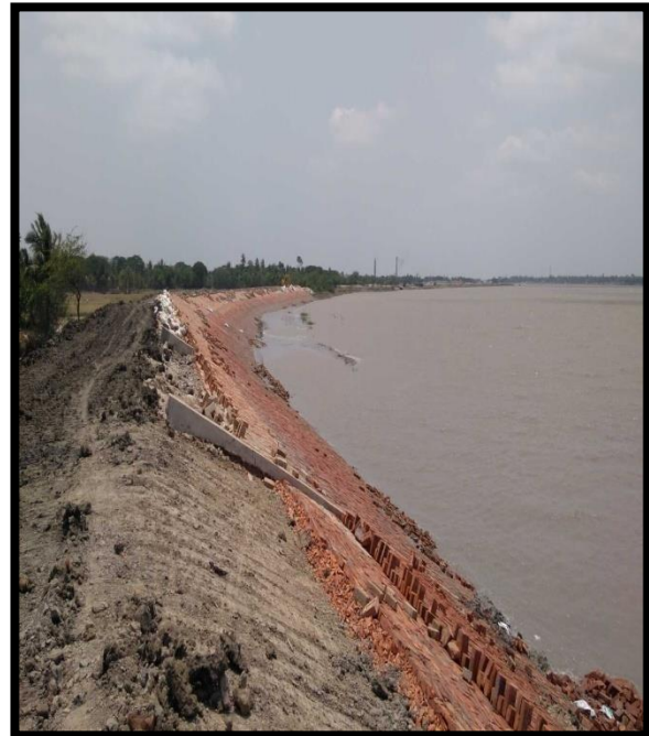
RIVER BANK PROTECTION AT CHAINAGE 40.8, RIGHT BANK
