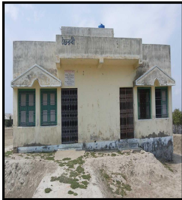
SCHOOL AT CHAINAGE 11.3, LEFT BANK
