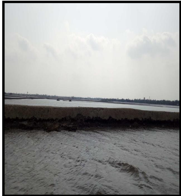
RIVER BANK AT CHAINAGE 23.5, RIGHT BANK
