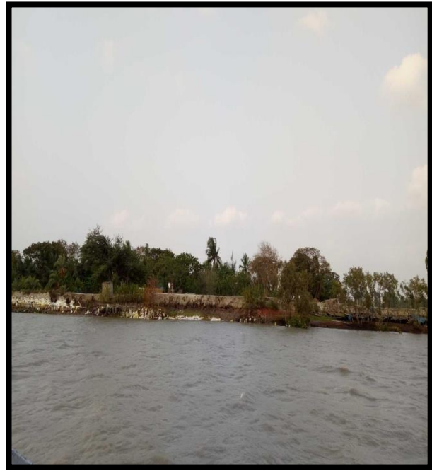
RIVER BANK AT CHAINAGE 25, RIGHT BANK
