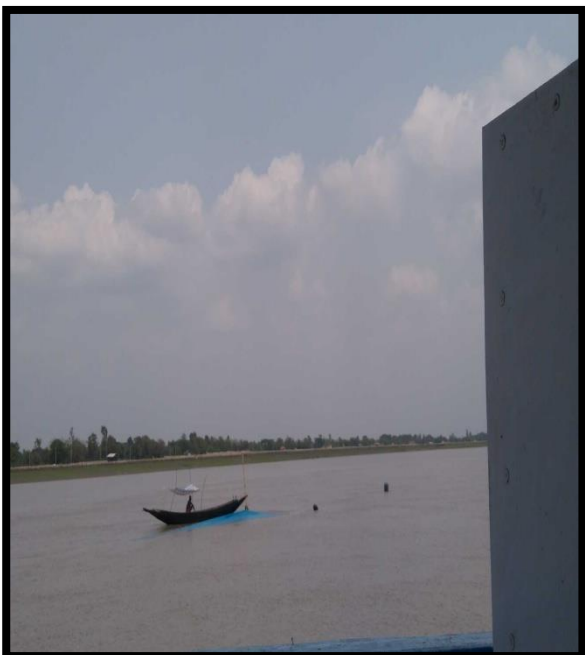
LEFT RIVER BANK AT CHAINAGE 33
