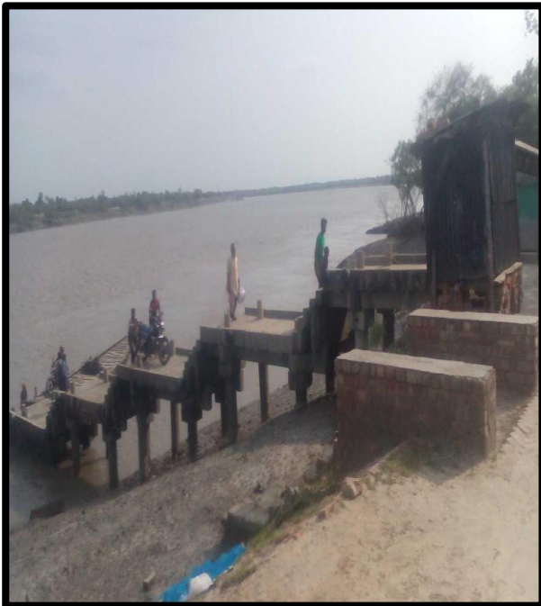
BOLAKALI JETTY AT CHAINAGE 24
