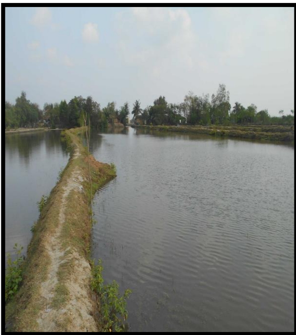
RIGHT RIVER BANK FISHING POND AT CHAINAGE 48
