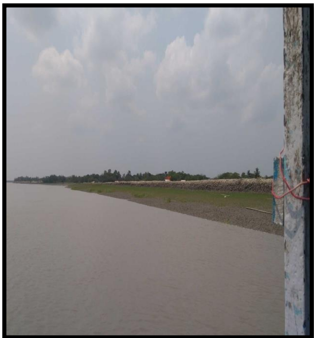
RIGHT RIVER BANK AT CHAINAGE 32.5
