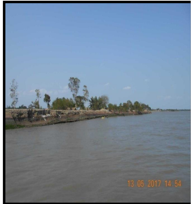
RIVER BANK AT CHAINAGE 14, RIGHT BANK
