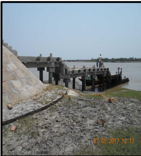
BINDADA JETTY AT CHAINAGE 33.5, RIGHT BANK
