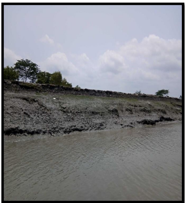
RIGHT RIVER BANK AT CHAINAGE 25
