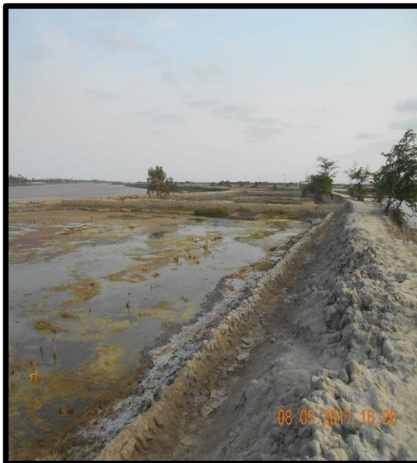
FISHING POND AT CHAINAGE 23.3, LEFT BANK
