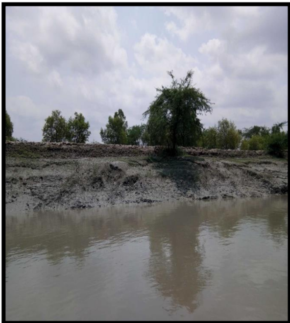
RIGHT RIVER BANK AT CHAINAGE 25.5
