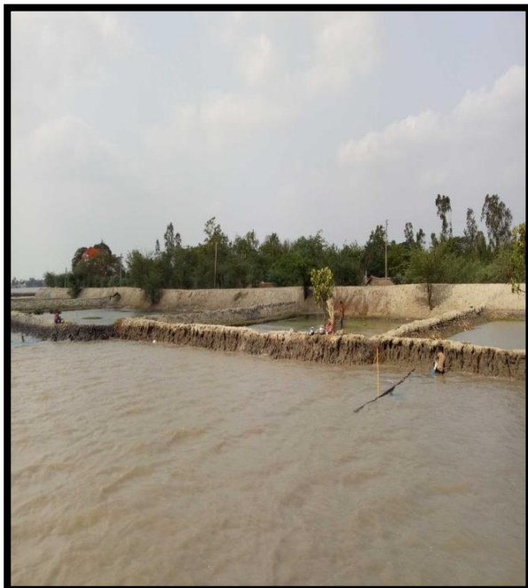
RIVER BANK AT CHAINAGE 23.5, LEFT BANK
