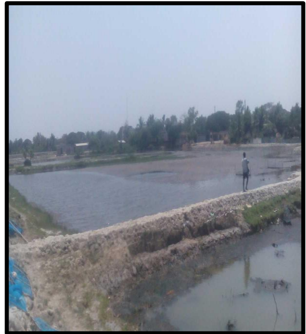
POND AT CHAINAGE 30.5, LEFT BANK
