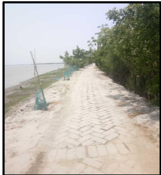
RIVER BANK AT CHAINAGE 35.5, LEFT BANK
