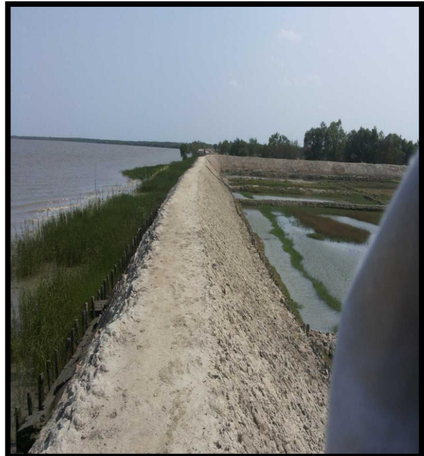
TEMPORARY PROTECTION AT CHAINAGE 9, LEFT BANK
