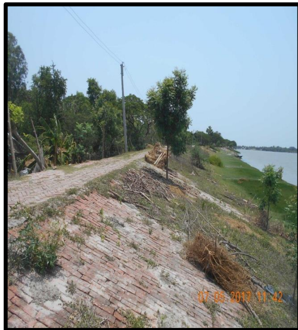
RIVER BANK PROTECTION AT CHAINAGE 34.5, RIGHT BANK
