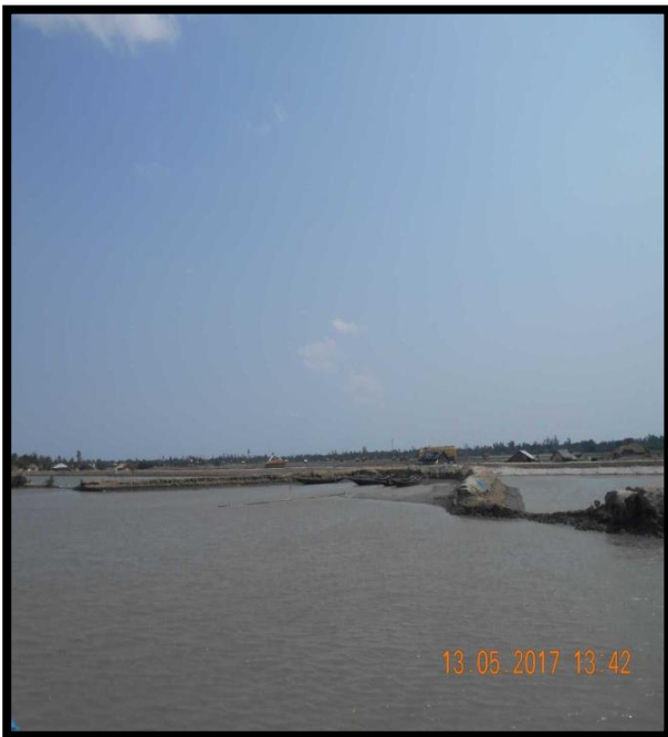
RIVER BANK AT CHAINAGE 16, RIGHT BANK
