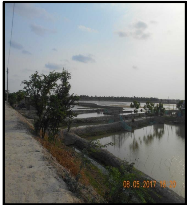
FISHING POND AT CHAINAGE 23.6, LEFT BANK
