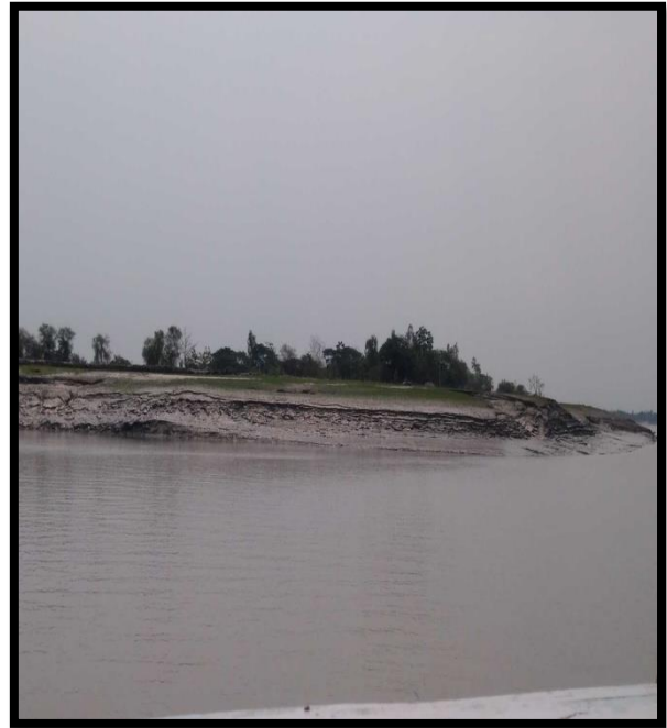
RIGHT RIVER BANK AT CHAINAGE 30
