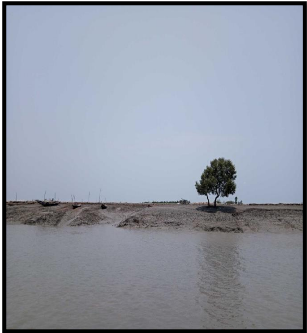
LEFT RIVER BANK AT CHAINAGE 25
