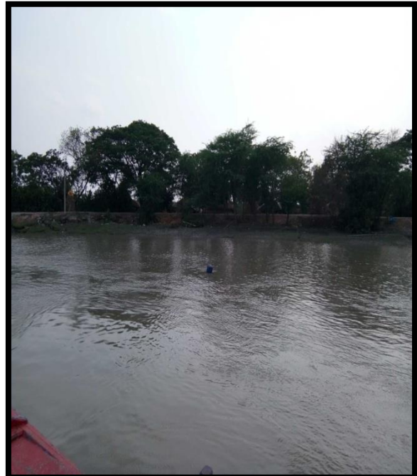
RIVER BANK AT CHAINAGE 45, RIGHT BANK
