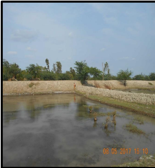
POND AT CHAINAGE 23.5, RIGHT BANK
