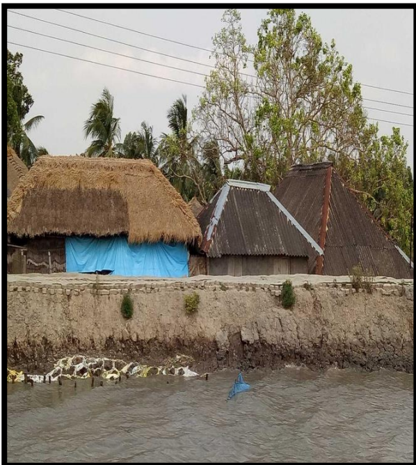
RIVER BANK AT CHAINAGE 21.5, LEFT BANK
