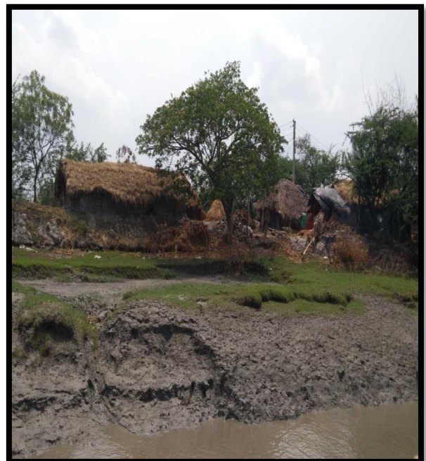
LEFT RIVER BANK AT CHAINAGE 33
