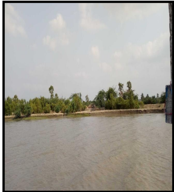
RIVER BANK AT CHAINAGE 24.5, RIGHT BANK
