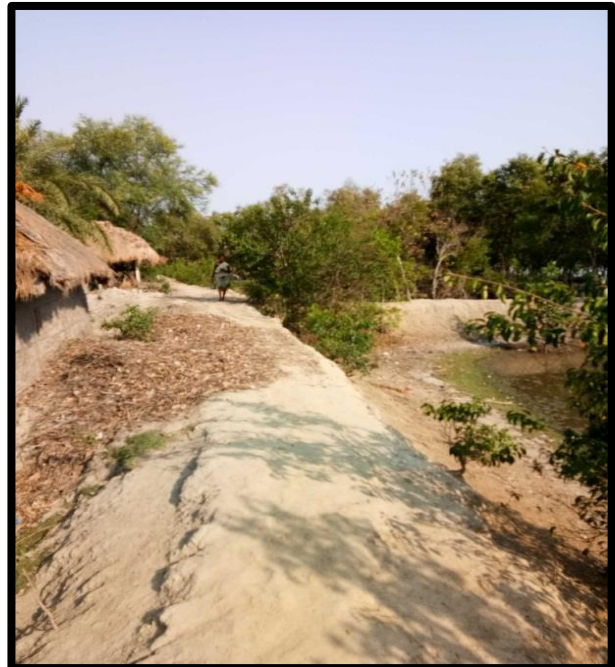
RIVER BANK AT CHAINAGE 5.5, RIGHT BANK
