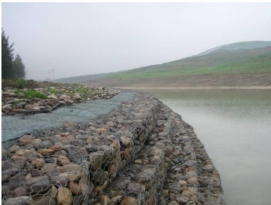
Figure 20: Photograph showing arrangement of Gabion Wall along River Bank
