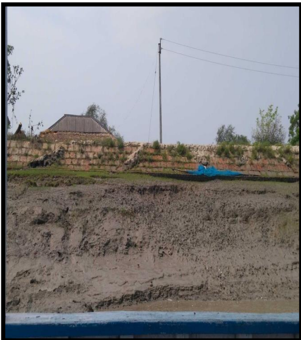
LEFT RIVER BANK AT CHAINAGE 29
