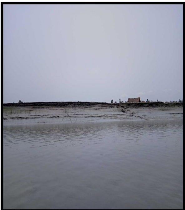
RIGHT RIVER BANK AT CHAINAGE 27
