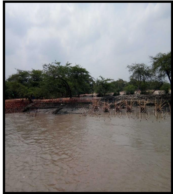
RIVER BANK AT CHAINAGE 49, LEFT BANK
