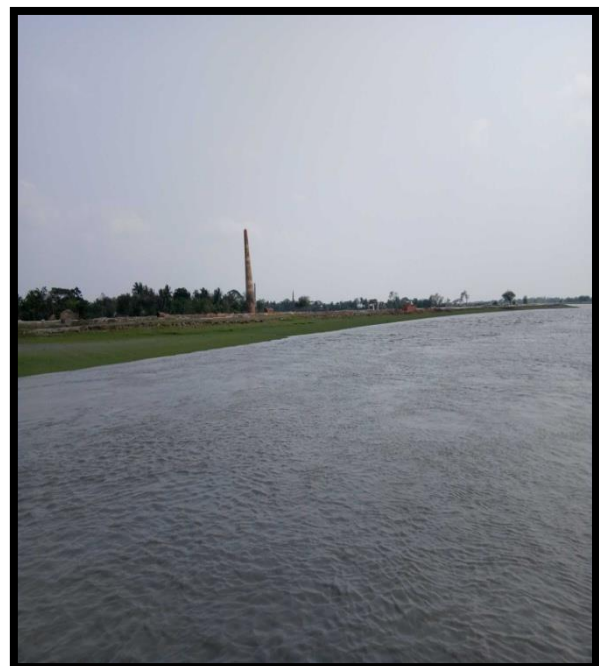
RIVER BANK AT CHAINAGE 45, LEFT BANK
