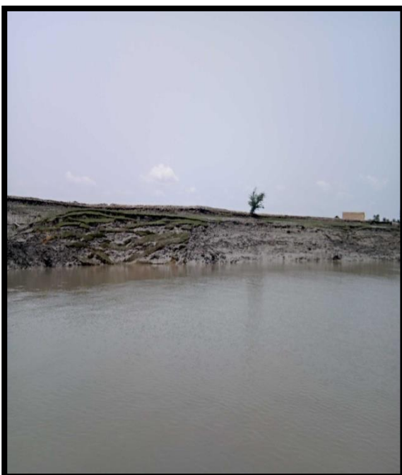
RIGHT RIVER BANK AT CHAINAGE 26.5
