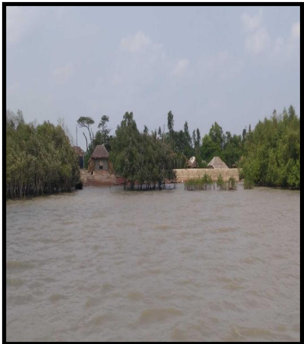
RIVER BANK AT CHAINAGE 2, LEFT BANK
