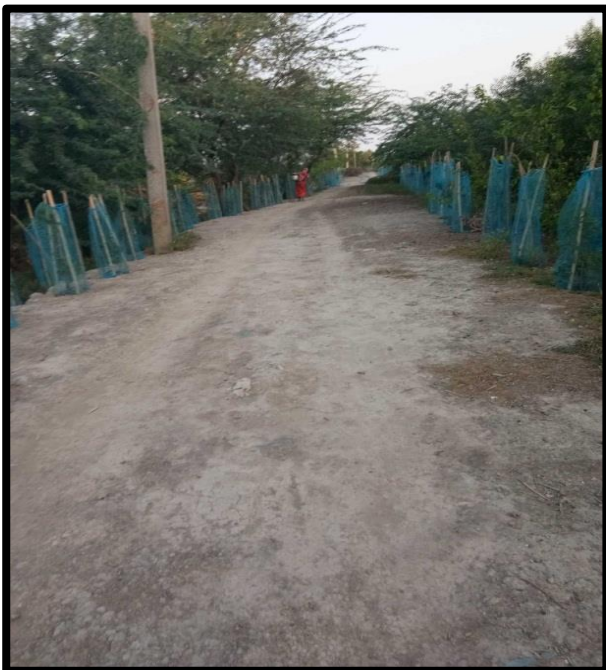
TREE COVER AREA AT CHAINAGE 4, RIGHT BANK
