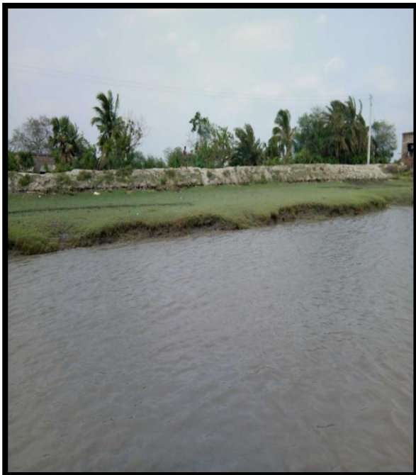
RIVER BANK AT CHAINAGE 45.5, LEFT BANK
