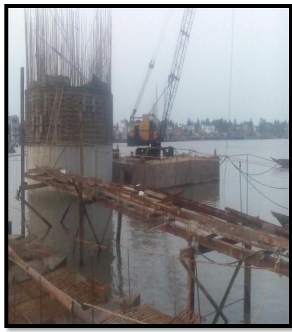
RIGHT RIVER BANK BRIDGE CONSTRUCTION CHAINAGE 50
