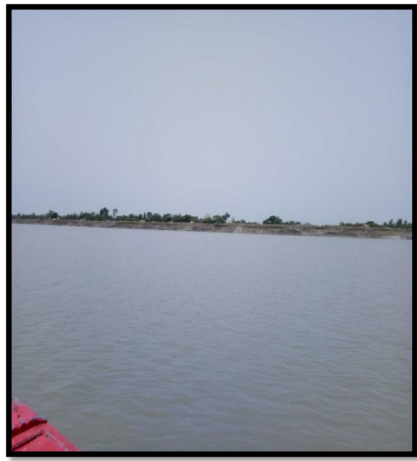
LEFT RIVER BANK AT CHAINAGE 27
