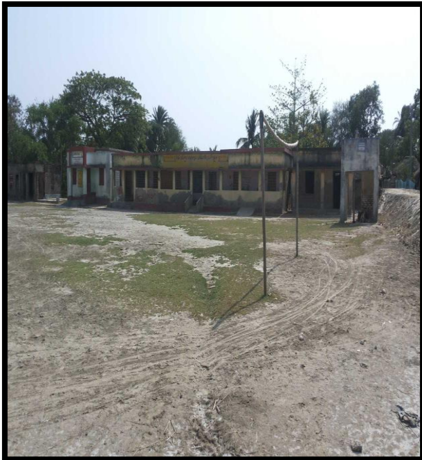
SCHOOL AT CHAINAGE 9.5, LEFT BANK
