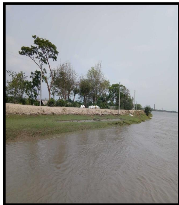
RIVER BANK AT CHAINAGE 46.5, LEFT BANK
