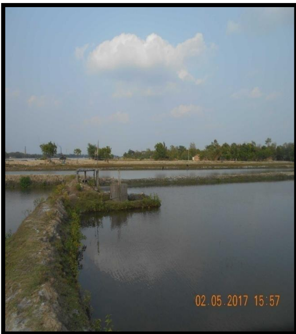
RIGHT RIVER BANK FISHING POND AT CHAINAGE 48.2
