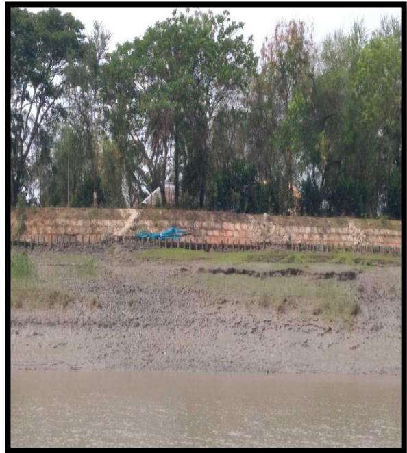
RIGHT RIVER BANK AT CHAINAGE 29
