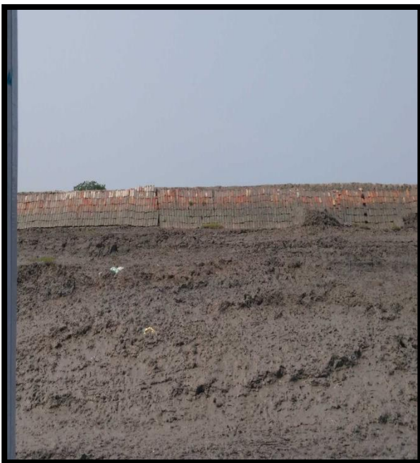
RIGHT RIVER BANK PROTECTION AT CHAINAGE 28.5
