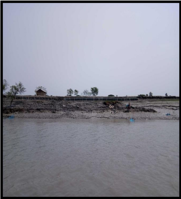
RIGHT RIVER BANK AT CHAINAGE 27.5
