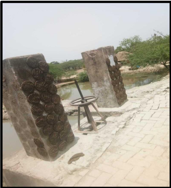
WATER LOCK AT CHAINAGE 34.7, LEFT BANK
