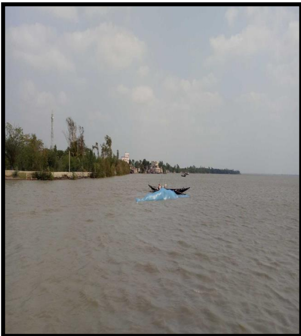
RIVER BANK AT CHAINAGE 20, LEFT BANK
