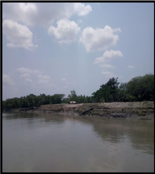
Left River Bank at Chainage 45.7
