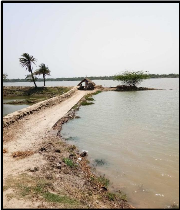
Jetty House at Left Bank Chainage 41.5
