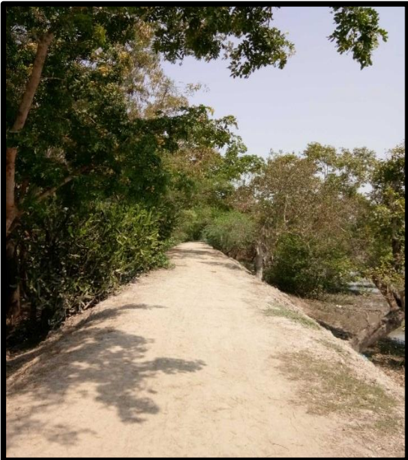
Road at Left Bank Chainage 50
