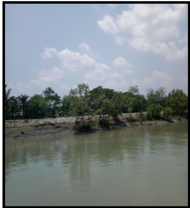
Right River Bank at Chainage 45.7
