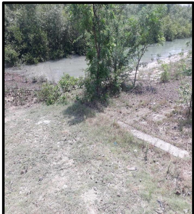
Left River Bank at Chainage 23.2
