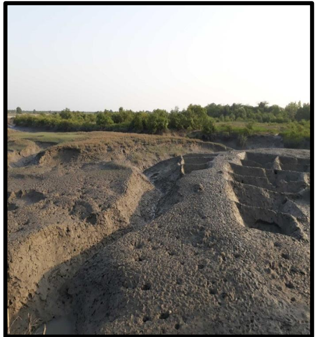
Creek at Left Bank Chainage 31
