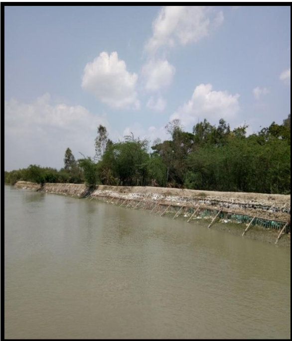
Right River Bank at Chainage 44
