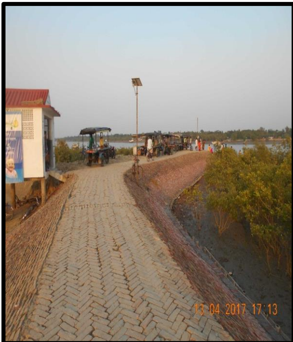
Chandipur Jetty Road at Left Bank Chainage 38
