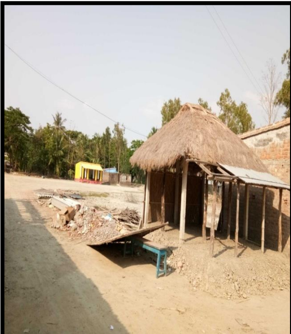
Structure at Right Bank Chainage 52
