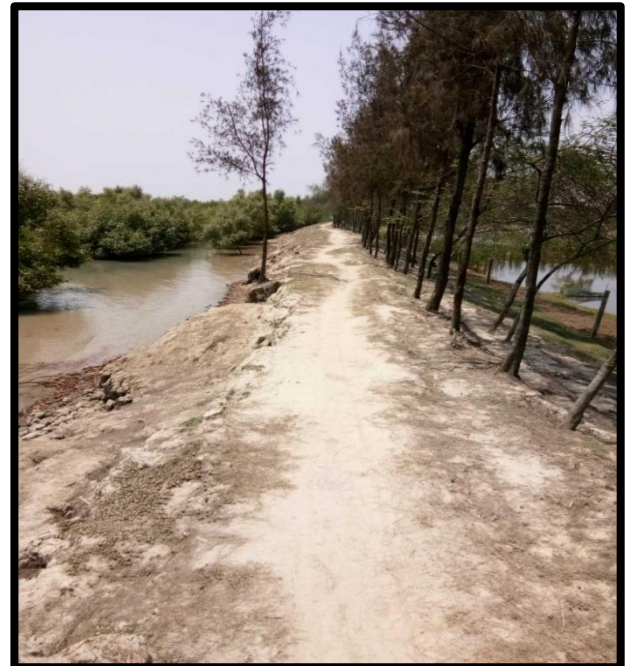
Left River Bank at Chainage 13
