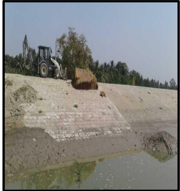
River Bank Protection at Chainage 29.7
