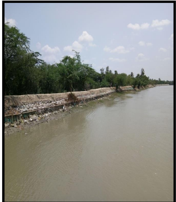
Right River Bank at Chainage 44
