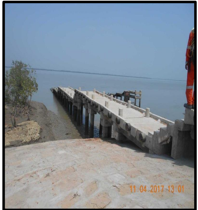
Jetty at Left Bank Chainage 15.7
