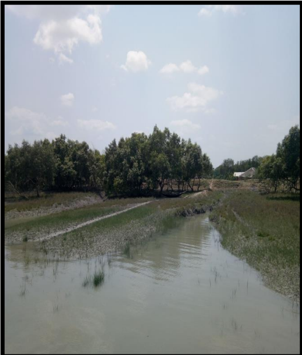
Left River Bank at Chainage 45
