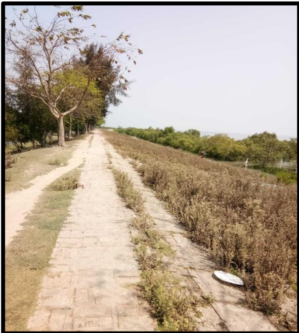
Left River Bank at Chainage 15
