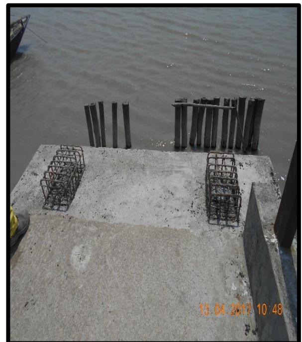
Under Construction Jetty at Left Bank Chainage 37.2
