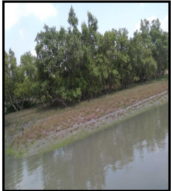
Mangroves Right Bank at Chainage 47.5
