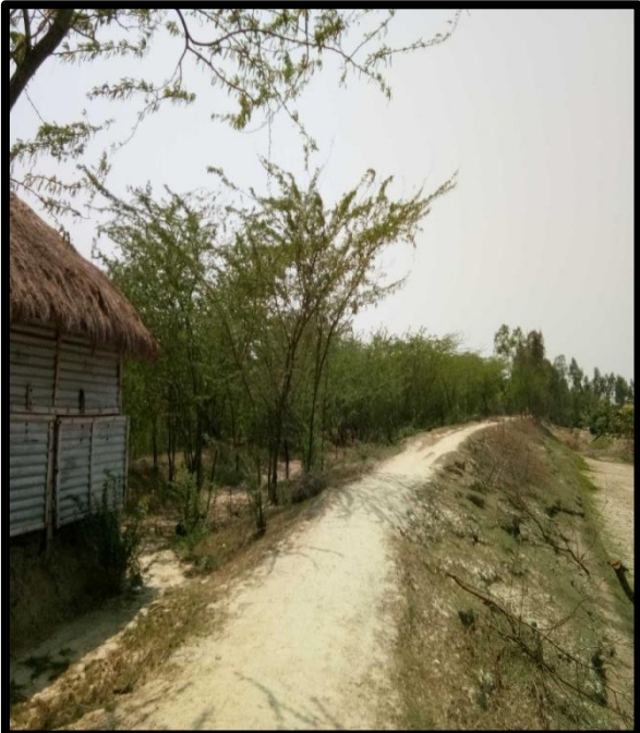
Left River Bank at Chainage 14
