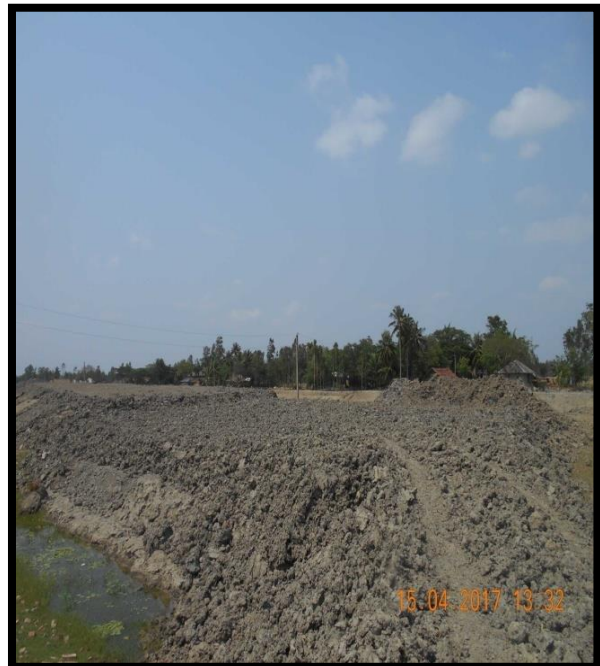
Construction Of New Road at Right Bank Chainage 46.7
