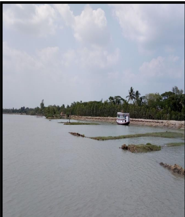
River Bank at Left Bank Chainage 40.5
