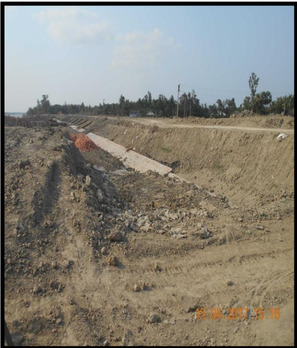
Construction of New Road at Right Bank Chainage 45.2
