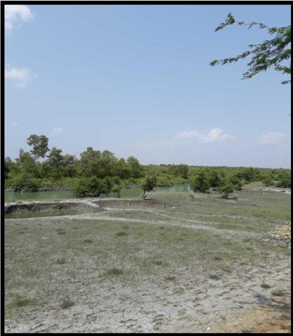
Mangrove at Right Bank Chainage 31.5
