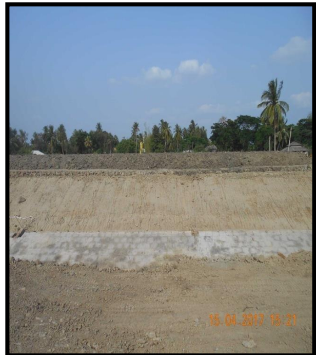
Construction of New Road at Right Bank Chainage 45.2
