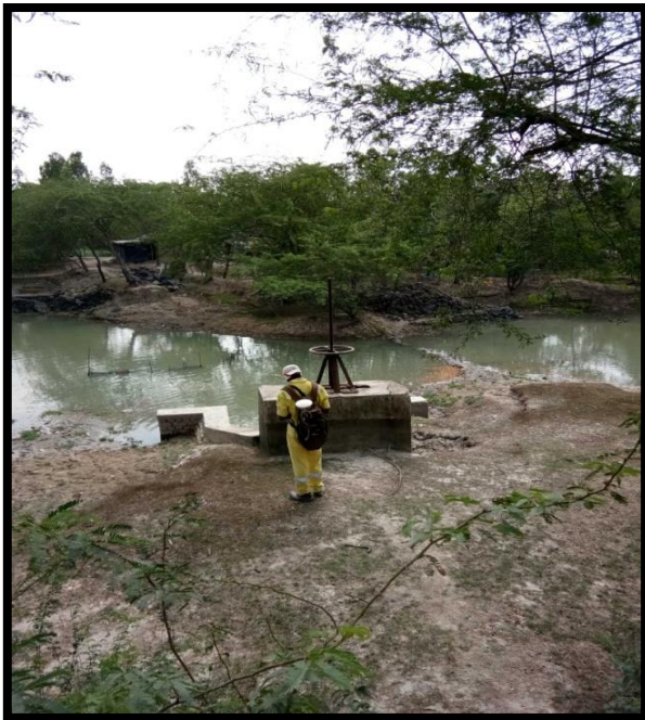
Water Lock at Right Bank Chainage 51.5
