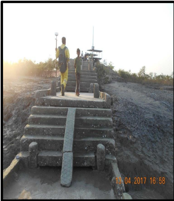
Chandipur Jetty Ghat at Left Bank Chainage 38
