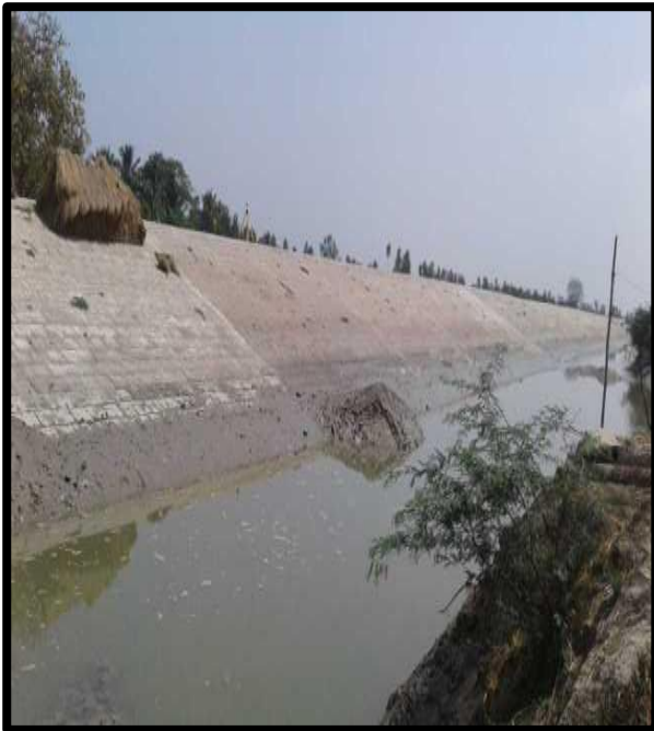
Right River Bank Protection at Chainage 29.7
