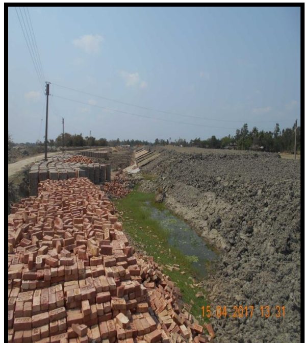
Construction of New Road at Right Bank Chainage 46.8
