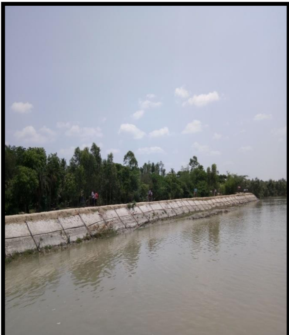
Right River Bank at Chainage 43.5
