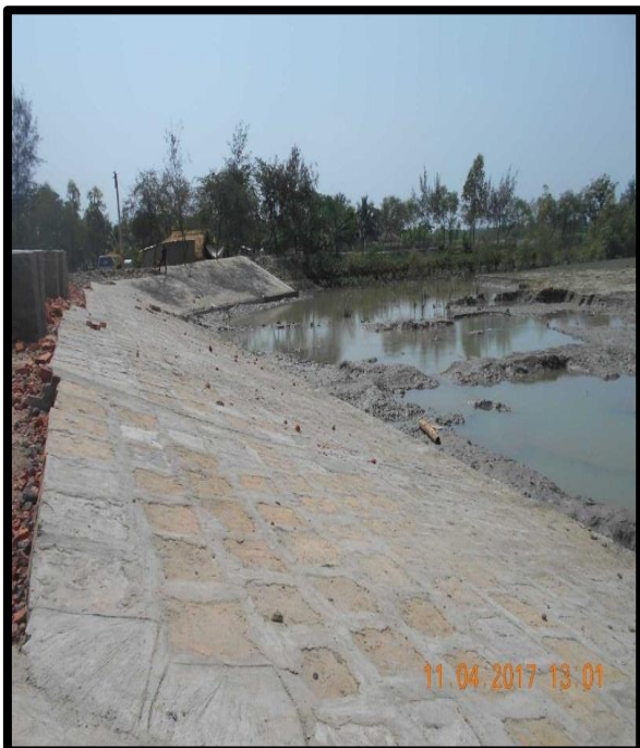
Left River Bank Protection at Chainage 15.7
