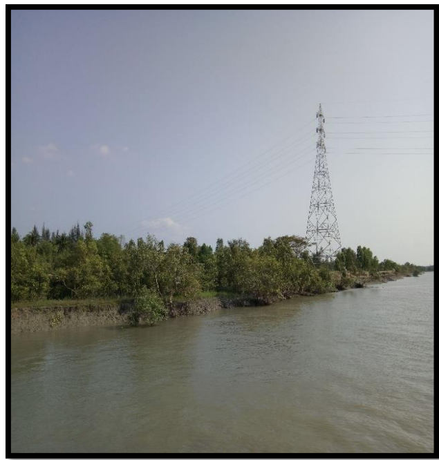
High Tension Line at Right Bank Chainage 35.6
