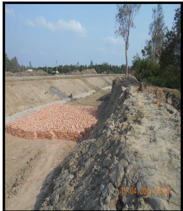
Construction of New Road at Right Bank Chainage 45.3
