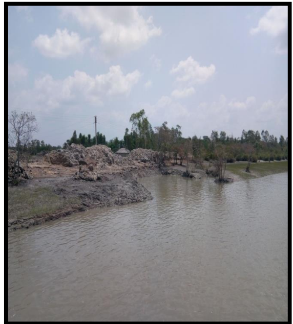
Right River Bank at Chainage 46.3
