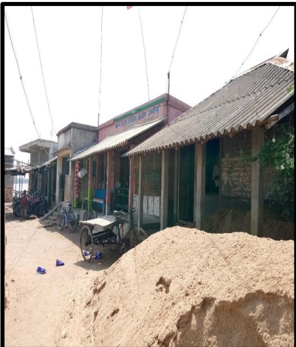
Structure at Left Bank Chainage 39.5
