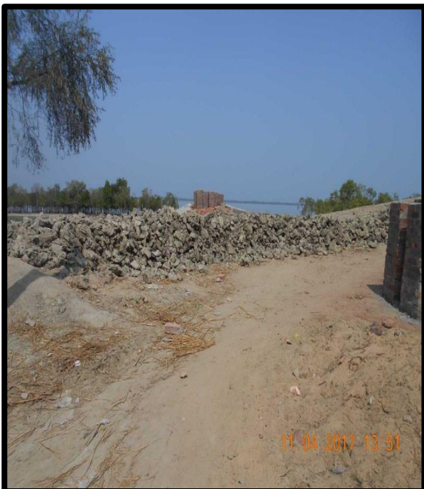
Under Construction Left River Bank at Chainage 15.8
