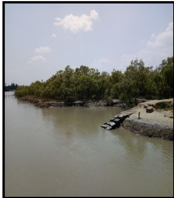
Jetty at Left Bank Chainage 43.5
