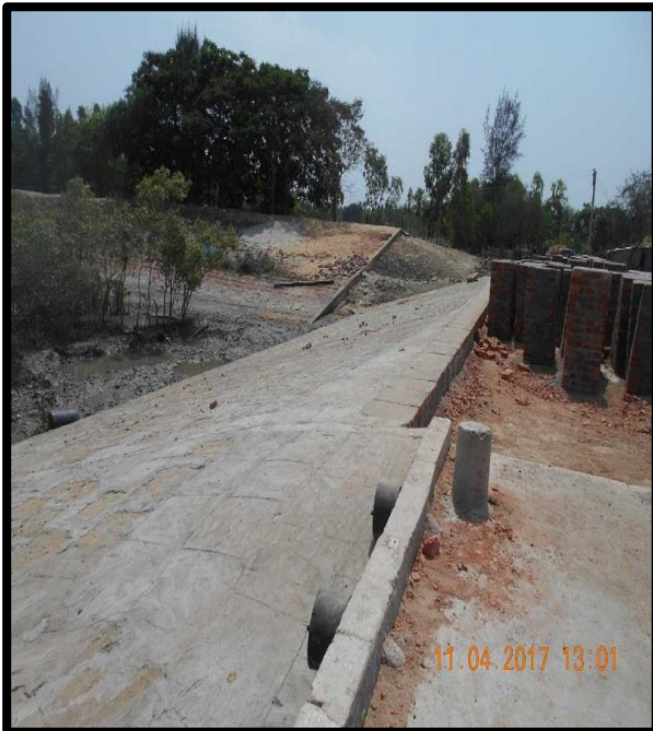
Left River Bank Protection at Chainage 15.7
