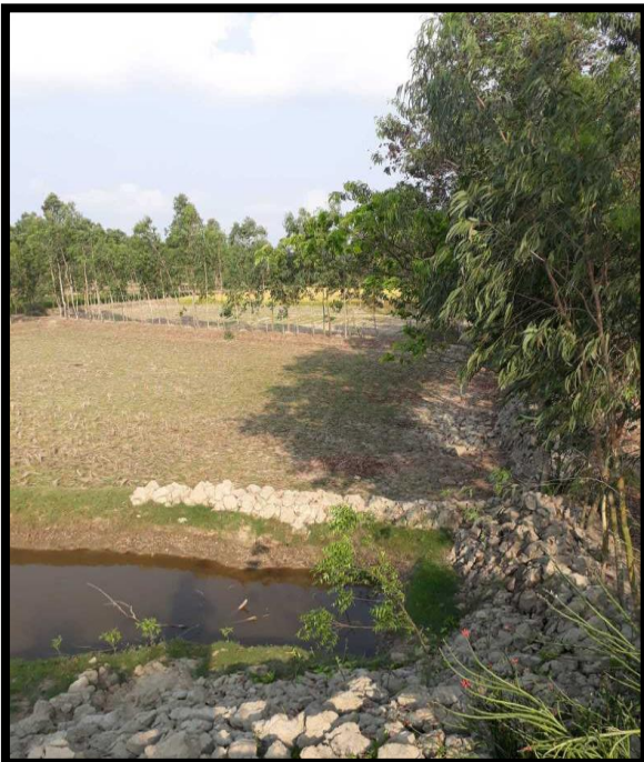
Land at Right Bank Chainage 35.4
