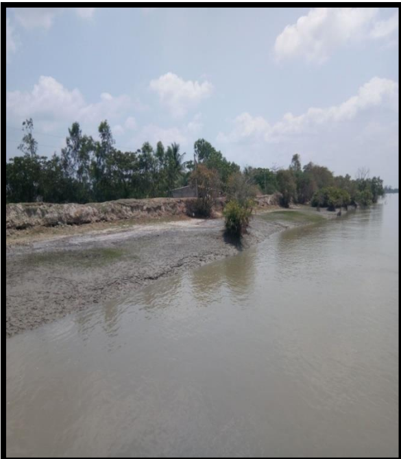
Left River Bank at Chainage 45.8
