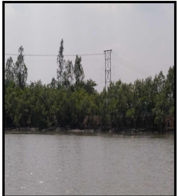
High Tension Line at Right Bank Chainage 48.5
