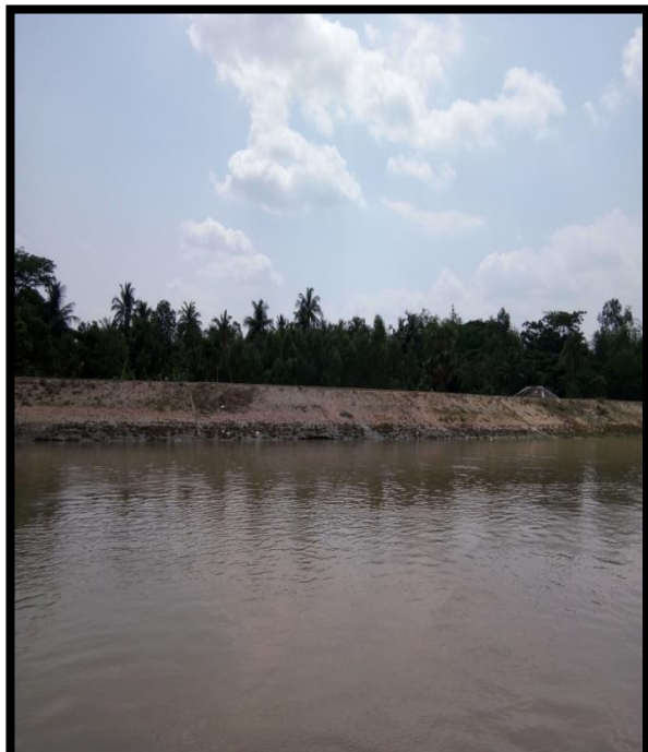
Right River Bank Protection at Chainage 42
