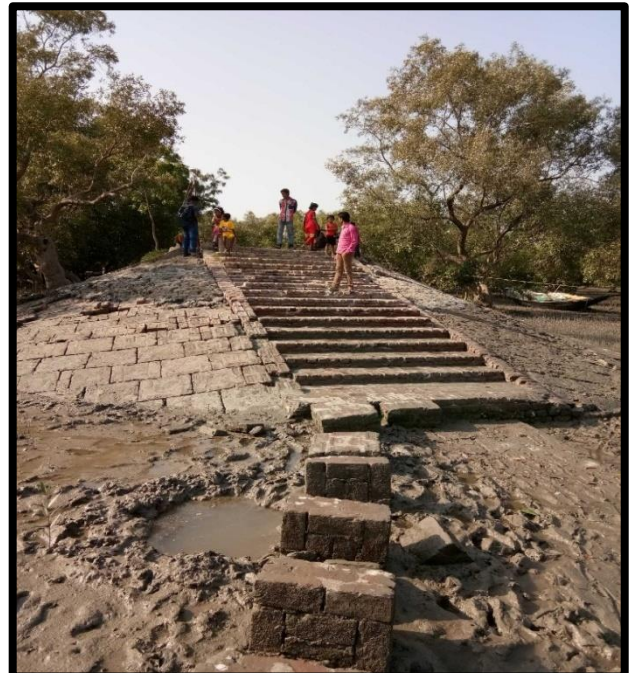
Radharanipur Jetty at Left Bank Chainage
