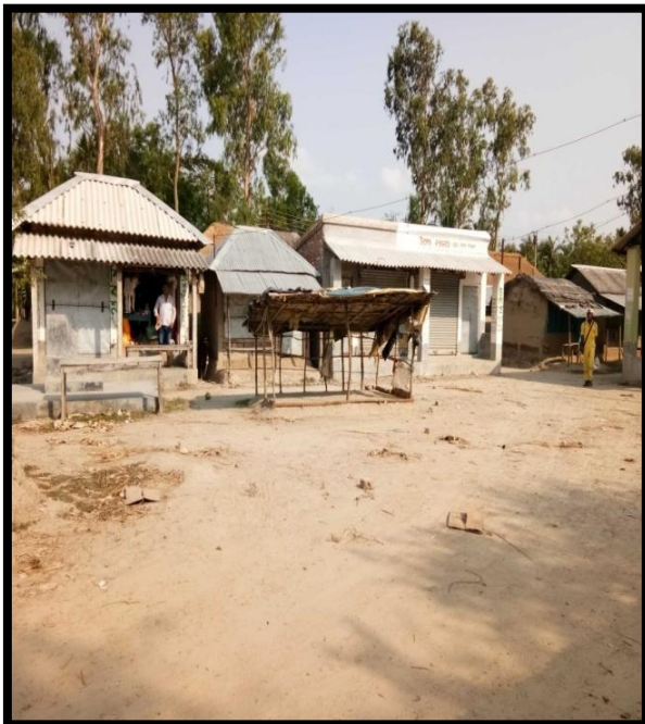
Structure at Right Bank Chainage 52
