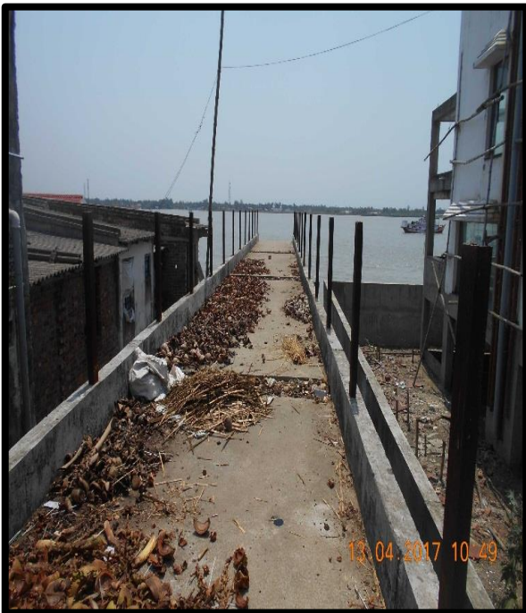
Under Construction Jetty at Left Bank Chainage 37.2
