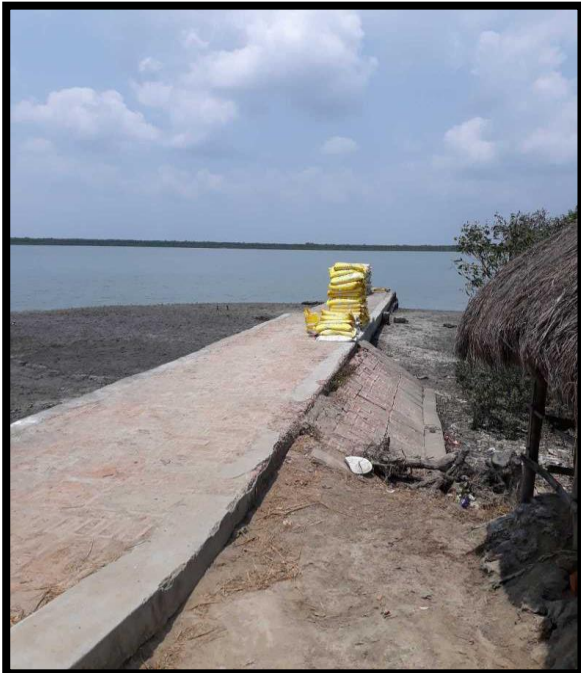
Jetty at Right Bank Chainage 30
