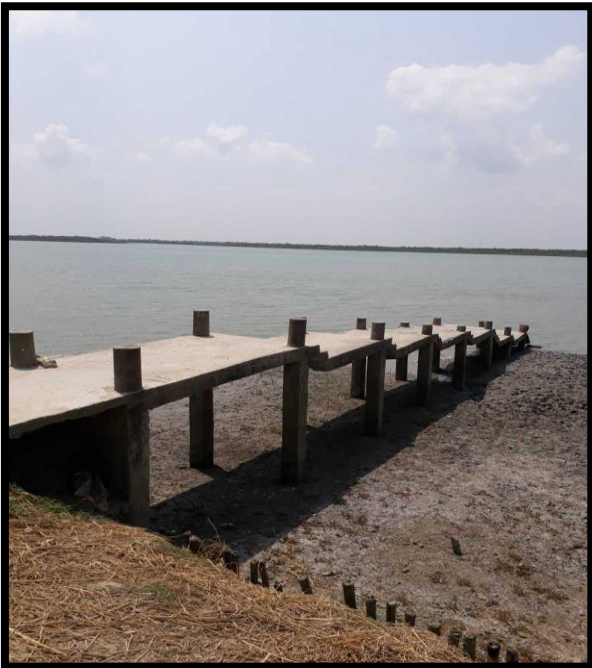
Balli Jetty at Right Bank Chainage 31
