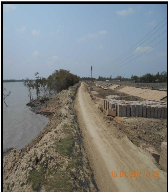
Construction Of New Road at Right Bank Chainage 46.7
