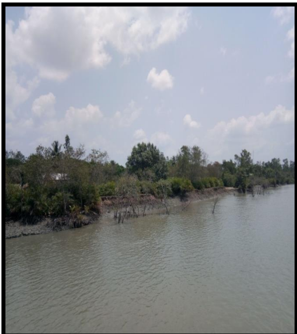
Right River Bank at Chainage 45.5
