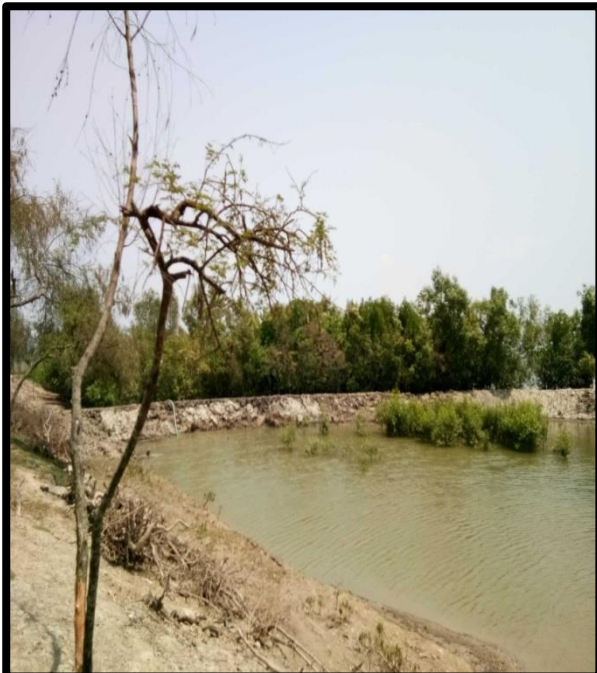
Creek at Left Bank Chainage 29.5
