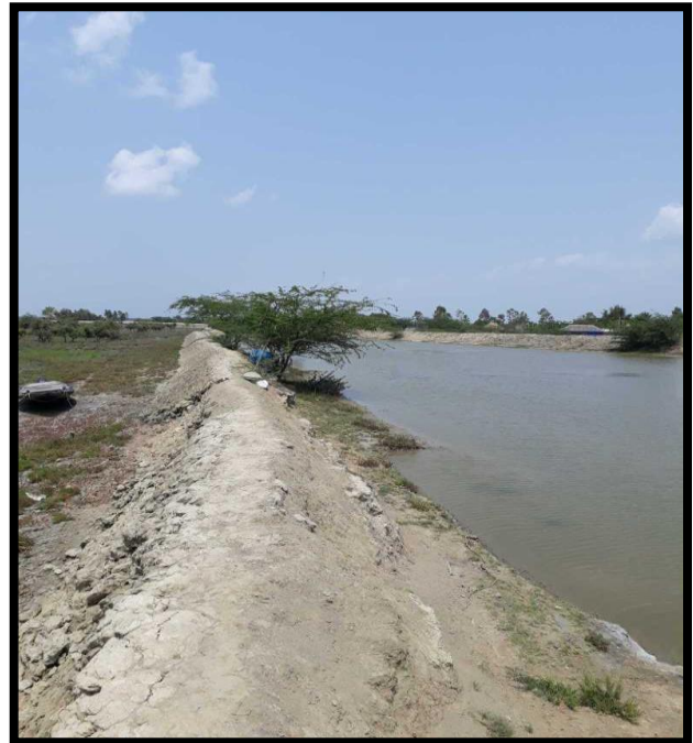
Pond at Right Bank Chainage 30.6
