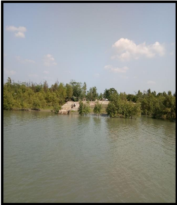
Right River Bank at Chainage 36.9
