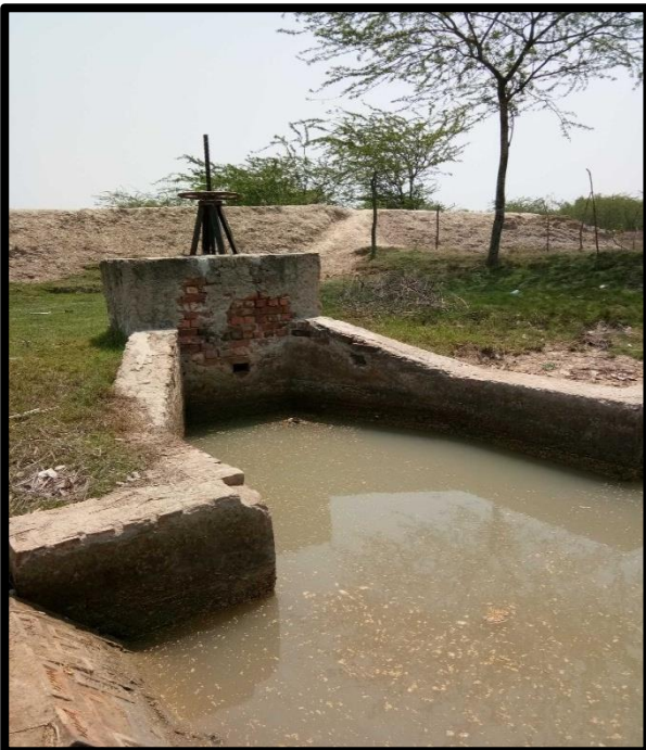
Water Lock at Left Bank Chainage 14
