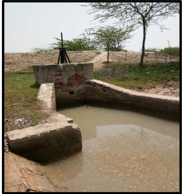
Water Lock at Left Bank Chainage 14
