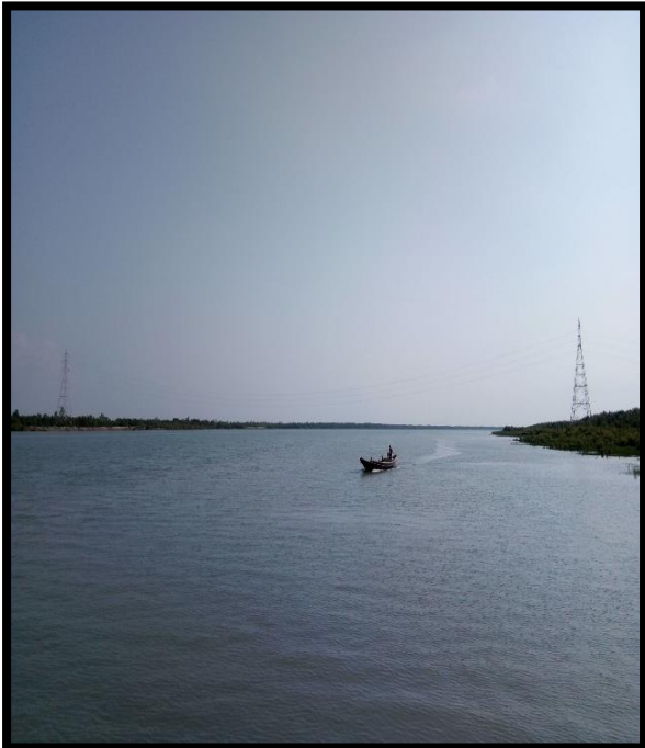
Left River Bank at Chainage 35.8
