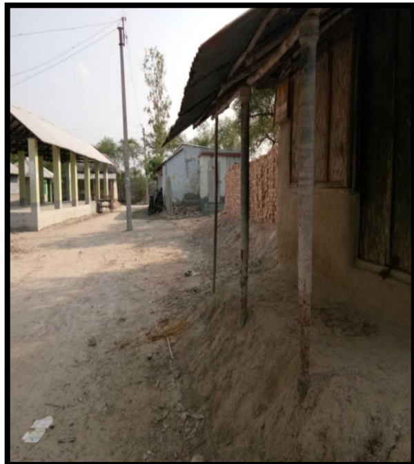
Structure Right Bank at Chainage 52
