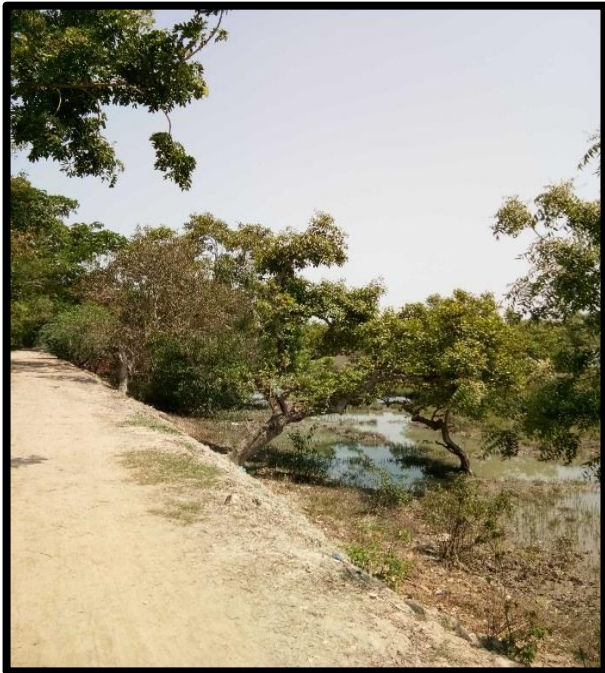
Road at Left Bank Chainage 48
