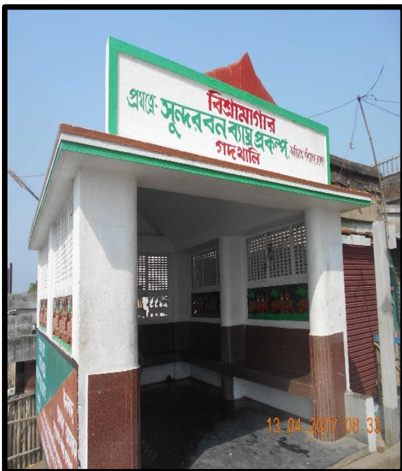
Gadkhali Jetty No.3 Waiting Shed at Left Bank Chainage 37.2
