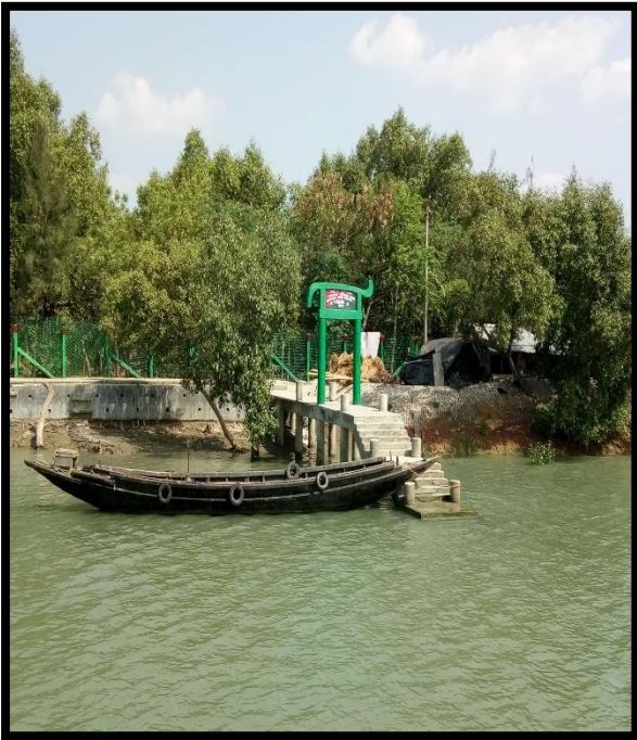
Right River Bank at Chainage 37.8
