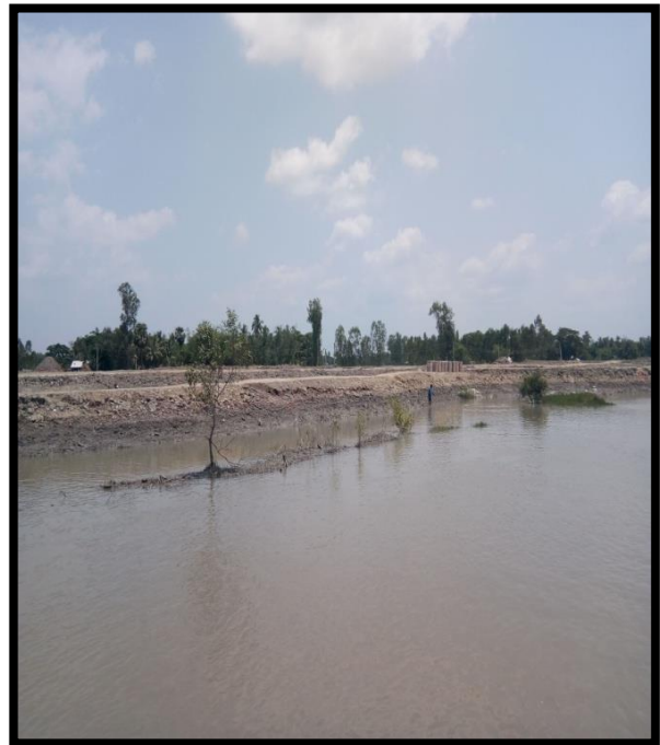
Right River Bank at Chainage 44.5
