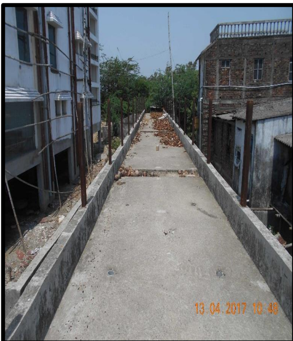
Under Construction Jetty at Left Bank Chainage 37.2
