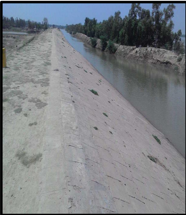
Right River Bank Protection at Chainage 29.7
