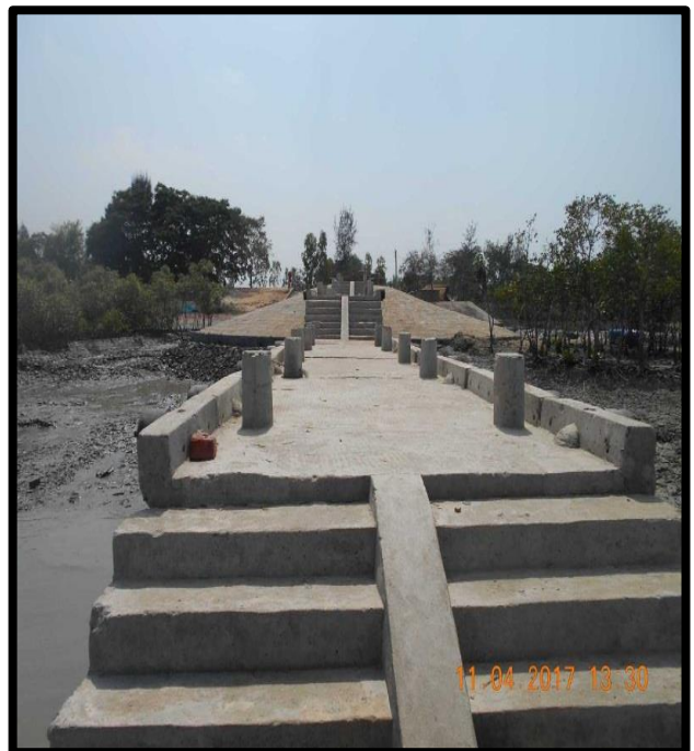
Jetty at Left Bank Chainage 15.7
