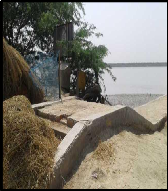
Bally Taltala Ghat at Chainage 29.7
