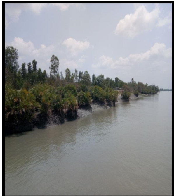
Right River Bank at Chainage 45.8
