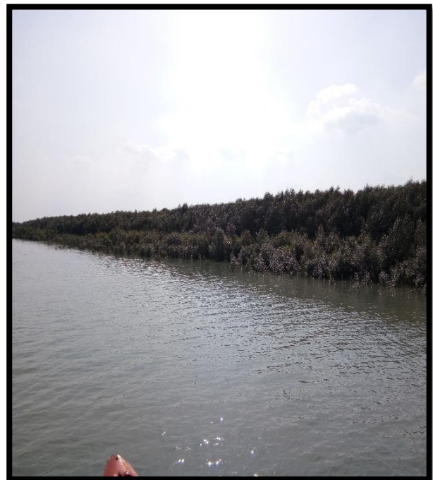
Left River Bank at Chainage 36.8
