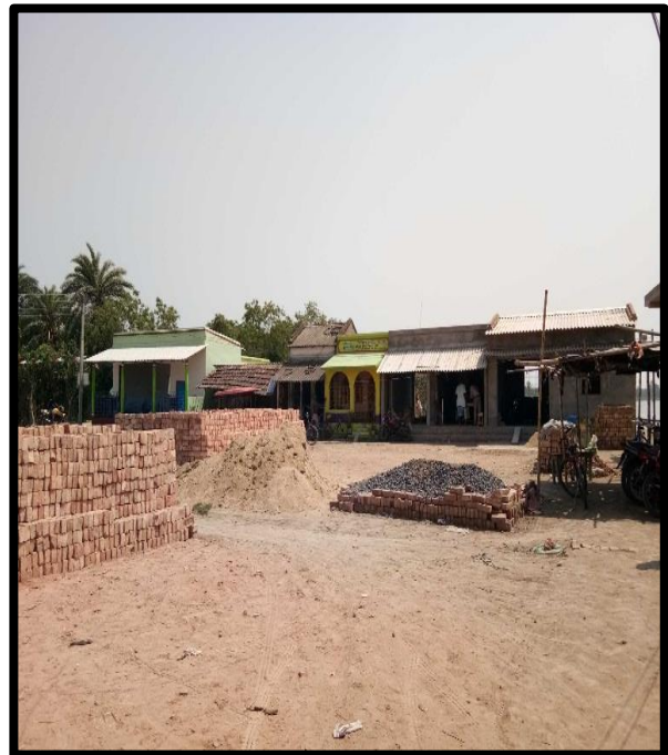
Structure at Left Bank Chainage 39.5
