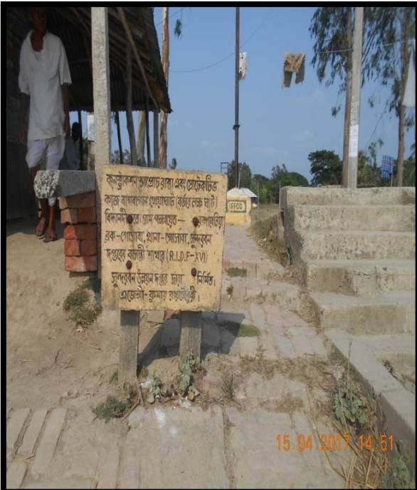
Bagbagan Jetty at Right Bank Chainage 45
