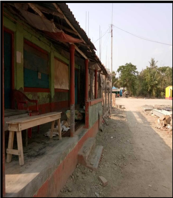
Structure at Right Bank Chainage 52.8
