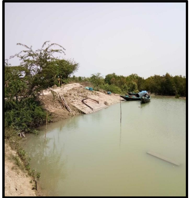
Left River Bank at Chainage 14
