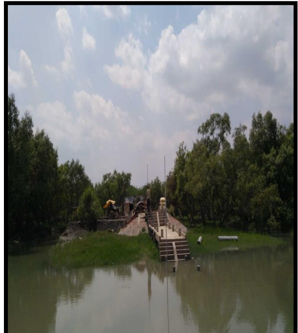
Jetty at Left Bank Chainage 52.5
