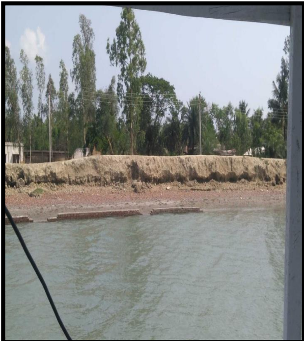
Right River Bank at Chainage 26
