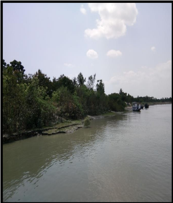
Right River Bank at Chainage 43
