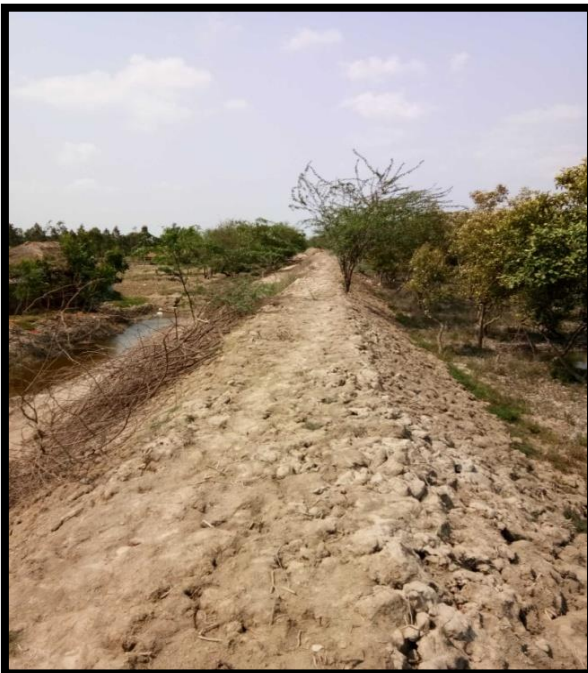
Right River Bank at Chainage 52.5
