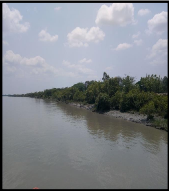
Right River Bank at Chainage 46
