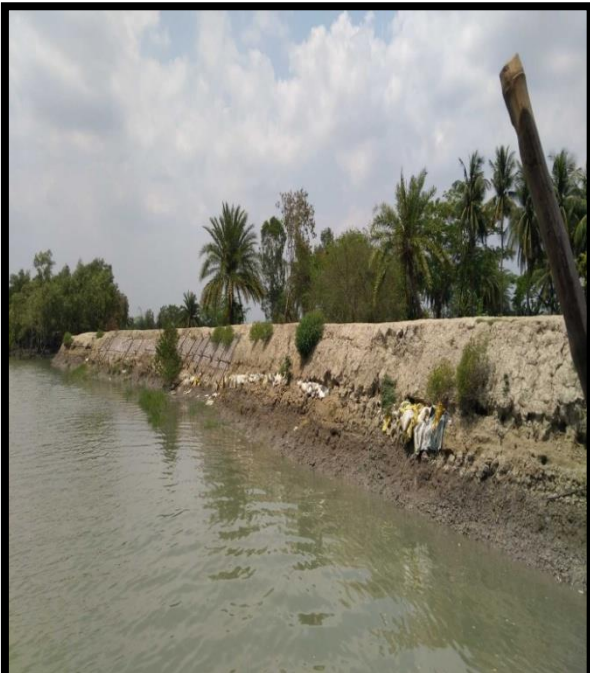
Right River Bank at Chainage 54.5
