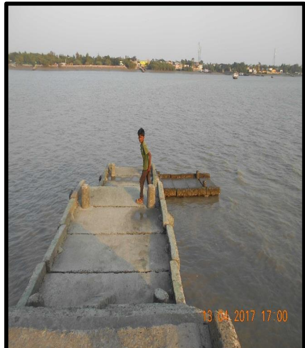
Chandipur Jetty Ghat at Left Bank Chainage 38
