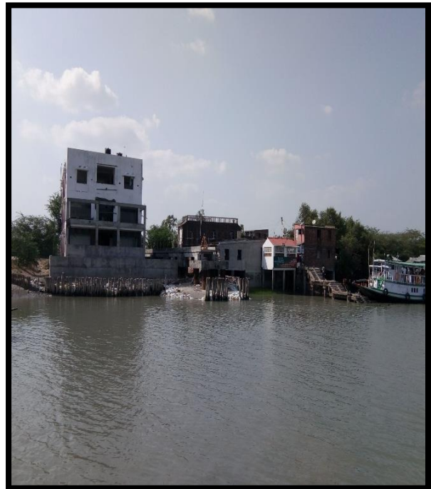
Left River Bank at Chainage 37
