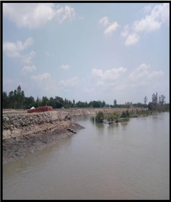
Right River Bank at Chainage 44.5
