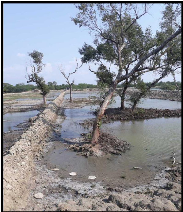
Pond at Right Bank Chainage 33.8
