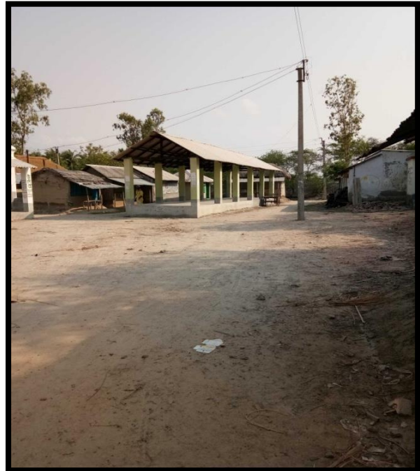
Structure at Right Bank Chainage 52
