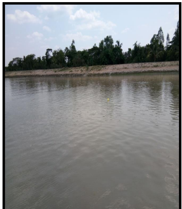
Right River Bank Protection at Chainage 42.2
