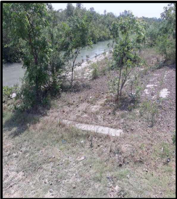
Left River Bank at Chainage 23.2
