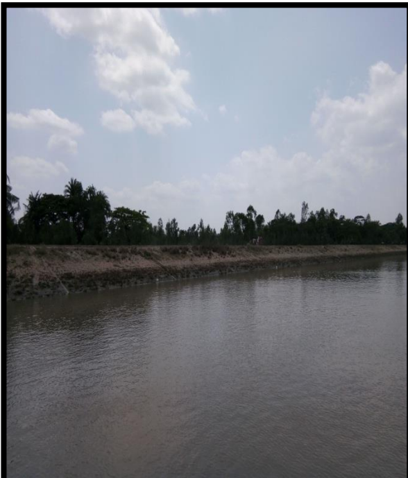
Left River Bank Protection at Chainage 42.5
