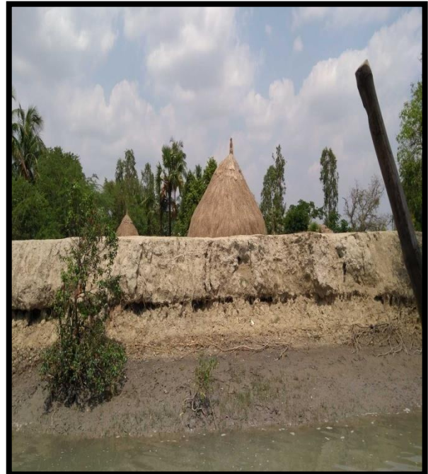
Left River Bank at Chainage 55
