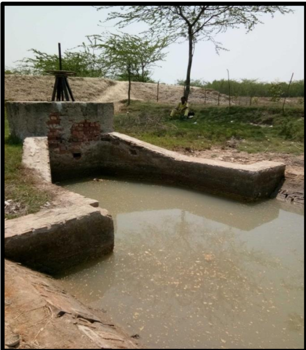
Water Lock at Left Chainage 14
