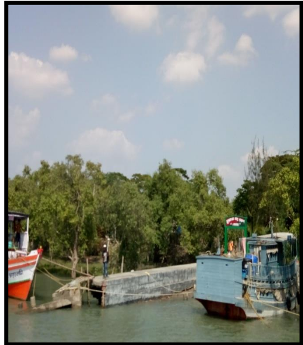
Right River Bank at Chainage 37.8
