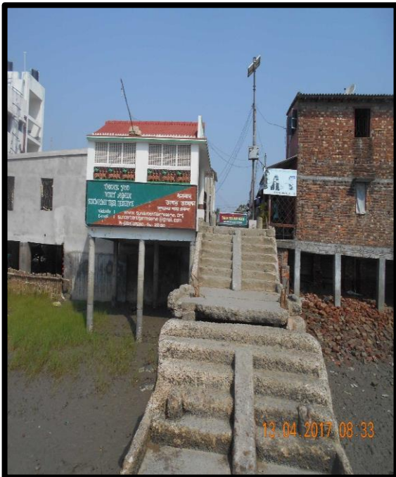
Gadkhali Jetty No. 3 at Left Bank Chainage 37.2
