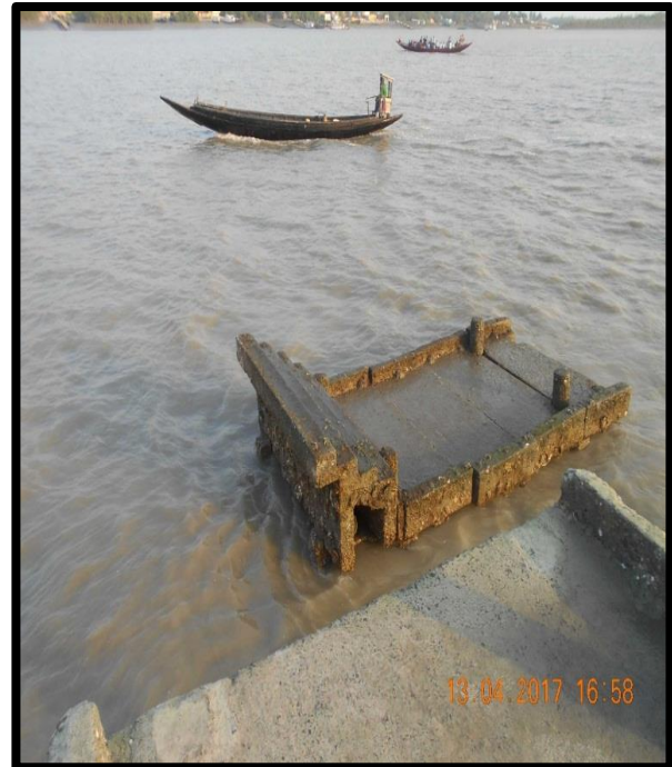
Chandipur Jetty Ghat at Left Bank Chainage 38
