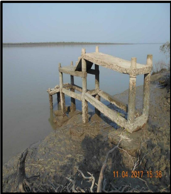
Unused Jetty at Left Bank Chainage 18.3
