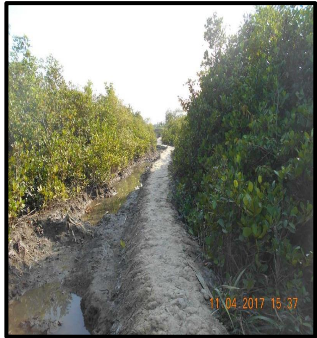
Road For Jetty at Left Bank Chainage 18.3
