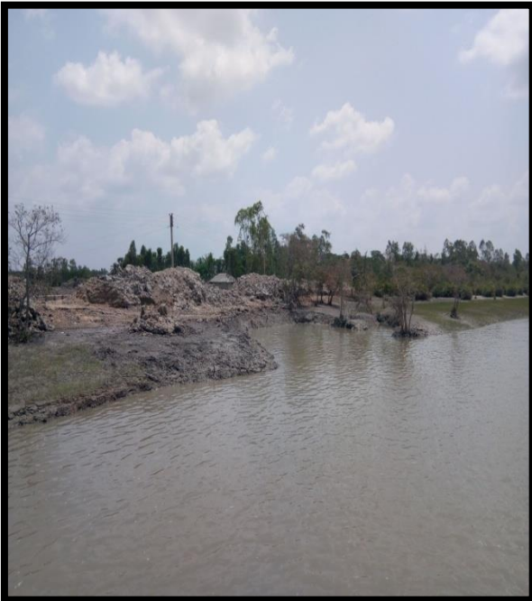
Left River Bank at Chainage 46.1
