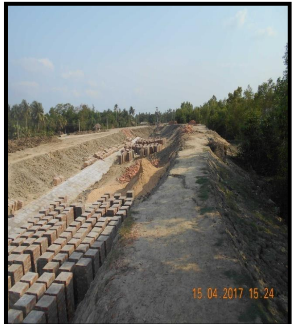
Construction of New Road at Right Bank Chainage 45.4
