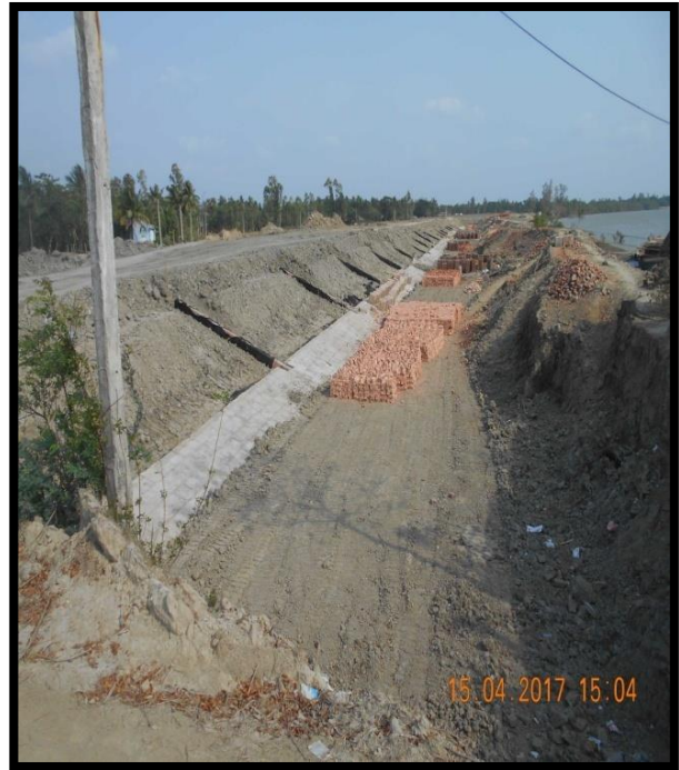
Construction of New Road at Right Bank Chainage 45
