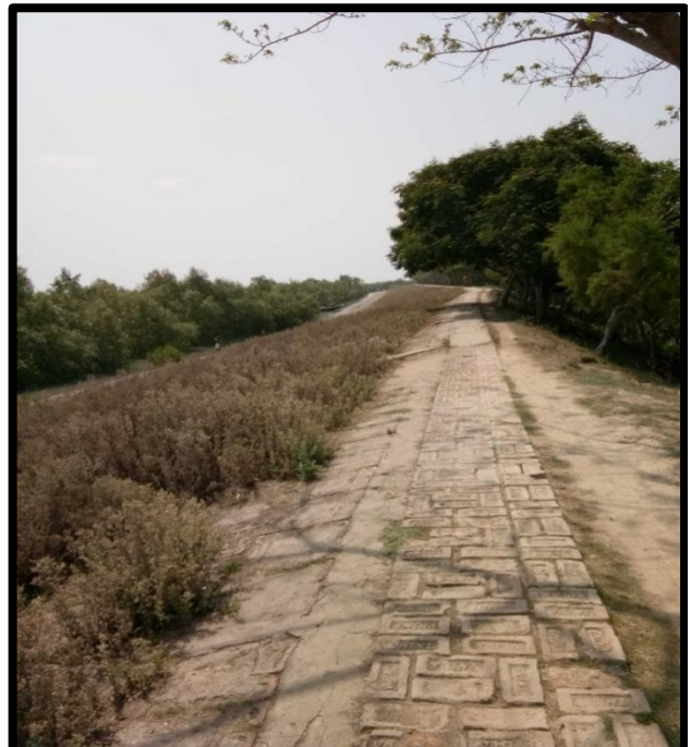
Left River Bank at Chainage 14.5
