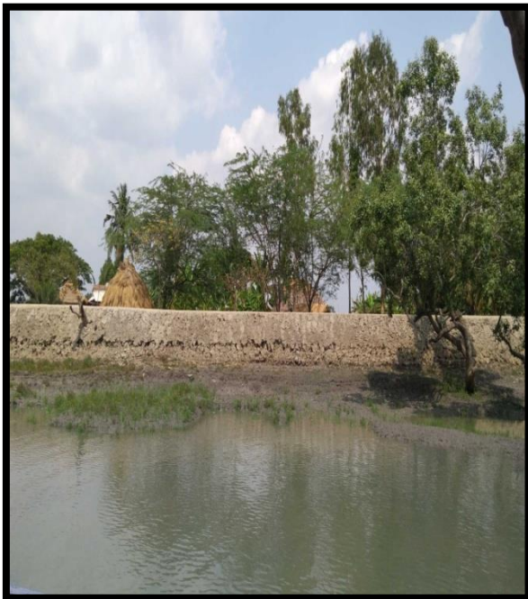
Left River Bank at Chainage 55
