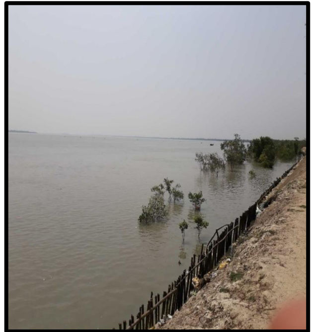
Left River Bank at Chainage 22.6
