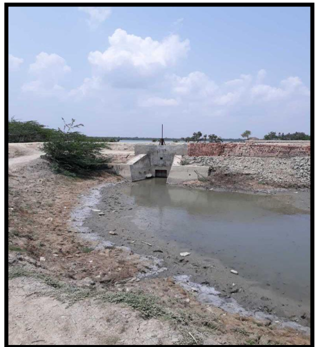
Water Lock at Right Bank Chainage 30.6
