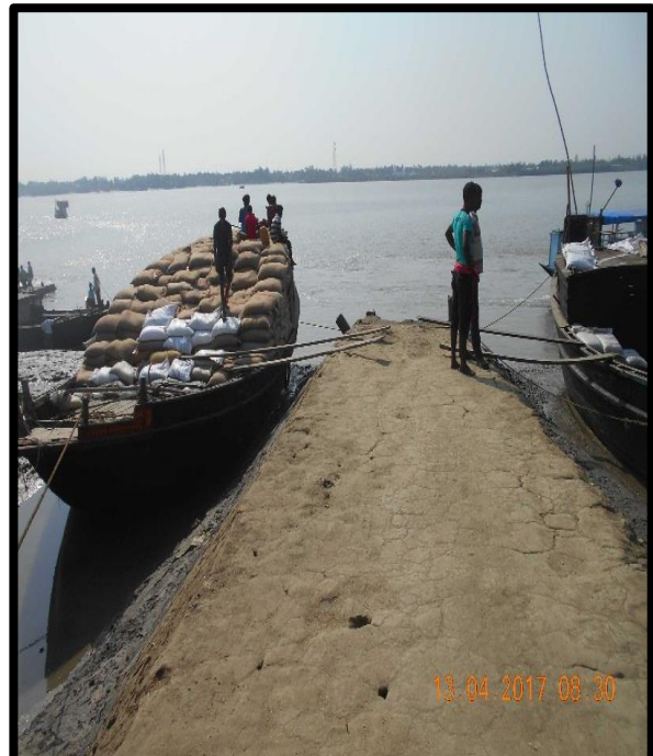
Gadkhali Jetty No.2 at Left Bank Chainage 37.2
