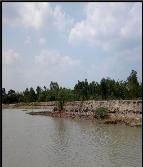
Right River Bank at Chainage 40
