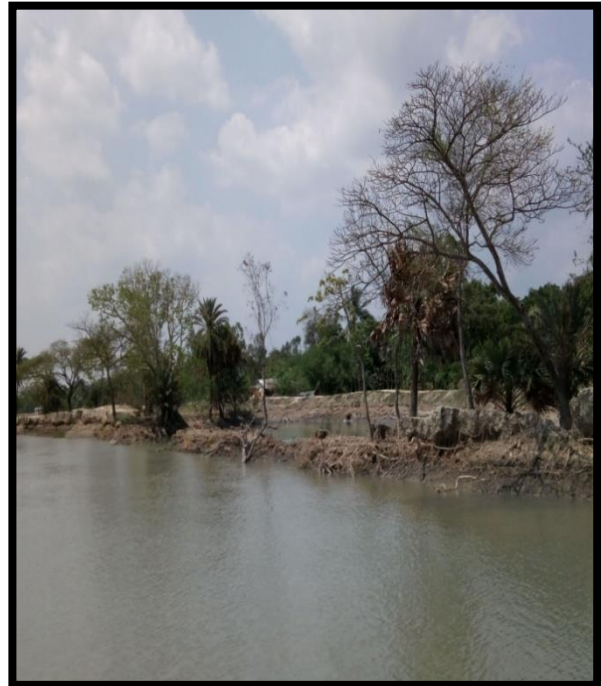
Left River Bank at Chainage 41
