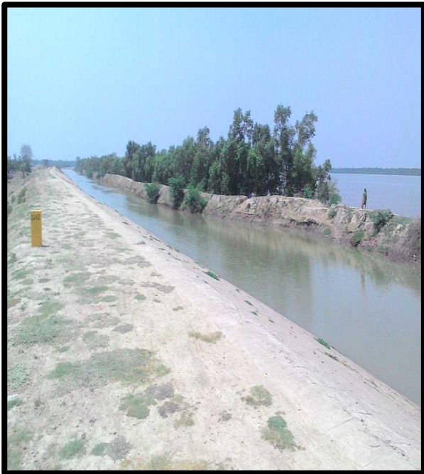
BD-03 inBally Village at Right Bank Chainage 29.7
