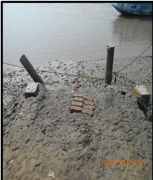
Gadkhali Jetty No.2 at Left Bank Chainage 37.2
