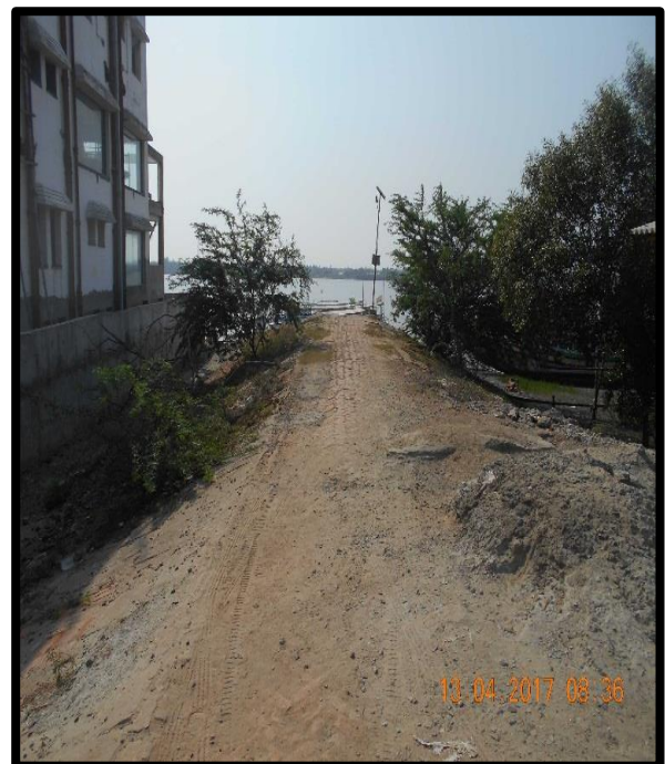
Gadkhali Jetty No.4 at Left Bank Chainage 37.2
