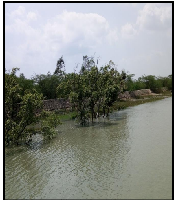
Right River Bank at Chainage 41.5
