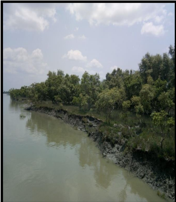
Left River Bank at Chainage 45.3
