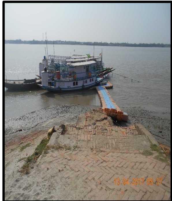
Gadkhali Jetty No. 4 at Left Bank Chainage 37.2
