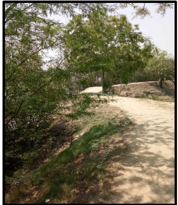
Road at Left Bank Chainage 39.5
