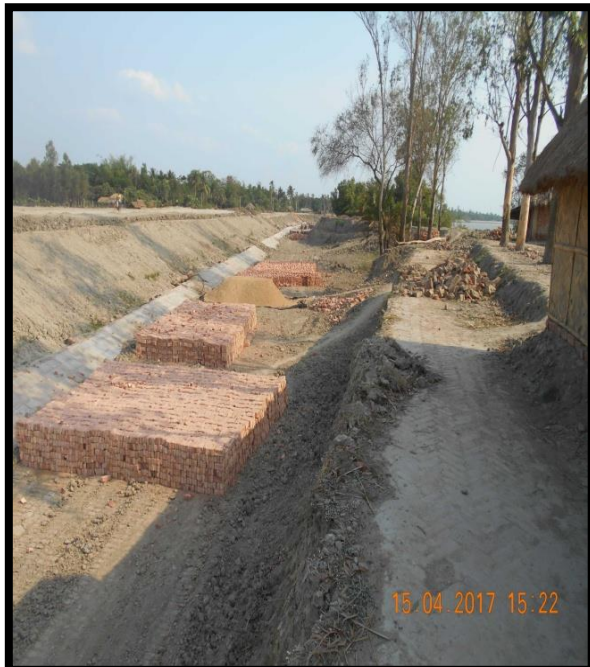
Construction of New Road at Right Bank Chainage 45.3
