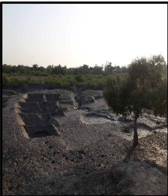
Creek at Left Bank Chainage 31
