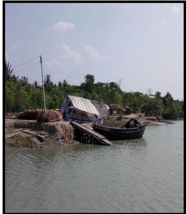
Jetty at Right Bank Chainage 38
