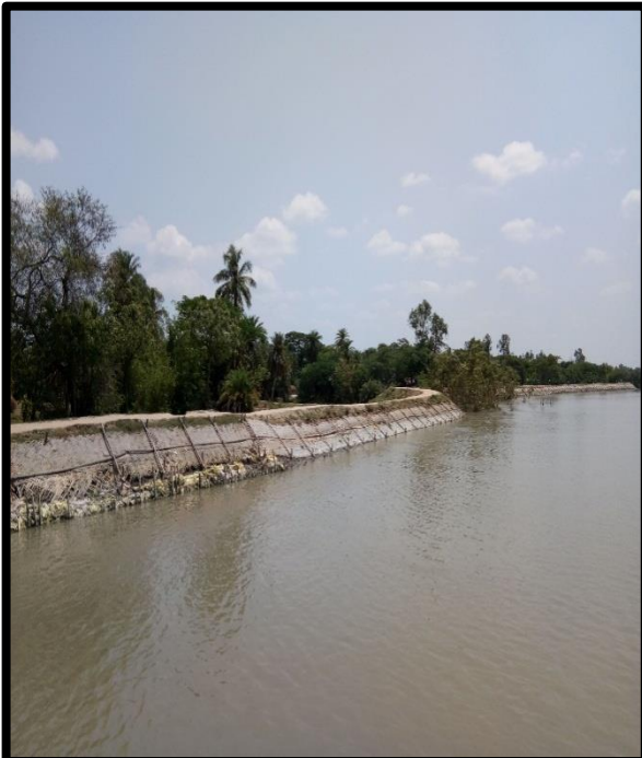
Left River Bank at Chainage 43.7
