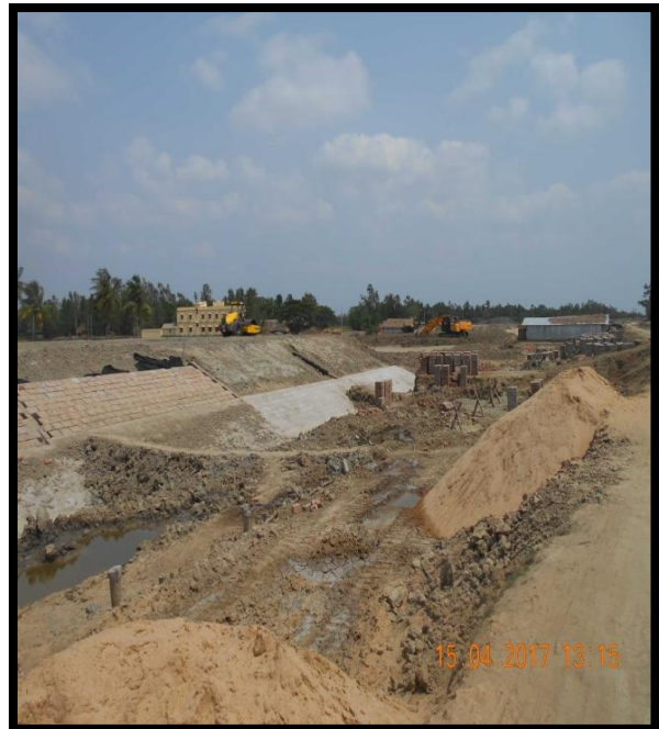
Construction Of New Road at Right Bank Chainage 46.5
