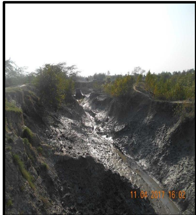
Canal at Left Bank Chainage 18.9
