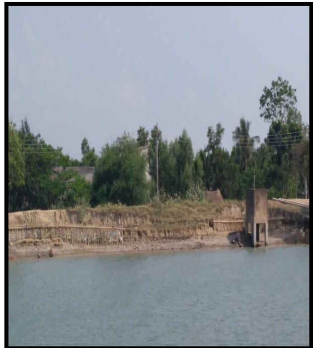
Right River Bank at Chainage 25.5
