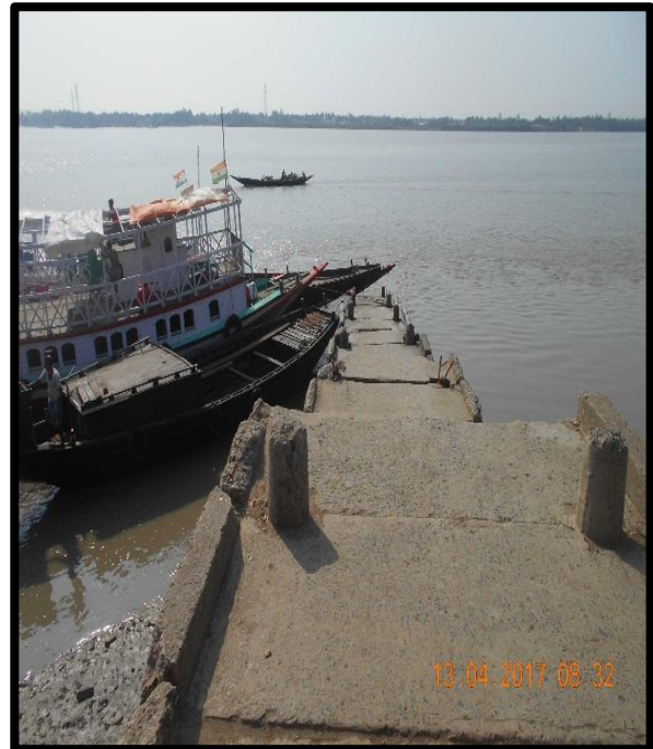
Gadkhali Jetty No. 3 at Left Bank Chainage 37.2
