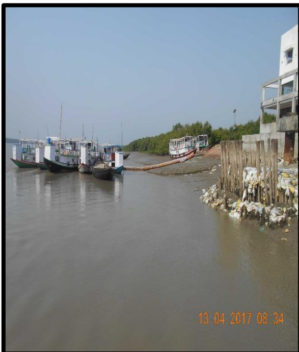
Gadkhali Jetty No.4 at Left Bank Chainage 37.2
