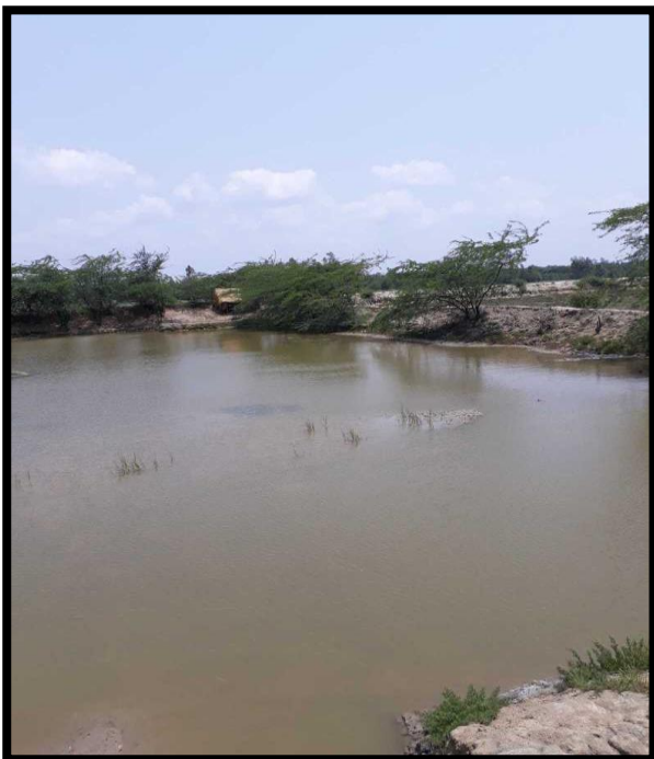
Pond at Right Bank Chainage 30.6
