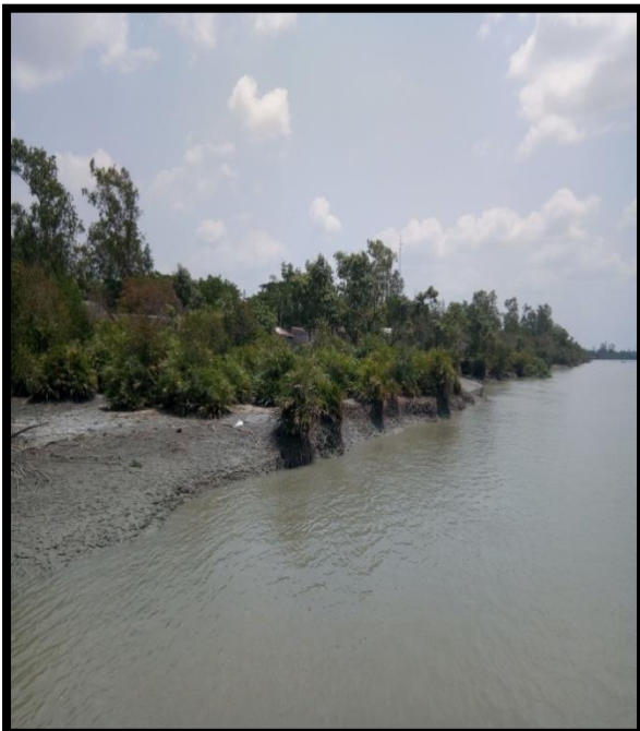
Left River Bank at Chainage 45.4
