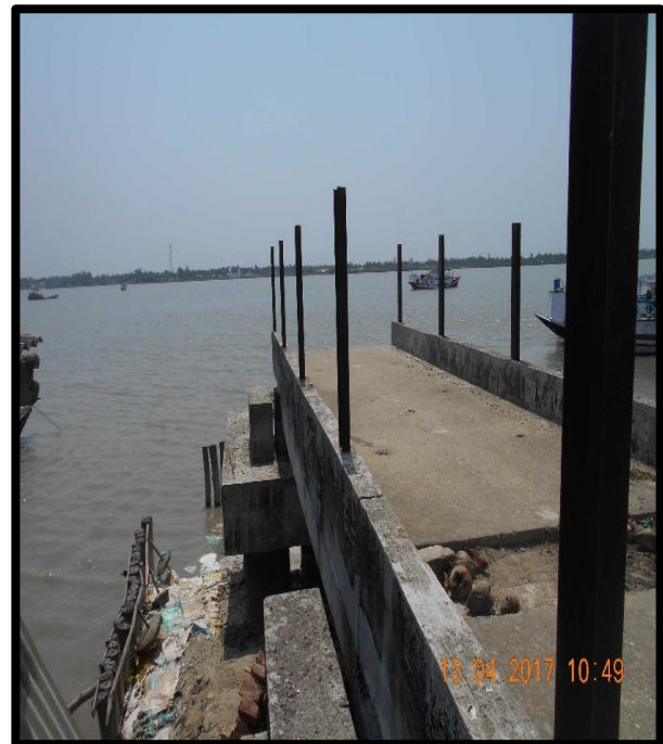
Under Construction Jetty at Left Bank Chainage 37.2
