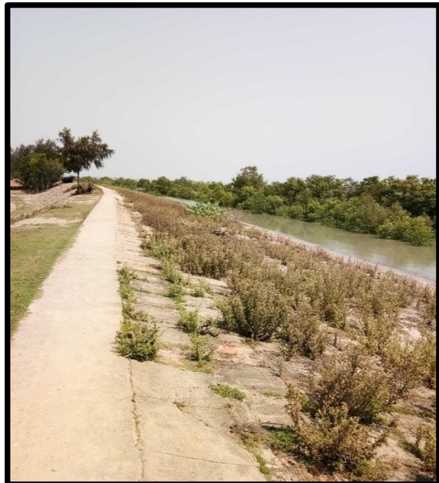
Left River Bank at Chainage 14
