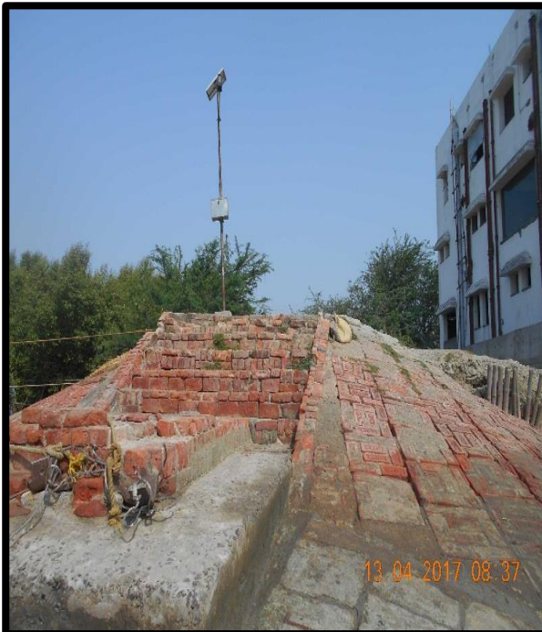
Gadkhali Jetty No.4 at Left Bank Chainage 37.2
