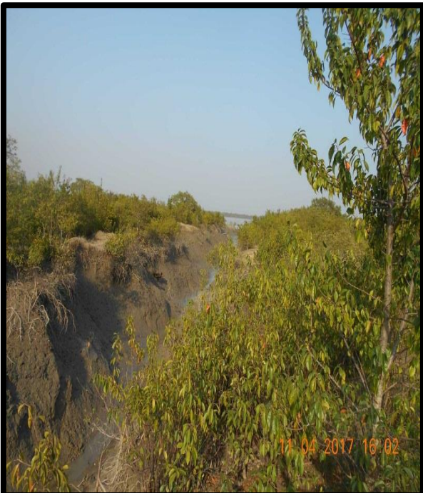
Canal at Left Bank Chainage 18.9
