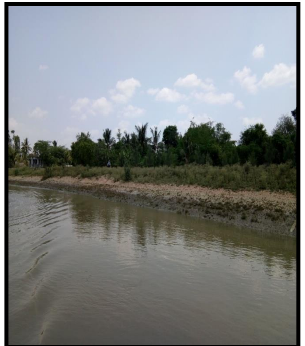
Right River Bank Protection at Chainage 42.5
