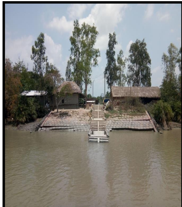
Bagbagan Jetty at Right Bank Chainage 45
