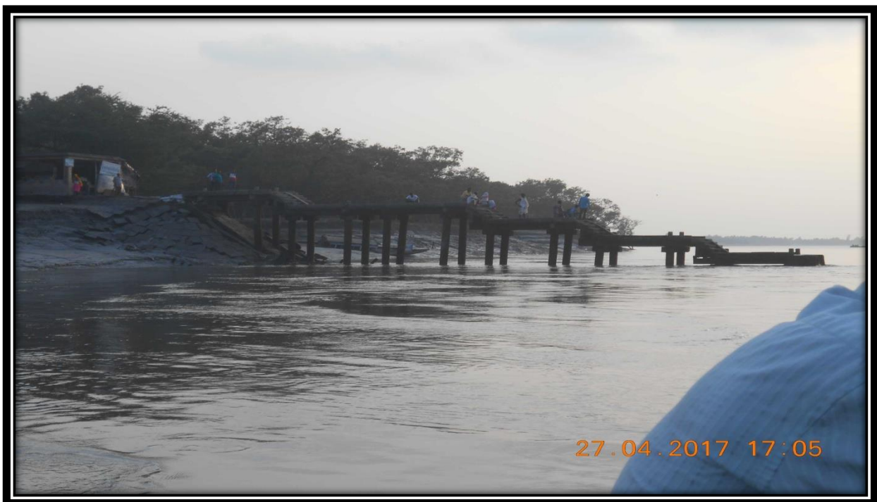
Gazikhali Ghat at Chainage 15.0 on left river bank during low water
