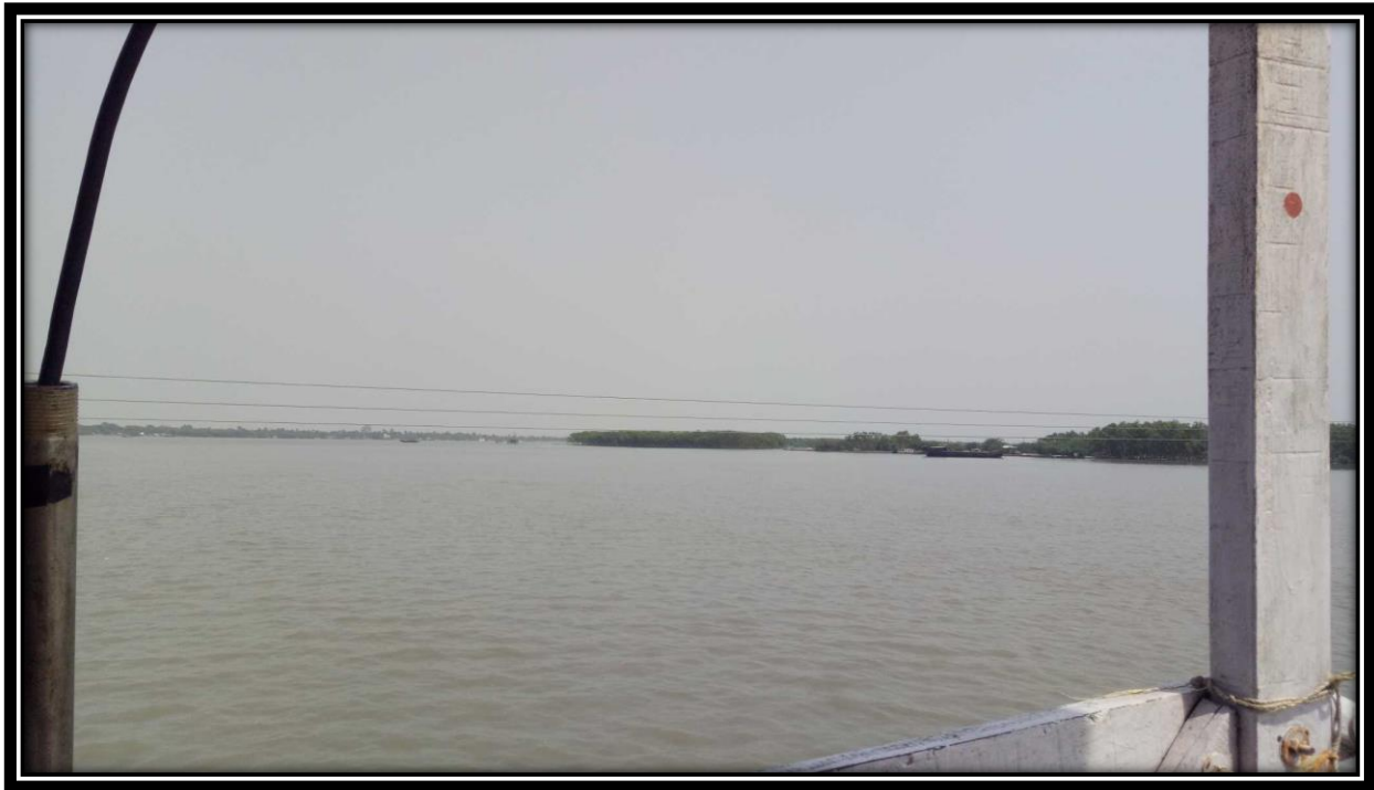
Electric Line Crossing at Chainage 15.0
