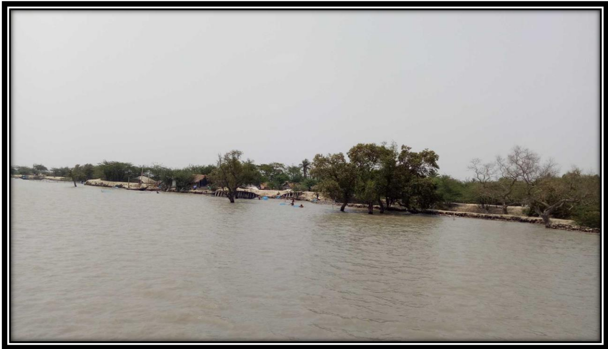
Right Bank Protection at Chainage 5.0
