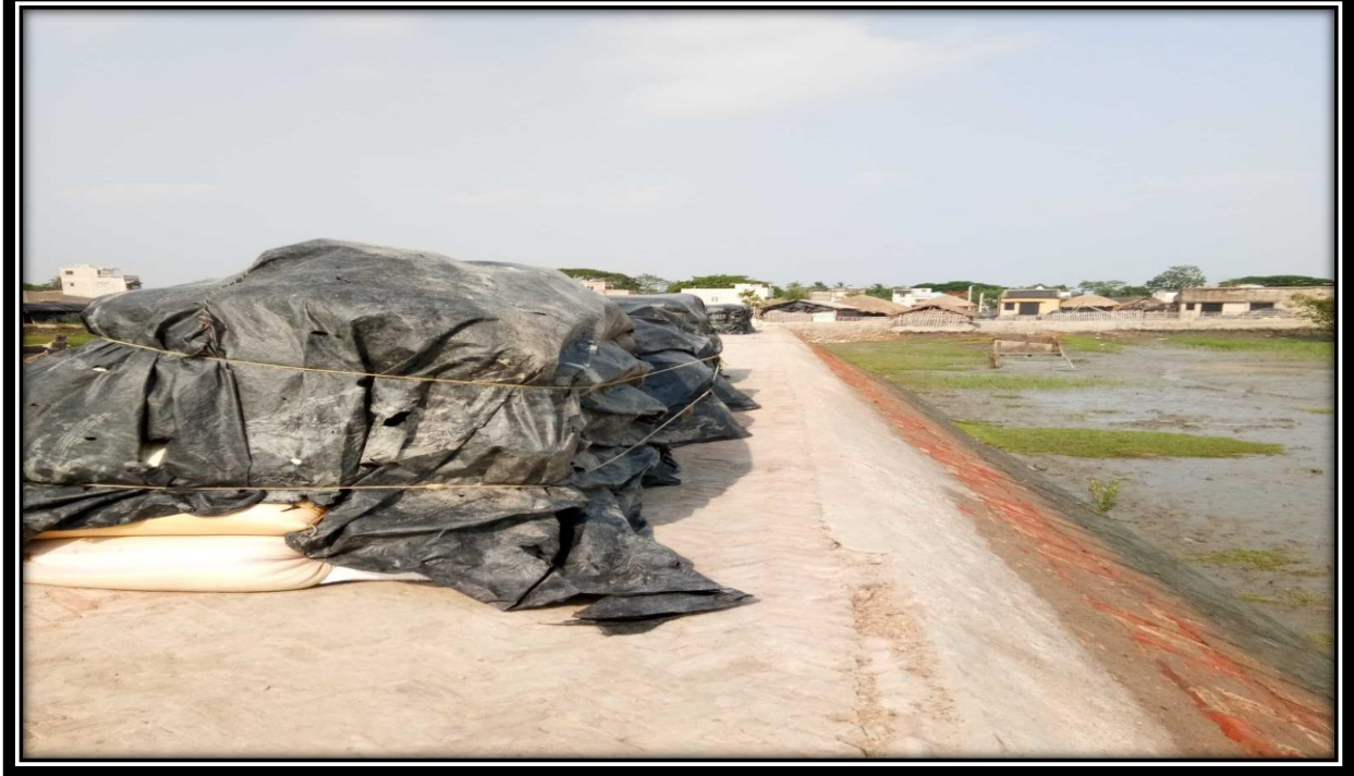
Local Jetty at Chainage 13.5
