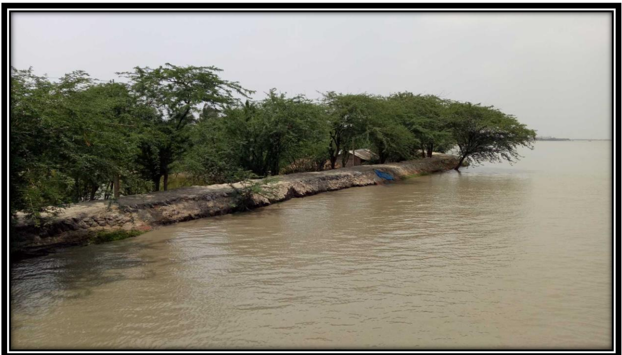
Right Bank View at Chainage 2.5
