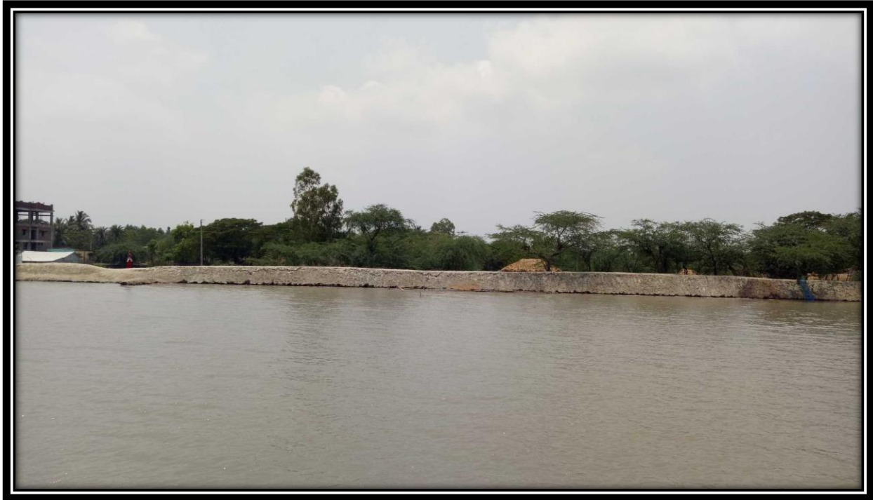
Bank Protection at Chainage 1.5
