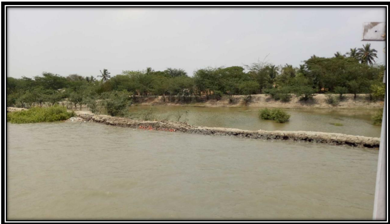
Right Bank Protection at Chainage 4.5
