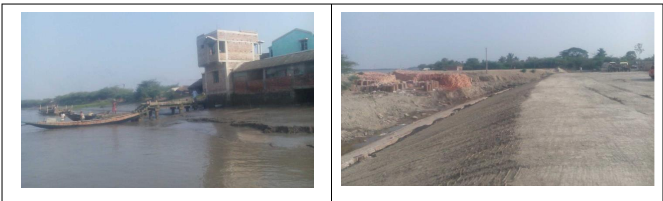
Figure 8: Photographs of Sub-stretch 2
