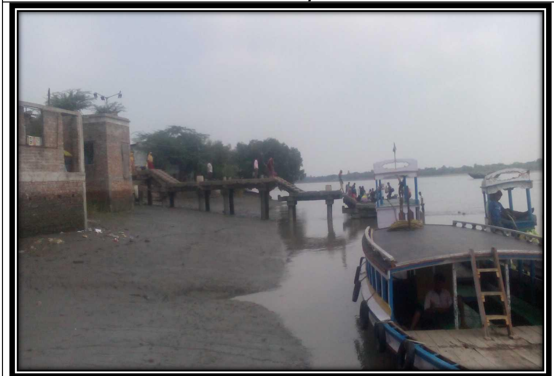
Dhamkhali Ferry Ghat at Chainage 4.0
