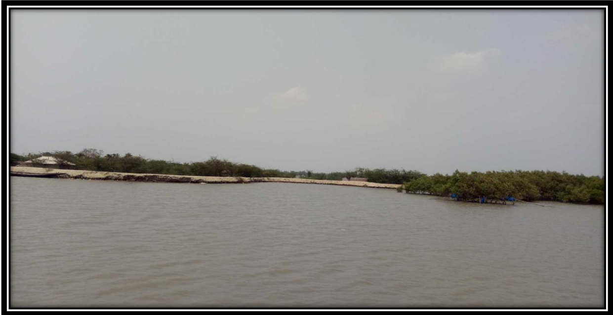
Right Bank Protection at Chainage 6.0
