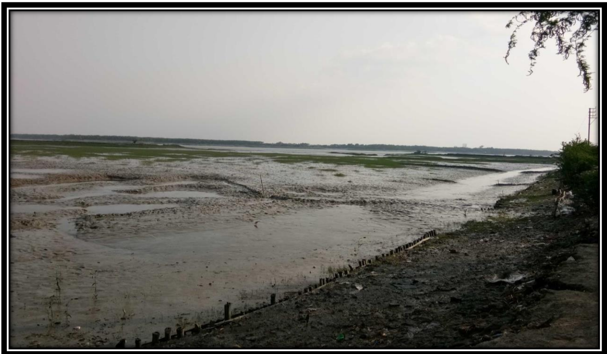
River bank at Chainage 13.9
