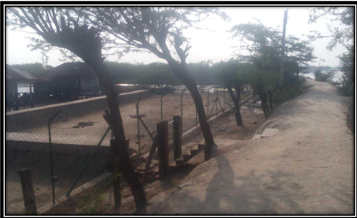
Kaccha Road at Chainage 3.2
