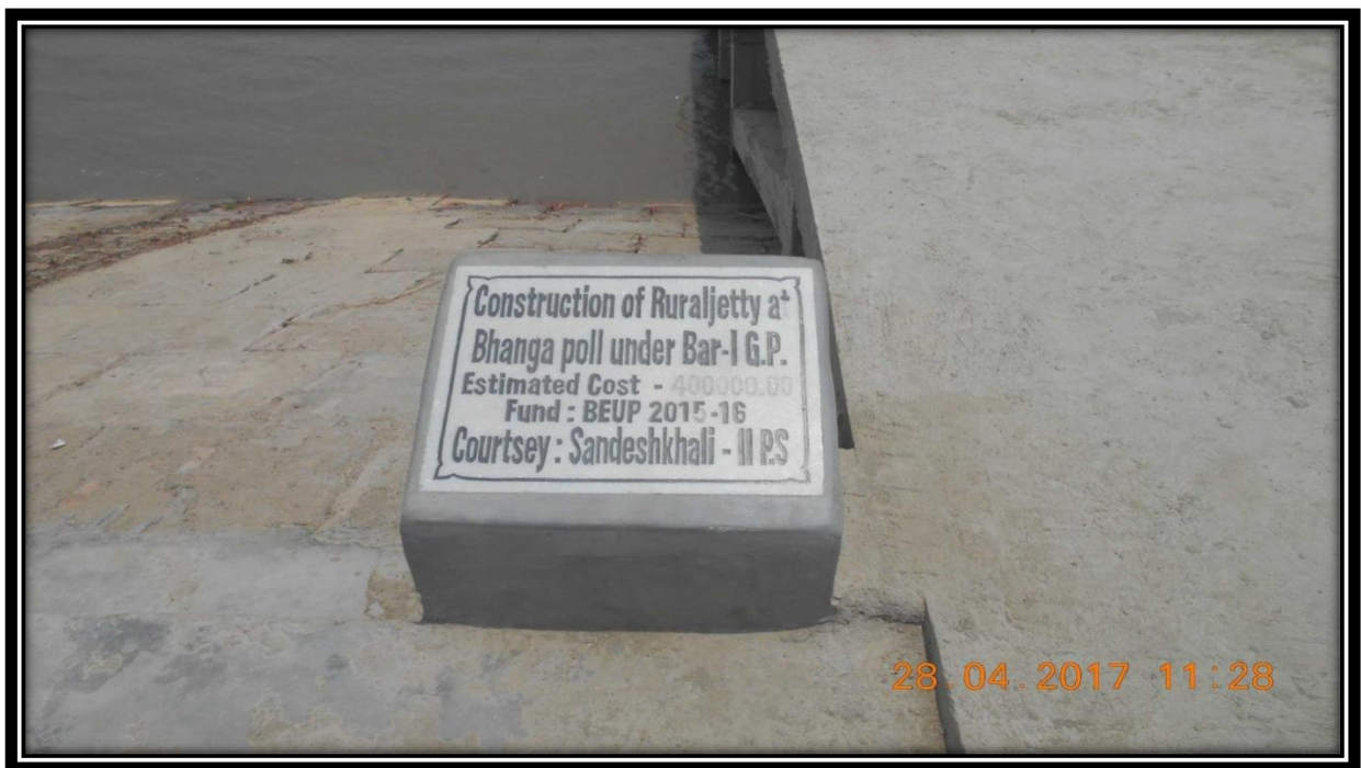
Rural Jetty Under Construction at Chainage 10.3
