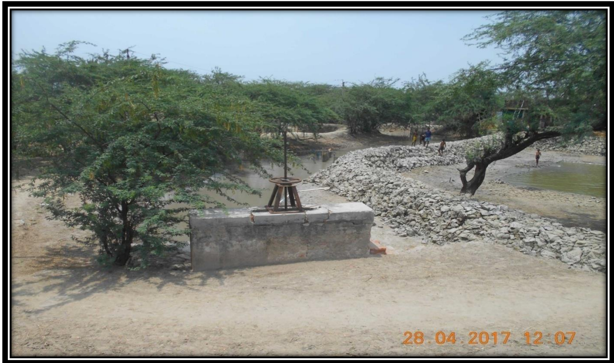
Water Lock gate at Chainage 10.0
