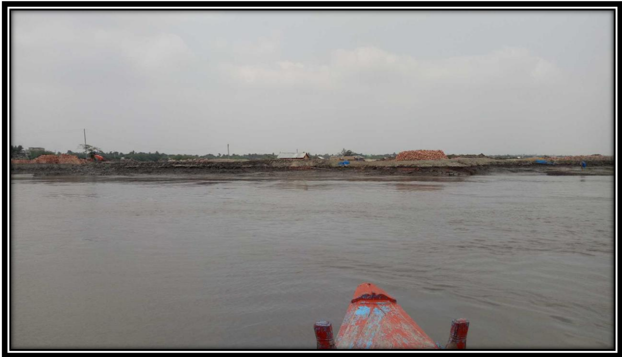
Bank Protection work under Progress at Chainage 7.5
