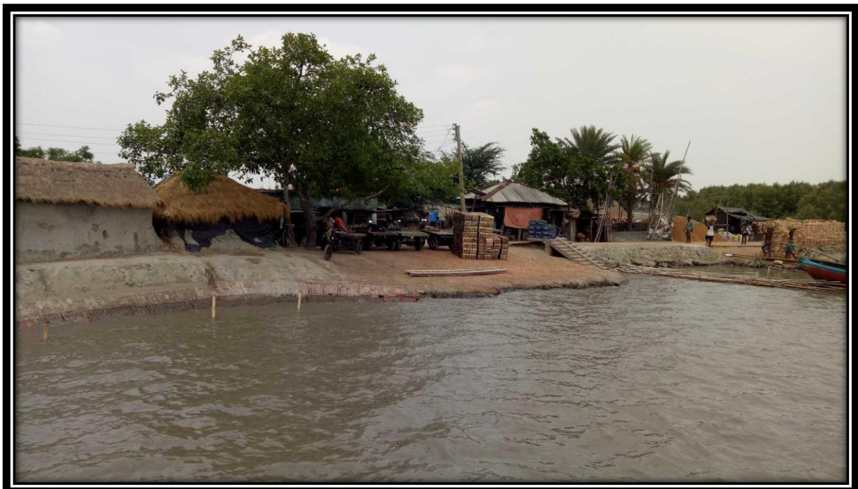
View of Bank Protection of Left bank and Village at Chainage 0.02
