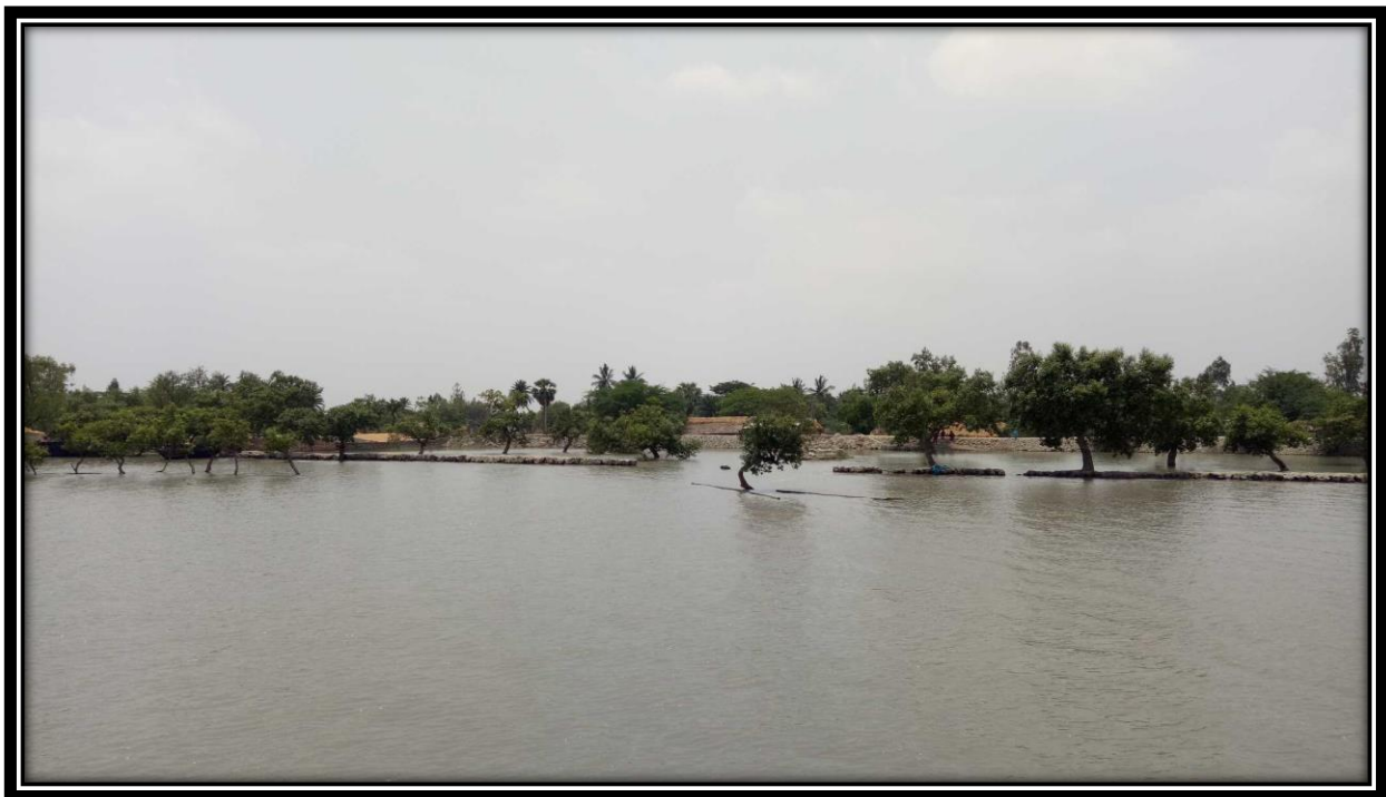
Bank Protection at Chainage 1.0
