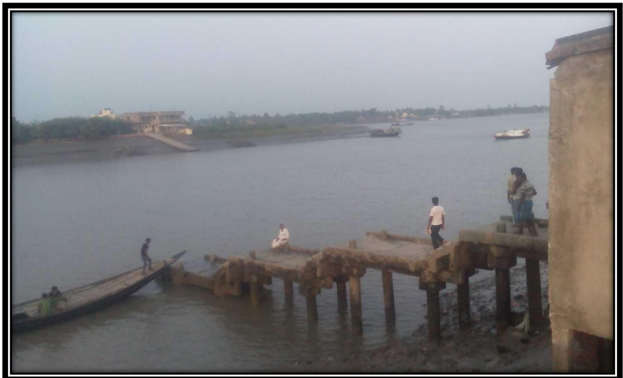
Bihangatushkhali Ferry Ghat at Chainage 3.6
