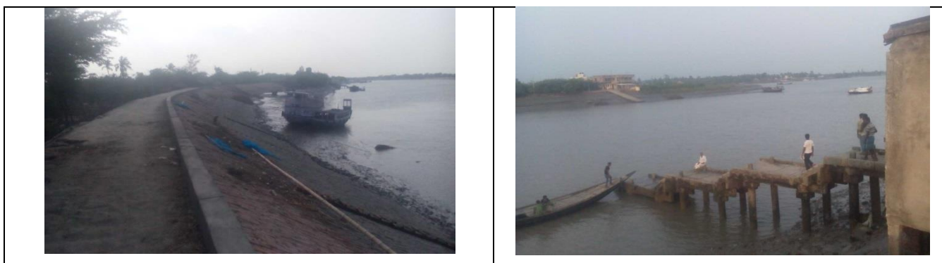
Figure 5: Photographs of Sub-Stretch 1
