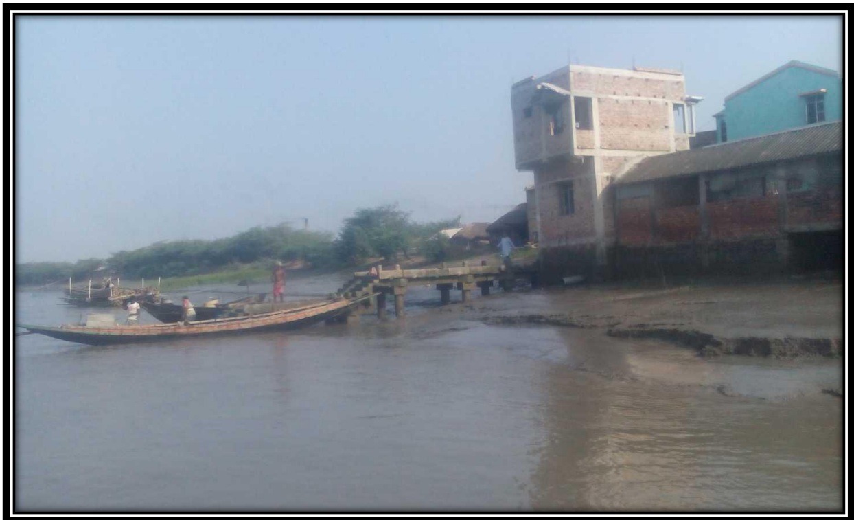
2 nd Jetty at Arsadmiya Ghat at Chainage 6.2
