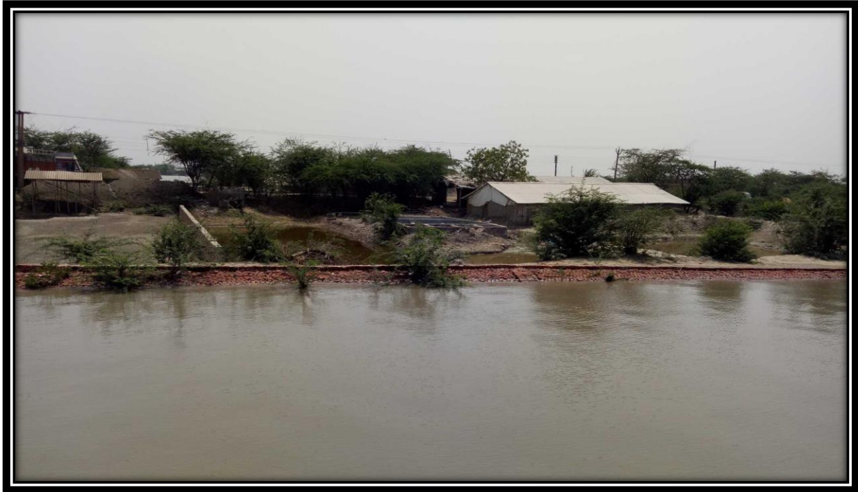
Left Bank Protection at Chainage 5.0
