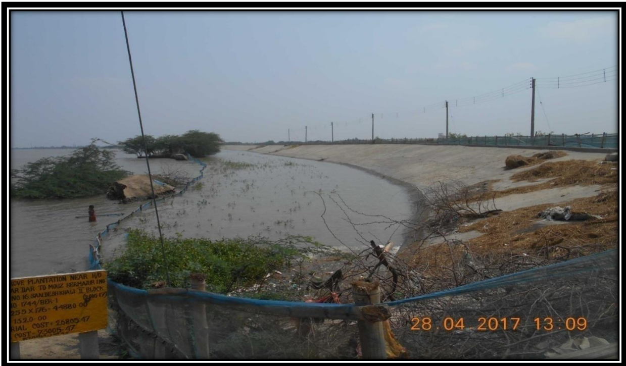
River Bank Protection at Chainage 8.8
