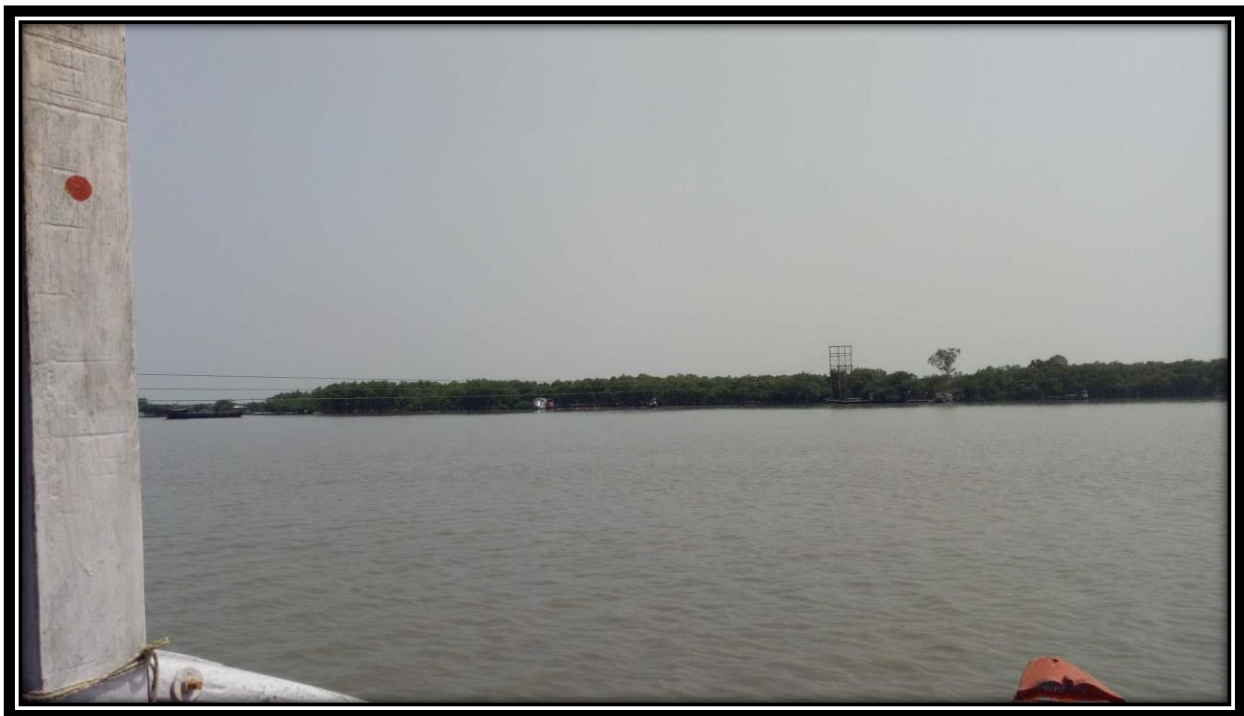
Electric Tower on Right Bank at Chainage 15.0
