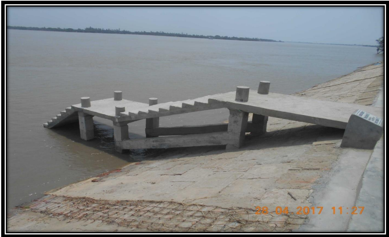
Rural Jetty Under Construction at Chainage 10.3
