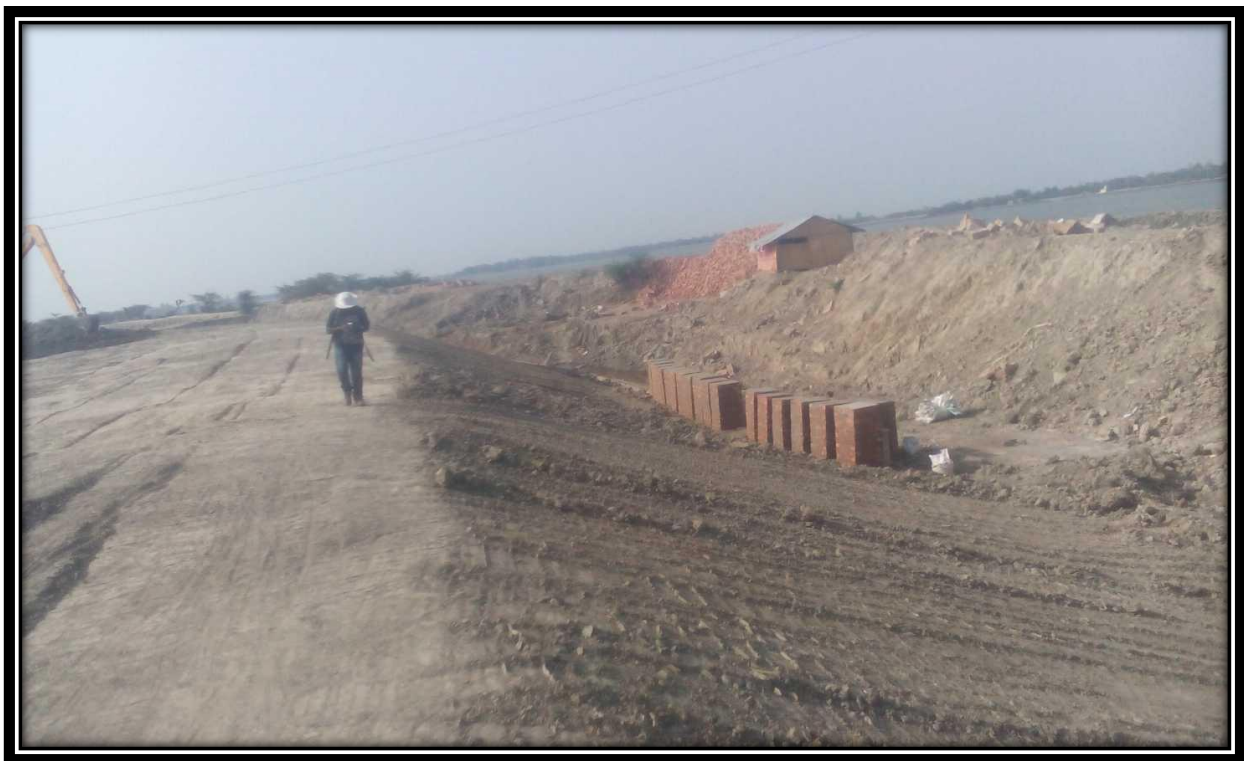
River Bank Protection work on right bank at Chainage 7.1
