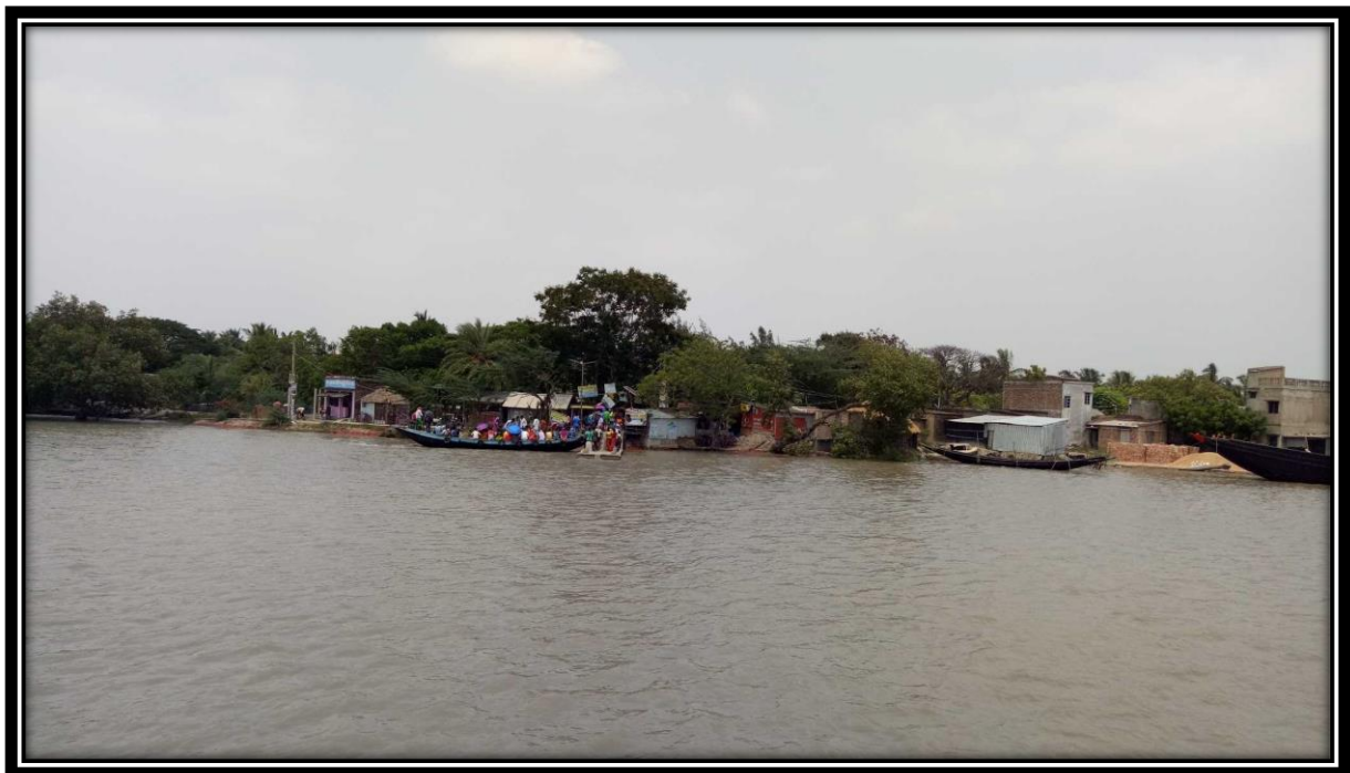
Dhamkhali Ferry Ghat at Chainage 4.0
