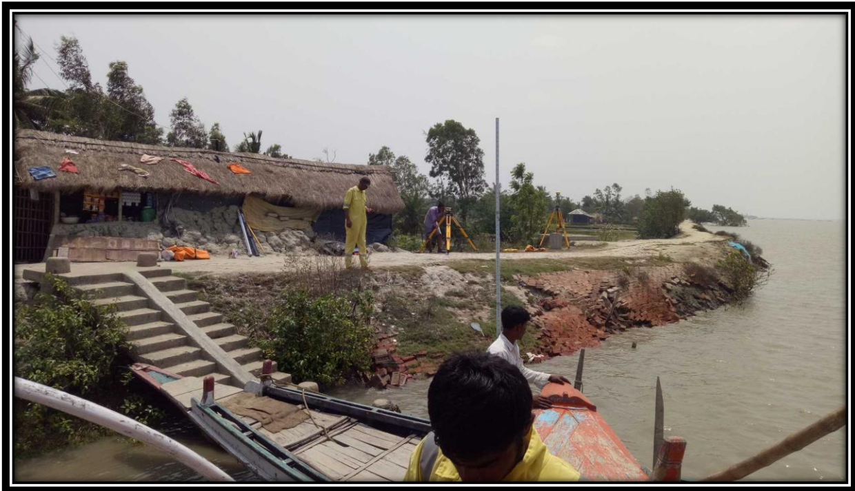
View at Right bank Chainage 0.03 – Carrying out Levelling, DGPS Observation
