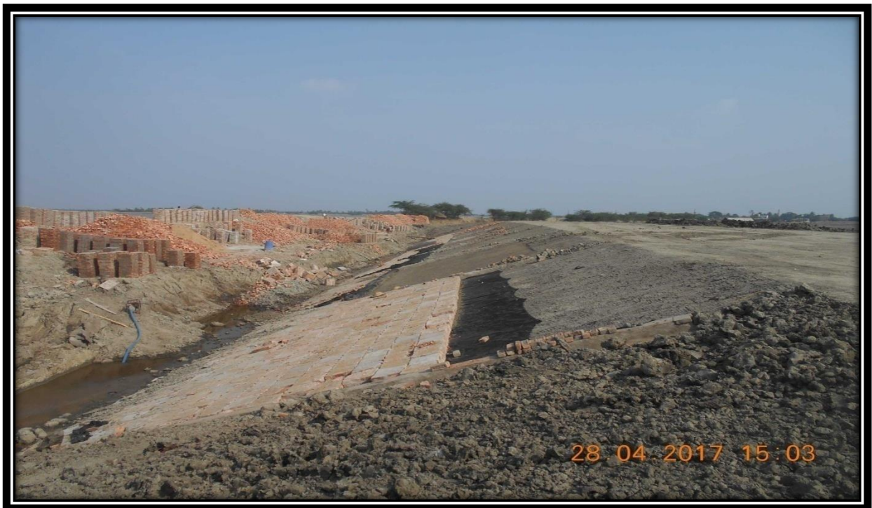
Bank Protection work under Progress at Chainage 7.4
