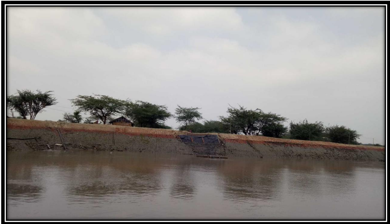
Protected Bank Chainage 6.5
