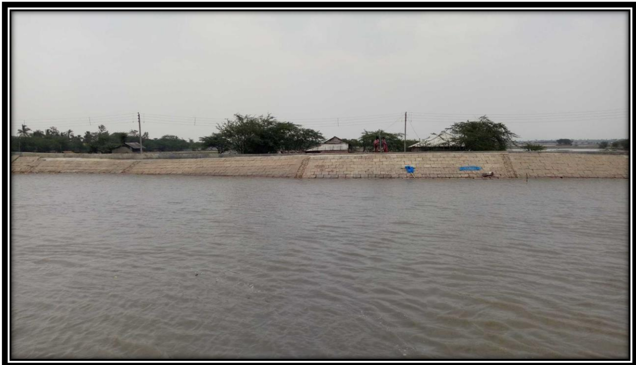
Protected Bank at Chainage 9.5
