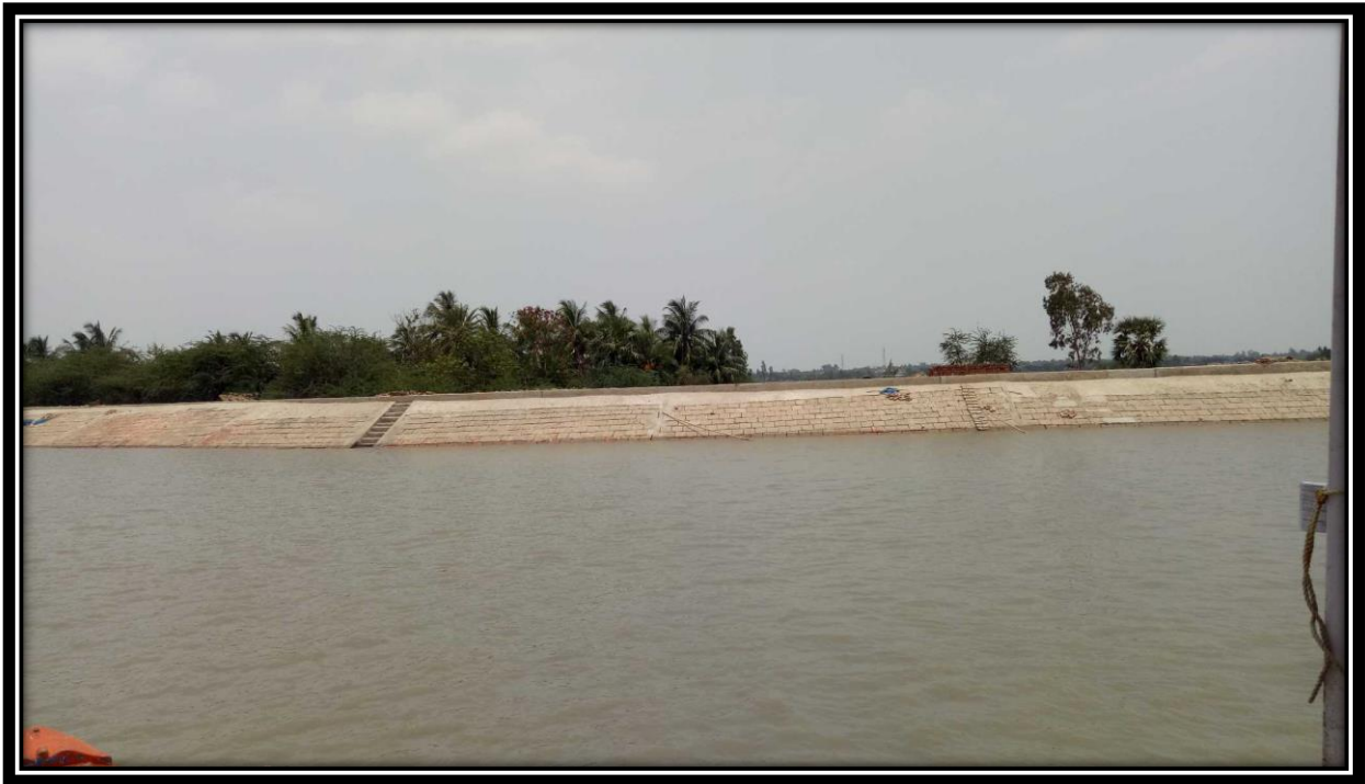
Right Bank Protection at Chainage 2.0
