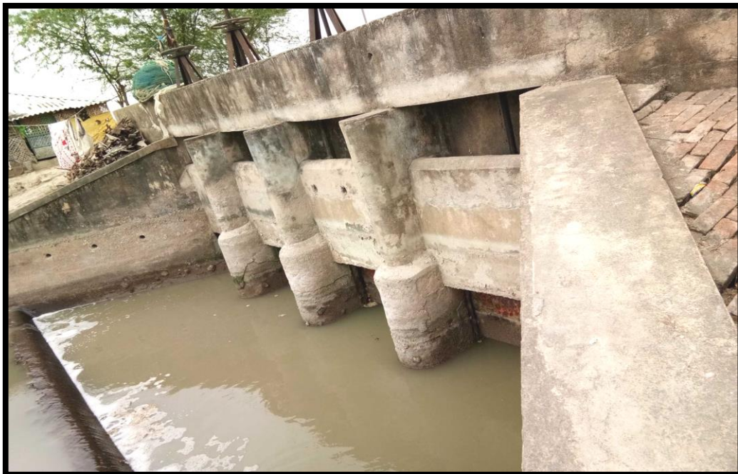
Water lock at chainage 4.5
