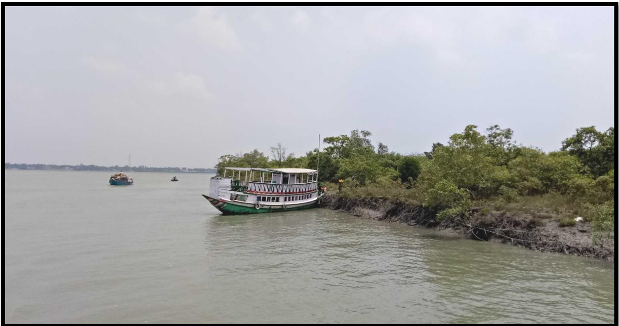
Unprotected Left Bank at Chainage 1.0
