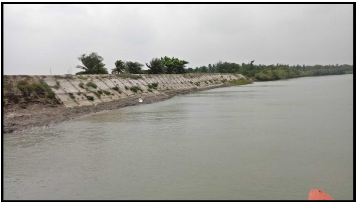
View of Right bank at Chainage 3.0
