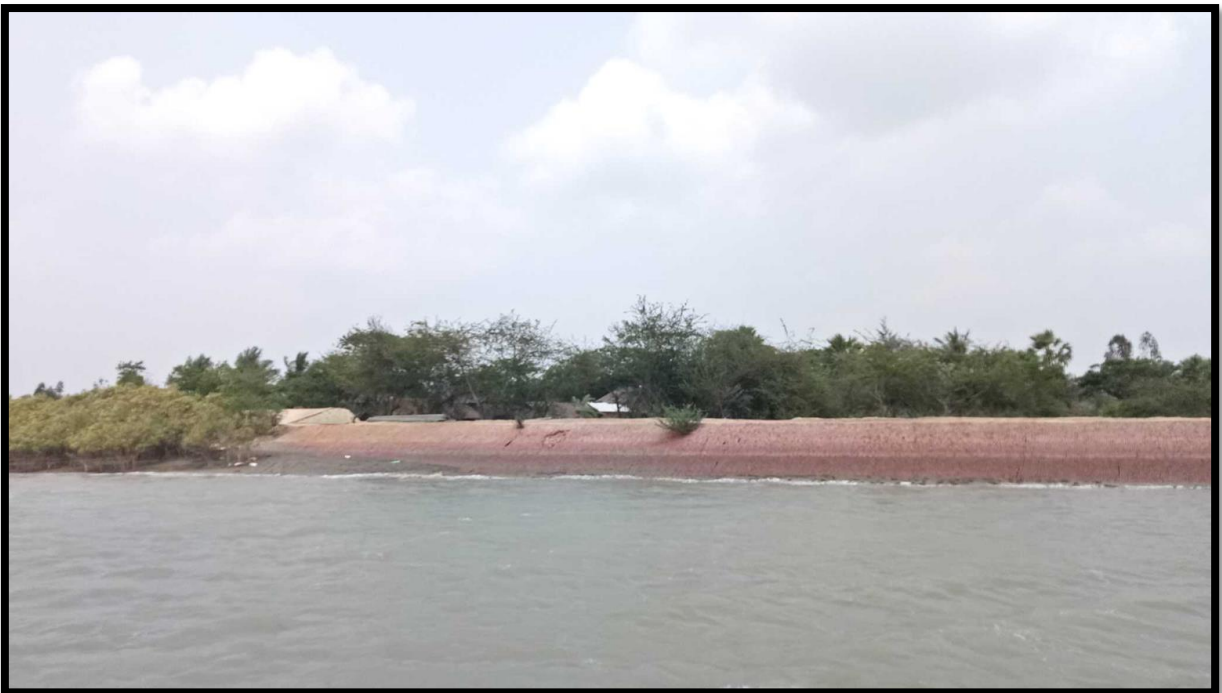
Protected Right Bank at Chainage 0.5
