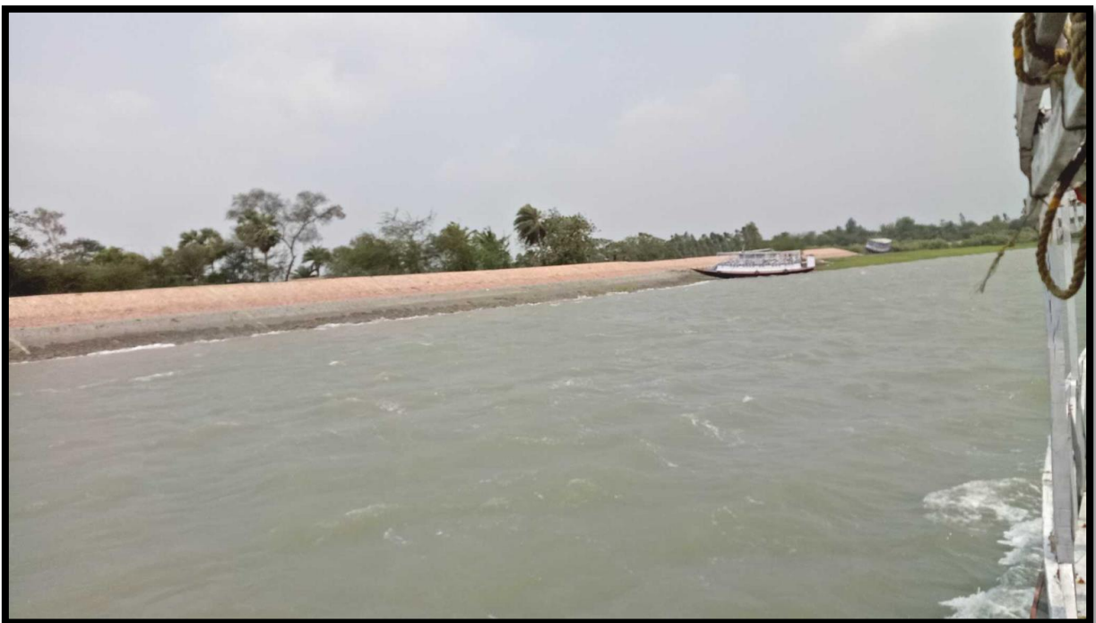
Protected Right Bank at Chainage 1.5
