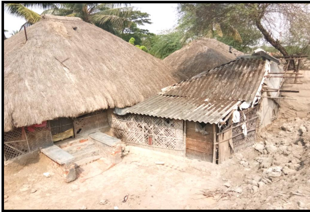
Hutments at chainage 5.7
