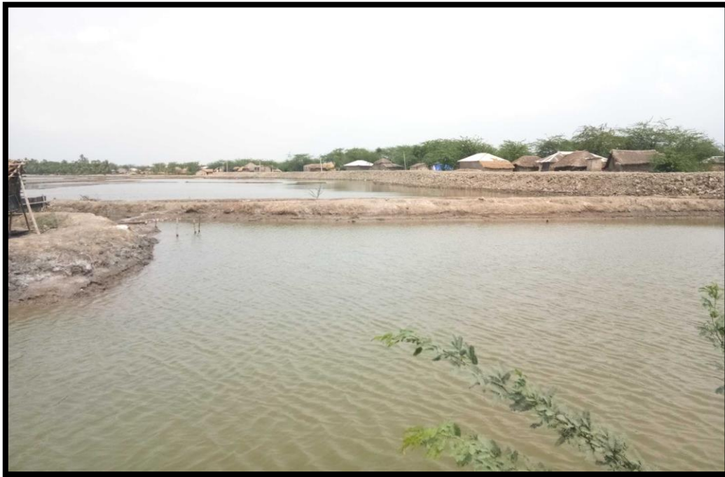
Pond along the river bank at chainage 5.0
