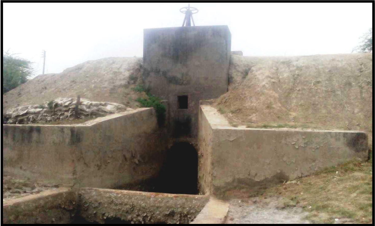
Water lock at chainage 5.8
