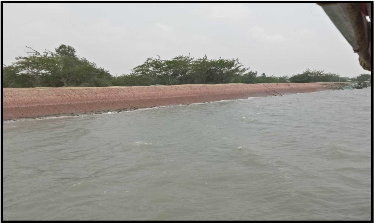
Protected Right Bank at Chainage 1.0
