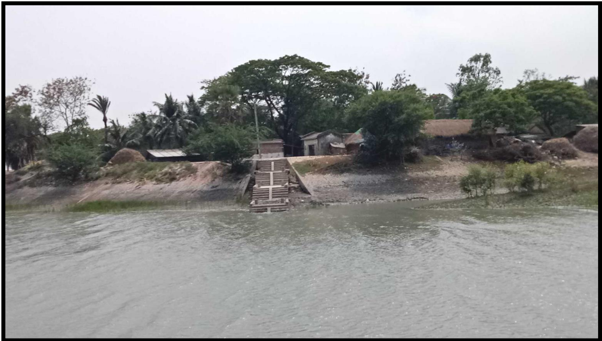
Ferry Jetty at Chainage 4.0
