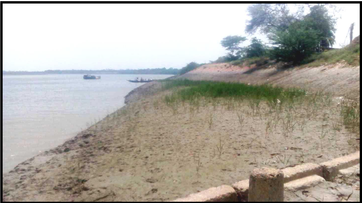
River bank at Chainage 3.6
