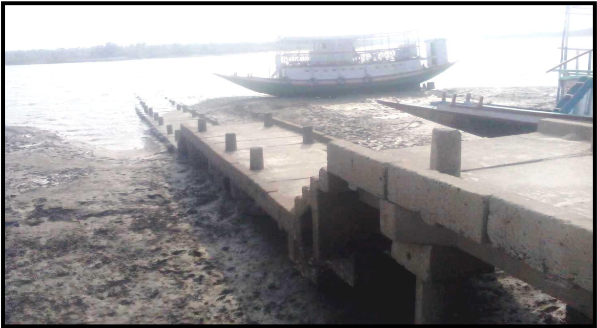
Jetty at Chandipur Chainage 4.2
