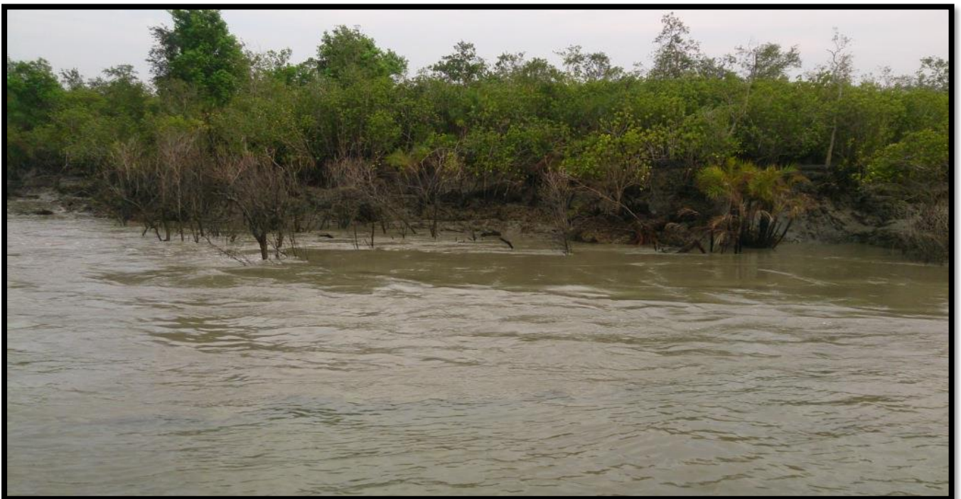
Unprotected Left Bank at CHAINAGE 13.5
