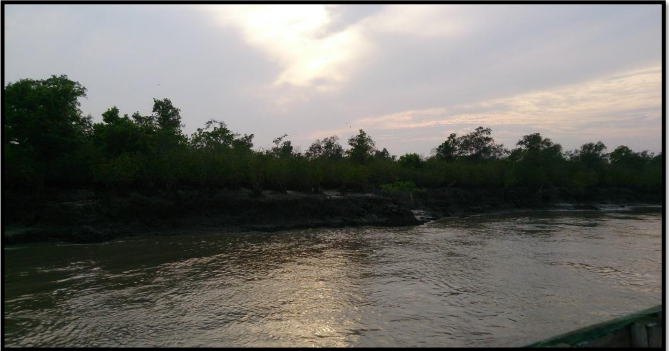
Unprotected Left Bank at CHAINAGE 11.8
