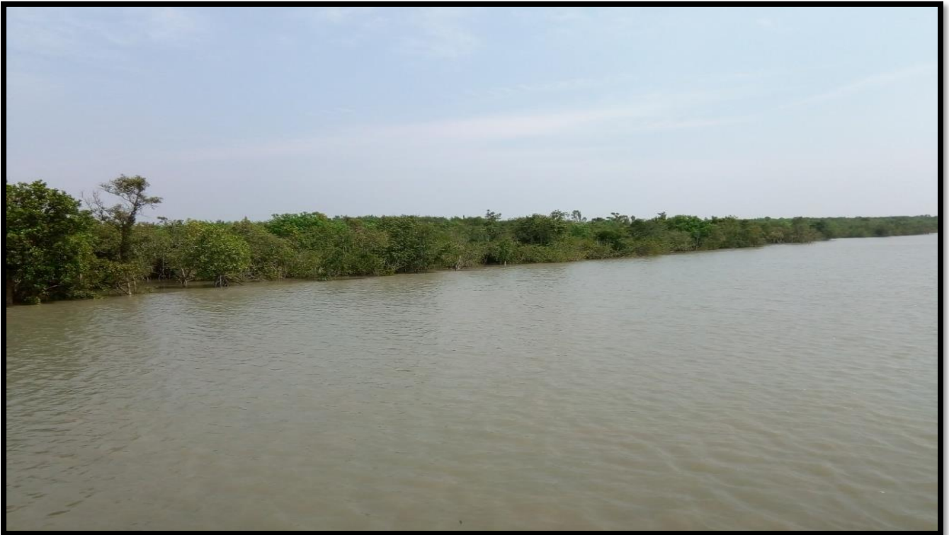
Unprotected Left Bank at CHAINAGE 15.827
