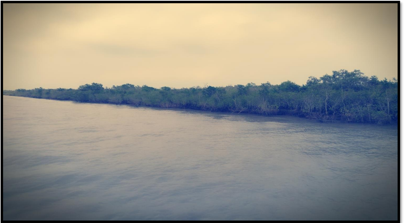
Unprotected Right Bank at CHAINAGE 13.5
