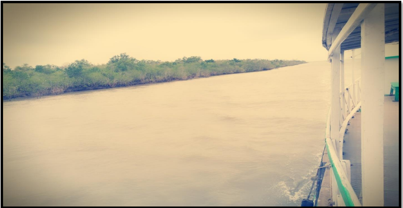
Unprotected Right Bank at CHAINAGE 7.5
