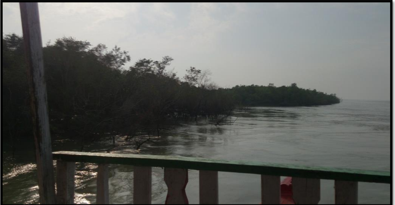
Unprotected Left Bank at CHAINAGE 12.8
