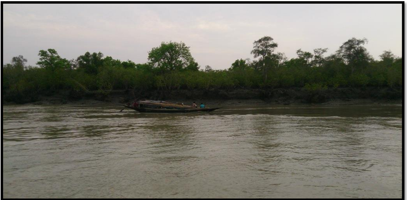
Unprotected Right Bank at Chainage 3.7
