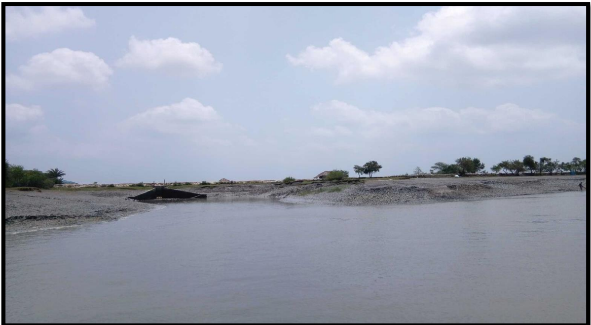
Lock gate on Right Bank at Chainage 4.0
