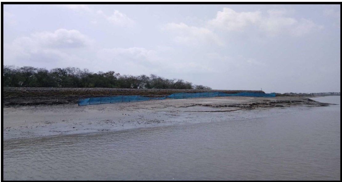
Bank Protection at Chainage 7.6
