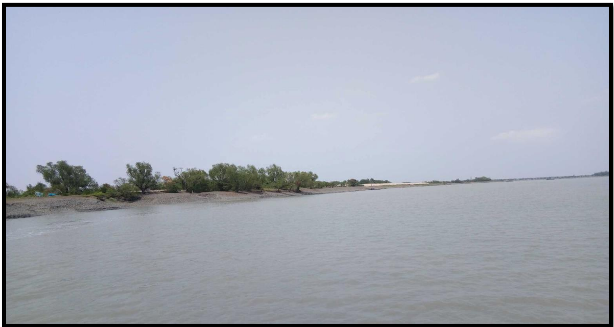
Bank Condition at Chainage 3.4
