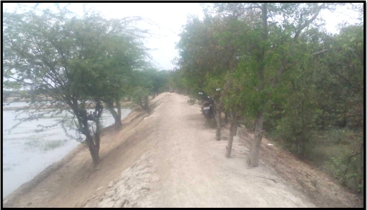
River Bank at Chainage 3.6
