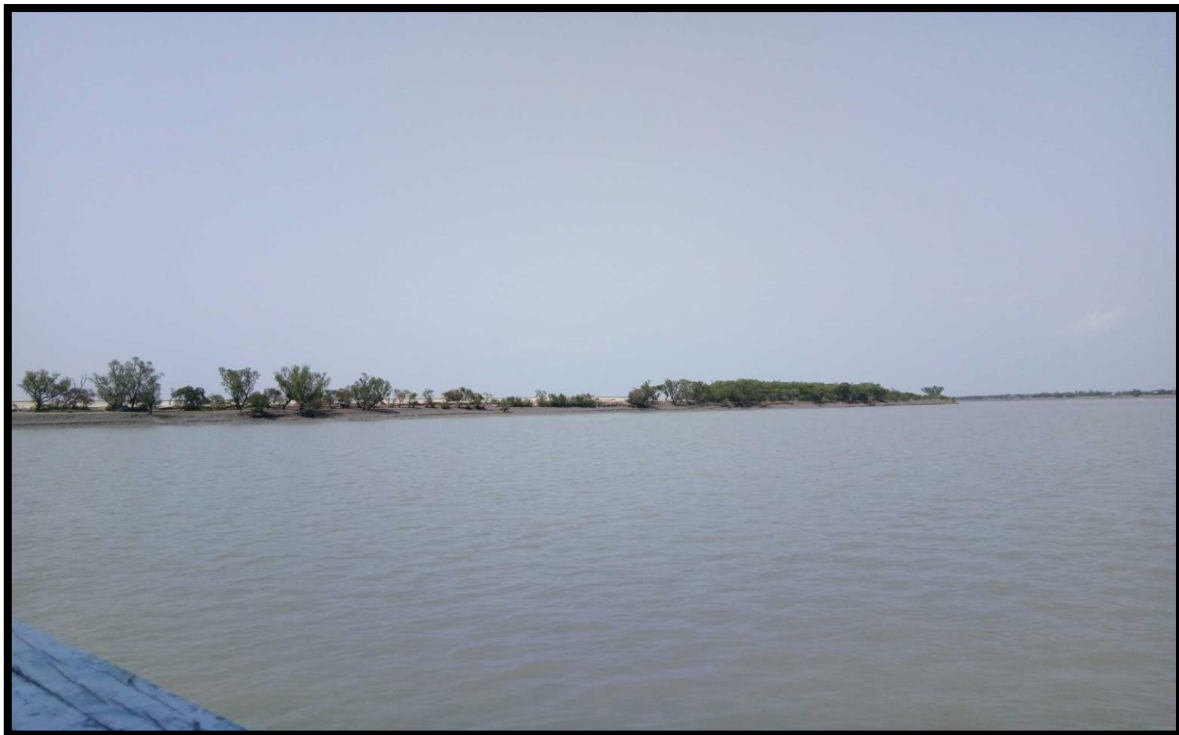
Unprotected Left bank at chainage 1.0
