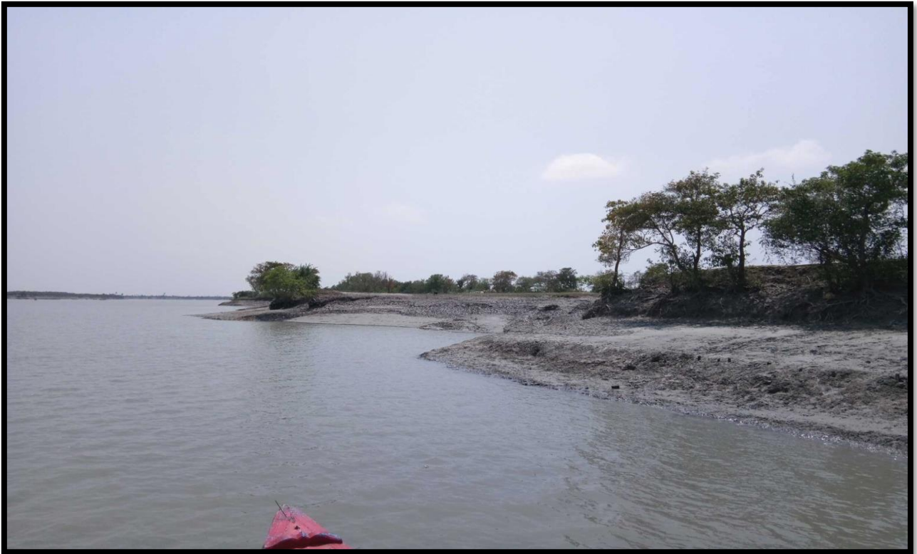
Unprotected Left bank at chainage 2.5
