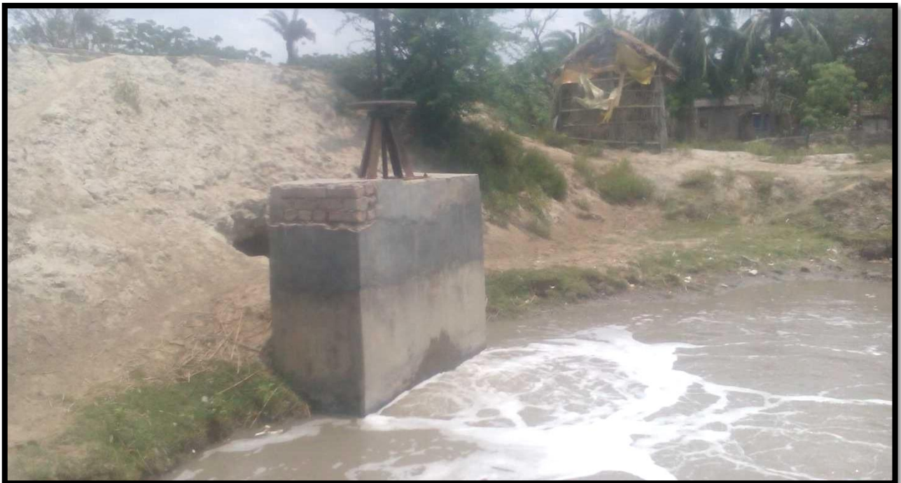
Lock gate at Chainage 4.7
