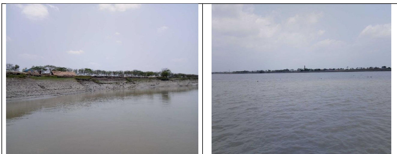
Figure 8: Photographs of Sub-stretch 2
