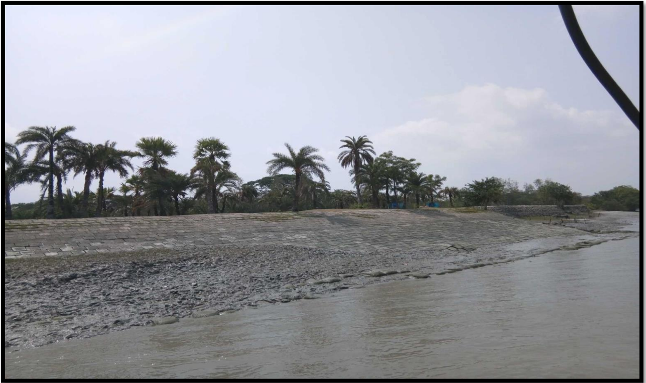
Bank Protection at Chainage 8.4
