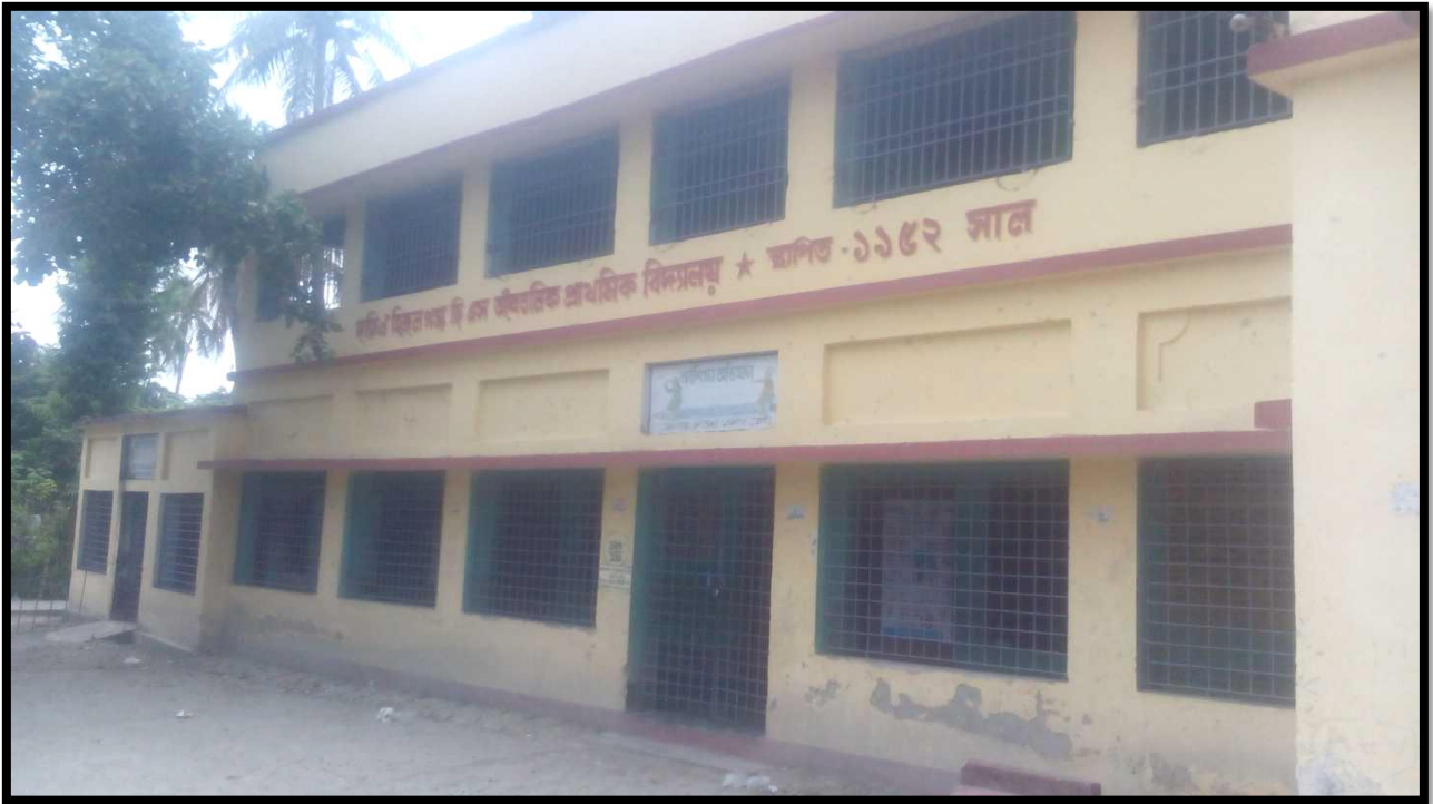
Govt School at Chainage 8.0
