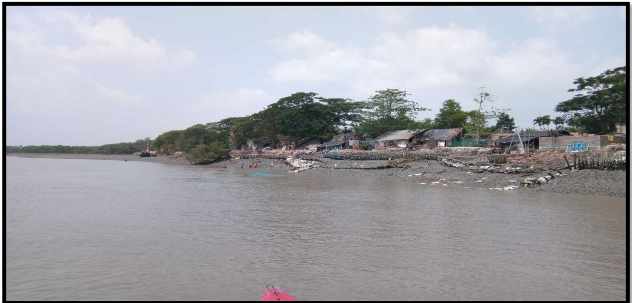
View at Chainage 8.4
