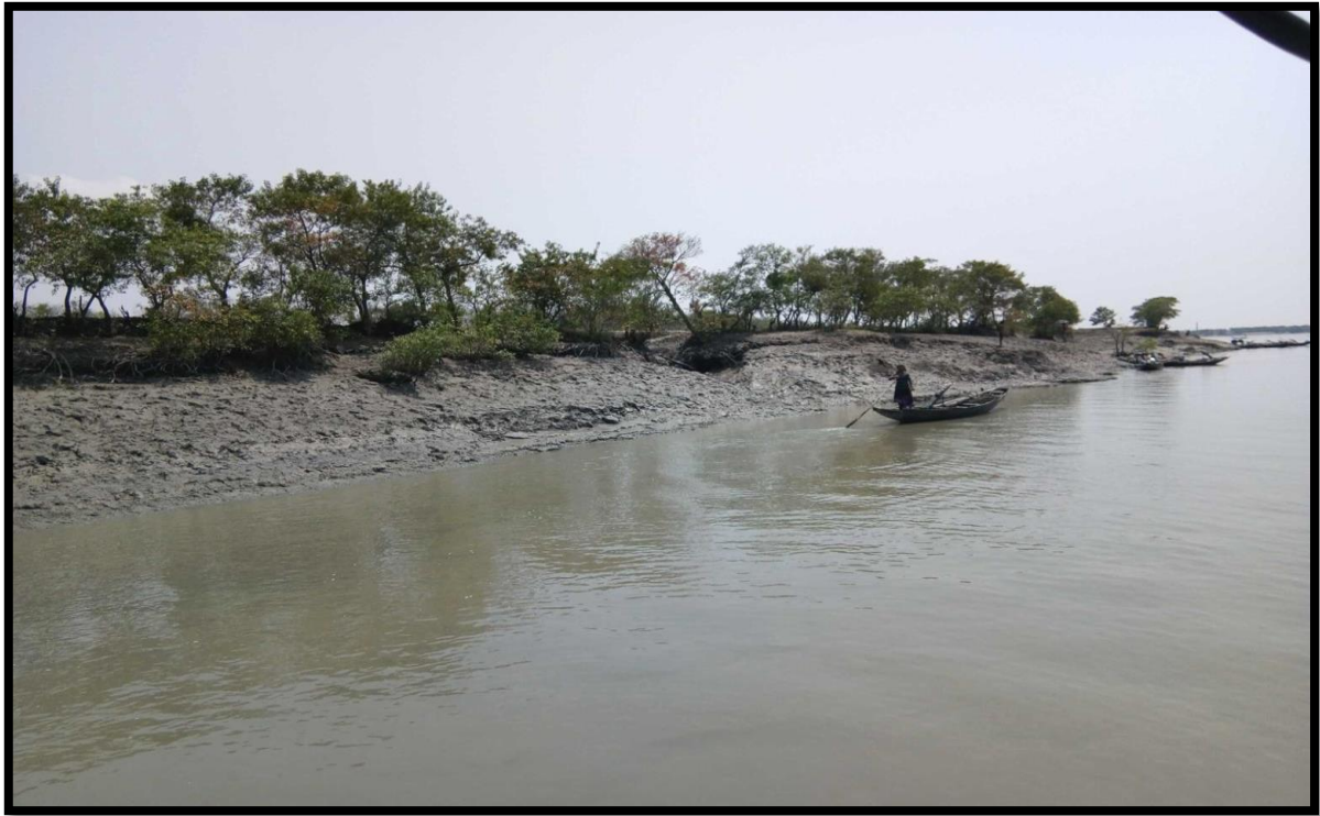
Unprotected Right bank at chainage 1.3
