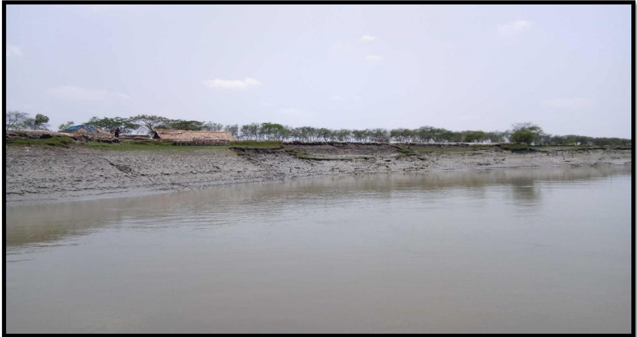
Bank Condition at Chainage 3.5
