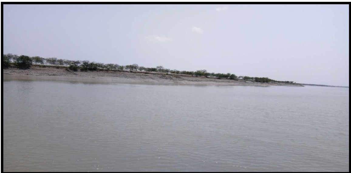
Unprotected Right bank at chainage 2.5
