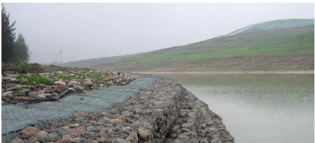
Figure 19: Photograph showing arrangement of Gabion Wall along River Bank
