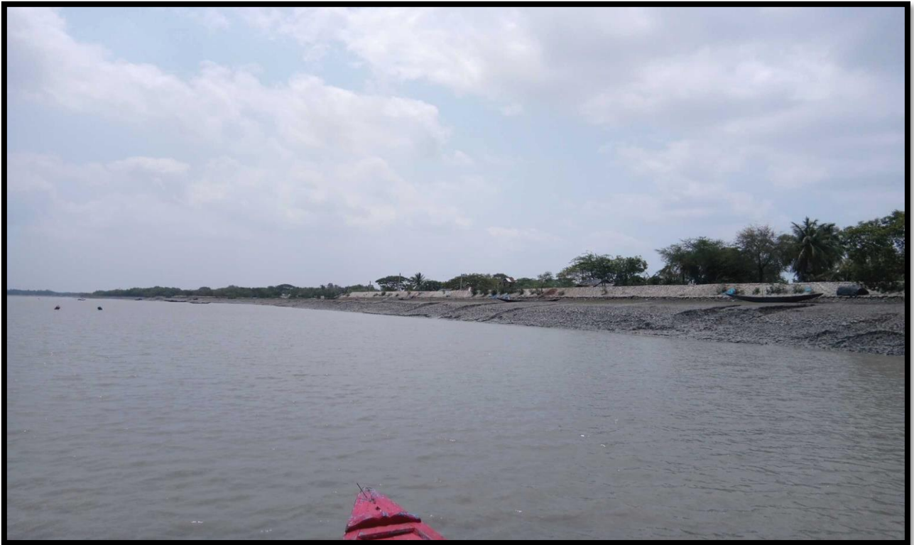
Protected Left bank at Chainage 5.0
