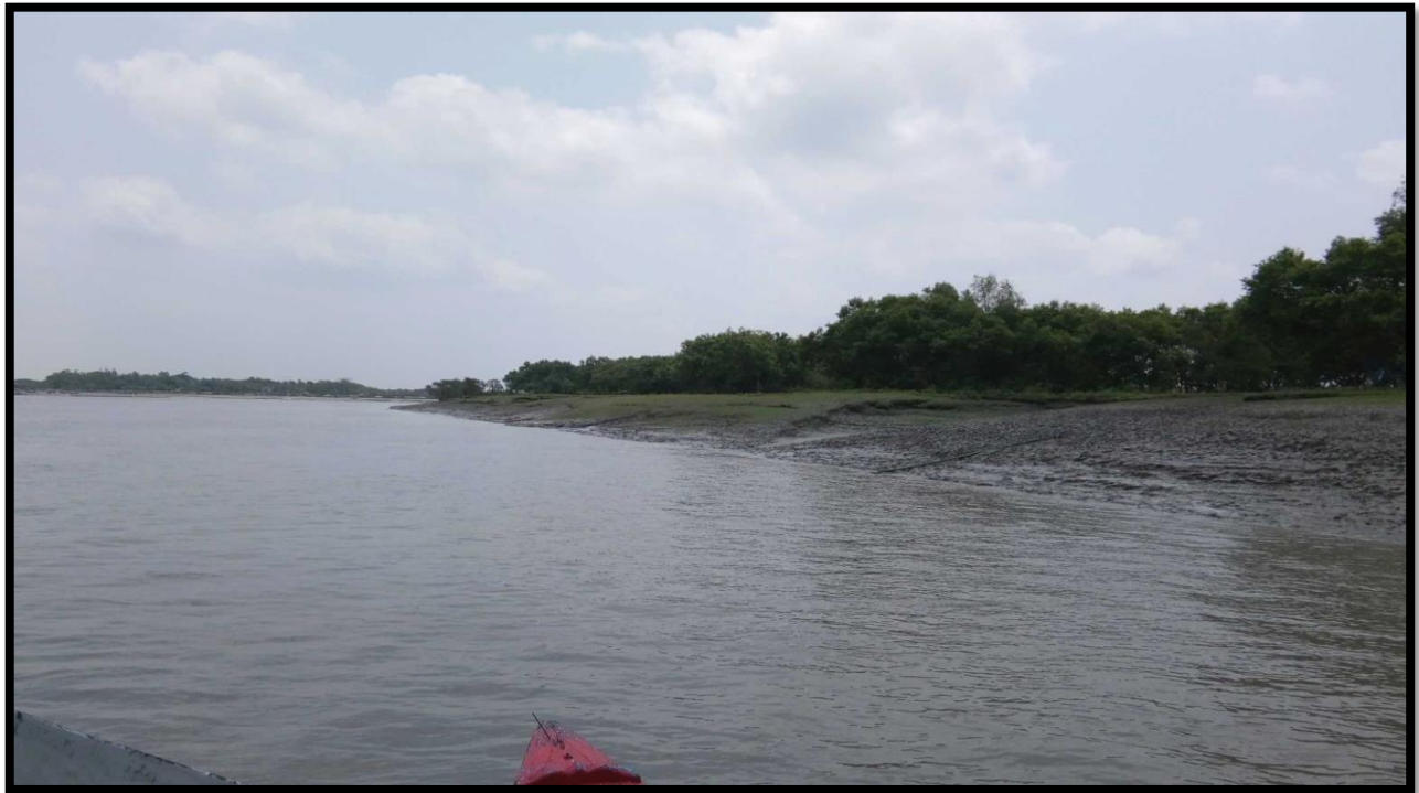
Bank Condition Left bank at Chainage 4.2
