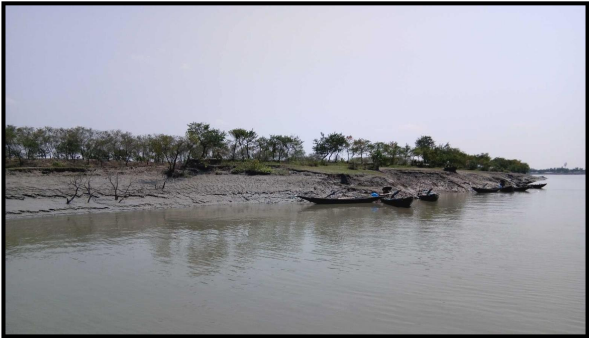
Unprotected Right bank at chainage 0.7
