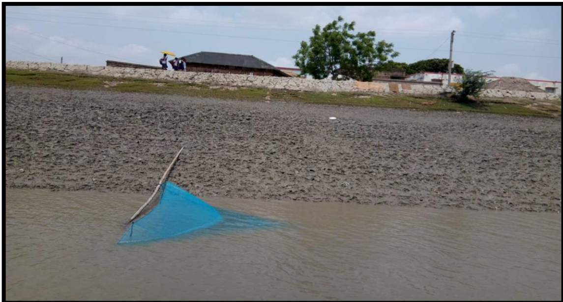
Unprotected Left Bank at CHAINAGE 4.0
