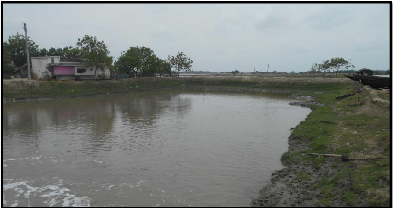
Pond on right bank at CHAINAGE 21.6
