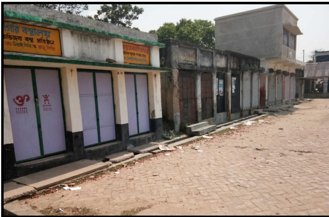
Shops on left bank at CHAINAGE 8
