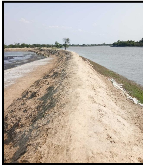
Right bank at CHAINAGE 6.5
