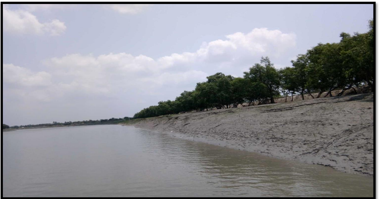
Unprotected Right Bank at CHAINAGE 8.5
