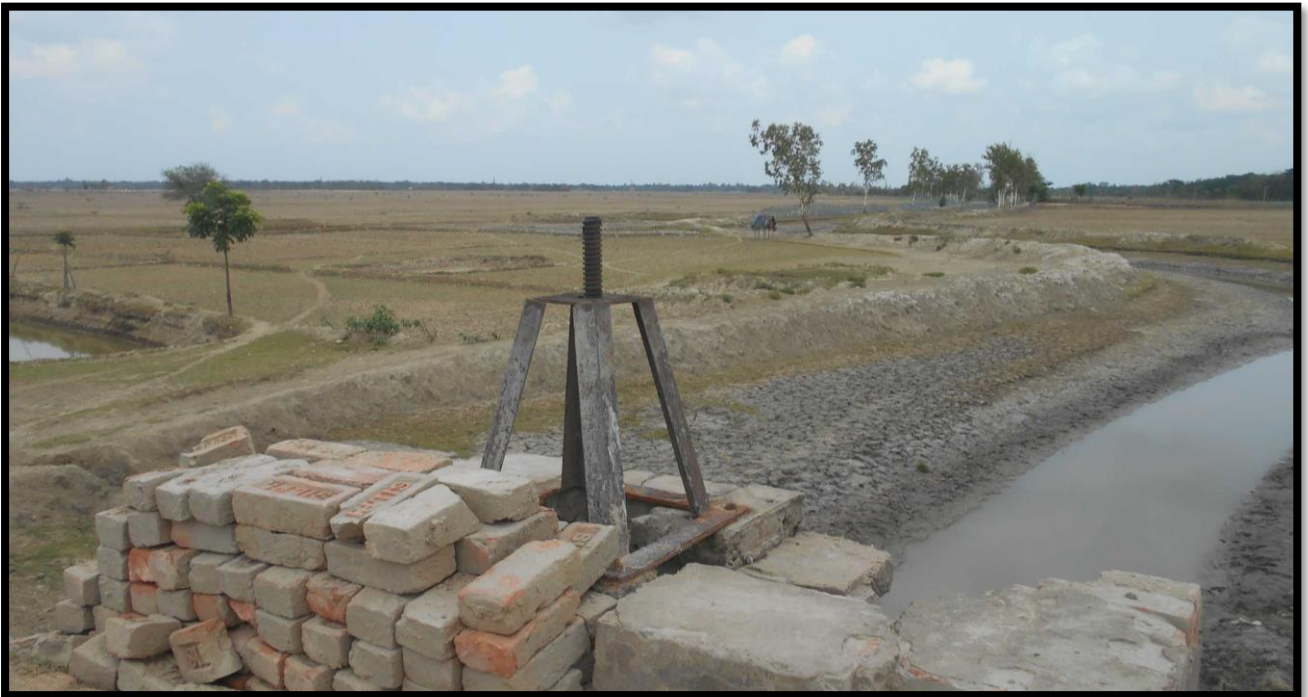
Water lock on right bank at CHAINAGE 17.8
