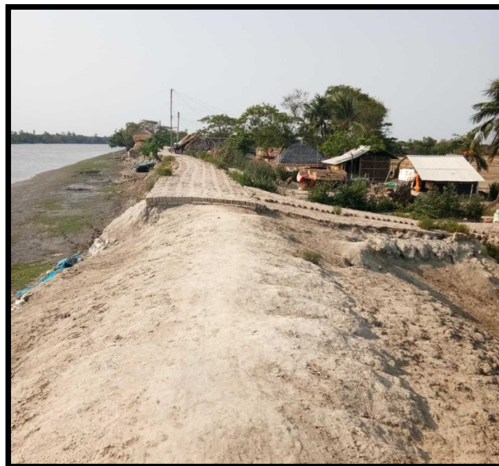
Right bank at 7.5 CHAINAGE
