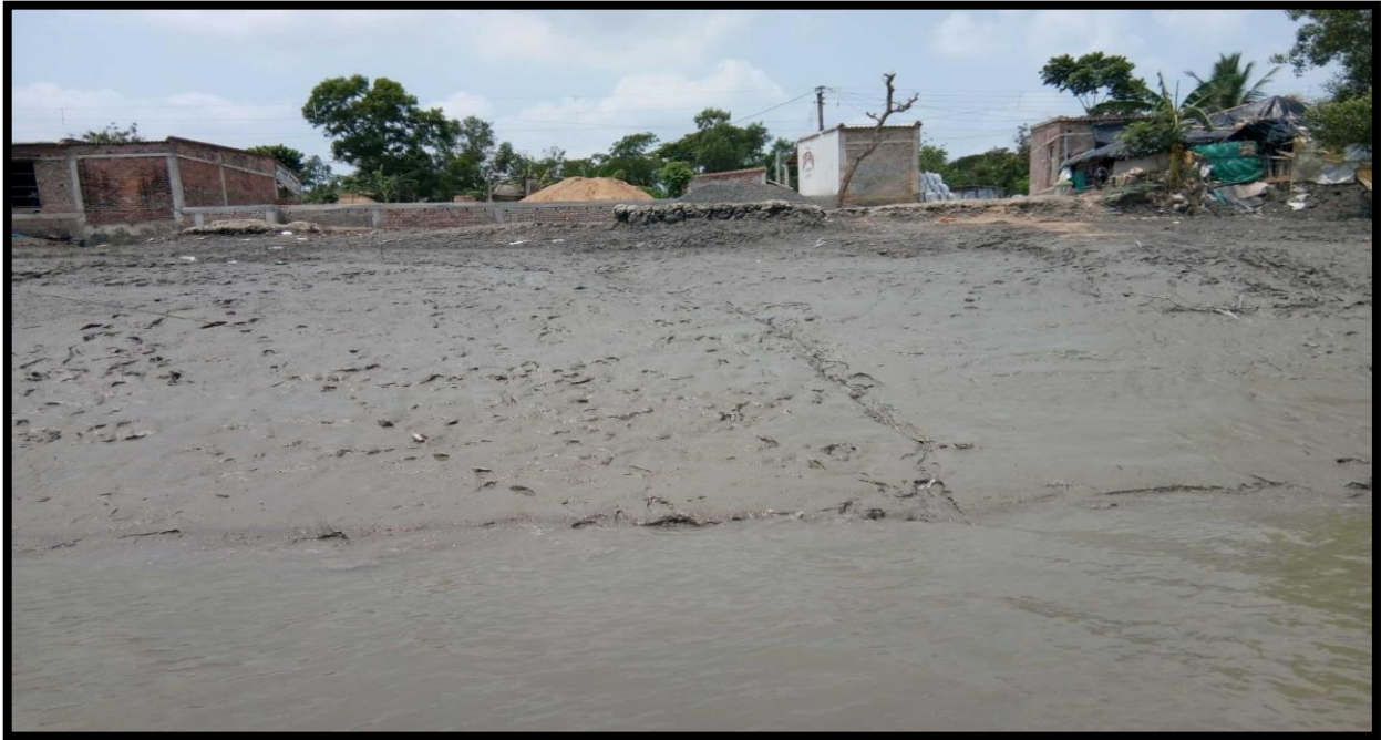
Unprotected Left Bank at CHAINAGE 4.7
