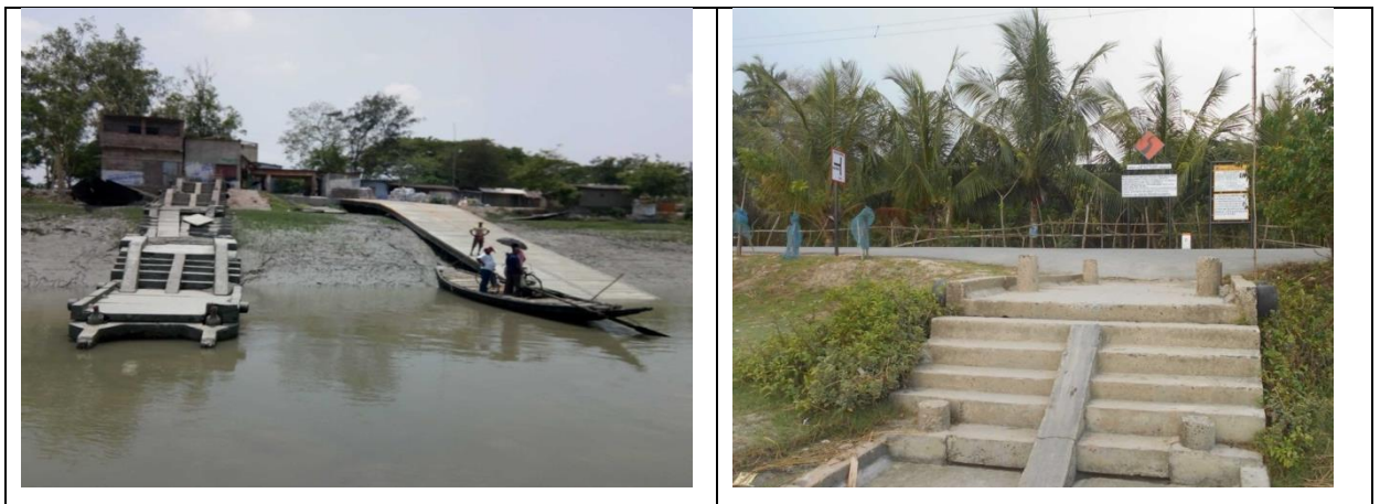
Figure 23: Photographs of Jettiy located along Katakhal Waterway
