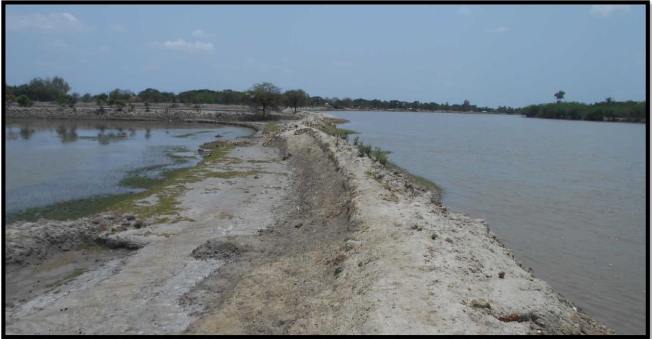
Right bank at CHAINAGE 9.0
