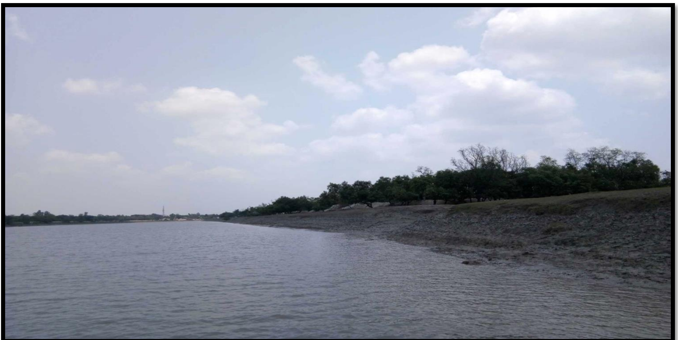
Unprotected Right Bank at CHAINAGE 7.0
