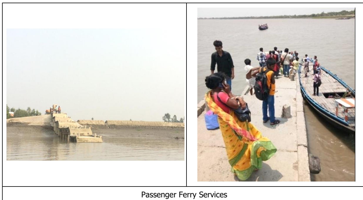
Figure 21: Photographs of IWT services along Katakhal Waterway
