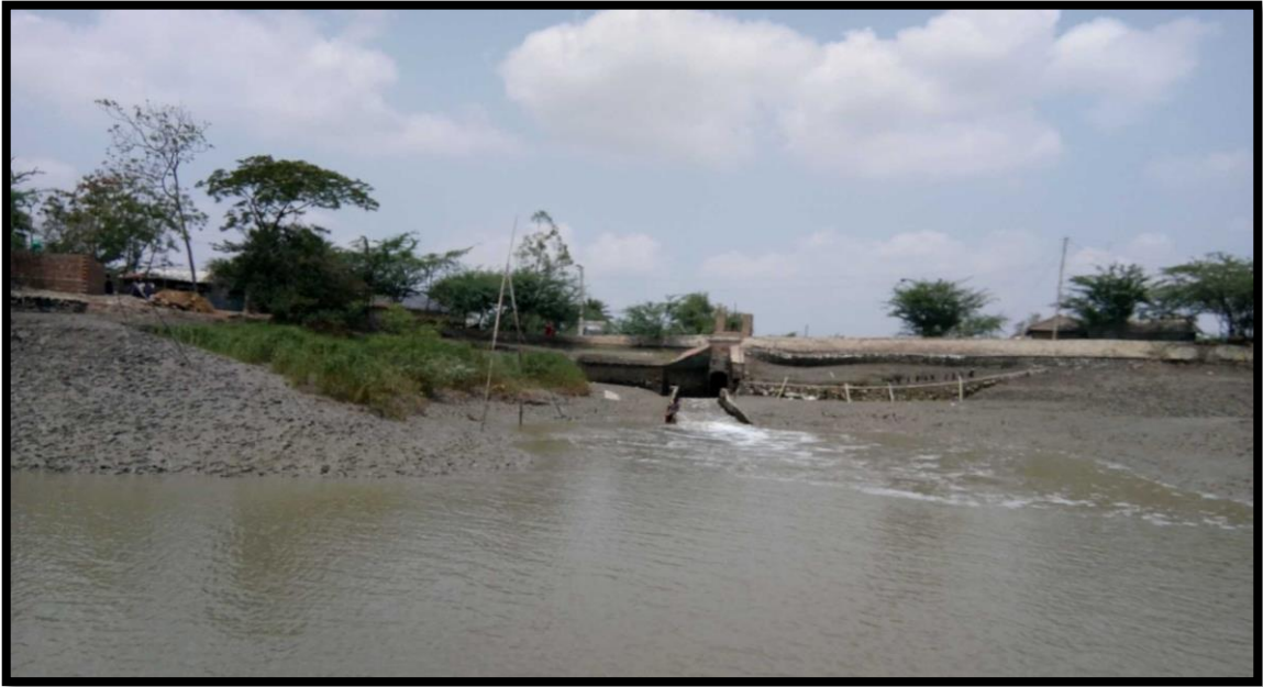
Lock Gate at 4.0 CHAINAGE
