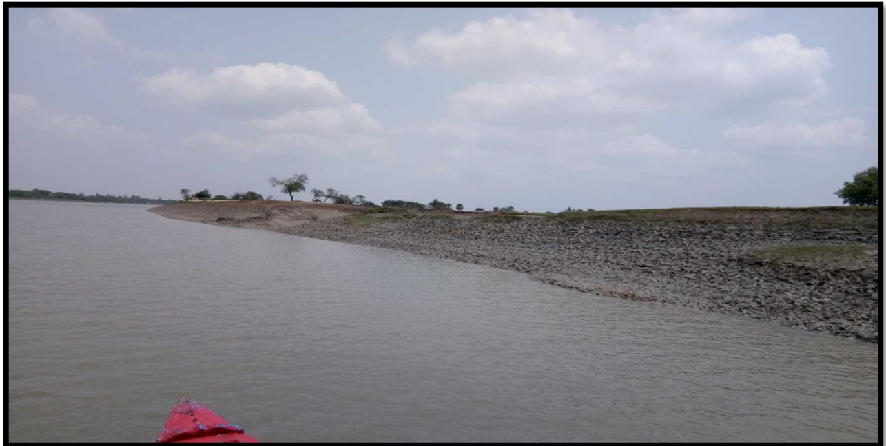
Unprotected Right Bank at CHAINAGE 6.0
