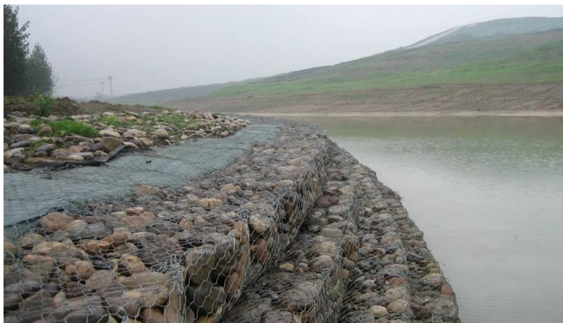
Figure 15: Photograph showing arrangement of Gabion Wall along River Bank
