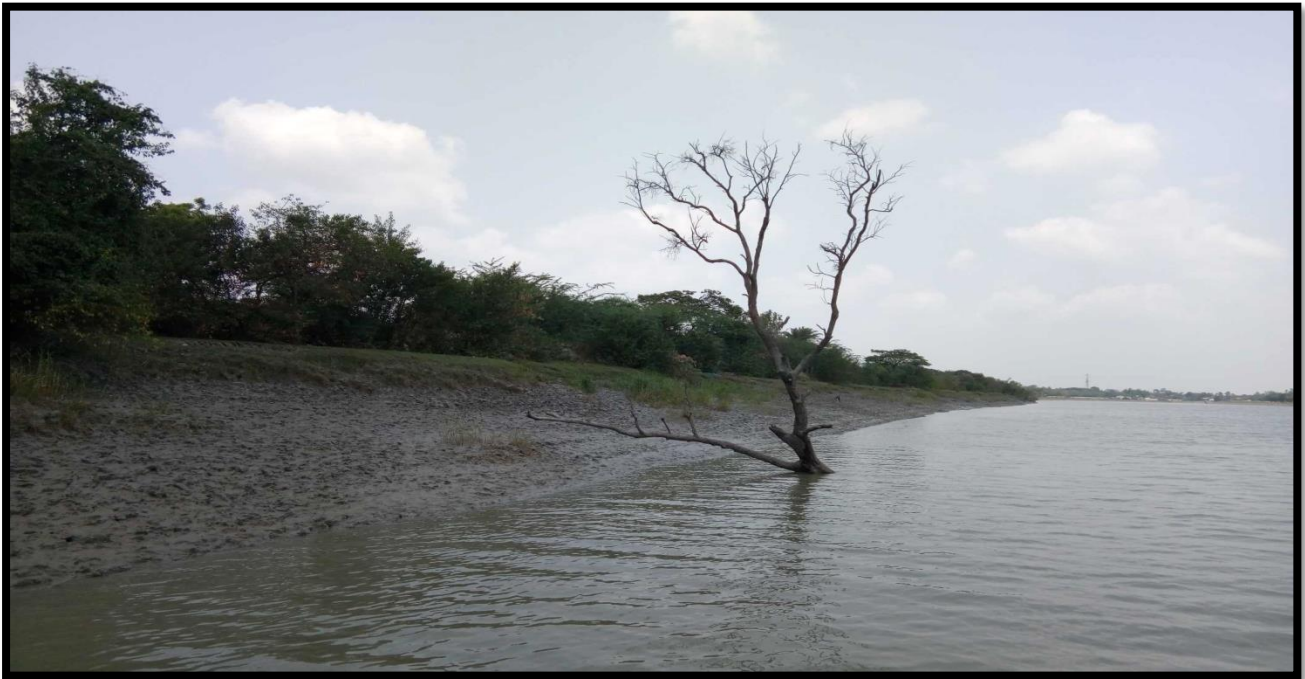
Unprotected Left Bank at CHAINAGE 7.0
