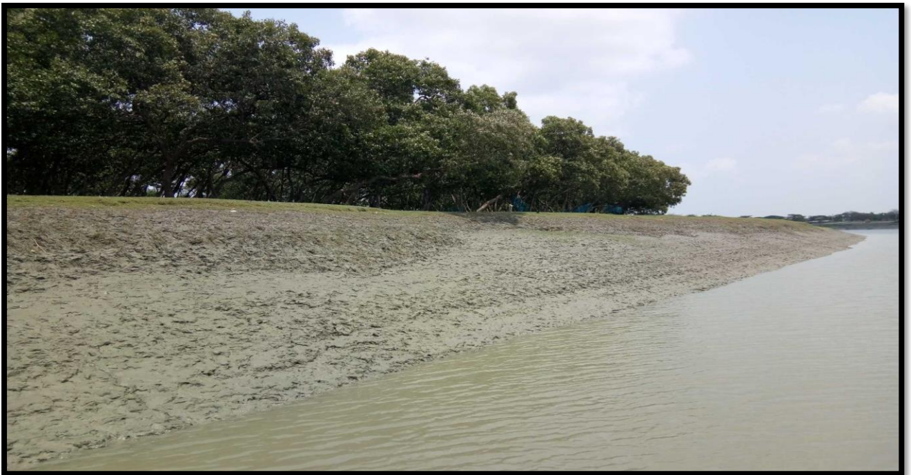
Unprotected Left Bank at CHAINAGE 9.0
