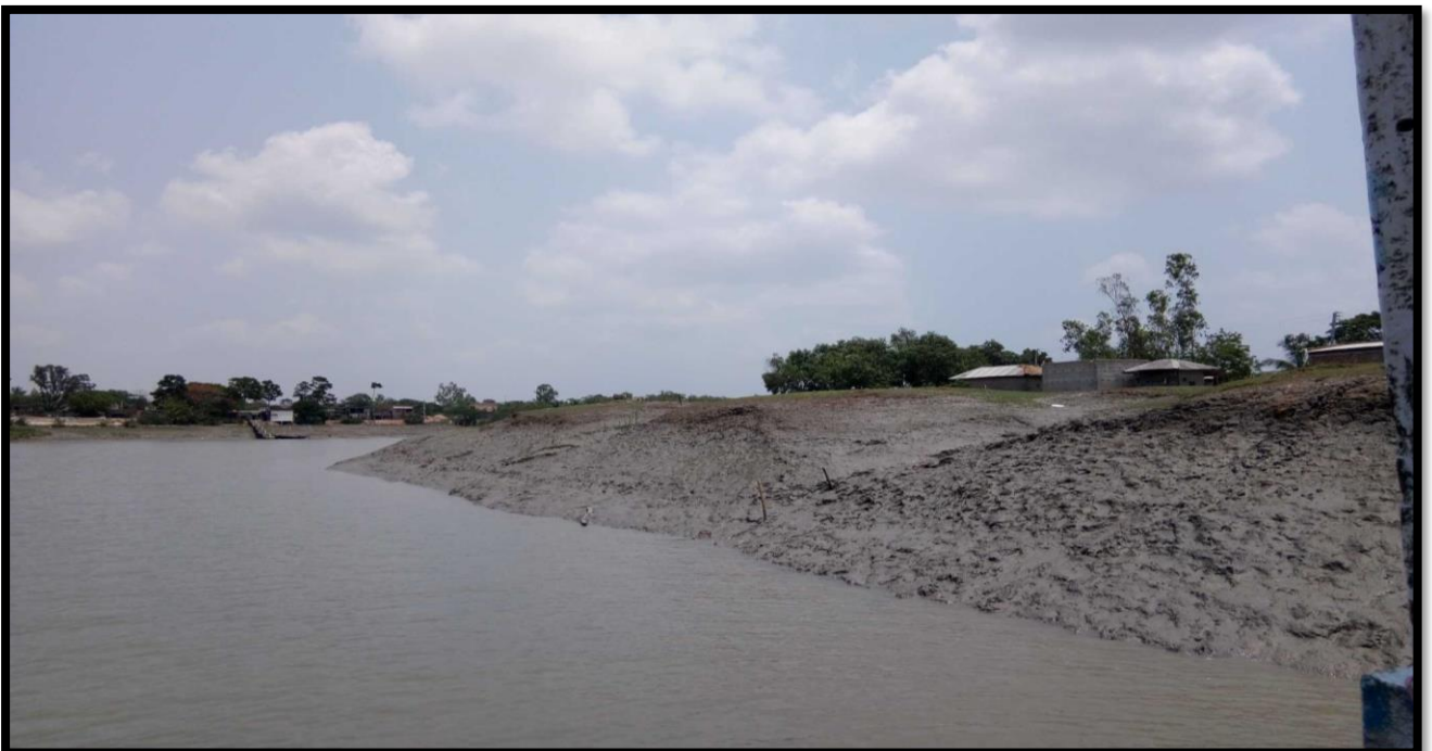
Unprotected Right Bank at CHAINAGE 8.0
