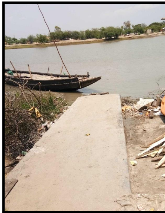
Small Jetty on left bank at CHAINAGE 12.9
