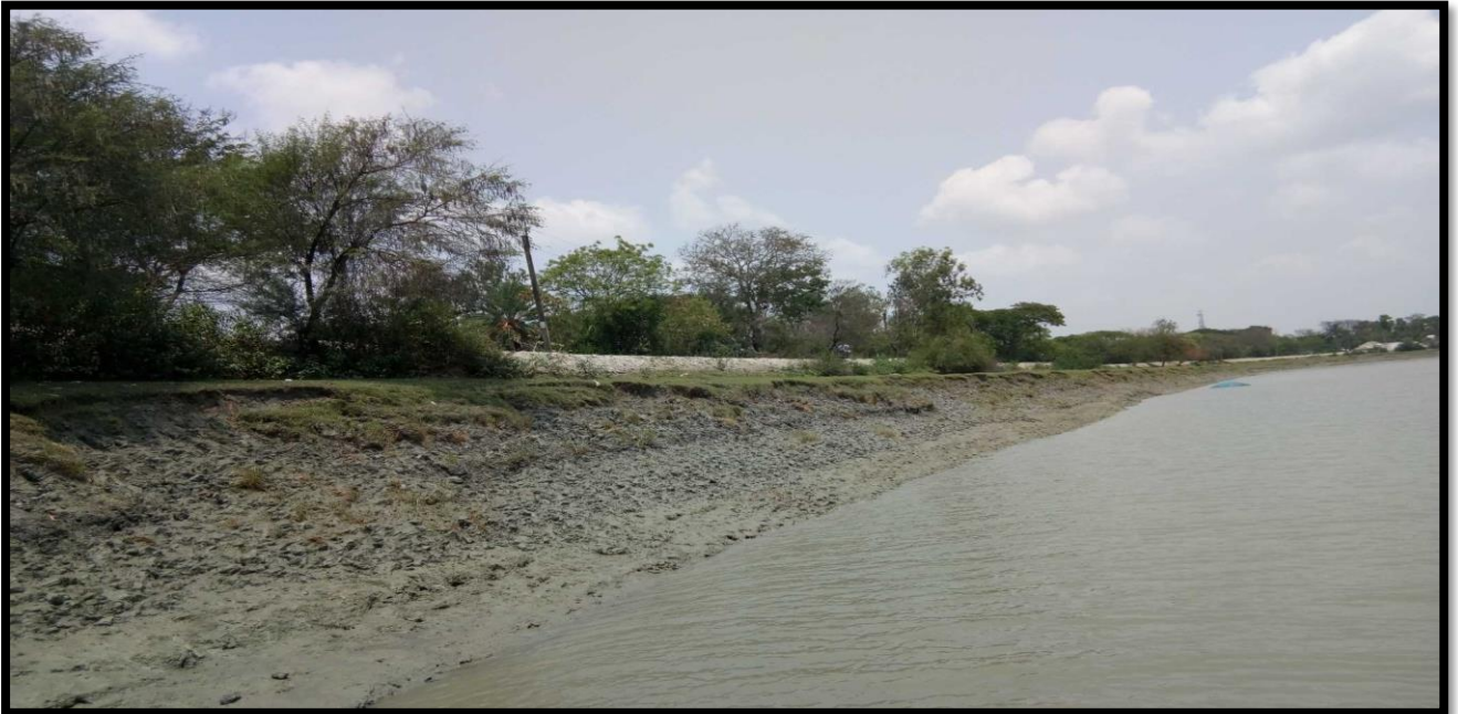
Unprotected Left Bank at CHAINAGE 7.5
