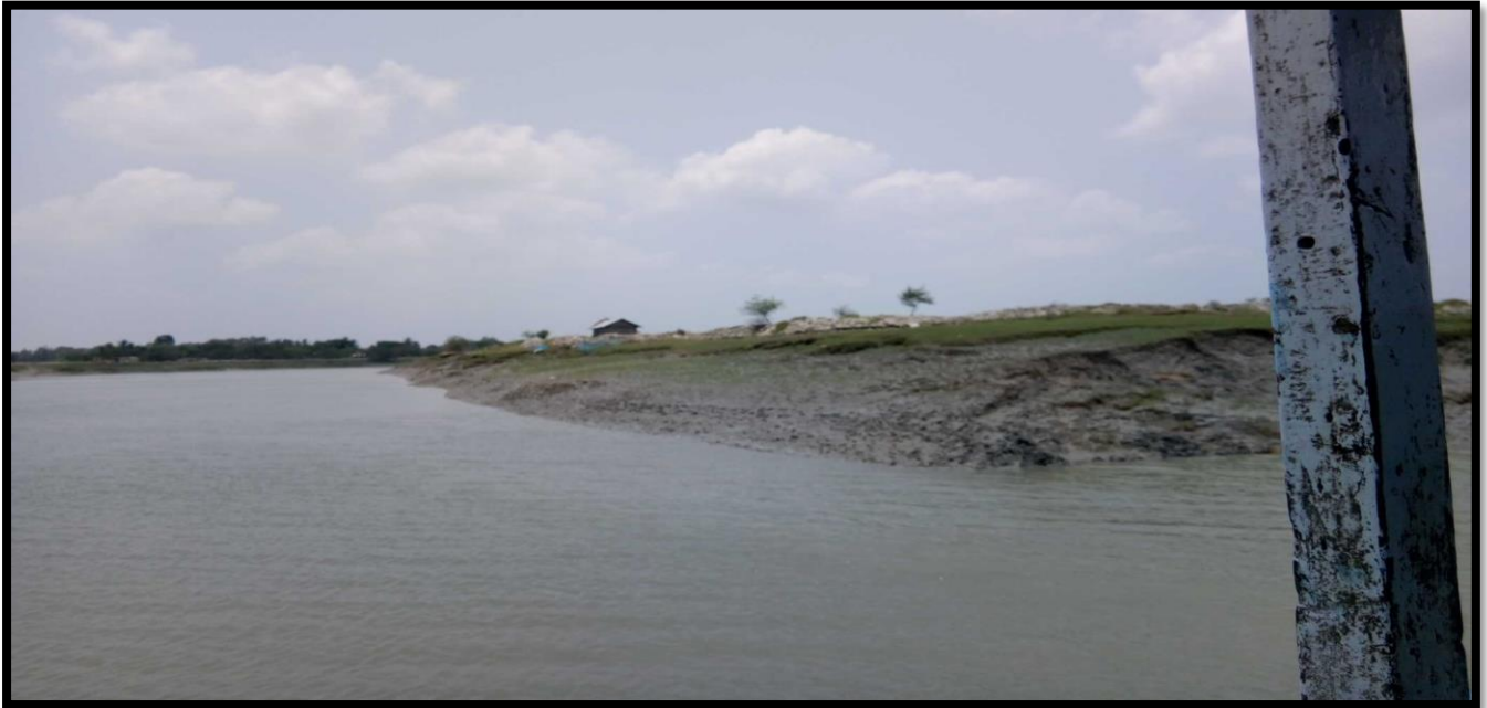
Unprotected Right Bank at CHAINAGE 11.5
