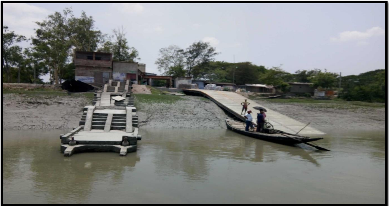
Ferry Jetty on Right Bank at CHAINAGE 16.5
