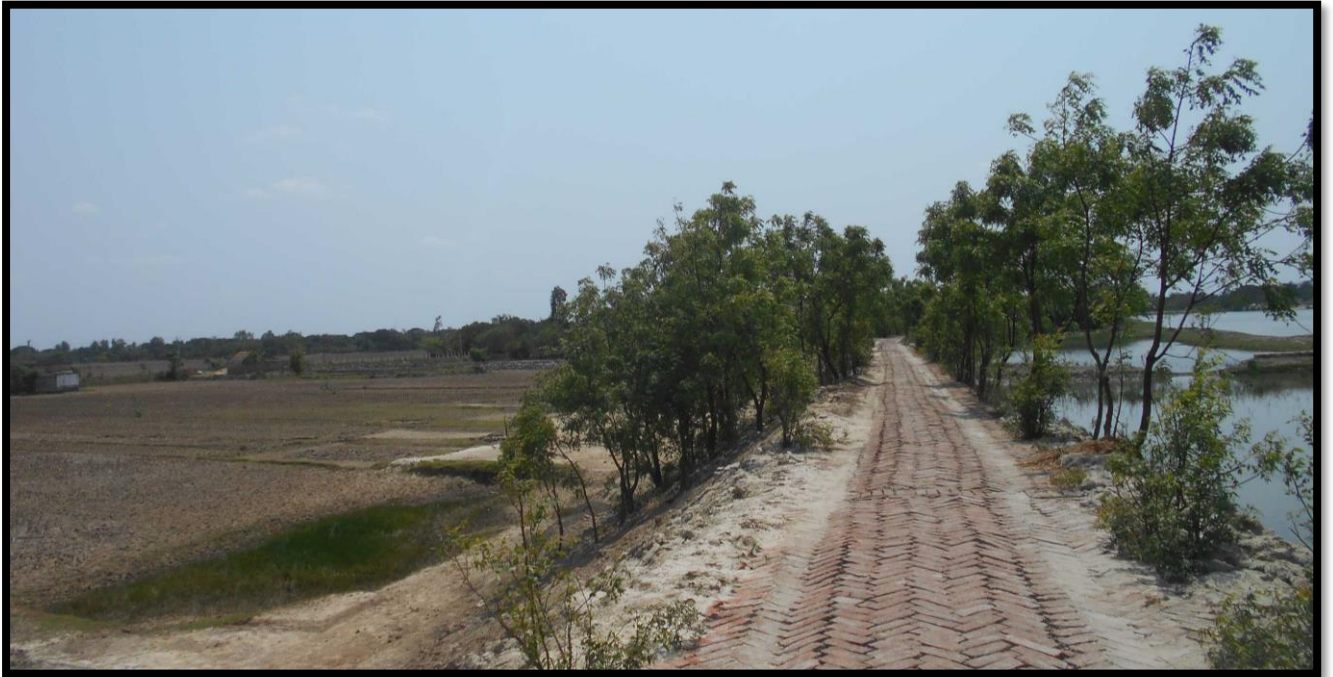
Walkway on right bank at CHAINAGE 8.5
