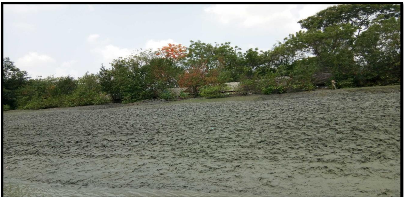
Unprotected Left Bank at CHAINAGE 5.5
