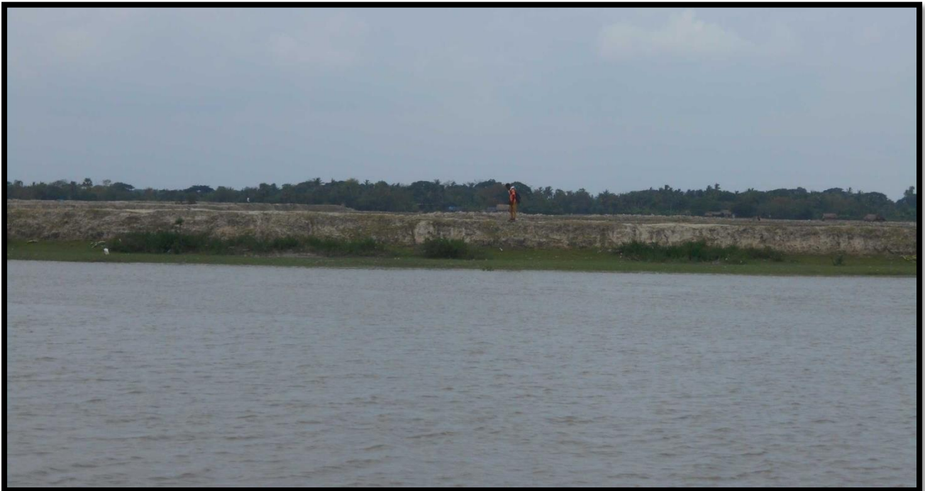
Pond on right bank at CHAINAGE 20.7
