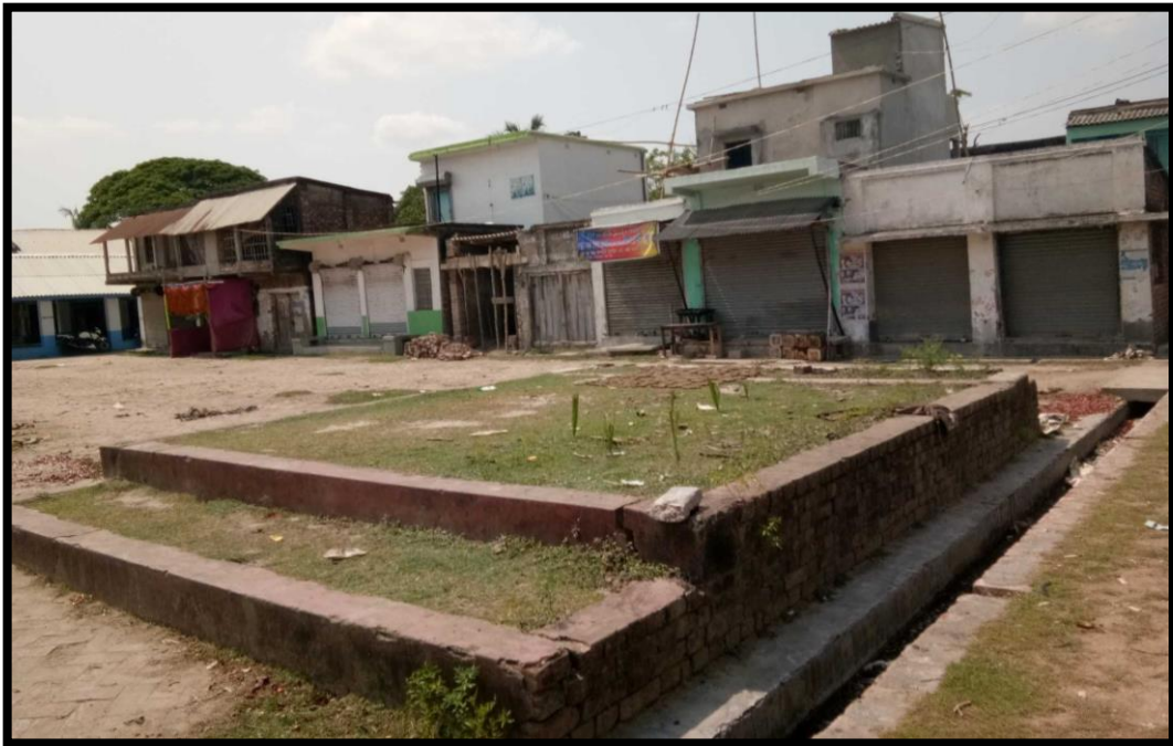
Shops on left bank at CHAINAGE 8
