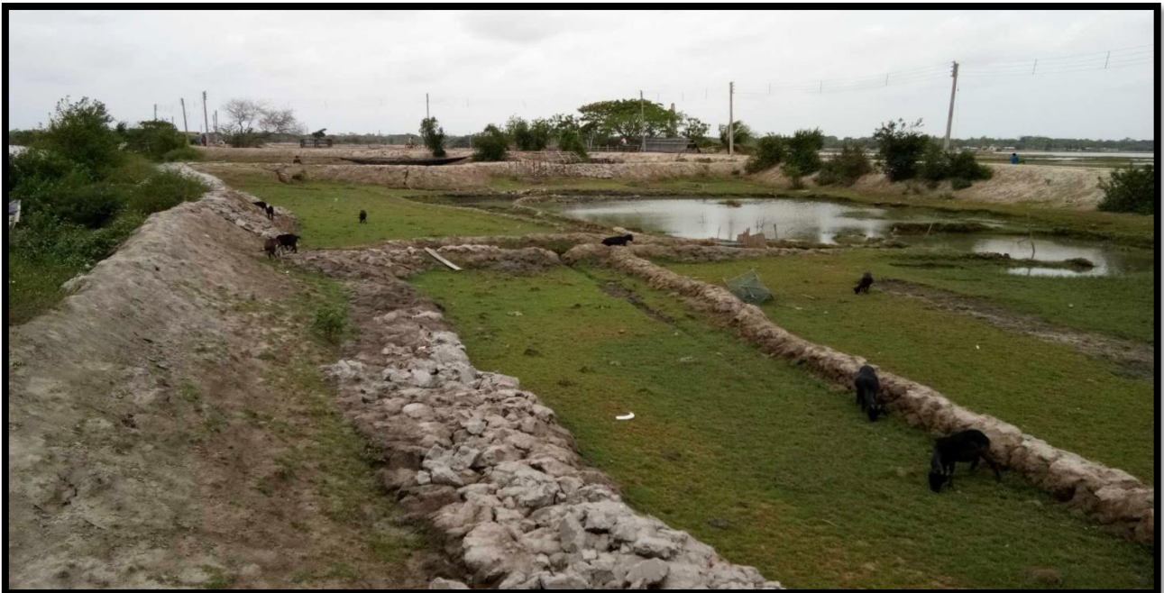
Pond on left bank at CHAINAGE 21.4
