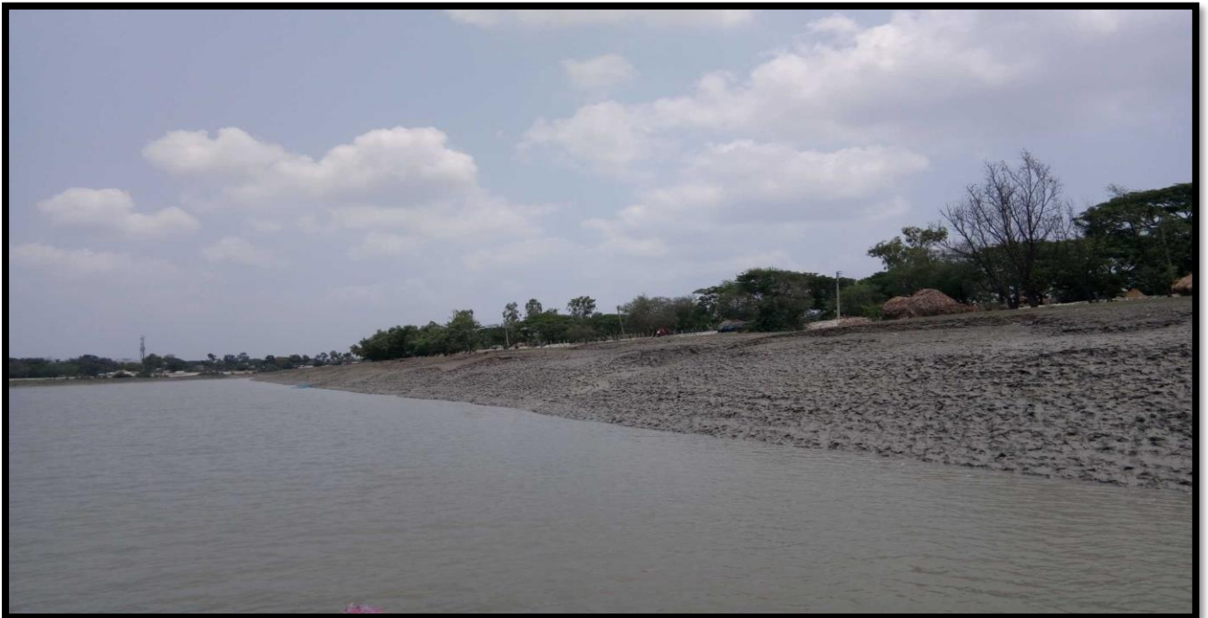
Unprotected Right Bank at CHAINAGE 7.5
