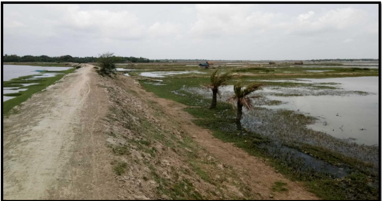
Pond on left bank at CHAINAGE 20.4
