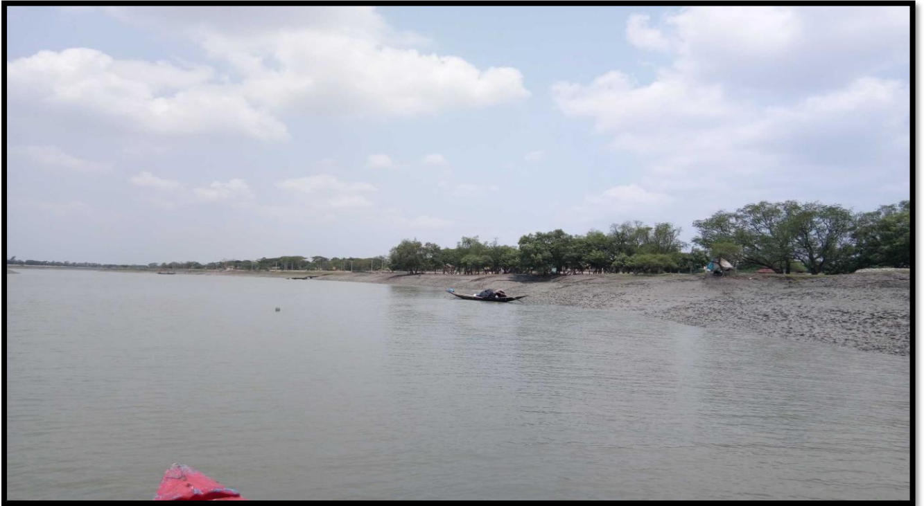
Unprotected Right Bank at CHAINAGE 10
