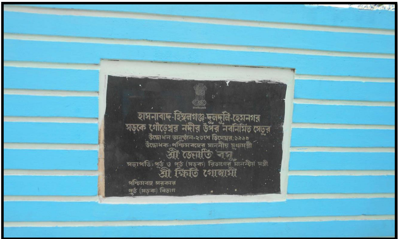
Bridge at CHAINAGE 22.1
