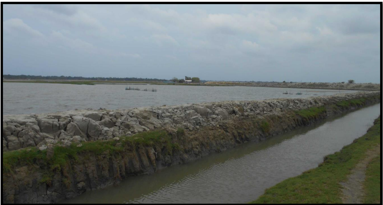
Pond on right bank at CHAINAGE 21.1
