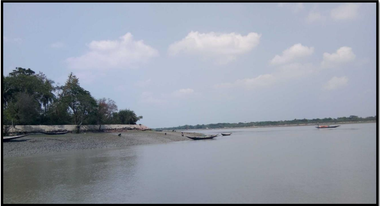
Unprotected Left Bank at CHAINAGE 22.5
