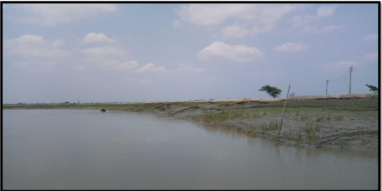
Unprotected Right Bank at CHAINAGE 20.0
