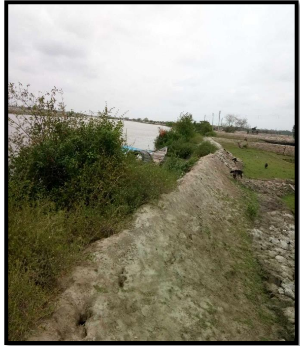
Left Bank at CHAINAGE
