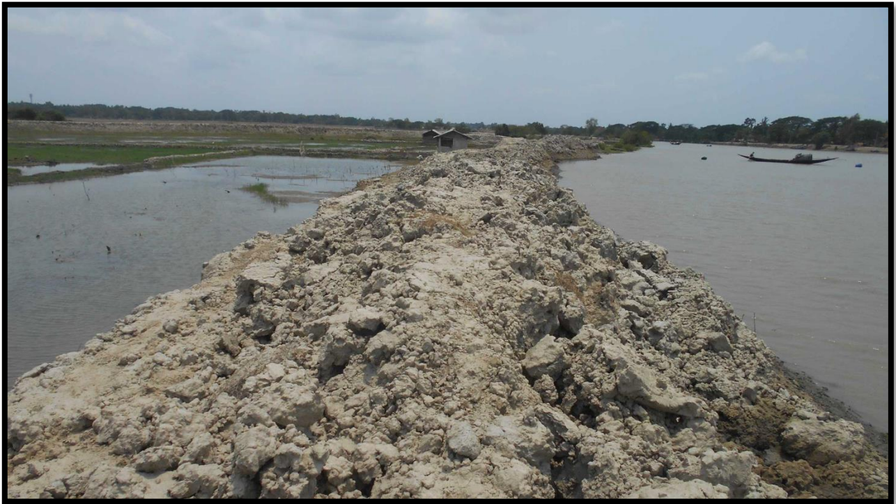
Right river bank at CHAINAGE 20.0
