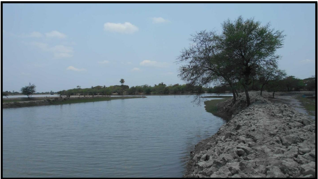
Creek on right bank at CHAINAGE 9.3
