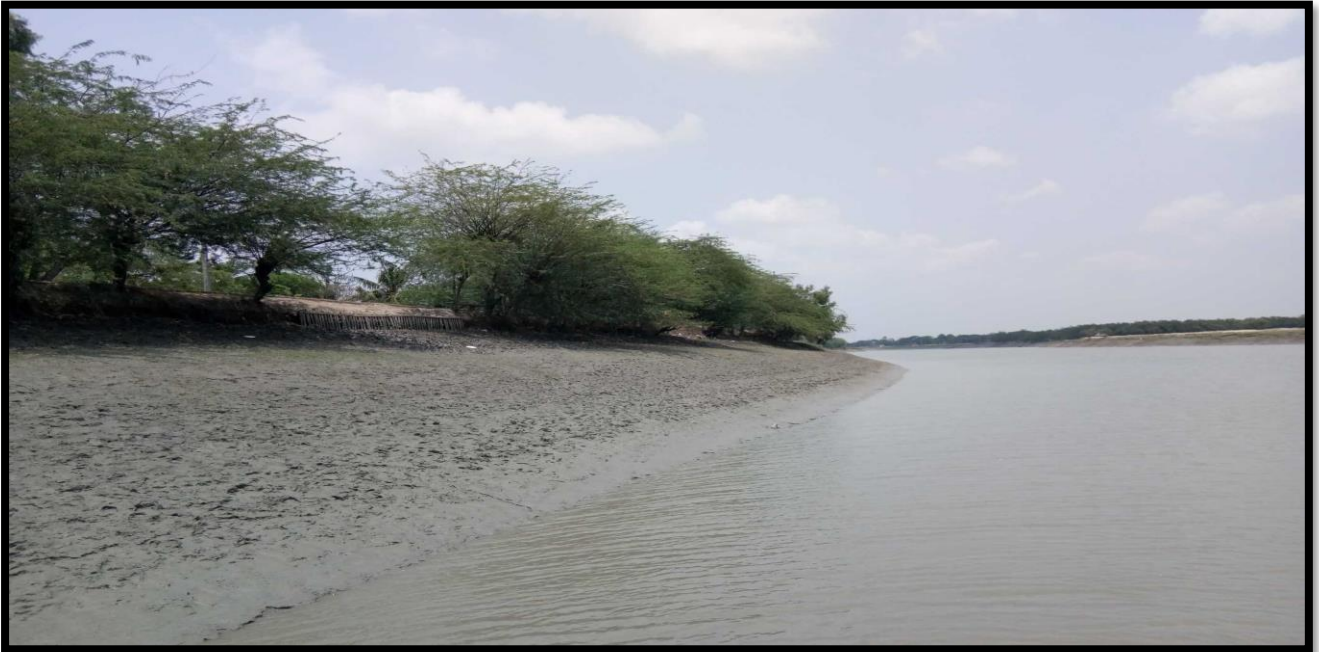
Unprotected Left Bank at CHAINAGE 9.5
