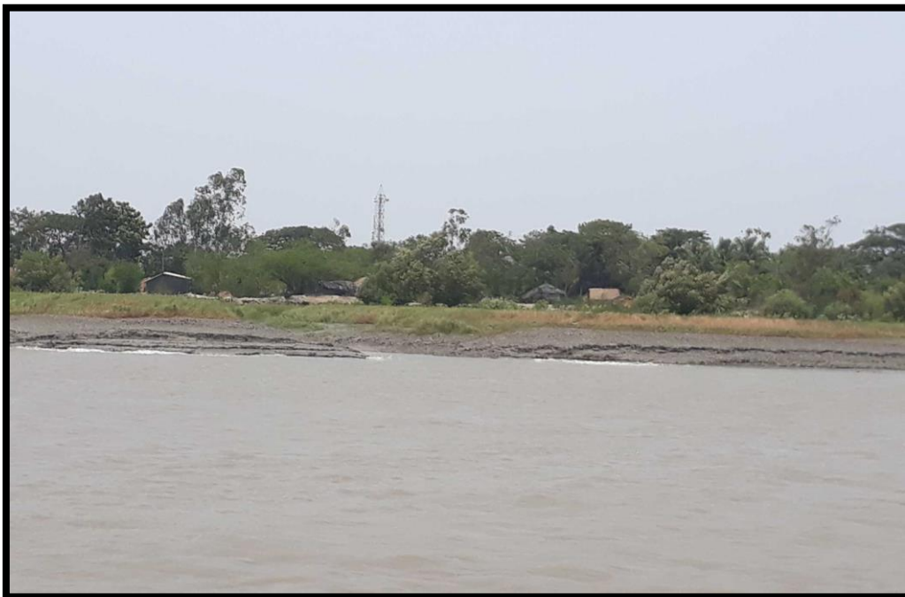
Telecommunication Tower at Chainage 7.5
