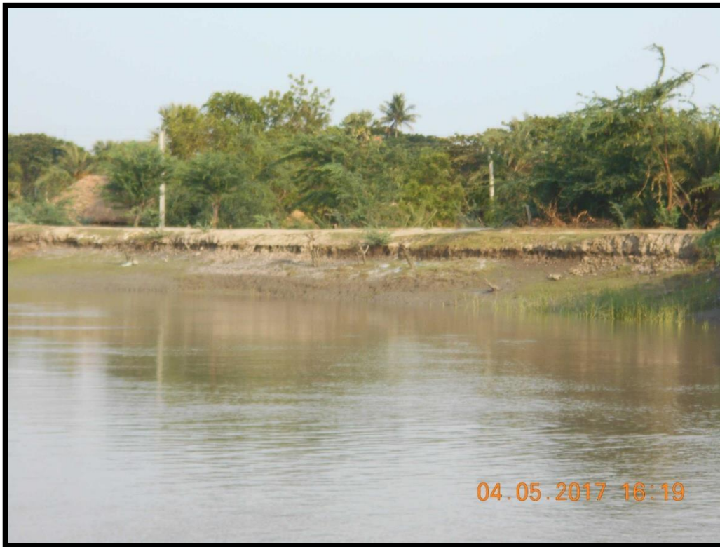
River Left Bank at chainage 8.4
