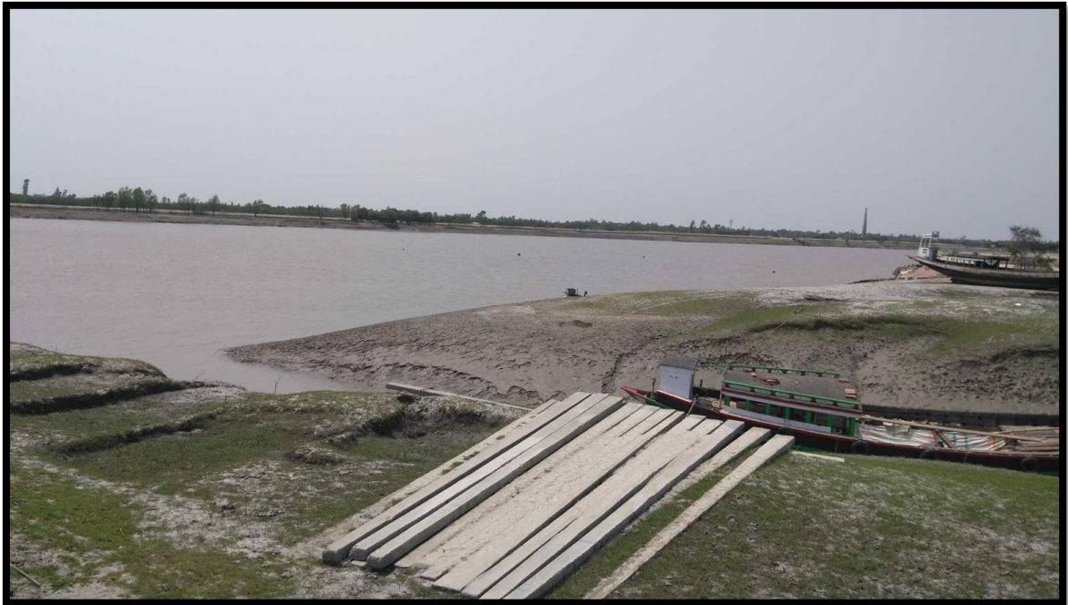
View on Right Bank at Chainage 9.7
