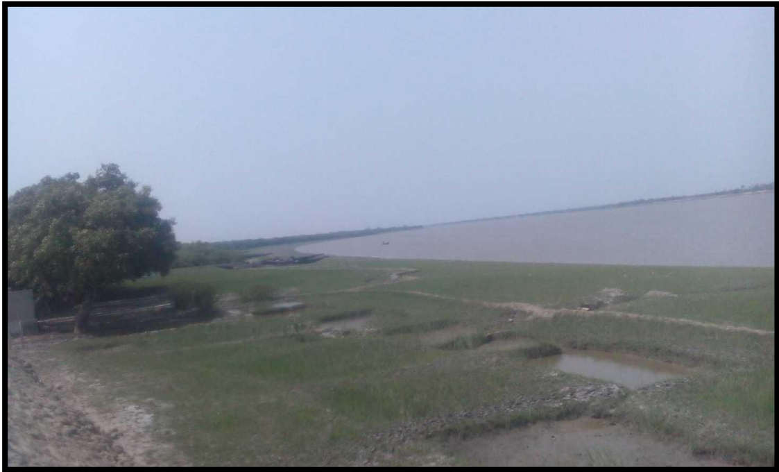
Bank Condition at Chainage 3.4
