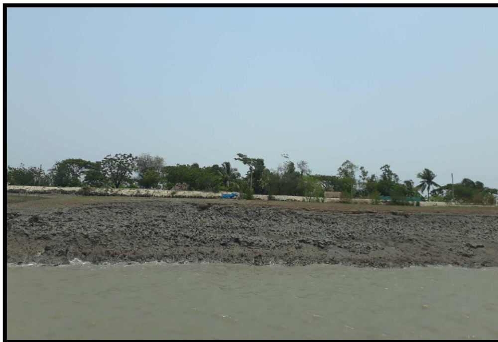
Bank Condition at Chainage 6.8
