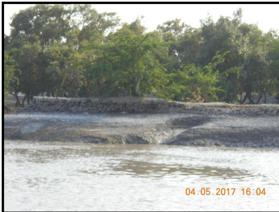
Left River Bank at chainage 9.4
