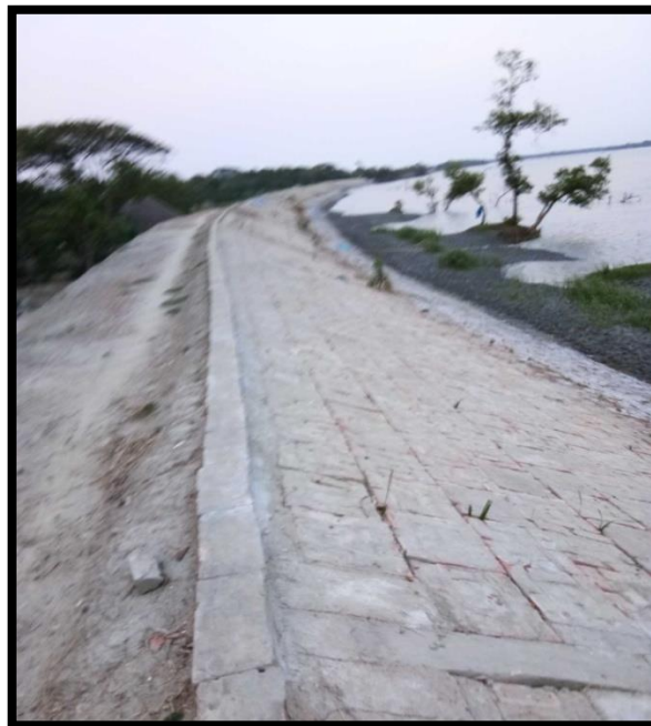
Protected River Bank at Chainage 14.5
