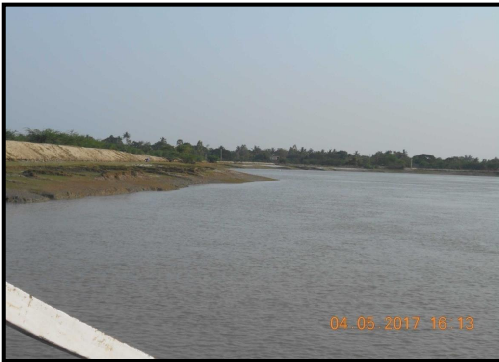
River Bank at chainage 8.6
