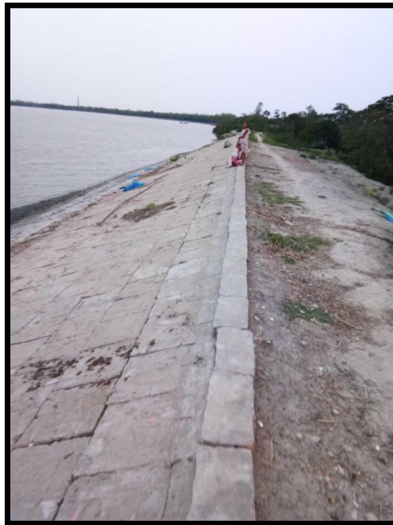
Right Bank Protection at Chainage 14.6
