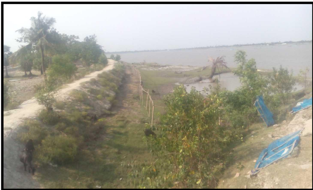
River bank at Chainage 5.0
