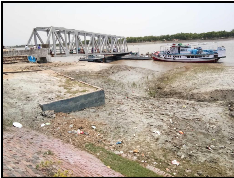
Vessel Jetty Bridge at chainage 8.0
