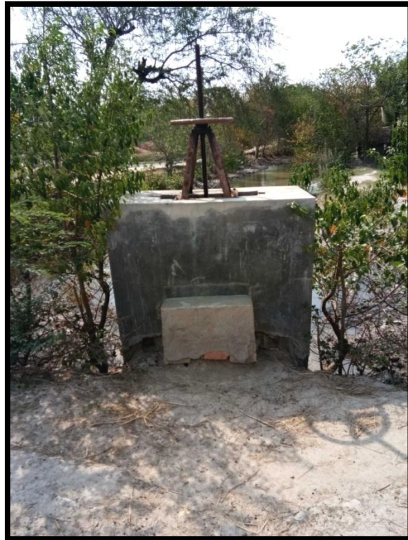
Lock Gate at Chainage 11.0
