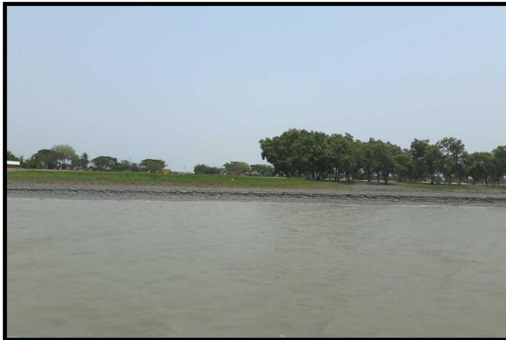
Unprotected bank at Chainage 6.4
