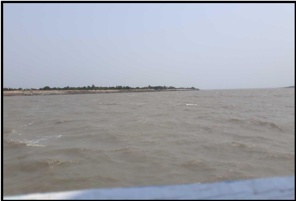
Protected River Bank at Chainage 4.0
