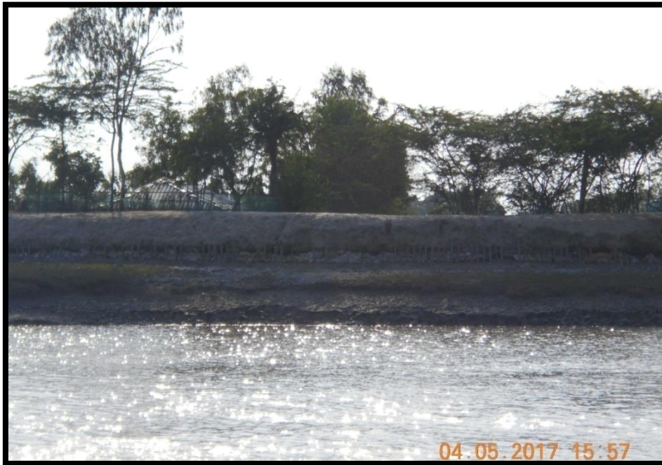
Left River Bank at chainage 9.7
