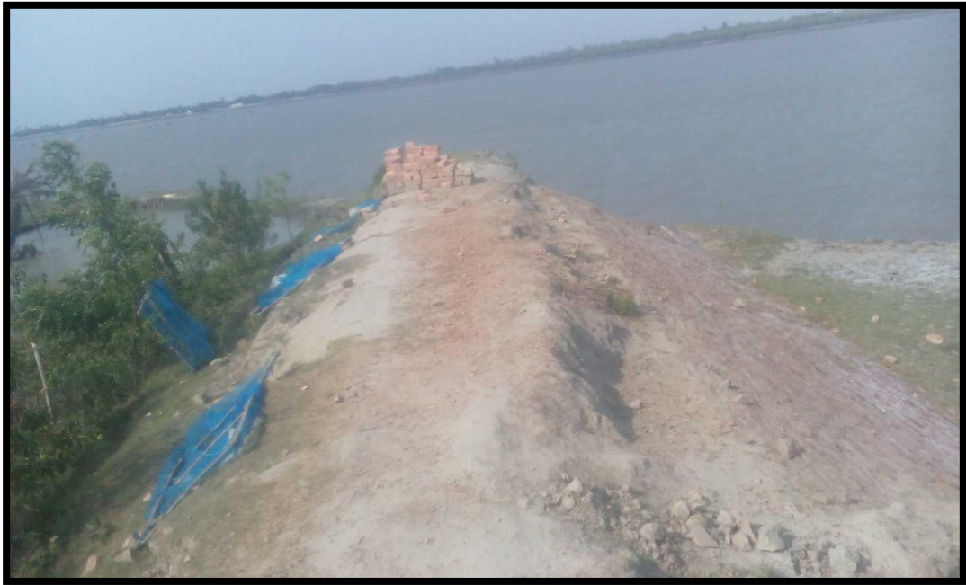
Bund on Left Bank at Chainage 4.8
