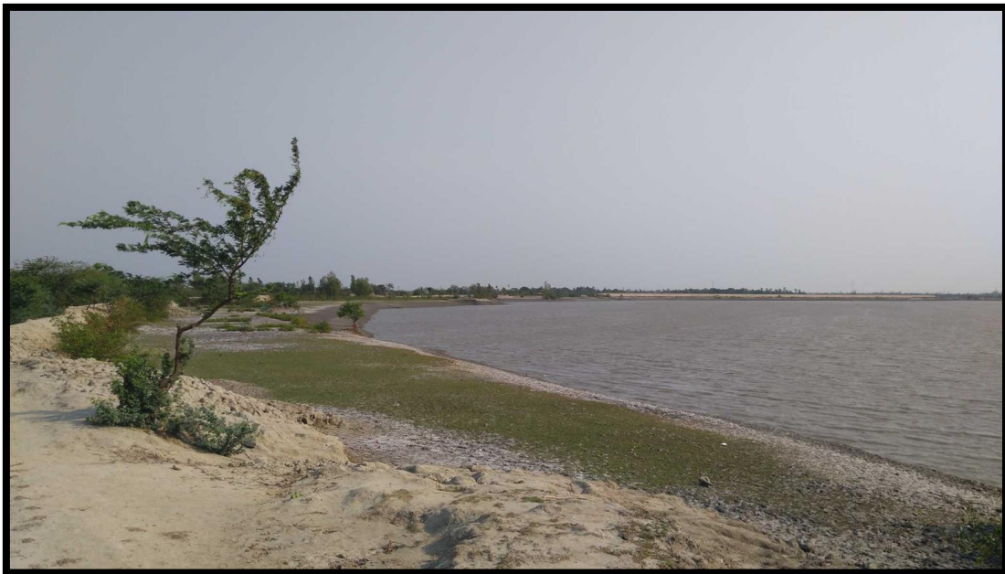
View of Right Bank at Chainage 12.7
