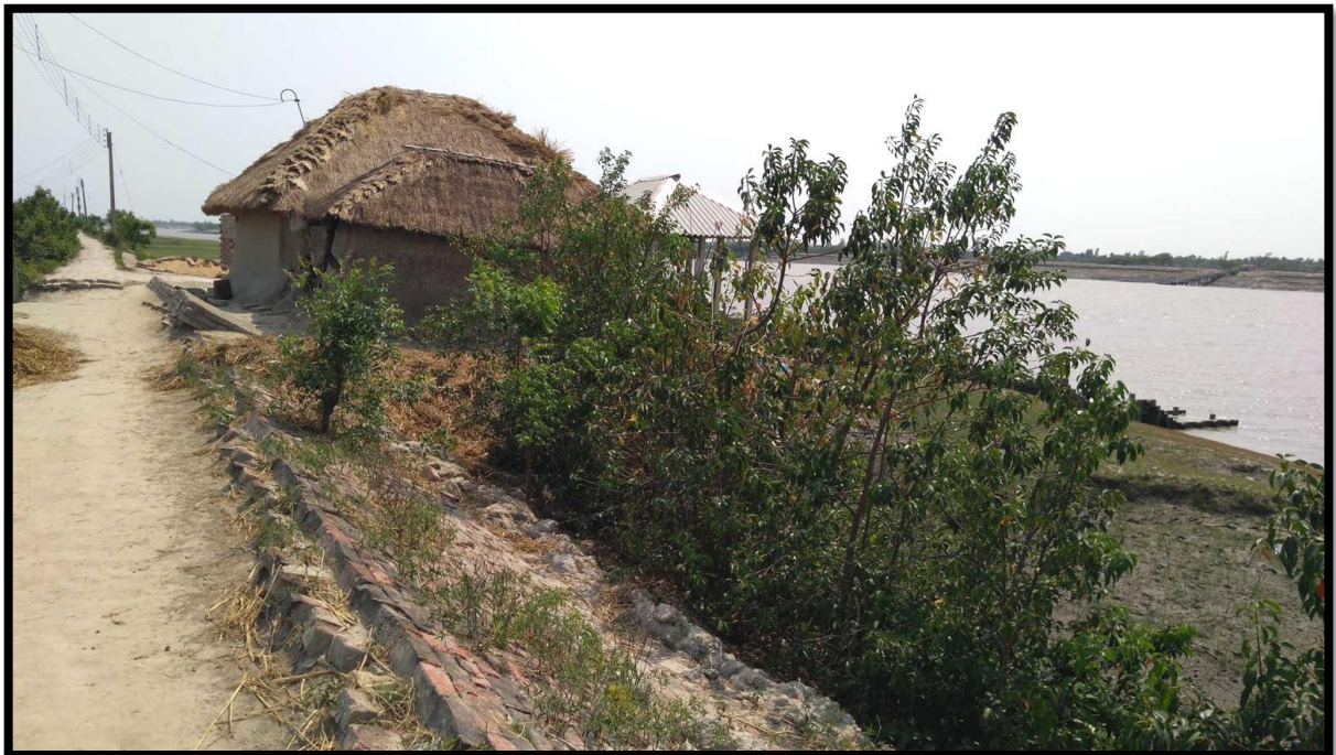
View of Right Bank at Chainage 10.4
