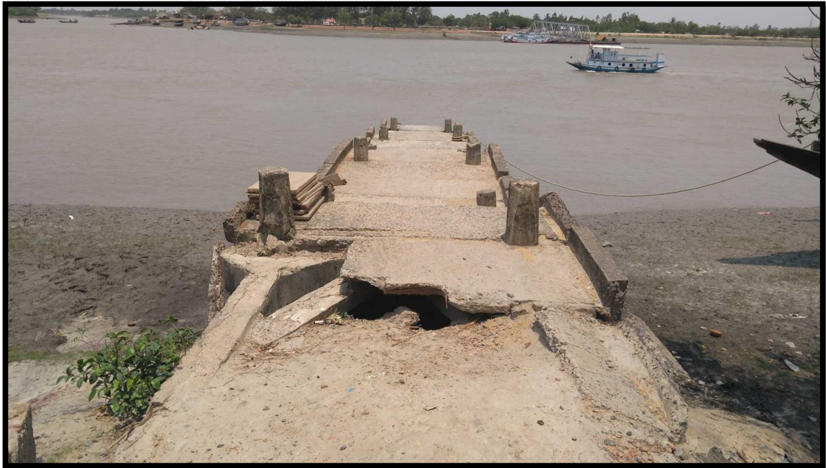
Local Jetty on the Right Bank at Chainage 8.1
