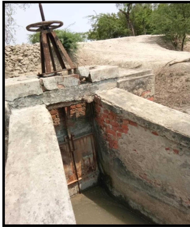
Lock gate at Chainage 9.5
