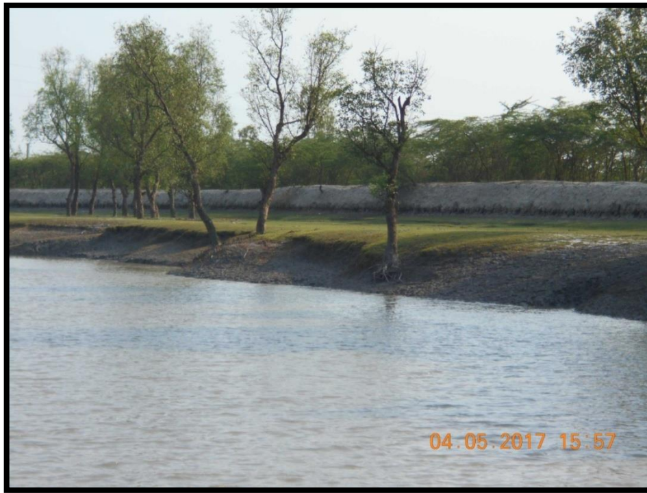
Left River Bank at chainage 9.6
