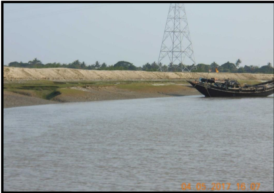
River Bank at chainage 8.8
