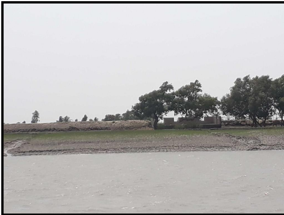
River Bank Protection at Chainage 3.0
