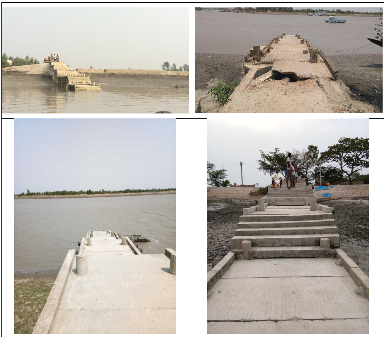
Figure 23: Photographs of Jetties located along Sahibkhali Waterway
