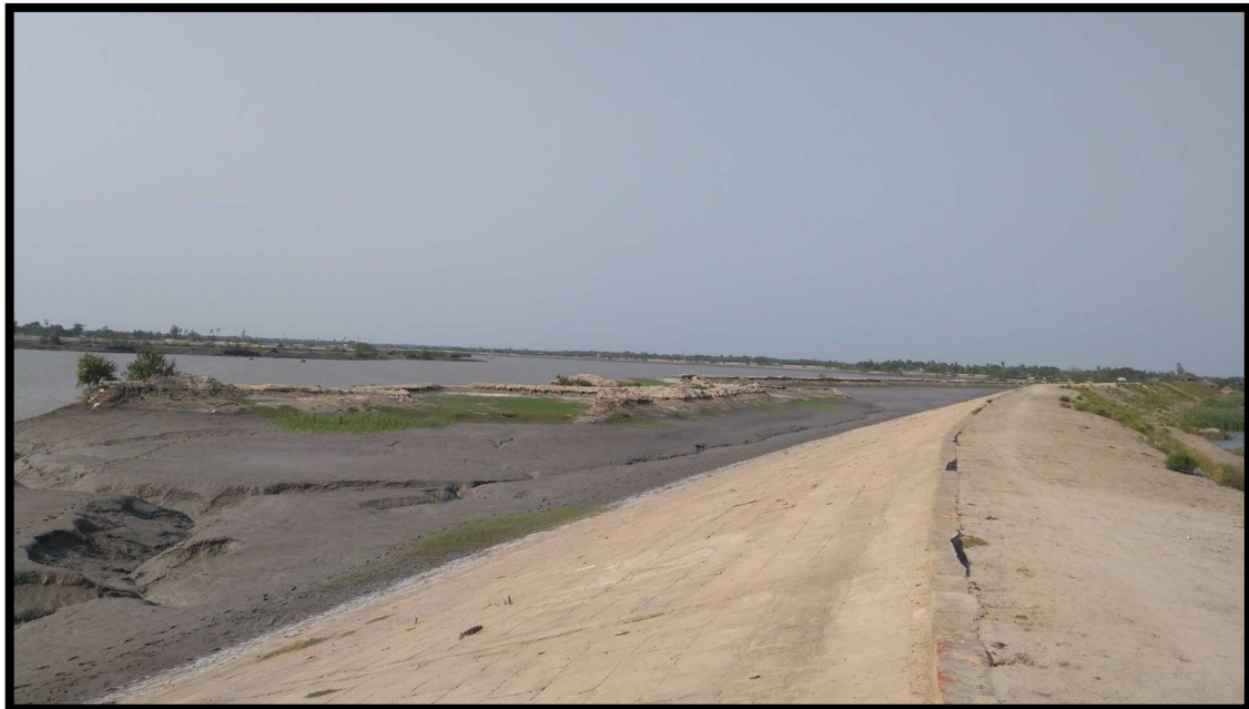
River Bank Protection at Chainage 11.4
