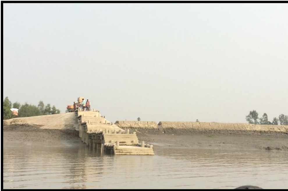
Ramapur Ferry jetty on Right Bank at Chainage 1.9
