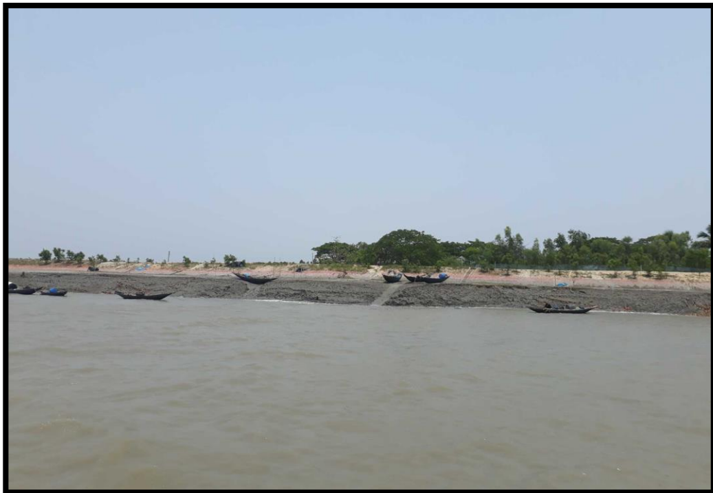
Protected River Bank at chainage 4.9
