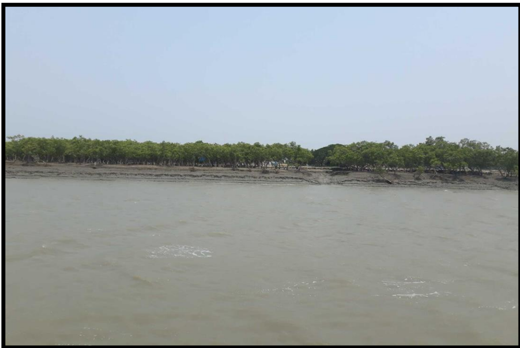
Bank Condition at Chainage 5.4
