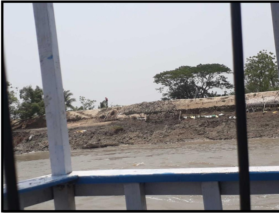
Bank Condition at Chainage 6.6
