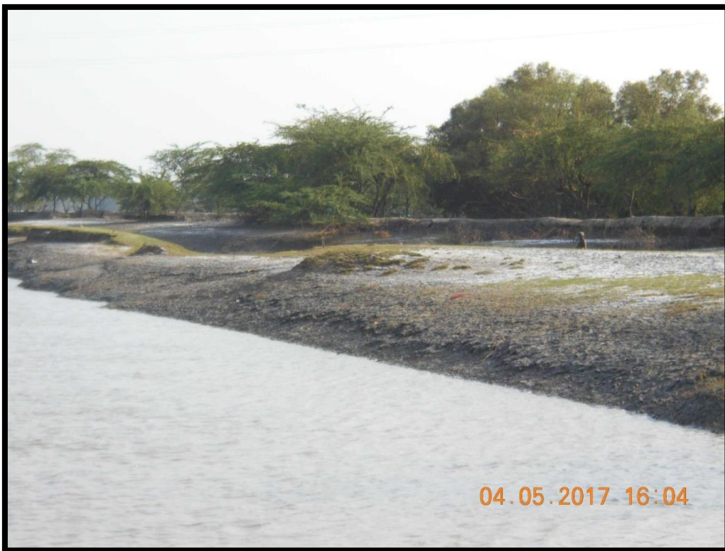
Left River Bank at chainage 9.2
