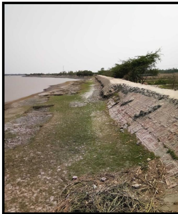
Right Bank Protection at Chainage 7.8
