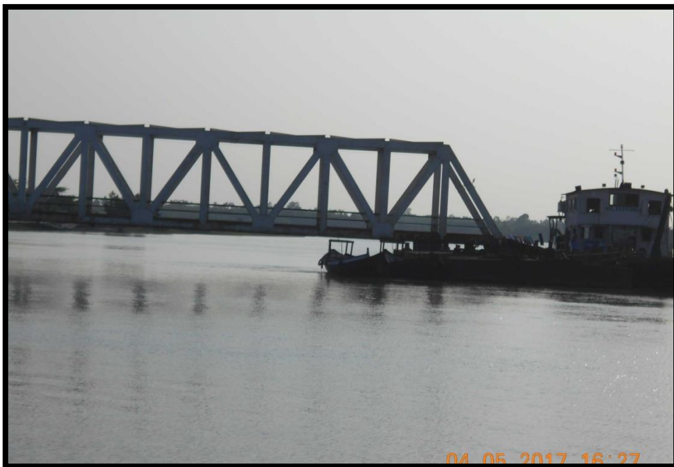
Vessel Jetty Bridge at chainage 8.0
