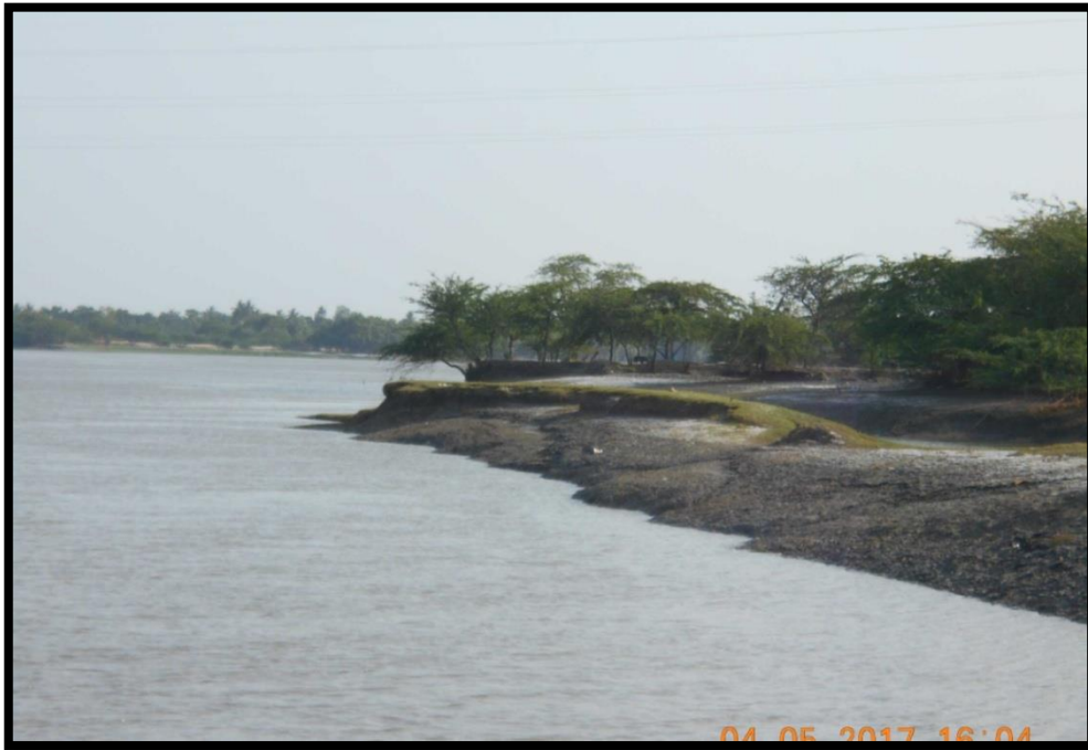
Left River Bank at chainage 9.0
