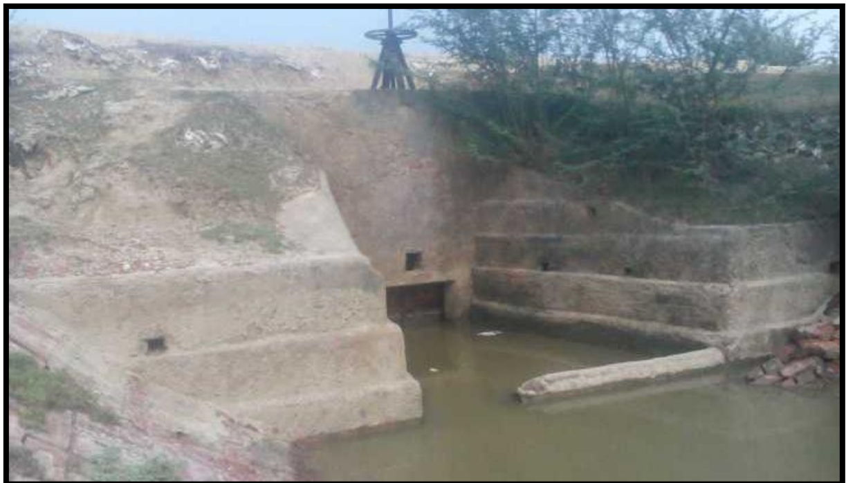
Water Lock on Left Bank at Chainage 5.3
