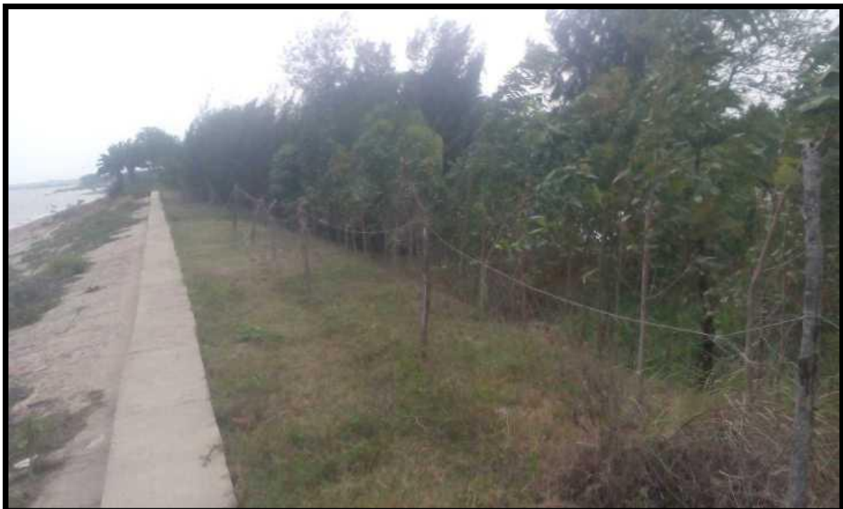
Protected Bank at Chainage 6.0
