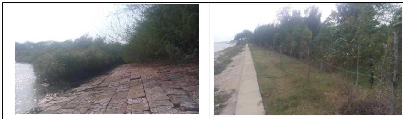
Figure 5: Photographs of Sub-Stretch 1
