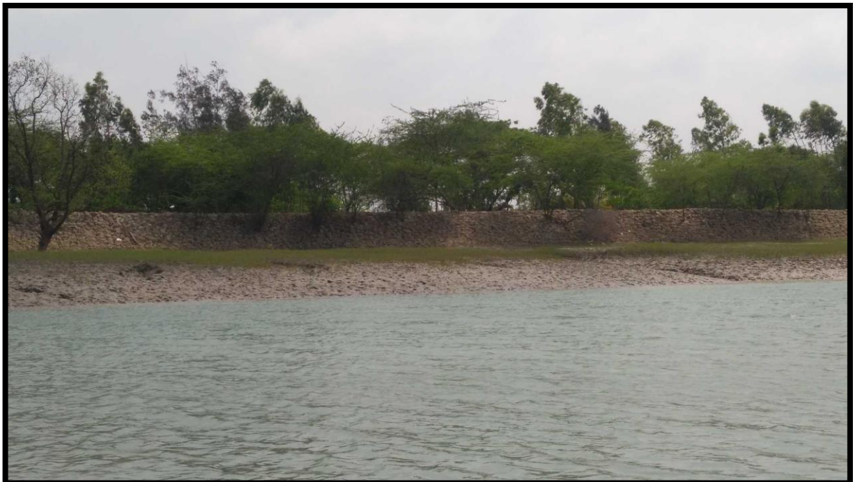
Bank Protection Wall at chainage 37.0
