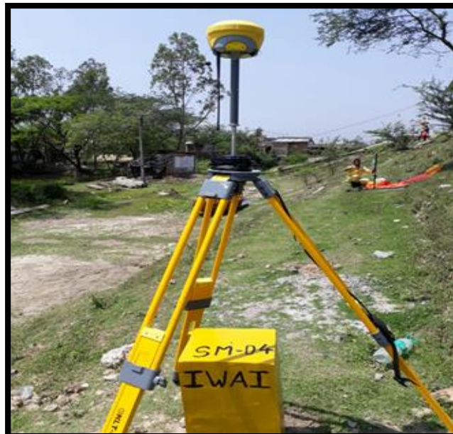
TBM SM-04 at Addhabazar Chainage 35.5
