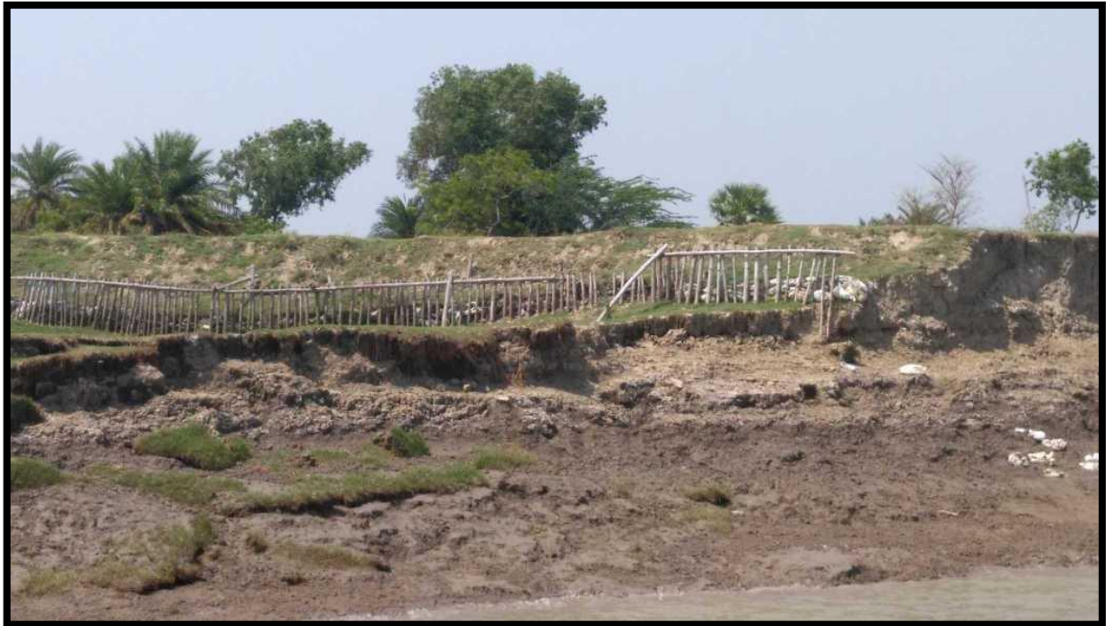
Bank Protection at Chainage 19.7
