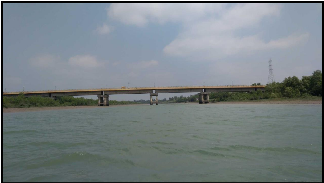
Road Bridge and HT wire tower at Addhabazar Chainage 36.0
