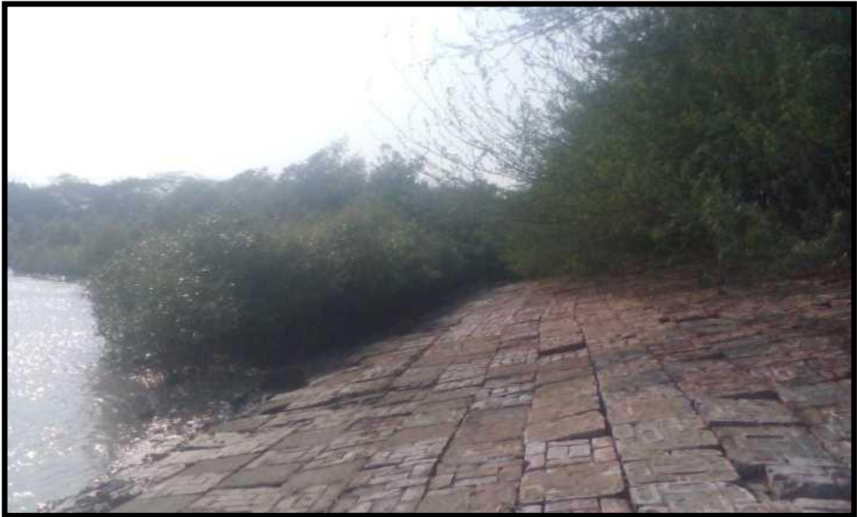
Mangroves at Chainage 5.1
