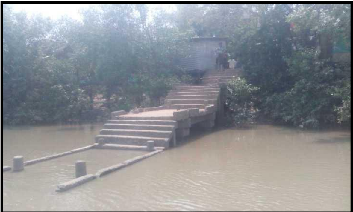
Jetty at Haripur Chainage 8.0
