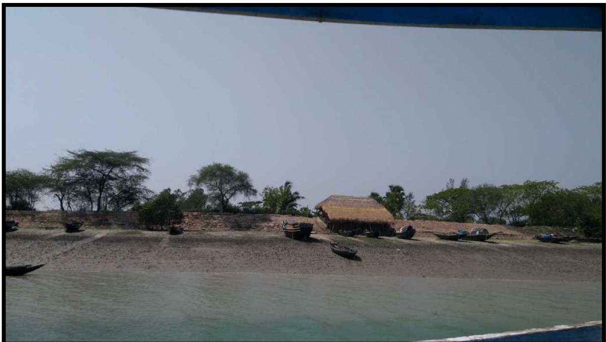
Bank Protection at Chainage 20.5
