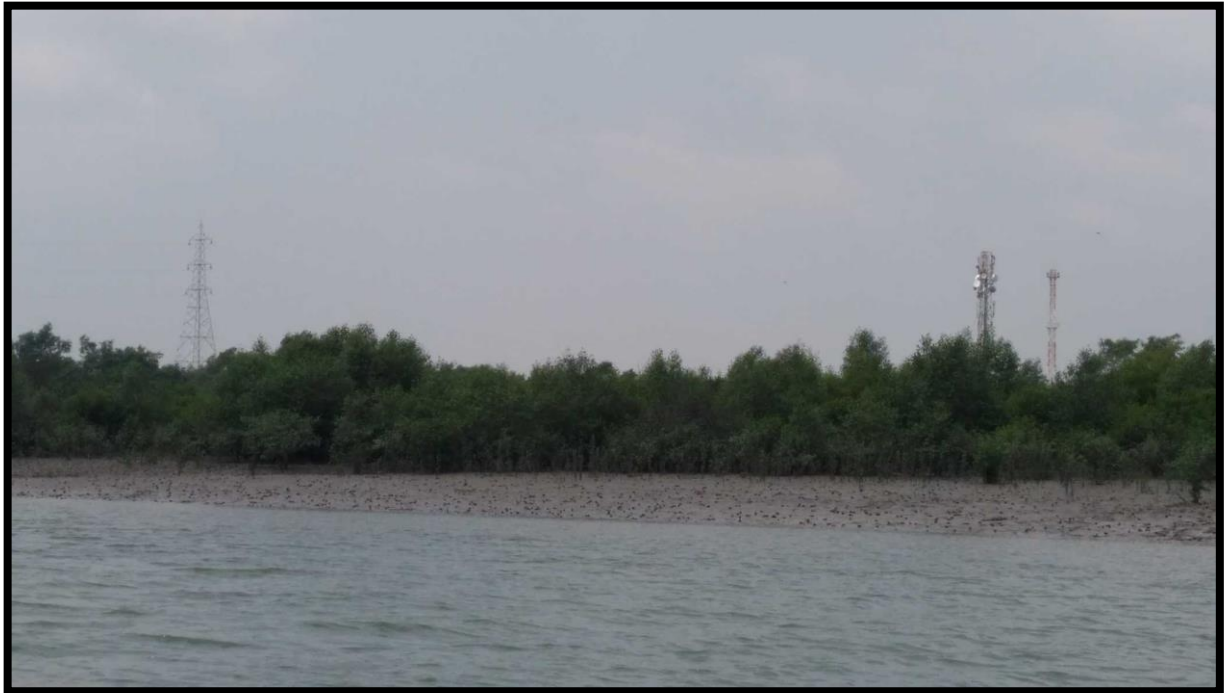
HT wires and mobile communication tower at Addhabazar Chainage 36.0
