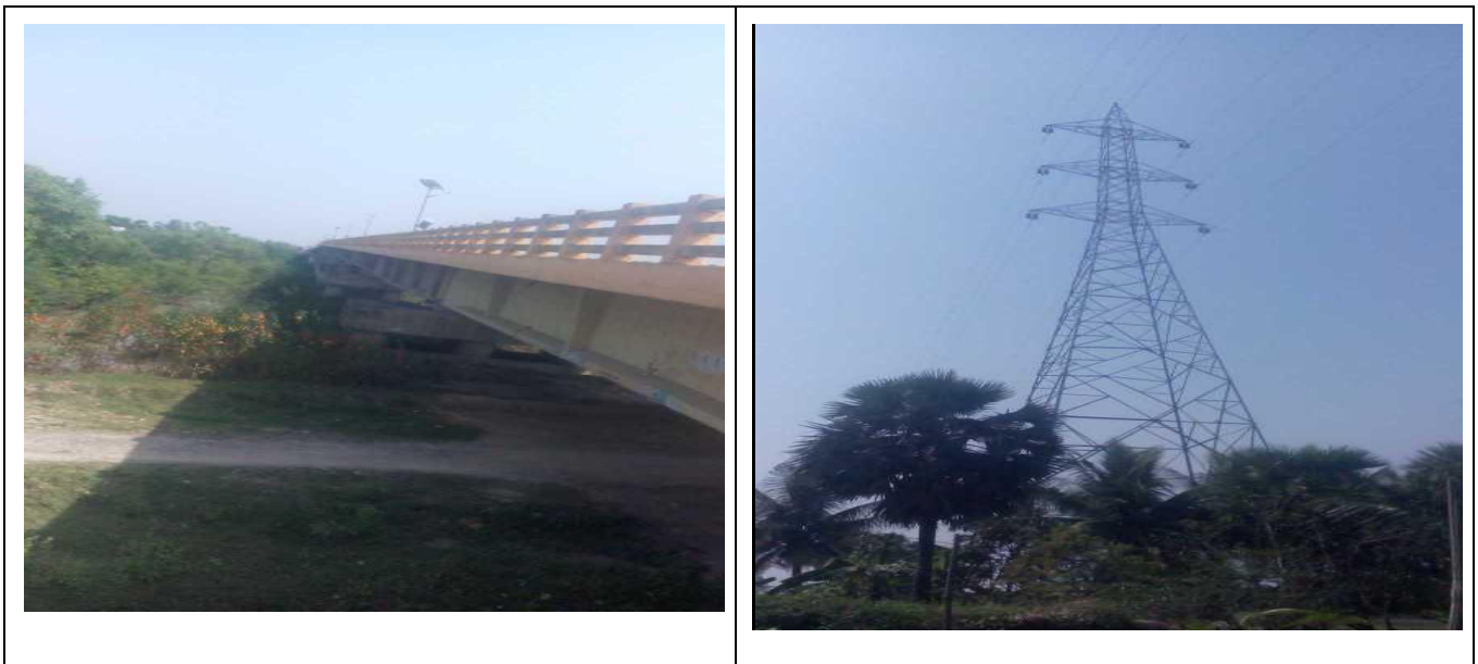
Figure 14: Photograph along Sub-Stretch 4
