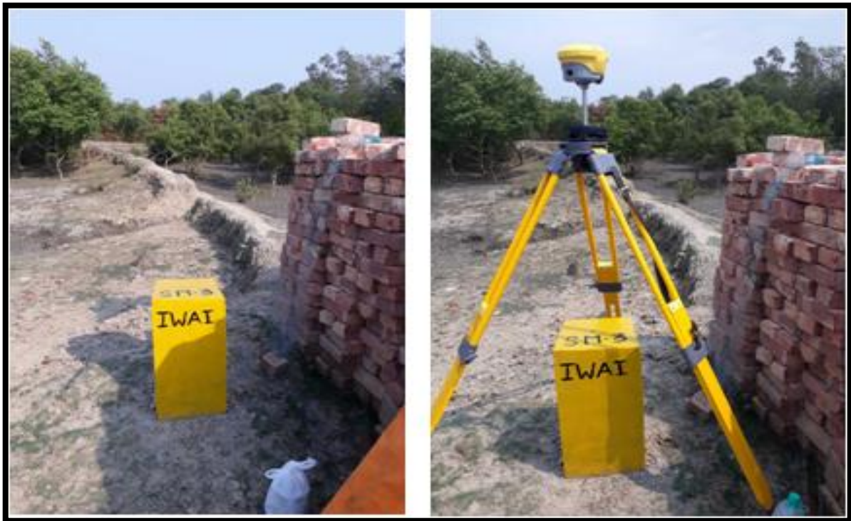
SM-03 at Dwarik Nagar Chainage 18.5
