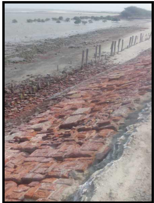
Protected River Bank at Chainage 4.5
