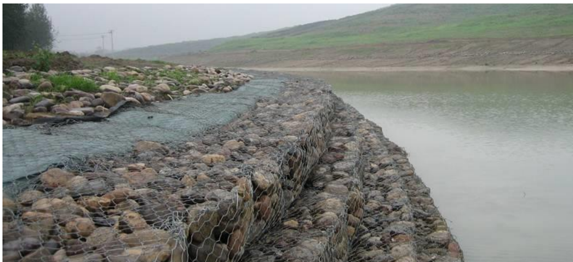
Figure 18: Photograph showing arrangement of Gabion Wall along River Bank
