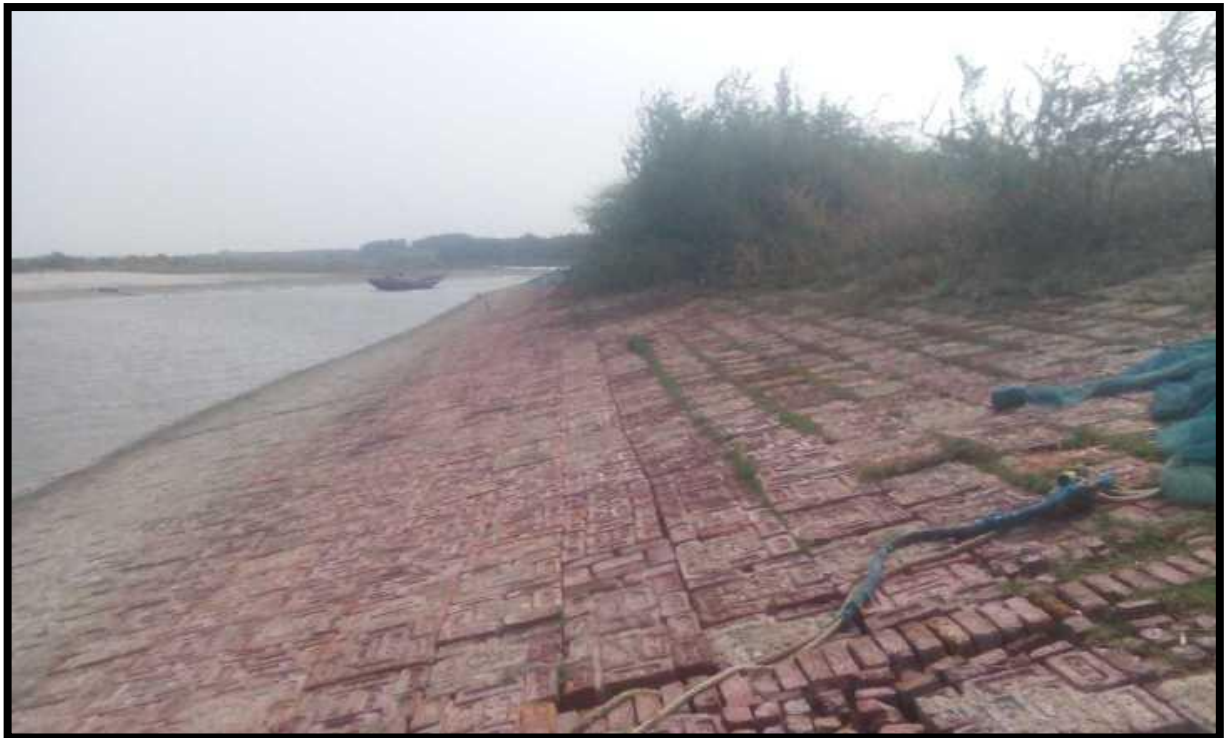
Protected Bank at Chainage 5.0
