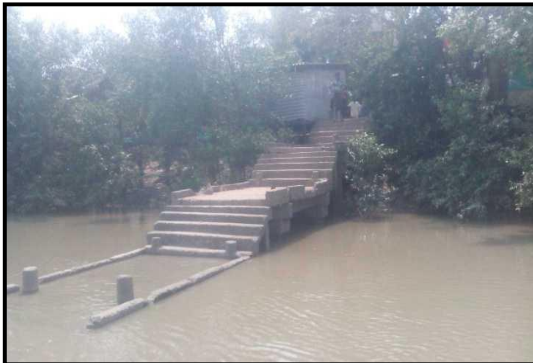
Figure 25: Photograph of Jetty located at Harinagar (Chainage 8.0 Km)
