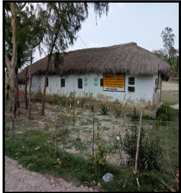
Mukti Head Office at Left Bank Chainage 40.1, Kurbha Shridhapur
