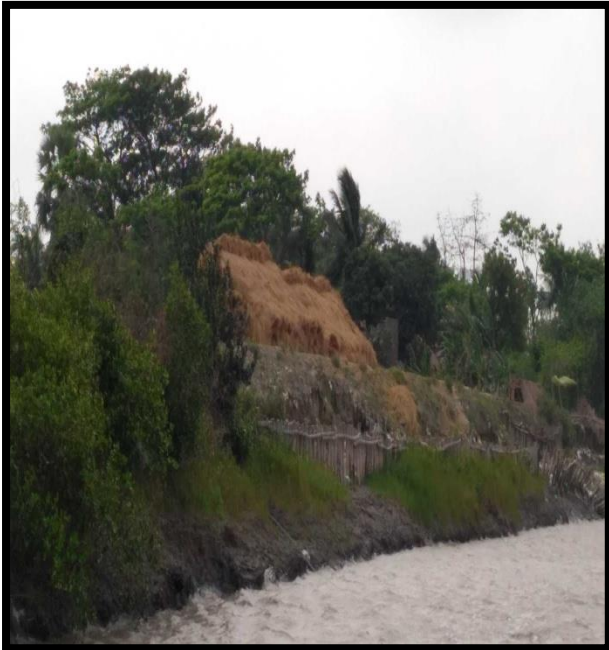
Temporary Right River Bank Protection at Chainage 44
