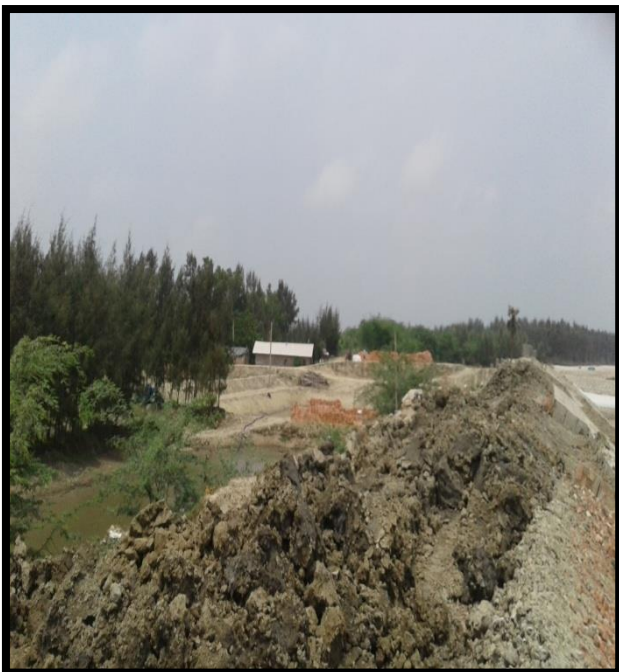
Land at Left Bank Chainage 3.7
