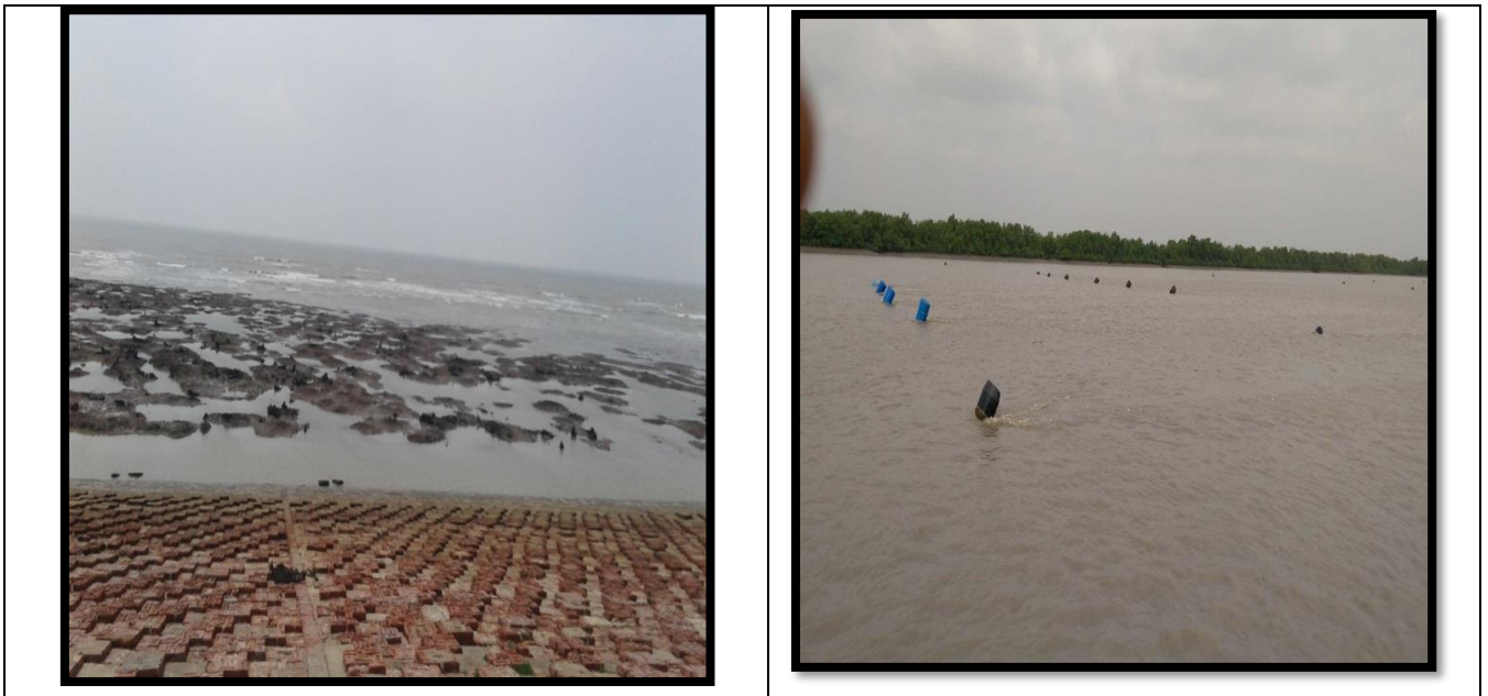
Figure 5: Photographs of Sub-Stretch 1
