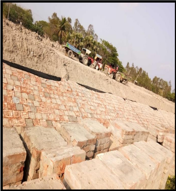
Left River Bank Protection at Chainage 53.5
