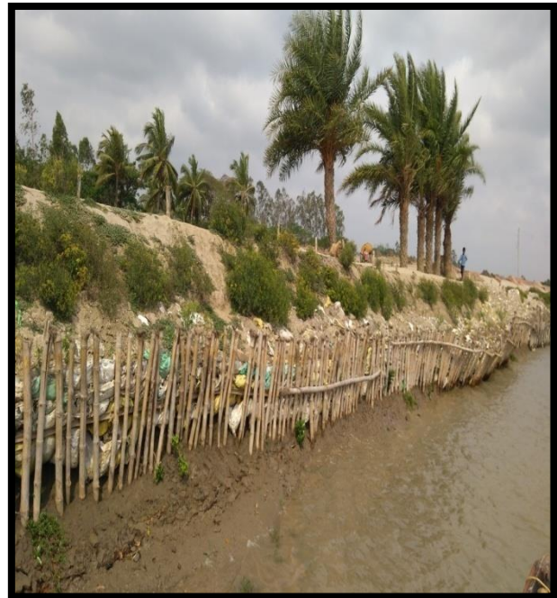
Left River Bank at Chainage 54
