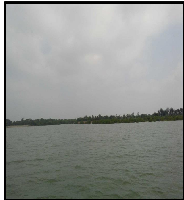
Left River Bank At Chainage 26.5
