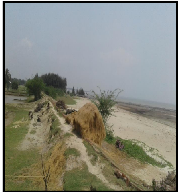
Land at Left Bank Chainage 3
