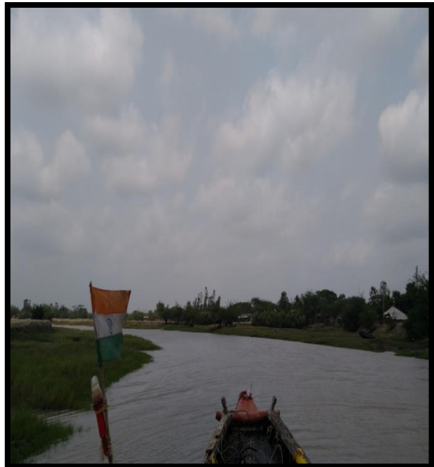
Left River Bank at Chainage 64
