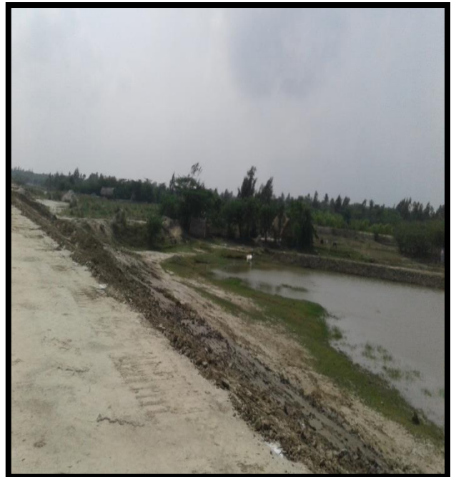
Pond at Left Bank Chainage 5.5
