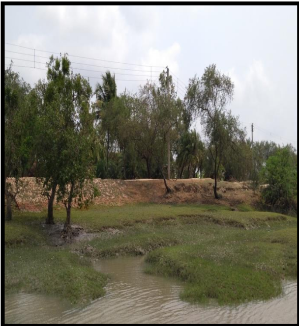
Left River Bank at Chainage 63.5
