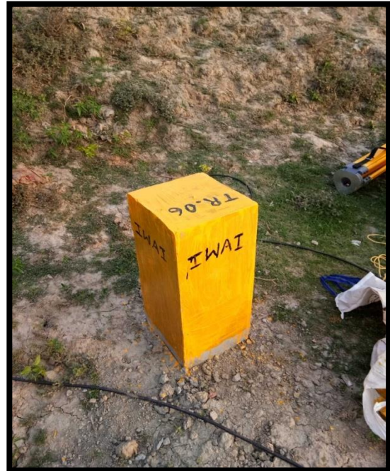
TR-06 At Left Bank Chainage 50.7
