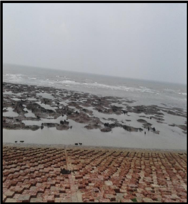
River Bank Protection at Left Chainage 2.8
