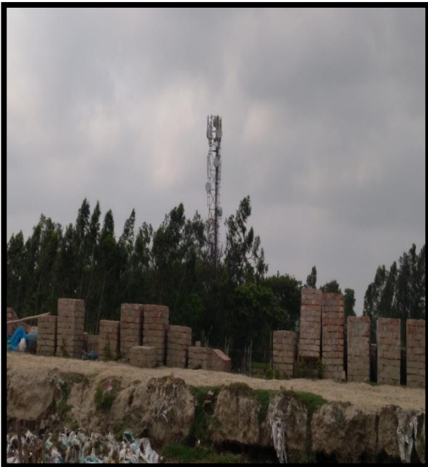
Mobile Tower at Left Bank Chainage 53.9
