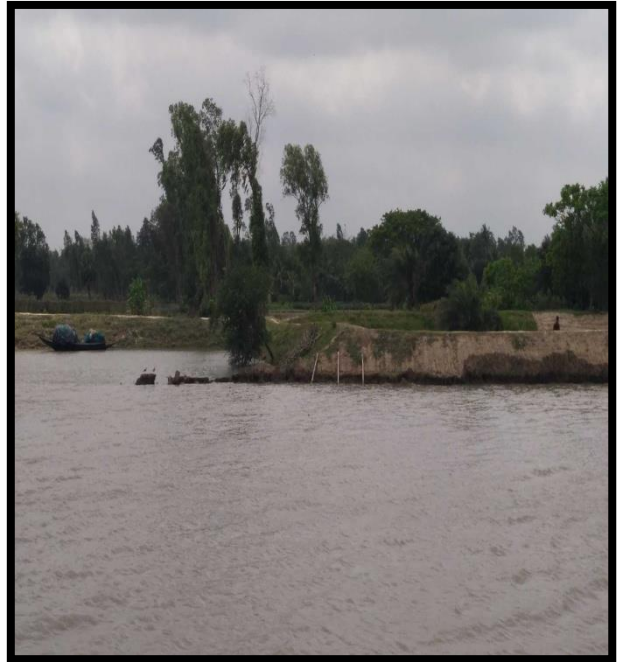
Right River Bank at Chainage 38.5
