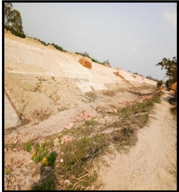
Left River Bank Protection at Chainage 53.6
