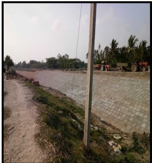
Left River Bank Protection at Chainage 53.8
