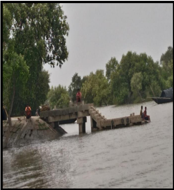
Jetty at Right Bank Chainage 59.4
