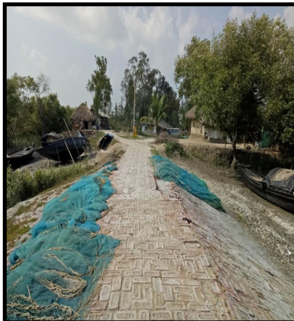
Road at Left Bank Chainage 40, Kurbha Shridhapur
