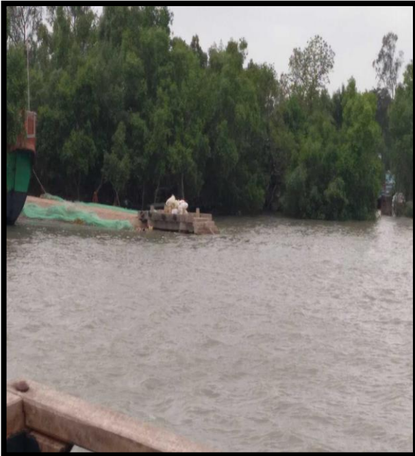
Jetty at Right Bank Chainage 38
