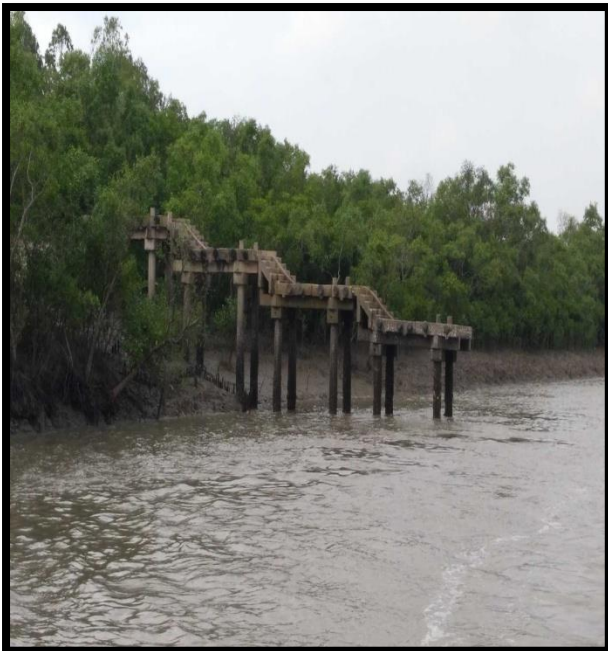
Right River Bank Bhunesvar Jetty at Chainage 41.4
