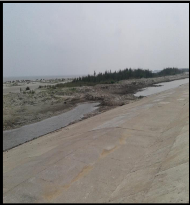
River Bank Protection at Left Chainage 5
