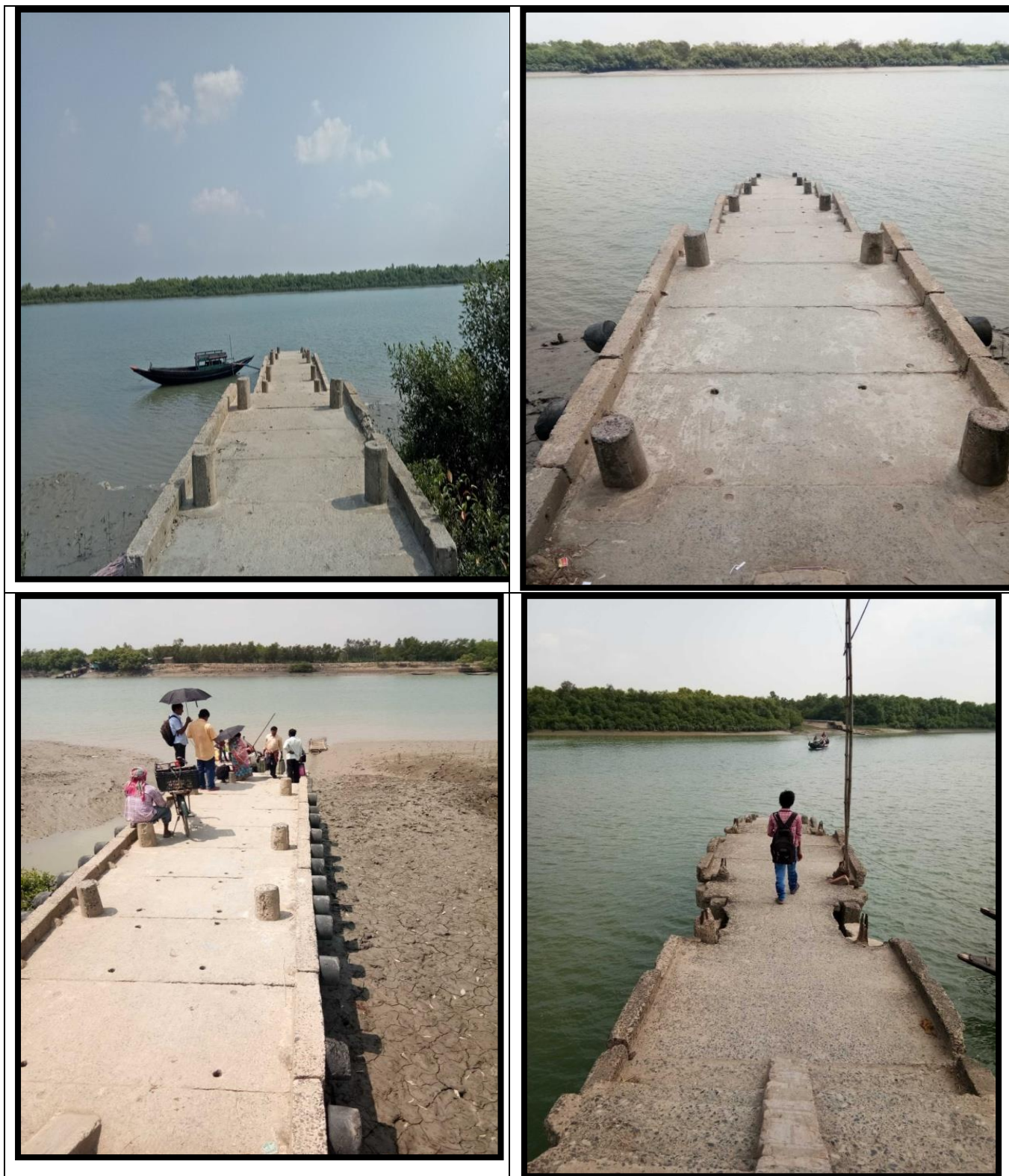
Figure 32: Photographs of Jetties located along Thakurran River Waterway
