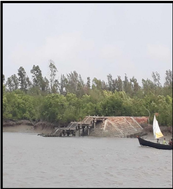
Jetty at Right Bank Chainage 39.2
