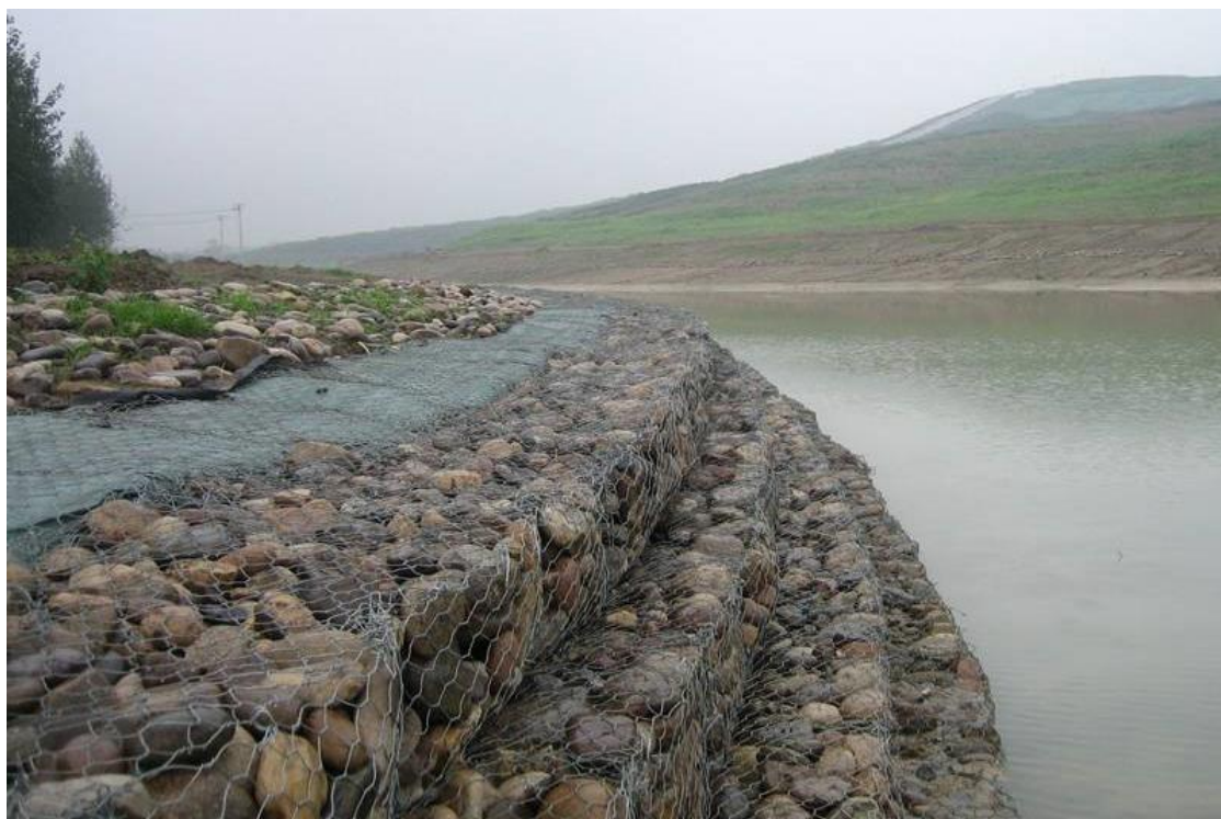
Figure 24: Photograph showing arrangement of Gabion Wall along River Bank
