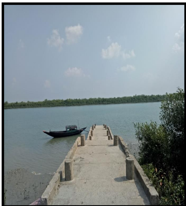
Jetty Ghat at Left Bank Chainage 40, Kurbha Shridhapur
