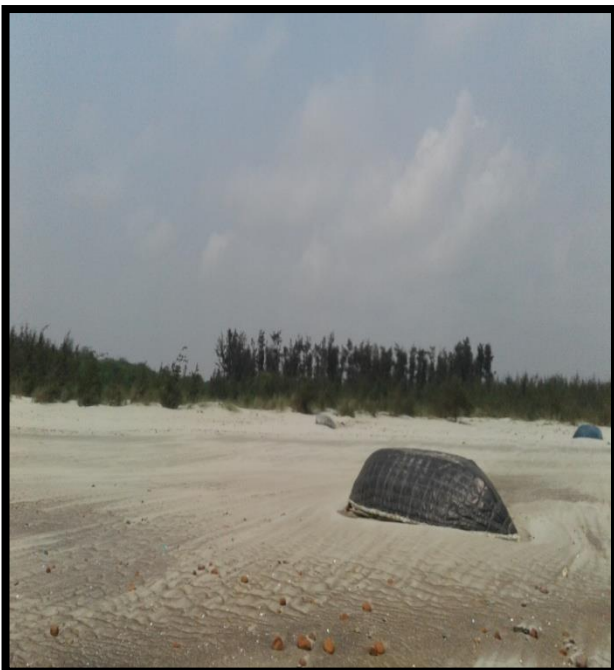
River Shore at Left Chainage 6.2
