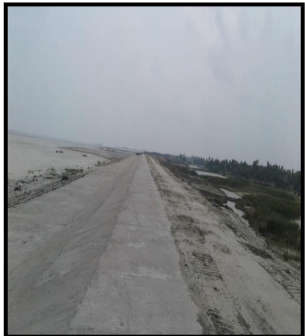
River Bank Protection at Left Chainage 4.1
