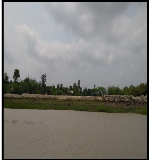
Left River Bank Protection at Chainage 63.2
