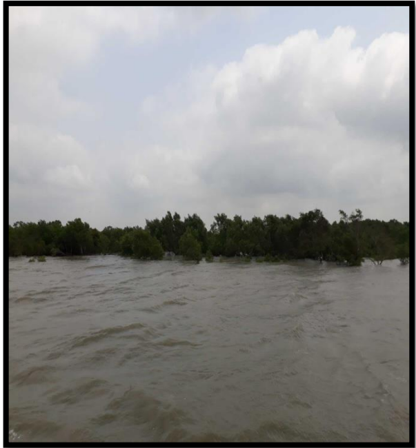
Right River Bank at Chainage 22.1
