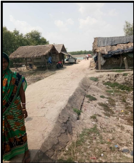
Debhipur Jetty Ghat at Right Bank Chainage 53.4
