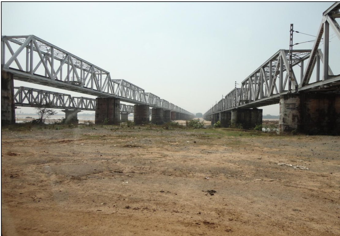
Photo 4 : Railway Bridge on River Brahmani near Jenapur /Pankpal
