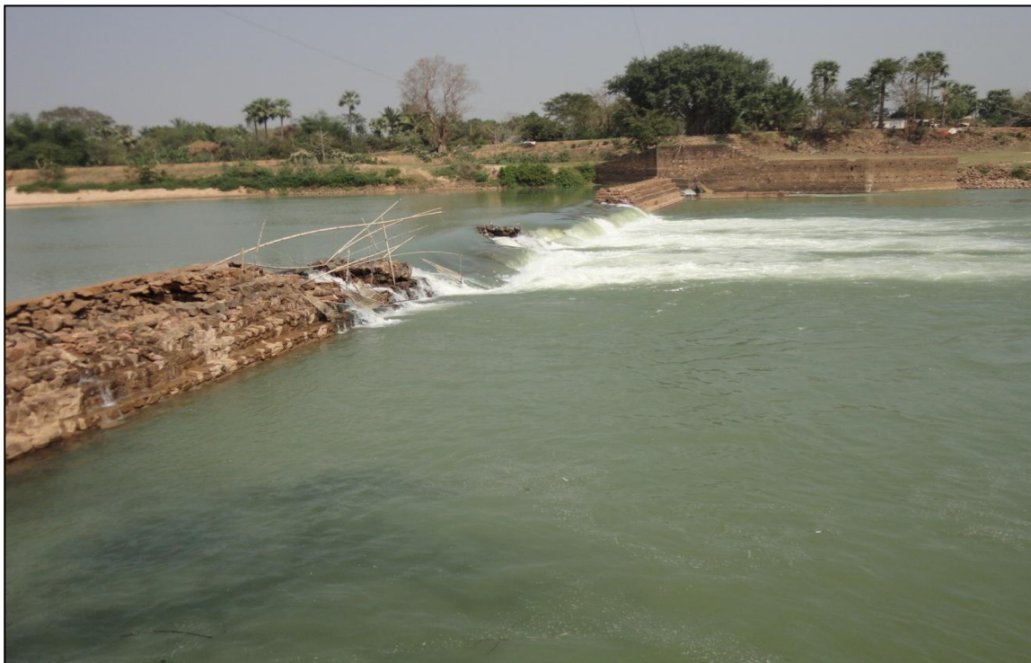
Photo 16 : Another View of Sujanpur Weir
