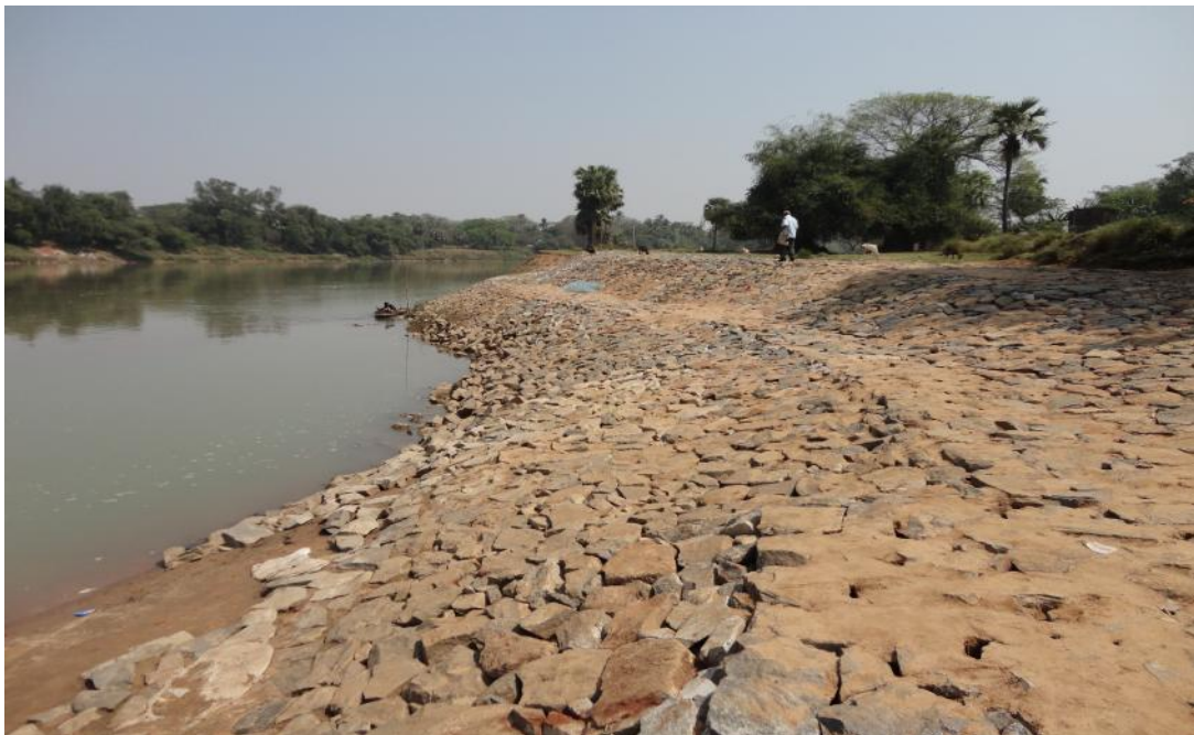
Photograph No. 13-3 Bank Protection along the river
