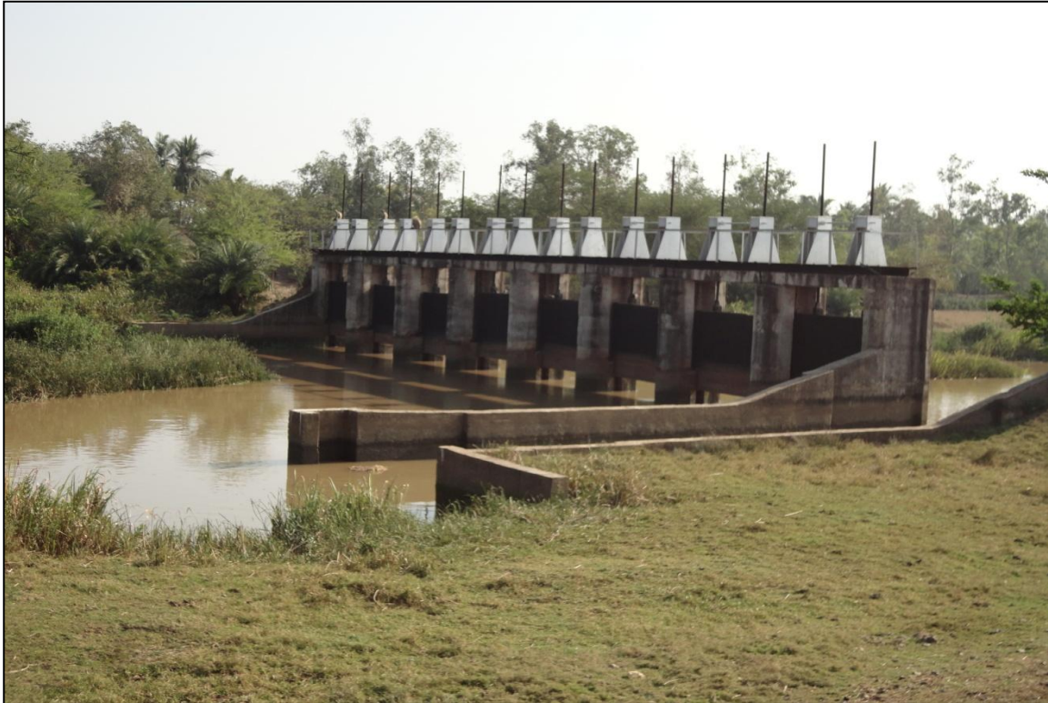
Photo 31 : Gated Weir with Navigational Lock at Tantipal
