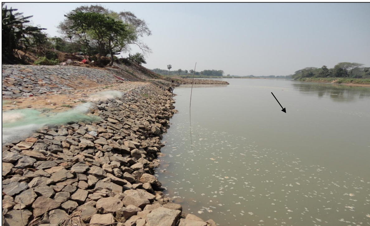
Photo 26 : Bank Protection Works along Right Bank of Kani River
