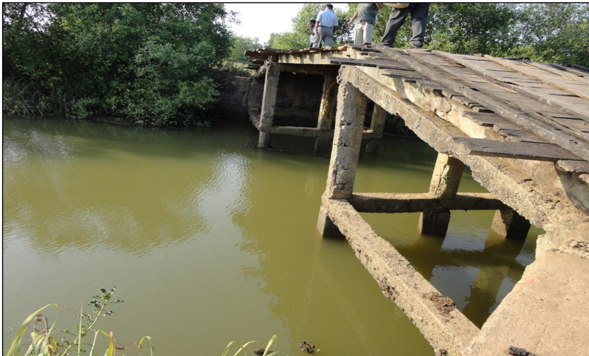
Photo 34 : Wooden Bridge with Concrete Pillars
