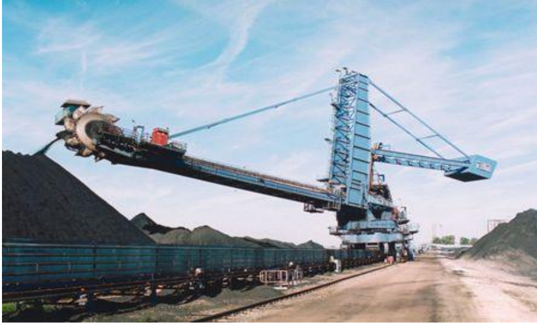
Figure No. 11- 13 Gantry Stacker and Reclaimer
