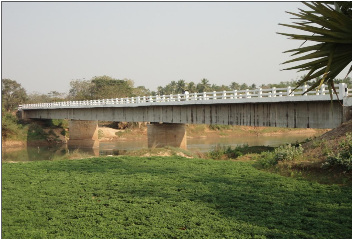
Photo 20- Bridge on Dudhia river near Rajapur
