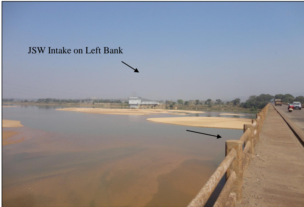
Photo 1 : SH 200 Bridge on River Brahmani near Pankpal
