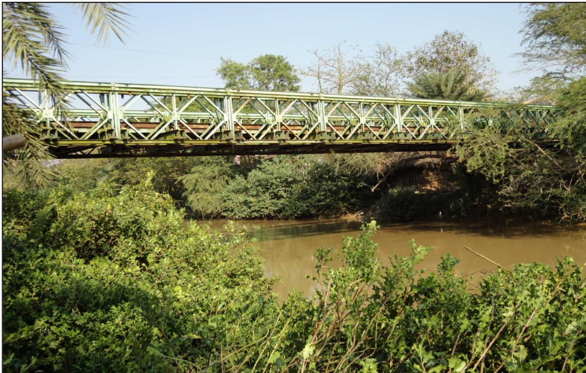
Photo 30 : Steel Bridge at Tantipal
