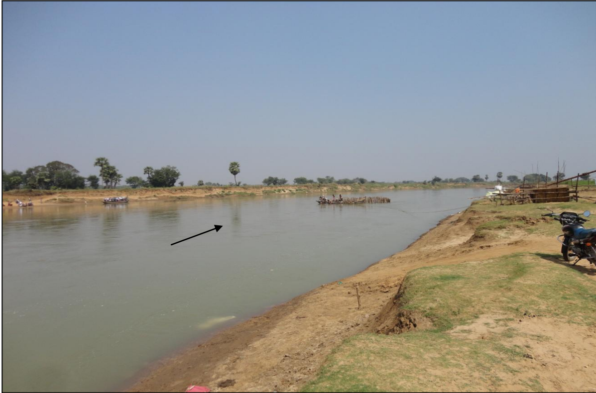
Photo 27 : Under Construction Bridge at Dandisia Village
