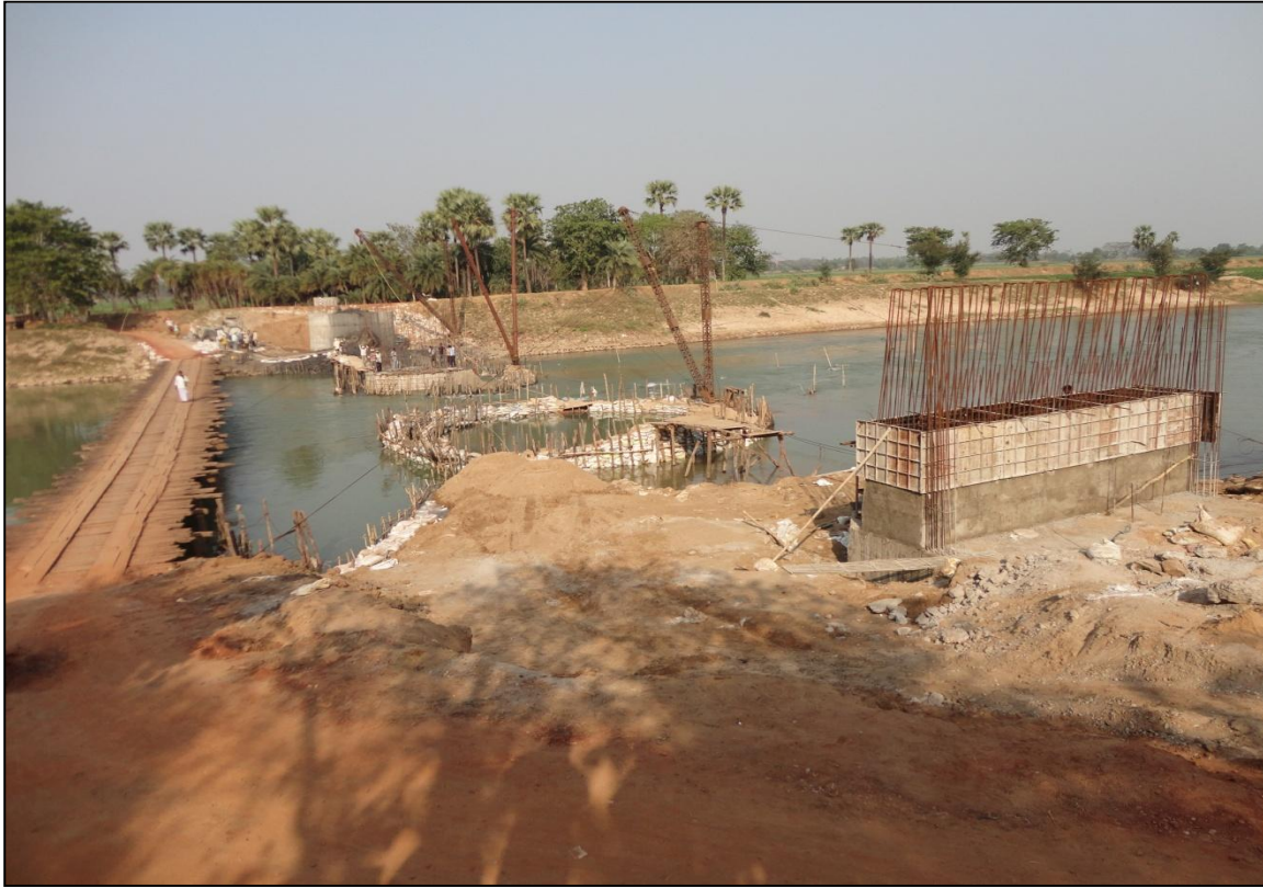
Photo 17 : Under Construction Road Bridge on Dudhia River at Aurangabad (Bari)
