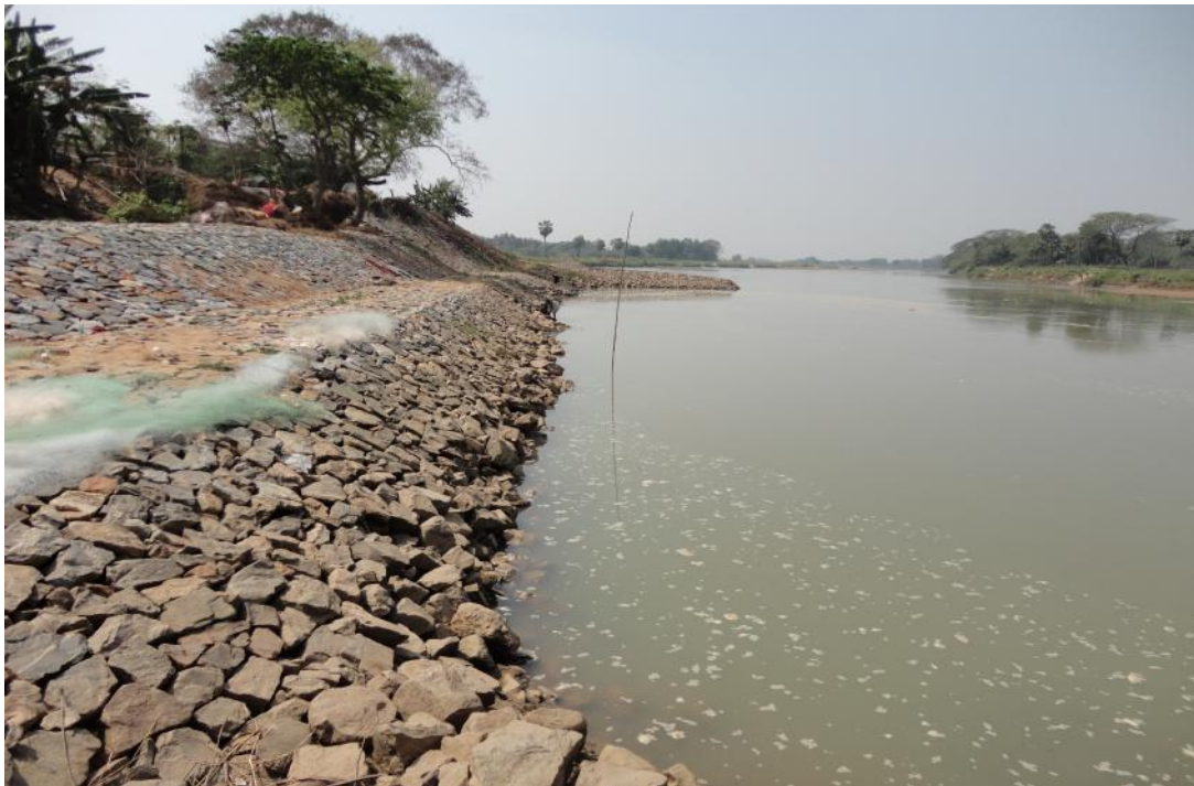
Photograph No. 13-5 Bank Protection along the river
