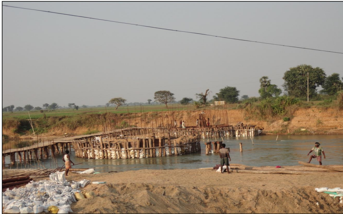
Photo 18 : Under Construction Road Bridge on Dudhia River near Bari
