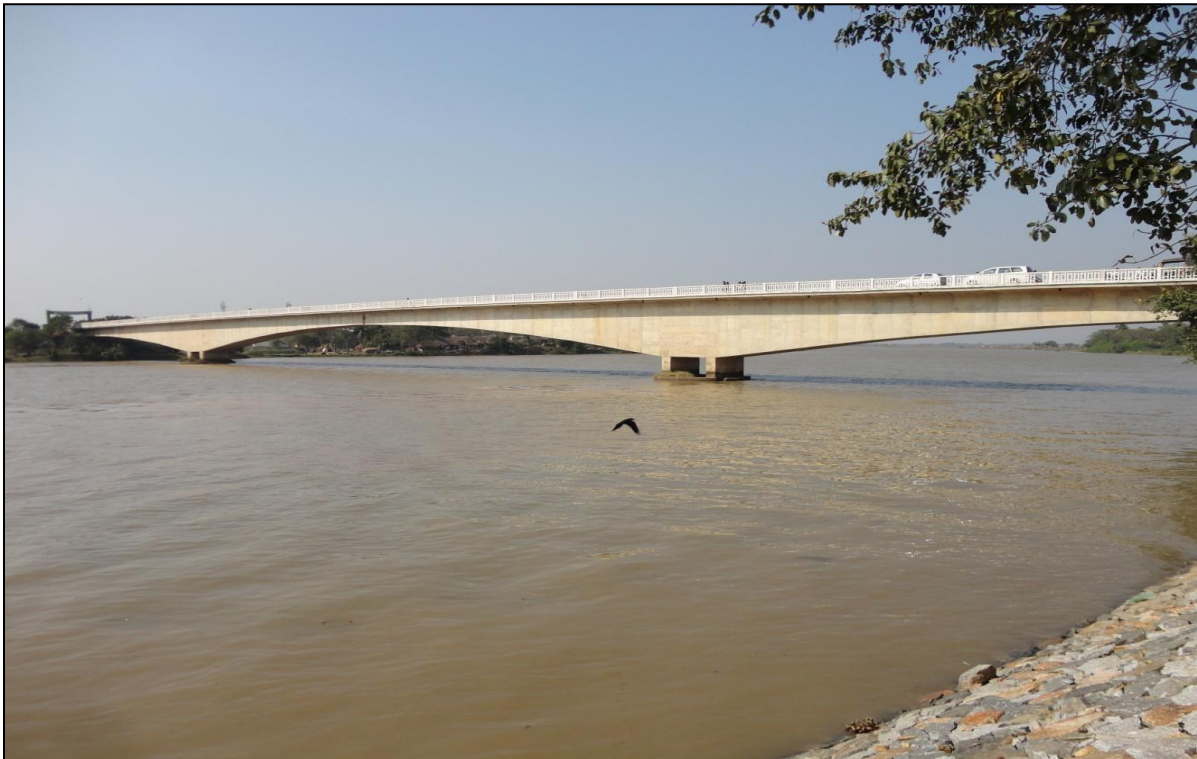
Photo 28 : Bridge on River Hansua at Rajnagar
