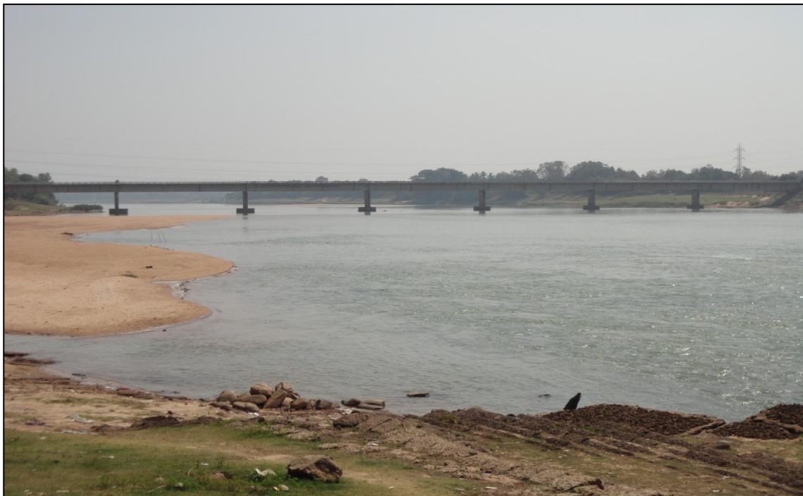
Photo 10 : Road Bridge on Downstream of Jokadia Barrage
