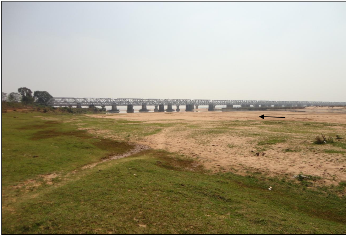
Photo 3 : Railway Bridge on River Brahmani near Jenapur/Pankpal
