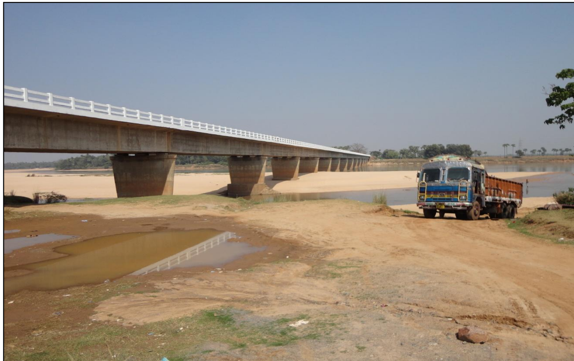
Photo 12 : Bridge on River Brahmani about 3 km Upstream of Sujanpur
