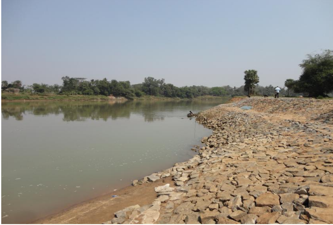
Photograph No. 13-5 Bank Protection along the river
