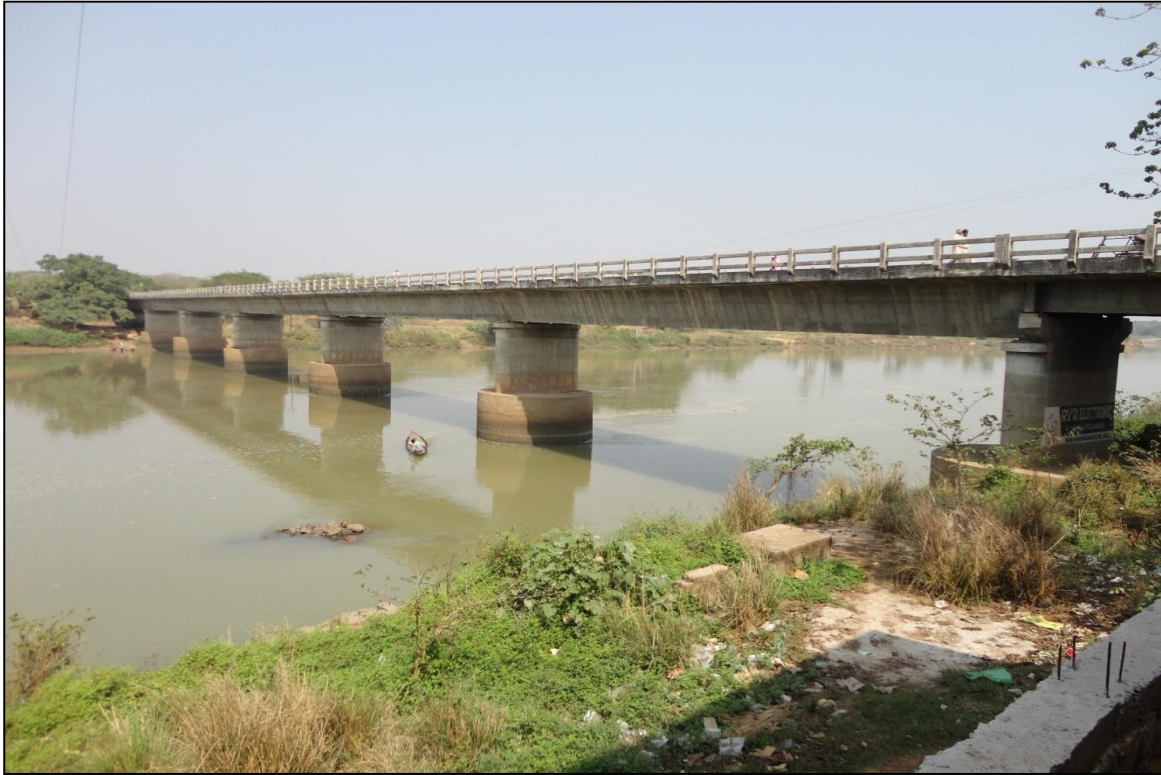
Photo 23 : Road Bridge on Kani River at Mangalpur
