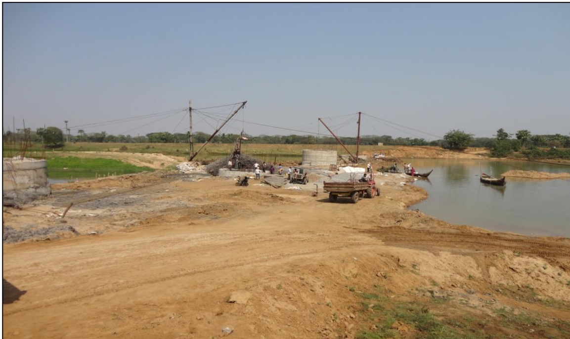
Photo 22 : Under Construction Bridge on Tantighai / Bhongra River at Raula/Aurangabad
