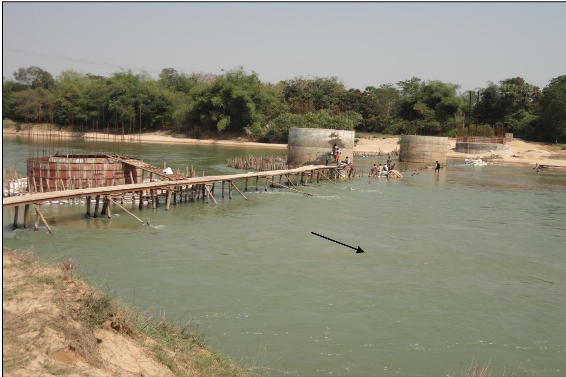
Photo 21 : Under Construction Bridge on Tantighai / Bhongra River near Erada
