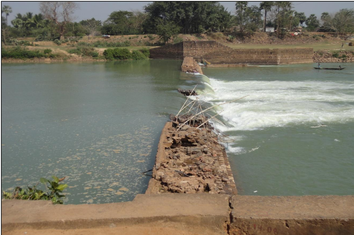
Photo 14 : Sujanpur Weir on Tantighai River
