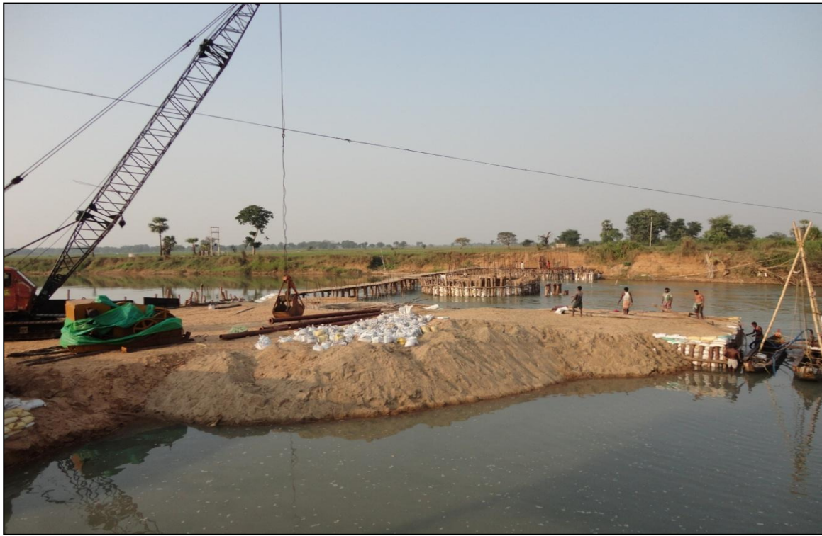
Photo 19- Bridge under construction on Dudhia river near Bari
