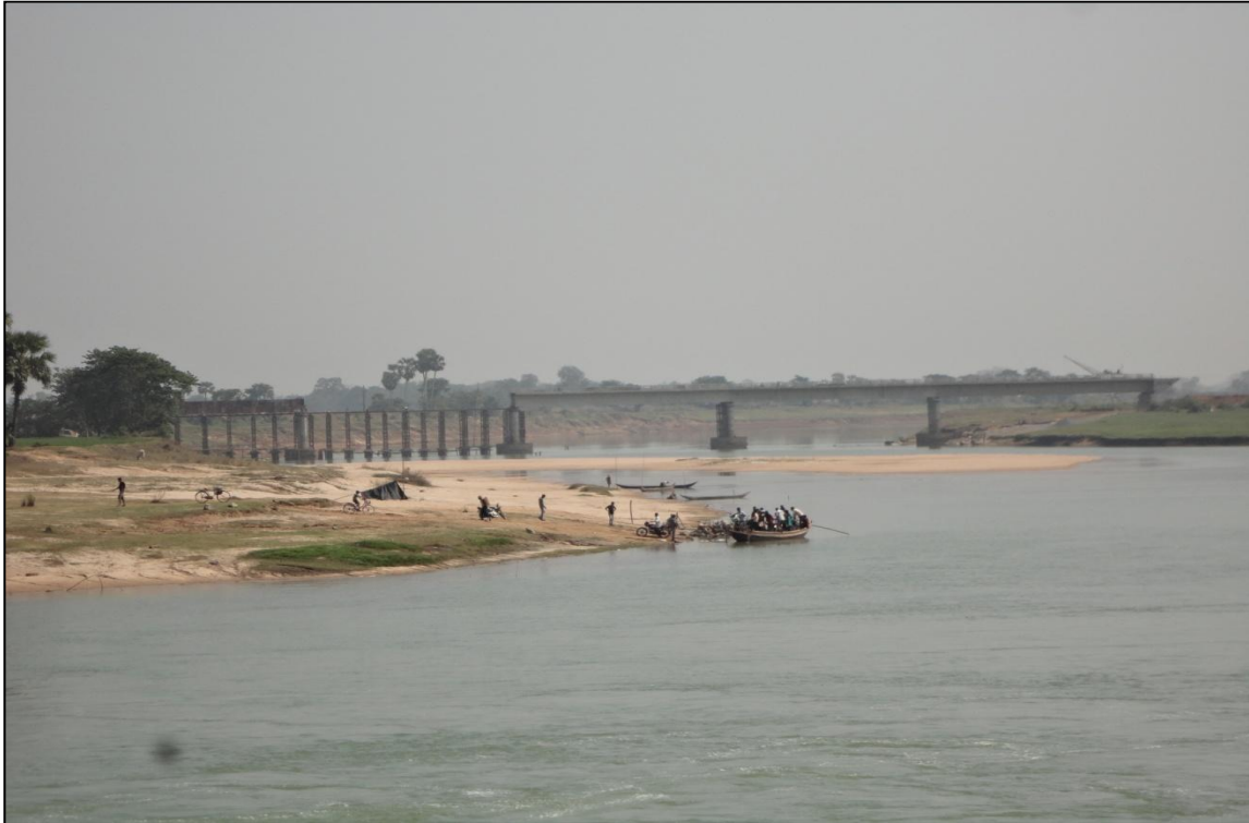
Photo 15 : Under Construction Road Bridge Downstream of Sujanpur Weir
