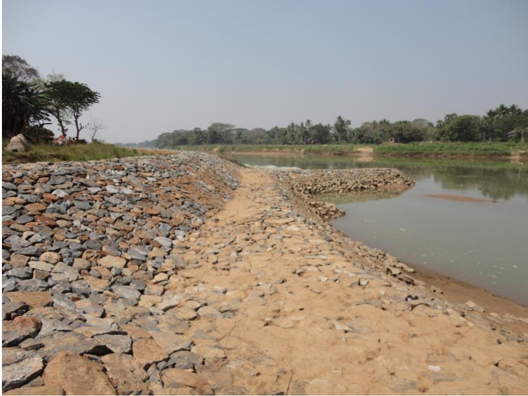
Photograph No. 13-3 Bank Protection along the river
