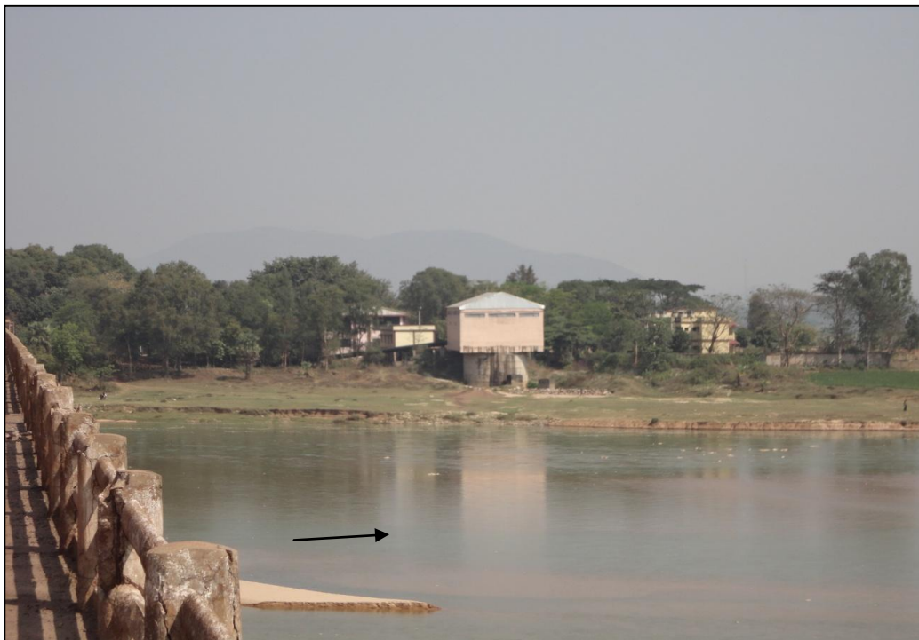
Photo 2 : Intake on Downstream of SH 200 Bridge on River Brahmani near Pankpal
