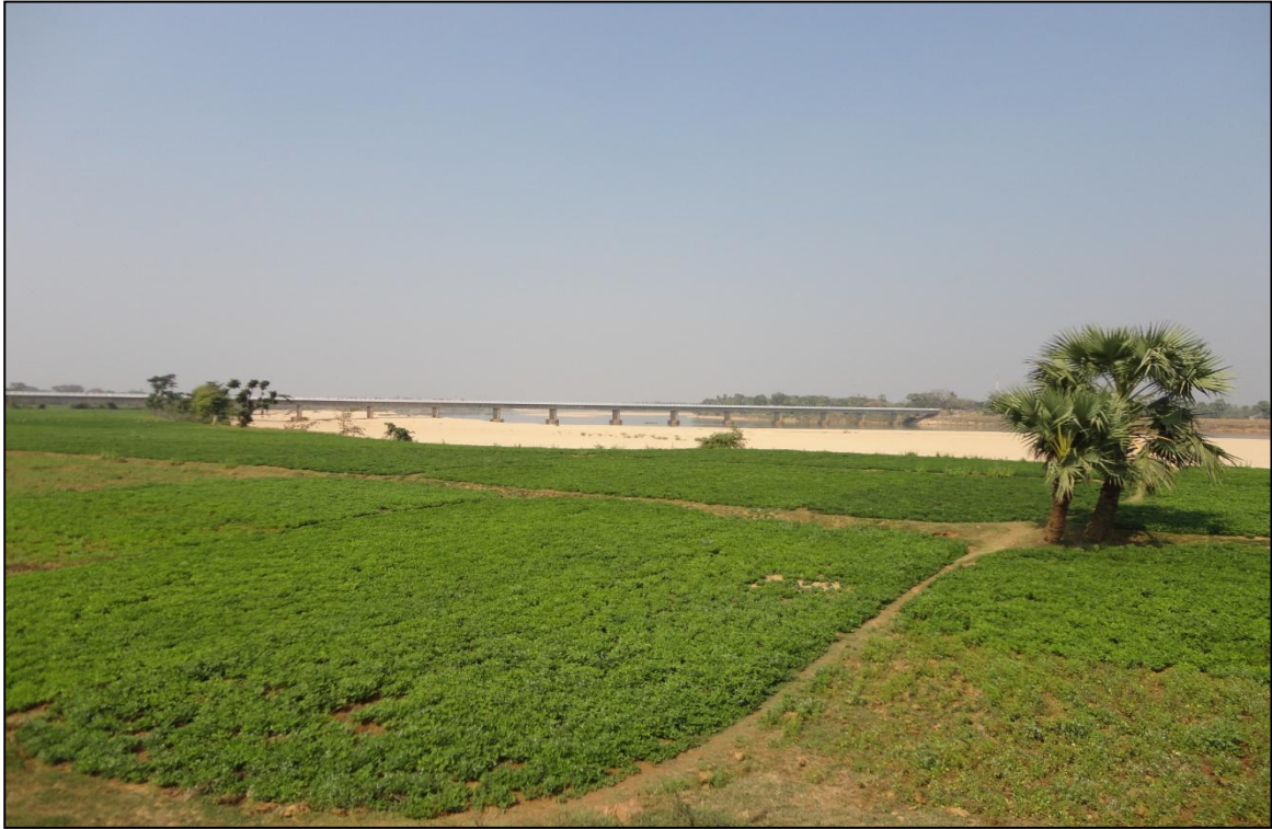
Photo 13 : Bridge on River Brahmani near Jalpur about 3 km Upstream of Sujanpur
