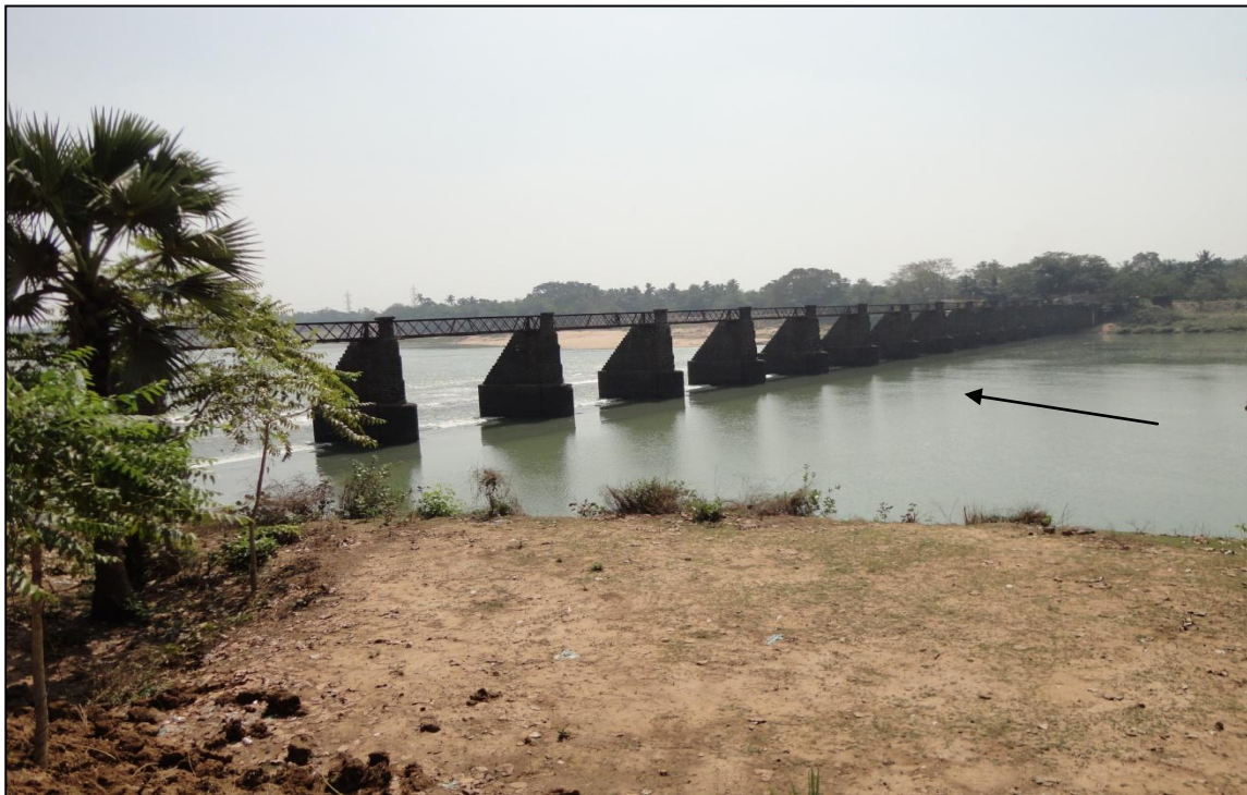
Photo 8 : View of Jokadia Barrage from Upstream
