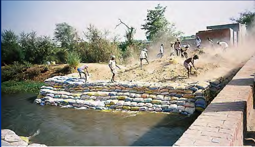
Bypass for a weak bridge is under construction
