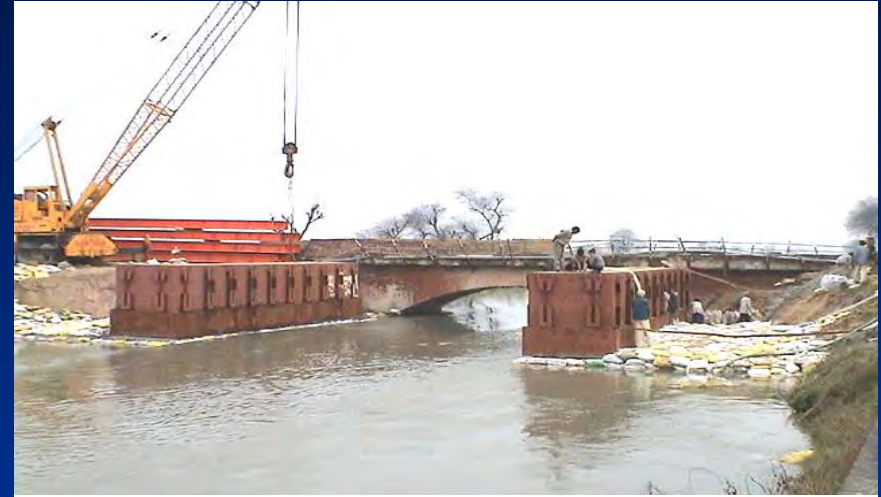
Pontoon bridge across Canal under construction
