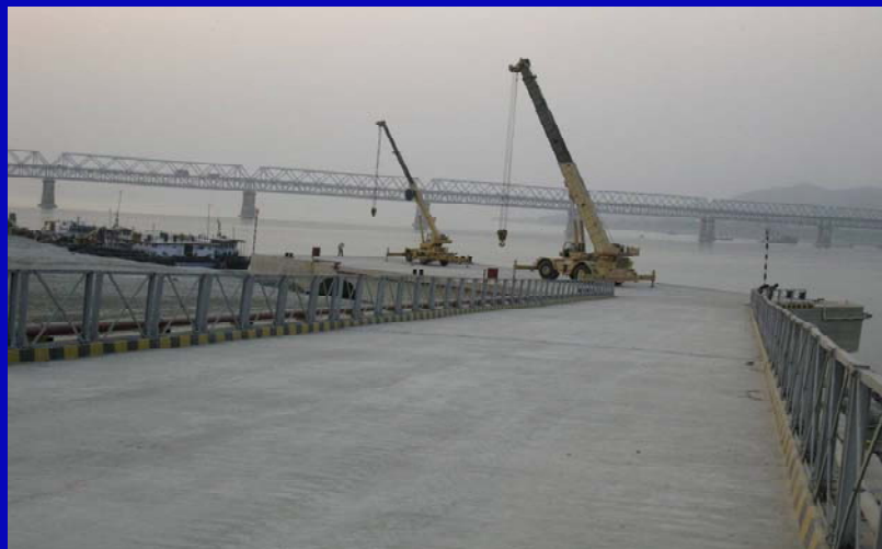
Low level jetty at Pandu
