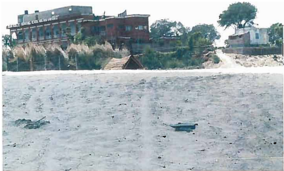
Plate 4.1 (a) Public Boarding School at New Ram Nagar By pass bridge ( Right bank)
