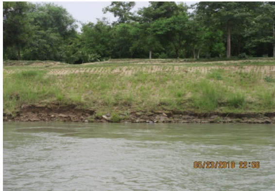
Grass Pitching Bank Protection at Udaychandpur
