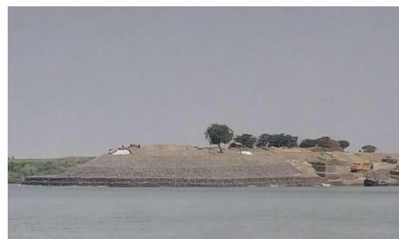
Spur Construction after Ismailpur Area
