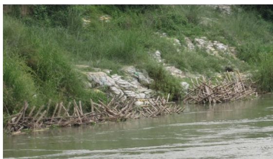
Bank Protection with Bamboo
