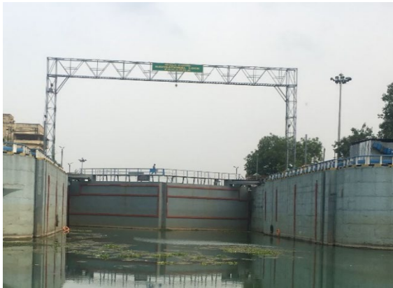
Farakka Barrage Lock gate Upstream Side
