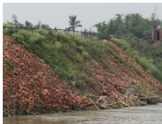
Bank Protection with Broken Bricks Near Kalna
