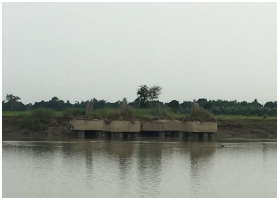
Foundations of collapsed tower line at Rukespur
