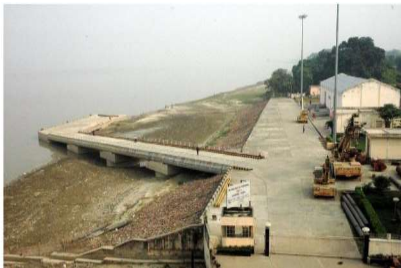
Figure 18: Existing Patna terminal
