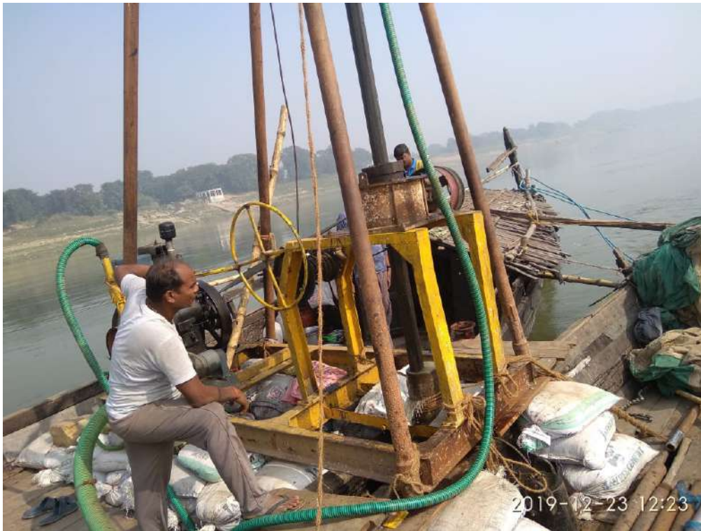
Figure 1: Drilling machine mounted on two boats
