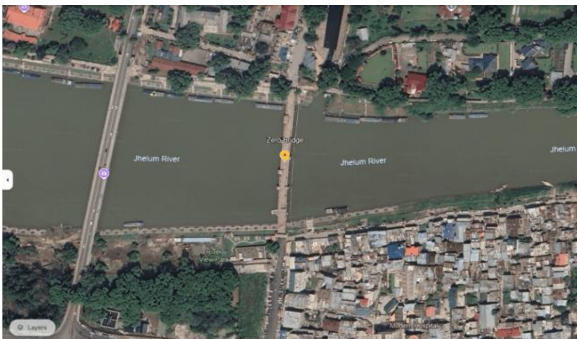
Fig 4. floating concrete jetty at Zero Bridge
