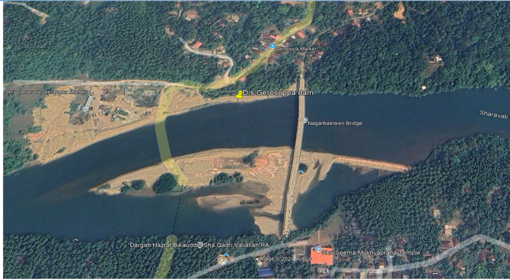
Fig 2. D/s Gerosappa Dam - floating jetty site
