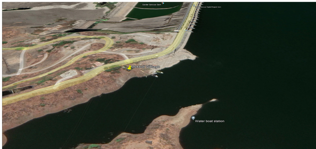
Fig 1. Mokhdi River Bank - floating jetty site
