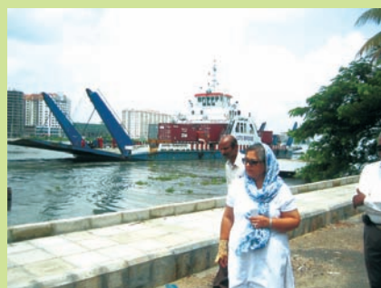
Inspection of Bolgatty Terminal by Chairperson, IWAI
