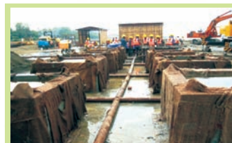
Pre casting of structural members for Port & IWT Jetty at Sittwe
