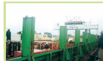
Unloading of cranes at Sittwe for construction work
