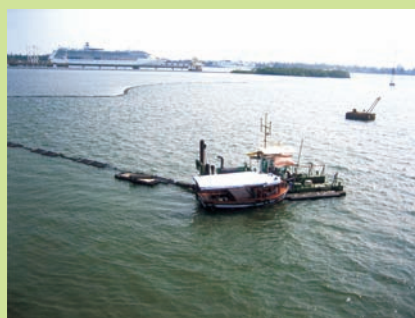
A view of IWAI's Cutter Suction Dredger at work in Bolghatty shoal on NW.3
