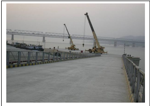
Fig-4, IWT terminal at Pandu, NW-2
