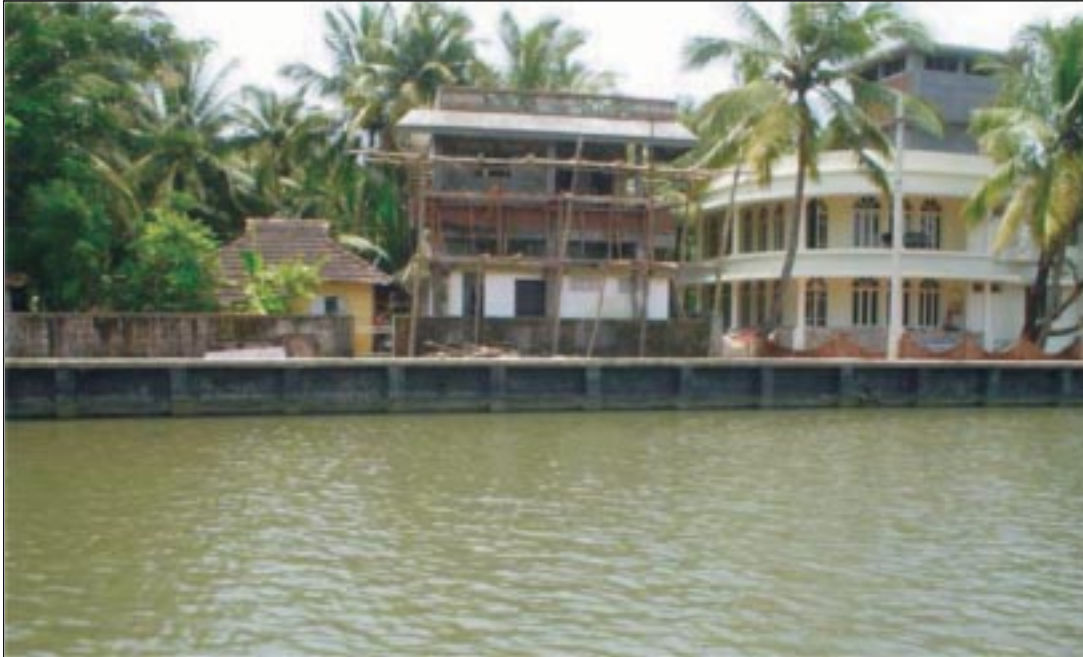
BANK PROTECTION WORK IN CHAMPAKKRA CANAL
