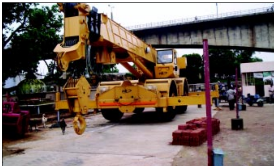
CONTAINER CRANE - PATNA
